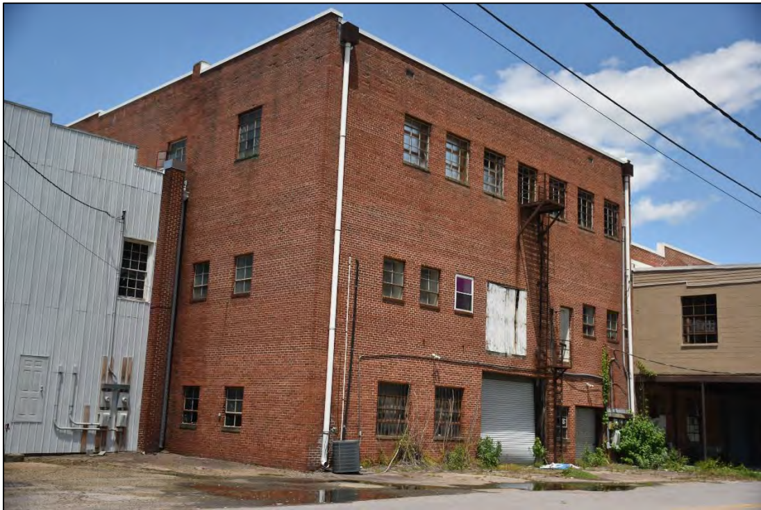
Figure 2.3.9. WK0452, 327 East Main Street, facing northeast.
