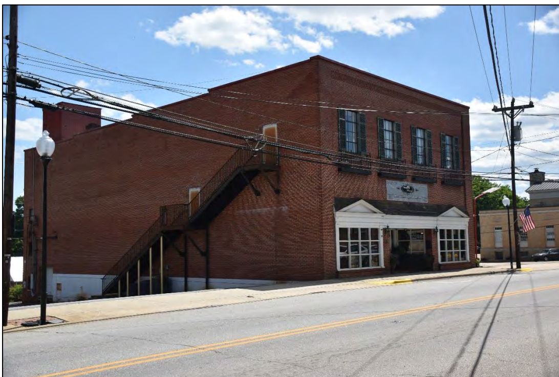
Figure 2.3.30. Gray Brothers Furniture Company Building (WK0253), facing southwest.
