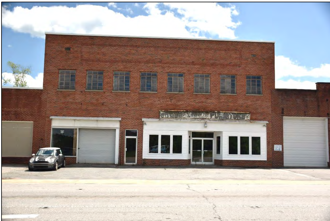
Figure 2.3.8. WK0452, 327 East Main Street, facing south.
