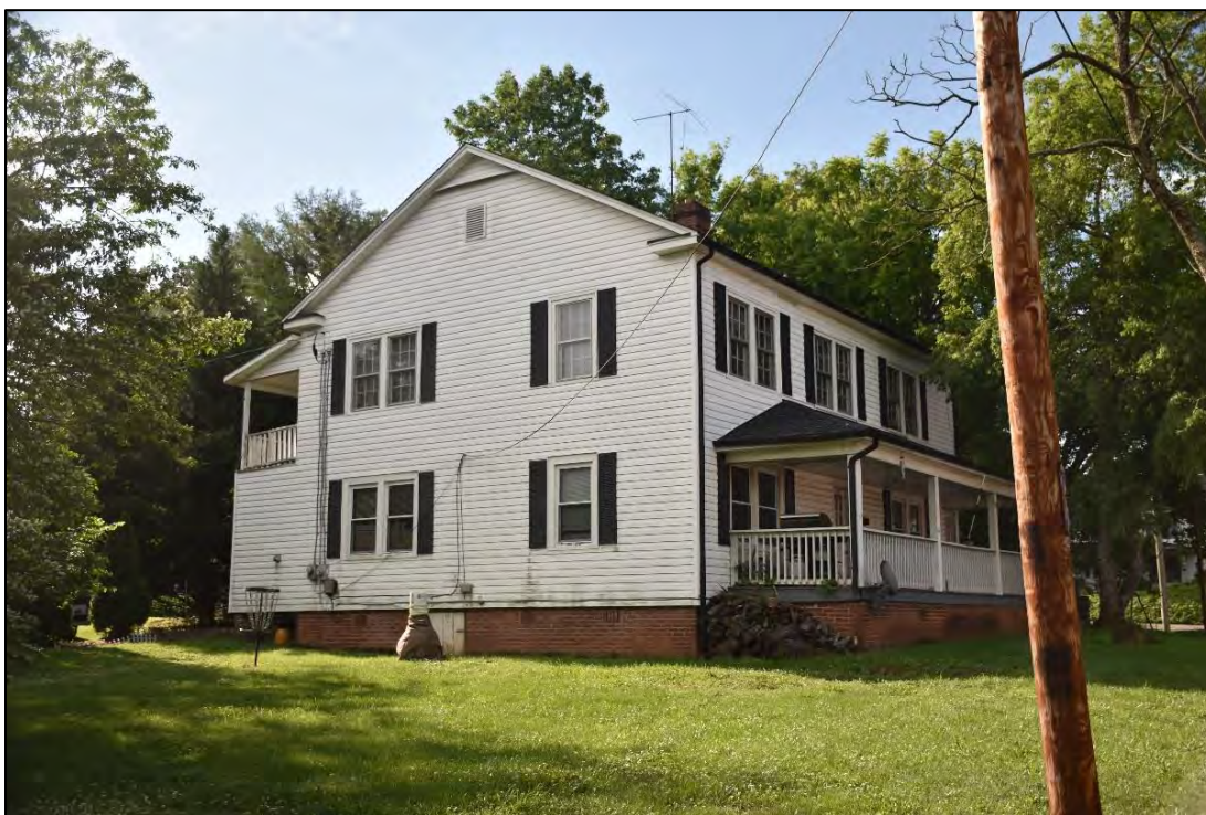
Figure 2.2.47. East Wilkesboro Historic District (WK0450), parcel 22, Greene House, facing southeast.
