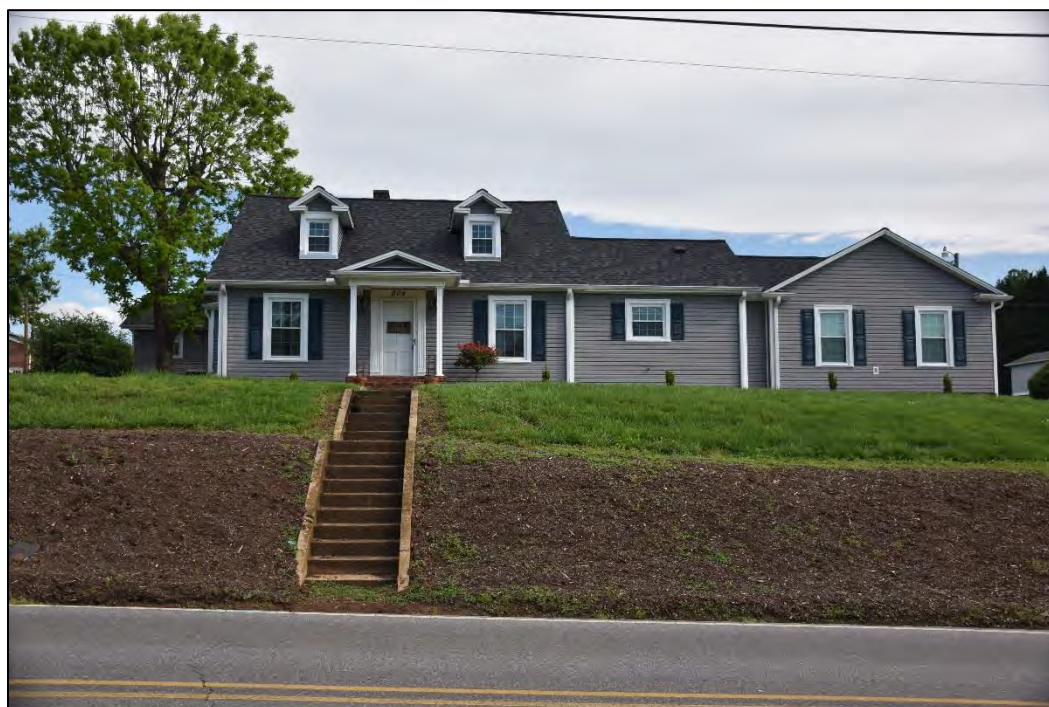
Figure 2.2.22. East Wilkesboro Historic District (WK0450), parcel 12, Garza House, facing north.
