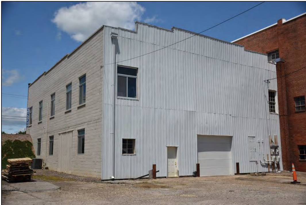
Figure 2.3.5. WK0451, 309 East Main Street, facing northeast.
