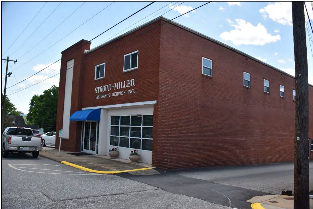
Figure 2.3.28. Wilkesboro Building and Loan Association Building (WK0219), facing southwest.
