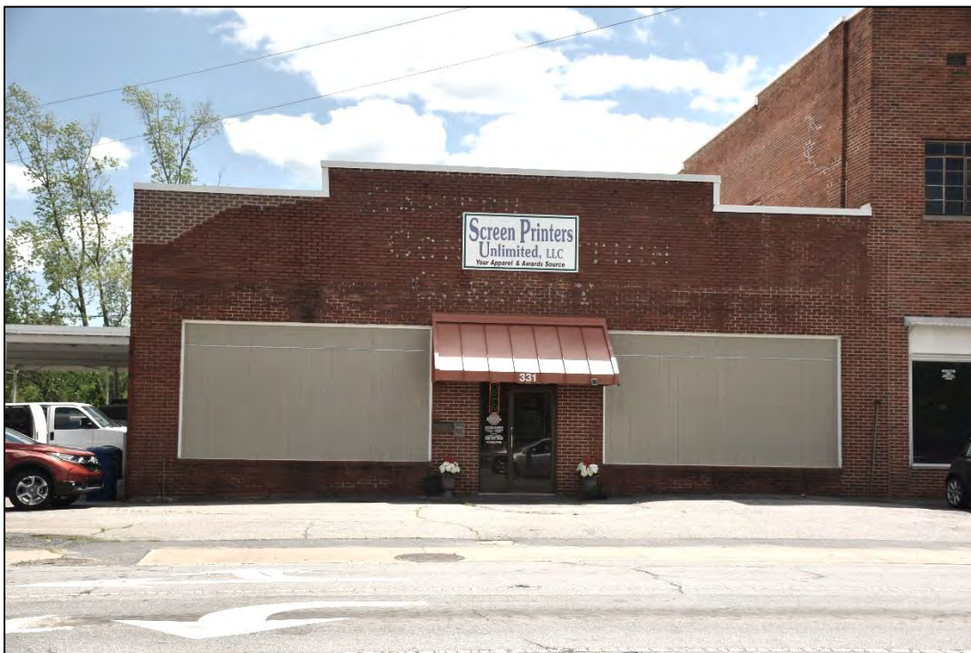
Figure 2.3.13. WK0453, 331 East Main Street, facing south.
