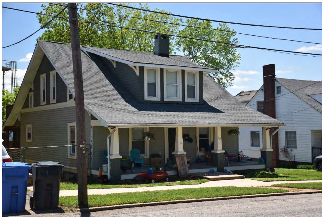
Figure 2.5.17. House at 507 C Street, North Wilkesboro (NSN), facing southwest.
