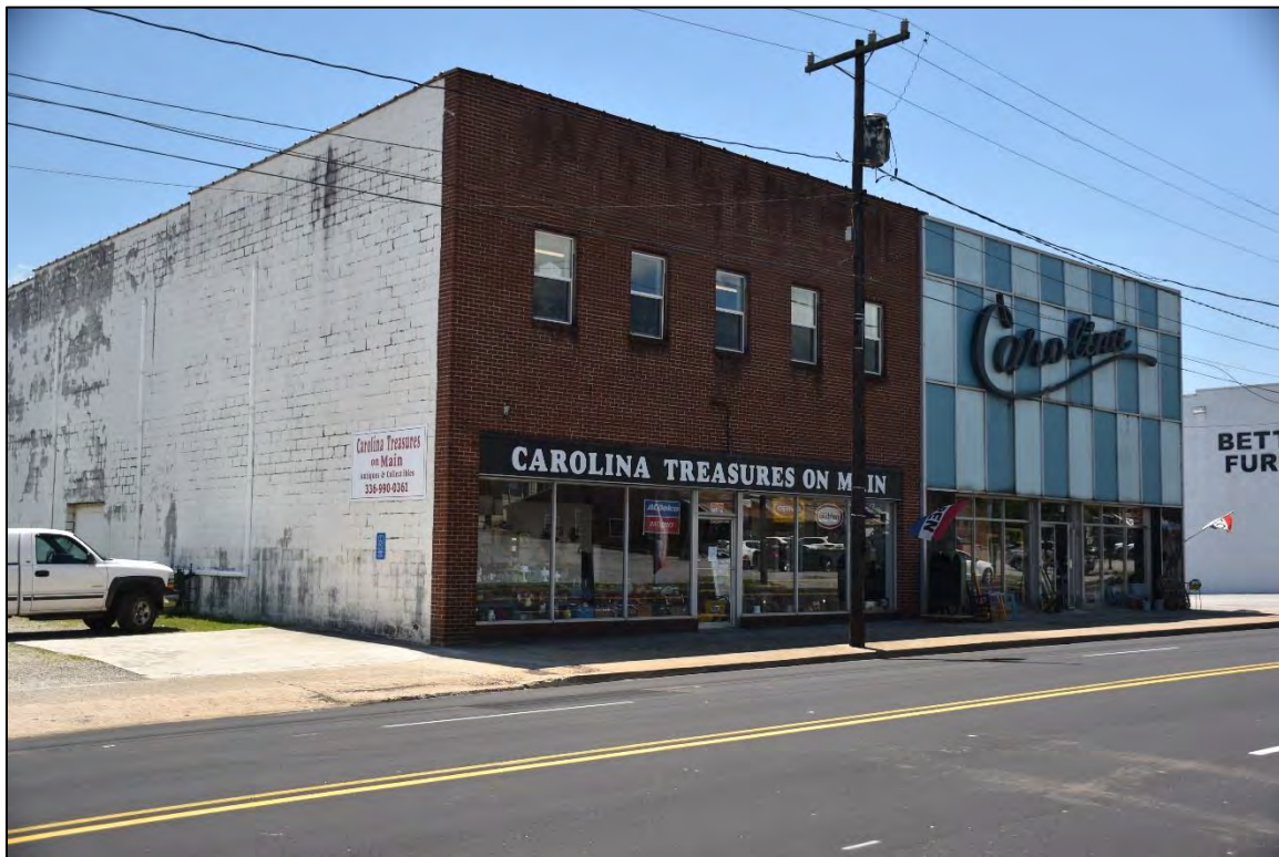
Figure 2.3.32. Commercial building, 515 Main Street, North Wilkesboro (NSN), facing southwest.
