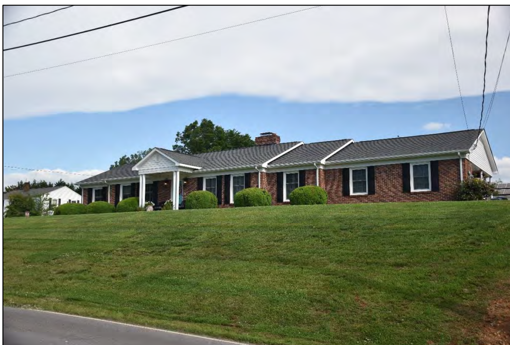
Figure 2.2.27. East Wilkesboro Historic District (WK0450), parcel 14, Jones-Parker House, facing northwest.
