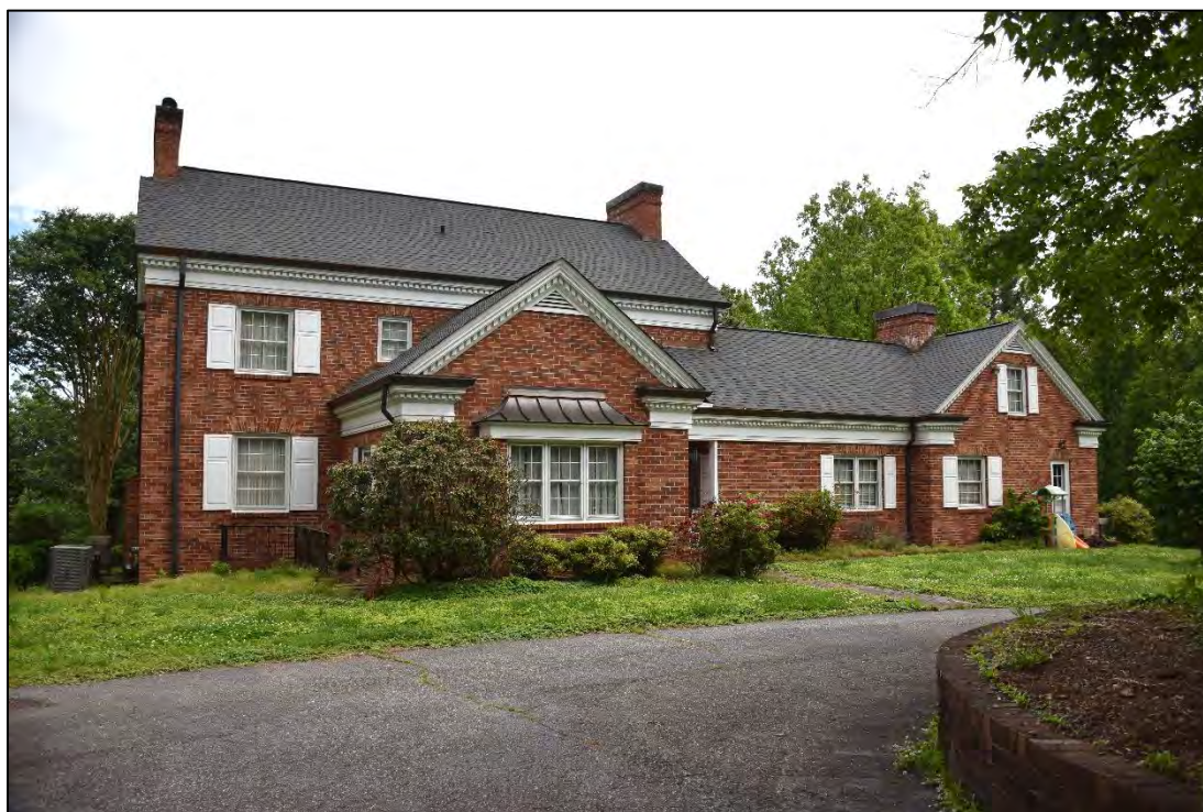
Figure 2.4.9. Julius A. Rousseau House (WK0454), facing northeast.
