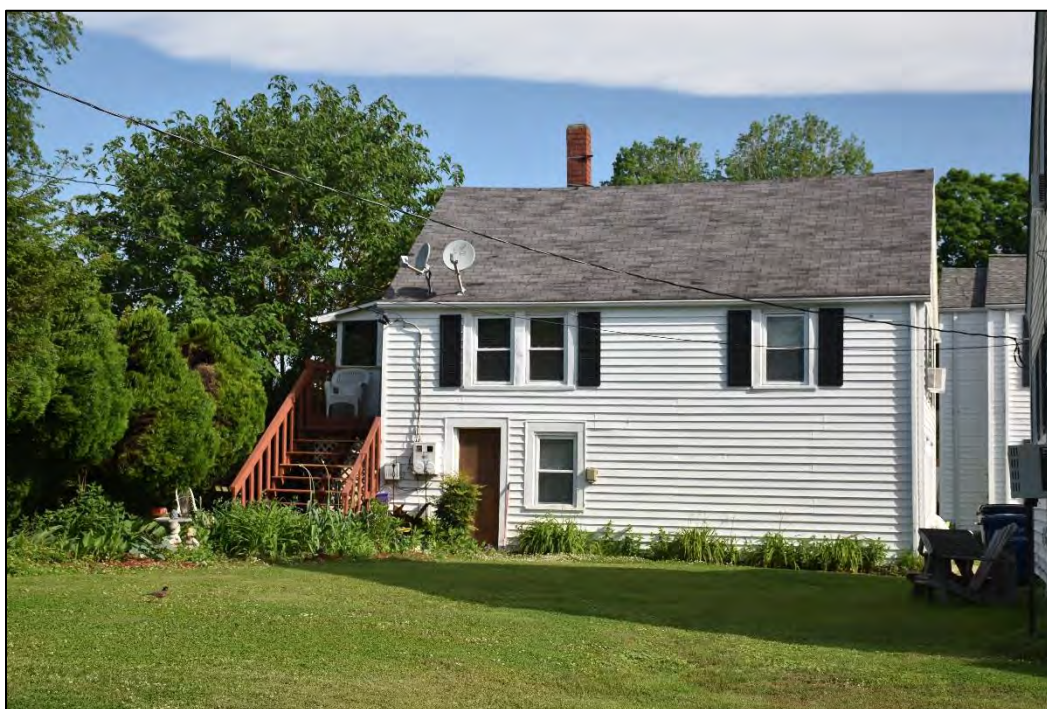
Figure 2.2.31. East Wilkesboro Historic District (WK0450), parcel 15, Forrester-Hayes House, garage apartment, facing north.
