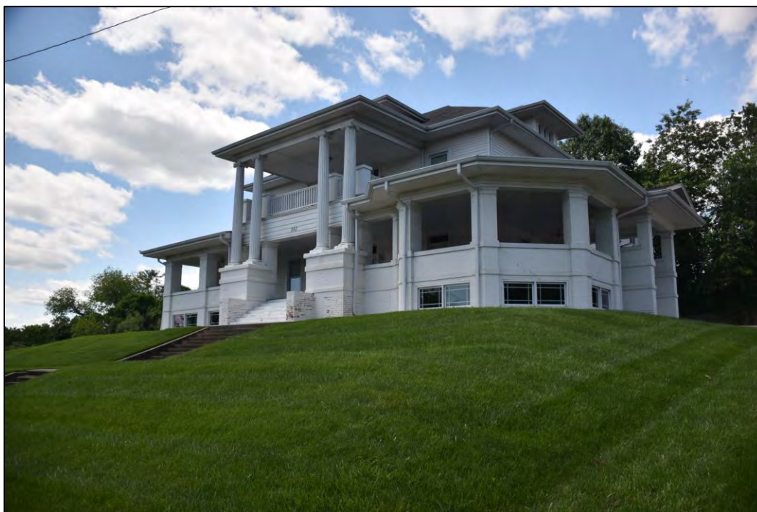
Figure 2.4.21. W. F. Trogden House (WK0169), facing northwest.
