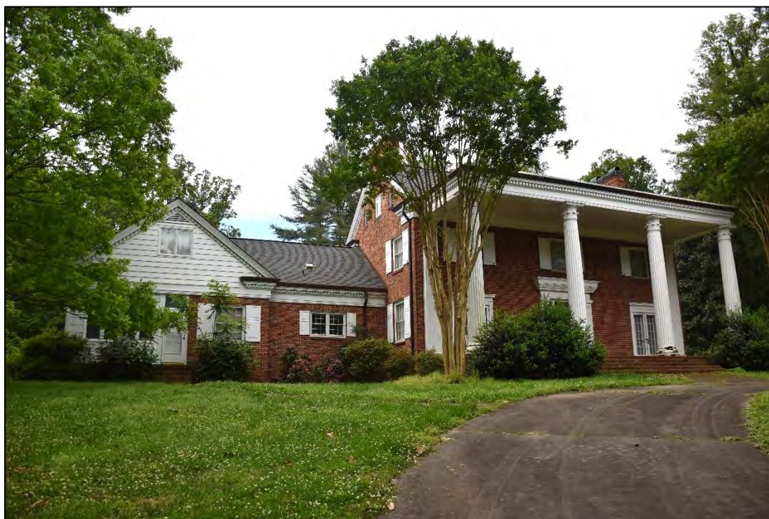
Figure 2.4.5. Julius A. Rousseau House (WK0454), facing southwest.
