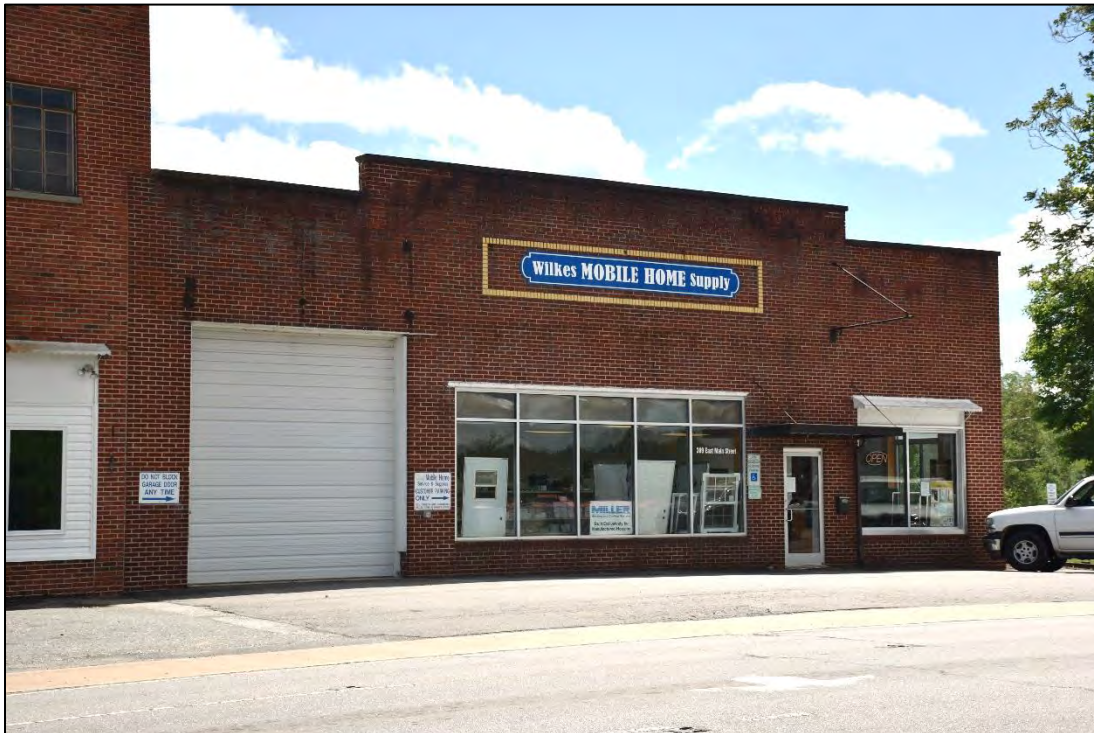
Figure 2.3.3. WK0451, 309 East Main Street, facing south.
