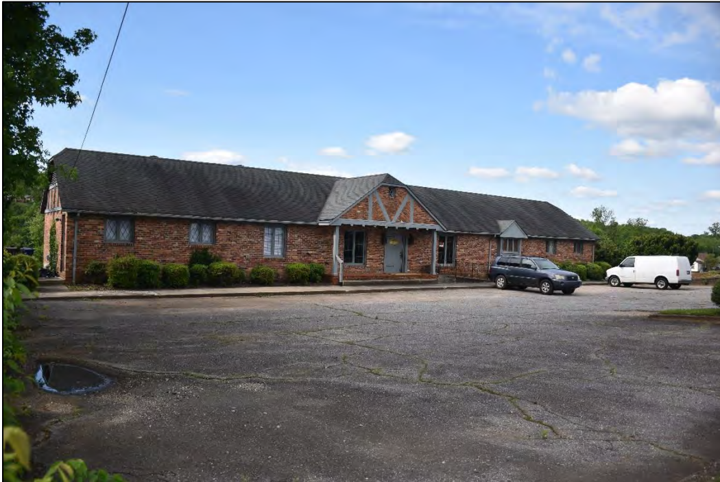
Figure 2.2.14. East Wilkesboro Historic District (WK0450), parcel 7, Hicks Building, facing southwest.
