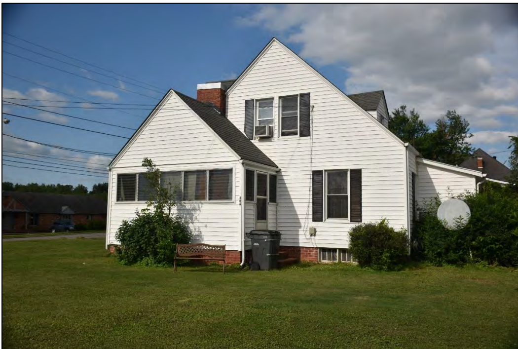
Figure 2.2.29. East Wilkesboro Historic District (WK0450), parcel 15, Forrester-Hayes House, facing west.
