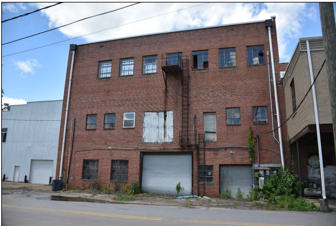
Figure 2.3.10. WK0452, 327 East Main Street, facing north.
