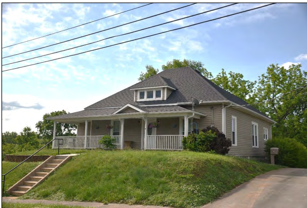
Figure 2.2.19. East Wilkesboro Historic District (WK0450), parcel 10, unnamed House (WK0030), facing southeast.
