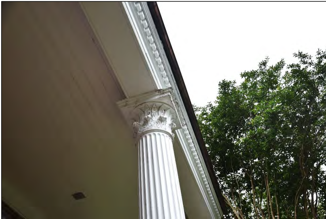
Figure 2.4.2. Julius A. Rousseau House (WK0454), porch detail, facing southwest.
