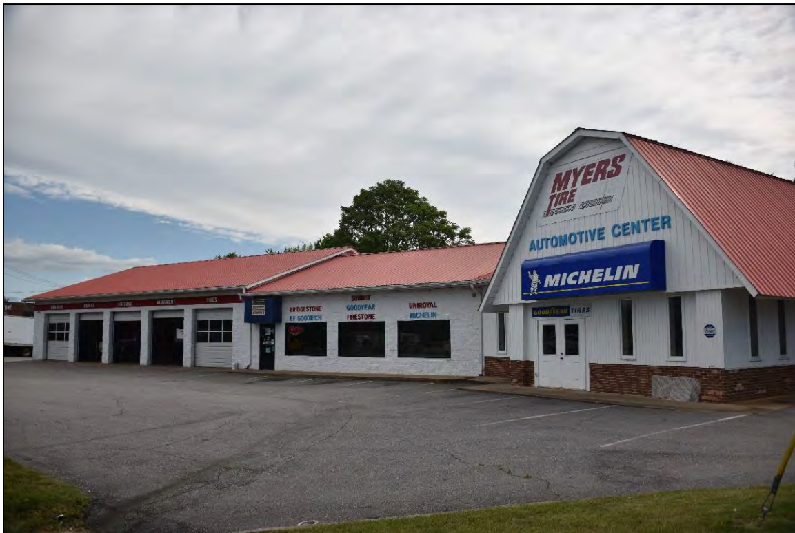
Figure 2.2.48. East Wilkesboro Historic District (WK0450), parcel 23, Myers Tire, facing north.
