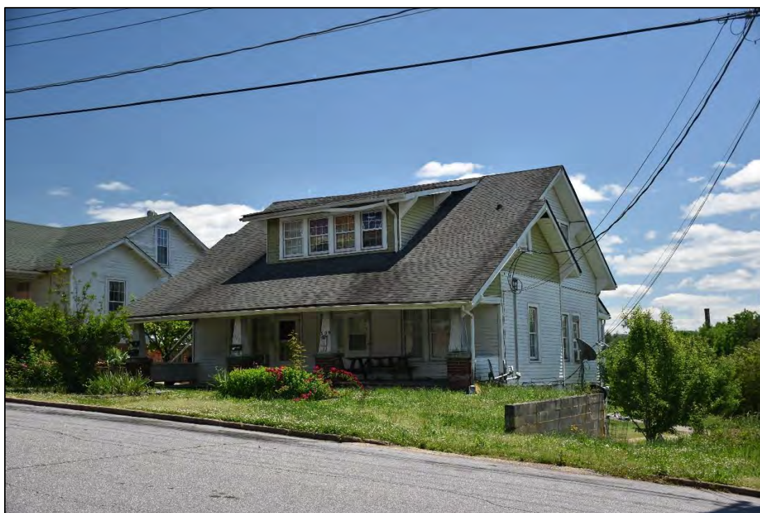
Figure 2.5.16. House at 309 D Street, North Wilkesboro (NSN), facing southeast.
