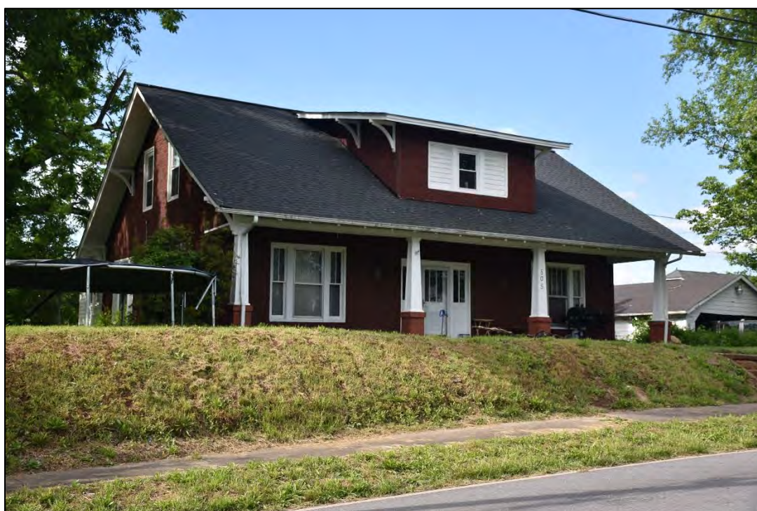
Figure 2.2.16. East Wilkesboro Historic District (WK0450), parcel 8, Henderson House, facing southwest.
