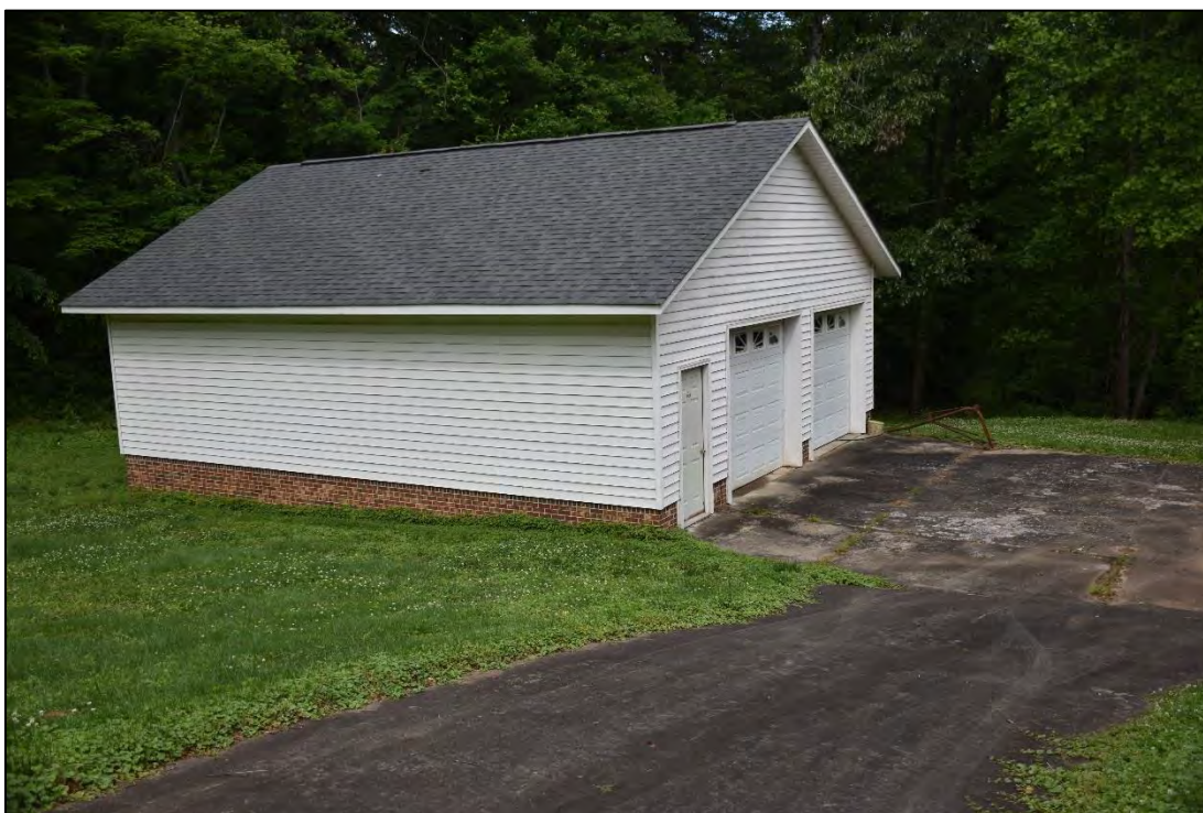
Figure 2.4.11. Julius A. Rousseau House (WK0454), modern garage, facing northwest.
