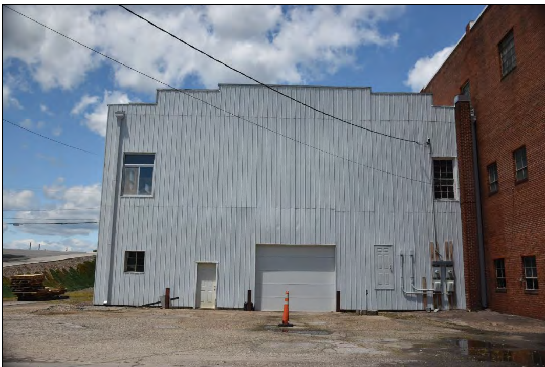
Figure 2.3.6. WK0451, 309 East Main Street, facing north.
