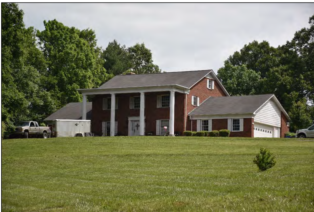
Figure 2.4.26. House at 1524 Dogwood Drive (NSN), facing north.
