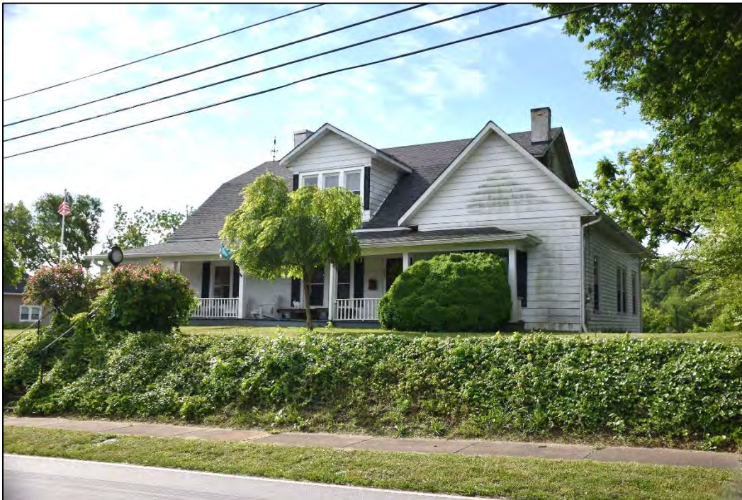
Figure 2.2.17. East Wilkesboro Historic District (WK0450), parcel 9, J. F. Jordan House (WK0042), facing southeast.
