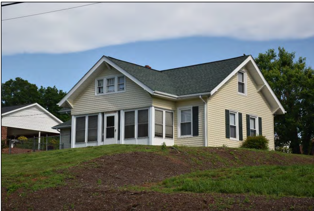
Figure 2.2.25. East Wilkesboro Historic District (WK0450), parcel 13, Hayes-Parker House, facing northwest.
