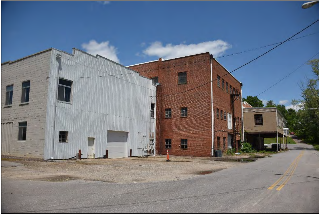
Figure 2.3.2. 300 East Main Commercial Block (WK0451, WK0452, and WK0453), facing northeast.
