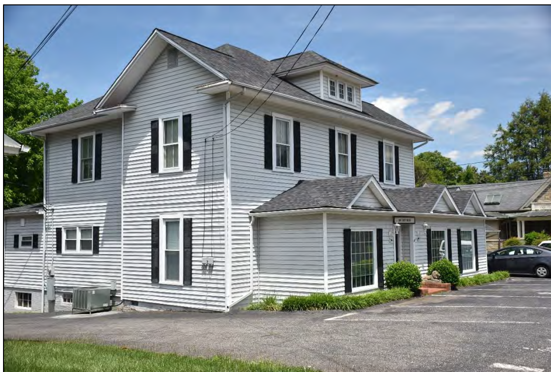
Figure 2.2.60. Somers-Bumgarner House (WK0232), facing northeast.
