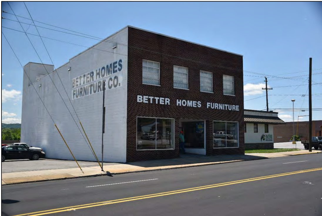
Figure 2.3.33. Commercial building, 527 Main Street, North Wilkesboro (NSN), facing southwest.
