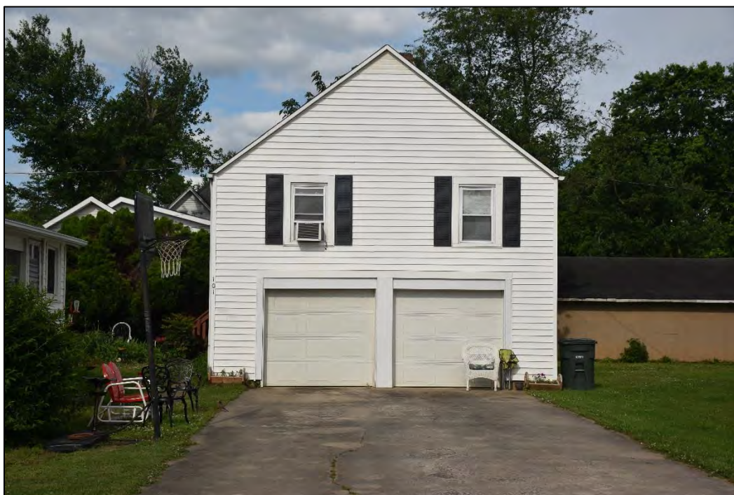
Figure 2.2.30. East Wilkesboro Historic District (WK0450), parcel 15, Forrester-Hayes House, garage apartment, facing west.
