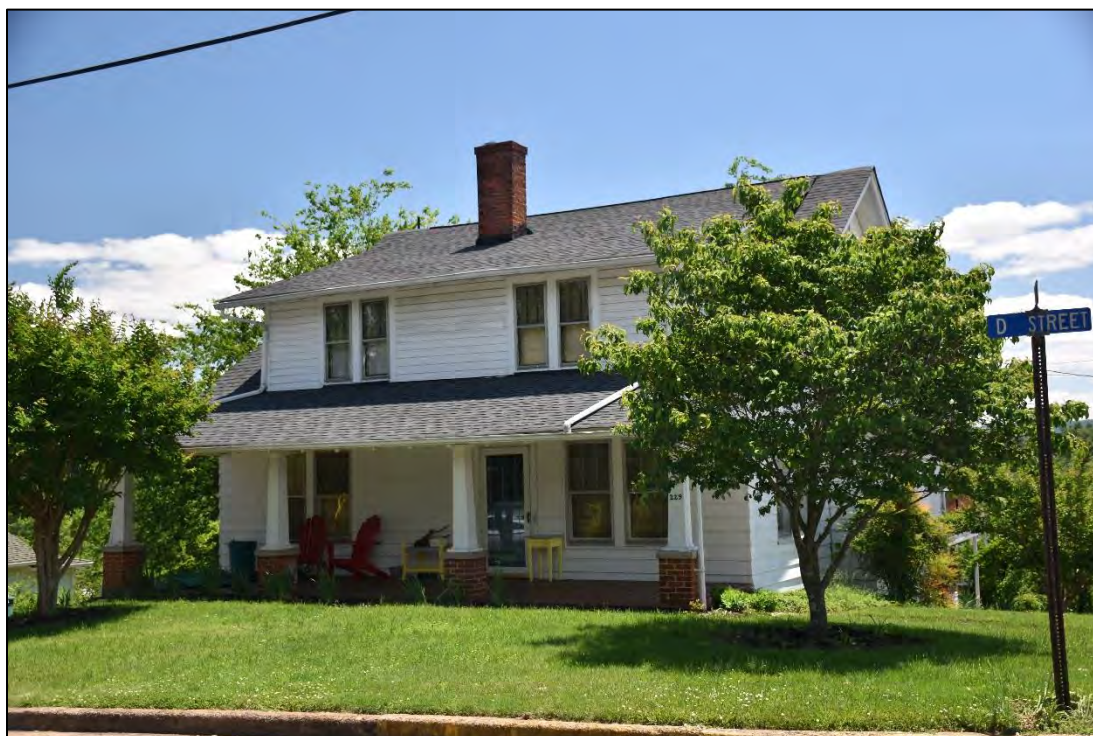
Figure 2.5.15. House at 229 D. Street, North Wilkesboro (NSN), facing southeast.
