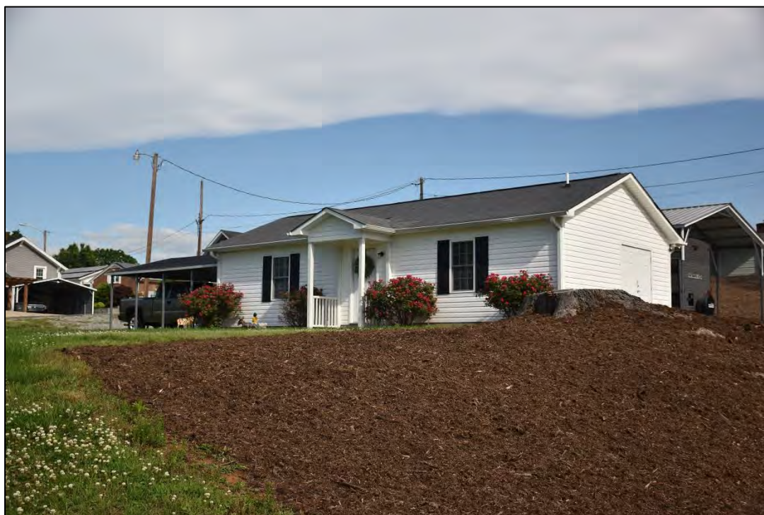
Figure 2.2.21. East Wilkesboro Historic District (WK0450), parcel 11, Parker House, facing northeast.
