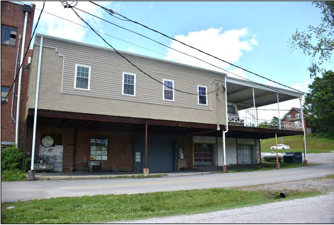
Figure 2.3.16. WK0453, 327 East Main Street, facing north.
