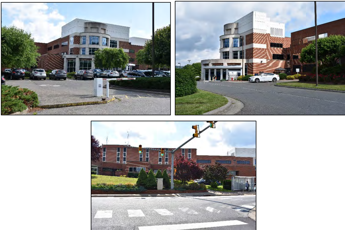
Figure 45. Watauga Medical Center principal buildings
