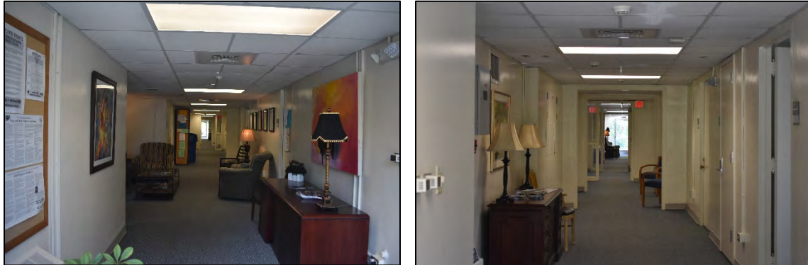
Figure 43. Left, looking east to west down ground floor corridor; right, looking west to east down corridor
