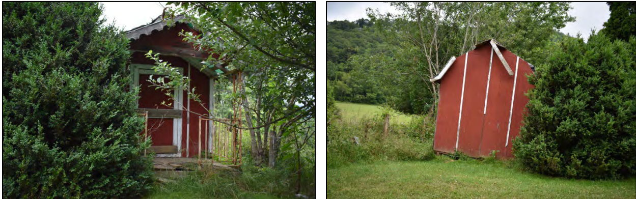
Figure 16. South front elevation of shed, at left, and north rear elevation, at right
