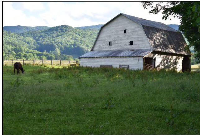
Figure 23. Barns at the Winfield Scott Farthing House (upper left), Rev. Ed Farthing House (upper right), and Henry Taylor Barns property (bottom)
