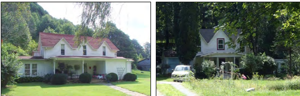
Figure 18. Eli and Louise Church House (WT-0434), left, and Jack Campbell House (WT-0434), right, in Mabel Historic District in 2016 (photographer: Sarah Woodard David)
