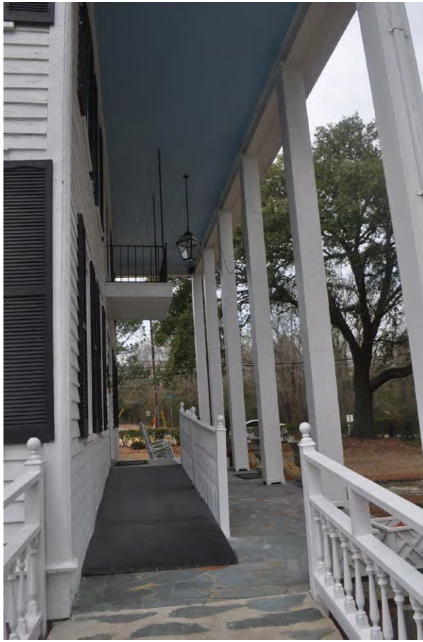
Plate 5.11: View under the front porch of the Moulder House.
