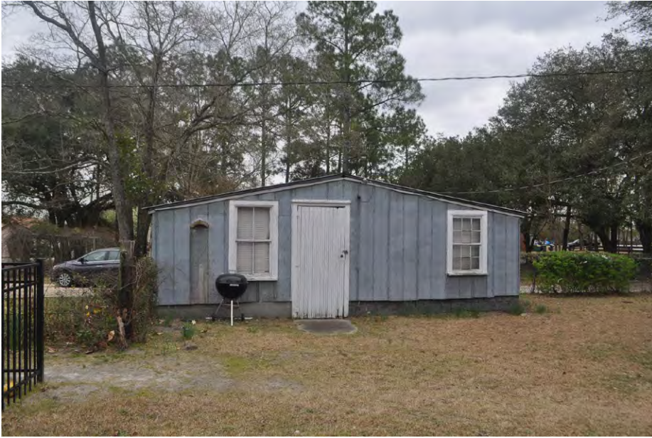
Plate 5.27: View of the workshop on the subject parcel.
