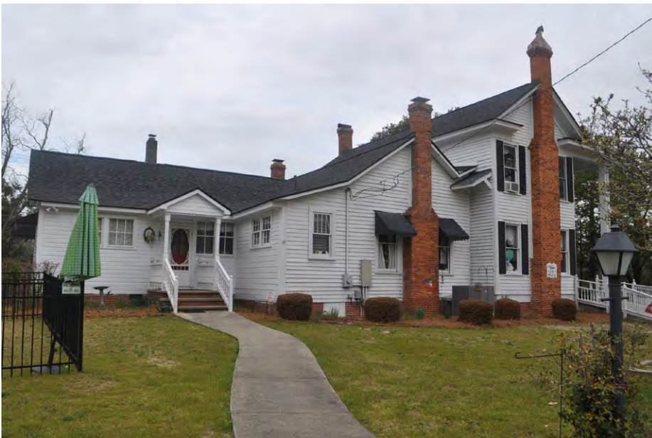
Plate 5.7: View of the southeast side of the Moulder House.
