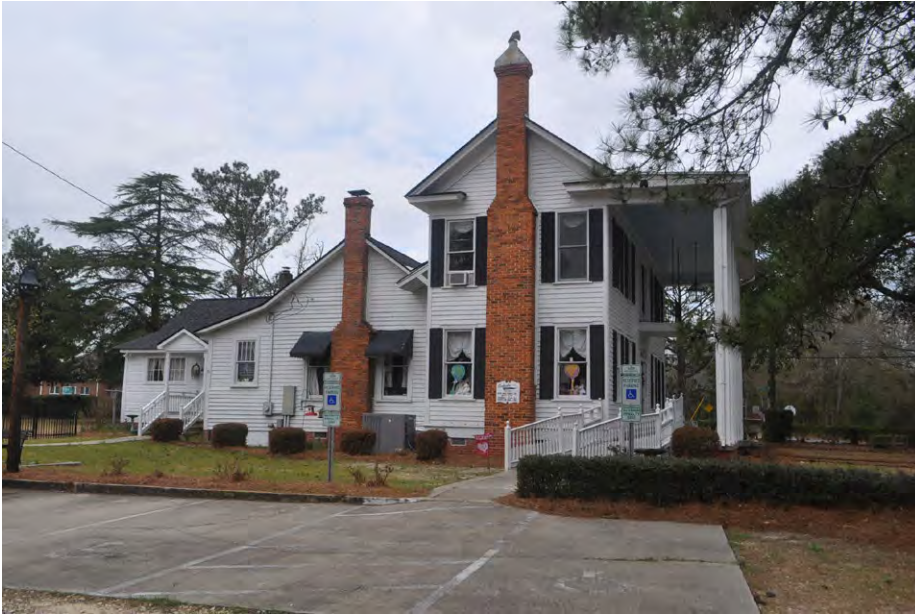
Plate 5.9: View of the southeast side of the Moulder House.
