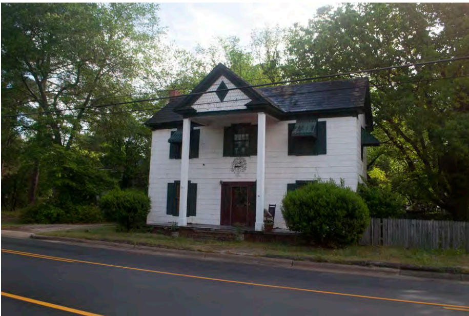
Plate 5.30: View of number 3957 South Main Street in Hope Mills.
