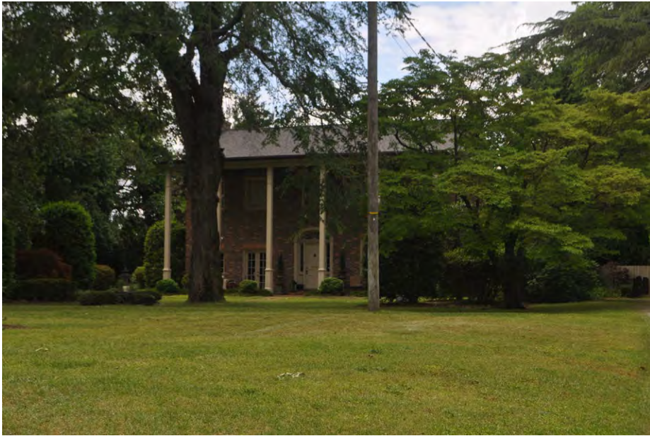
Plate 5.31: View of number 218 Bradford Avenue in Fayetteville.
