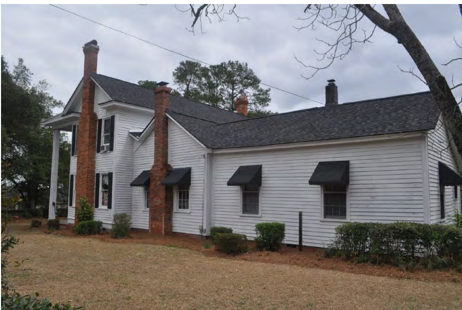
Plate 5.5: View of the northwest side of the Moulder House.
