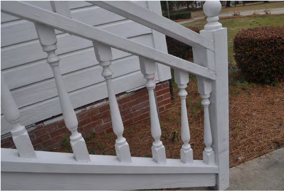
Plate 5.16: View of the stair on the apartment addition's porch.
