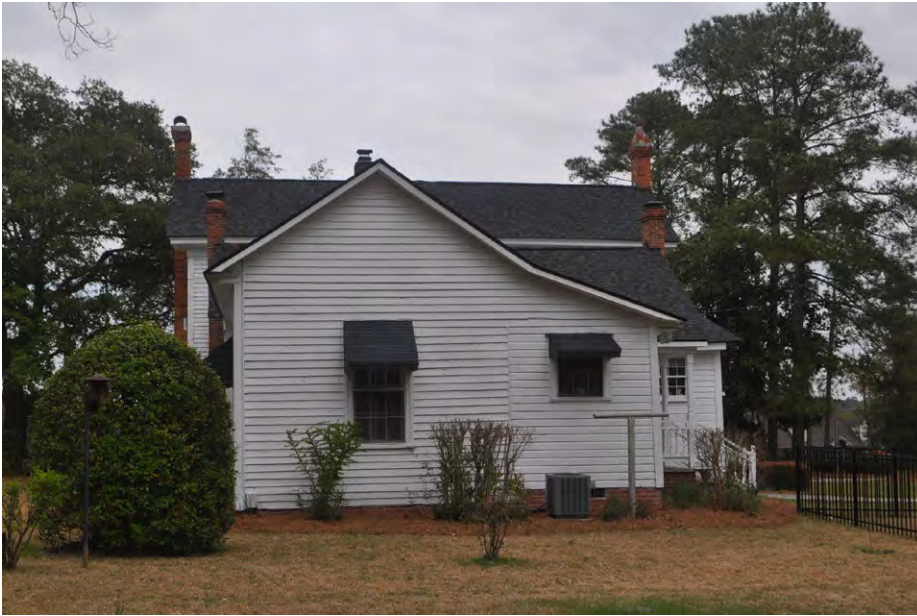
Plate 5.6: View of the rear (southwest side) of the Moulder House.
