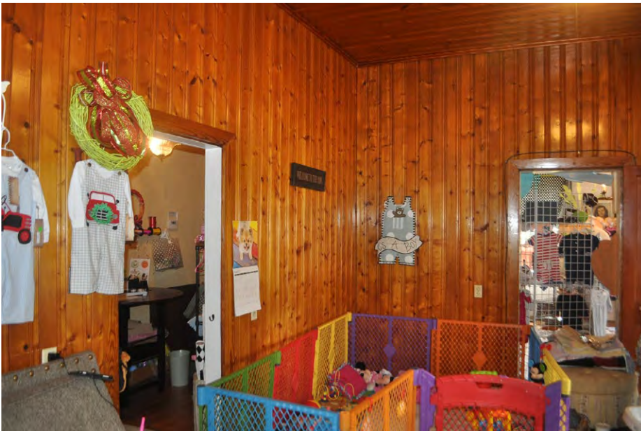
Plate 5.24: View of the southeast middle room.
