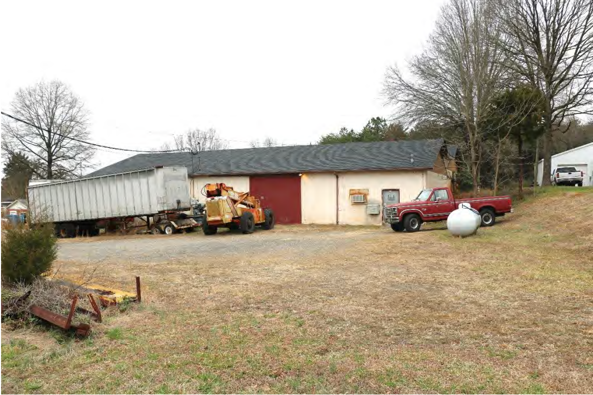
20. Storage Building, 129 Victory Grove Church Road, ca.1965, PIN 3632-26-4974,view facing north.
