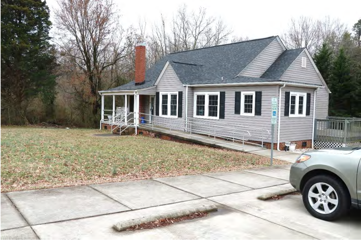
19. Cutting House Salon, garage, and shed, 1704 Gastonia Highway, ca.1945, PIN 3632-26-1702, view facing southwest.
