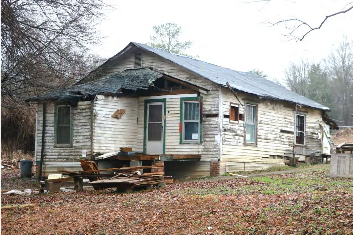
11. House, 1537 S. Aspen Street, ca.1940, PIN 3632-18-2240, view facing east.
