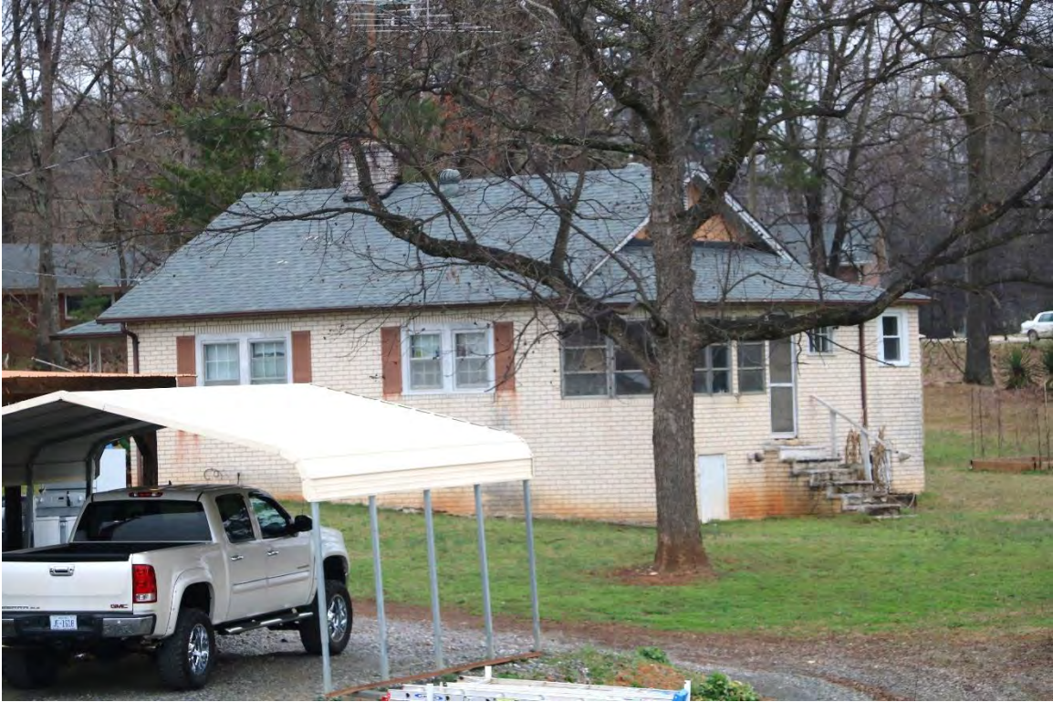
24. House and shed, 1285 Rocky Hill Lane, ca.1945, PIN 3632-27-1385, view facing east.
