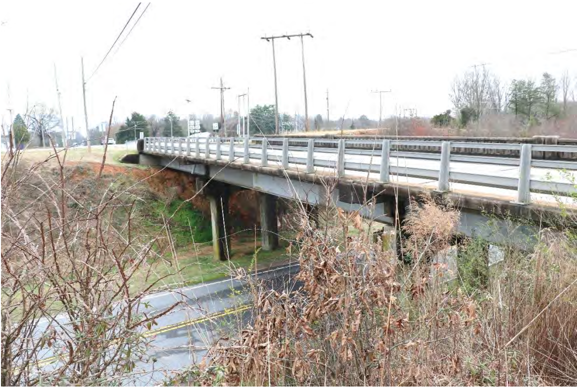
Bridge No. 30, constructed 1955, view facing southwest.
