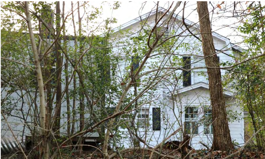
Figure 7. Side (north) elevation, view facing southeast. Mead & Hunt photograph.
