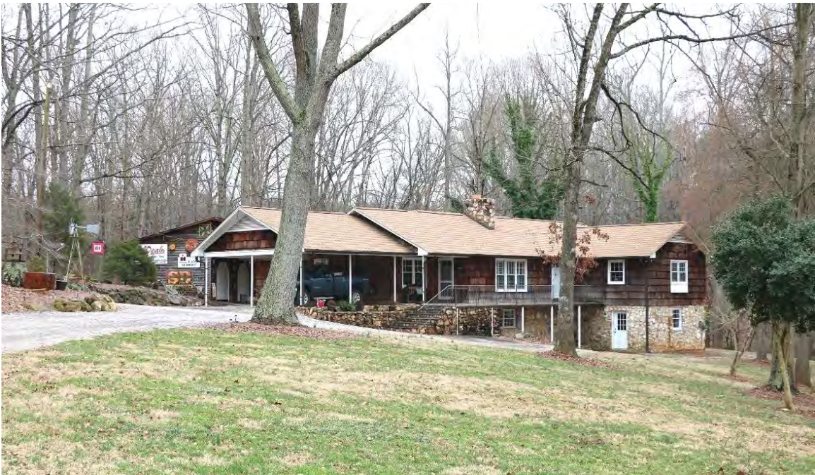
16. House, garage, and sheds, 229 Rocky Lane, 1965, PIN 3632-16-0702, view facing south.
