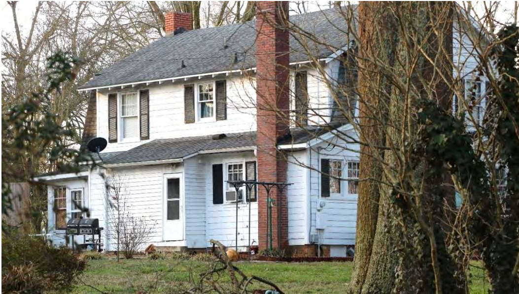
Figure 6. Rear (east) and side (north) elevations, view facing south. Mead & Hunt photograph.
