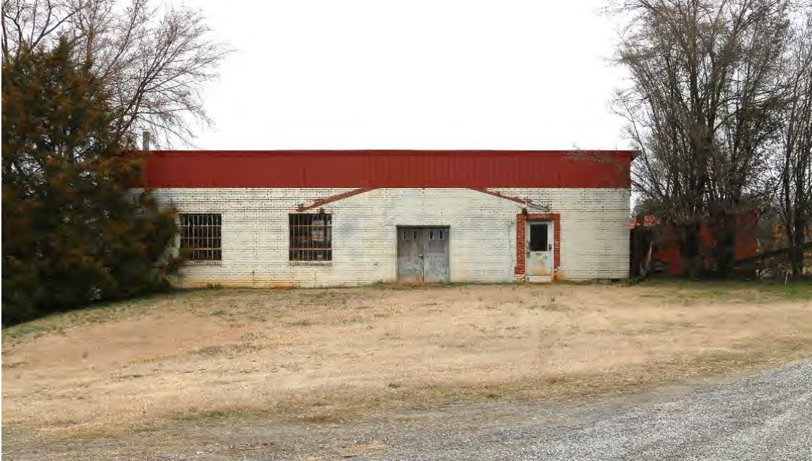
15. Deal Construction, Inc., 210 W. NC 150 Bypass, ca.1950, PIN 3632-07-6775, view facing north.
