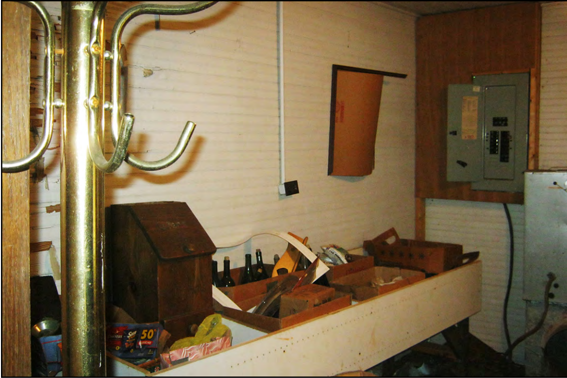
PLATE 8: Former Gulf Gas Station (RK1128), Interior View of Living Room, Rockingham County, North Carolina
