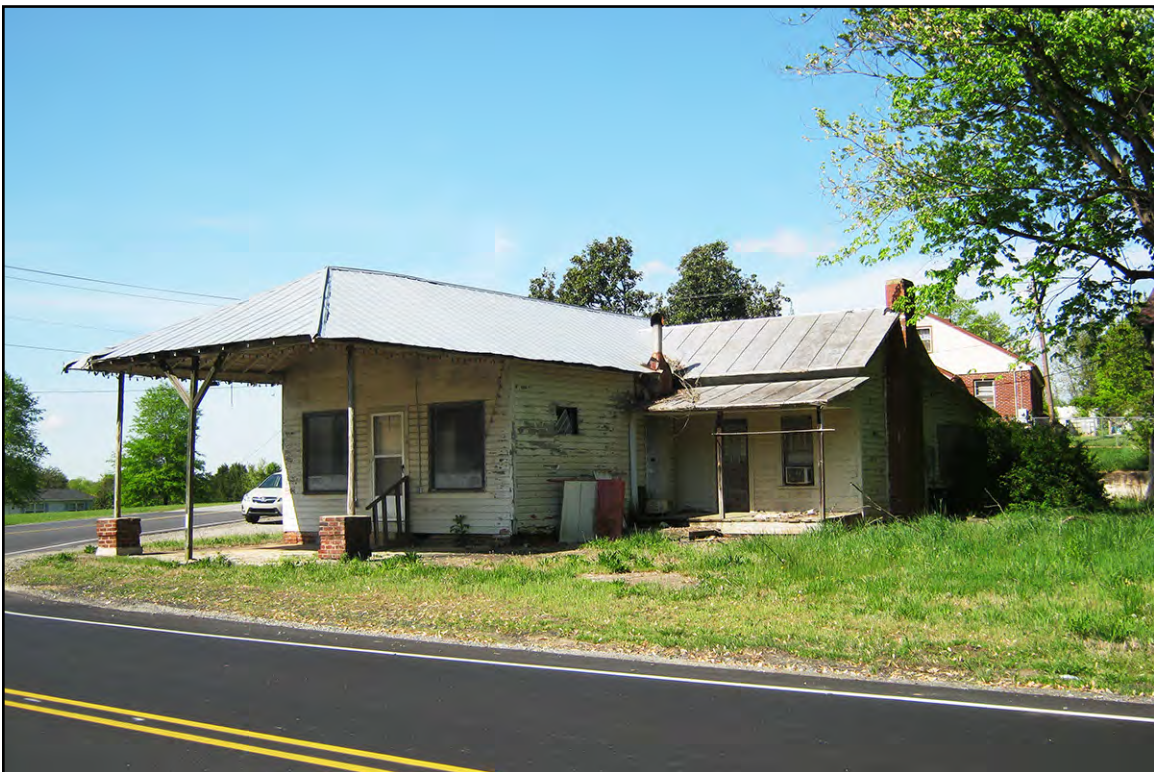
PLATE 2: Former Gulf Gas Station (RK1128), Oblique View of North and East Elevations, Rockingham County, North Carolina
