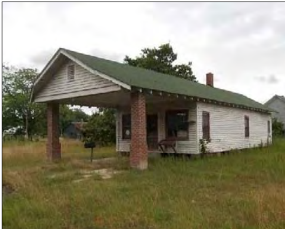
PLATE 14: Creekmore Store/Gas Station (CM0009), Looking West, Camden County, North Carolina (Dovetail 2013)
