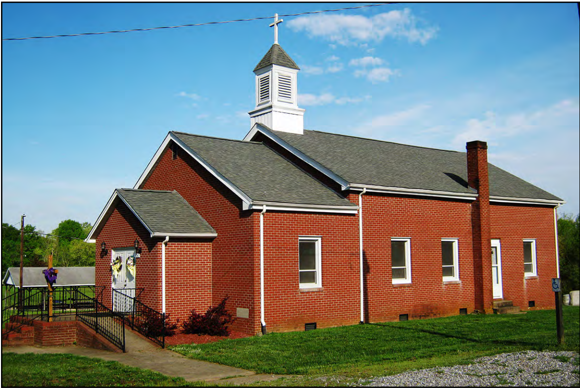
PLATE 30: Matthews Chapel United Methodist Church (RK1826), Looking Northwest, Rockingham County, North Carolina
