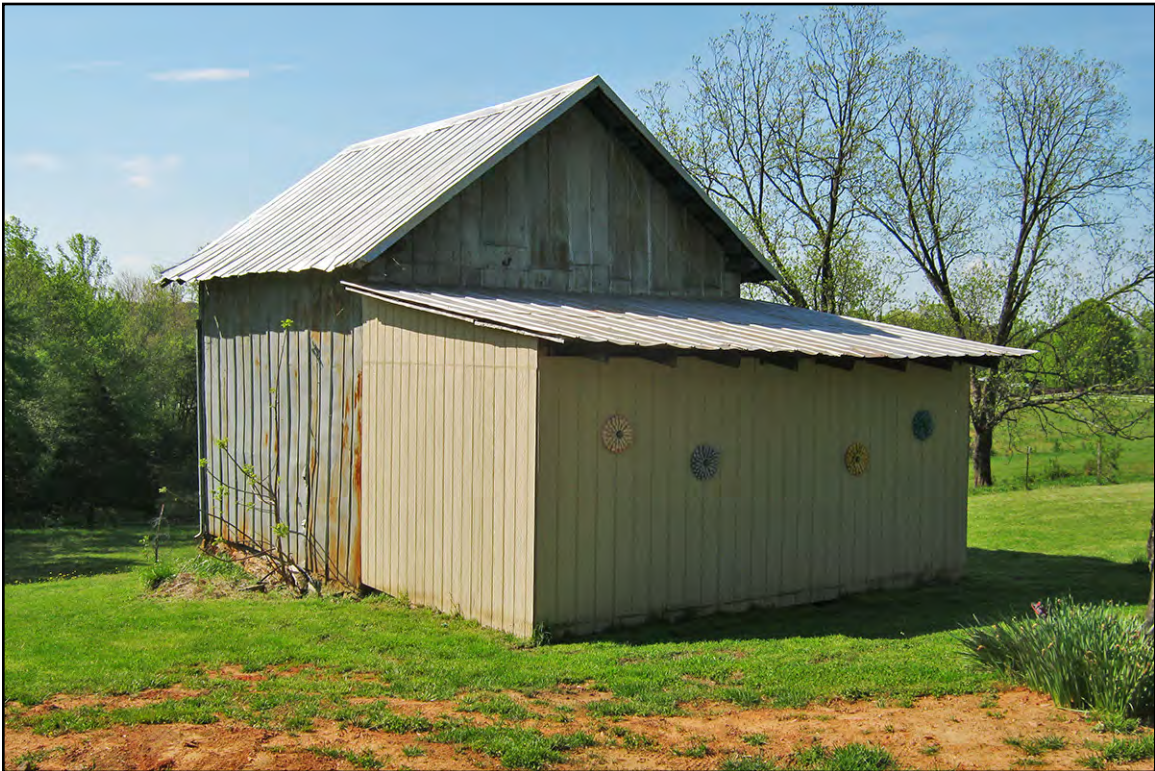
PLATE 23: Barn, Looking Southwest, Ed Matthews House (RK1130), Rockingham County, North Carolina
