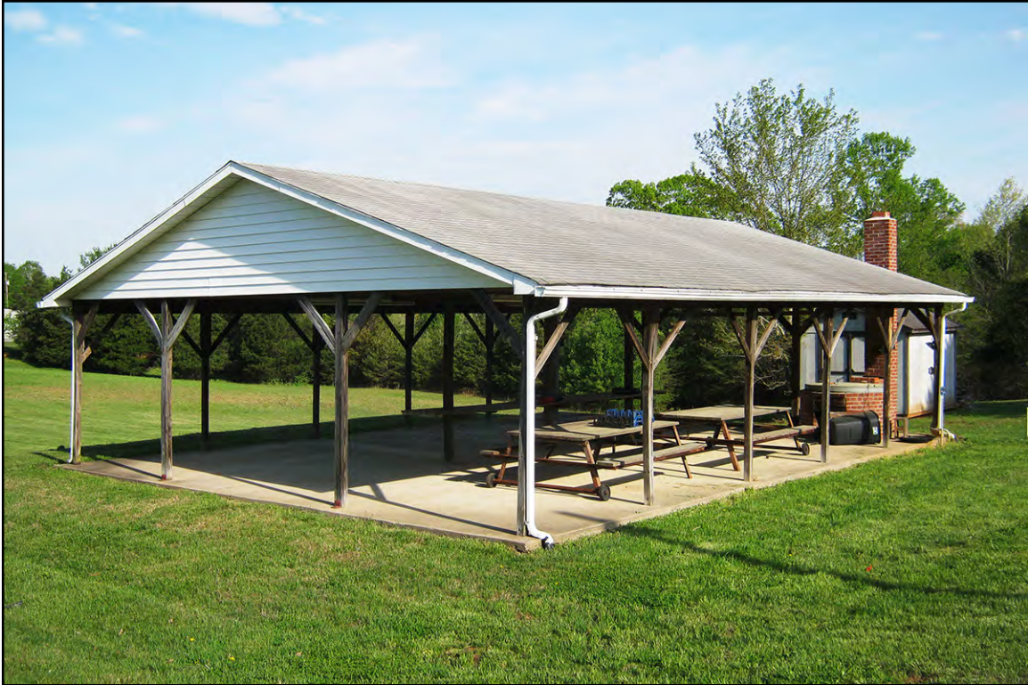
PLATE 36: Picnic Shelter, Matthews Chapel United Methodist Church (RK1826), Looking Northwest, Rockingham County, North Carolina
