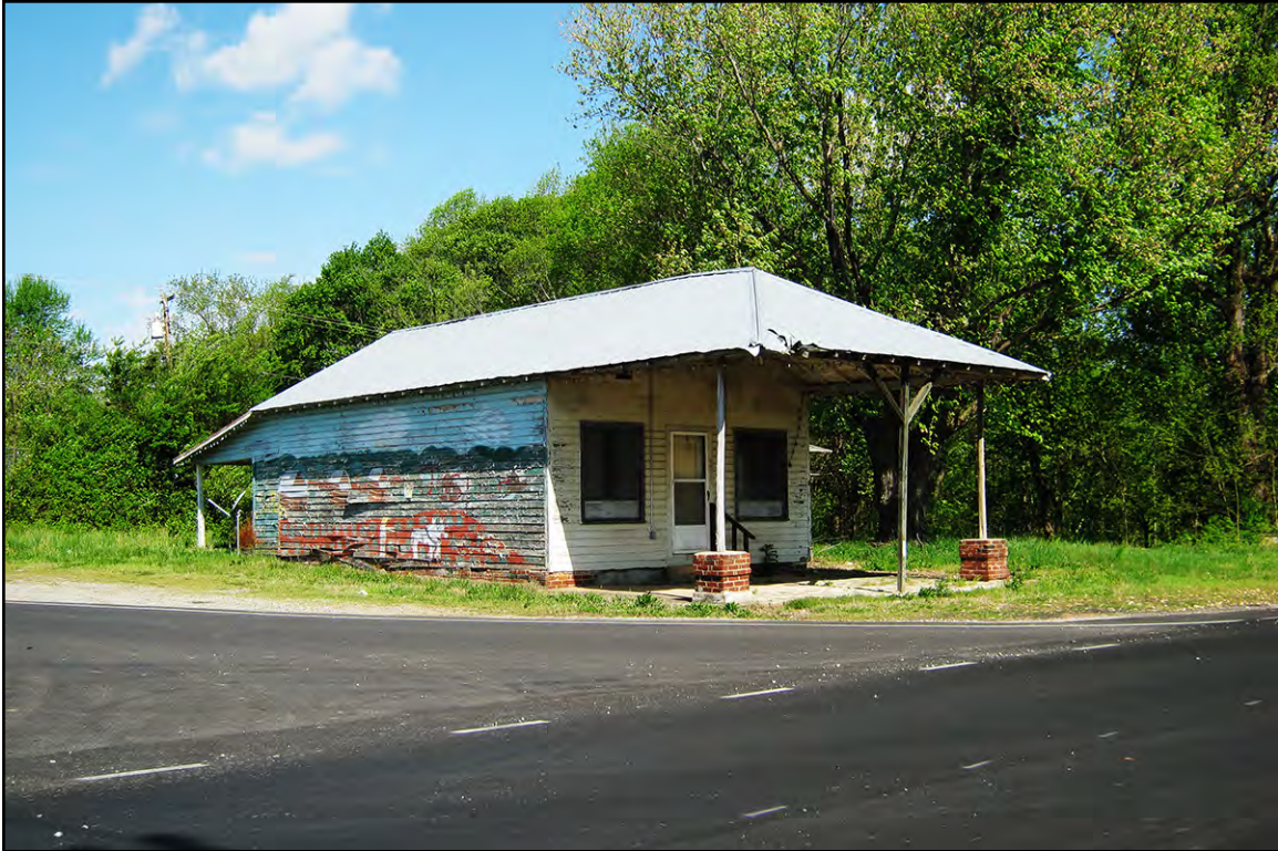
PLATE 1: Former Gulf Gas Station (RK1128), Oblique View of South and East Elevations, Rockingham County, North Carolina
