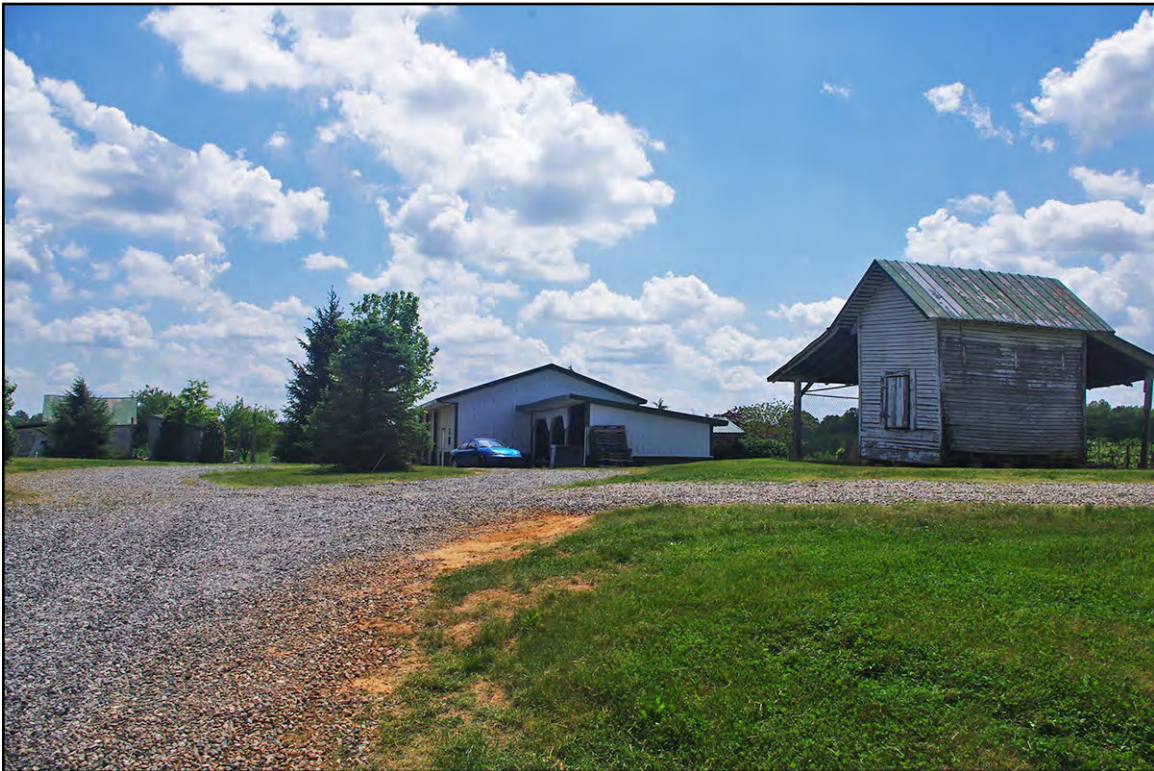
PLATE 28: Outbuildings on Rob Benton Joyce Farm, 364 Means Creek Road (RK1156), Looking West, Rockingham County, North Carolina
