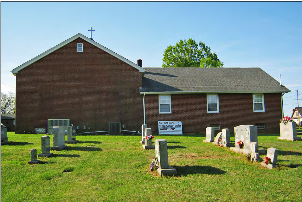
PLATE 32: Matthews Chapel United Methodist Church (RK1826), Looking South, Rockingham County, North Carolina
