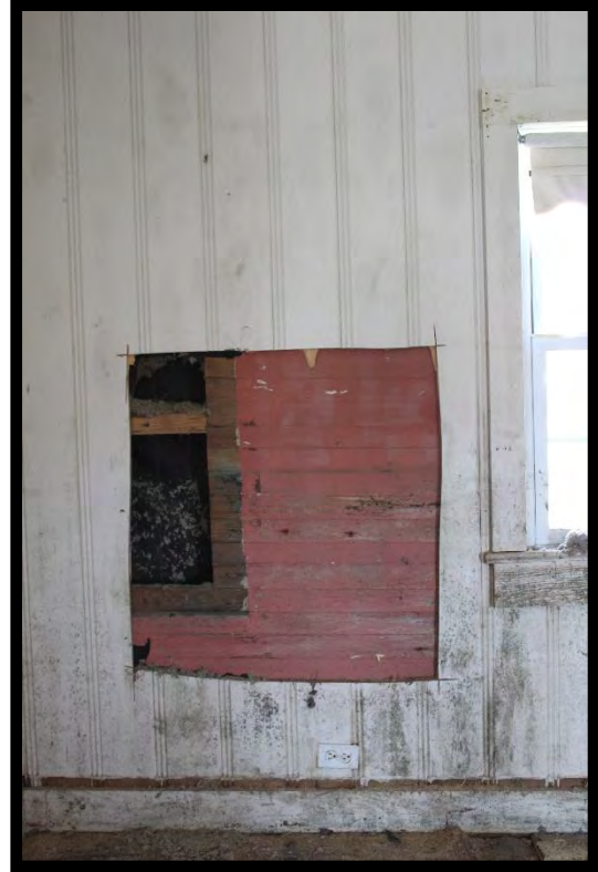
Figure 22: Maulsby and Susan Stephens House, Original Flush Boards and Window Opening.
