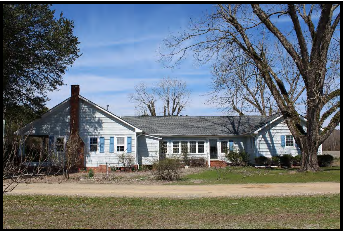
Figure 14: Mulsby and Susan Stephens House, Looking North.
