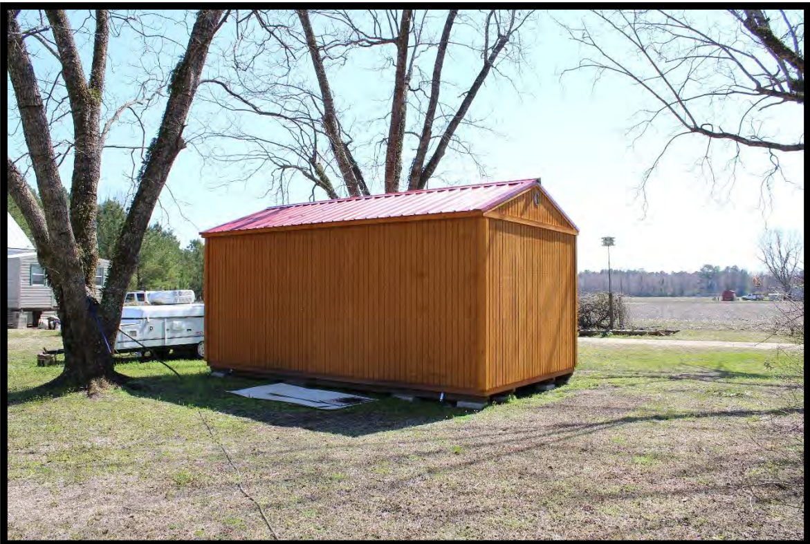
Figure 27: Maulsby and Susan Stephens House, Secondary Dwelling, Looking Southeast.
