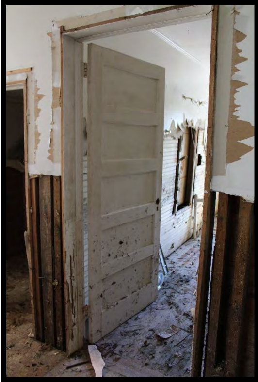
Figure 21: Maulsby and Susan Stephens House, Original Door and Window Opening.
