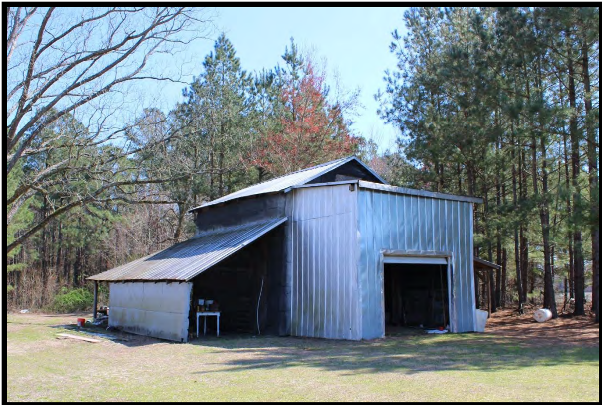
Figure 31: Maulsby and Susan Stephens House, Tobacco Barn and Additions, Looking Southeast.
