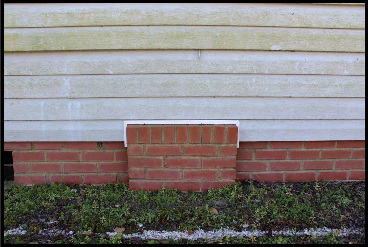
Figure 6: Maulsby and Susan Stephens House, Foundation and Piers.
