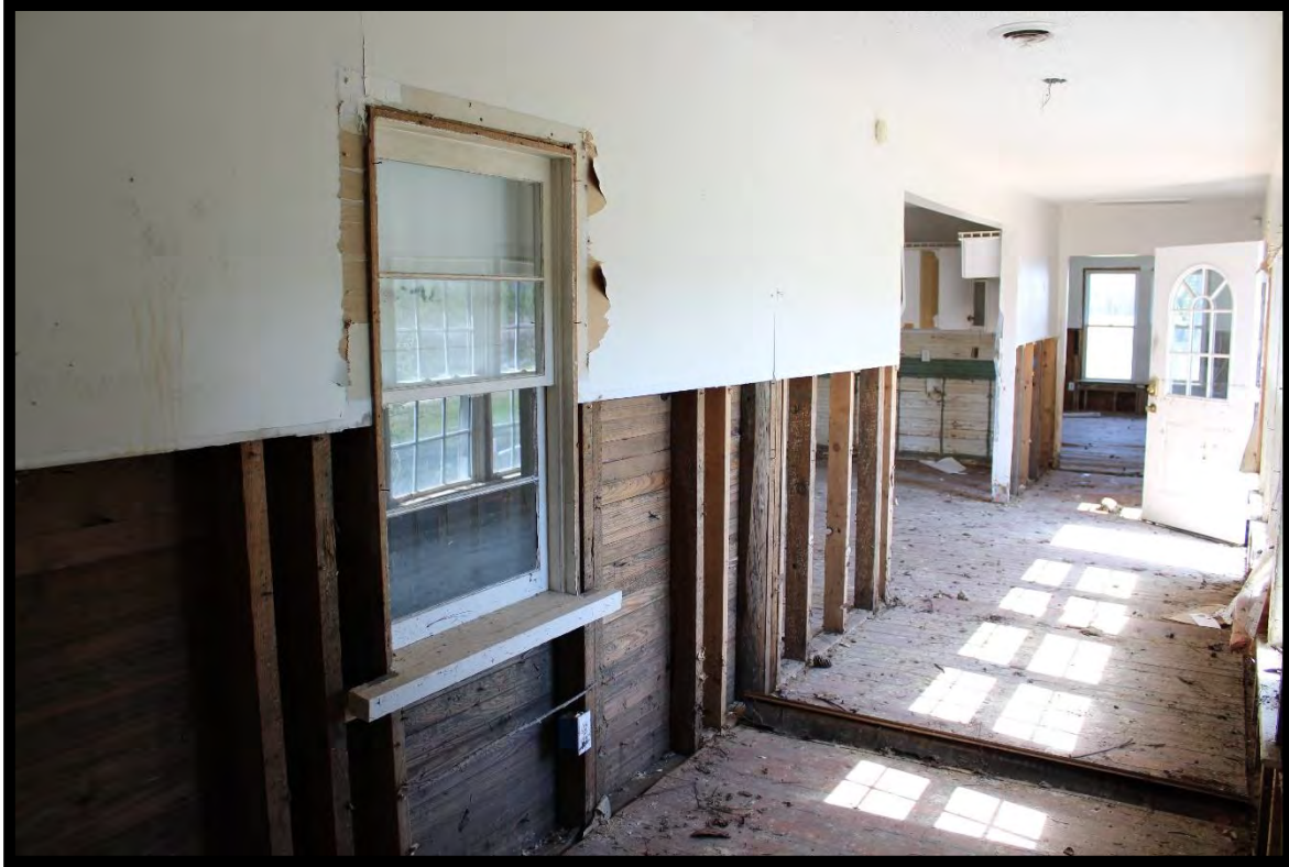
Figure 23: Malsby and Susan Stephens House, Original Window and Hall to Rear Addition.
