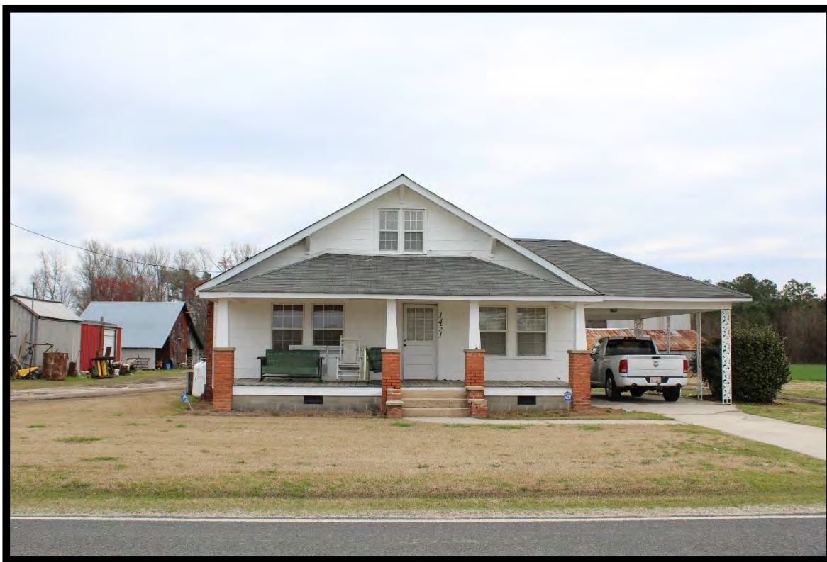
Figure 63: 1451 Long Branch Road, Lumberton, North Carolina, Looking East.
