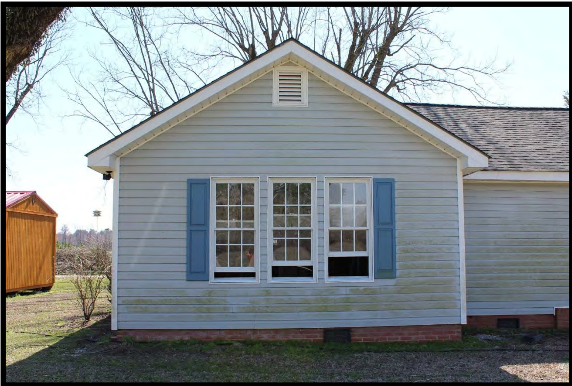
Figure 12: Maulsby and Susan Stephens House, Looking South.
