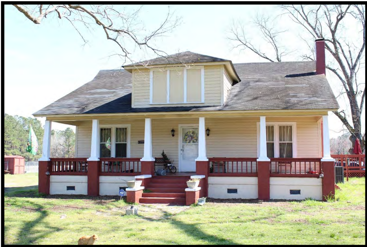
Figure 42: Giles Stephens Homeplace, Looking North-Northeast.
