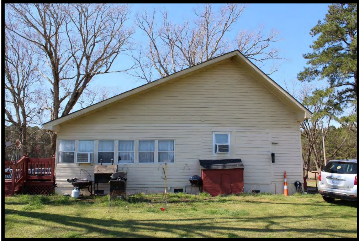
Figure 47: Giles Stephens Homeplace, Looking West.
