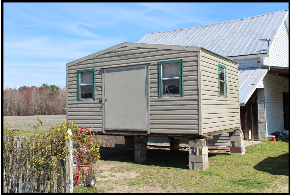
Figure 28: Maulsby and Susan Stephens House, Secondary Dwelling, Looking Northeast.
