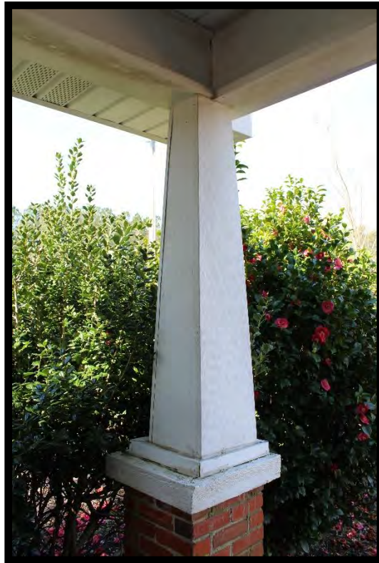
Figure 9: Maulsby and Susan Stephens House, Porch Column.
