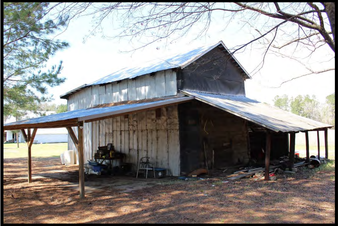
Figure 32: Maulsby and Susan Stephens House, Tobacco Barn, Looking Northwest.
