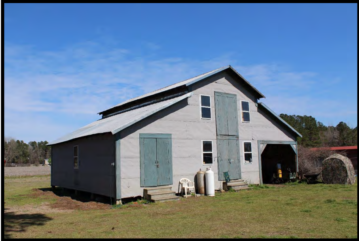
Figure 54: Giles Stephens Homeplace, Barn, Looking Northeast.
