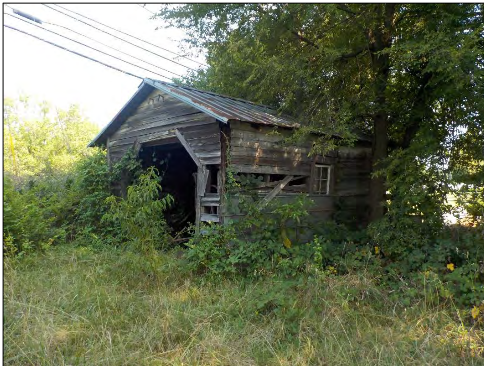
Figure 12. Garage, facing northwest.
