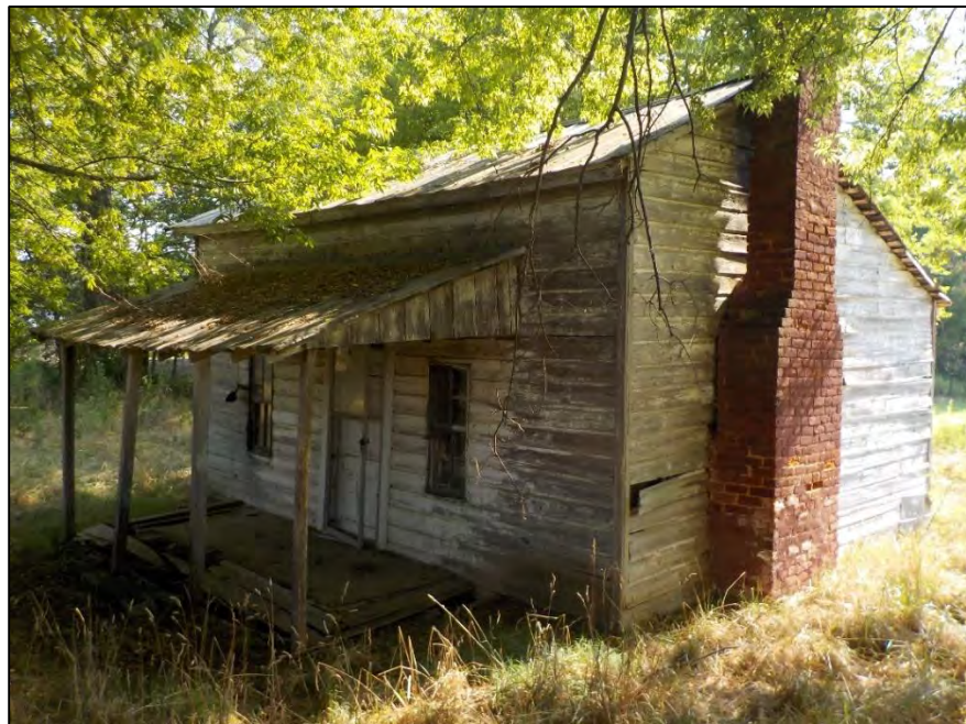
Figure 8. Resource No. MK2293, facing northeast.
