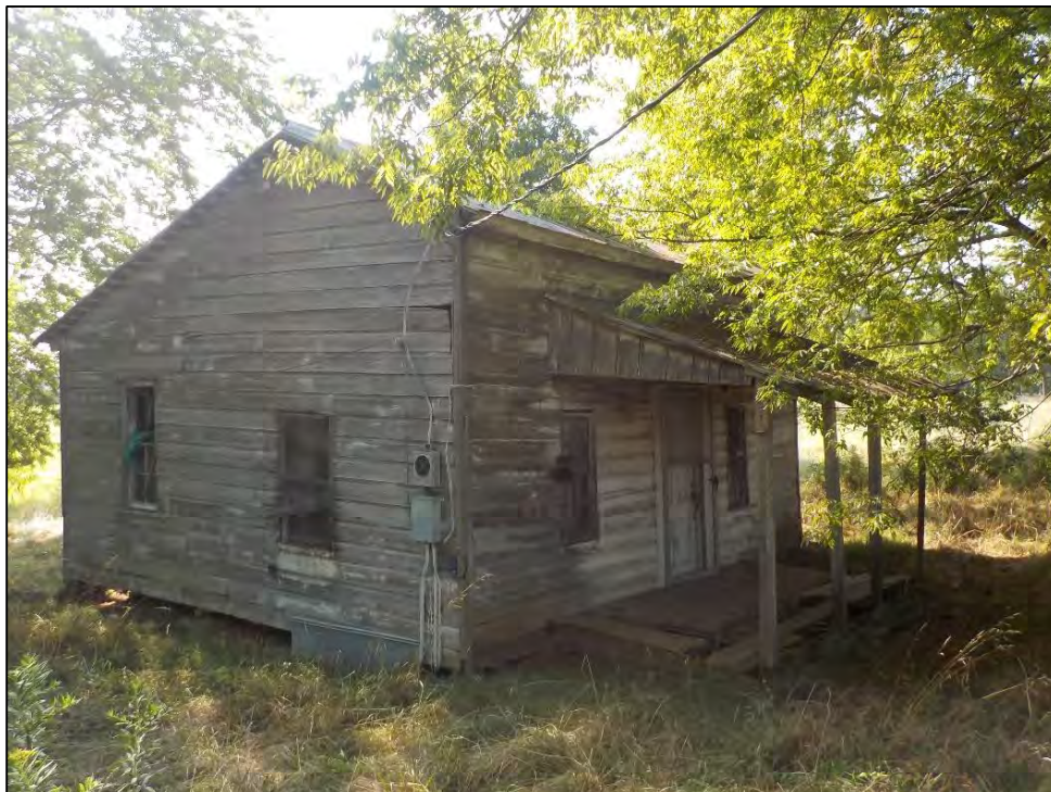
Figure 10. Resource No. MK2293, facing southeast.
