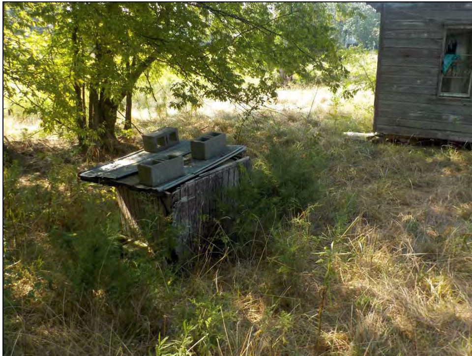
Figure 11. Wellhouse, facing southeast.
