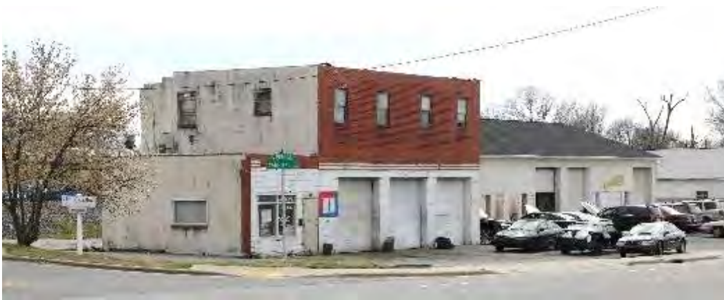
Figure 9. Front (north) facade and side (east) elevation of 2832 East Market Street, view facing southwest. Mead & Hunt photograph.
