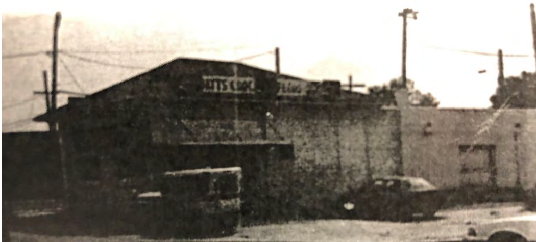
Figure 14. 1990 photograph of the Batts Grocery and Transfer Company building. Photograph from 1990 survey.
