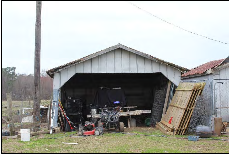
Figure 13. Garage, View Looking Northwest.
