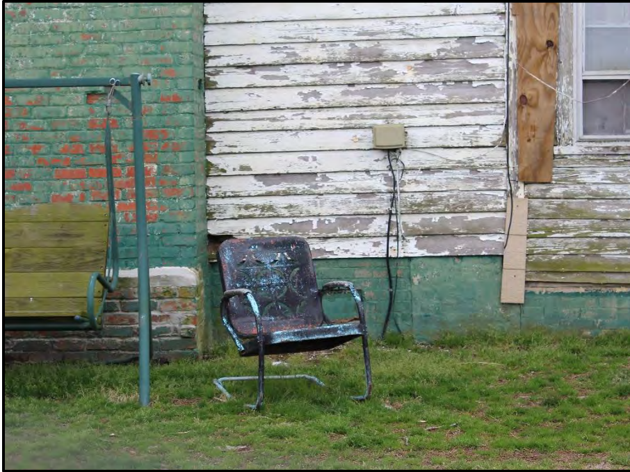
Figure 10. Detail of Foundation of Main Block and EII, Looking Southwest.
