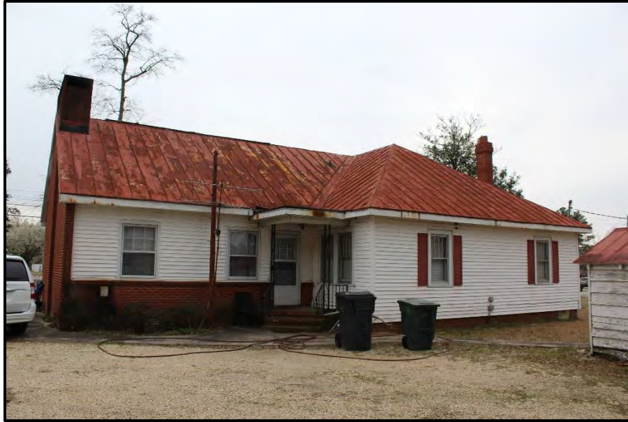
Figure 28. House, Looking Northwest.
