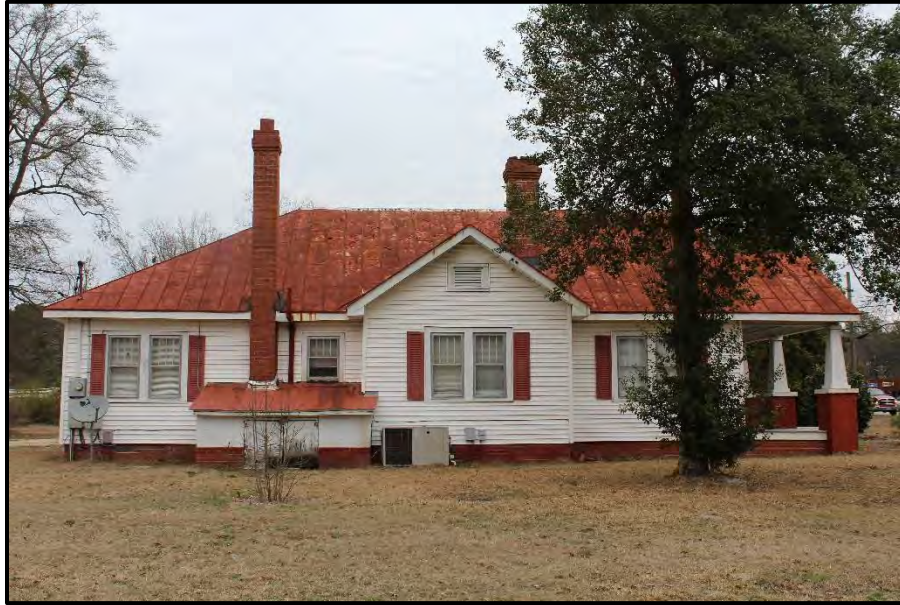
Figure 26. House, Looking South.
