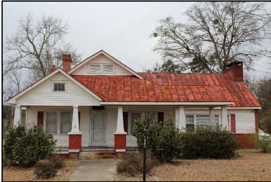
Figure 25. House, Looking Southeast.
