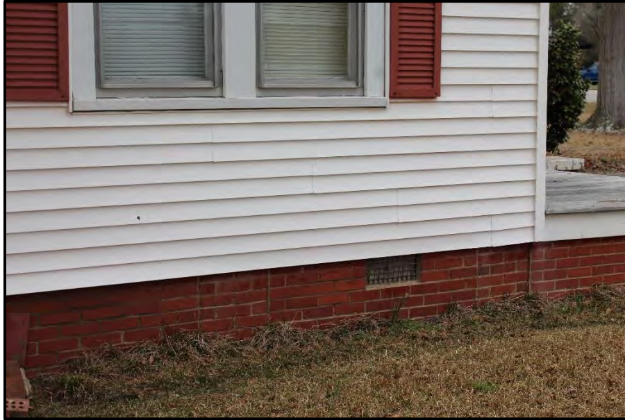
Figure 32. Detail of Foundation, Looking East.
