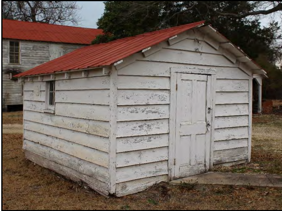
Figure 37. Shed, Looking North.
