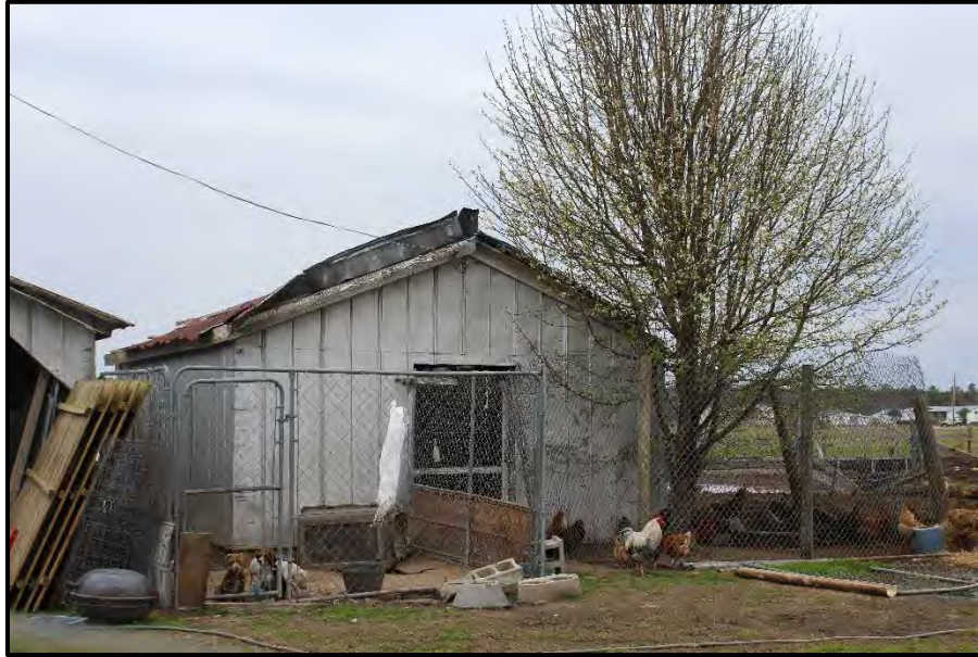
Figure 14. Workshop/Washhouse, View Looking Northwest.
