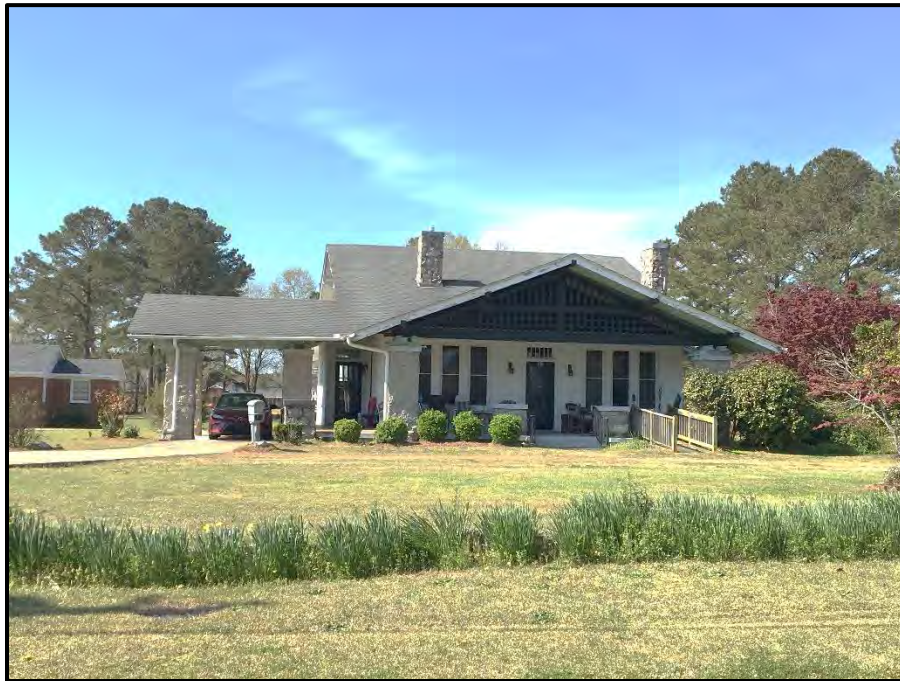
Figure 40. Thad Yelverton House (WY0769), 115 N. Church Street, Eureka, NC, Looking Southwest.
