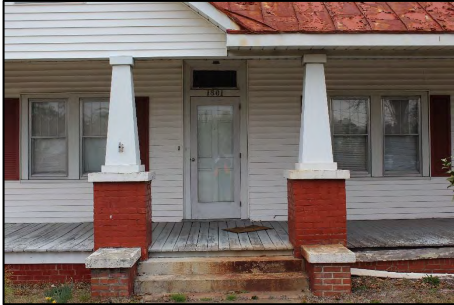
Figure 30. Detail of Porch and Front Entry Door, Looking Northwest.
