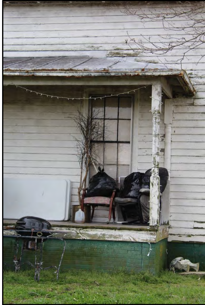
Figure 9. Detail of Front Porch, Looking Northwest.
