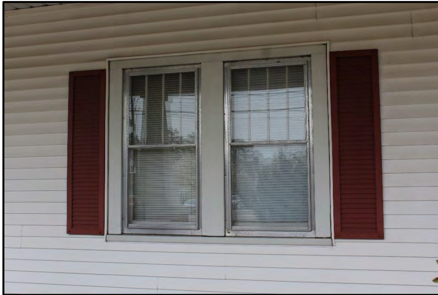
Figure 33. Detail of Paired Window on Façade, Looking West.
