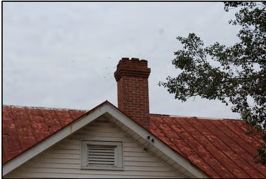
Figure 31. Detail of Chimney, Looking Northeast.
