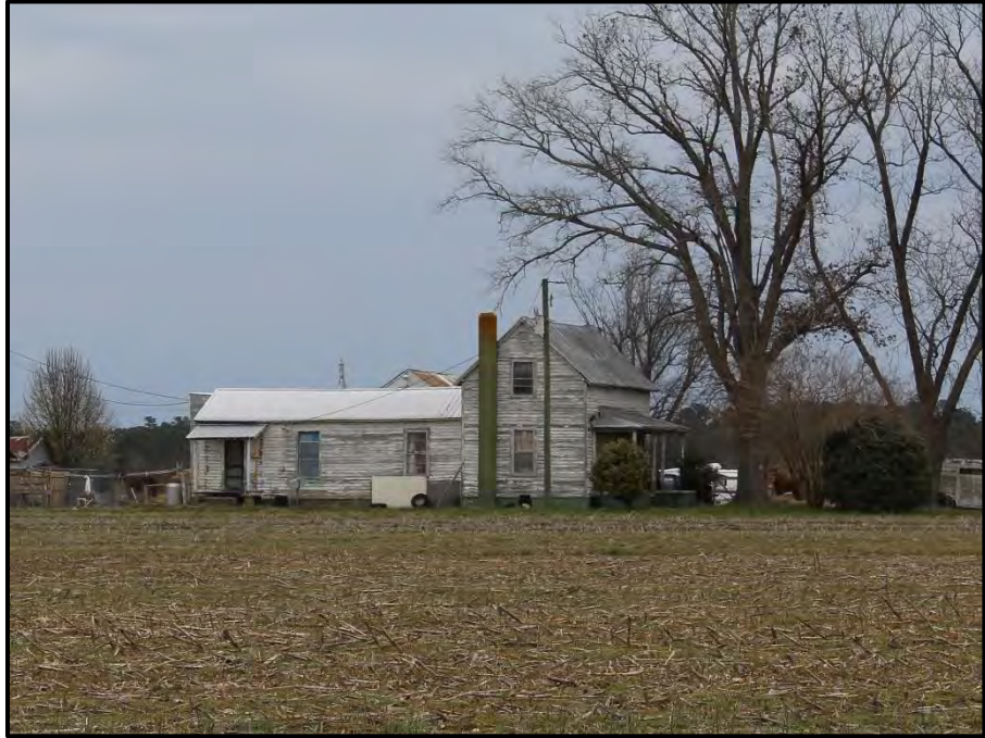
Figure 5. Anderson House, Looking Northeast.
