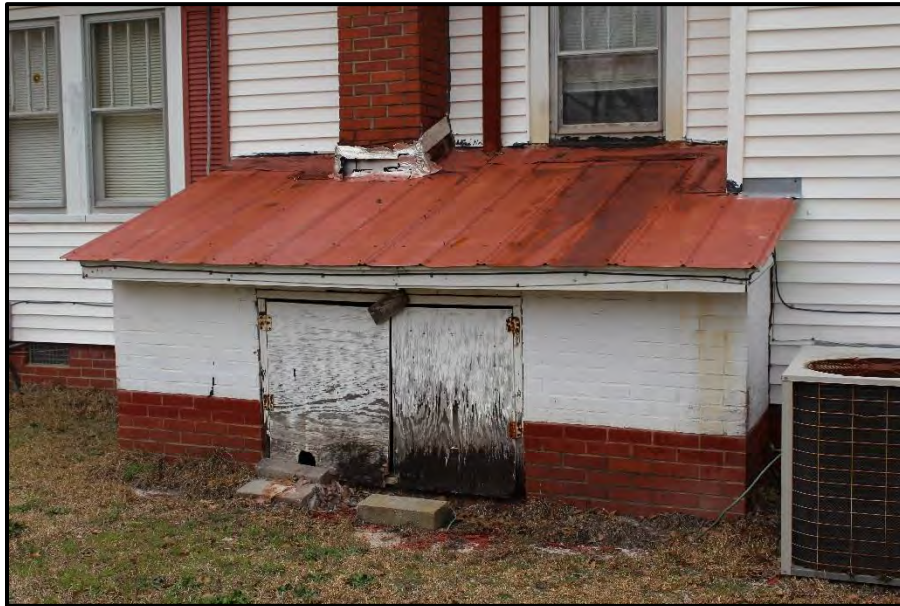
Figure 29. Detail of Bulkhead, Looking North.
