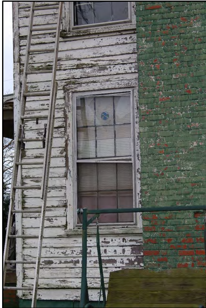
Figure 11. Detail of Window on Southeastern Gable End, Looking Southwest.
