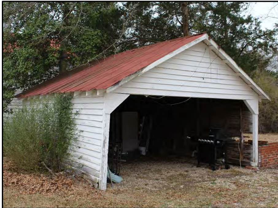
Figure 36. Garage, Looking North.
