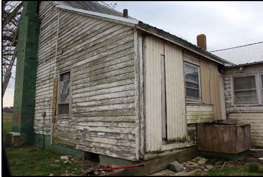
Figure 7. Anderson House Shed-Roofed Ell, Looking South.
