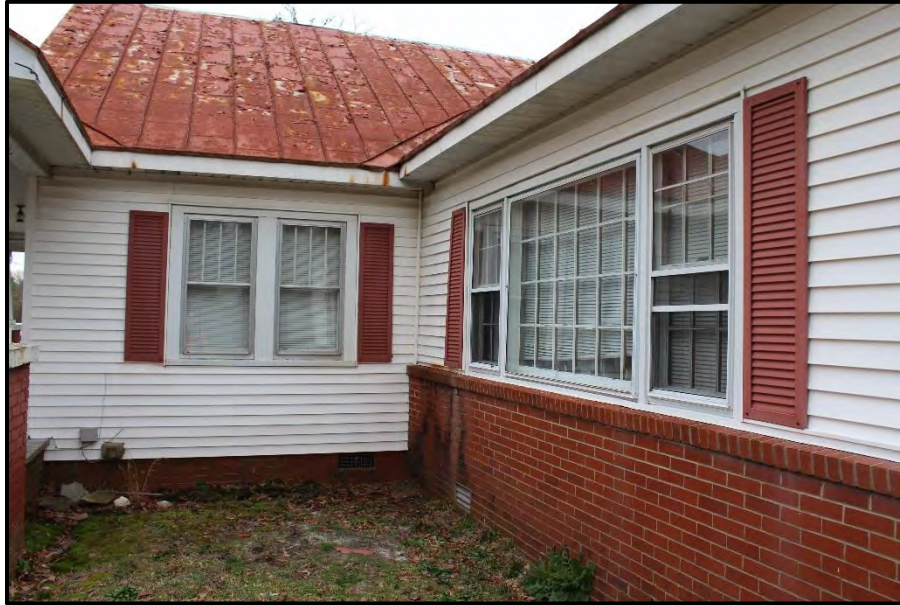
Figure 34. Detail of Windows on Southeast Elevation and Ell, Looking West.
