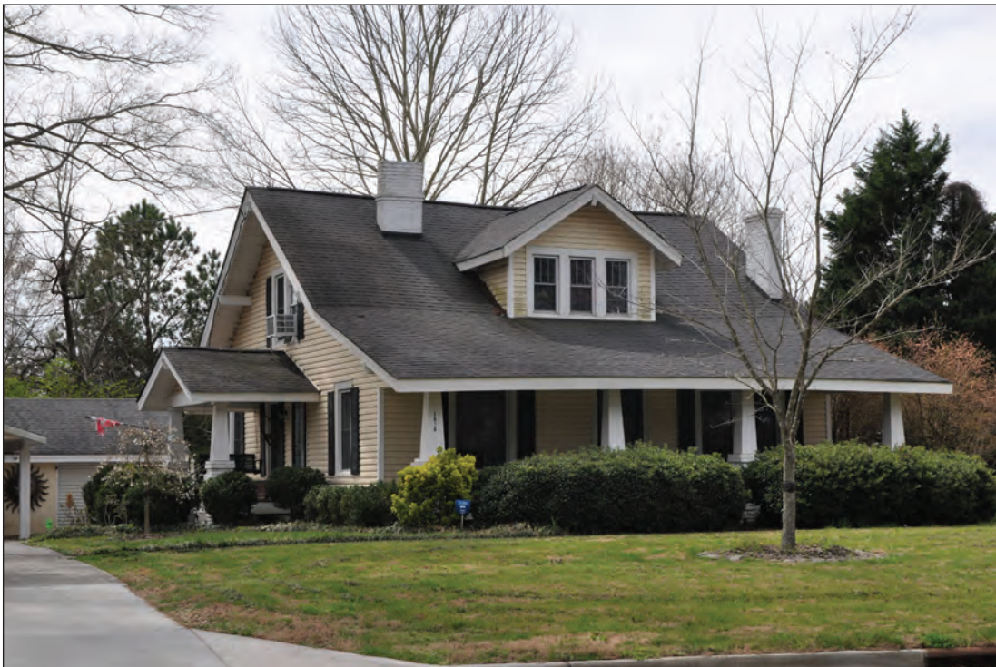
Figure 3.1. Paxton-Price House, Façade and East Elevation, Looking Southwest
