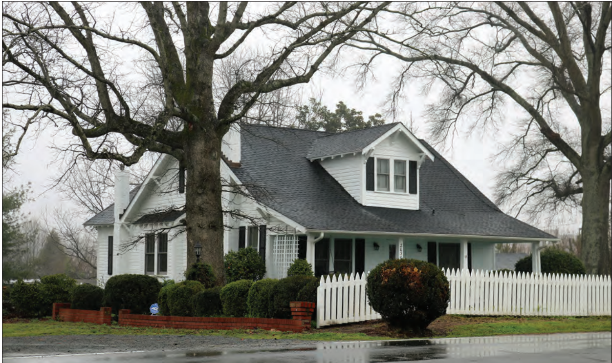
Figure 3.11 Photograph of MK3401 at 2030 McKee Road, circa 2015, Looking Northeast
