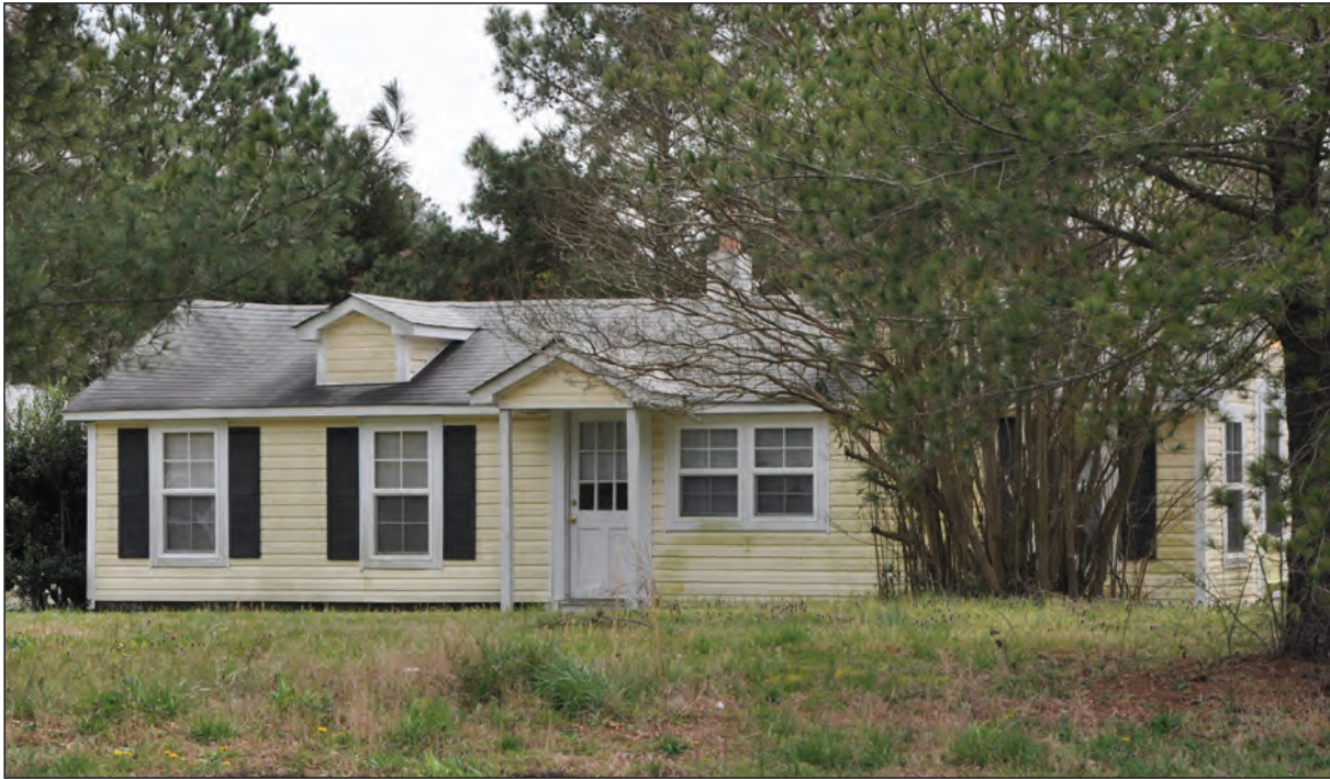
Figure 3.6. Secondary Dwelling, Façade, Looking Southeast
