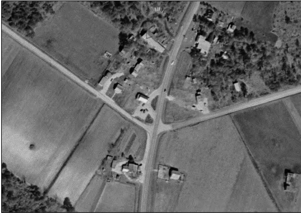
Figure 4.18. USGS aerial photograph (1957) showing structure BF2510 and outbuildings.
