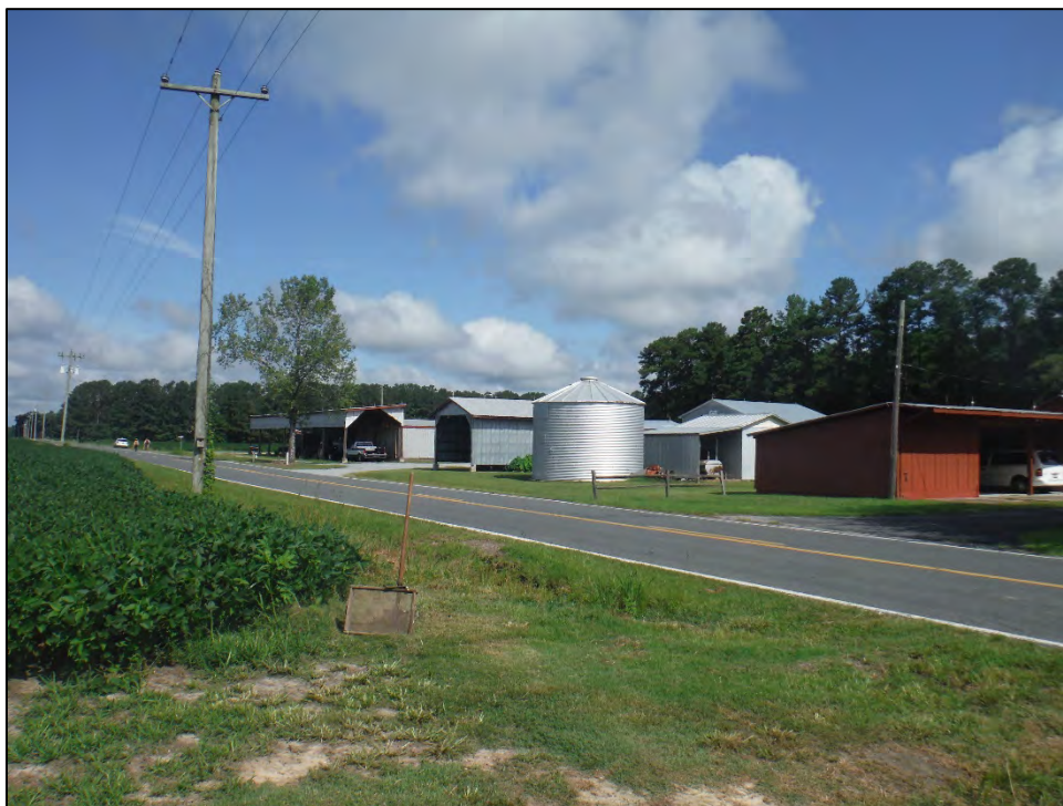
Figure 4.17. Structure BF2510, outbuildings, facing northwest
