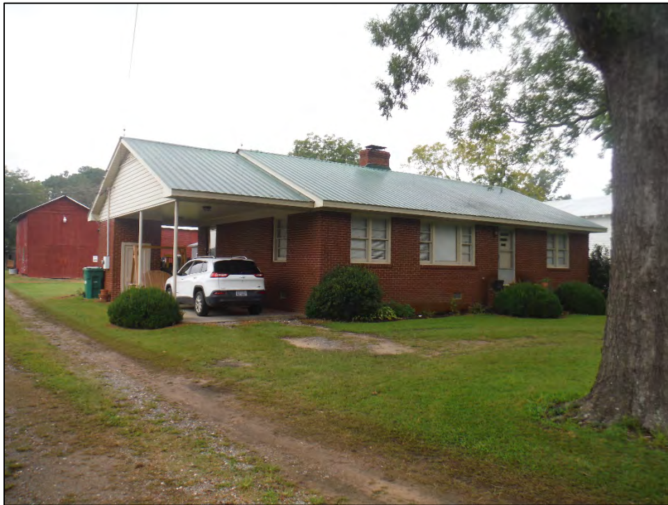
Figure 4.11. Structure MT1223, facing northwest.
