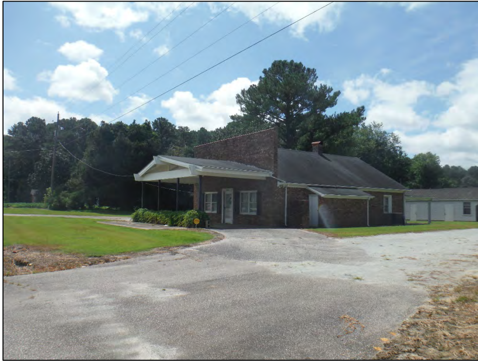
Figure 4.22. House (BF1618), facing south.
