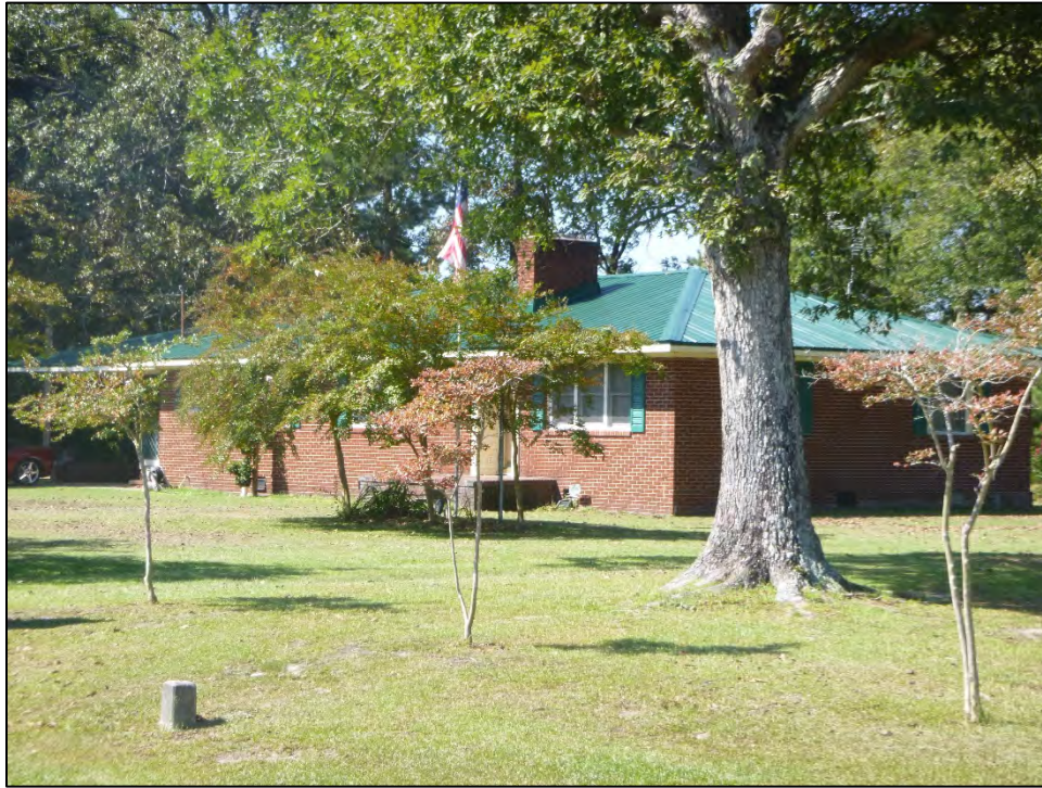
Figure 4.5. Structure MT1221, facing southwest.
