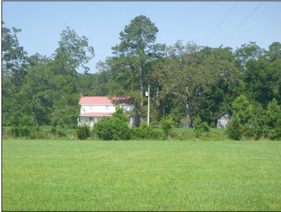
Figure 4.14. Ward House (MT1037), facing southwest.
