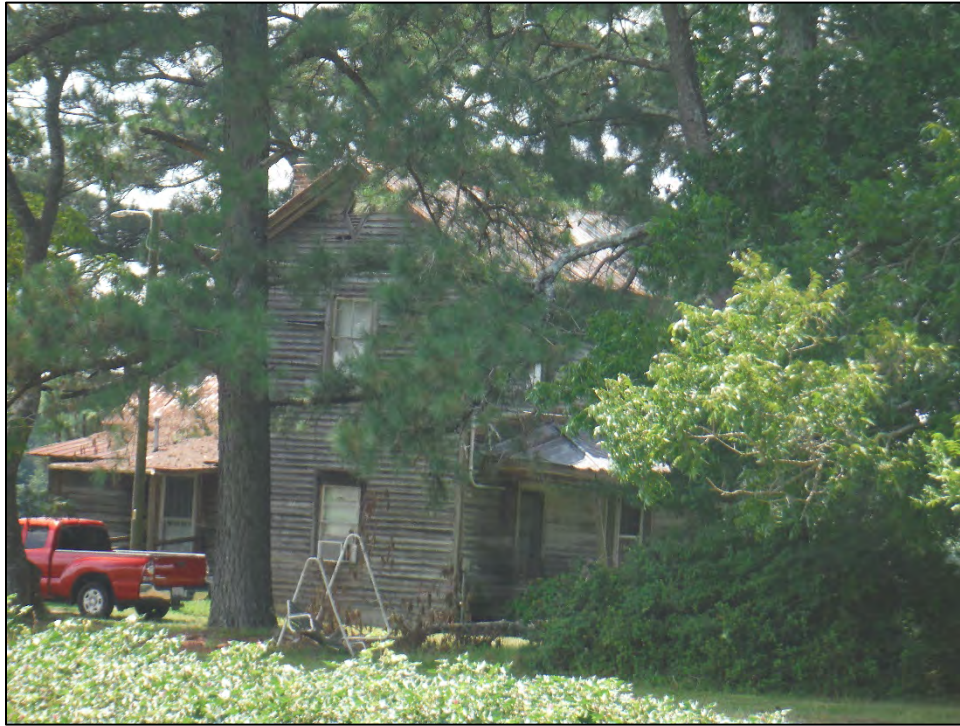
Figure 4.3. Structure MT1212, facing southwest.
