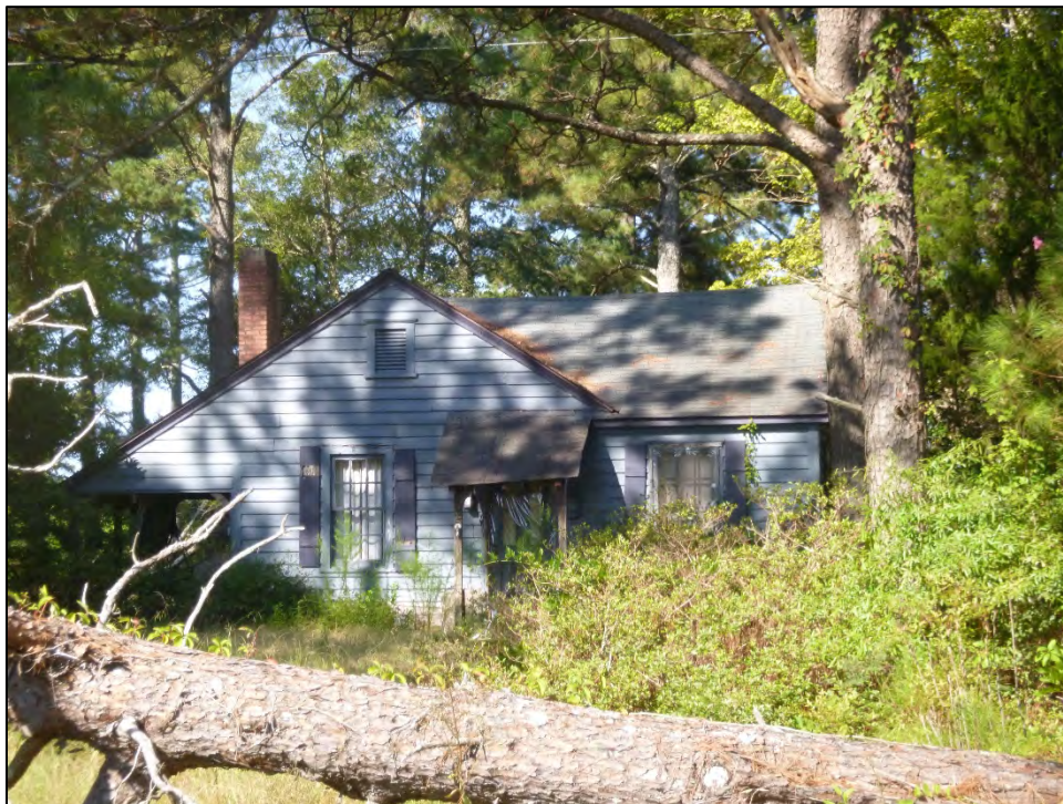
Figure 4.26. Structure BF2511, facing west.
