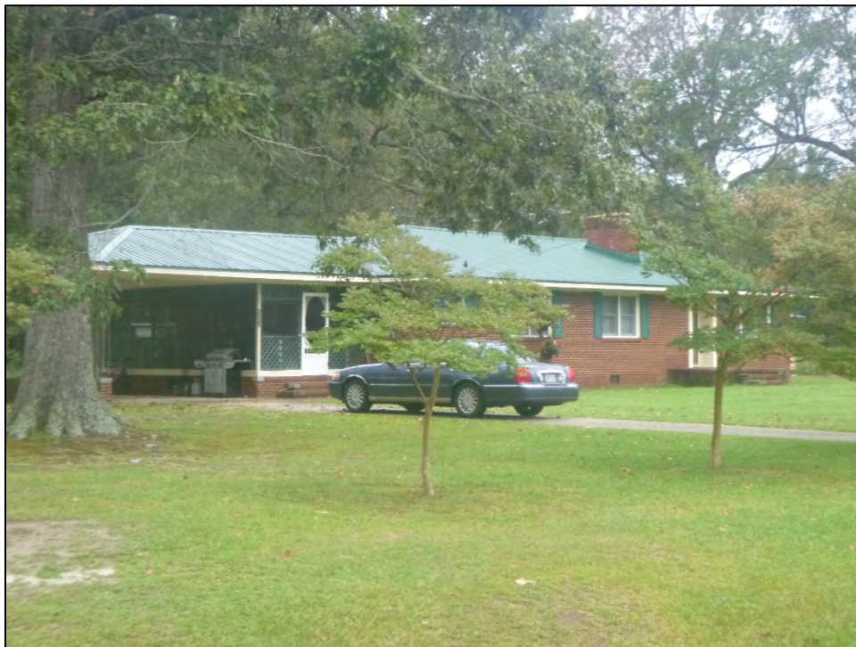
Figure 4.6. Structure MT1221, facing northwest.
