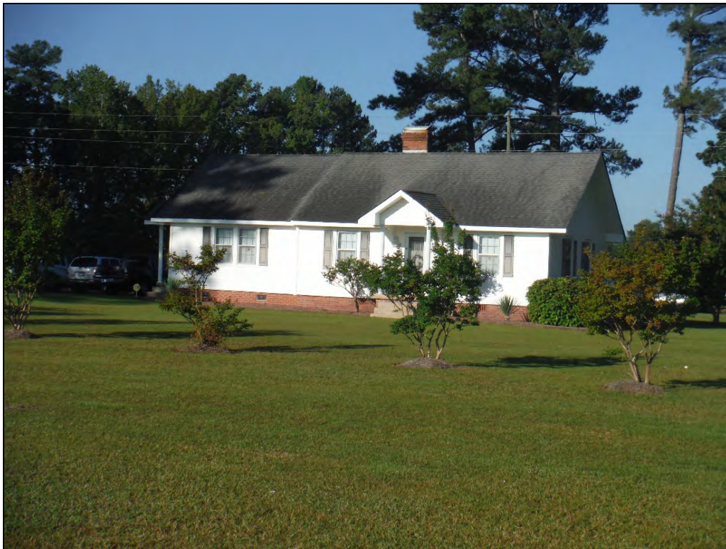
Figure 4.24. House (BF1613), facing west.
