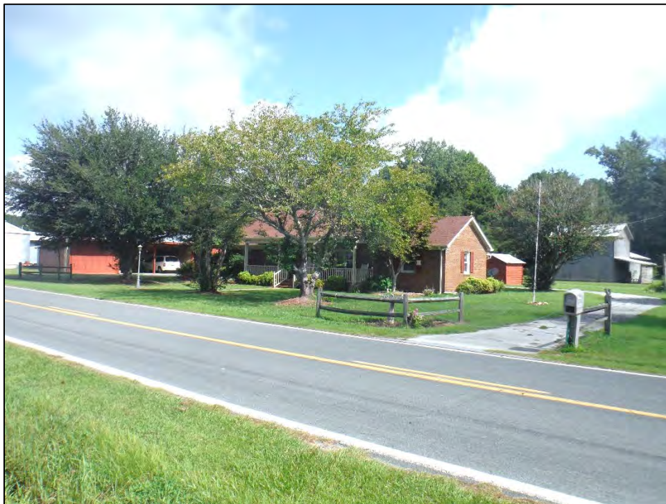
Figure 4.15. Structure BF2510, house, facing northwest.
