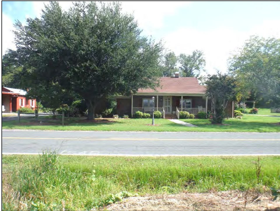
Figure 4.16. Structure BF2510, house, facing north.
