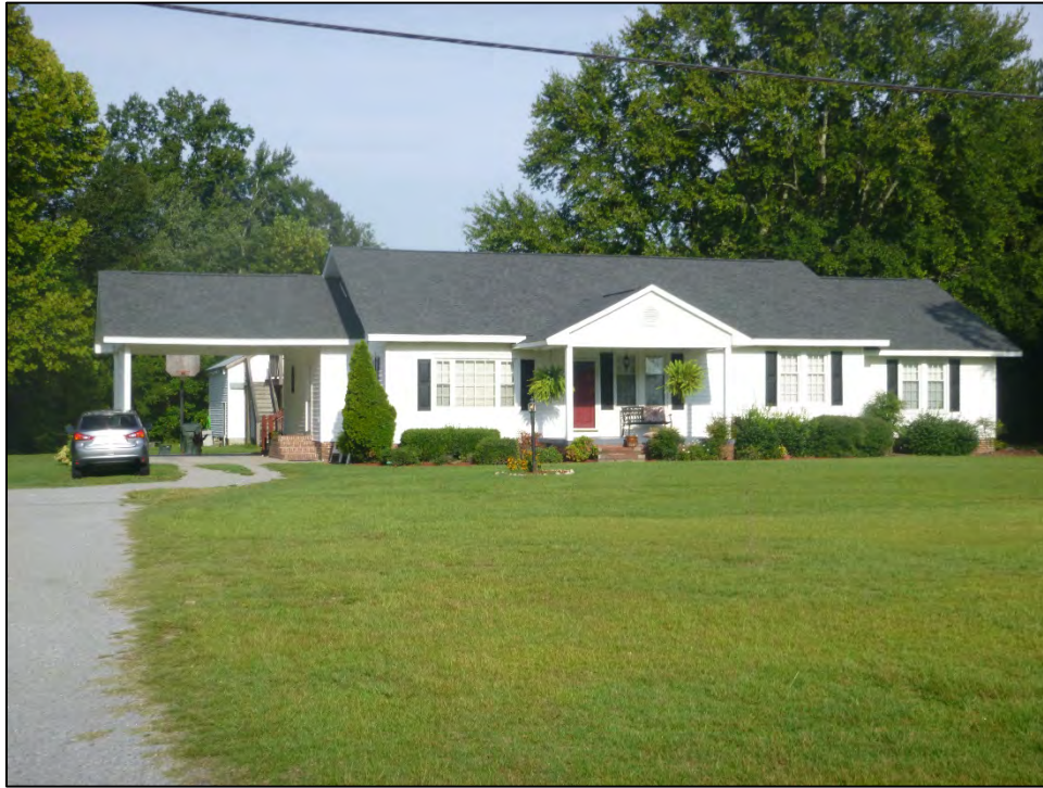
Figure 4.1. Structure MT1225, facing northwest.
