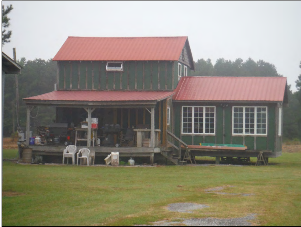
Figure 4.12. Structure MT1224, facing west.
