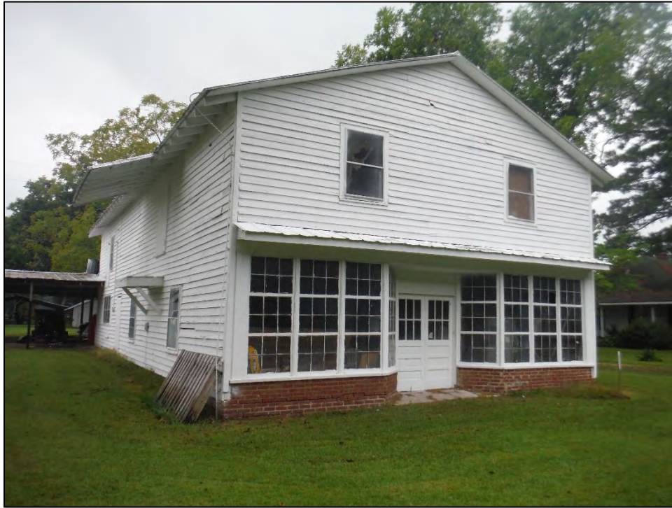
Figure 4.9. Griffin's Hatchery (MT0298), facing northwest.
