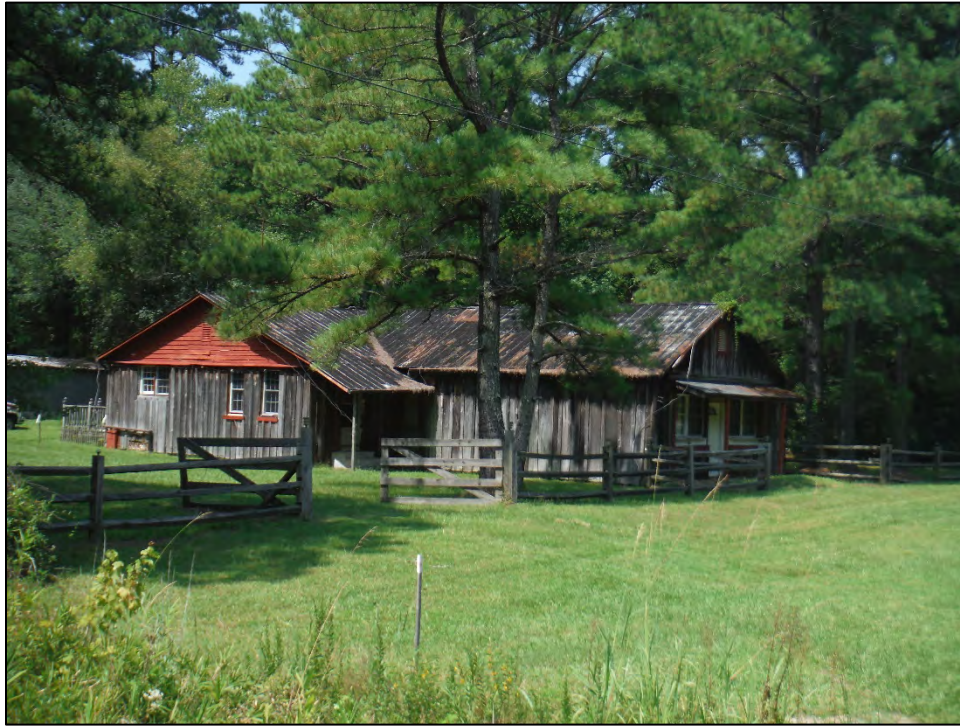
Figure 4.7. Structure MT1222, facing northwest.
