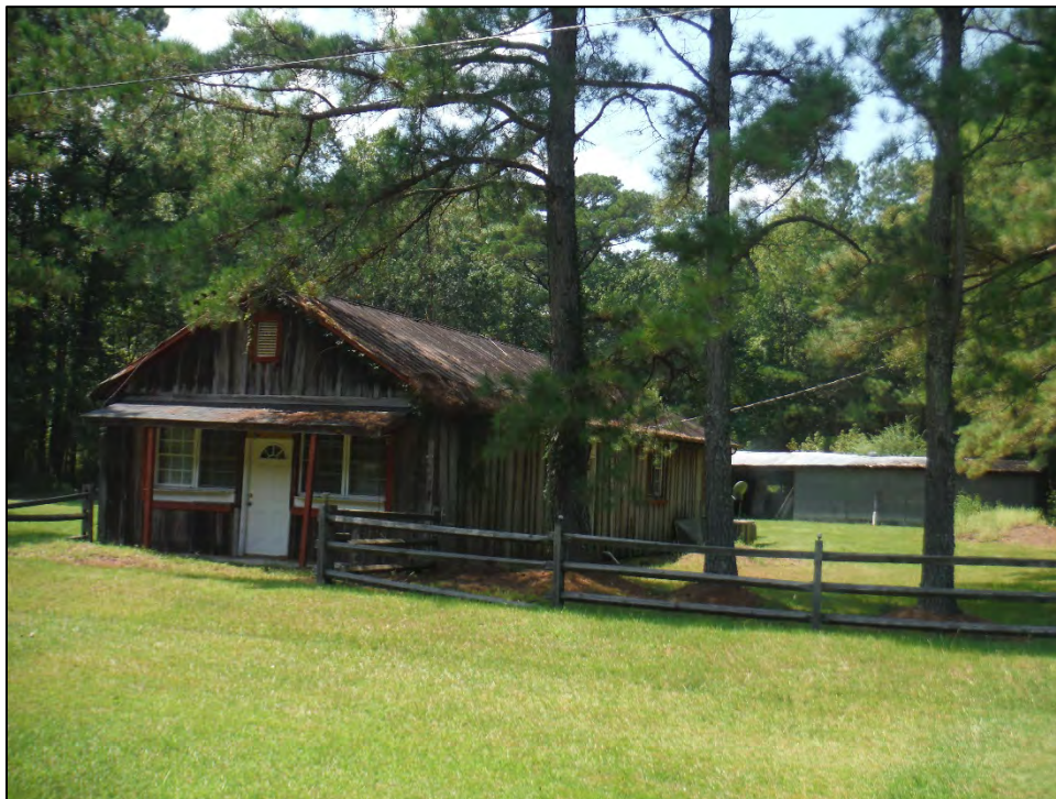
Figure 4.8. Structure MT1222, facing southwest.
