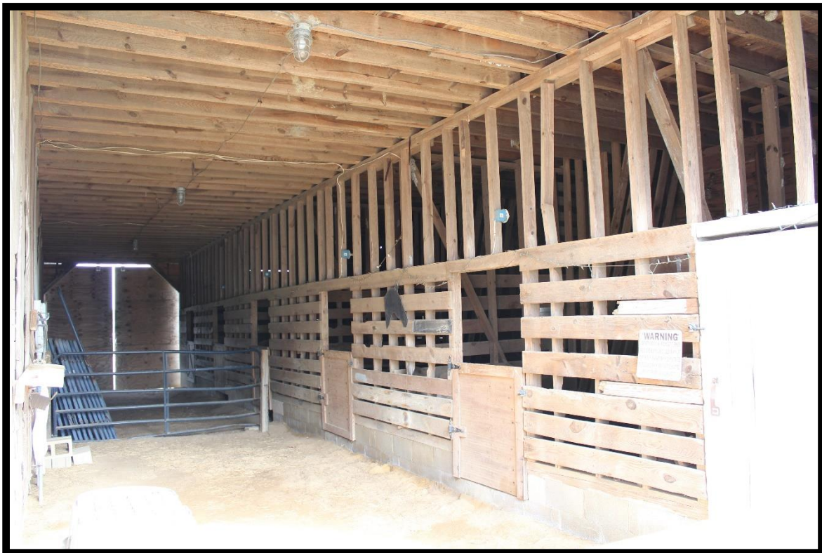
Figure 19: Embro Bass Farm, Interior Horse Barn, Looking East.
