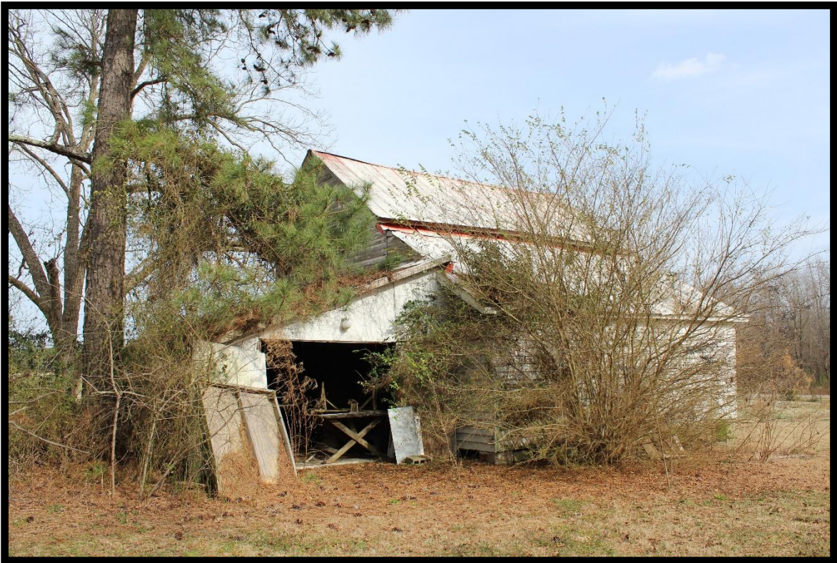
Figure 17: Embro Bass Farm, Barn, Looking East-Northeast.
