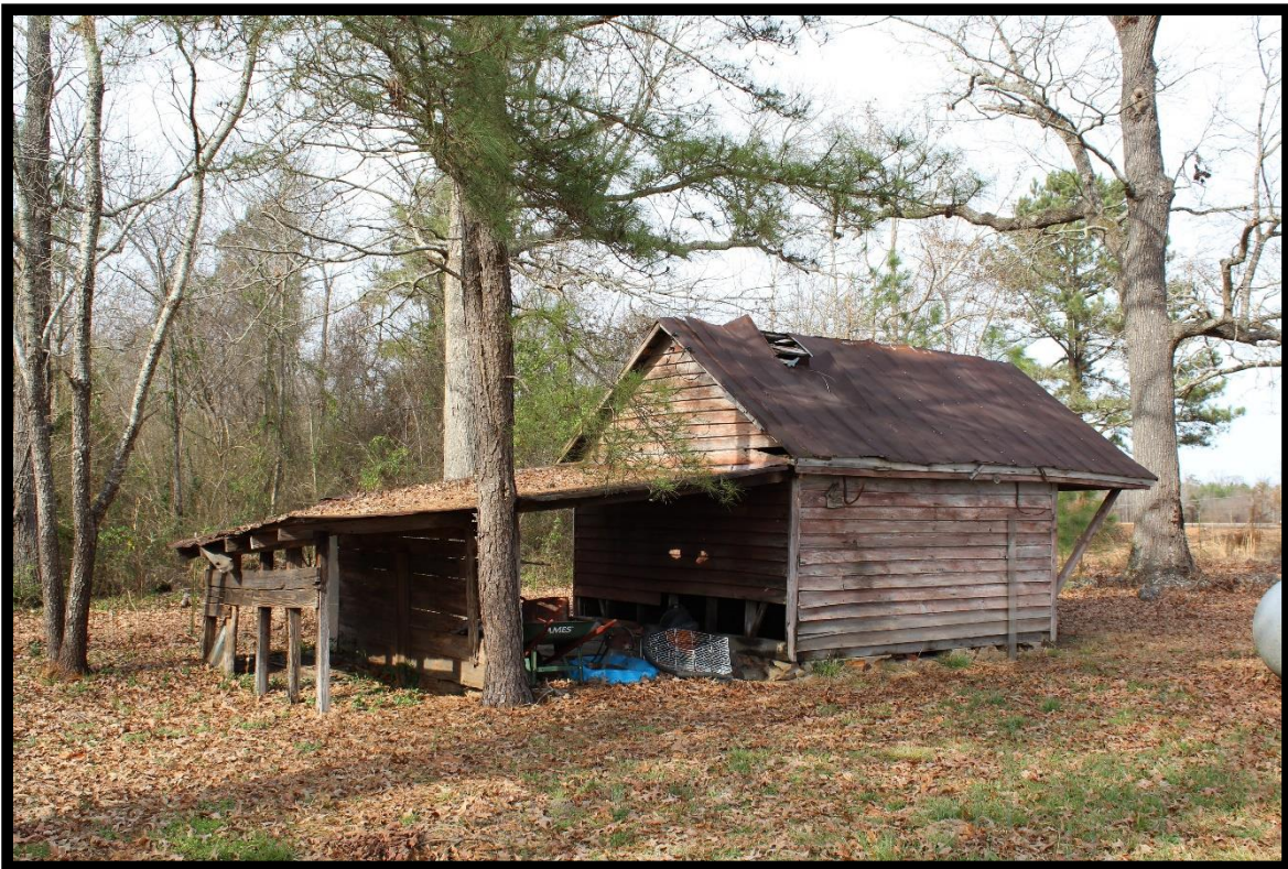
Figure 13: Embro Bass Farm, Ancillary Structure, Looking North.
