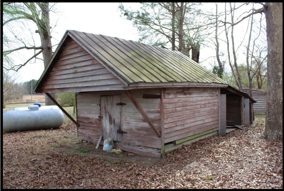
Figure 12: Embro Bass Farm, Ancillary Structure, Looking South.
