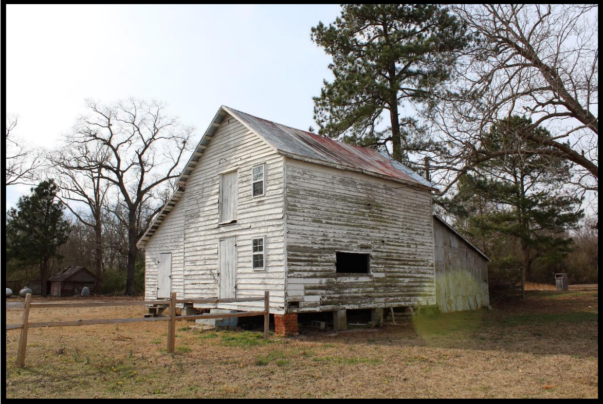
Figure 16: Embro Bass Farm, Barn, Looking West.
