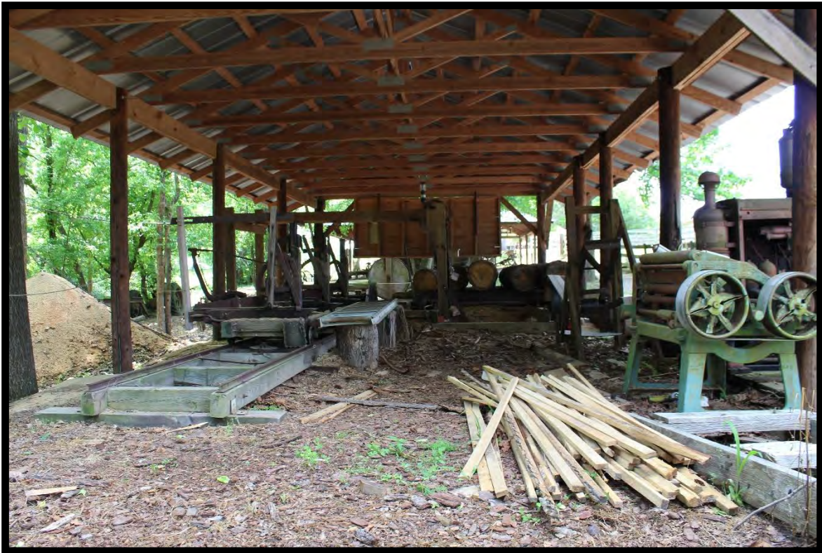
Figure 30: William John Gillis Farmstead, Saw Mill, Interior Setup, Looking West.
