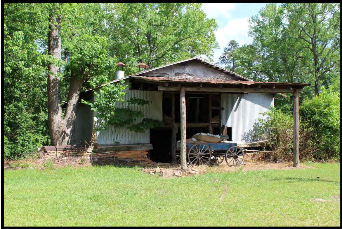
Figure 100: Gillis Cotton Gin No. 2, Looking Northeast.
