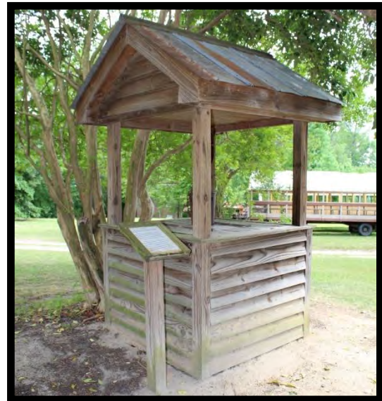
Figure 17: William John Gillis Farmstead, Modern Well, Looking Southwest.
