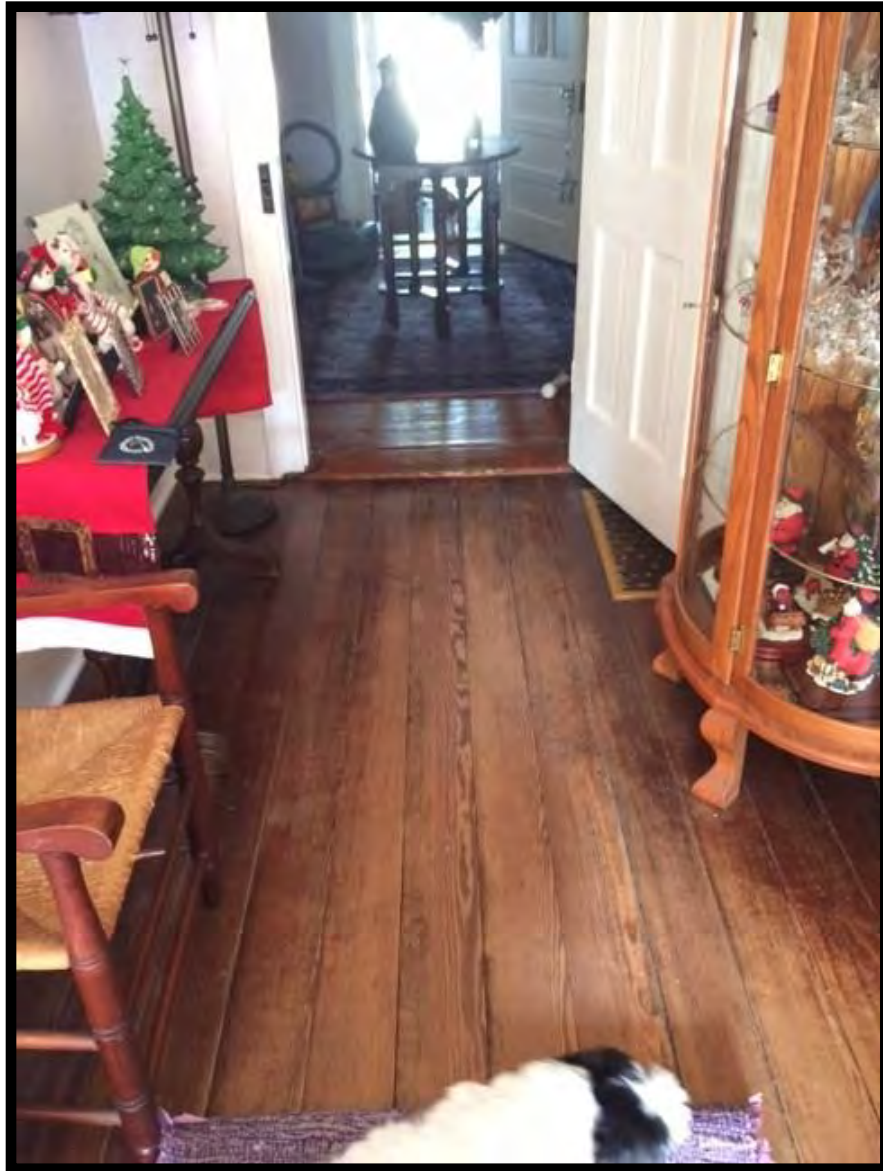
Figure 63: McInnis House, Central Hall, Floorboard Detail, Looking Northeast (Neill McInnis, 2019).
