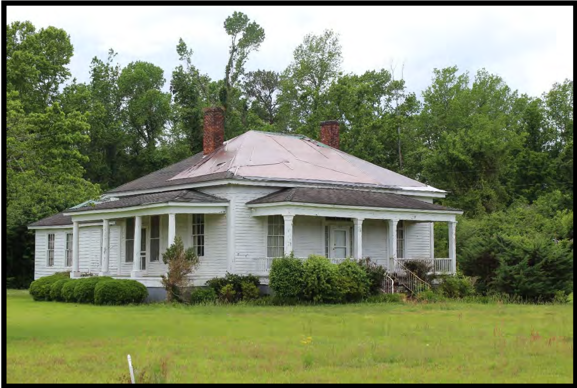
Figure 80: Robeson-Stevens House (BL0233), Looking Northwest.
