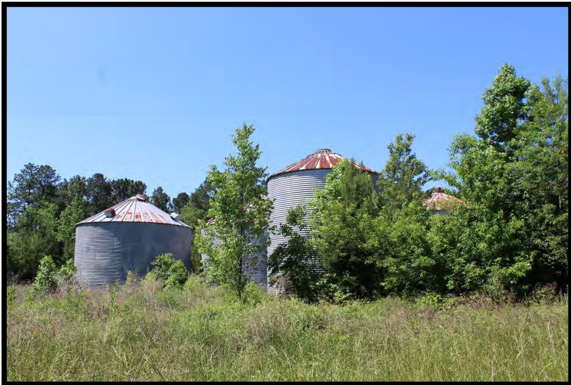
Figure 88: Gillis Cotton Gin, Metal Storage Bins, Looking Northwest.
