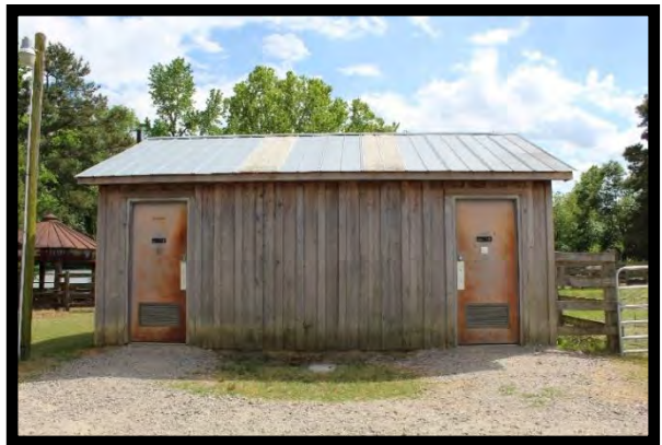
Figure 21: William John Gillis Farmstead, Modern Toilets, Looking South.
