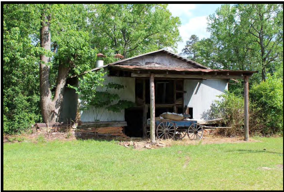
Figure 37: Gillis Cotton Gin No. 2, Looking Northeast.
