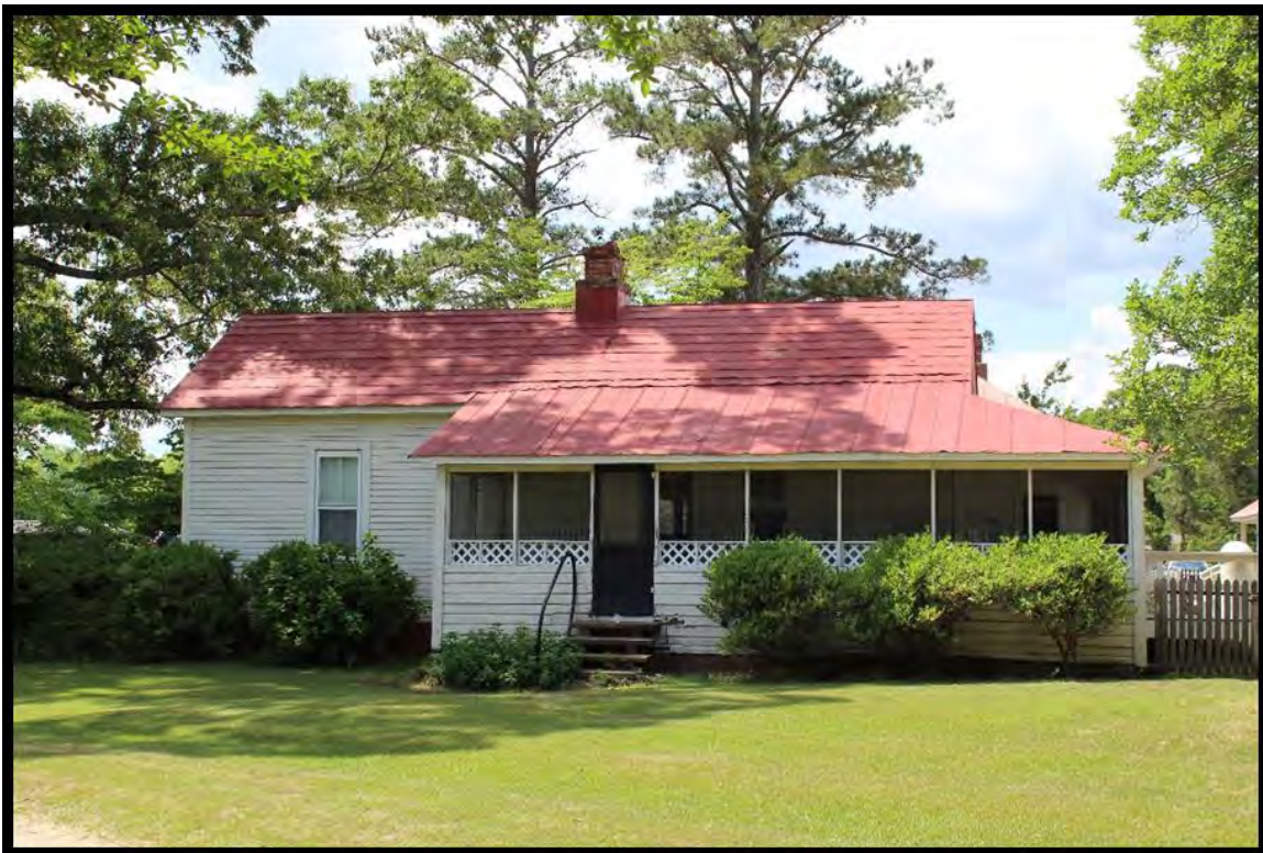
Figure 8: William John Gillis Farmstead, Dwelling, Looking Northwest.
