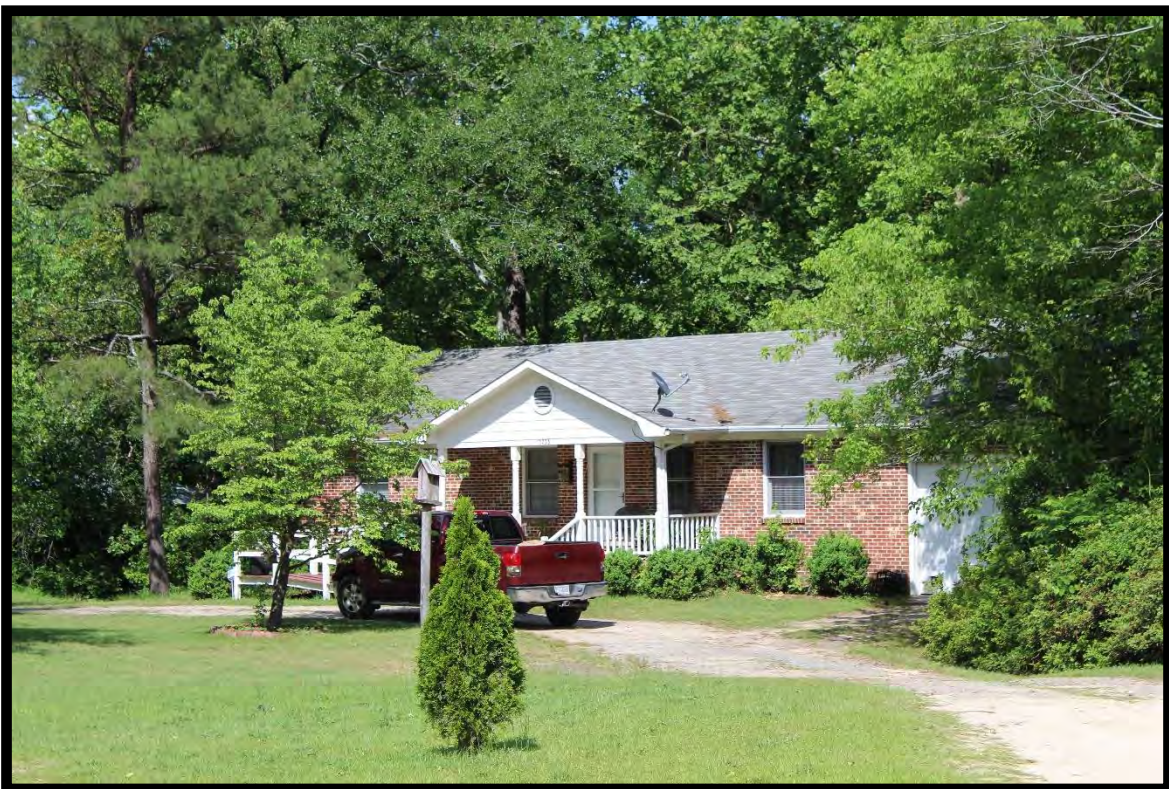
Figure 36: William John Gillis Farmstead, Modern Dwelling, Looking Northeast.
