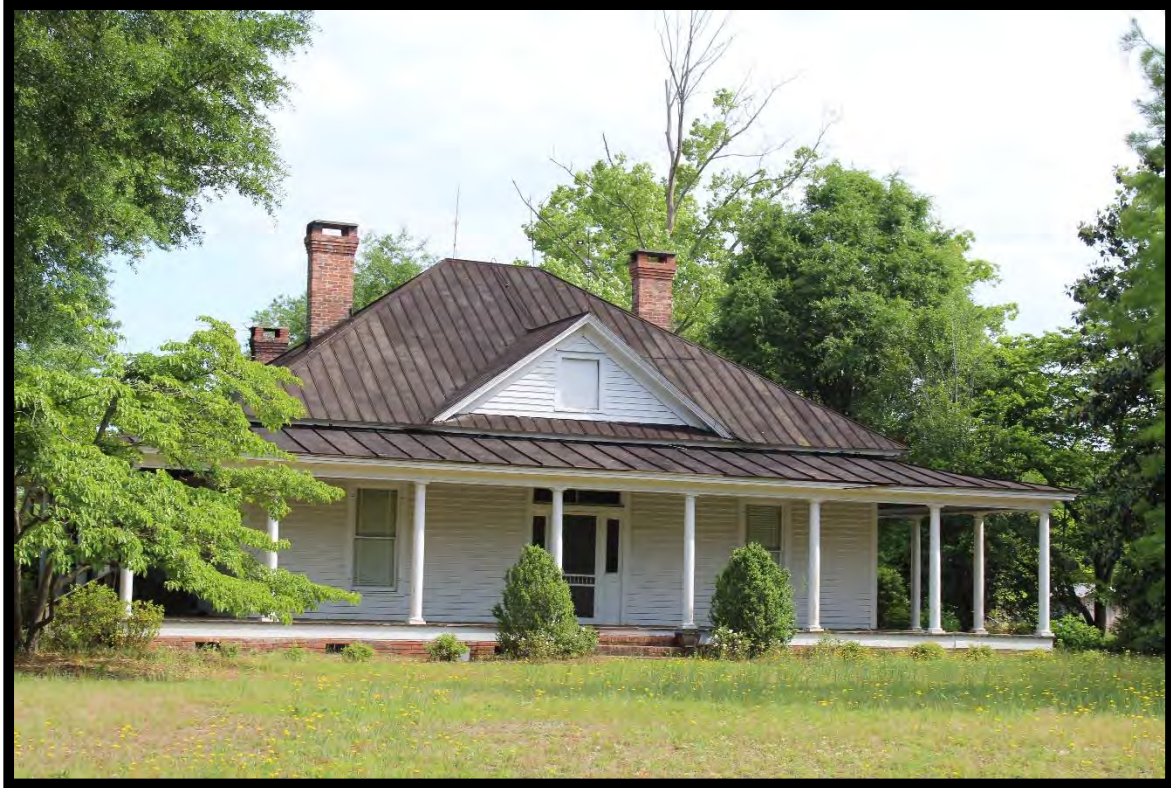
Figure 81: James L. Cooley House (SC0039), Looking Northeast.
