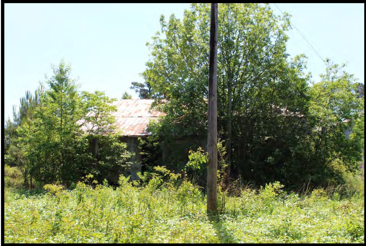
Figure 87: Gillis Cotton Gin, Gin Stand Shelter, Looking Southeast.
