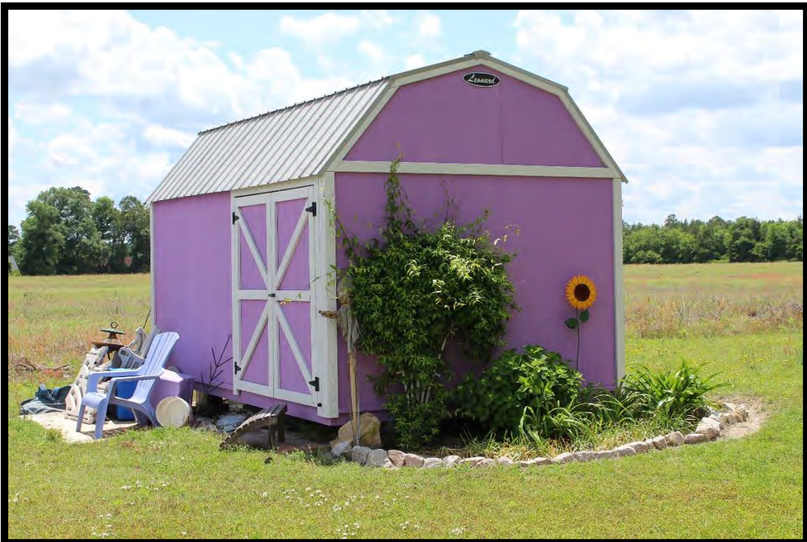
Figure 70: McInnis House, Gambrel-Roofed Modern Storage Shed, Looking Southwest.
