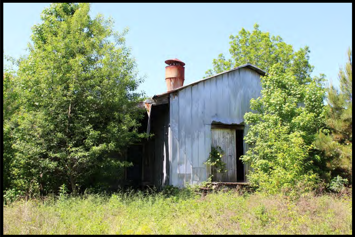
Figure 83: Gillis Cotton Gin, Structure, Looking Southwest.
