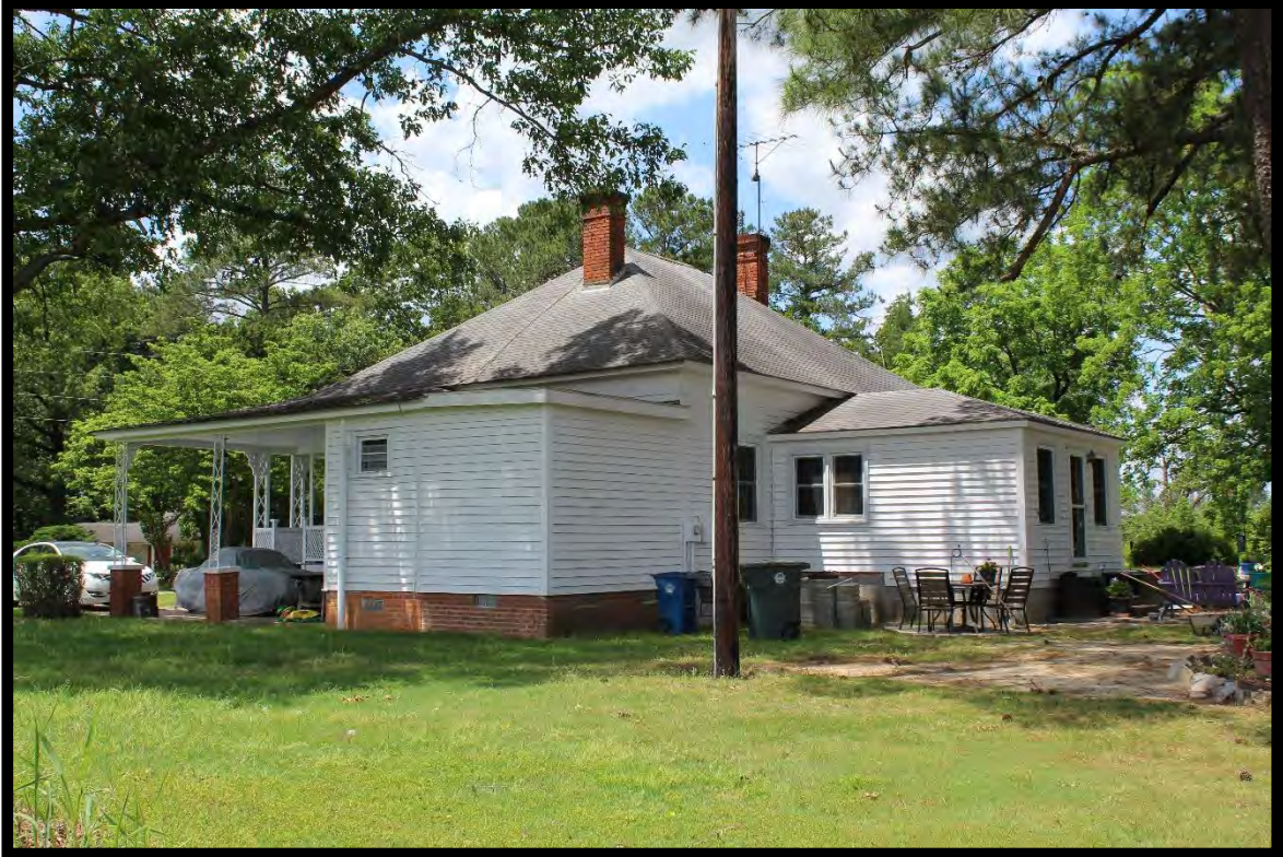
Figure 61: McInnis House, Looking Northwest.
