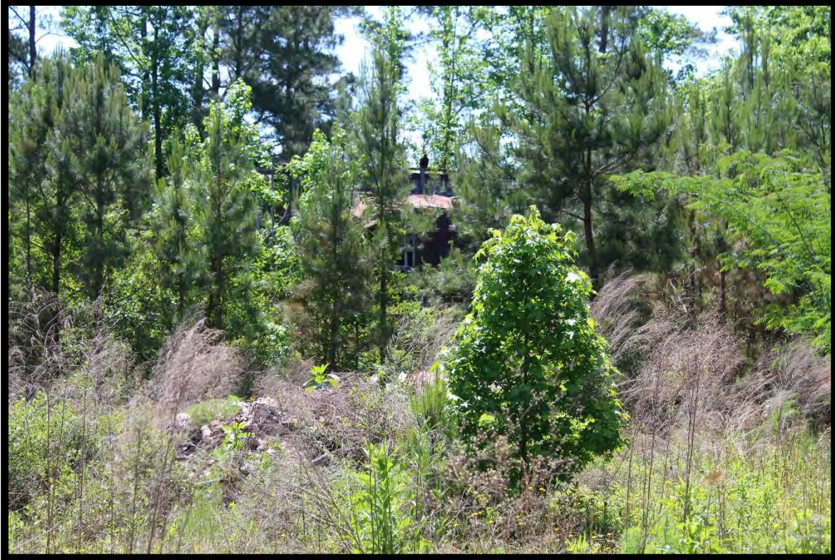
Figure 93: Gillis Cotton Gin, Partial View of Inaccessible Structure, Looking South.
