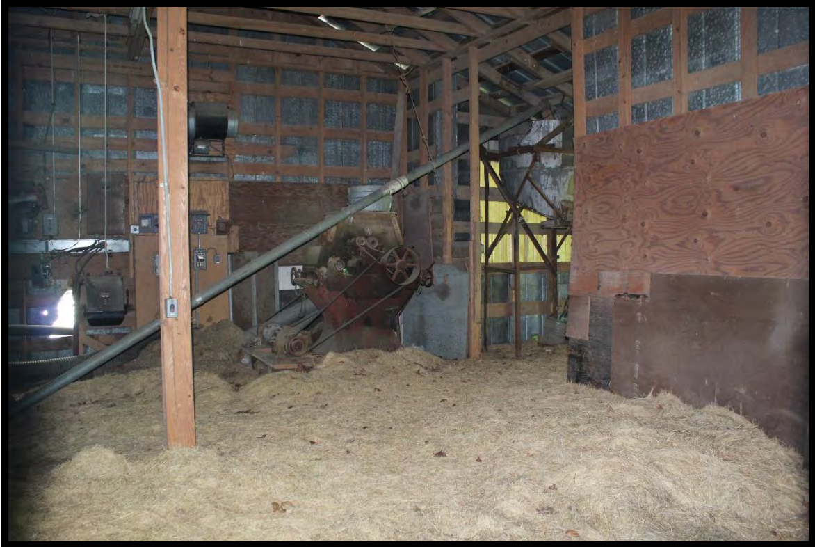
Figure 90: Gillis Cotton Gin, Interior Main Room and Machinery, Looking West.
