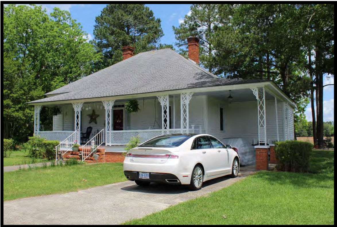
Figure 62: McInnis House, Looking Northeast.
