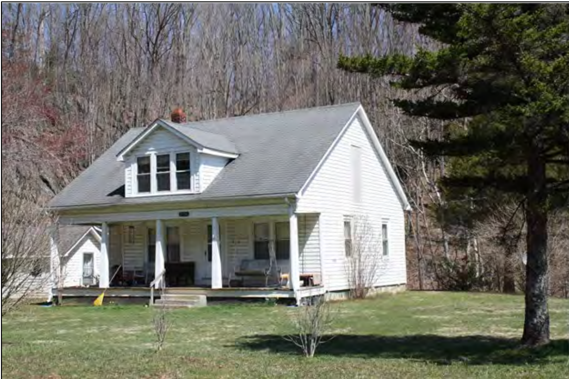
Figure 17: Bungalow, ca. 1930, 2556 NC HWY 88, W. Jefferson
