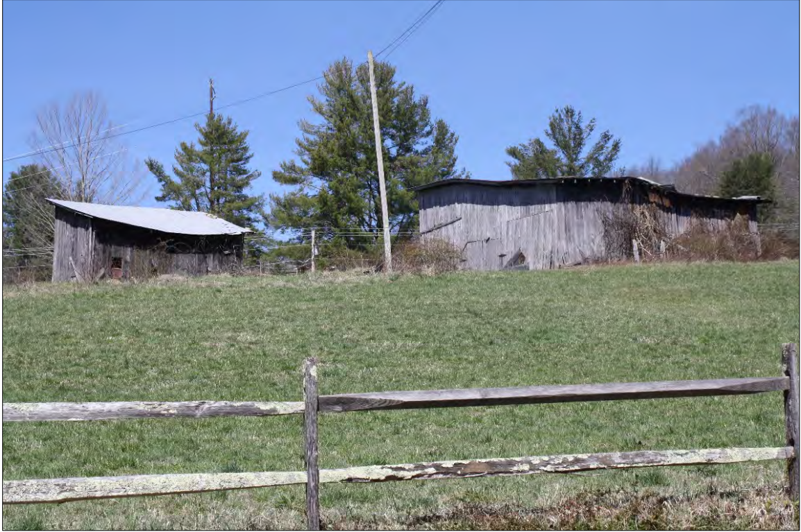
Figure 10: Two original outbuildings, now on adjacent subdivided parcel, looking southwest
