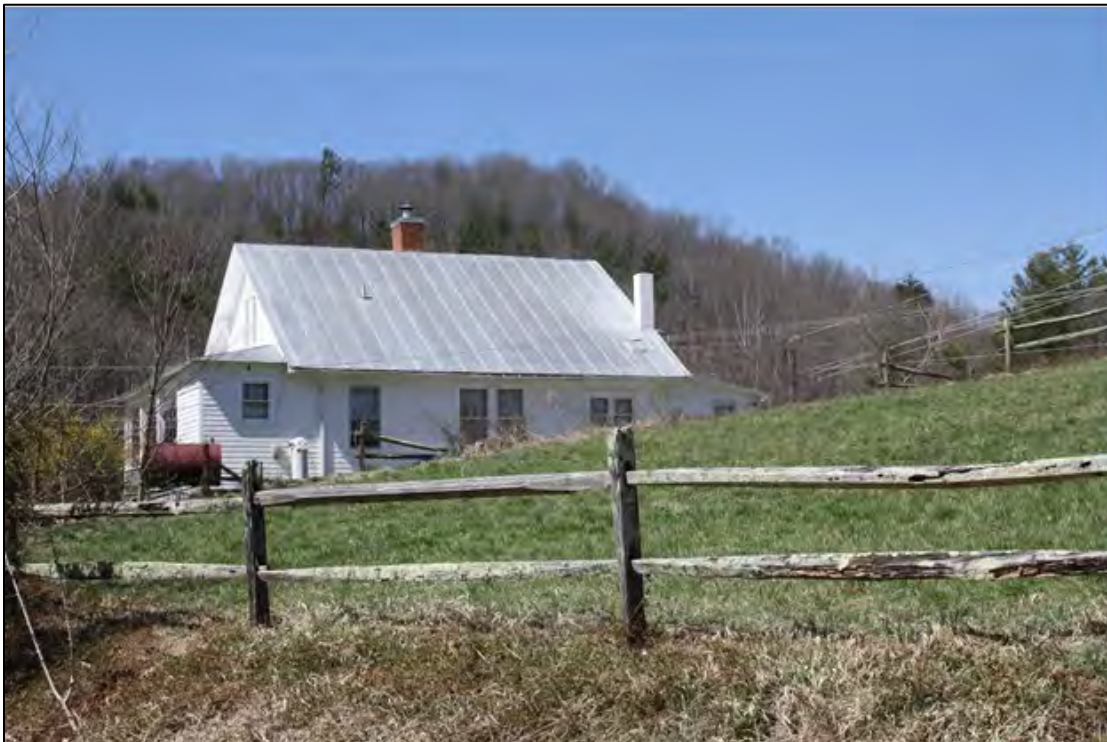
Figure 6: North (rear) elevation
