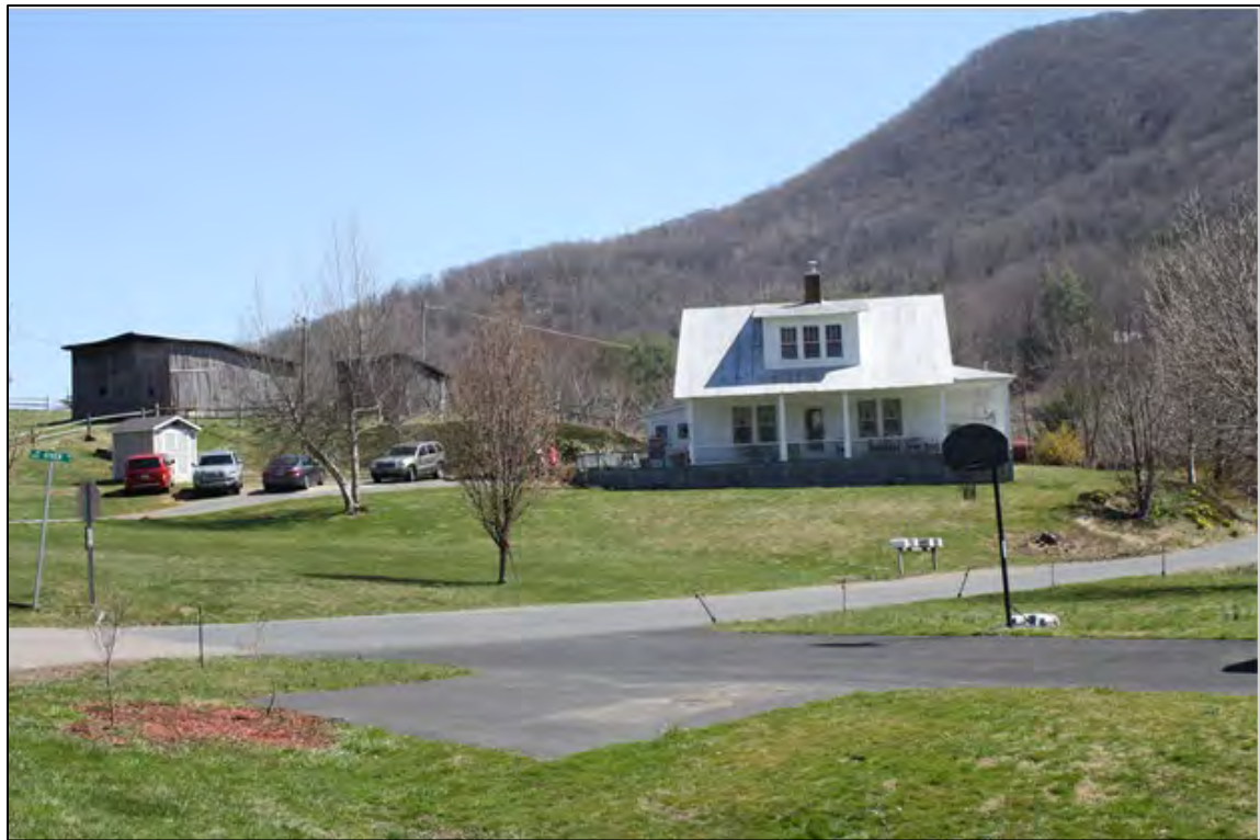
Figure 2: Looking northeast. Two original barns historically associated with the property to the northwest behind the house are extant, though now located on a subdivided adjacent parcel.
