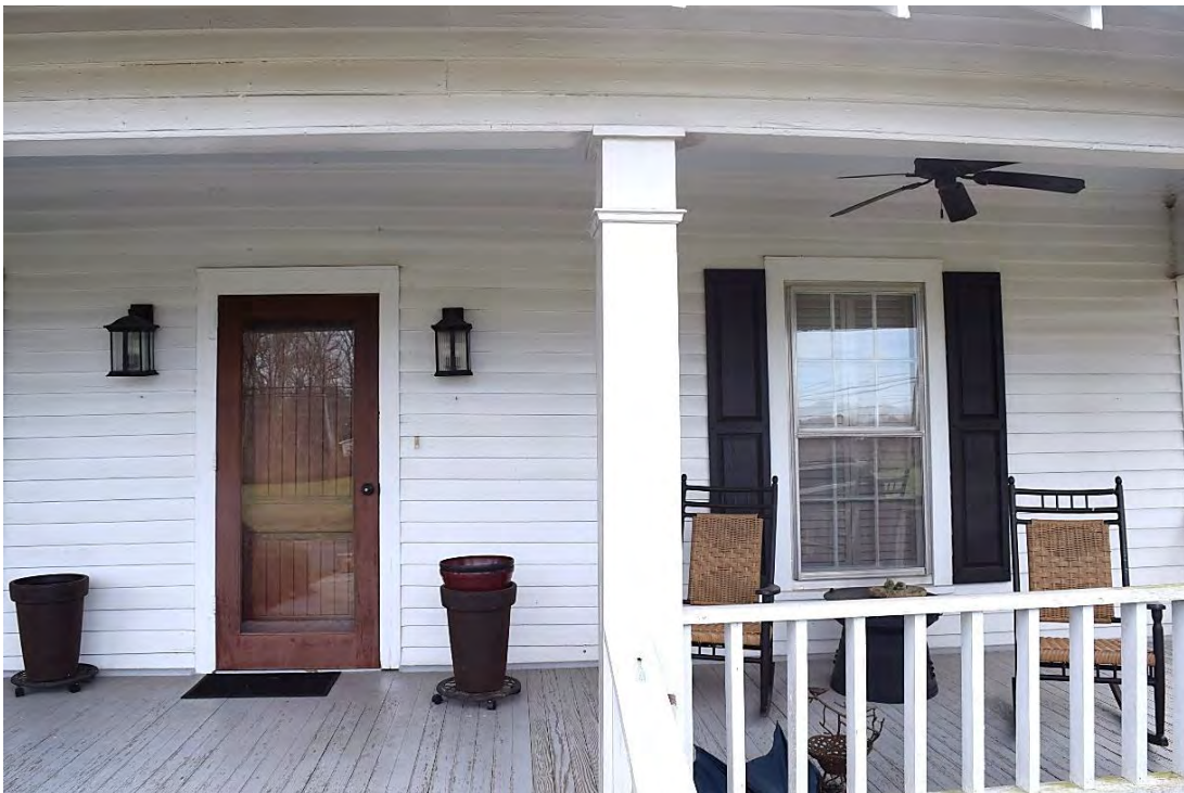
Plyler Family Homeplace, Front Porch with Modern Front Door and Modern Railing.
