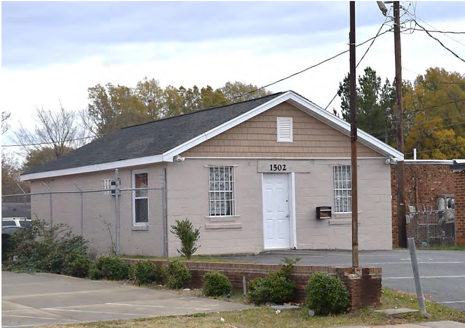
No. 20 Commercial Building (PIN 09226037), 1504 Concord Avenue, Monroe, Union County
