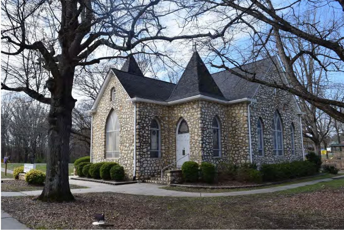
Indian Trail Presbyterian Church (UN0199), 1913, Stone Veneer 1935, 200 Indian Trail Road, Indian Trail, Union County.
