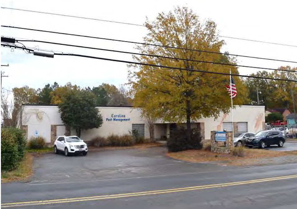
No. 21 Commercial Building (PIN 09226040), 1410 Concord Avenue, Monroe, Union County
