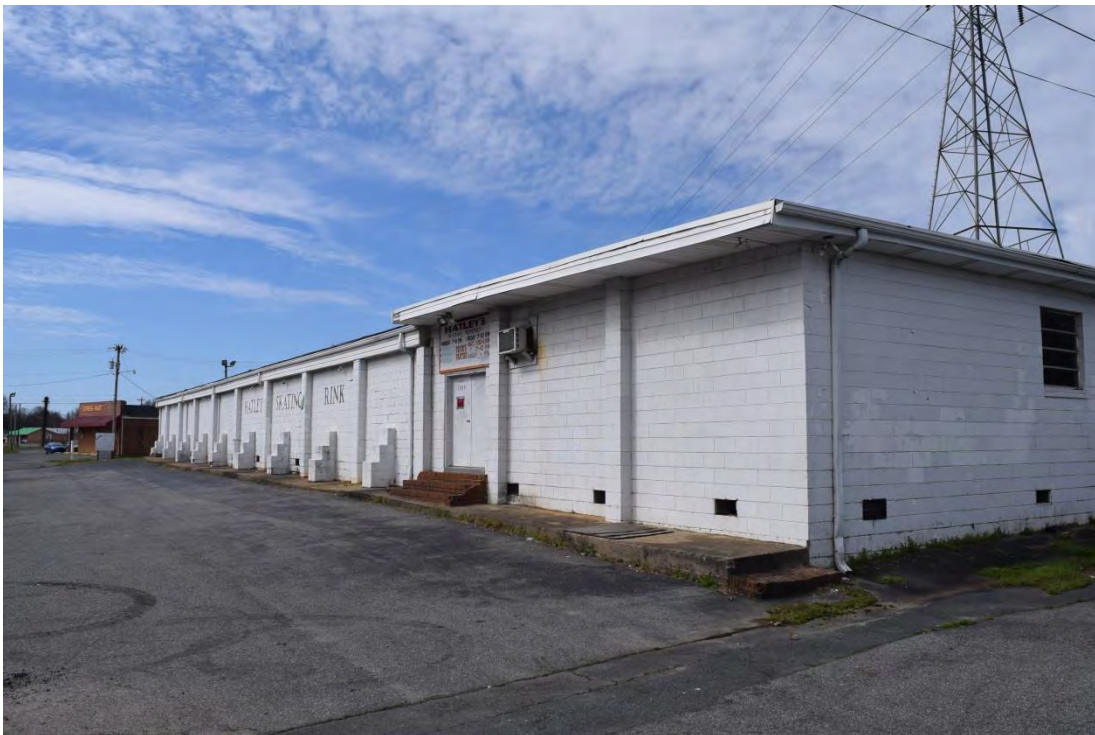
Hatley's Skating Rink, North Section Containing Office and Ticket Lobby, Looking Southwest from Concord Avenue.
