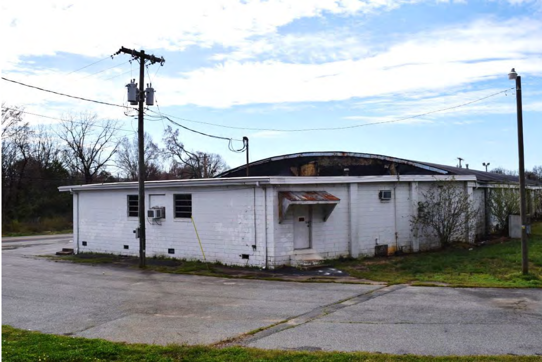
Hatley's Skating Rink, North and West Elevations, Looking South.
