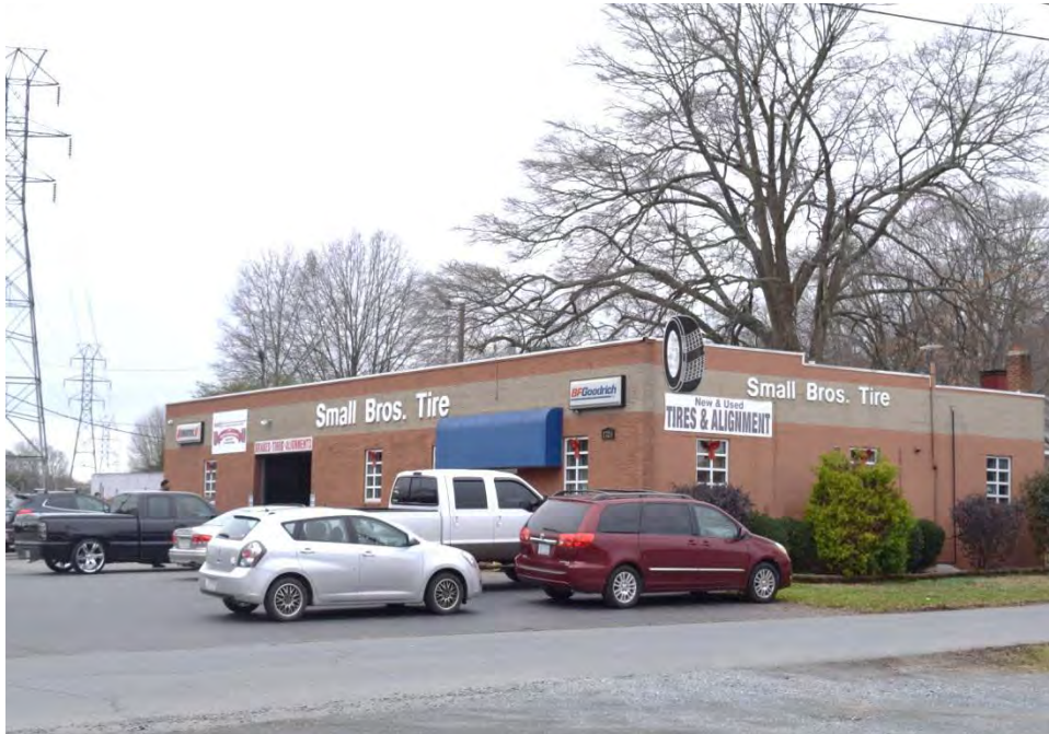
No. 15 Automobile Service Garage (PIN 09223052), 1725 Concord Avenue, Monroe, Union County
