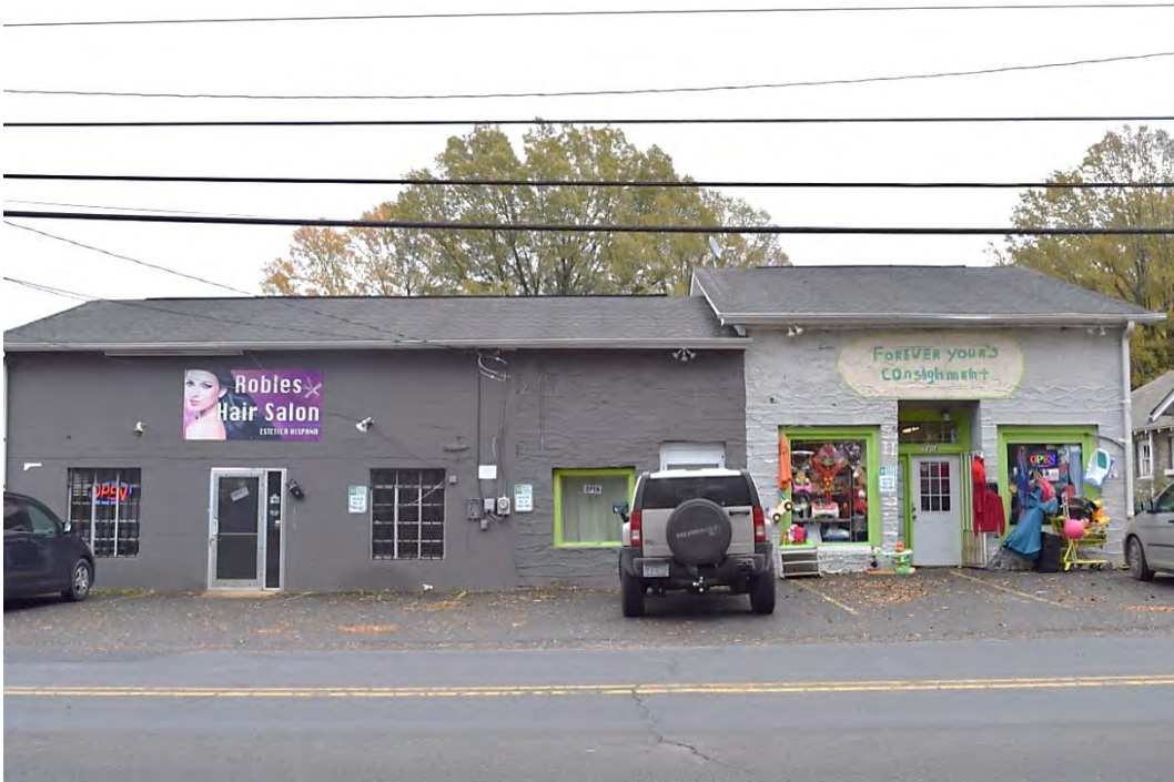
J.P. King Store (No. 25), Excluded from Historic District, Looking East,
