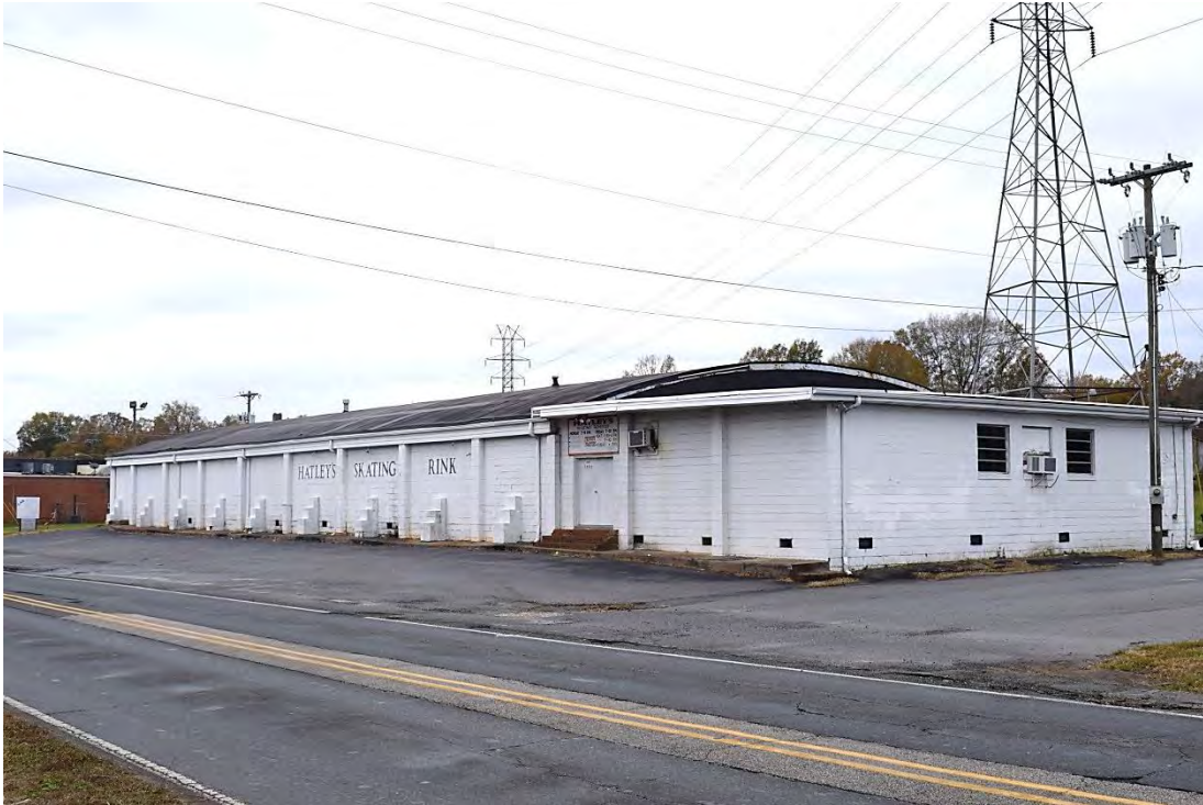
Hatley's Skating Rink, Overall View, Looking Southwest from Concord Avenue.
