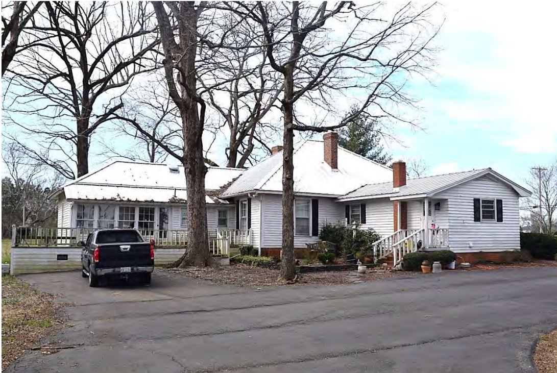
Plyler Family Homeplace, Main Block, 1954 Wing, and Rear Ell, Looking Southwest.
