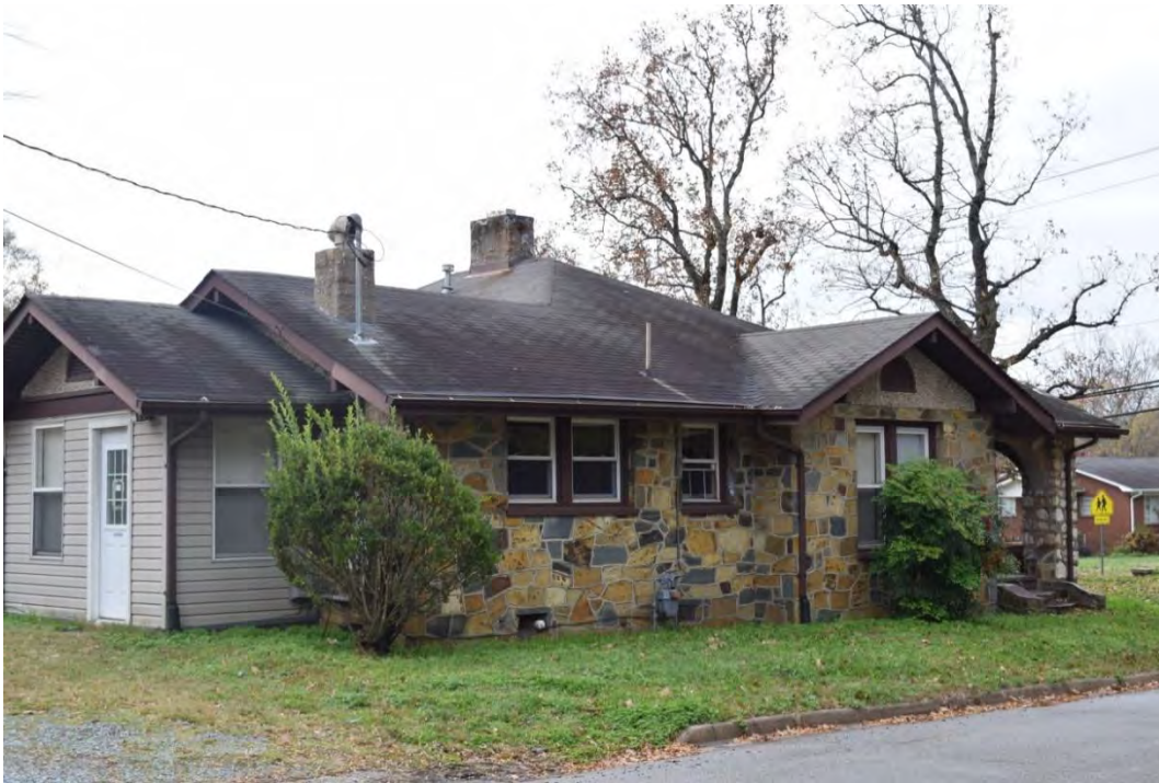
Concord Avenue Stone Bungalows Historic District, House (No. 28), Looking Southwest.
