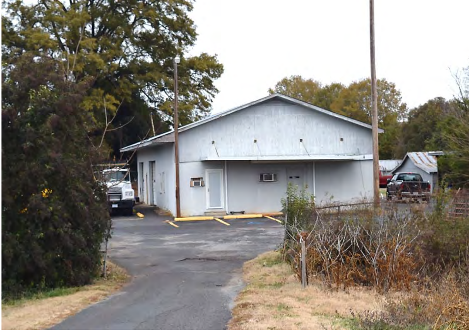
No. 3 Commercial Building (PIN 091800041), 2170 Concord Avenue, Monroe, Union County
