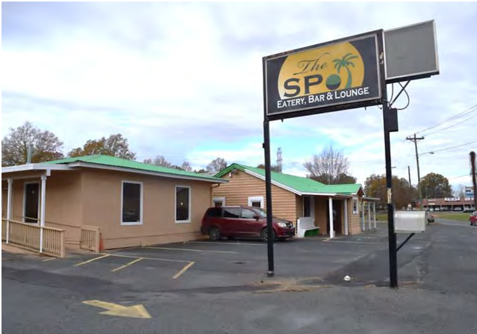
No. 19. Commercial Buildings (PIN 09226195), 1513 Concord Avenue, Monroe, Union County
