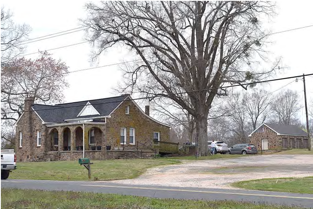
Thomas Griffin House (UN0143), 1936, Stone Exterior 1946, 614 West Main Street, Marshville, Union County.
