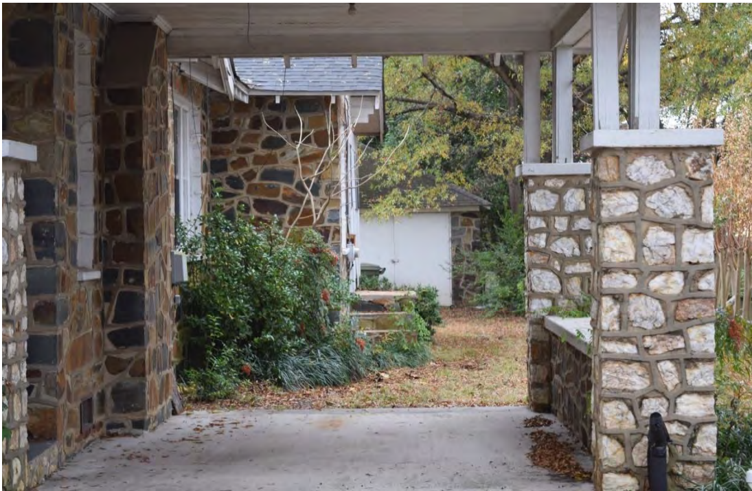
Concord Avenue Stone Bungalows Historic District, House (No. 30), Garage in Background, Looking West.
