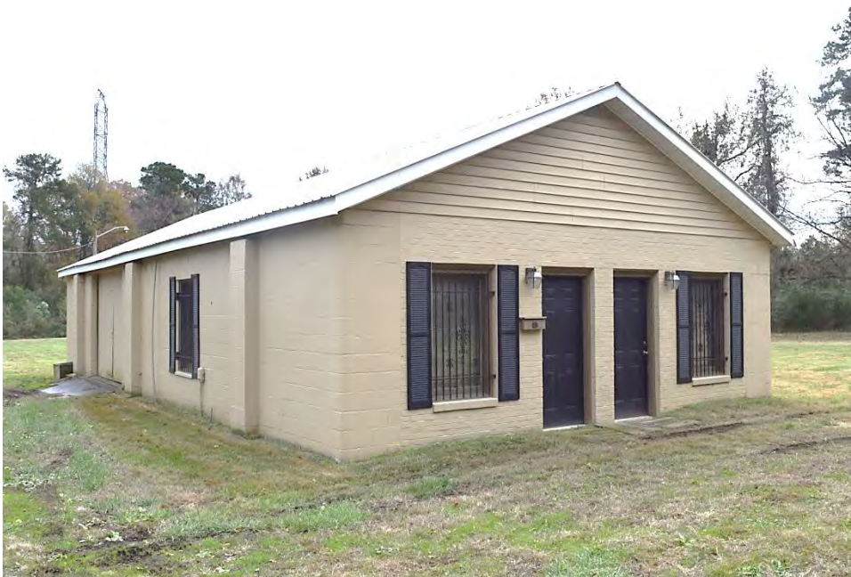
No. 9 Commercial Building (PIN 09223003), 1900 Concord Avenue, Monroe, Union County
