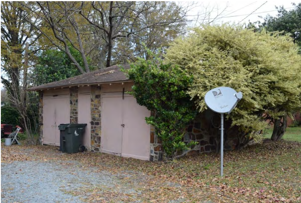
Concord Avenue Stone Bungalows Historic District, J.P. and Ida King House No. 2 (No. 27), Garage, Looking North from King Street.
