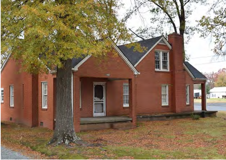
No. 22 Duplex (PIN 09226192A), 1409 Concord Avenue, Monroe, Union County
