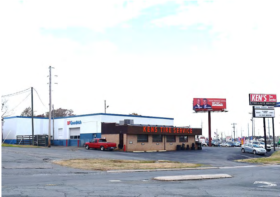
No. 14 Automobile Service Garage (PIN 09223069), 2001 West Roosevelt Boulevard, Monroe, Union County
