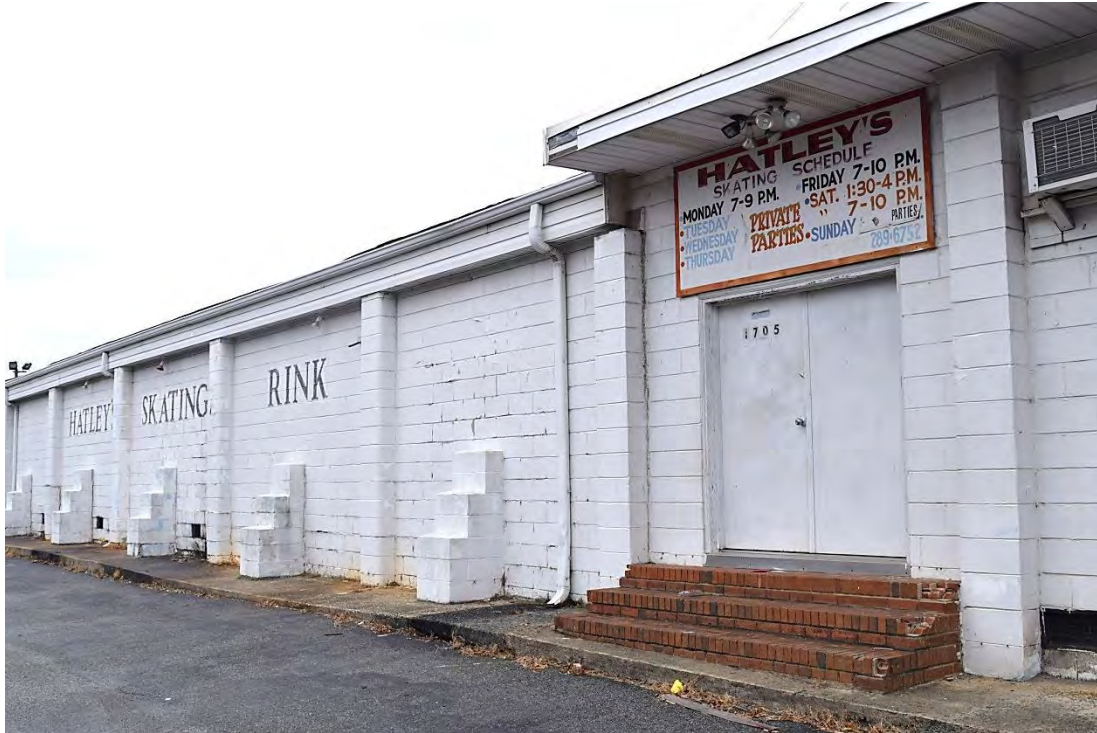
Hatley's Skating Rink, East Elevation and Entrance.
