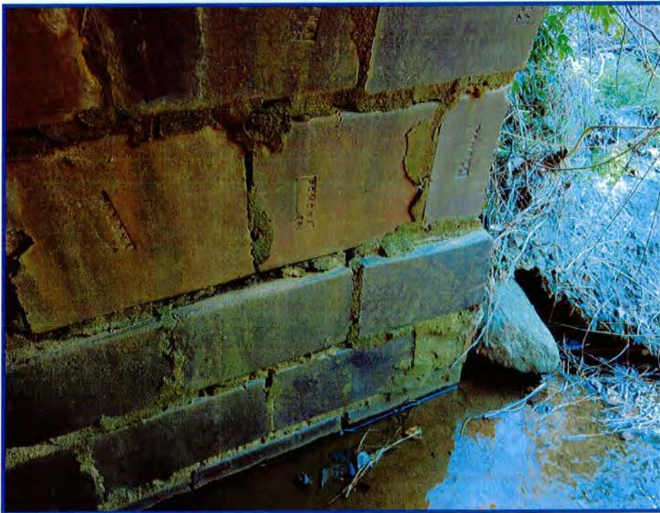
Arch Culvert (Pipe #40 2112) SR 2735 (Sockwell Road) Guilford County Looking south (above).
