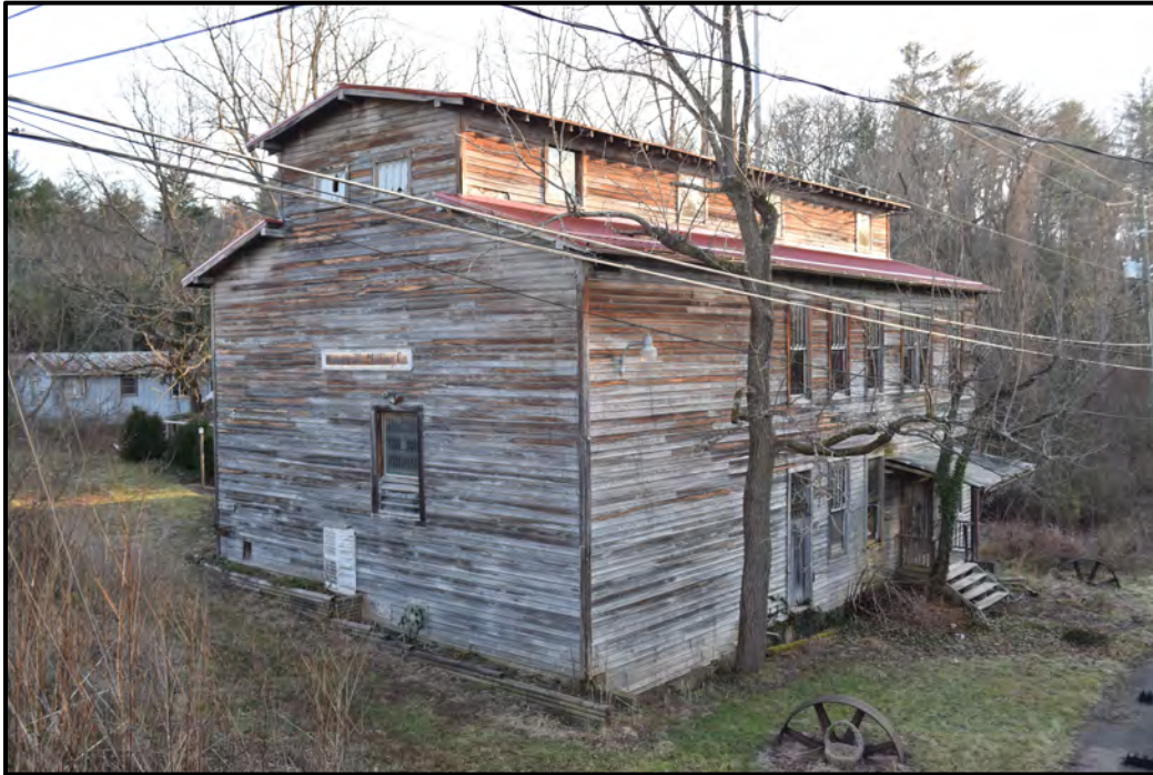
Weaverville Milling Company, north corner, view to the south
