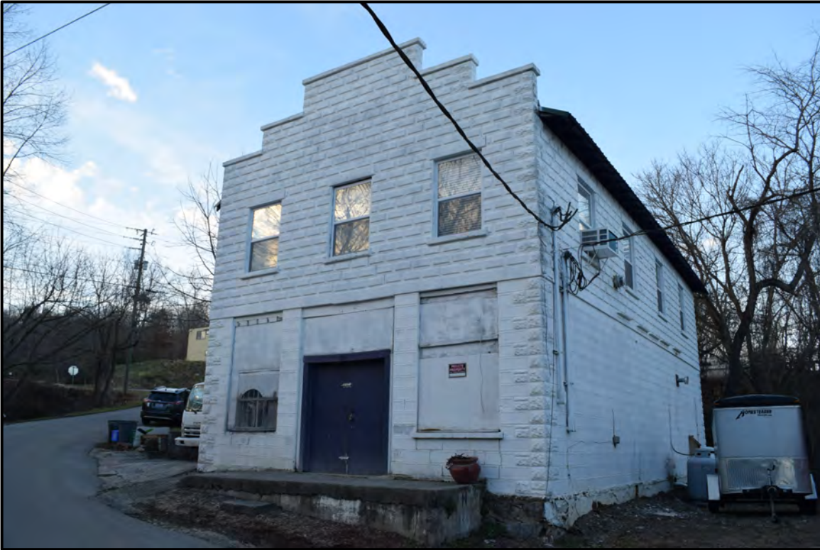
Southeast corner, view to the northwest
