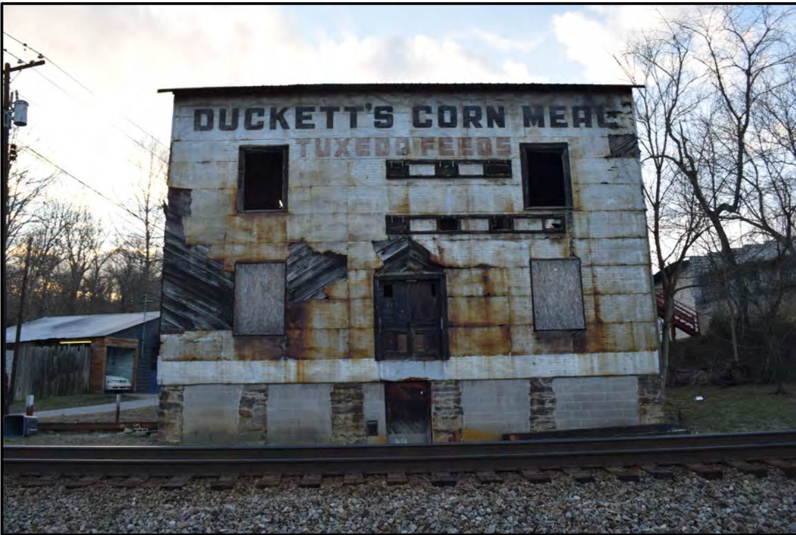
East elevation, view to the west
