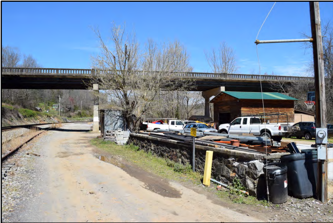
Modern garage north of house, view to the north-northeast
