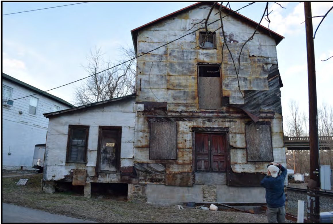
Facade, view to the north
