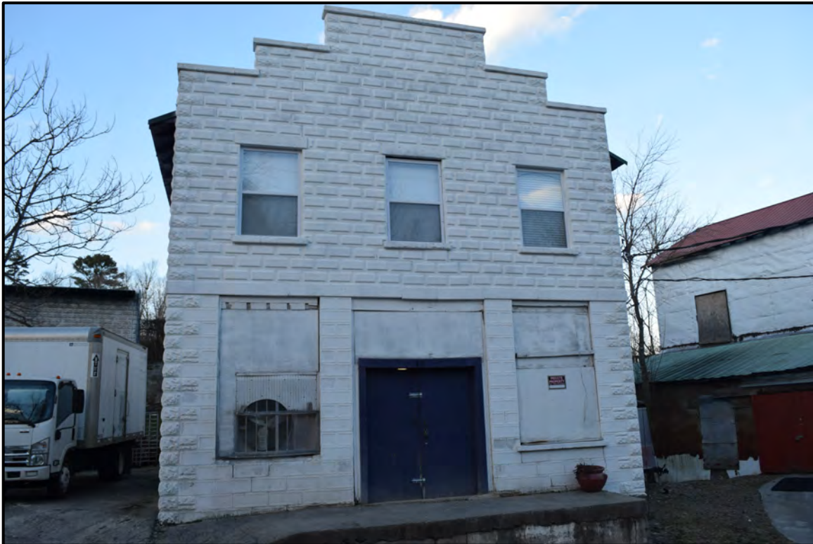
Facade, view to the north
