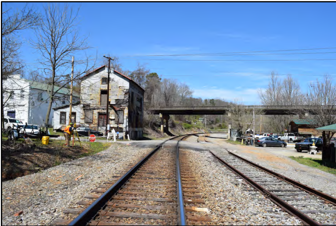
Lower portion of Craggy with Bridge No. 649 in background and Craggy Milling Company (BN0345) to the left, view to the south
