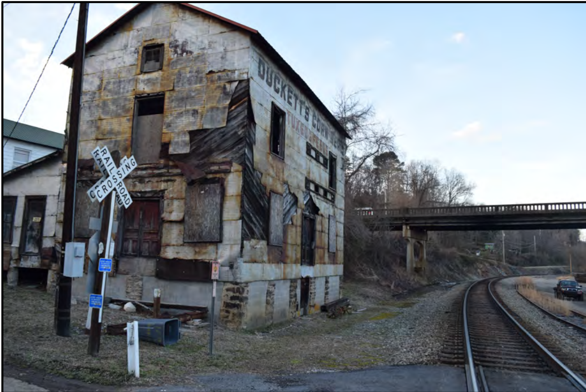
Craggy Milling Company's south side, view to the north
