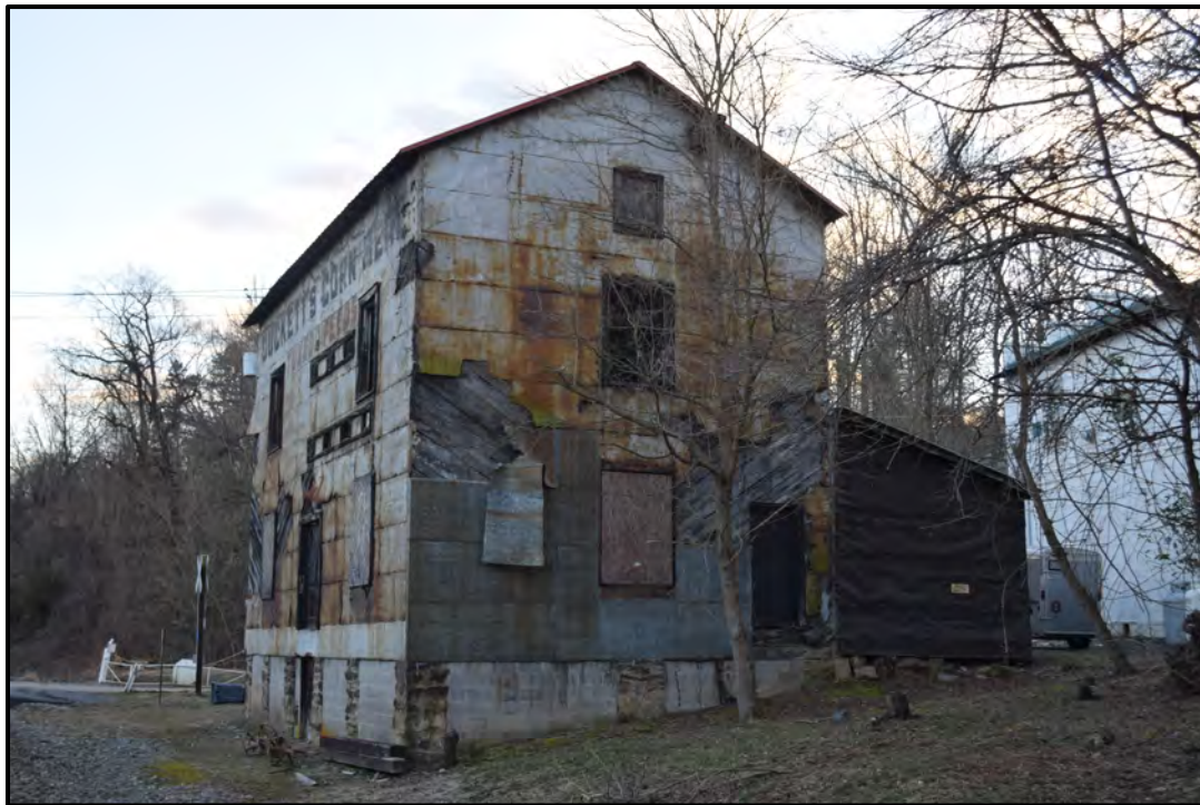
Rear elevation (northeast corner), view to the south-southwest
