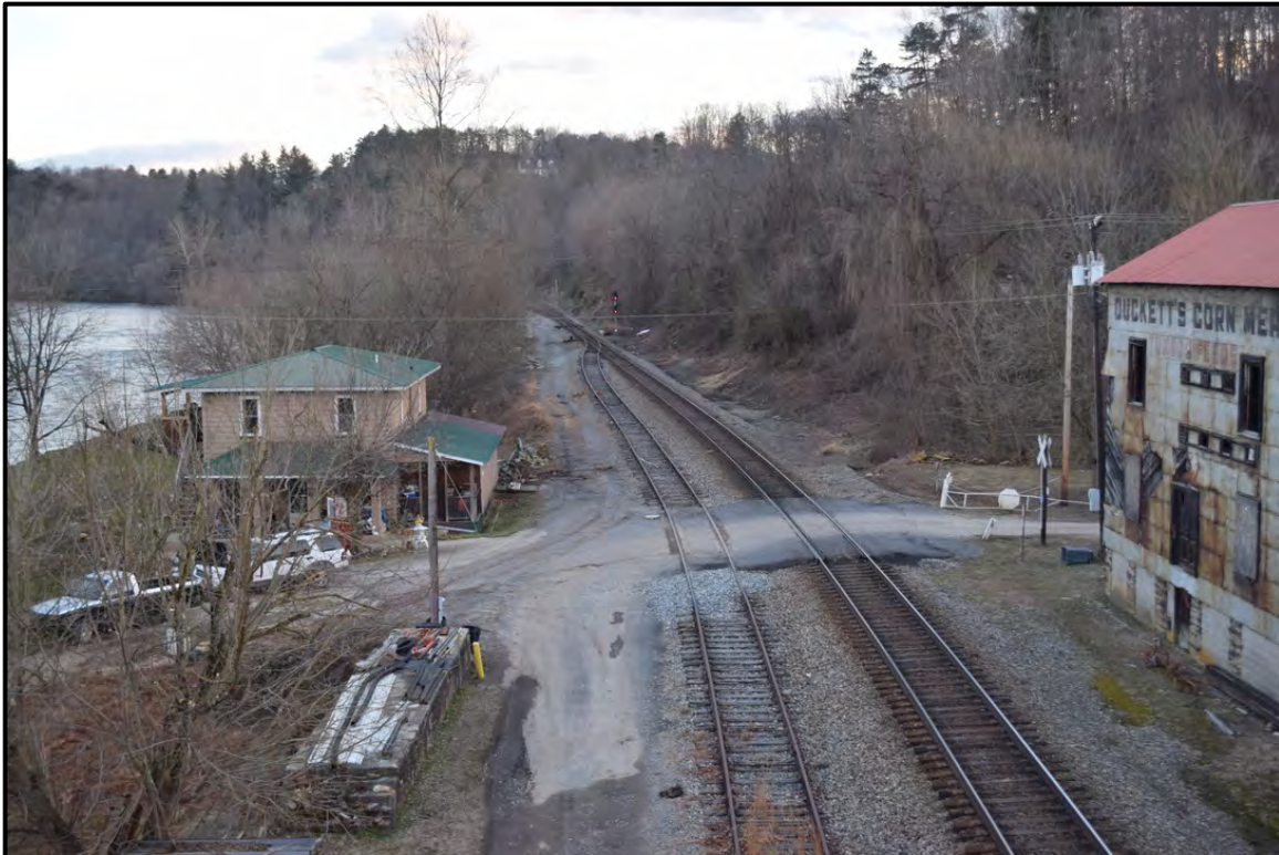
George Mayo House (left) and Craggy Milling Company (right) flanking tracks of the former Southern Railway, view to the south
