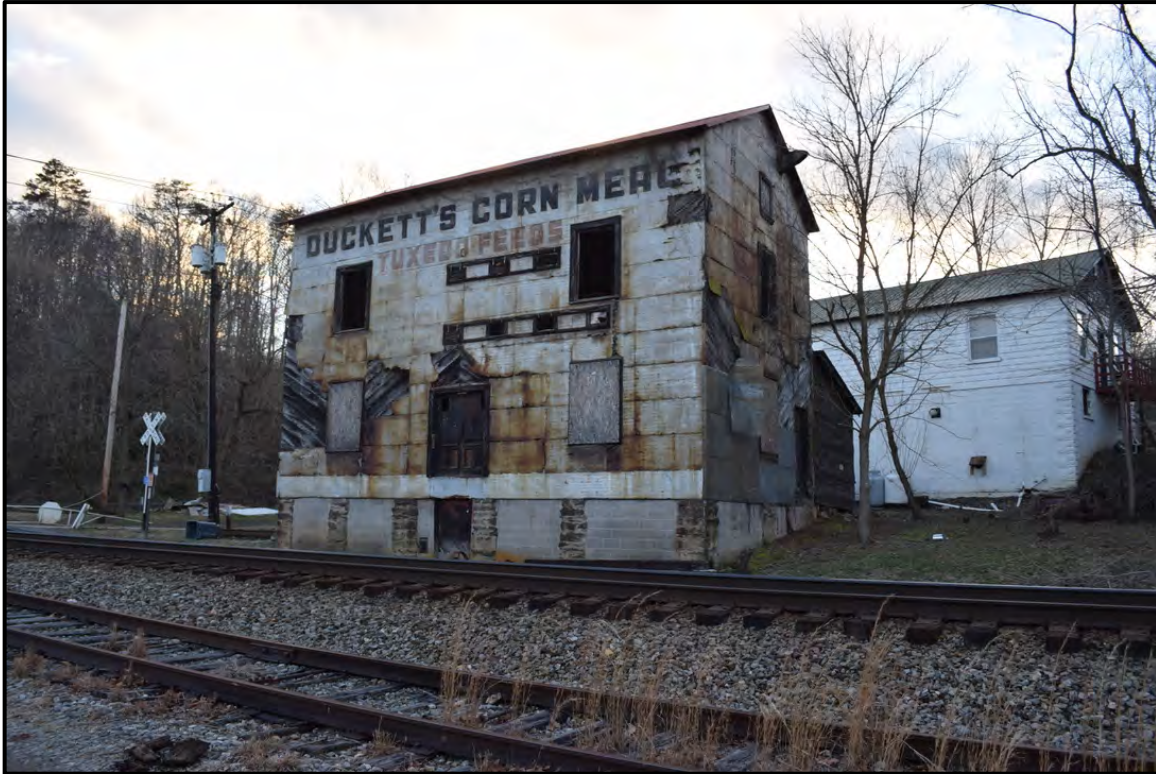
Craggy Milling Company, view to the southwest
