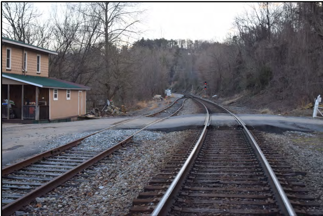
Railroad tracks at Craggy. Those on the left likely date to circa 1906, the period when Southern Railway took over this route. The rails on the right likely date to 1958. View to the south
