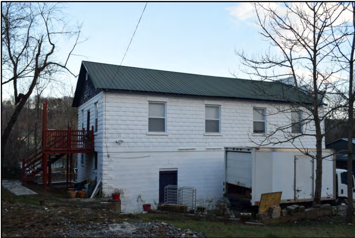
West elevation, view to the east-southeast
