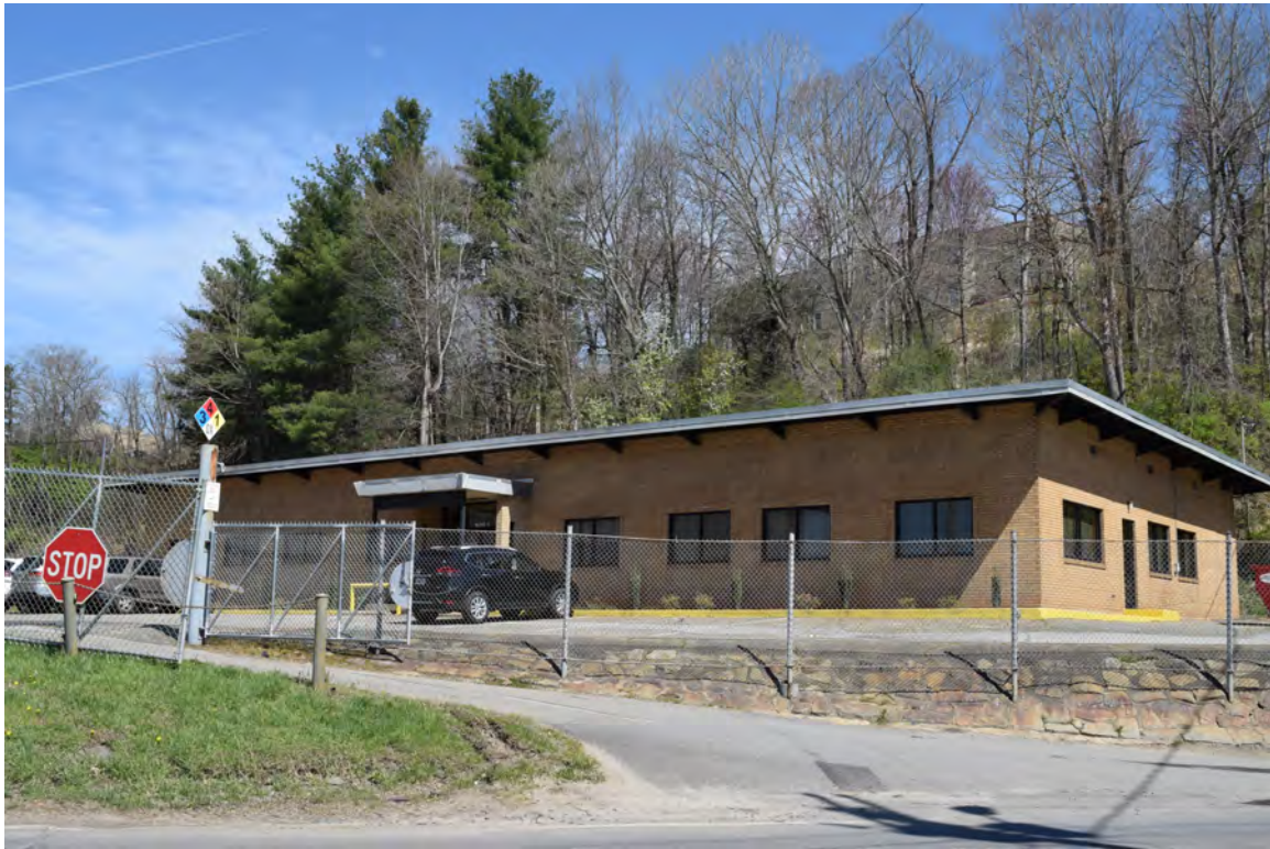
1964 office, view to the northeast
