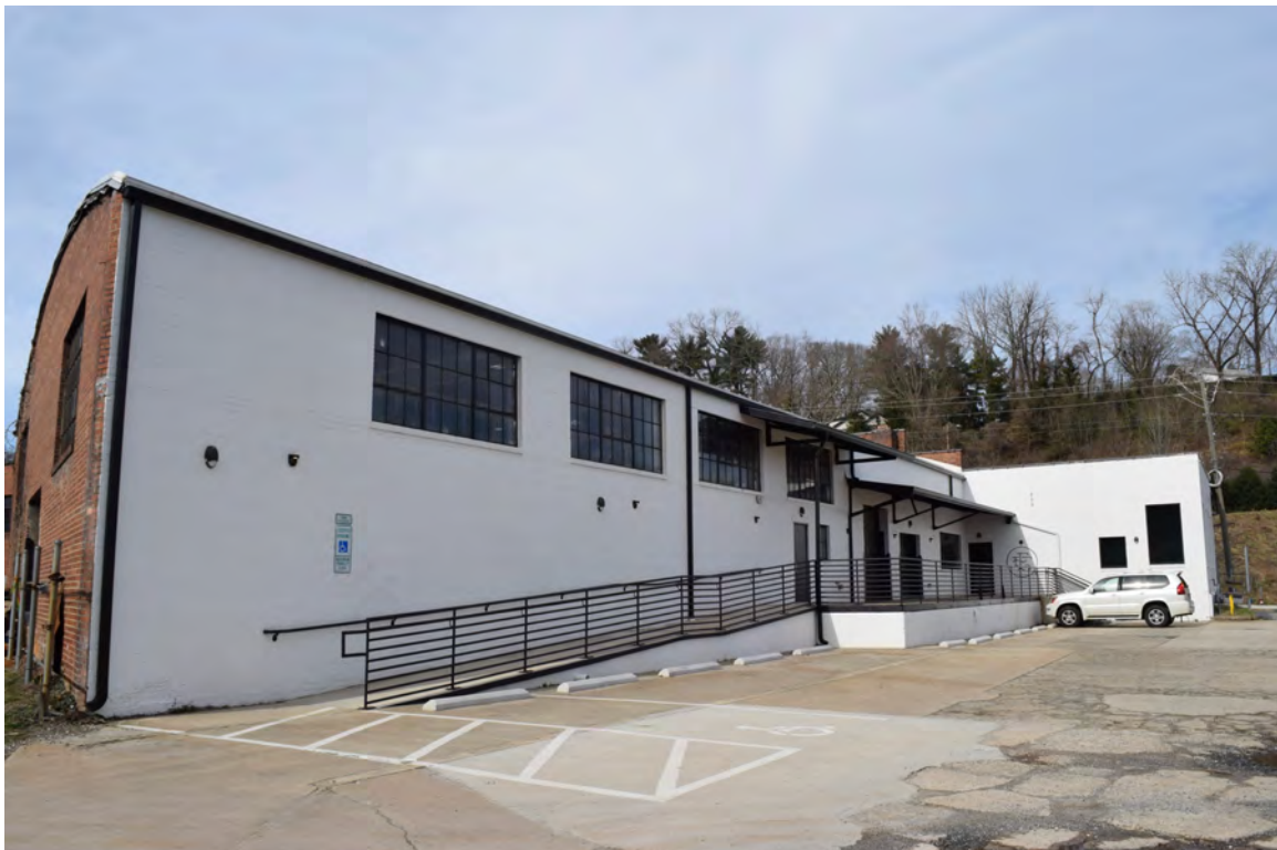
Southwest corner of warehouse and loading dock, view to the north
