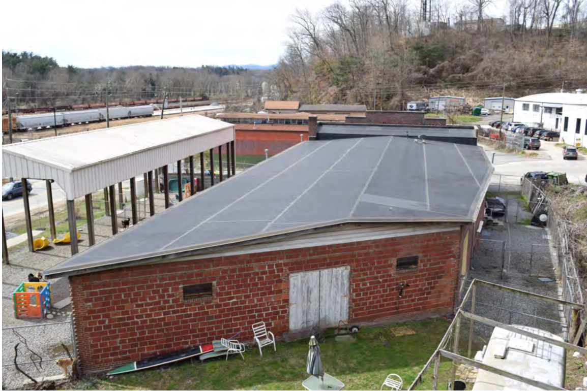
Rear elevation, view to the west
