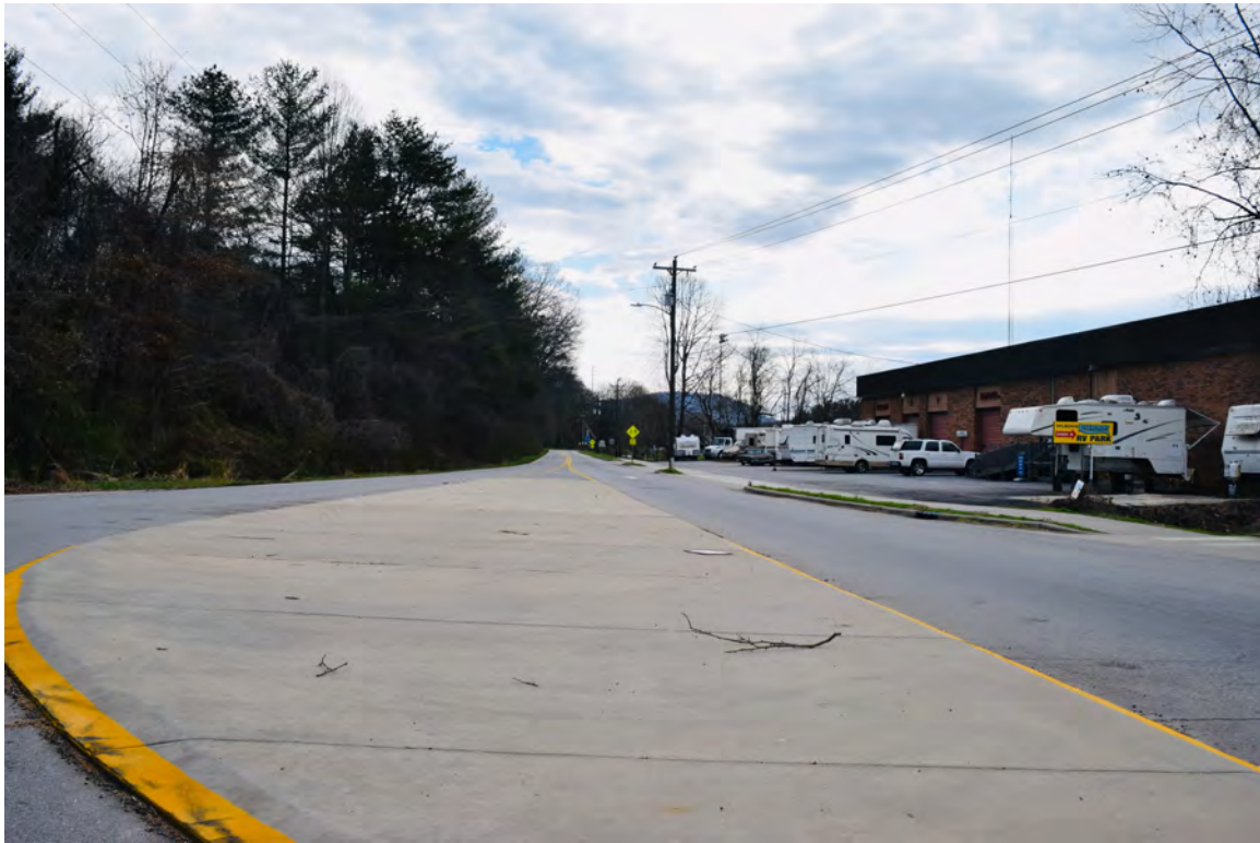
West End of Project Area on Amboy Road, view to the East
