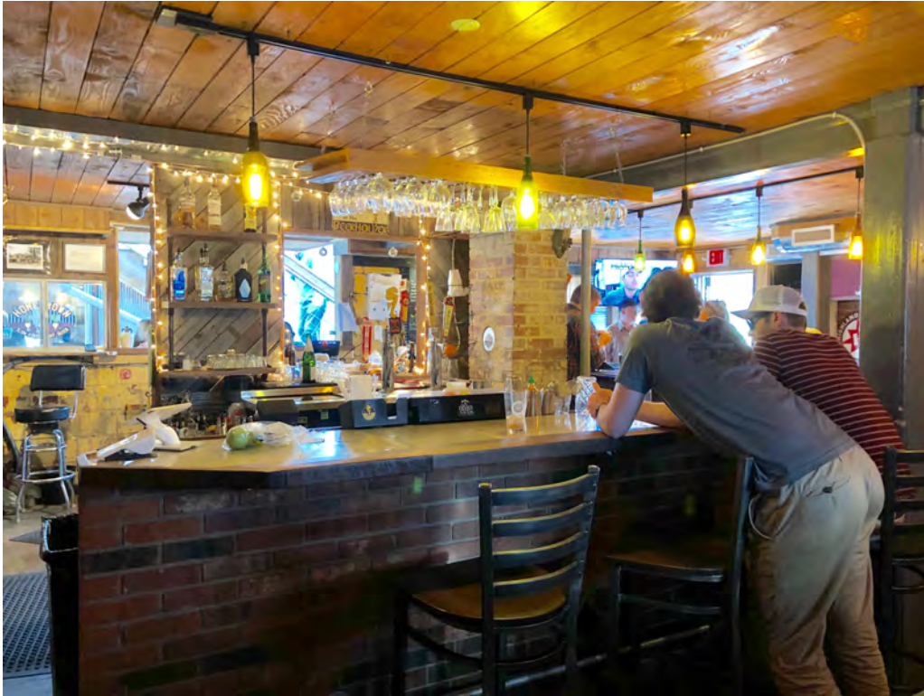
Original bar foundation in west building, view to the east-southeast
