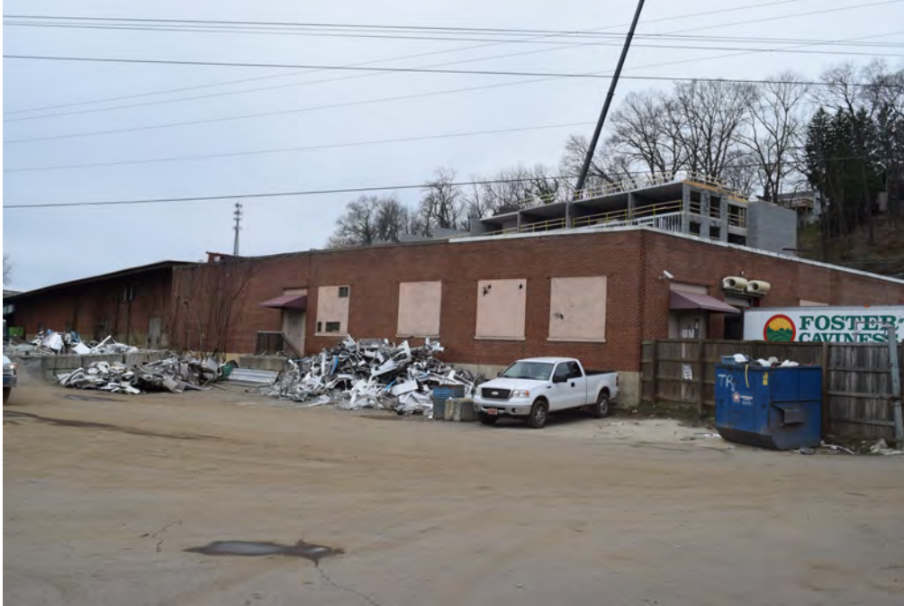
Rear (southeast) elevation, view to the northwest
