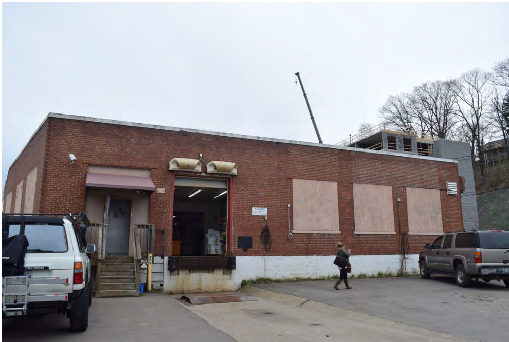
Northeast end loading dock, view to the southwest
