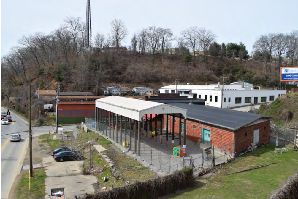
Southeast (rear) corner with Meadow Road to the left, view to the west-northwest
