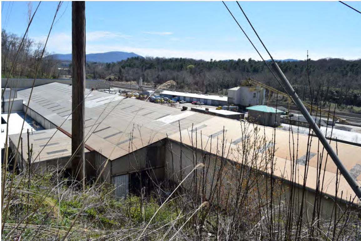
1964 portions of plant, view to the southeast
