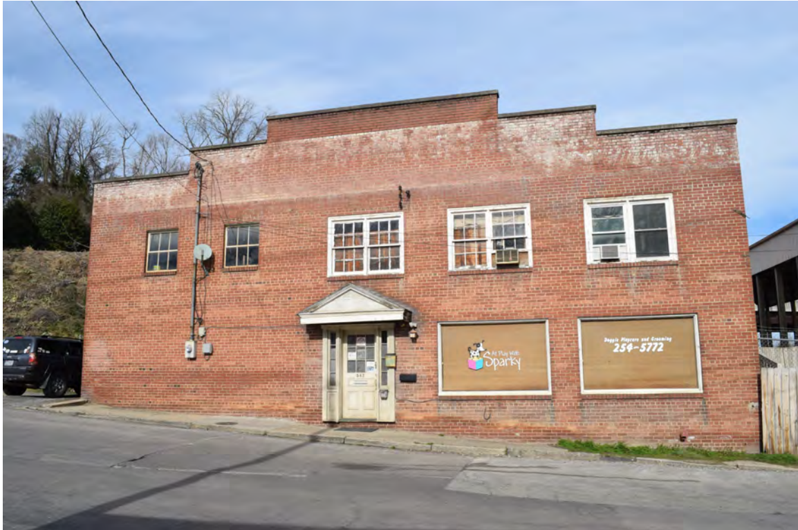
Façade of Colonial Mica Corporation, view to the east
