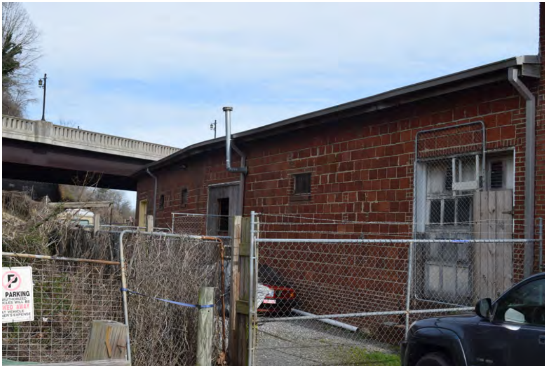
North side of the warehouse, view to the southeast
