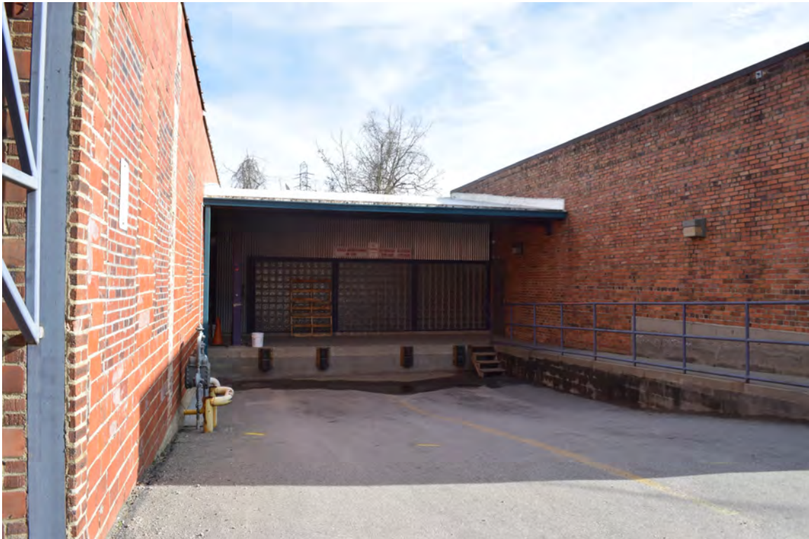
Loading dock and hyphen between the buildings, view to the southeast
