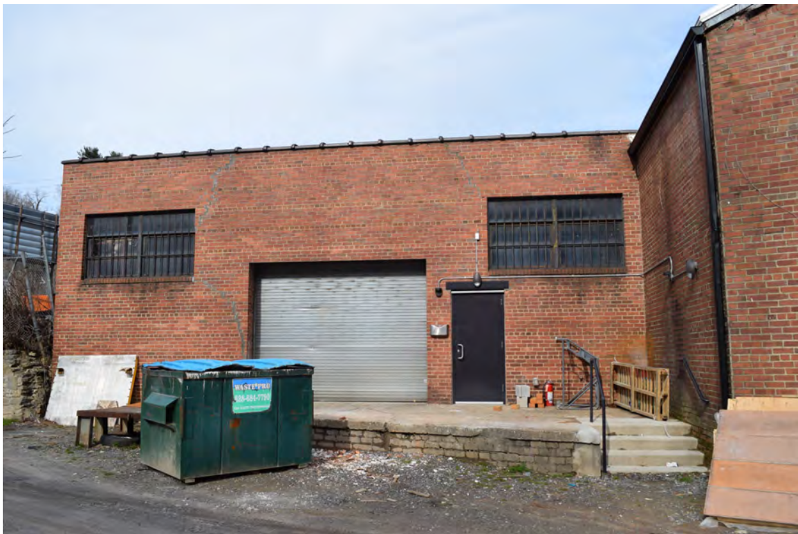
Rear of north warehouse, view to the northwest
