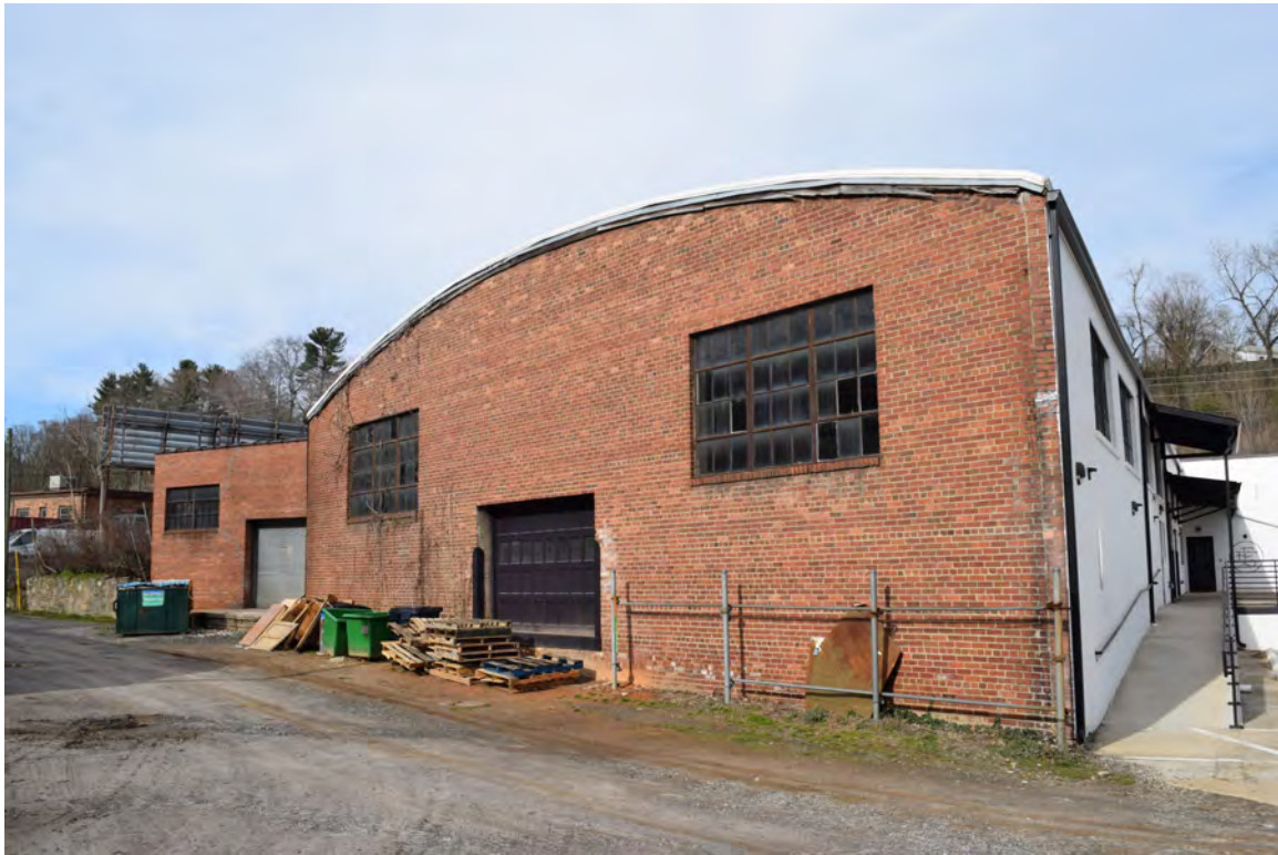
Rear of warehouse and loading dock, view to the northwest
