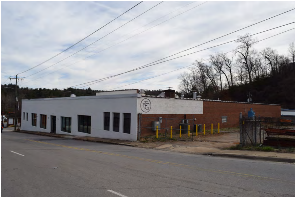
North side of the Crane Company Wholesale Plumbing Supplies, view to the south
