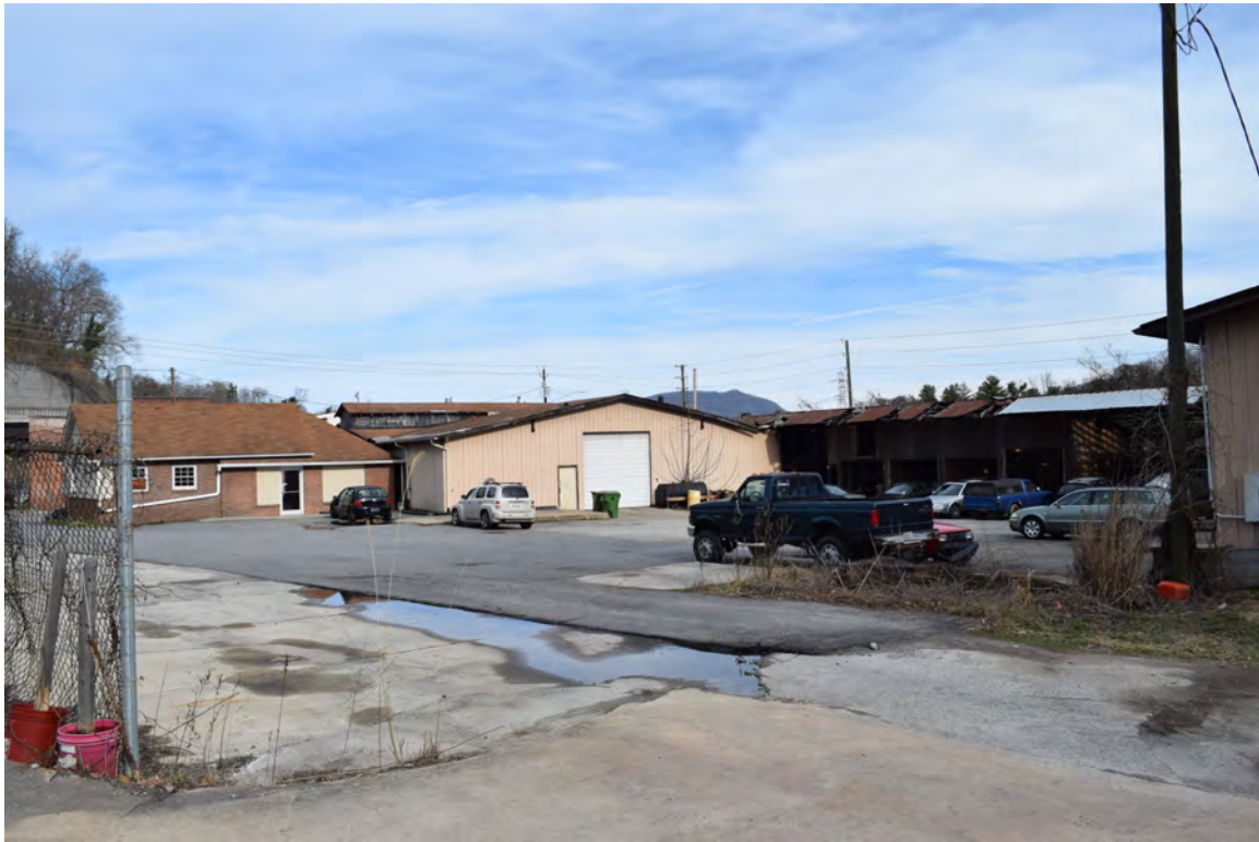
Overall north side of complex with modern warehouse at center and the rear of the office to the left, view to the southeast
