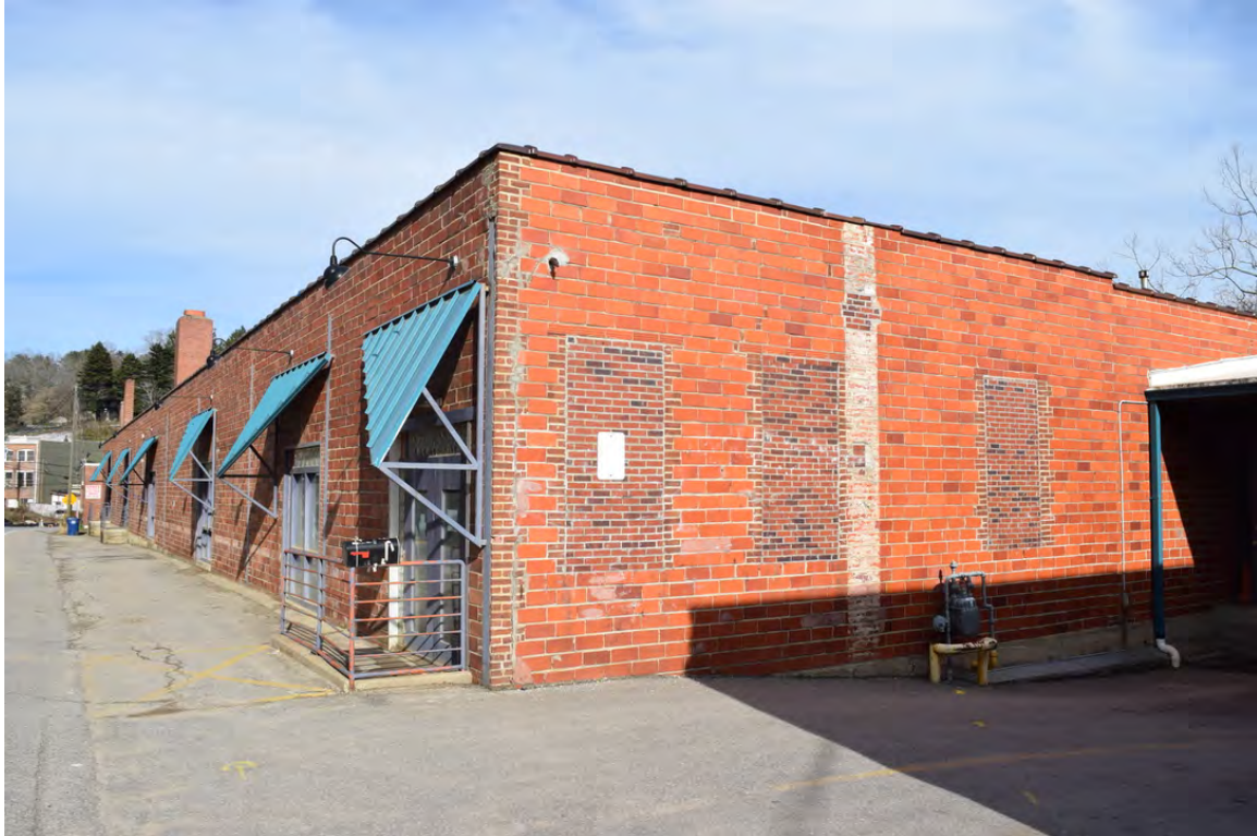
West corner of north building, view to the east
