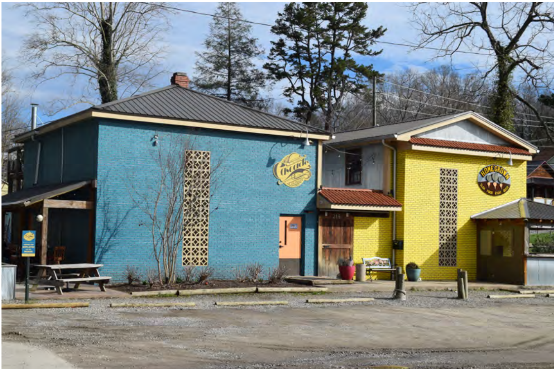
Facade, view to the Northeast
