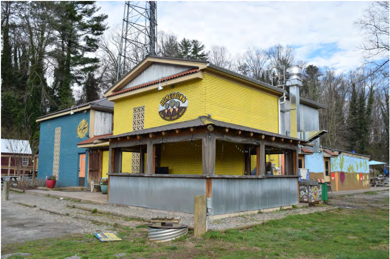
Southeast (front) corner, view to the northwest
