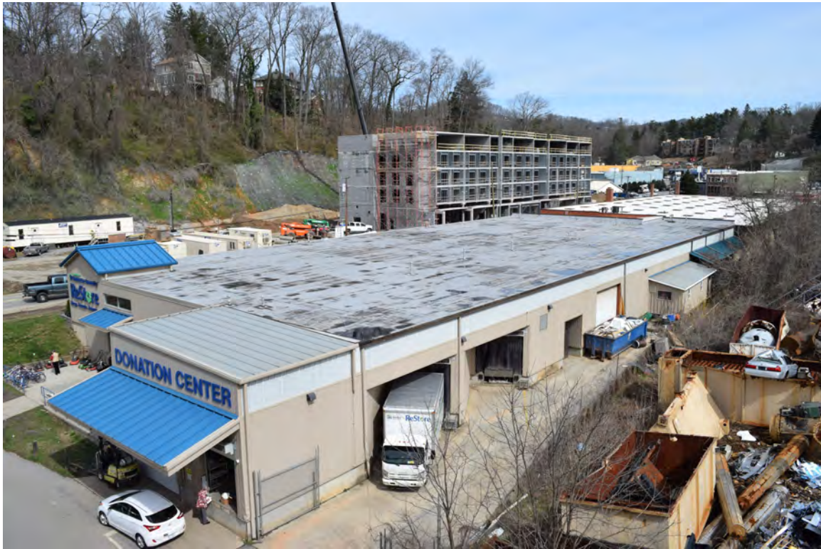
Southern section of warehouse, view to the northeast
