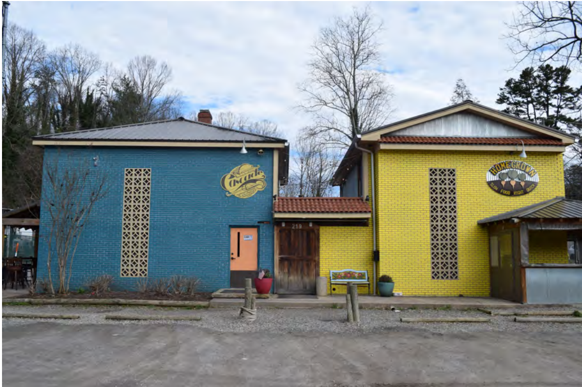
Facade, view to the North
