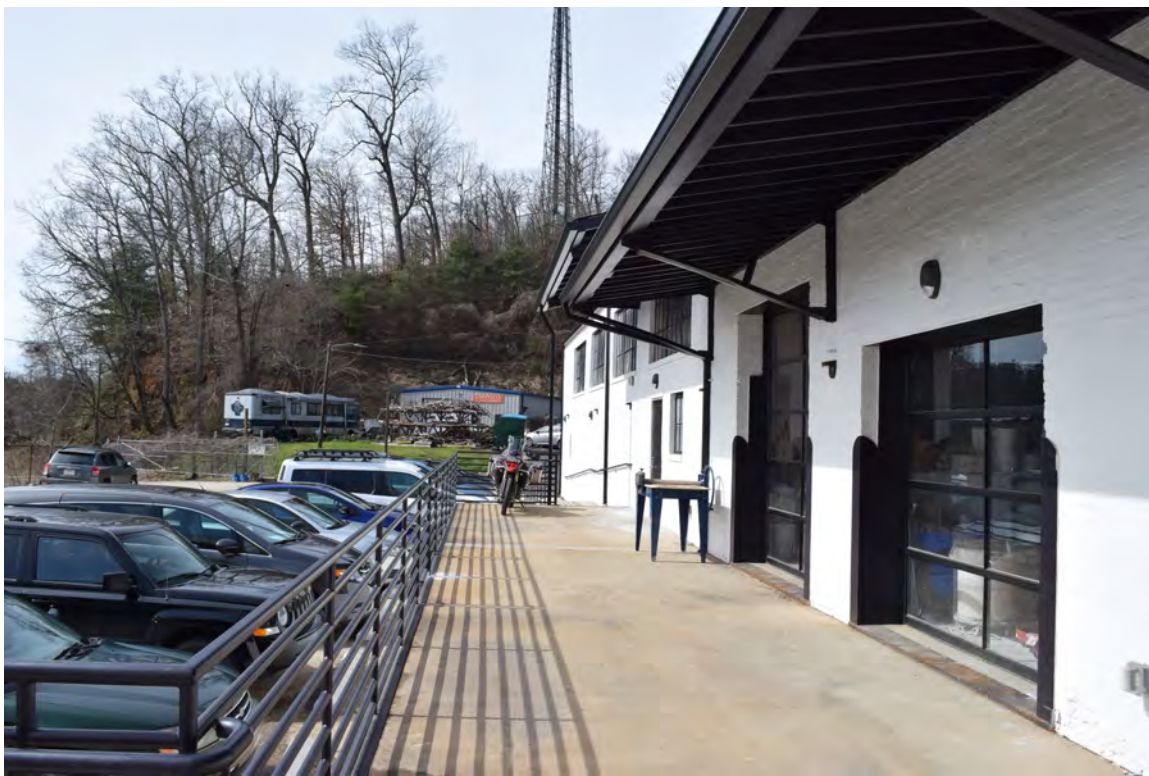
Loading dock, view to the southwest
