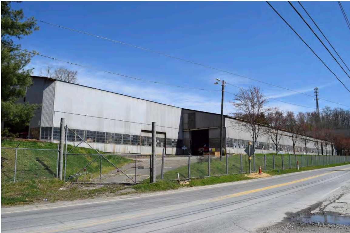
Original (1964) section of Asheville Steel and Salvage Company, view to the northeast
