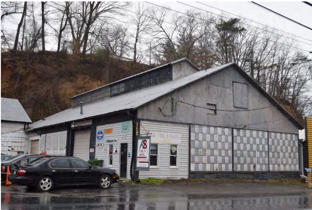
North Carolina State Highway Commission division garage built in 1930, view to the northwest
