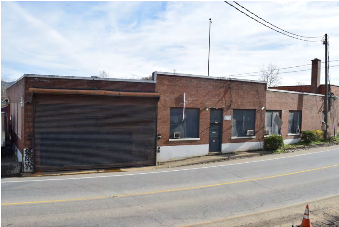
Northwest elevation along Meadow Road, view to the southeast
