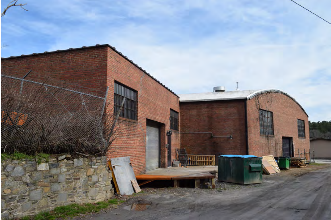
Rear of warehouses, view to the south
