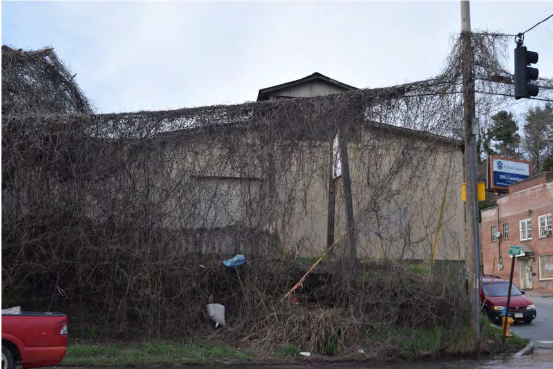
Original warehouse, south elevation, view to the northwest
