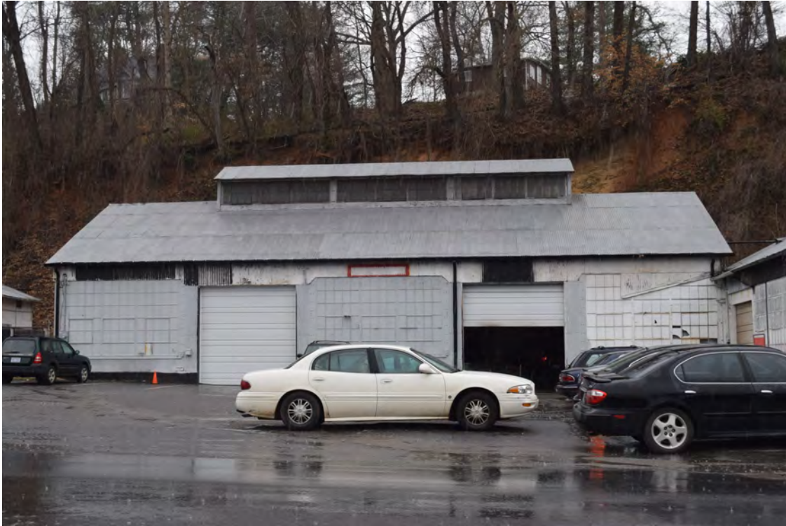
North Carolina State Highway Commission garage built in 1930, view to the west
