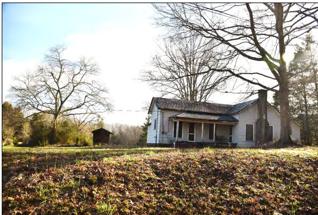
Figure 2.44. Thomas Joyner House (CA0449), facing south.
