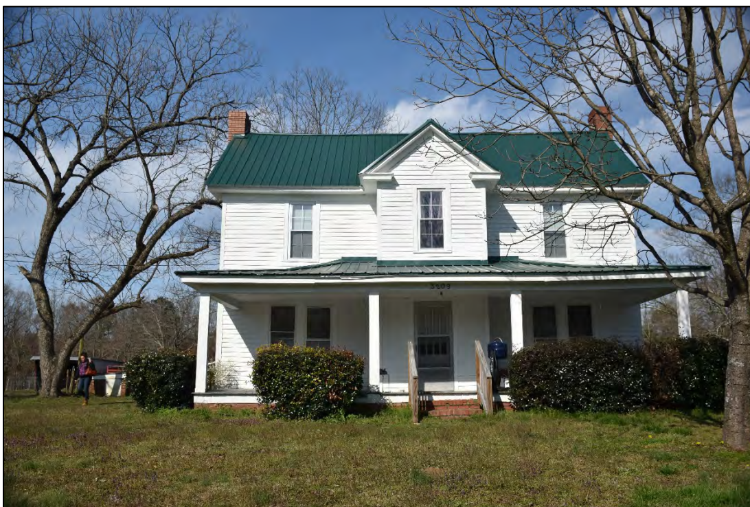
Figure 2.39. Jackson Safrit House (CA0543), facing west.
