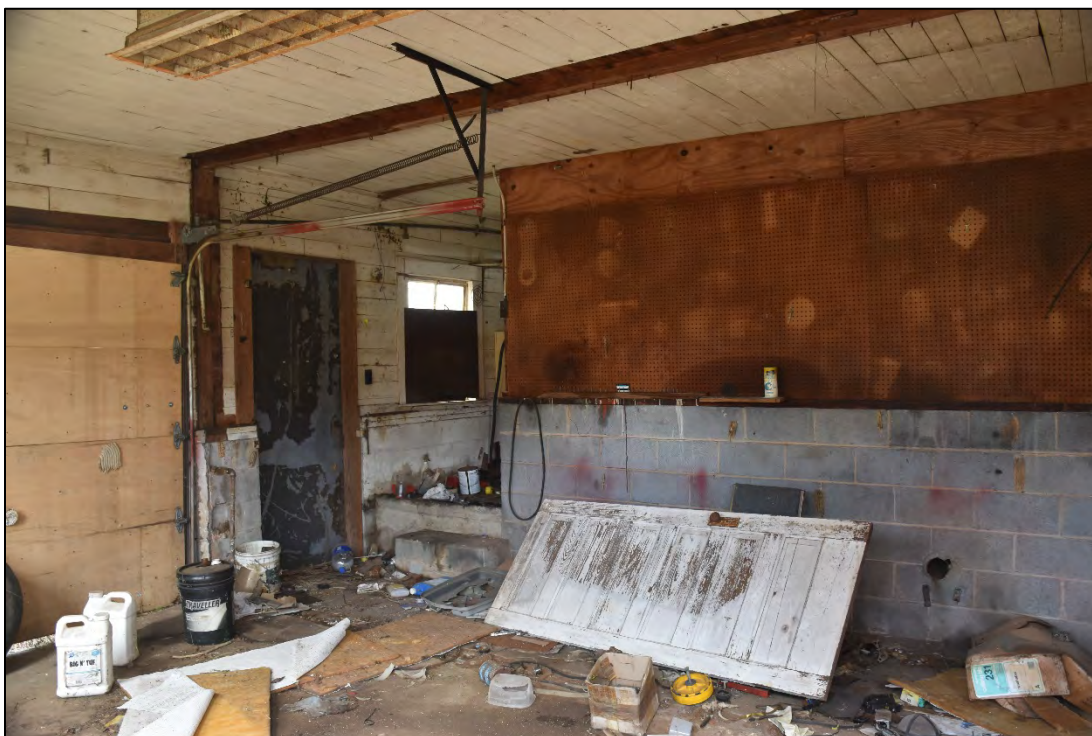
Figure 2.20. Henry Wallace House (CA0597), mid-twentieth-century dairy, interior.
