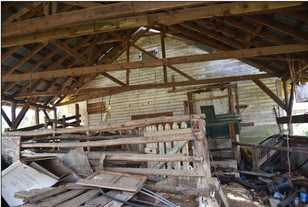
Figure 2.21. Henry Wallace House (CA0597), mid-twentieth-century dairy and barn, interior, facing south.
