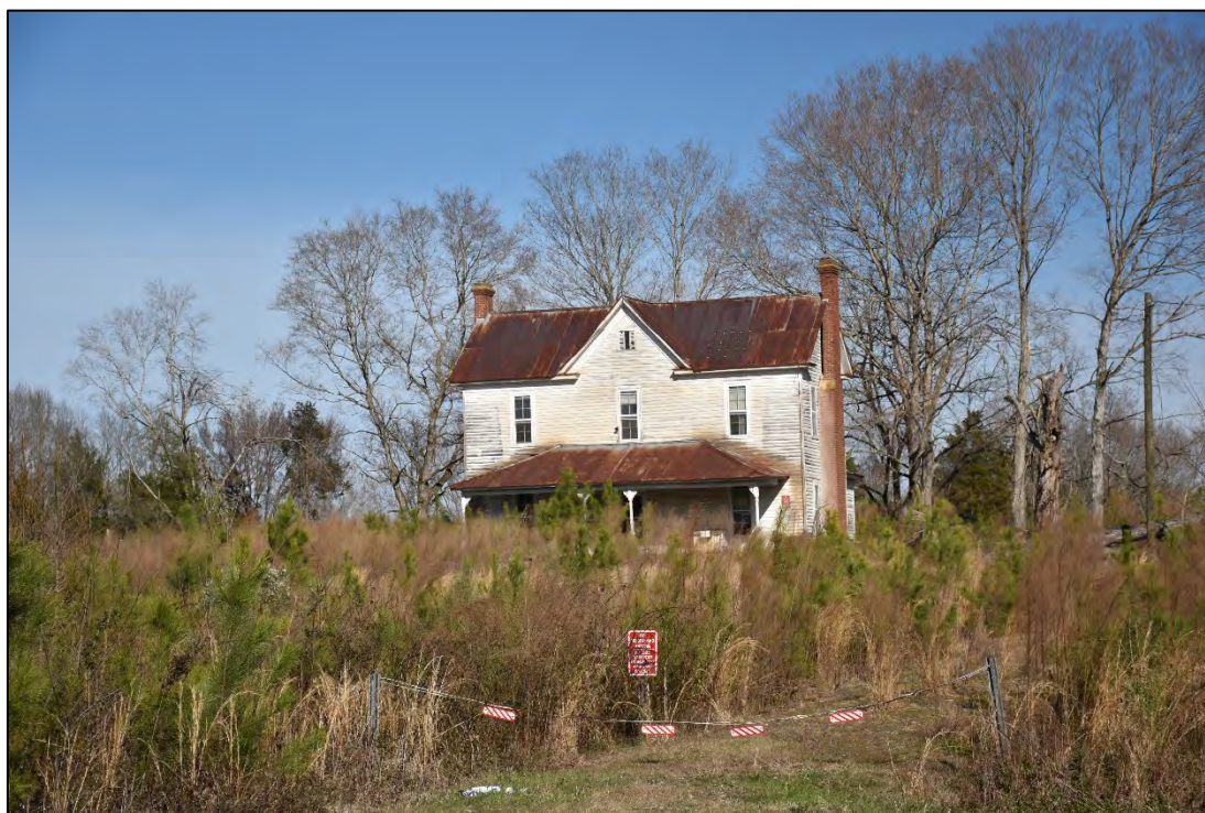
Figure 2.37. Unsurveyed house, 6009 US Highway 601, facing east.
