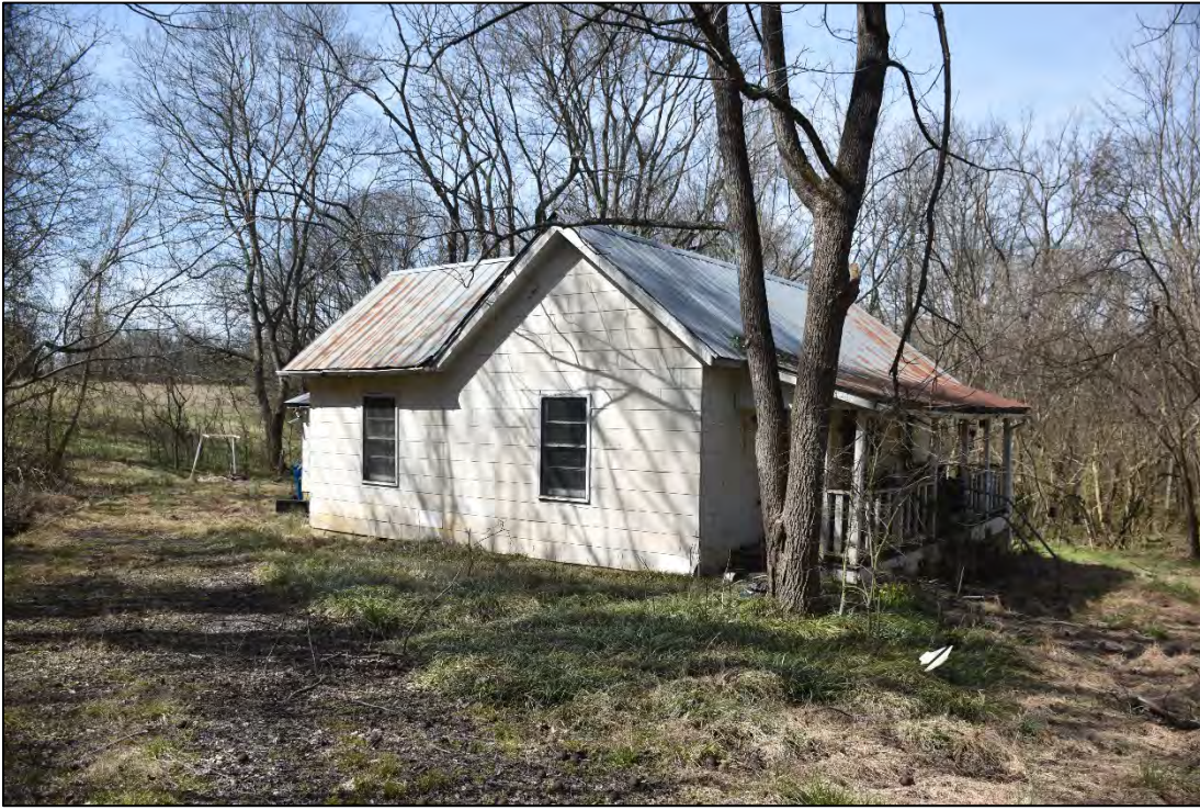
Figure 2.11. Henry Wallace House (CA0597), early-twentieth-century house, facing southwest.
