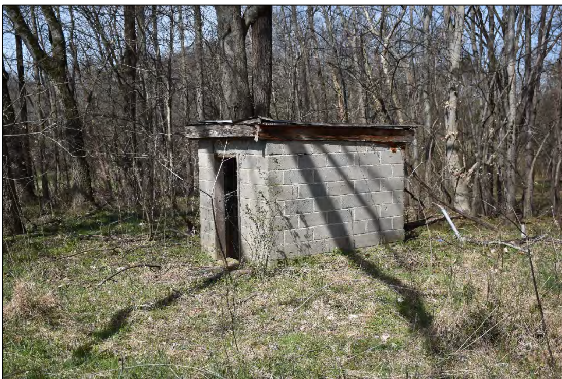
Figure 2.12. Henry Wallace House (CA0597), twentieth-century well house, facing southwest.
