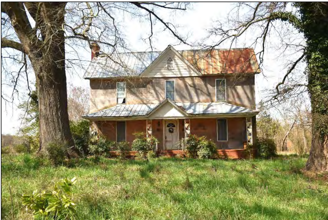
Figure 2.1. Henry Wallace House (CA0597), house, facing east.
