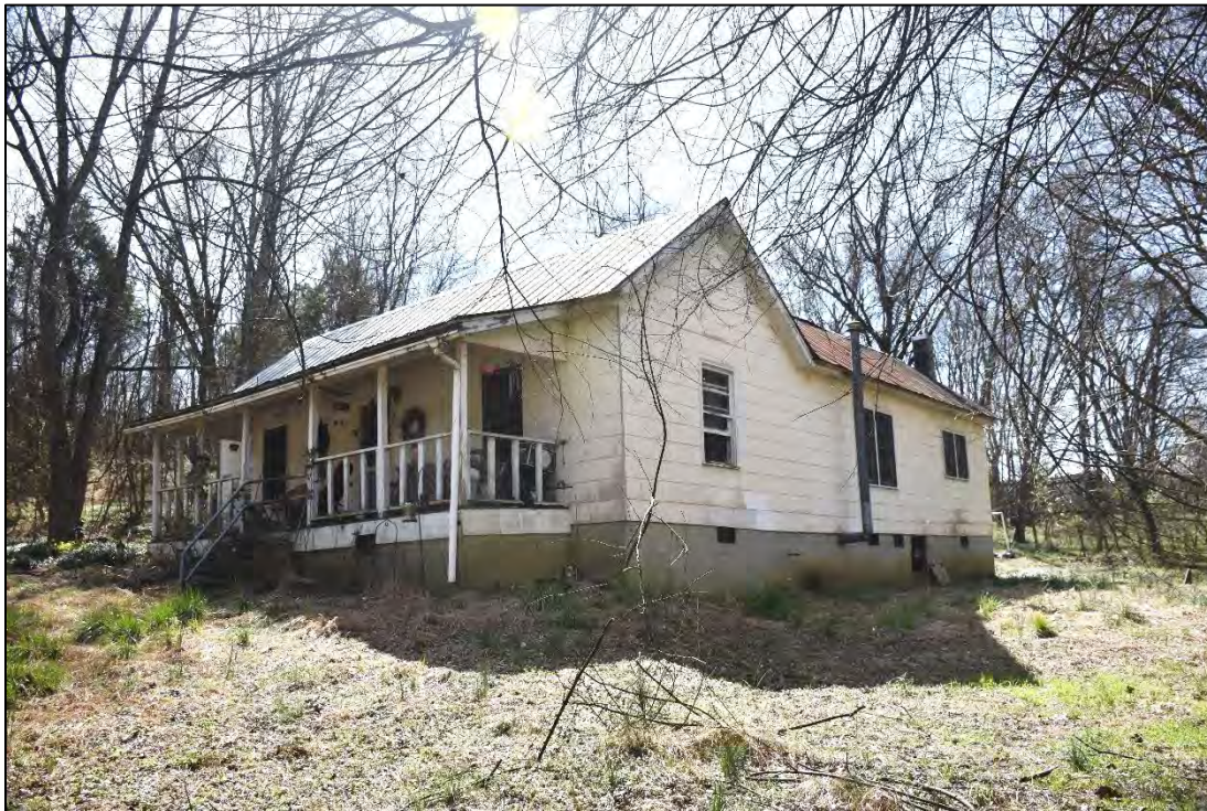
Figure 2.9. Henry Wallace House (CA0597), early-twentieth-century house, facing southeast.
