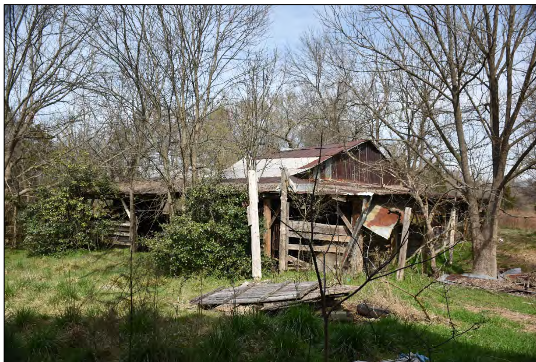
Figure 2.24. Henry Wallace House (CA0597), mid-twentieth-century agricultural building, facing southwest.
