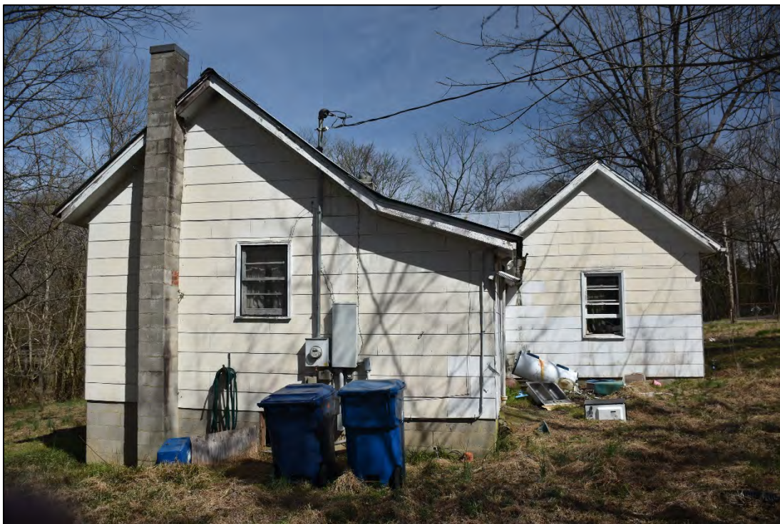
Figure 2.10. Henry Wallace House (CA0597), early-twentieth-century house, facing north.
