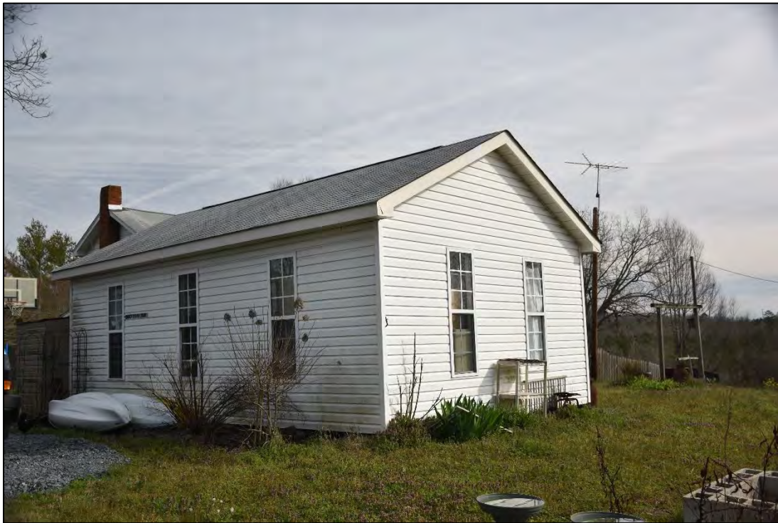
Figure 2.8. Small-Black House (CA1593), garage/workshop, facing northeast.
