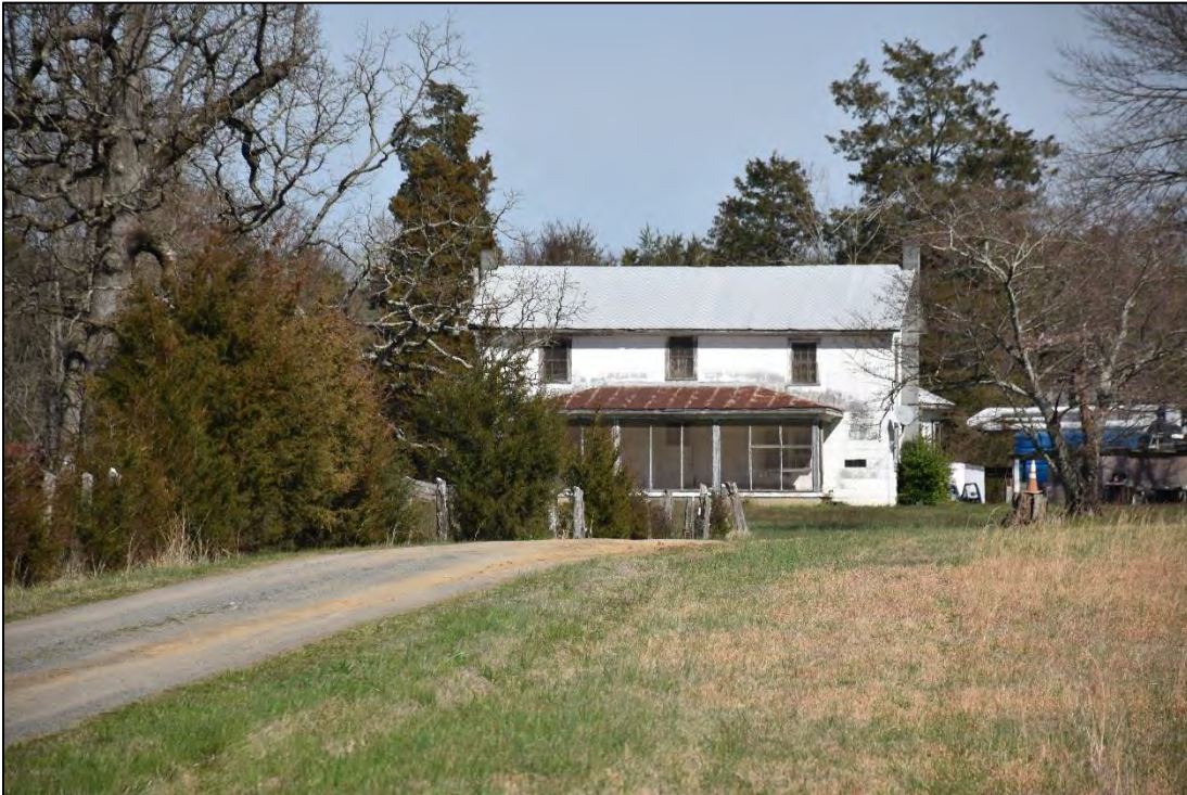
Figure 2.49. Unsurveyed House, 11475 Hickory Ridge Road, facing east.
