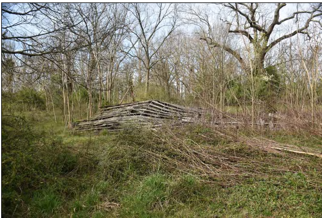
Figure 2.12. Small-Black House (CA1593), remains of a wooden outbuilding, facing west.
