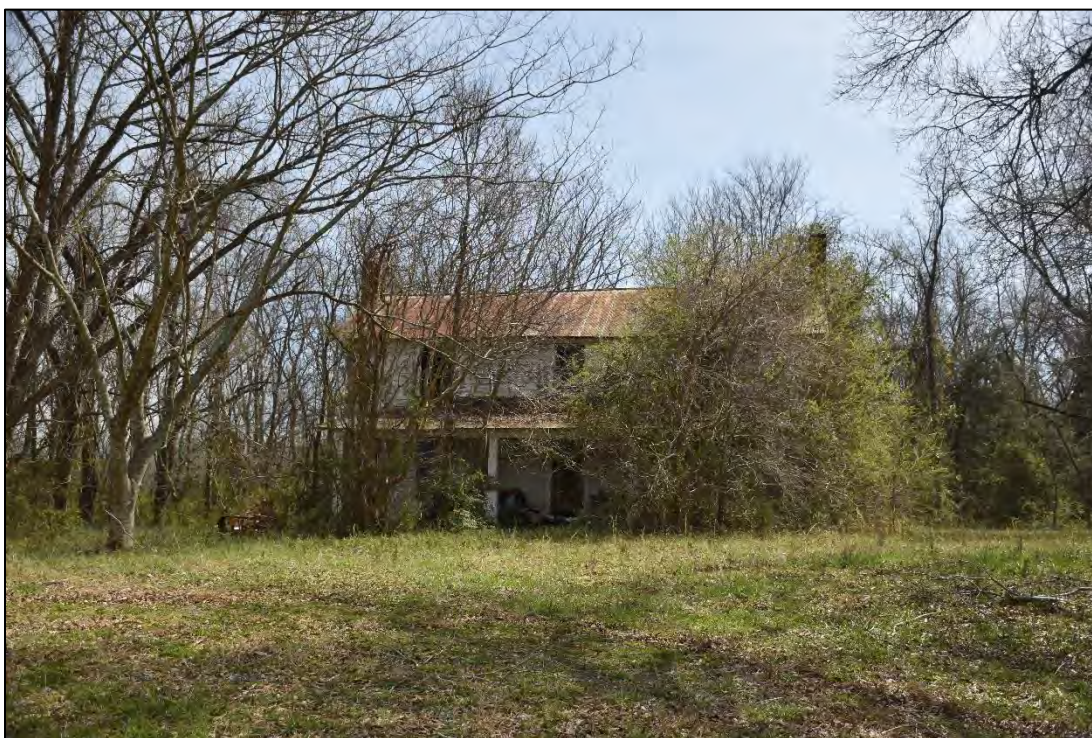
Figure 2.47. Sehorn Small Farm (CA0547), facing southeast.
