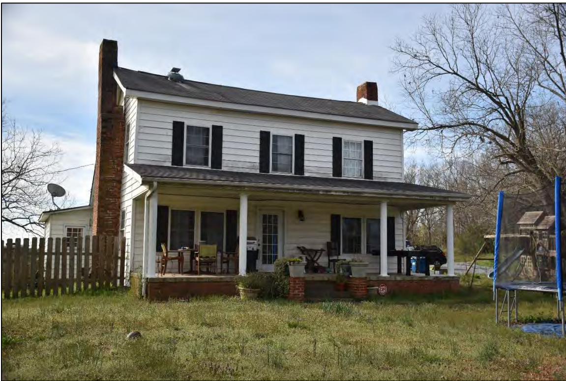
Figure 2.1. Small-Black House (CA1593), house, facing south.
