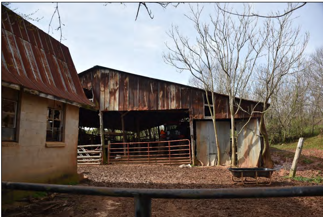
Figure 2.20. Small-Black House (CA1593), livestock barn, facing southwest.
