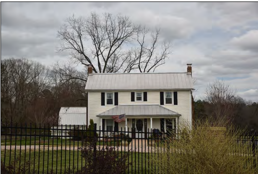
Figure 2.50. Unsurveyed House, 7051 Bost Cutoff Road, facing north.
