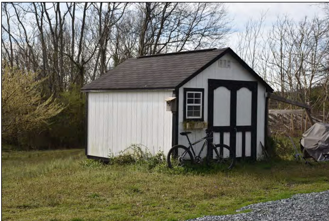
Figure 2.10. Small-Black House (CA1593), late-twentieth-century shed, facing south.
