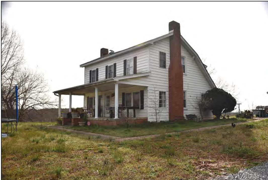
Figure 2.3. Small-Black House (CA1593), house, facing southeast.
