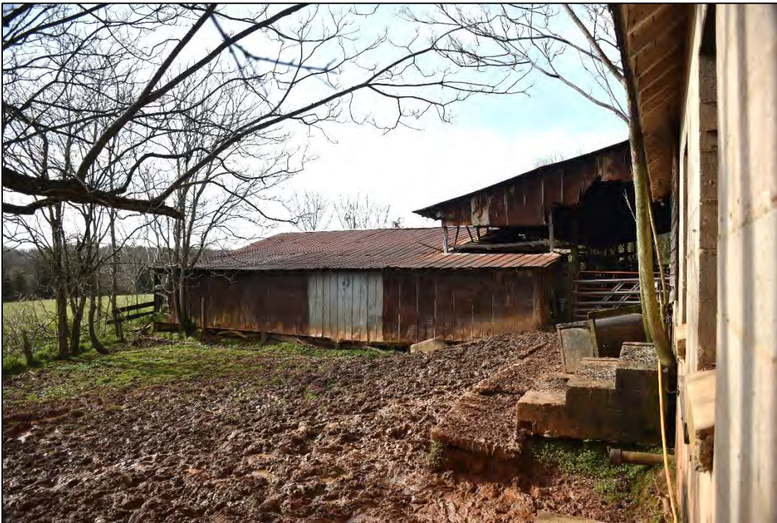
Figure 2.21. Small-Black House (CA1593), livestock barn, facing south.
