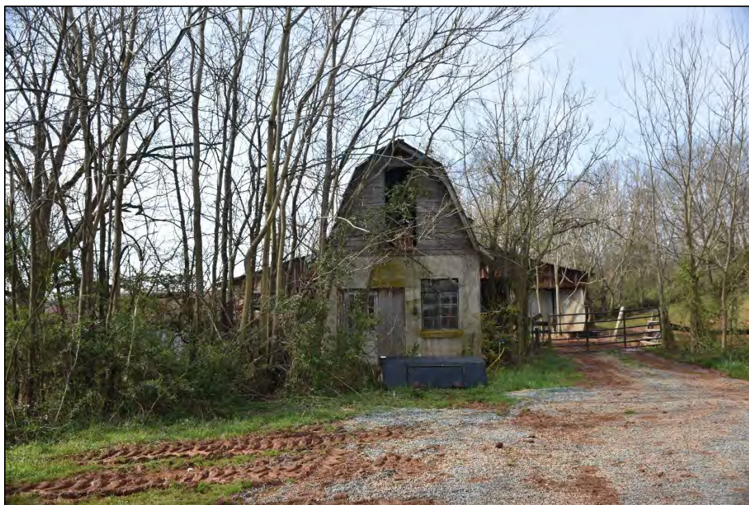
Figure 2.18. Small-Black House (CA1593), dairy barn, facing southwest.
