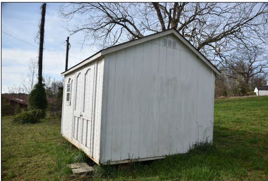
Figure 2.14. Small-Black House (CA1593), twenty-first-century shed, facing south.
