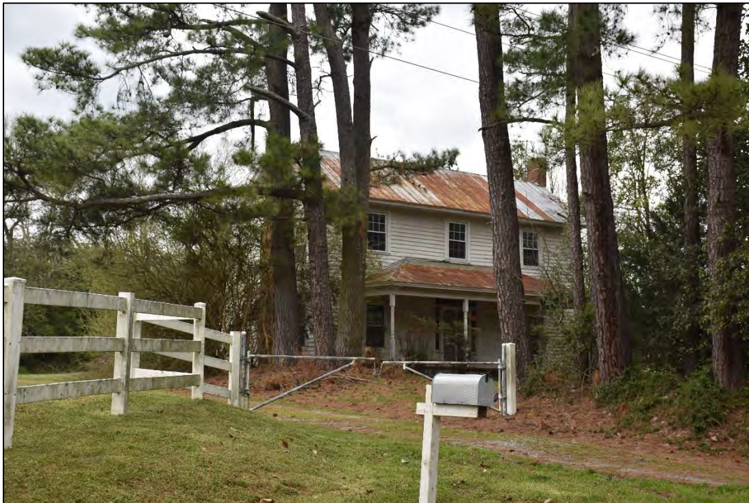
Figure 2.43. Unnamed House (CA0433), facing northwest.
