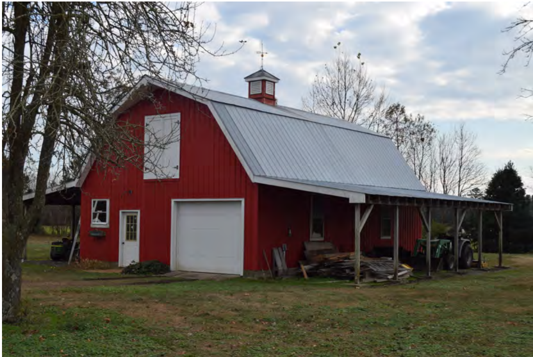
Modern barn and workshop, view to the southeast
