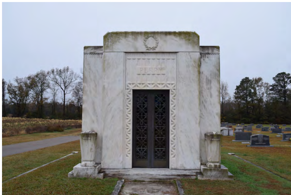
Perry Mausoleum, view to the west
