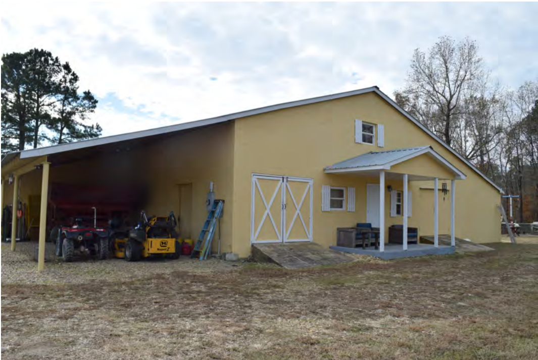
Mule barn, view to the southwest
