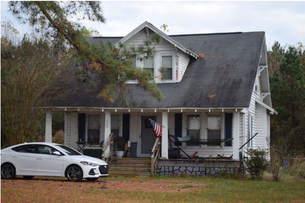
Facade, view to the east
