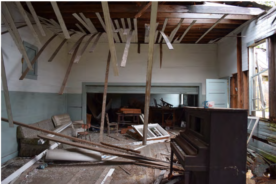
Interior, view to the north-northeast
