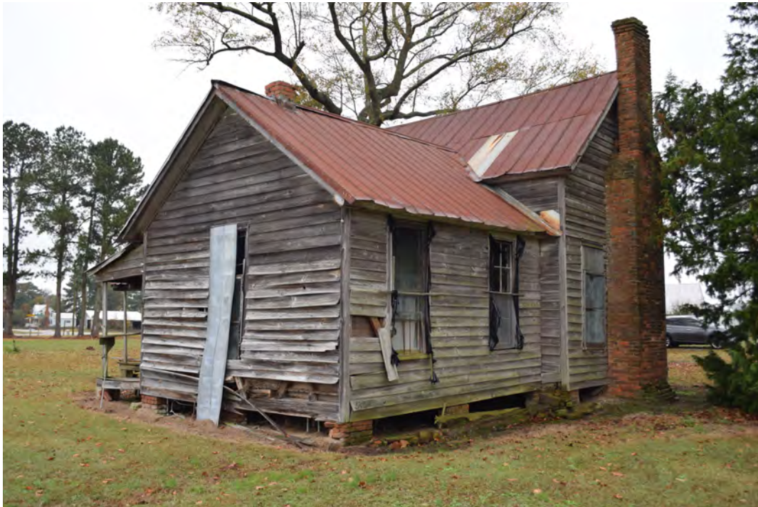
Northeast corner, view to the southwest
