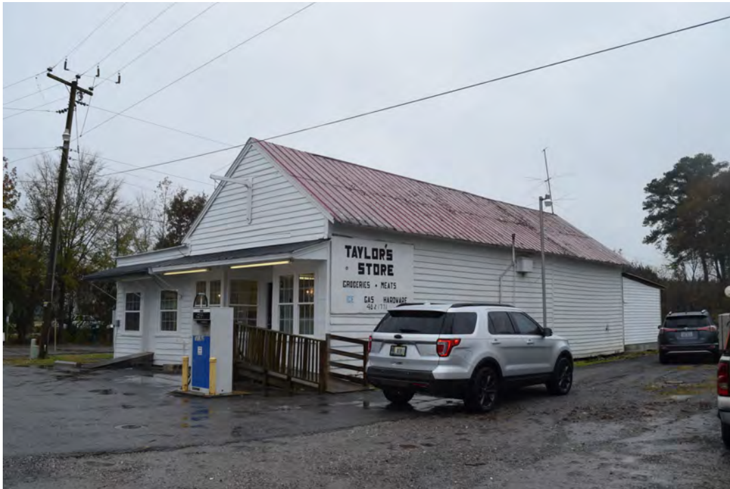
Front (northeast) corner, view to the southwest
