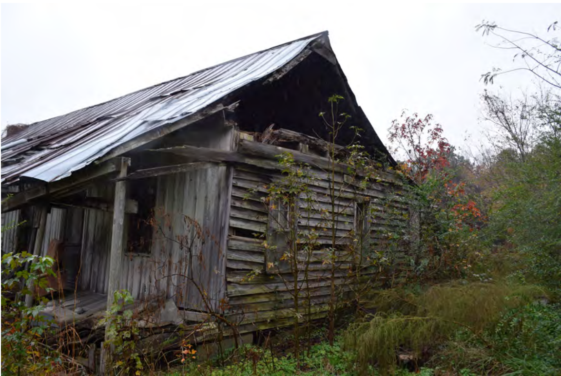
North gable end, view to the southwest
