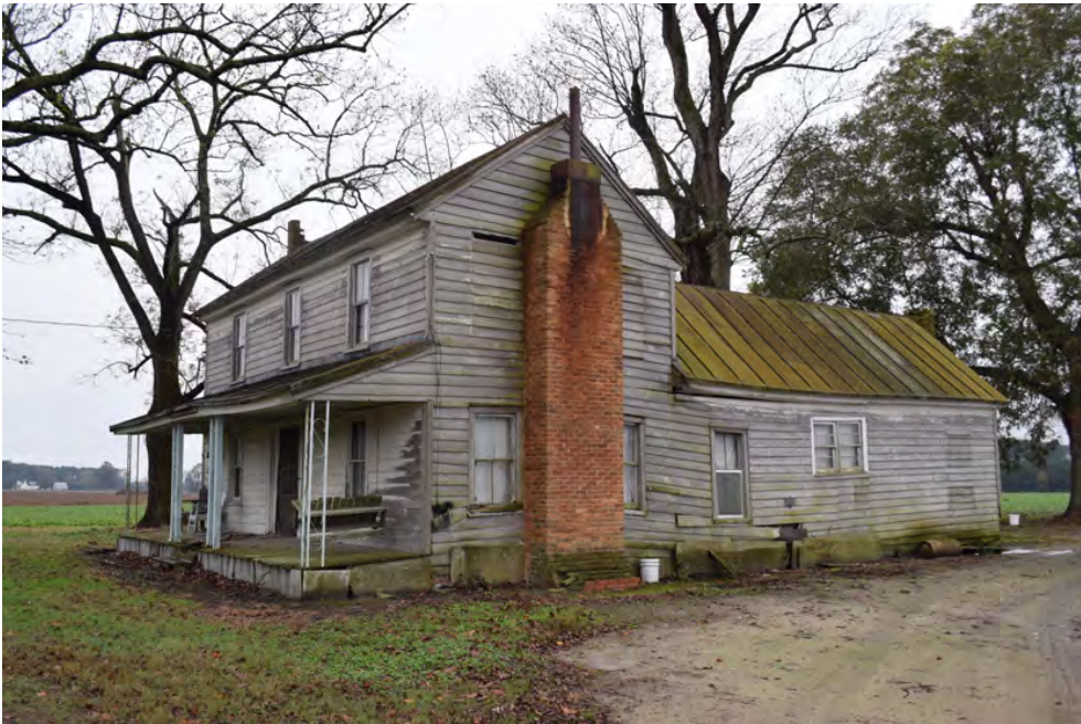
Northeast corner, view to the southwest
