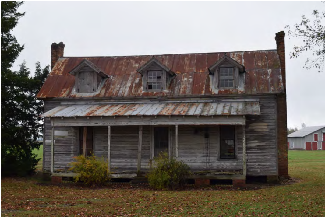
Facade, view to the east
