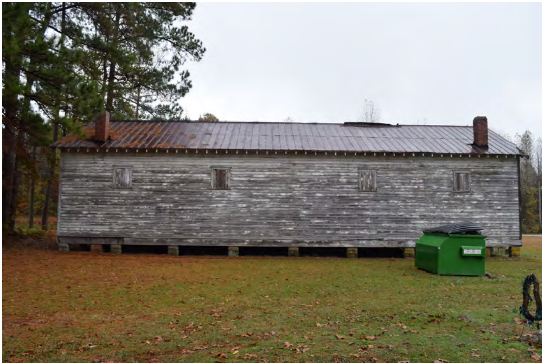
Rear elevation, view to the east-southeast
