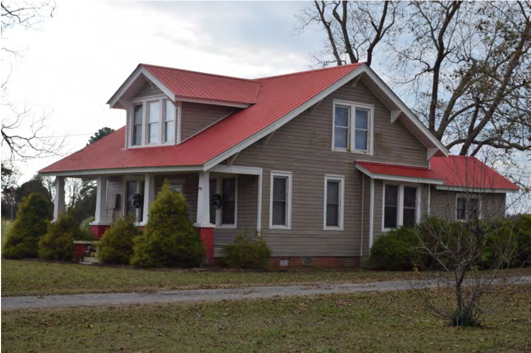
Northeast (front) corner, view to the southwest
