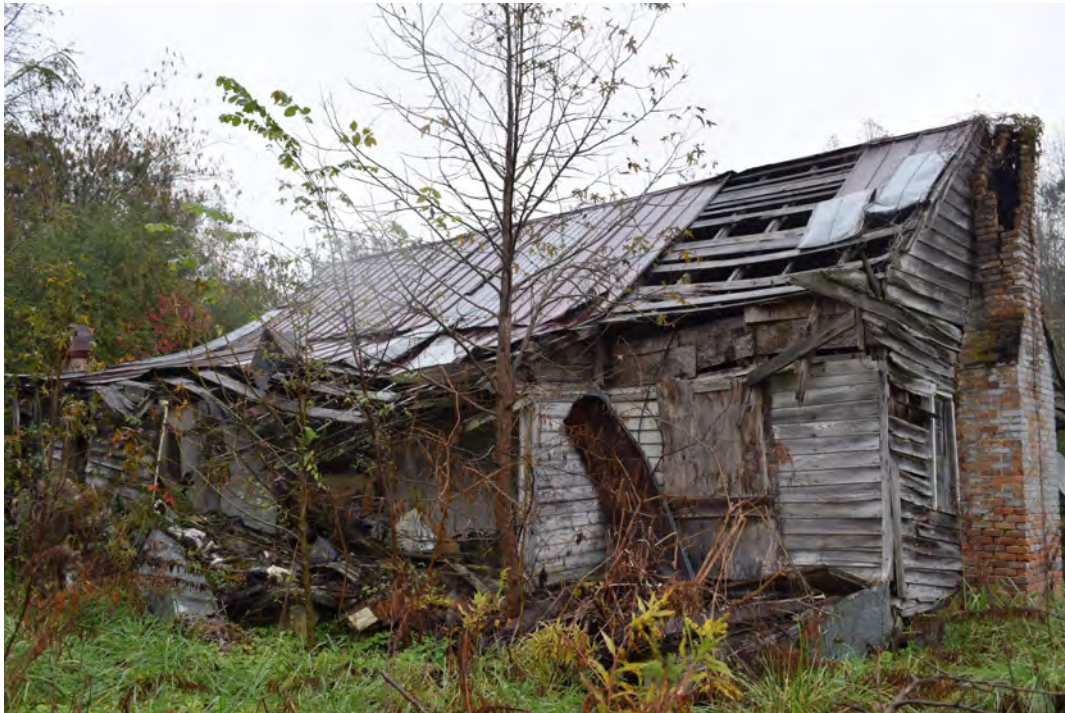
Rear elevation, view to the east-northeast
