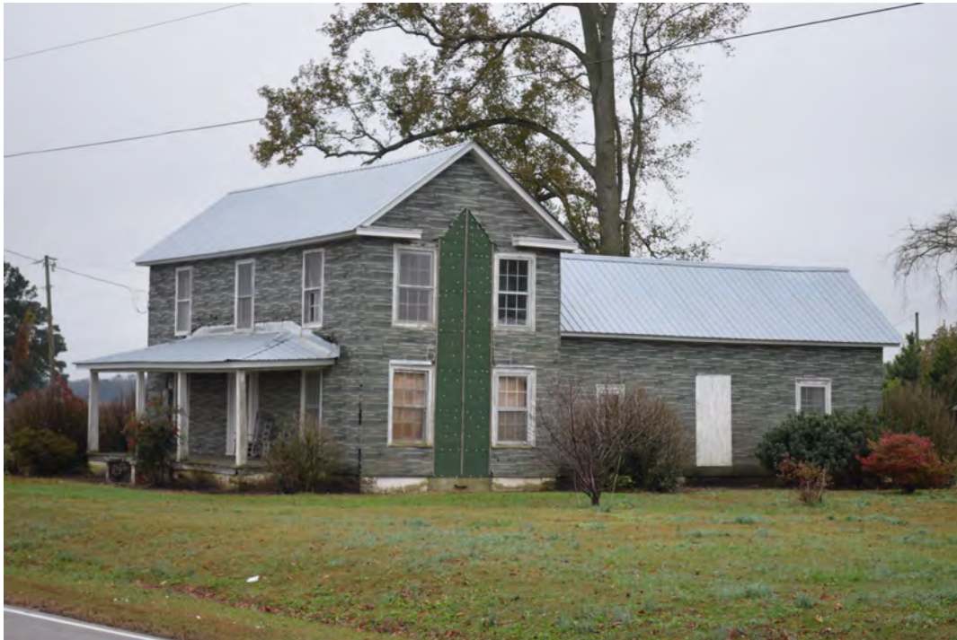
Northeast corner, view to the southwest
