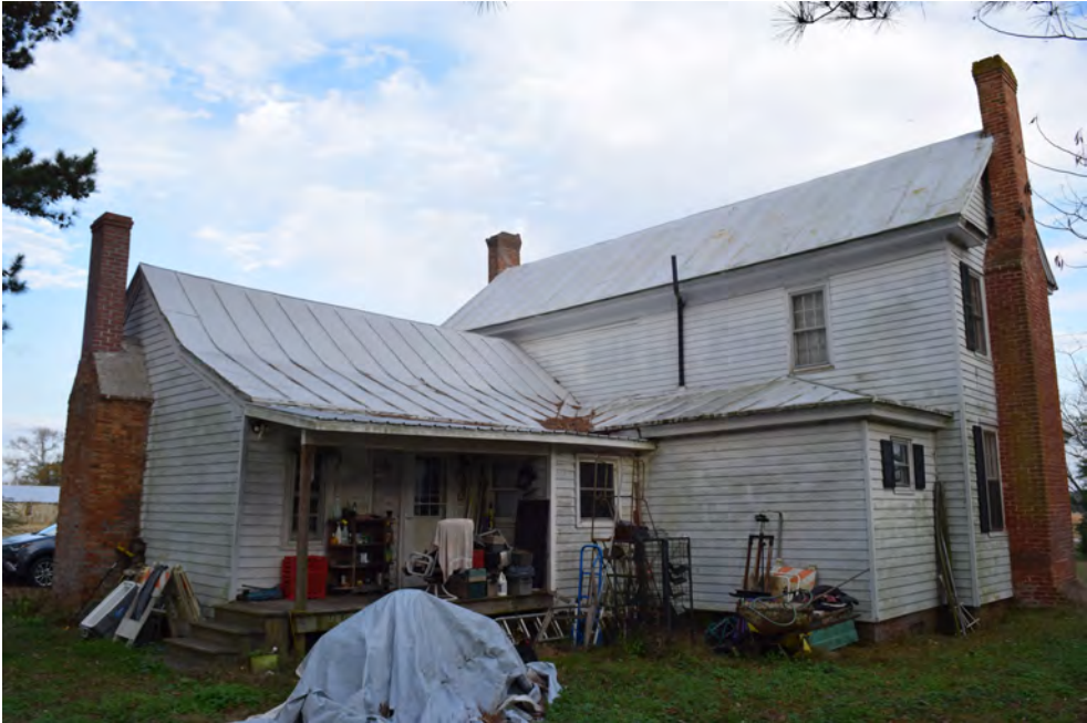
Southwest (rear) corner, view to the northeast
