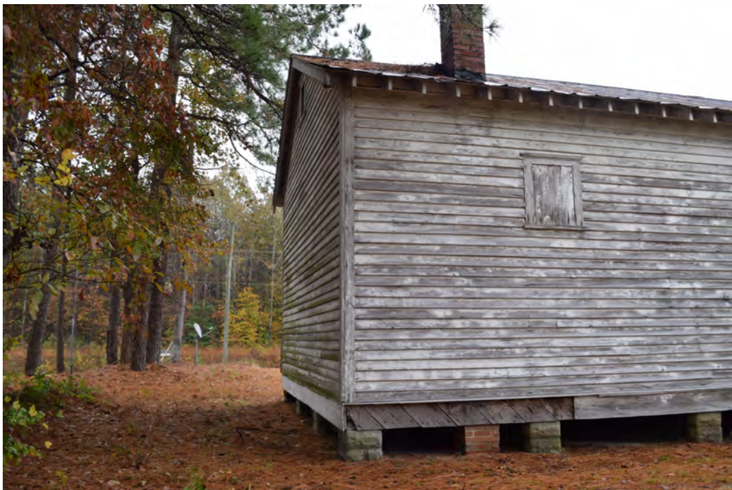
North gable end, view to the east
