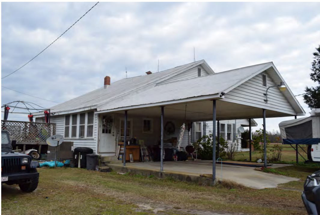
Southwest (rear) corner showing carport addition, view to the northeast
