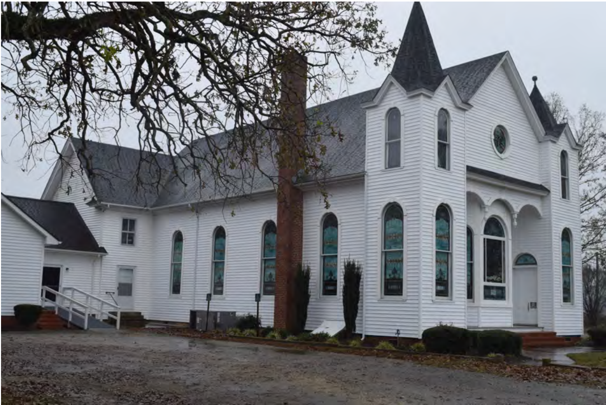
Northeast corner, view to the southwest
