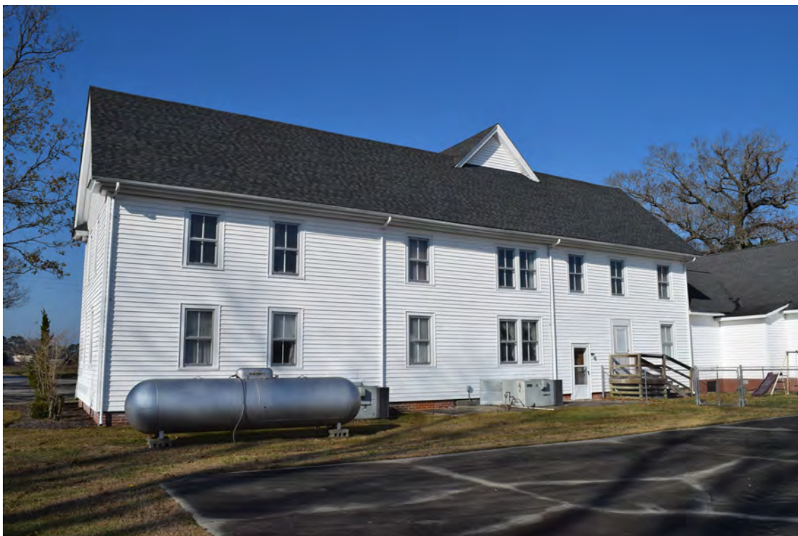
Rear of 1927 classroom wing, view to the north-northeast
