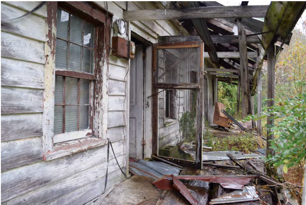
Front porch, view to the north-northwest
