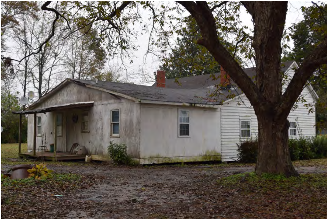
Southwest (rear) corner, view to the northeast
