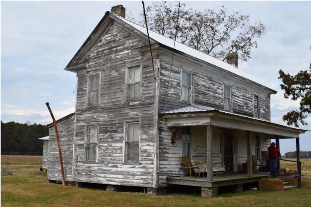
Southeast (front) corner, view to the northwest
