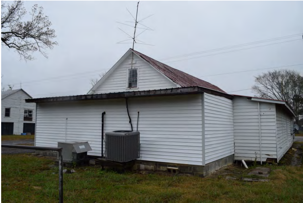
Nearly flat-roofed addition on rear, view to the northeast
