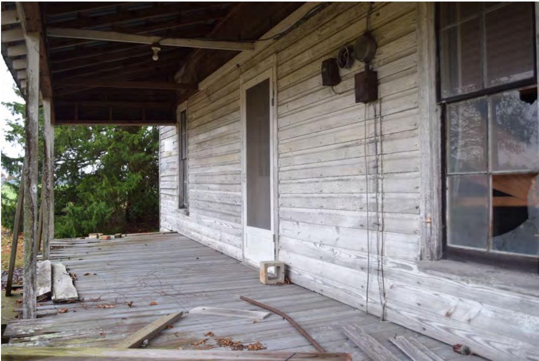
Detail of front porch, view to the north-northeast
