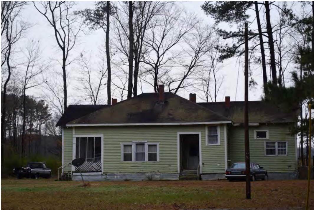
St. Francis School (BR1123) view to the south
