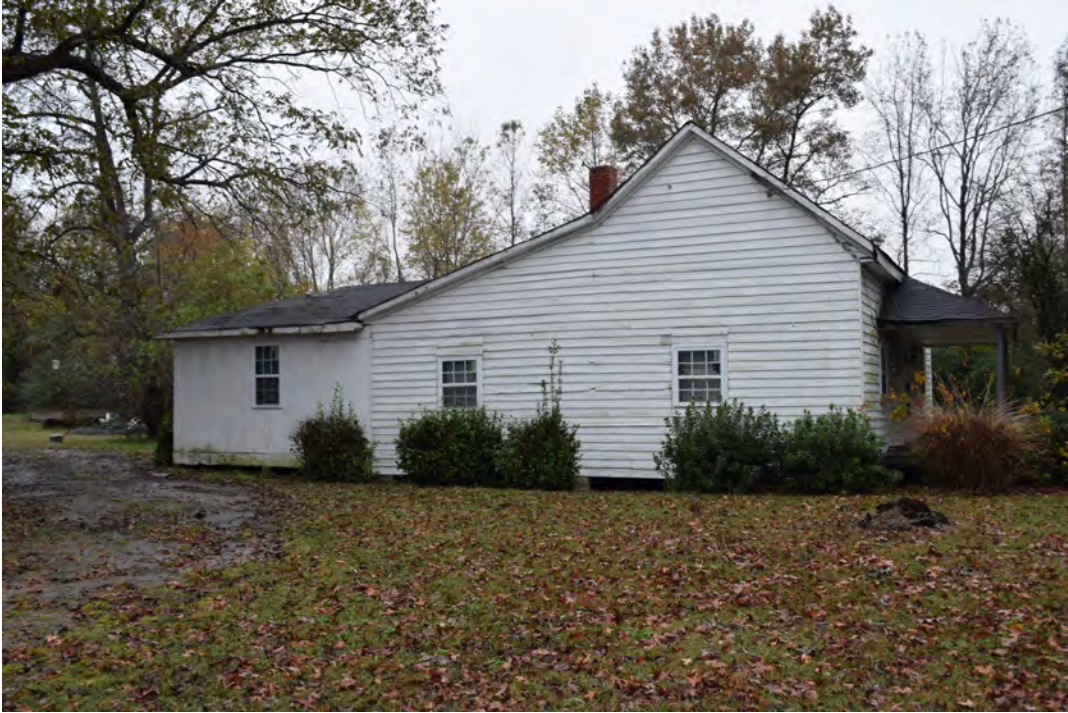
South (side) elevation, view to the north
