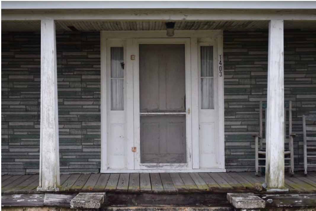
Front door, view to the west-northwest
