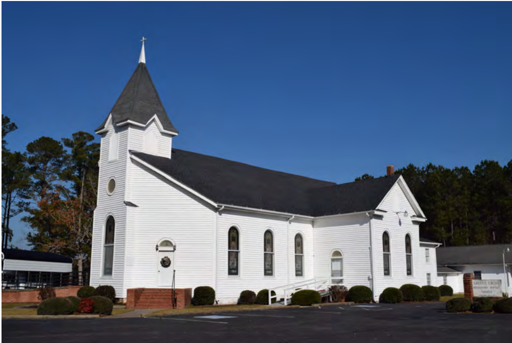
Greens Cross Missionary Baptist Church (BR0174), view to the north-northwest
