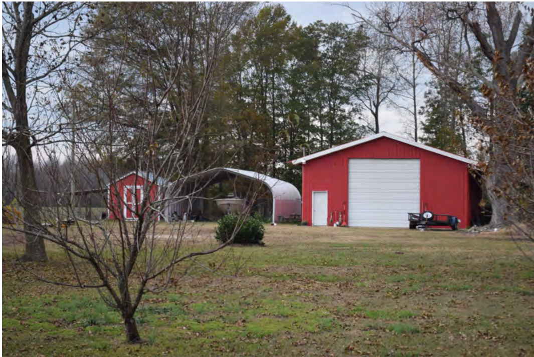
Three outbuildings in rear yard, view to the west
