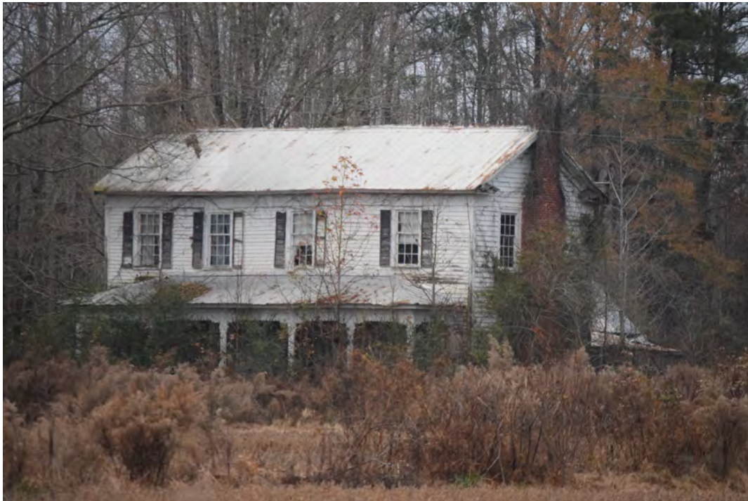
Taylor-Simmons House, view to the northeast
