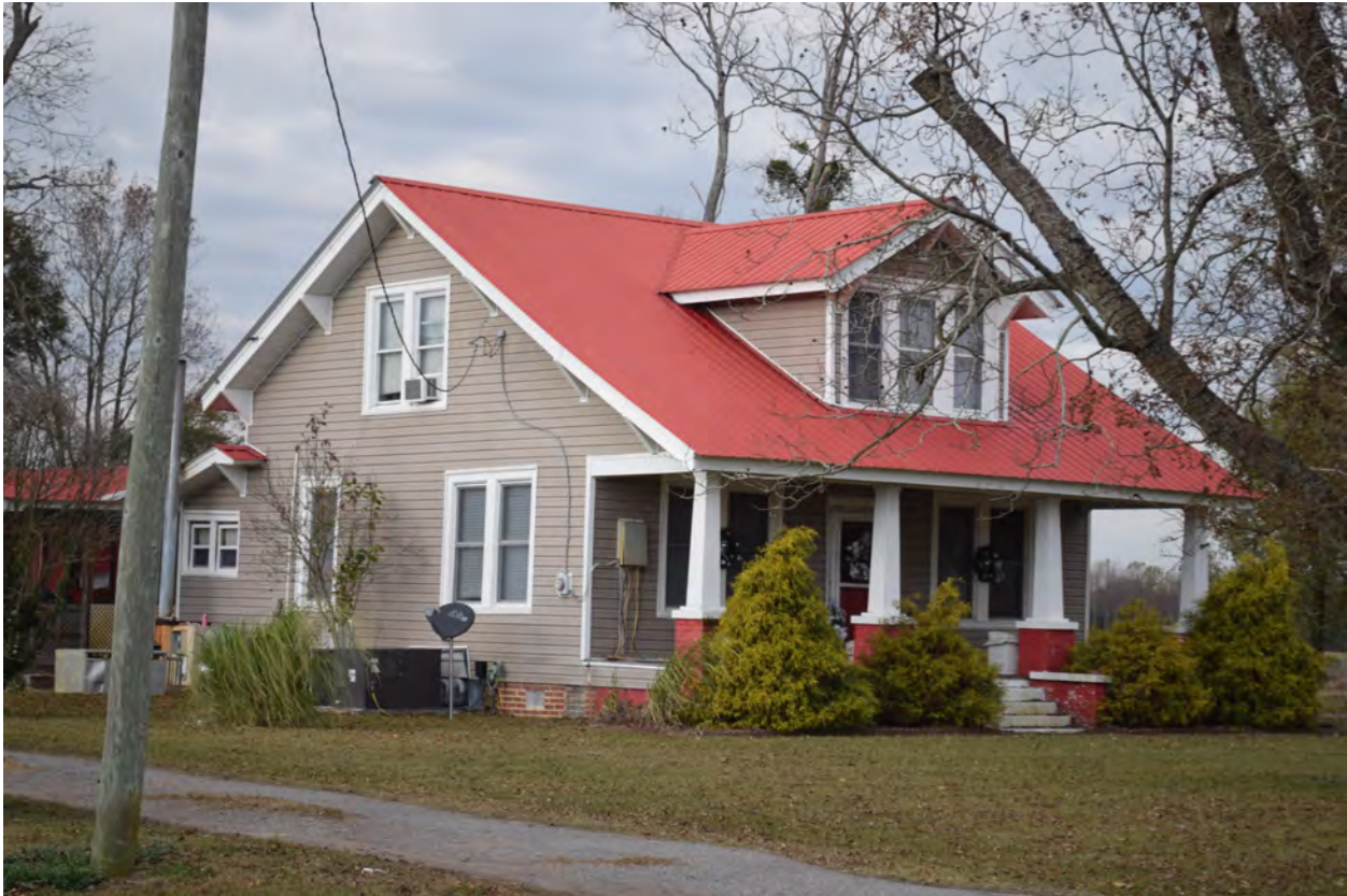
Southeast (front) corner, view to the northwest
