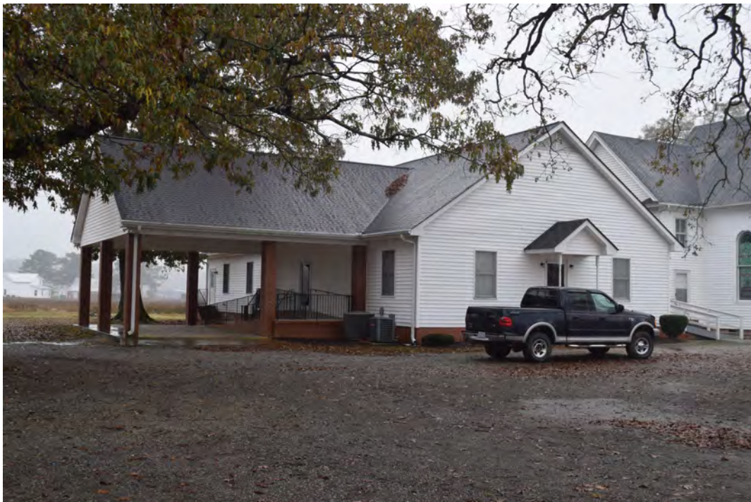
1964 addition and carport, view to the south-southwest
