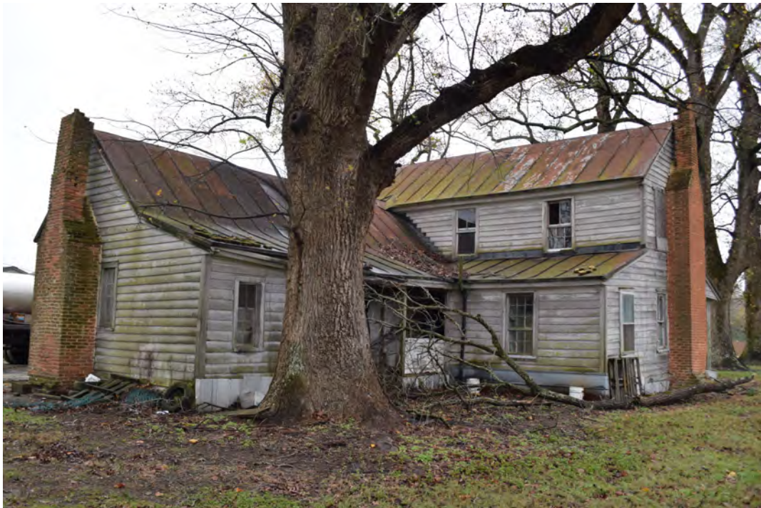
Southwest (rear) corner, view to the northeast
