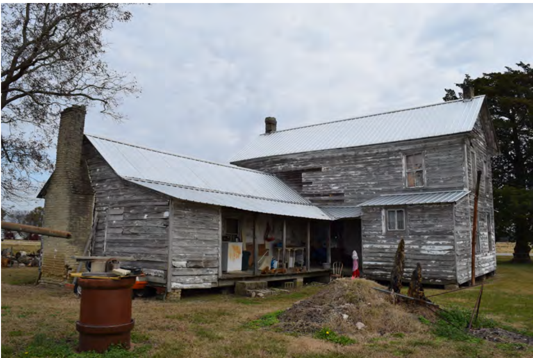
Southwest corner, view to the northeast
