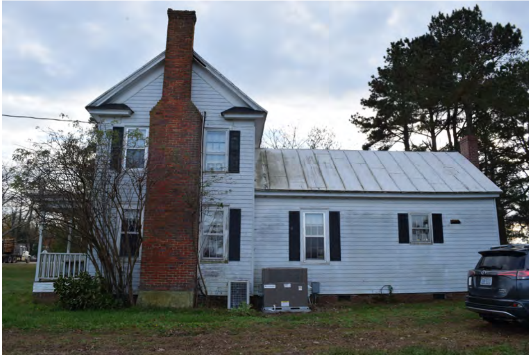
North gable end, view to the south
