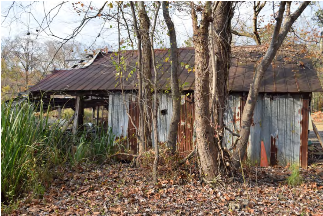
Guy Smith fish house, south elevation, view north-northwest
