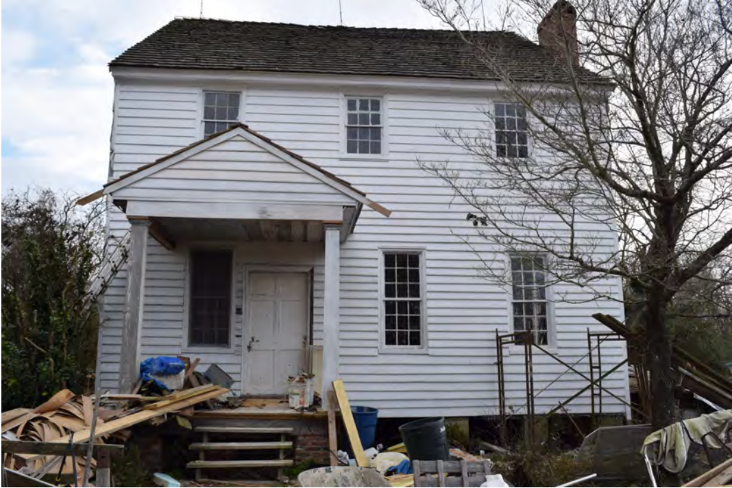
Facade, view to the east
