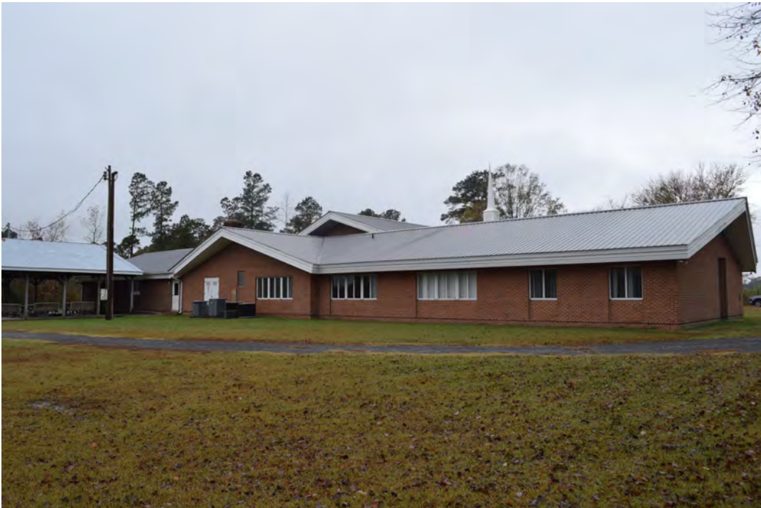
Rear of north wing and portion of 1990 picnic shelter, view to the southwest
