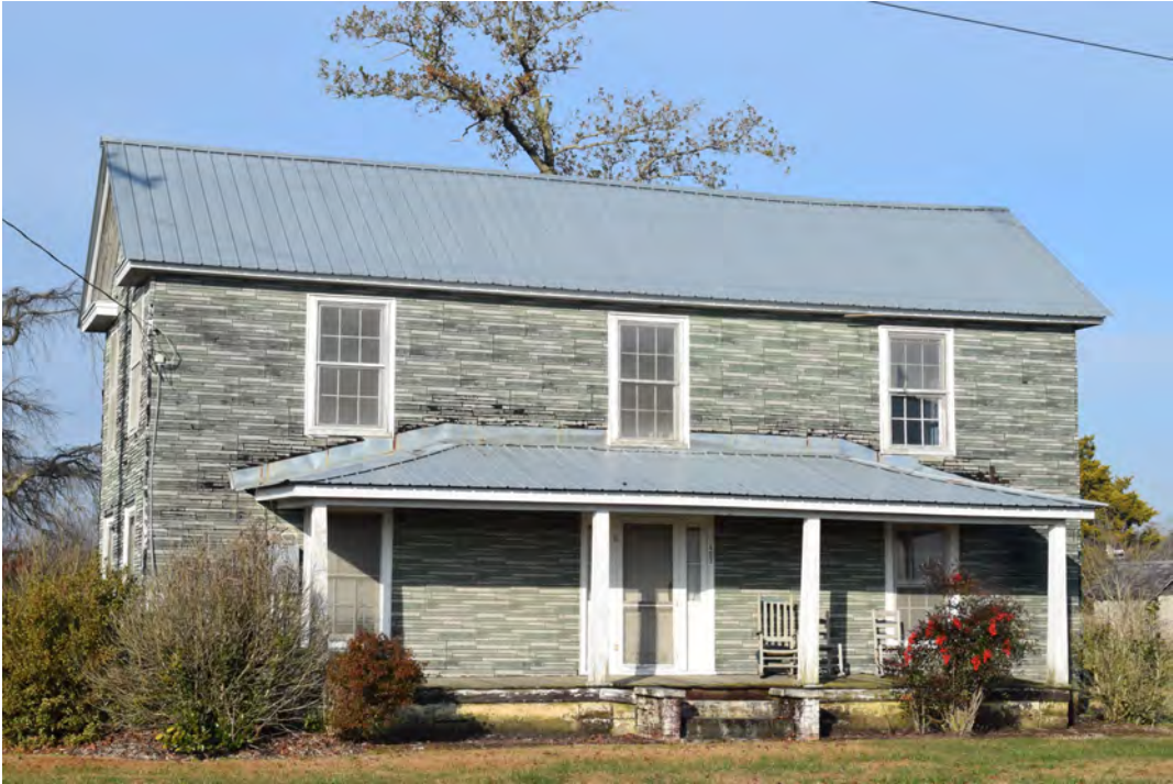
Facade, view to the west-northwest
