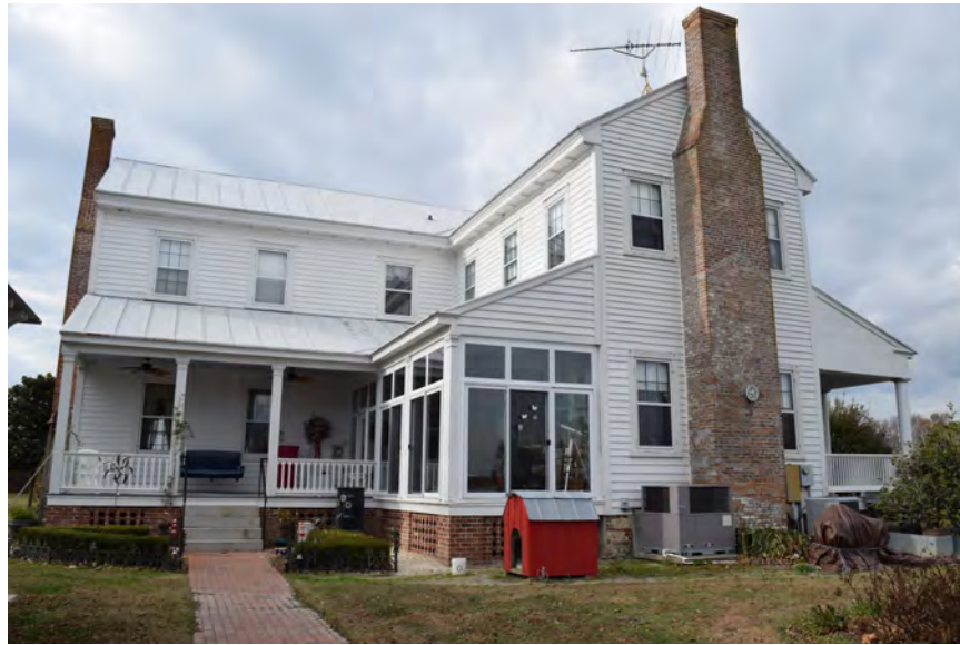
Rear elevation, view to the west
