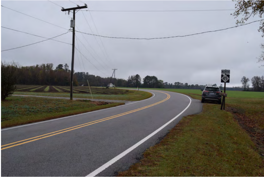
One of the few curves in NC 45 in the project area, near its intersection with Mount Gould River Road, view to the north
