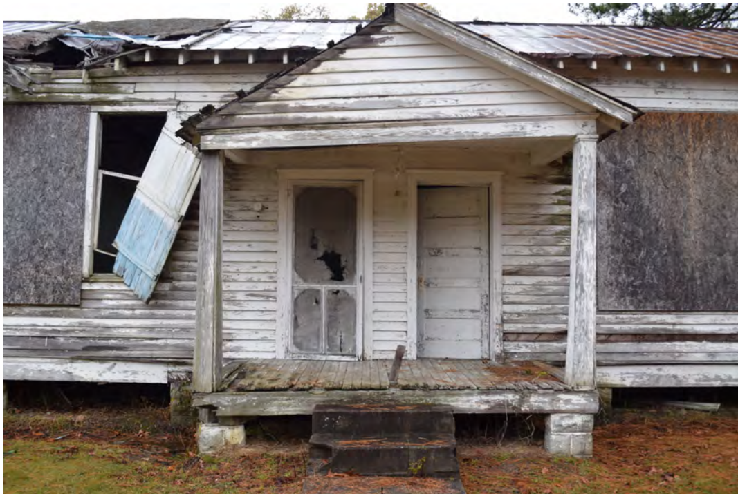
Detail of front portico, view to the west-northwest
