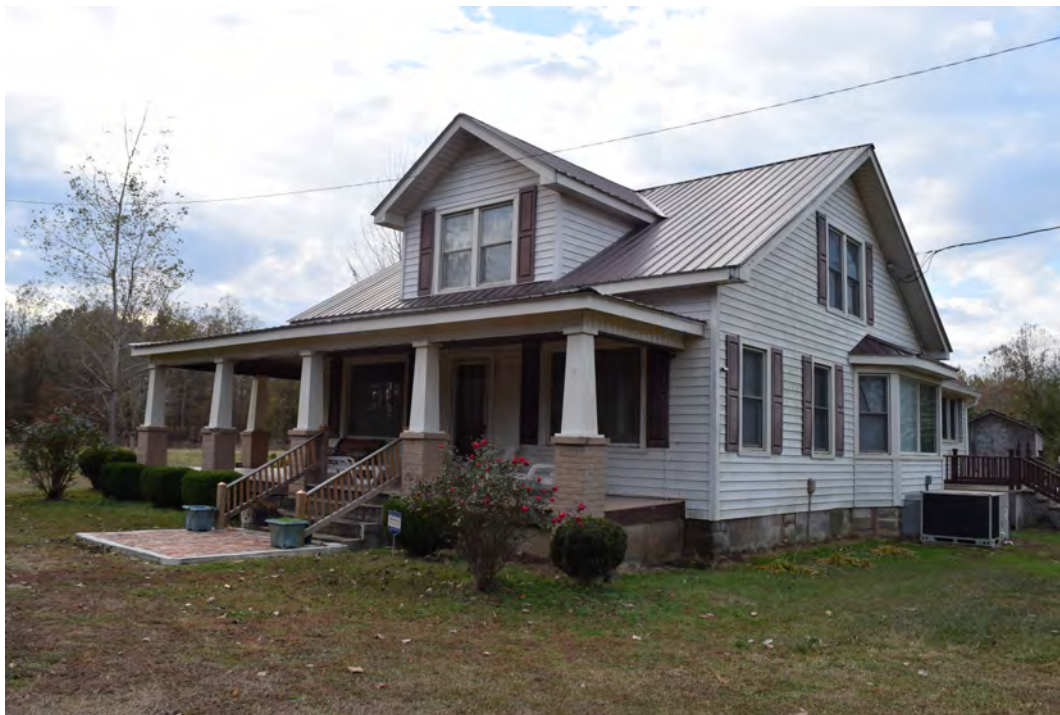
Southeast corner, view to the northwest
