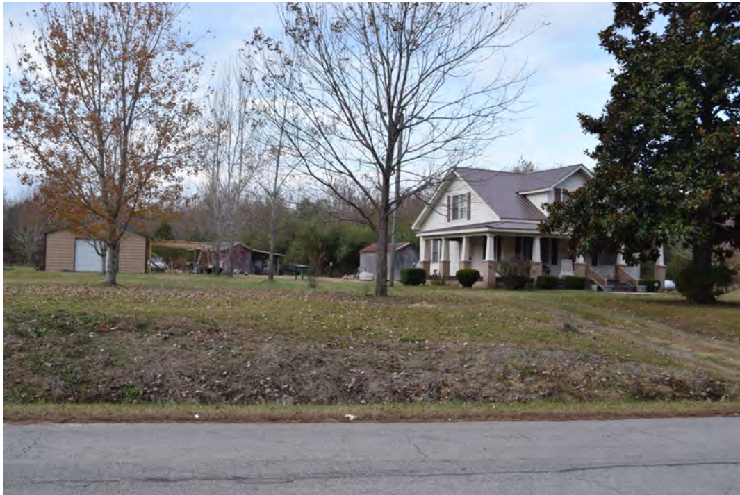
Southwest corner of the dwelling and outbuildings, view to the north-northeast
