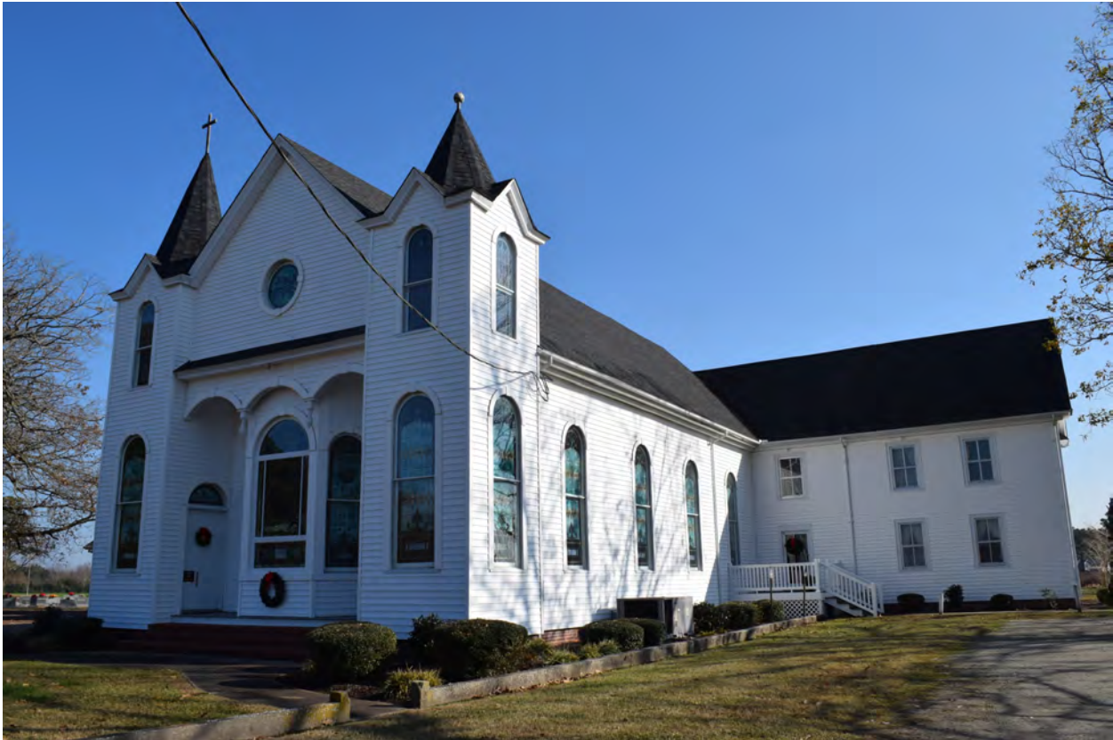
Front (northwest) corner, view to the south-southeast
