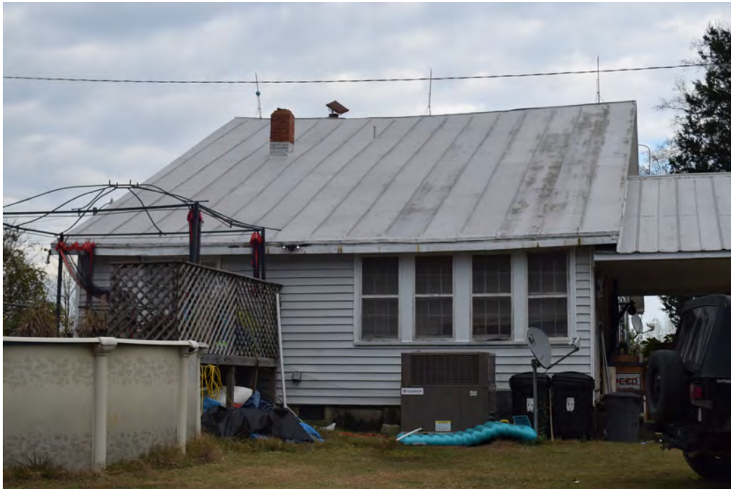
West (rear) elevation, view to the east
