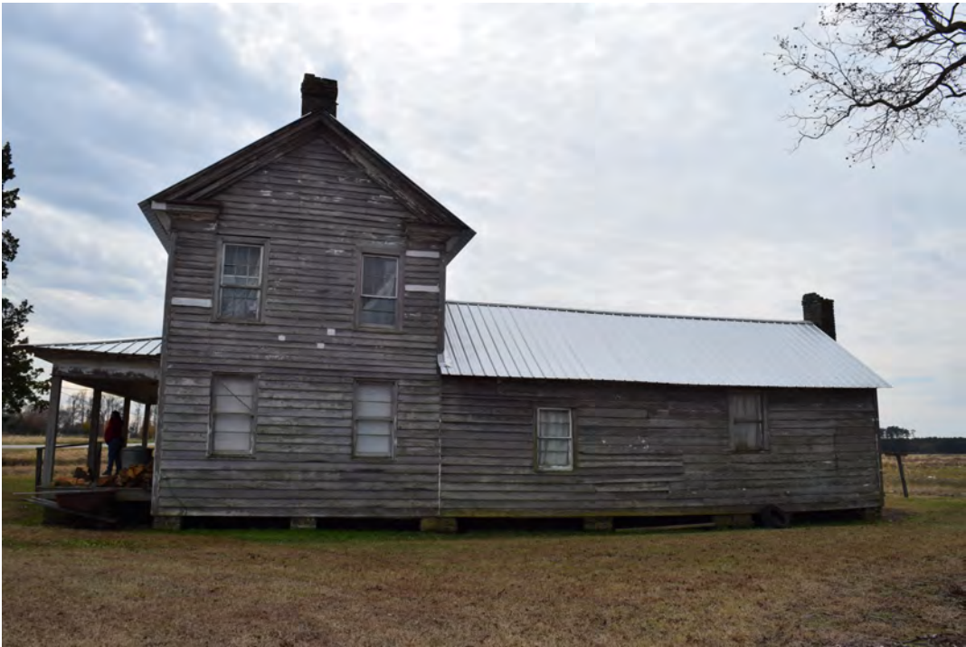
North gable end, view to the south
