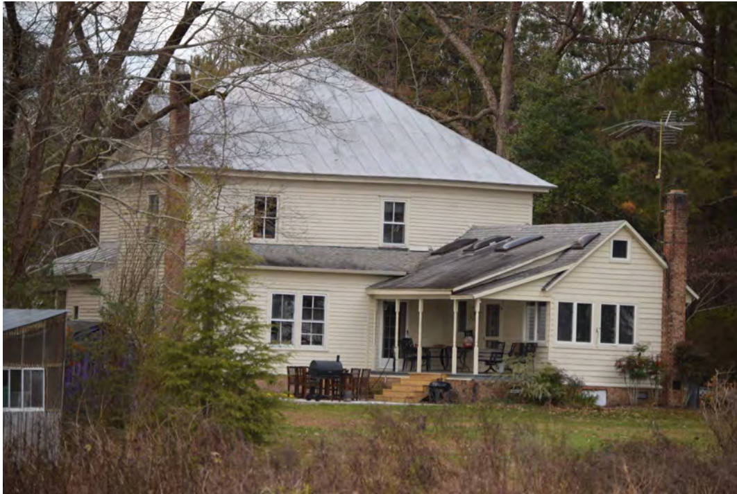
Southeast (rear) elevation, view to the north-northwest
