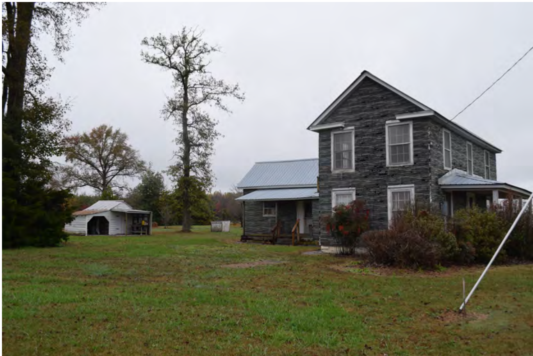
South elevation and outbuilding, view to the northwest
