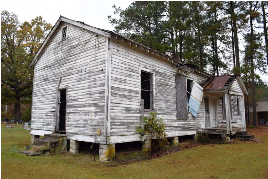
Southeast (front) corner, view to the northwest
