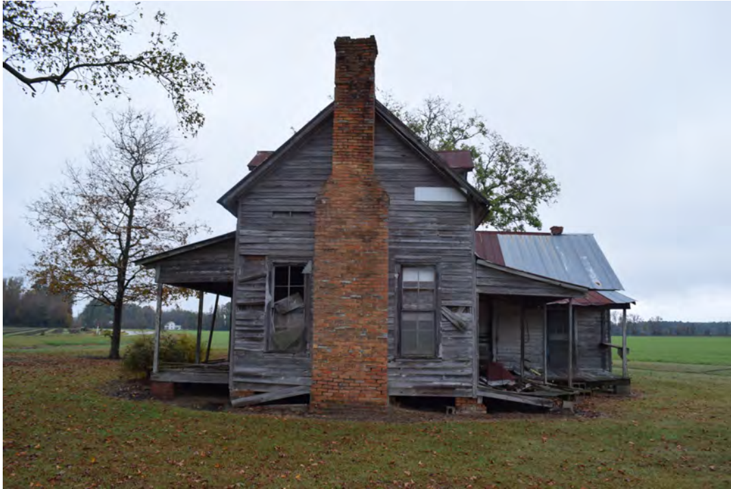
South gable end, view to the north
