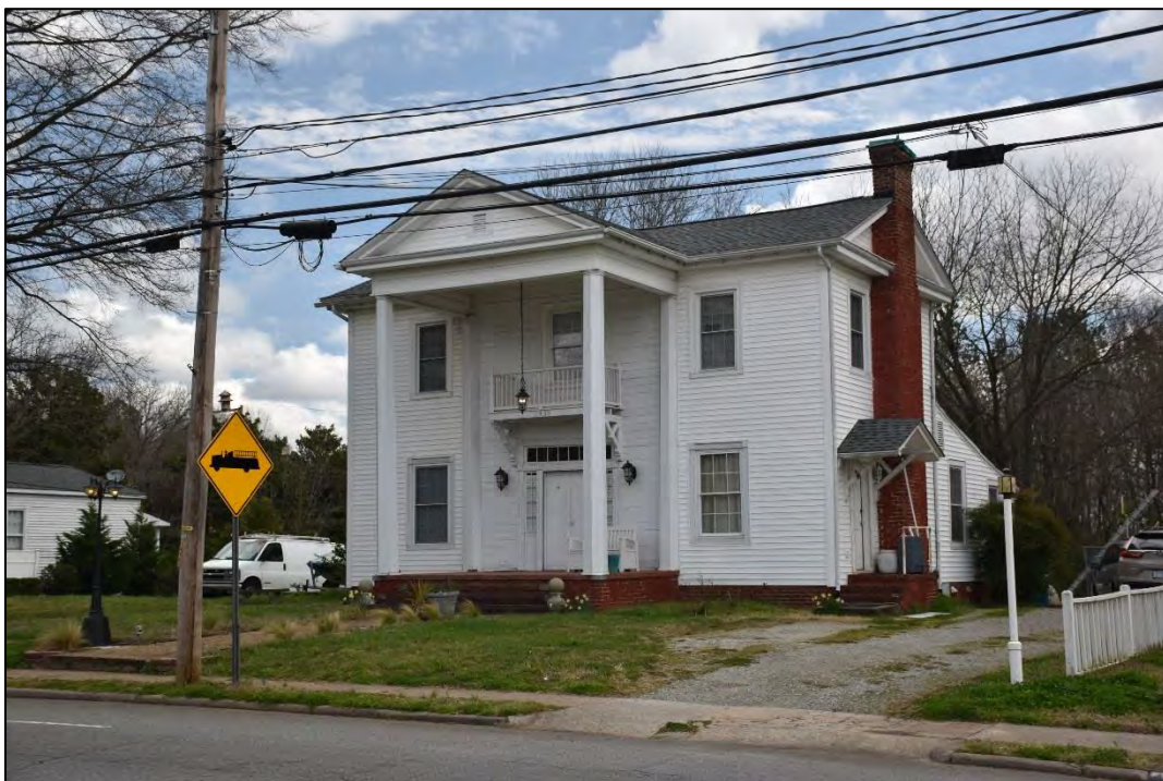
Figure 2.43. Matthew Cook House (CA0156), facing northeast.
