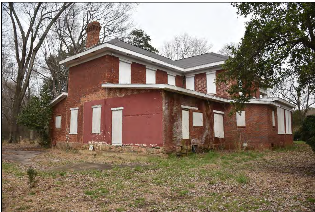
Figure 2.5. Boxwood Manor House (CA0322), house, facing northeast.
