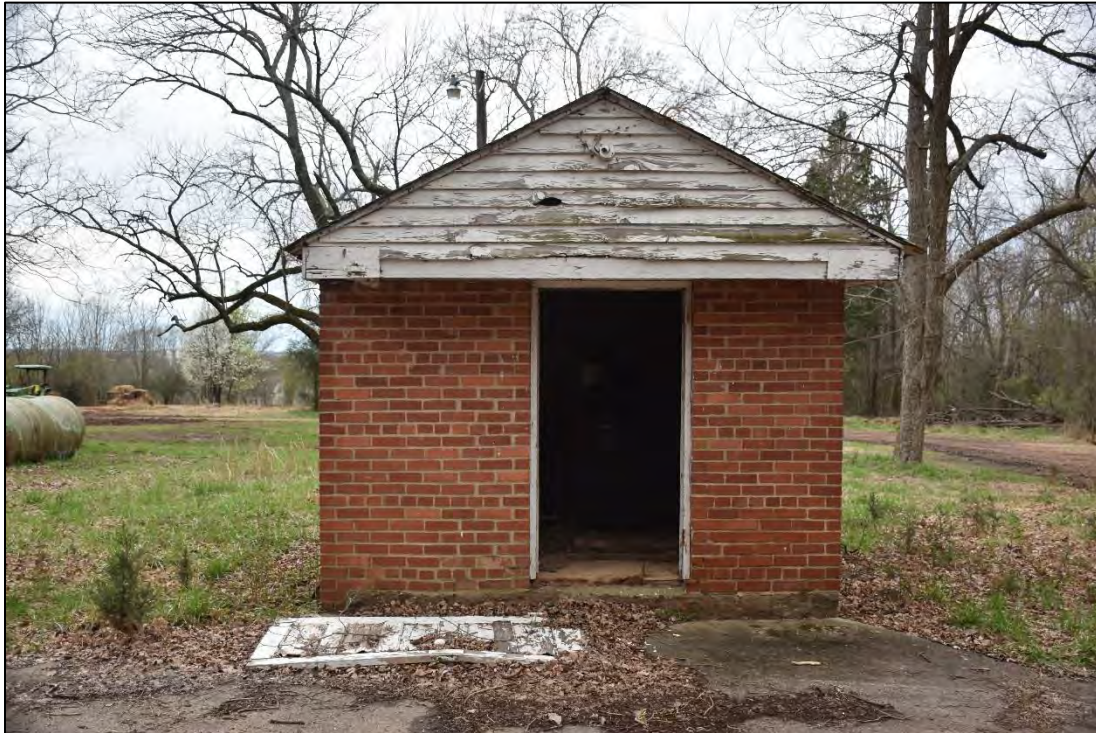
Figure 2.12. Boxwood Manor (CA0322), circa-1850/1910 dairy/well house, facing west.
