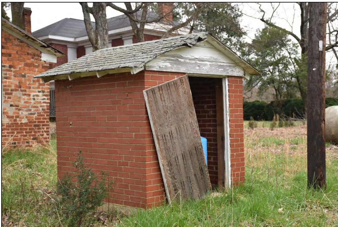
Figure 2.15. Boxwood Manor (CA0322), circa 1930 pump house, facing southeast.
