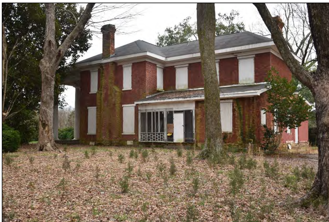
Figure 2.7. Boxwood Manor House (CA0322), house, facing southeast.
