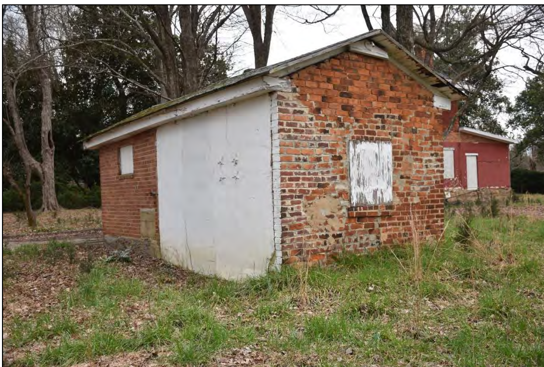
Figure 2.10. Boxwood Manor (CA0322), circa-1850/1910 dairy/well house, facing southeast.
