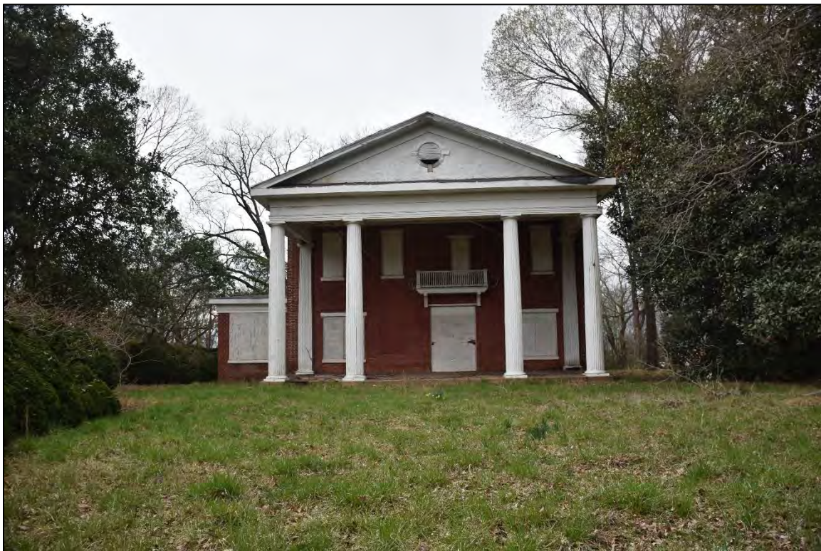
Figure 2.1. Boxwood Manor House (CA0322), house, facing west.
