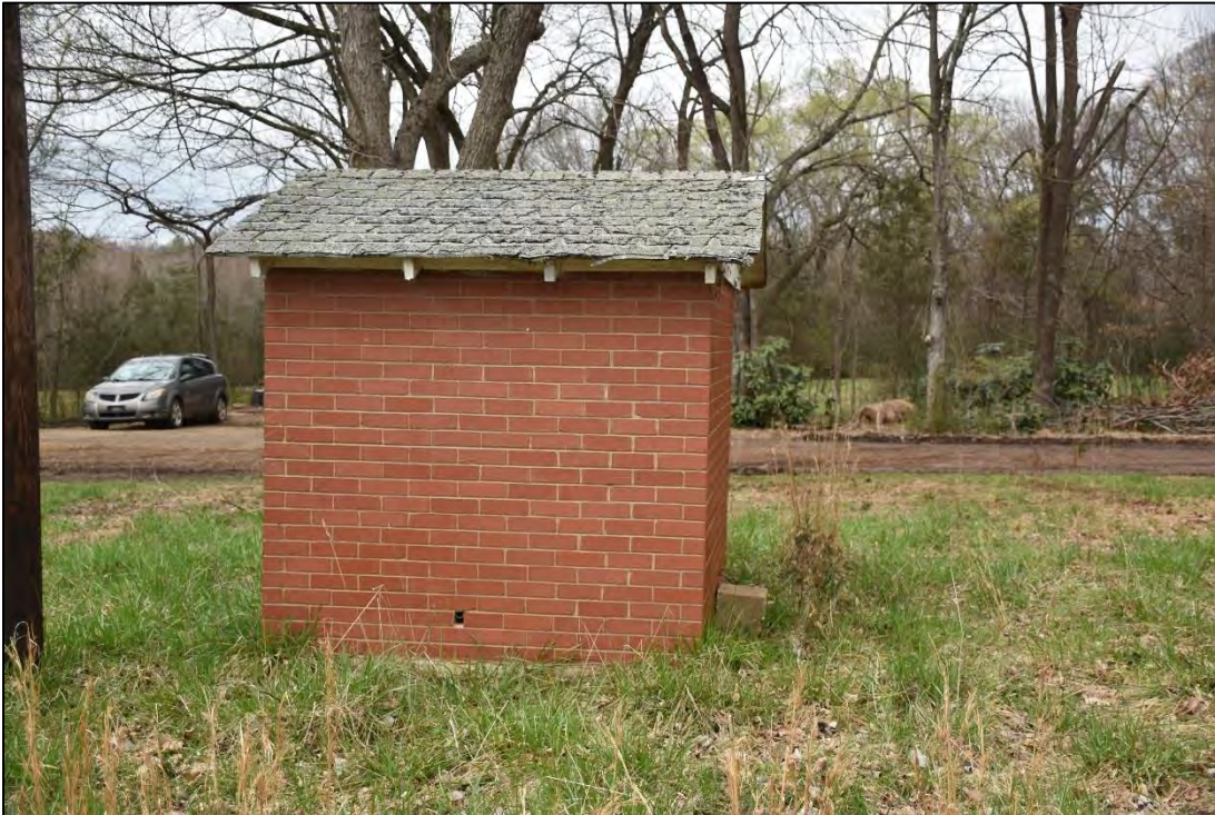
Figure 2.16. Boxwood Manor (CA0322), circa 1930 pump house, facing north.
