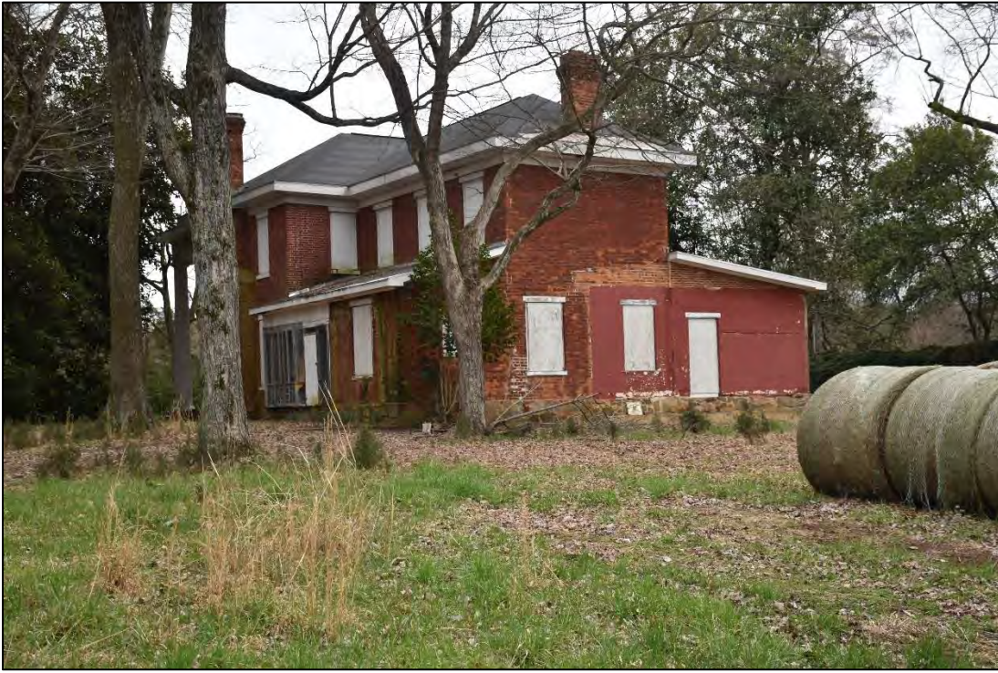
Figure 2.6. Boxwood Manor House (CA0322), house, facing southeast.
