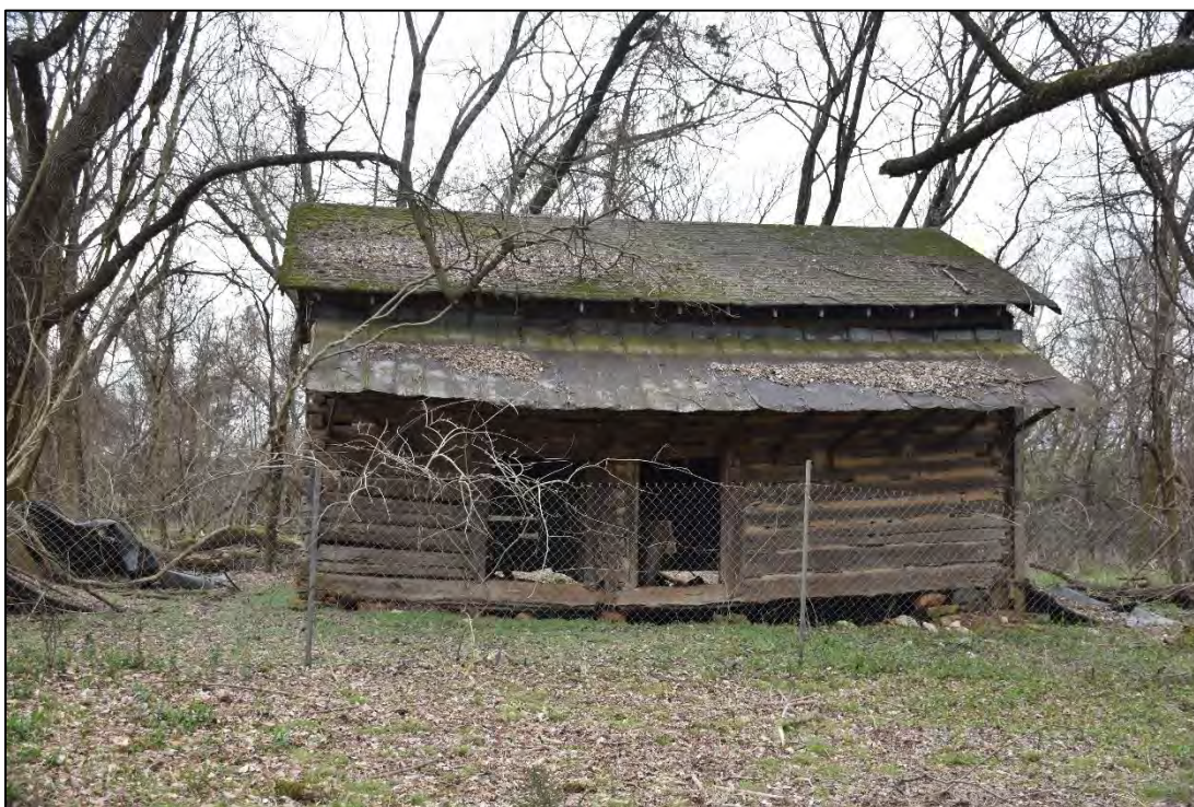
Figure 2.17. Boxwood Manor House (CA0322), log outbuilding, facing south.
