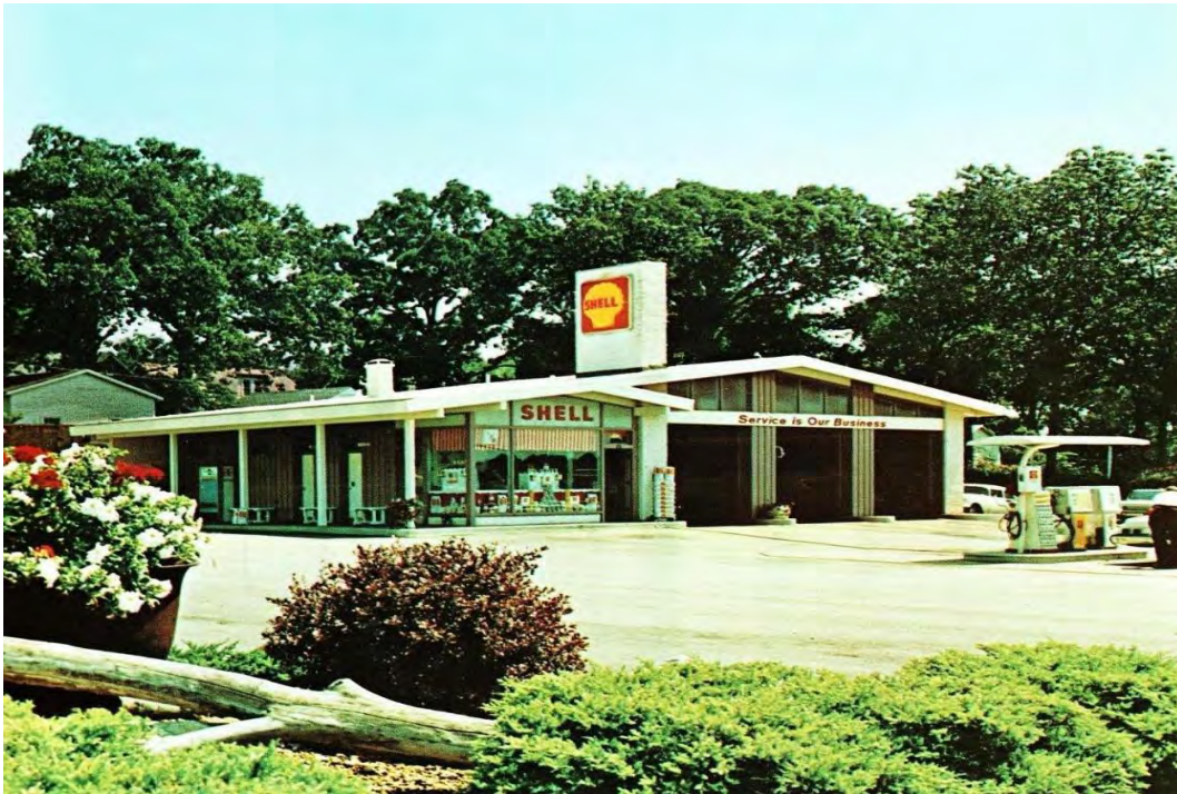
Prototypical Shell Oil Company Ranch-Style Station with Projecting Office Bay. Location Unknown. (Source: National Petroleum News , September 1969; www.flickr.com/photos/mark_potter_2000/3342084311/in/pool-1149631@N22 ).
