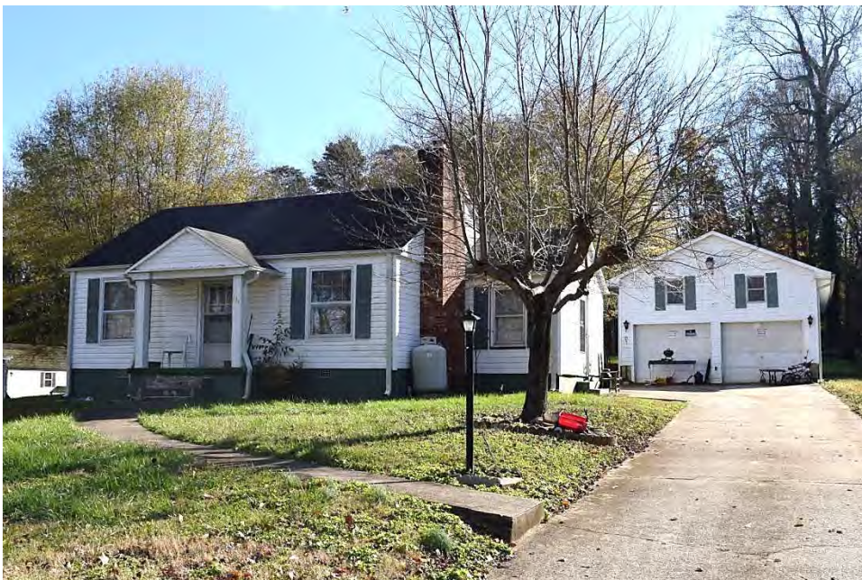
No. 36 House (PIN 6828-70-6663), 124 Garner Road, Winston-Salem, Forsyth County
