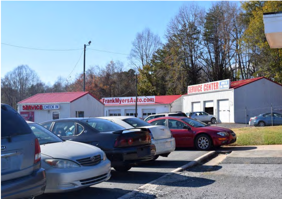
No. 13 Automobile Sales Building (PIN 6828-72-5432), Auxiliary Service Buildings, 4200 North Patterson Avenue, Winston-Salem, Forsyth County
