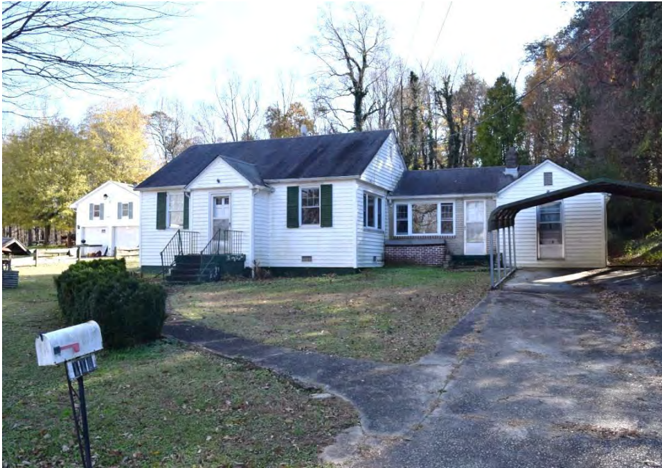
No. 35 House (PIN 6828-70-5663), 116 Garner Road, Winston-Salem, Forsyth County
