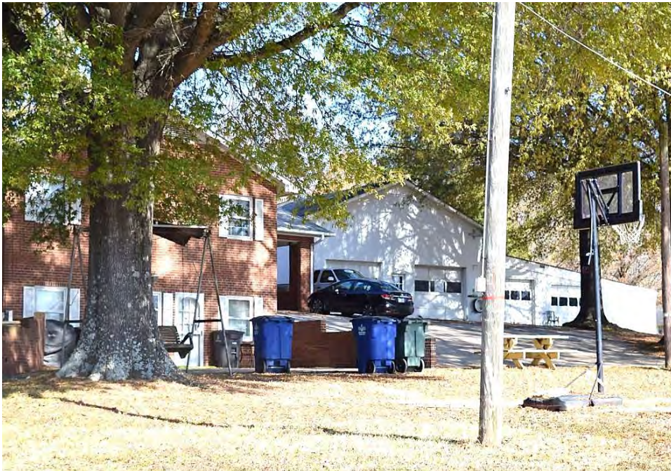
No. 9 House (PIN 6828-82-3711), Rear Garage, 5217 Germanton Road, Winston-Salem, Forsyth County
