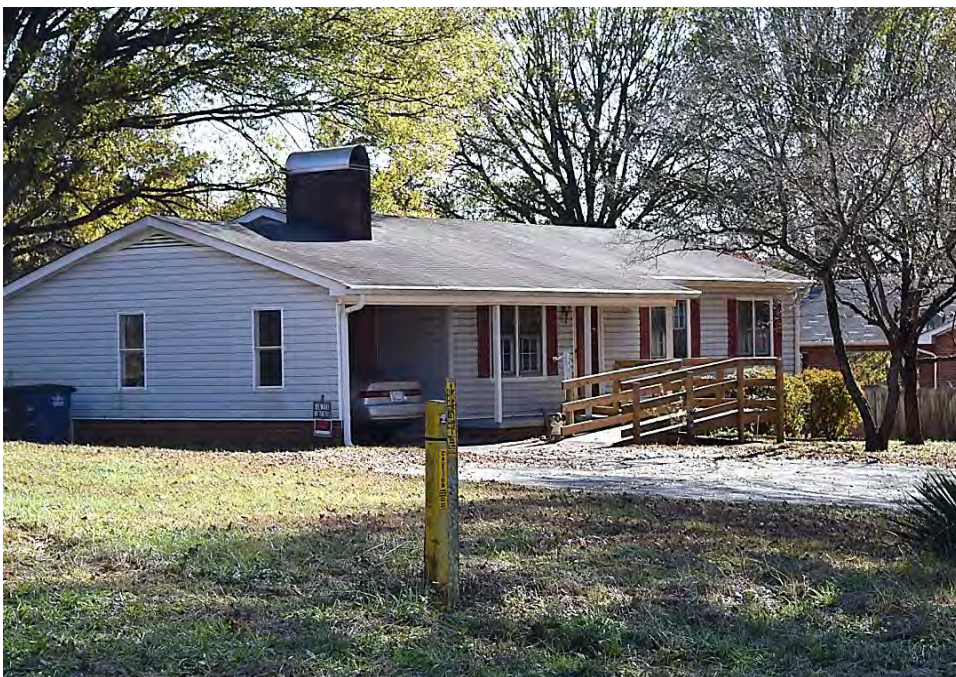
No. 8 House (PIN 6828-82-4885), 5221 Germanton Road, Winston-Salem, Forsyth County
