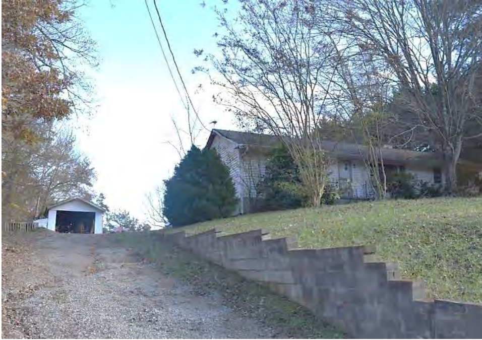
No. 33 House (PIN 6828-70-5149), 4943 Germanton Road, Winston-Salem, Forsyth County
