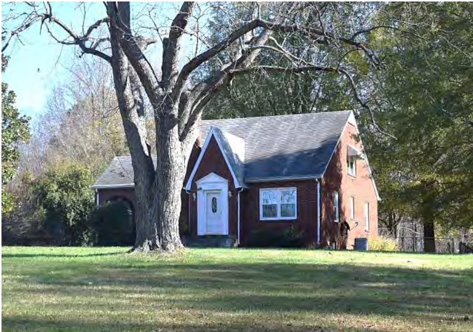
No. 6 House (PIN 6828-83-5314), 5245 Germanton Road, Winston-Salem, Forsyth County
