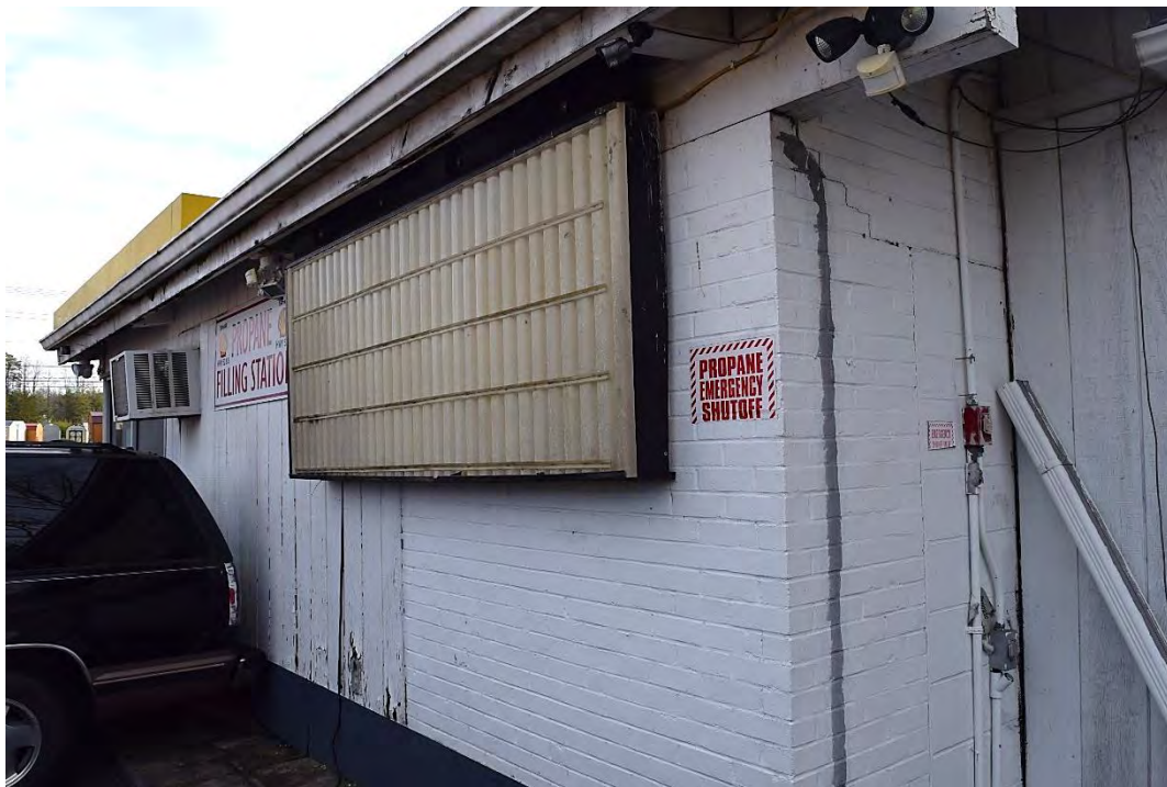
Knotts Shell Service Station No. 1, Side (North) Elevation, Looking East.
