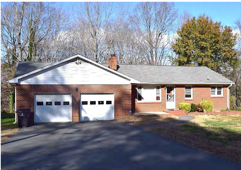
No. 40 House (PIN 6828-70-5886, 115 Garner Road, Winston-Salem, Forsyth County
