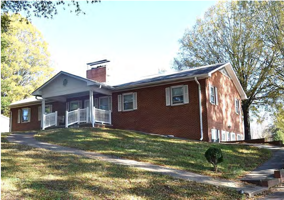
No. 9 House (PIN 6828-82-3711), 5217 Germanton Road, Winston-Salem, Forsyth County
