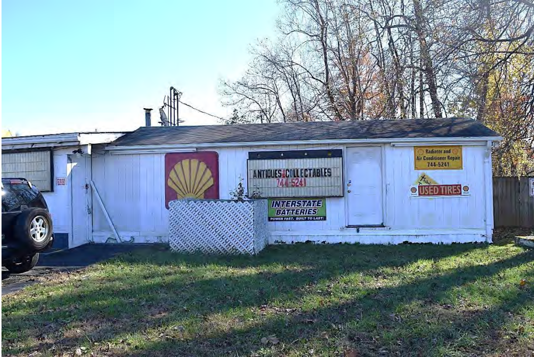
Knotts Shell Service Station No. 1, Rear Storage Wing, Side, (North) Elevation with Shell Sign, Looking South.
