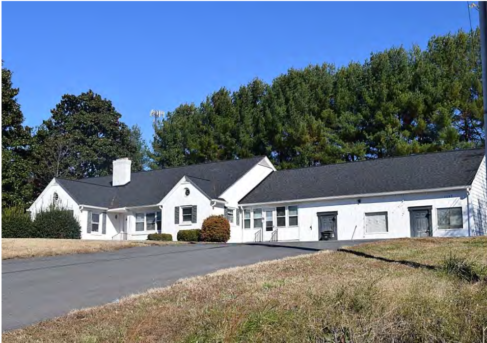
No. 10 House (PIN 6828-81-2923), 4187 North Patterson Avenue, Winston-Salem, Forsyth County
