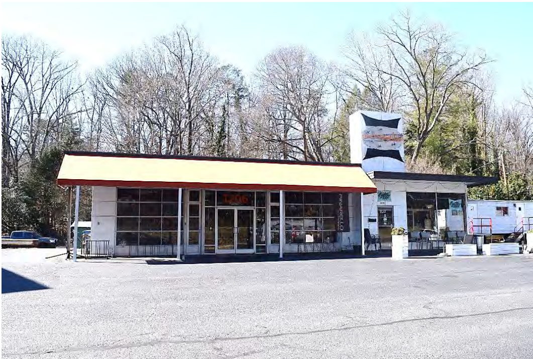
Texaco Service Station (1962), 1206 Reynolda Road, Winston-Salem, Looking West.
