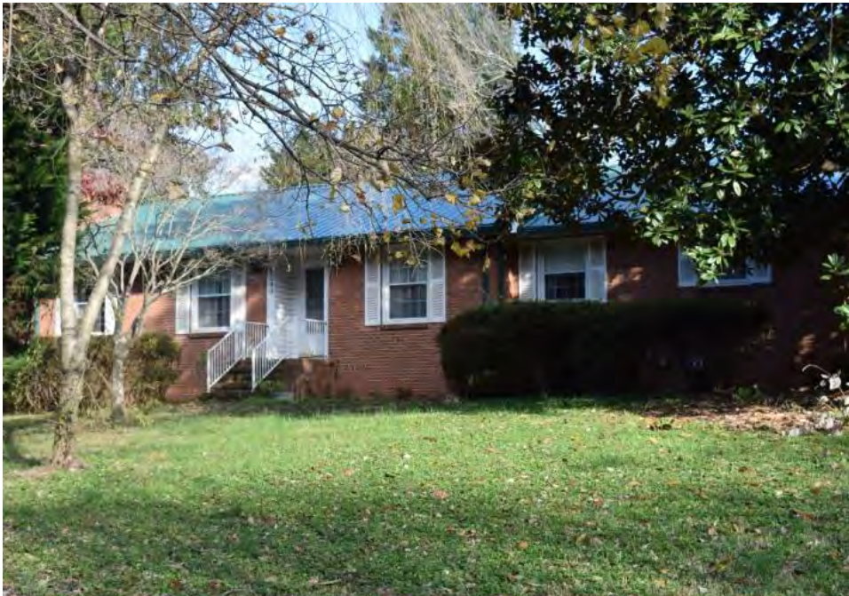
No. 32 House (PIN 6827-79-7969), 4925 Germanton Road, Winston-Salem, Forsyth County
