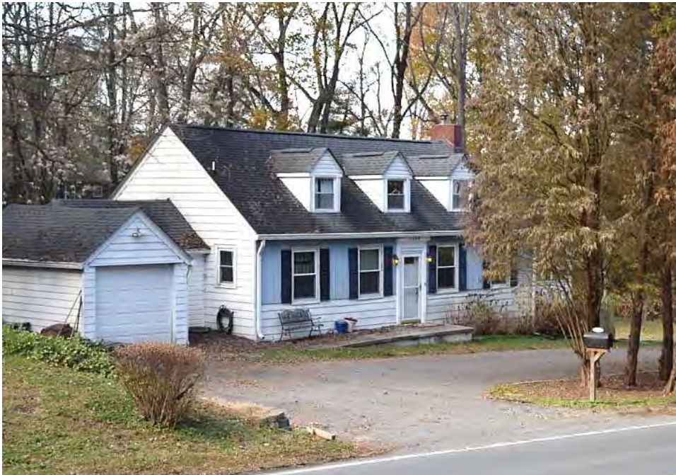
No. 42 House (PIN 6828-70-0285), 4944 Germanton Road, Winston-Salem, Forsyth County
