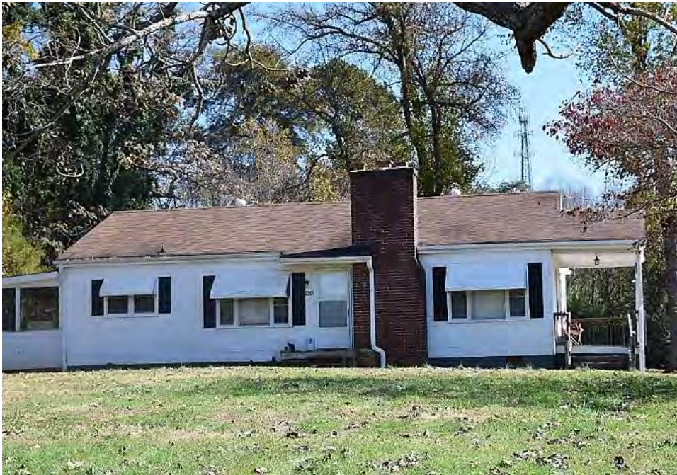
No. 4 House (PIN 6828-83-5782), 5261 Germanton Road, Winston-Salem, Forsyth County
