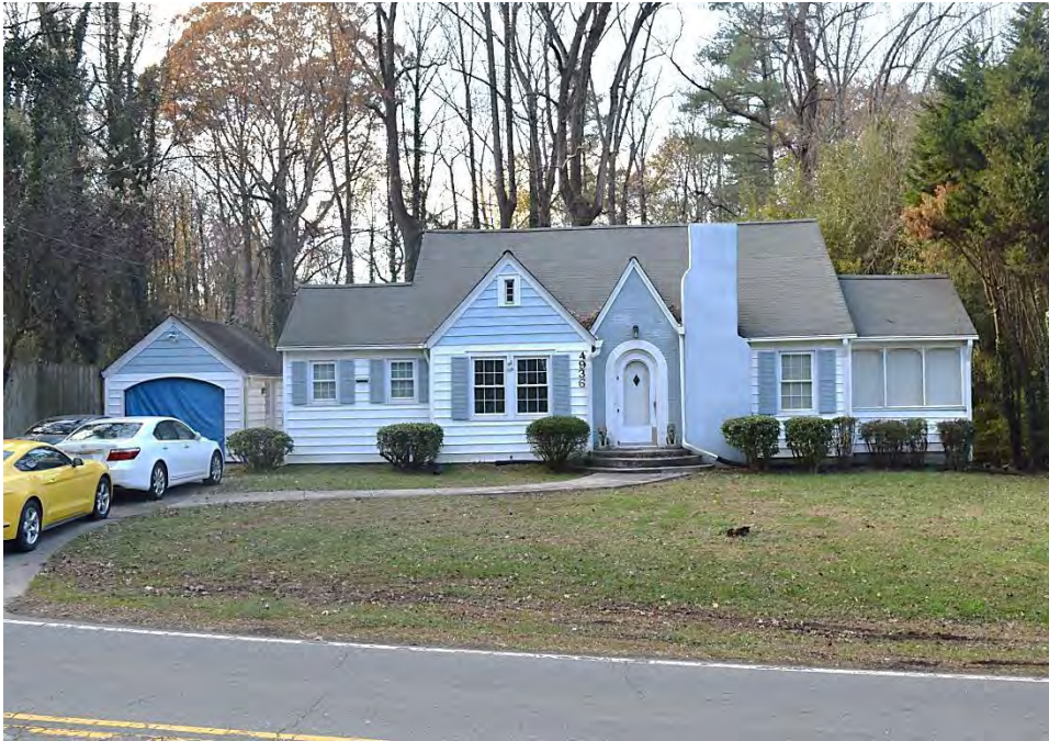
No. 43 House (PIN 6828-70-0165), 4936 Germanton Road, Winston-Salem, Forsyth County
