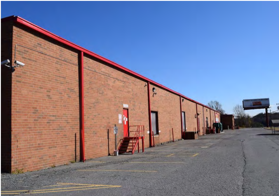
No. 15 Cook's Flea Market (PIN 6828-63-9091), 4250 North Patterson Avenue, Winston-Salem, Forsyth County
