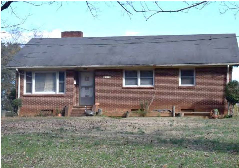
No. 30 House (PIN 6827-79-3767), 4911 Germanton Road, Winston-Salem, Forsyth County
