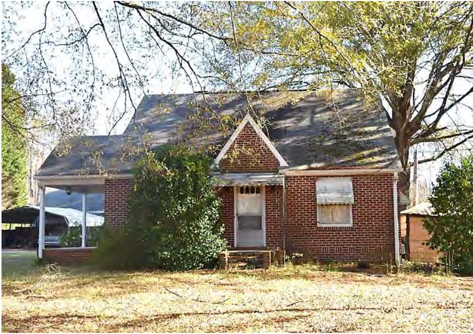
No. 7 House (PIN 6828-83-5006), 5237 Germanton Road, Winston-Salem, Forsyth County
