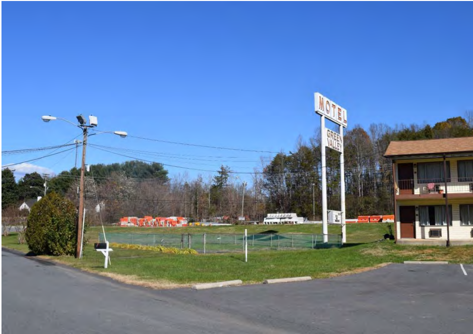
No. 11 Green Valley Motel (PIN 6828-81-0485), Infilled Swimming Pool, 4170 North Patterson Avenue, Winston-Salem, Forsyth County
