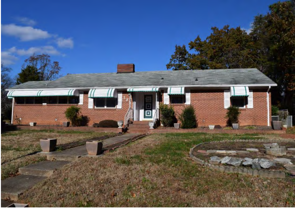
No. 26 House (PIN 6827-69-8432), 152 Otis Drive, Winston-Salem, Forsyth County
