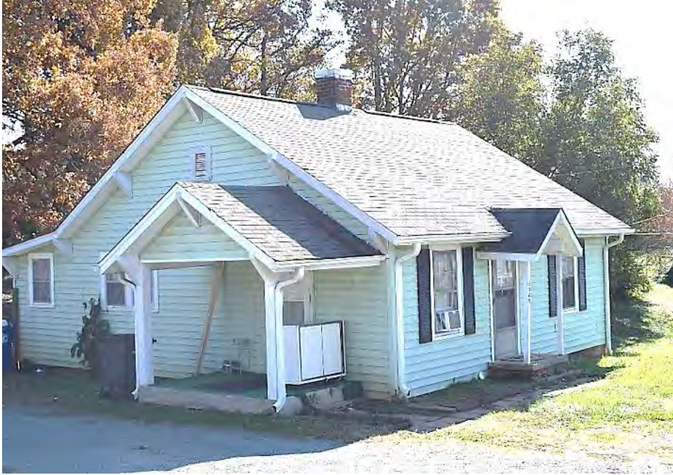
No. 3 House (PIN 6828-83-2987), 5269 Germanton Road, Winston-Salem, Forsyth County
