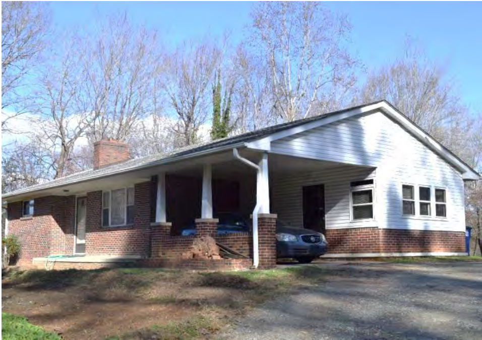
No. 41 House (PIN 6828-70-4960), 5001 Germanton Road, Winston-Salem, Forsyth County
