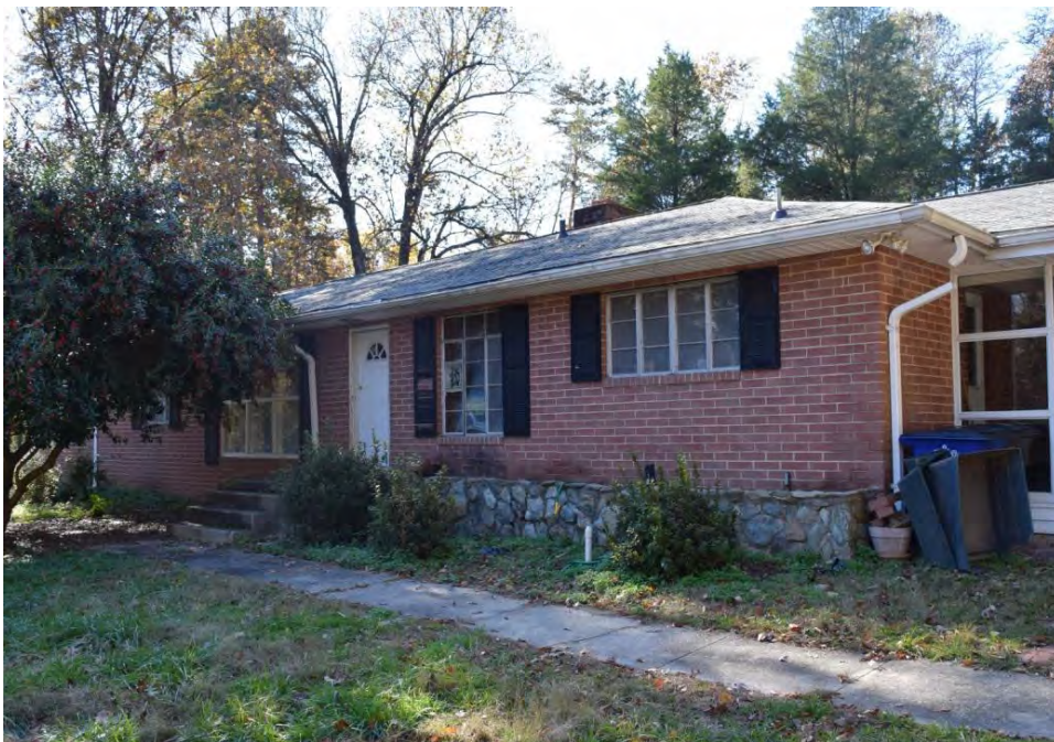
No. 17 House (PIN 6828-71-1089), 5030 Germanton Road, Winston-Salem, Forsyth County
