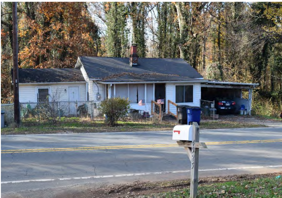
No. 44 House (PIN 6827-79-1839), 4922 Germanton Road, Winston-Salem, Forsyth County
