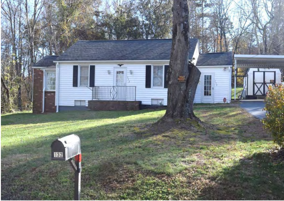
No. 37 House (PIN 6828-70-7663), 132 Garner Road, Winston-Salem, Forsyth County
