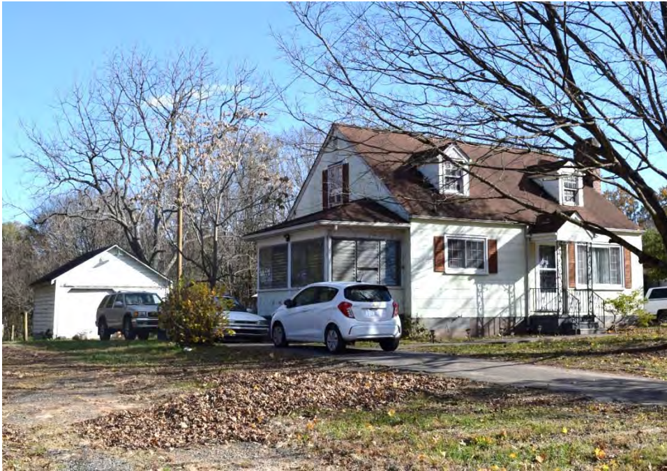
No. 28 House (PIN 6827-79-3431), 4855 Germanton Road, Winston-Salem, Forsyth County
