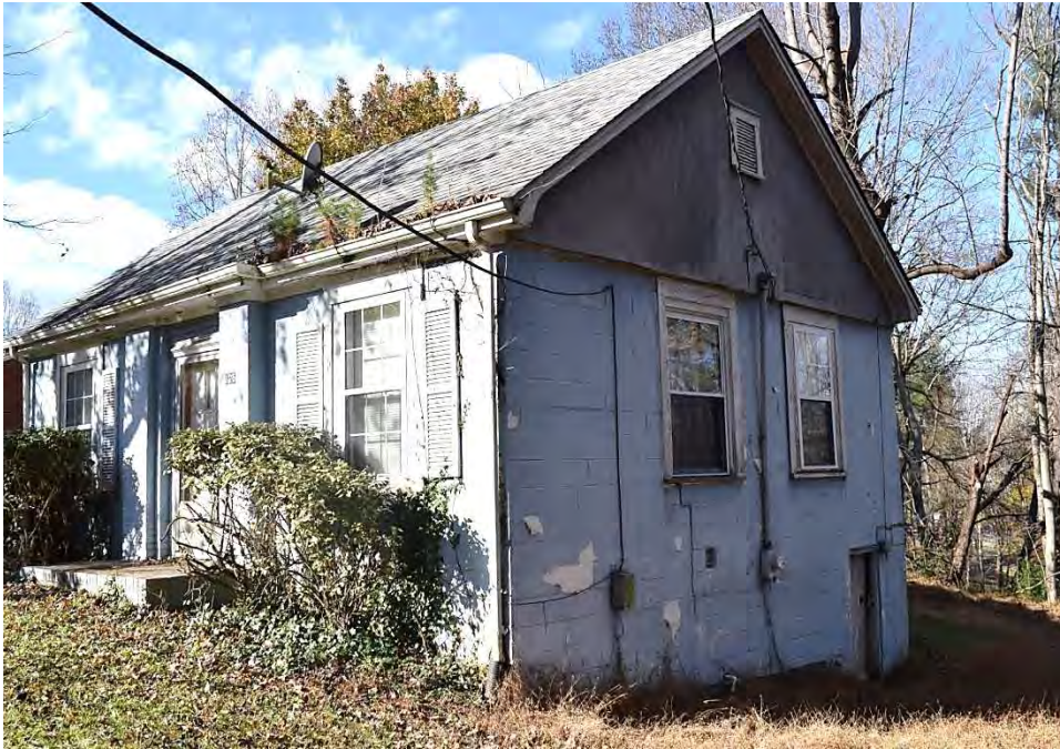
No. 39 House (PIN 6828-70-7831), 125 Garner Road, Winston-Salem, Forsyth County
