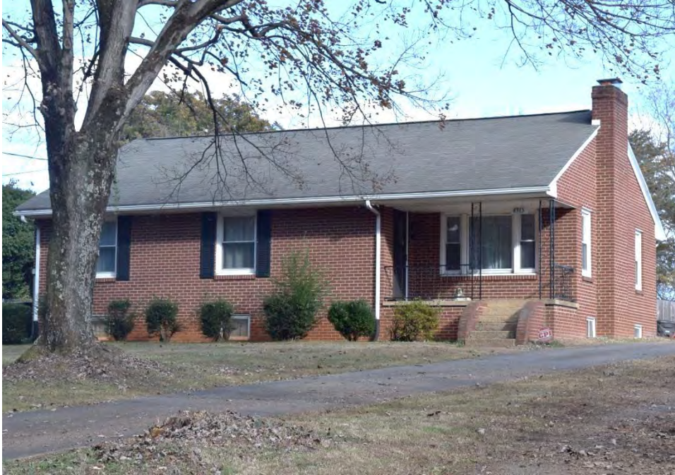
No. 31 House (PIN 6827-79-4804), 4915 Germanton Road, Winston-Salem, Forsyth County
