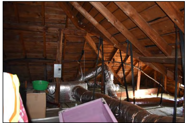
Figure 56: Attic with original well-preserved common rafters, roof boards, and other framing members
