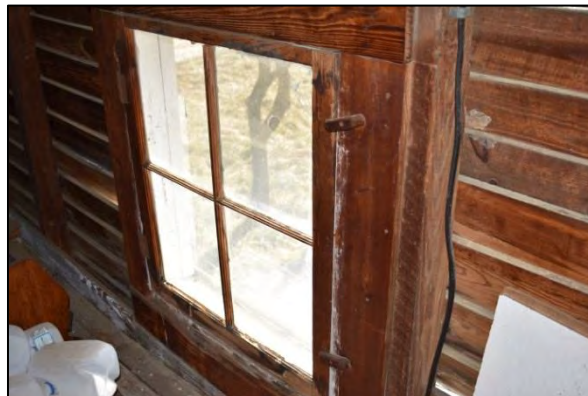
Figure 37. Casement attic window with hinges and wooden latches in place
