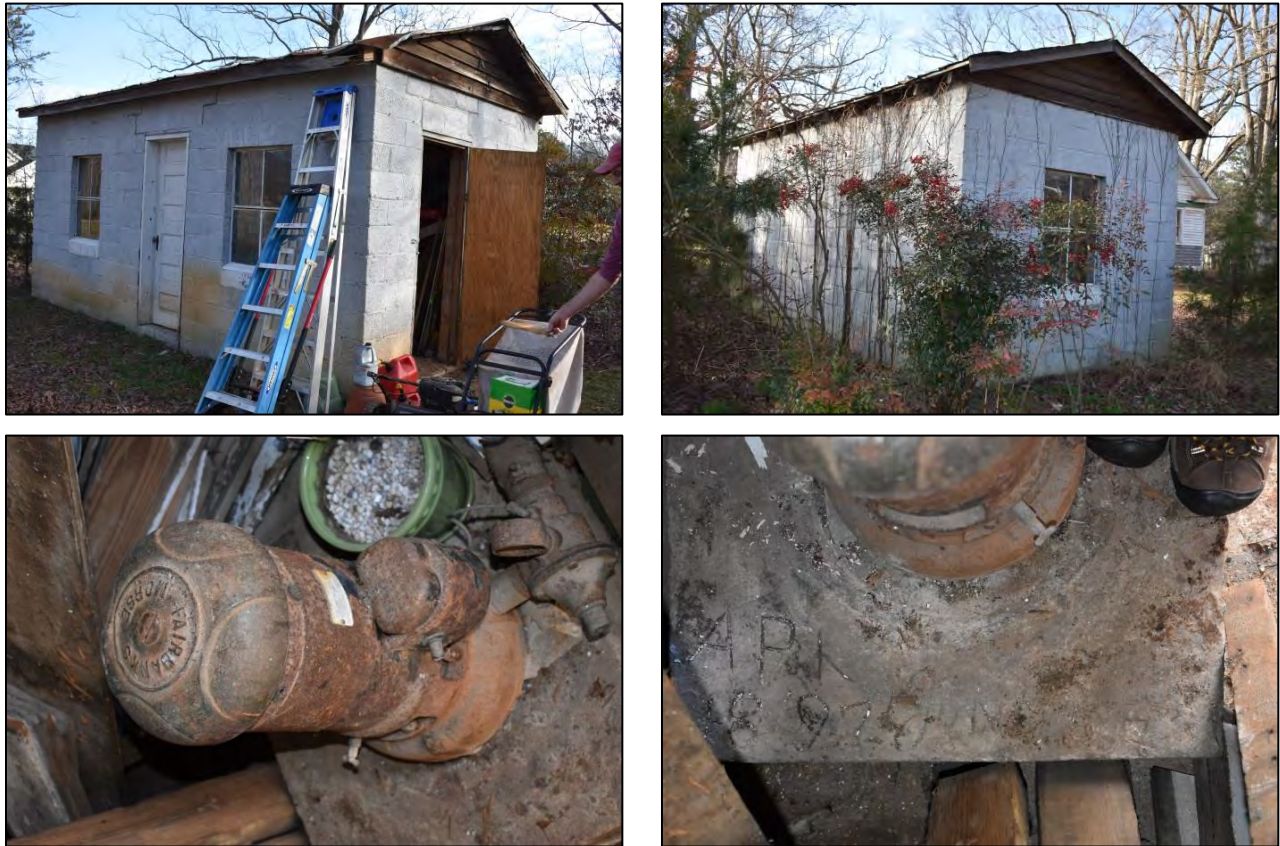
Figure 57: At top, concrete-block body of shed; at bottom, Fairbanks-Morse light plant or well pump fixture standing upon and 1897-dated concrete
