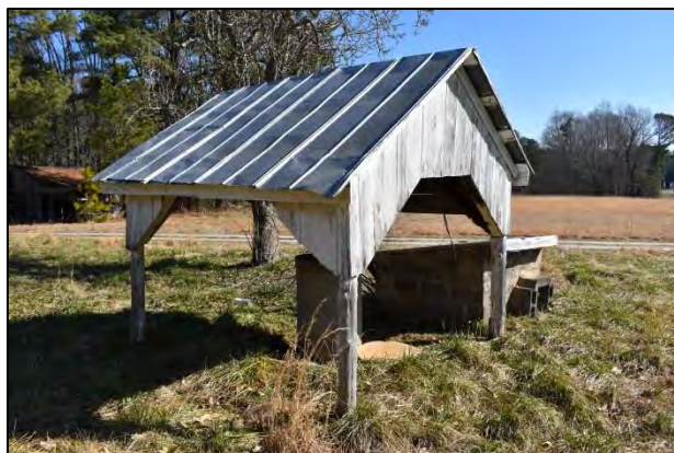
Figure 38: View of frame shed and low concrete-block wellhouse looking to northeast
