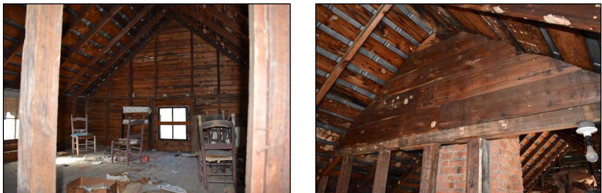
Figure 36: Common rafter system, wood floor, and partition in loft
