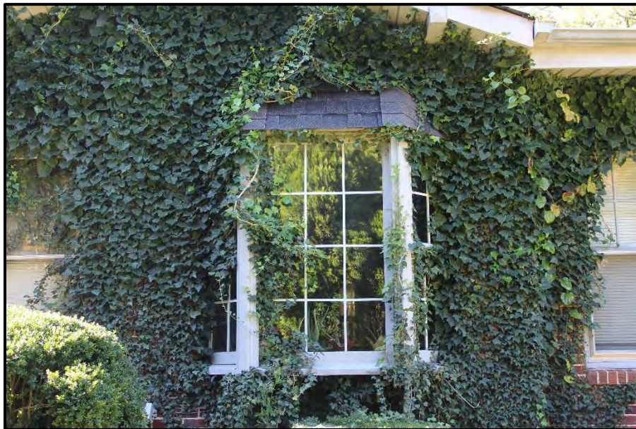
Figure 32. Detail of Bay Window on East Elevation, Looking Southwest.
