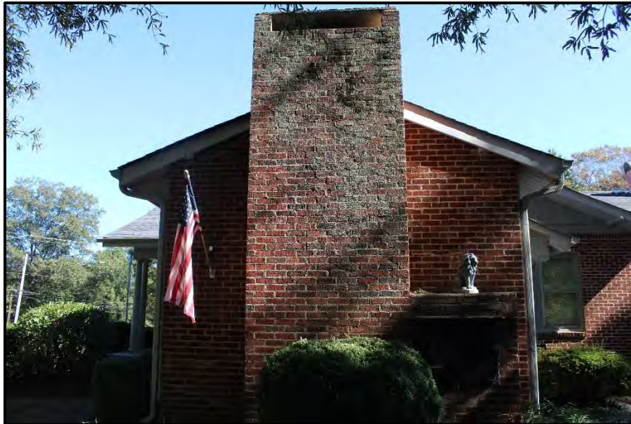
Figure 28. Detail of Chimney, Looking Northeast.
