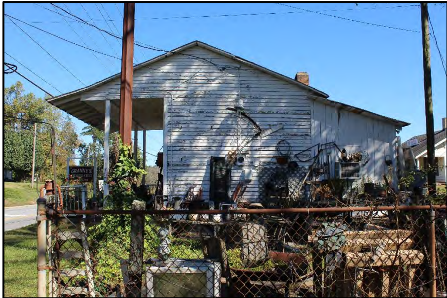
Figure 6. R. L. Hastings Store, Looking Northeast.
