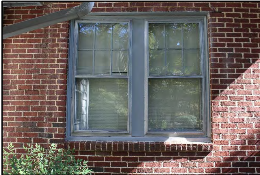
Figure 31. Detail of Paired Window on West Elevation, Looking Northeast.
