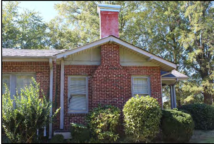
Figure 27. Detail of Northeast Gable End, Looking Southwest.
