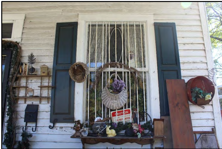
Figure 10. Detail of Bay Window on Southwestern Elevation, Looking North.
