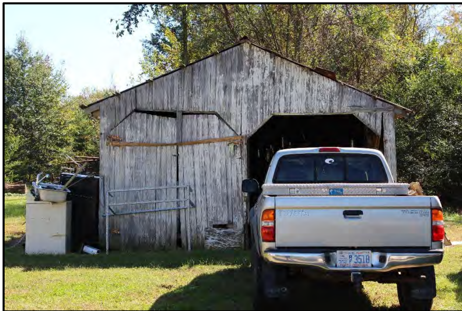
Figure 13. Vehicle Shed/Garage, Looking South.
