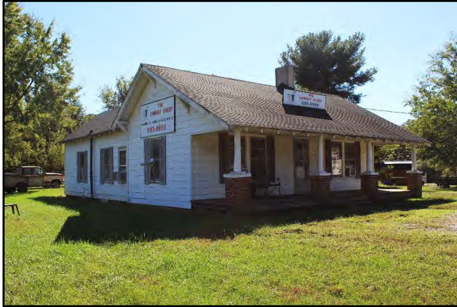
Figure 12. Dwelling, Looking Southwest.
