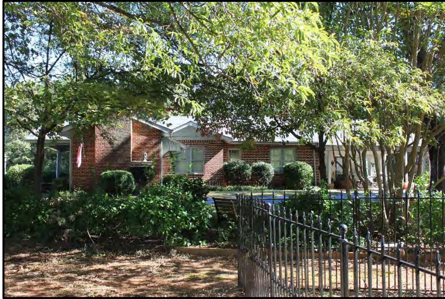
Figure 25. Ebert House, Looking Northeast.
