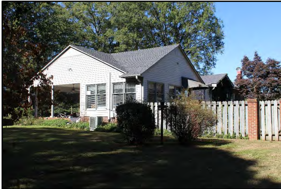
Figure 26. Ebert House, Looking Northwest.
