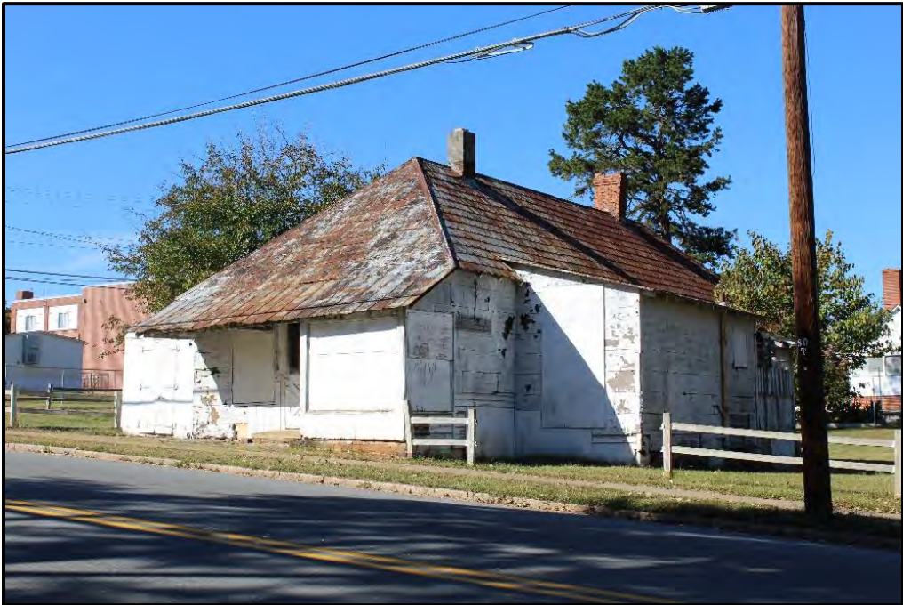
Figure 18. Store (FY3049), 1601 Sprague Street, Winston-Salem, NC, Looking Northwest.
