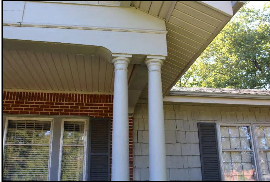
Figure 29. Detail of Front Porch, Looking Southeast.
