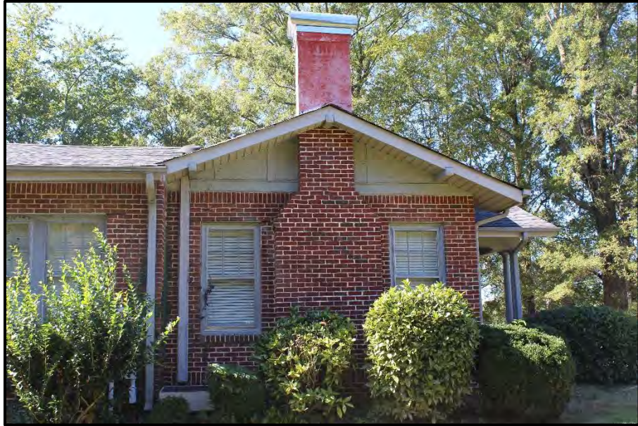
Figure 27. Detail of Northeast Gable End, Looking Southwest.
