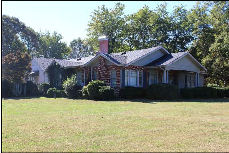
Figure 24. Ebert House, Looking South.
