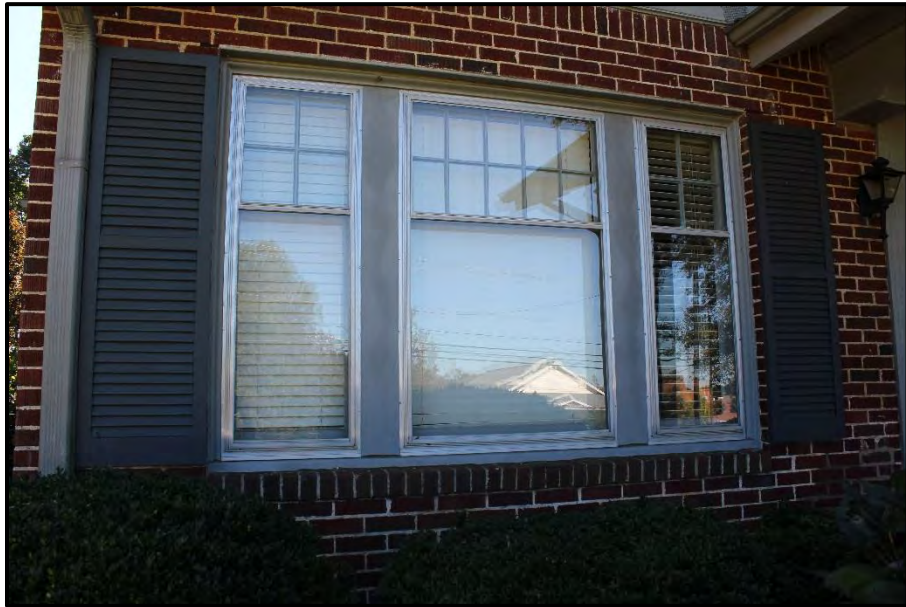
Figure 30. Detail of Tripartite Window on the Facade, Looking Southeast.
