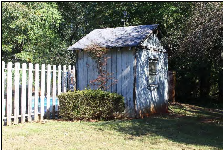
Figure 35. Shed, Looking West.
