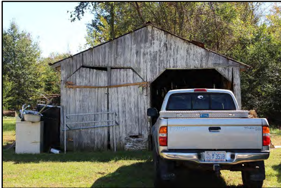
Figure 13. Vehicle Shed/Garage, Looking South.
