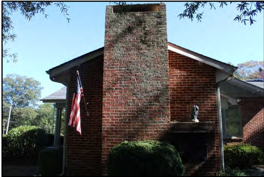
Figure 28. Detail of Chimney, Looking Northeast.
