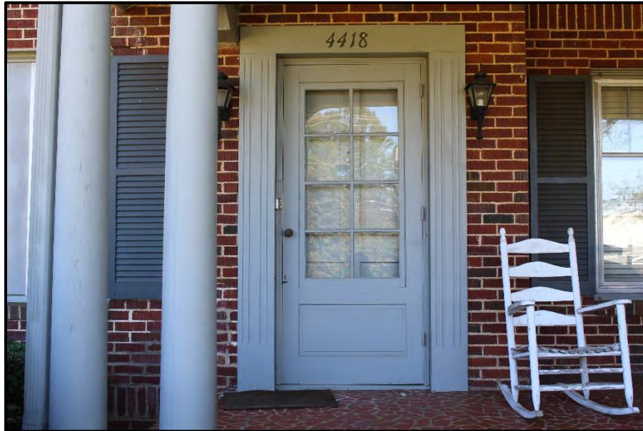
Figure 33. Detail of Entry Door on Front Facade, Looking Southeast.
