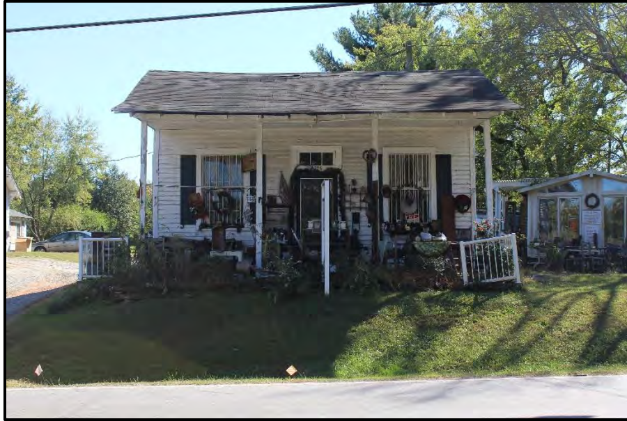
Figure 5. R. L. Hastings Store, Looking Southeast.
