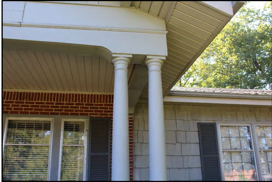
Figure 29. Detail of Front Porch, Looking Southeast.
