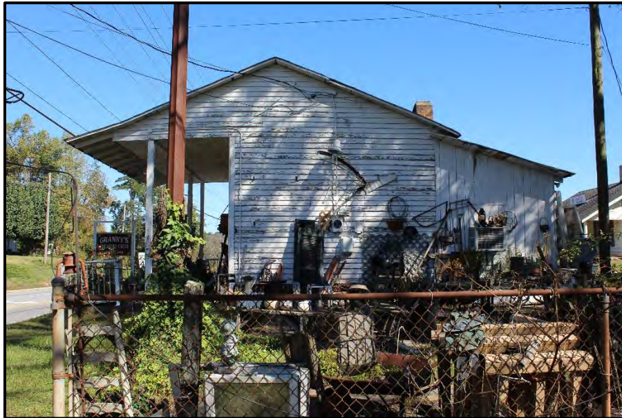
Figure 6. R. L. Hastings Store, Looking Northeast.
