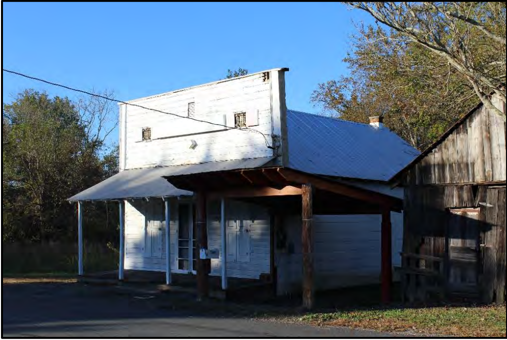
Figure 17. Long's Store (FY1490), 4916 Vienna-Dozier Road, Dozier, NC, Looking Southwest.
