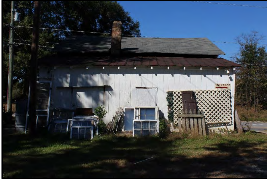
Figure 7. R. L. Hastings Store, Looking Northeast.
