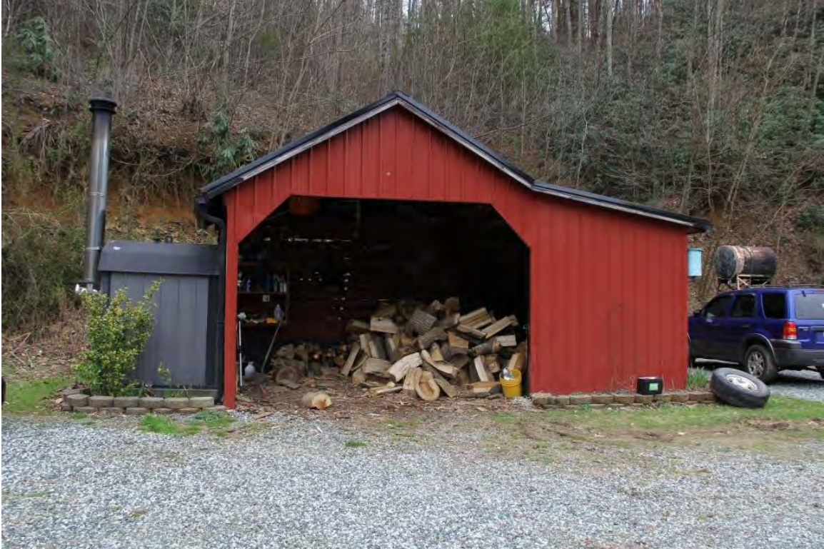
Woodshed, view to east
