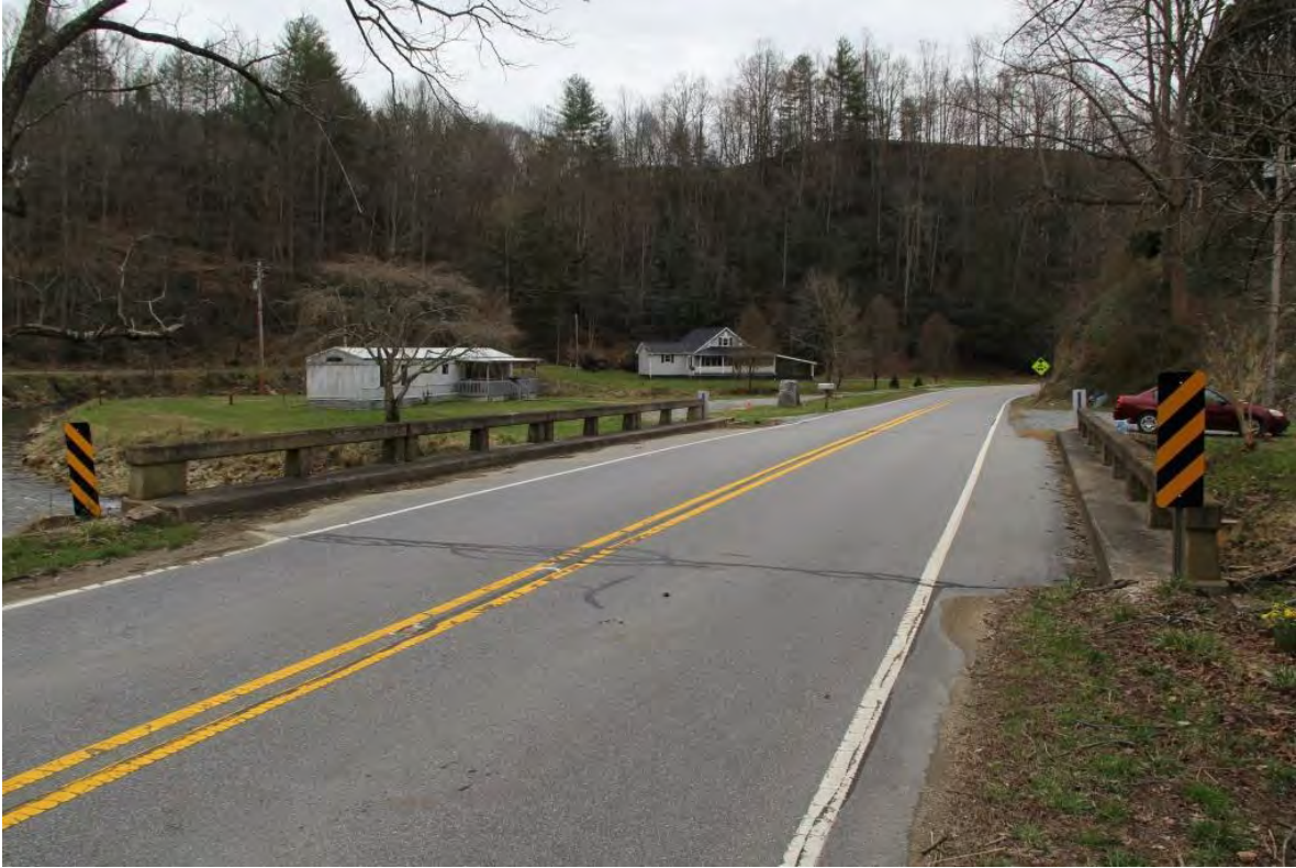
Bridge No. 15 over Shelton Laurel Creek, view to south along NC 212
