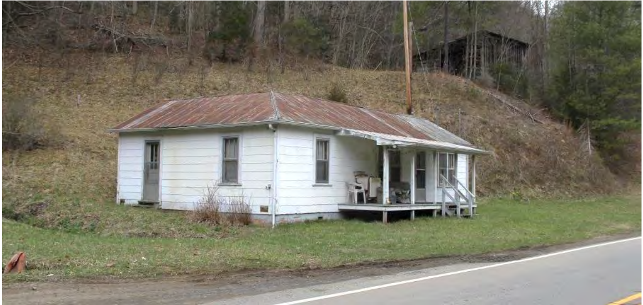
House and barn, 1969 NC 212 Hwy, view to northwest
