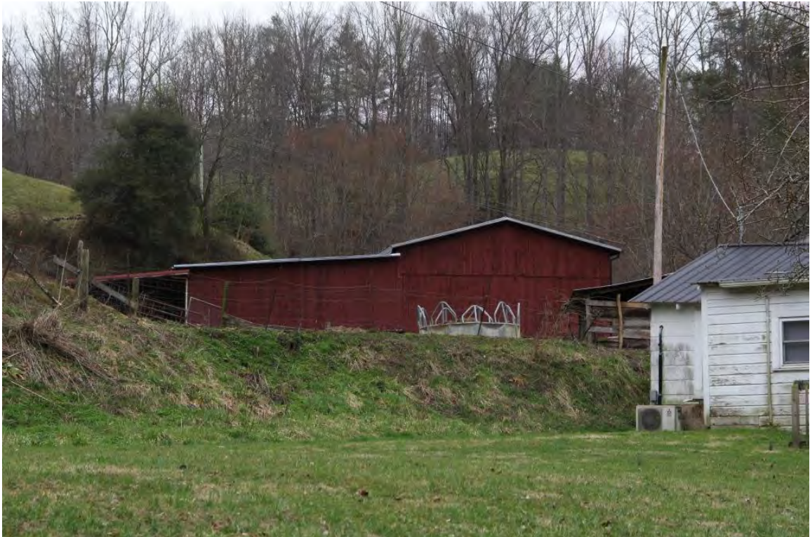
Barn, view to southeast
