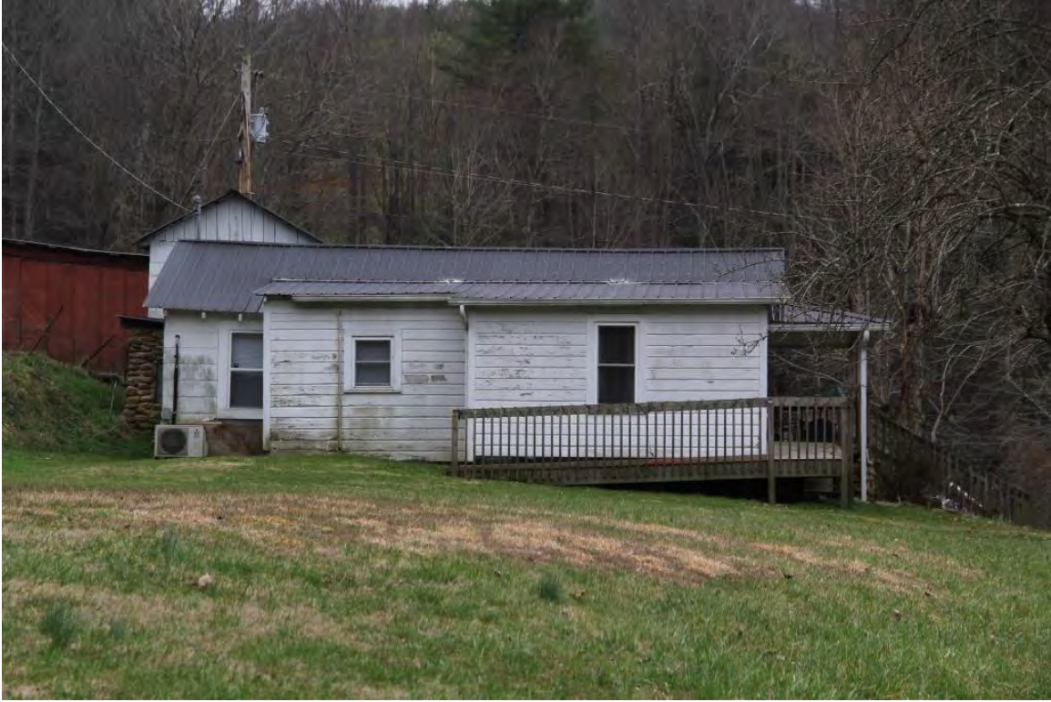
Gentry-Tweed Homestead, north elevation, view to south
