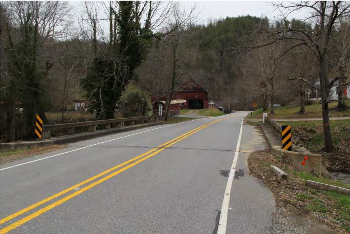
Bridge No. 15 over Shelton Laurel Creek, view to north along NC 212
