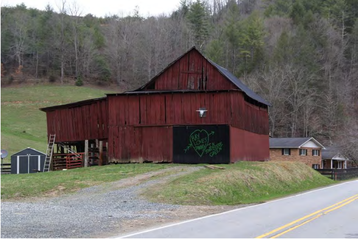
Tweed Barn, south elevation, view to north
