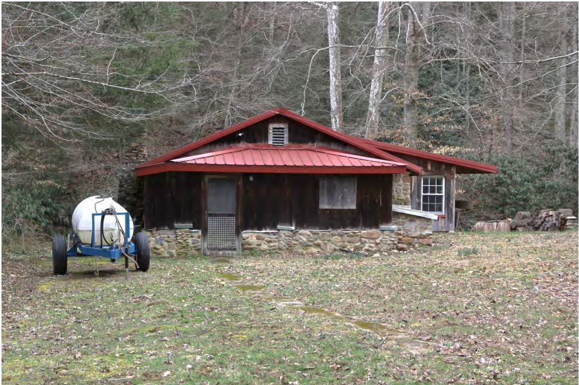
House, 3689 NC 212 Hwy, façade, view to west
