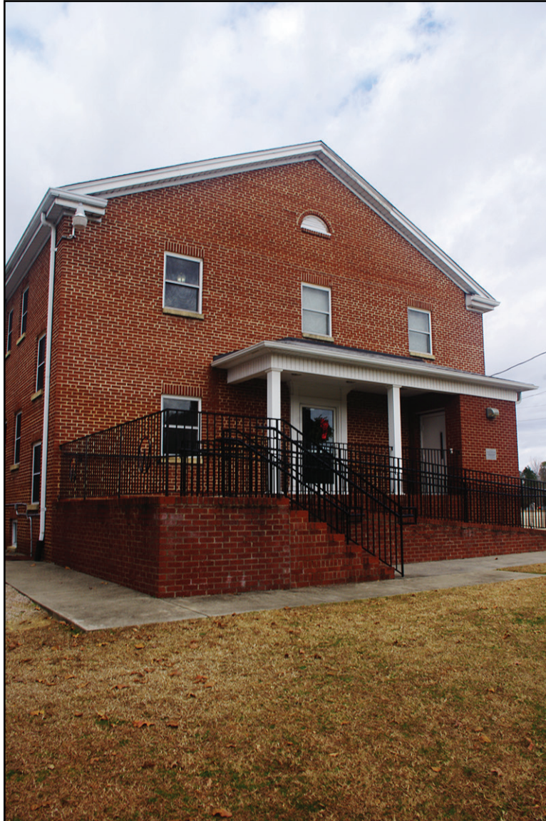
PLATE 6: South Elevation of Rear Wing, White Oak Baptist Church (JT1994), Johnston County, North Carolina
