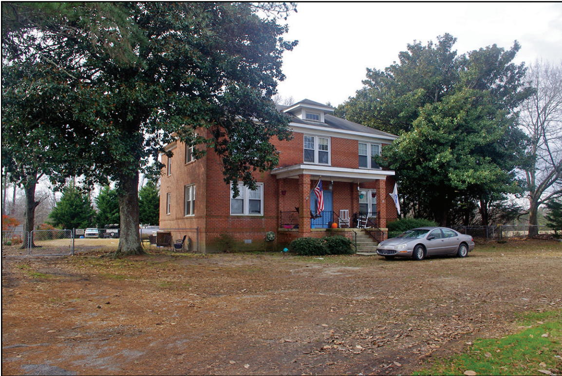
PLATE 32: Oblique View of South and East Elevations, Former Archer Lodge School Teacherage (JT1995), Johnston County, North Carolina
