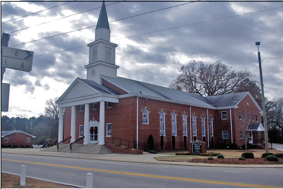
PLATE 1: Oblique View of North And East Elevations, White Oak Baptist Church (JT1994), Johnston County, North Carolina
