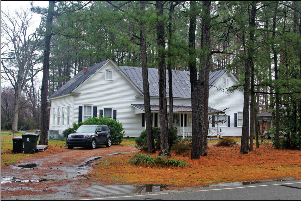
PLATE 44: Brogden Teacherage (JT1299), Southwest Elevation, Johnston County, North Carolina
