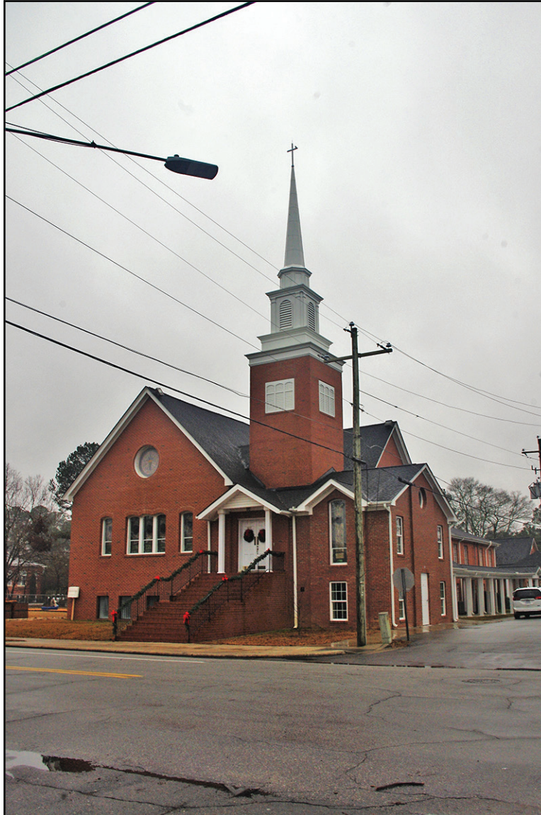
PLATE 30: Four Oaks Baptist Church (JT1110), East Elevation, Four Oaks, Johnston County, North Carolina
