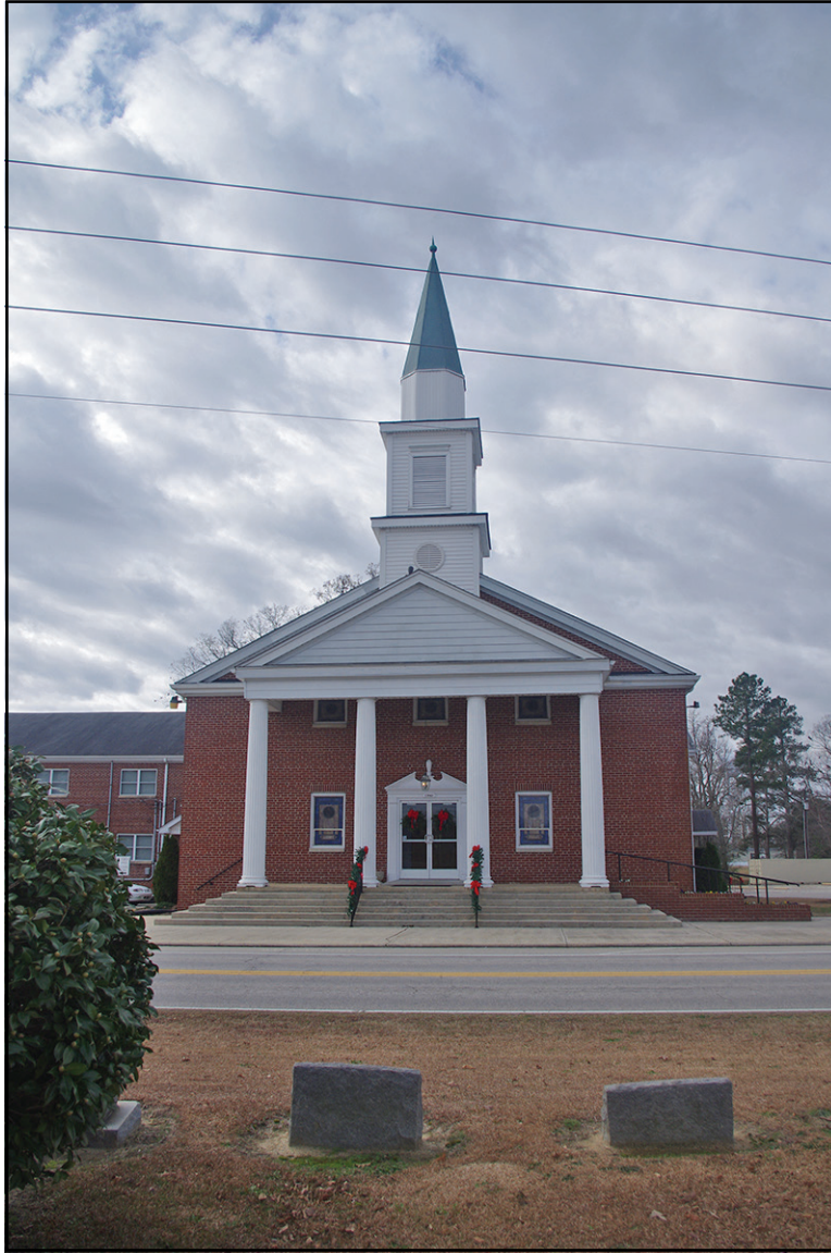
PLATE 2: East Elevation, White Oak Baptist Church (JT1994), Johnston County, North Carolina
