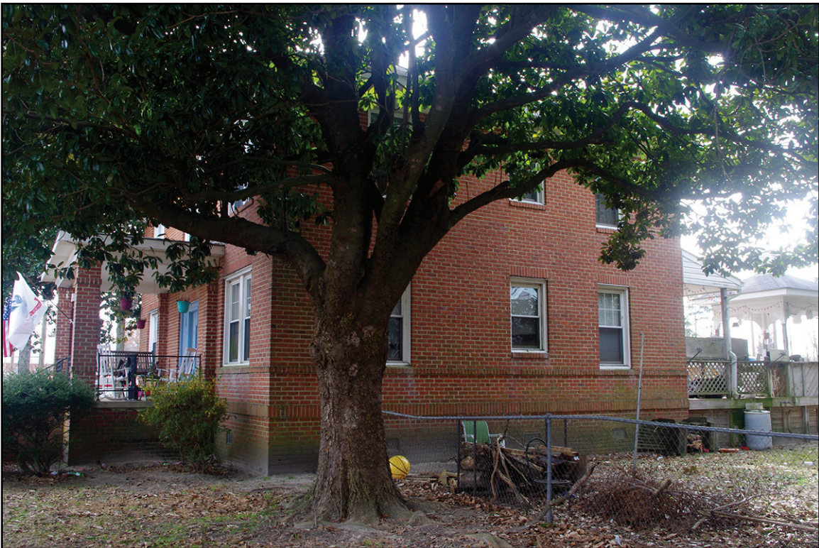
PLATE 35: Oblique View of North Elevation, Former Archer Lodge School Teacherage (JT1995), Johnston County, North Carolina
