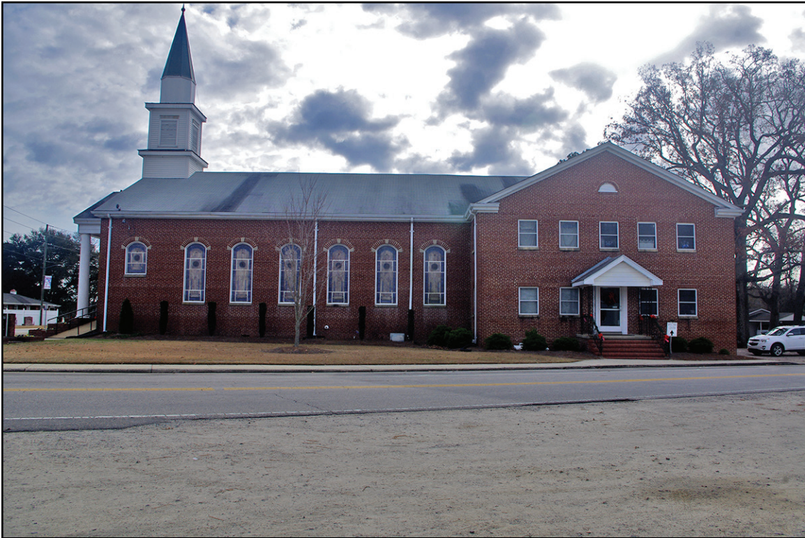
PLATE 4: North Elevation, White Oak Baptist Church (JT1994), Johnston County, North Carolina
