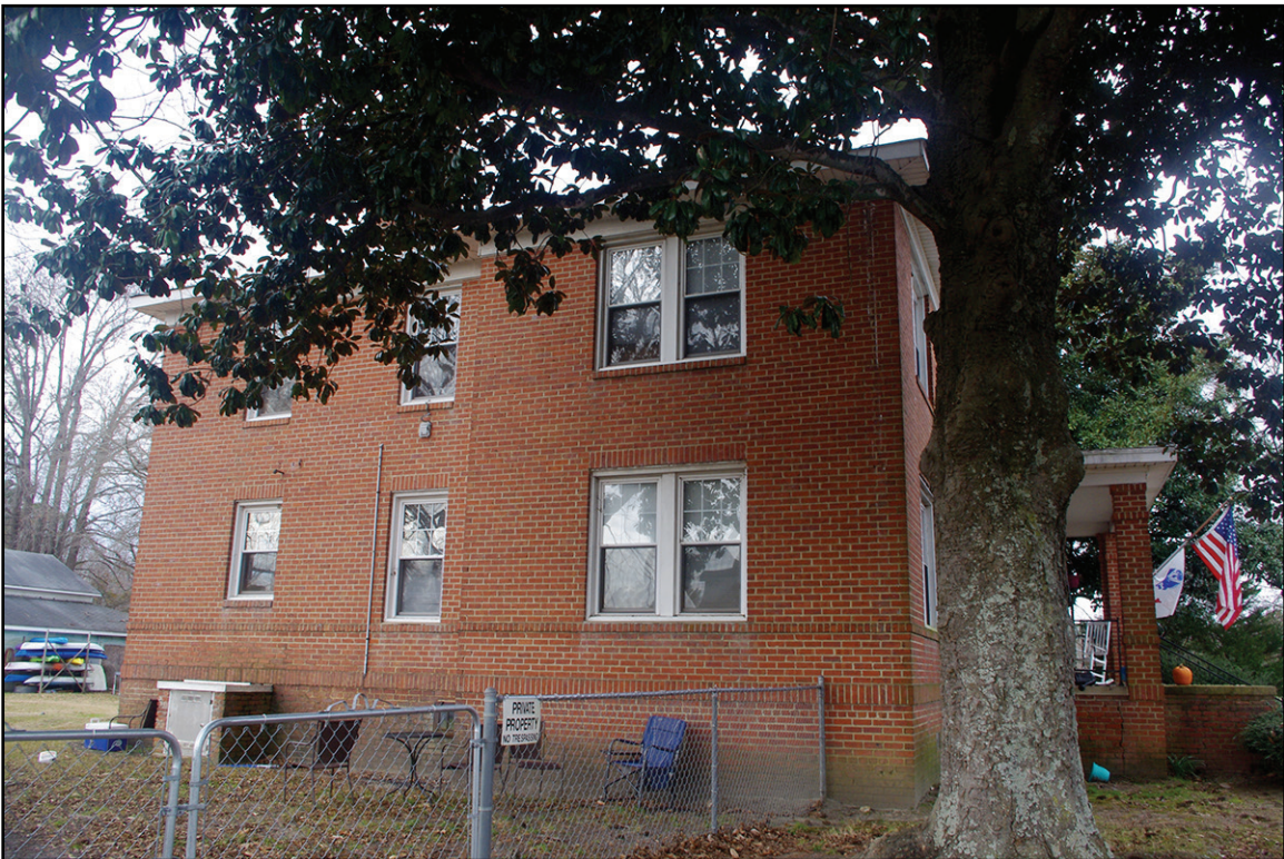
PLATE 37: South Elevation, Former Archer Lodge School Teacherage (JT1995), Johnston County, North Carolina
