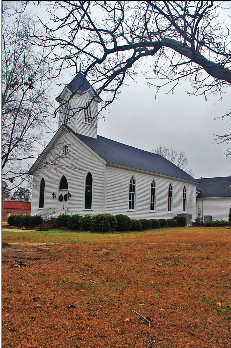
PLATE 28: Wilson's Mills Disciples of Christ Church (JT1006), Southeast Elevation, Johnston County, North Carolina
