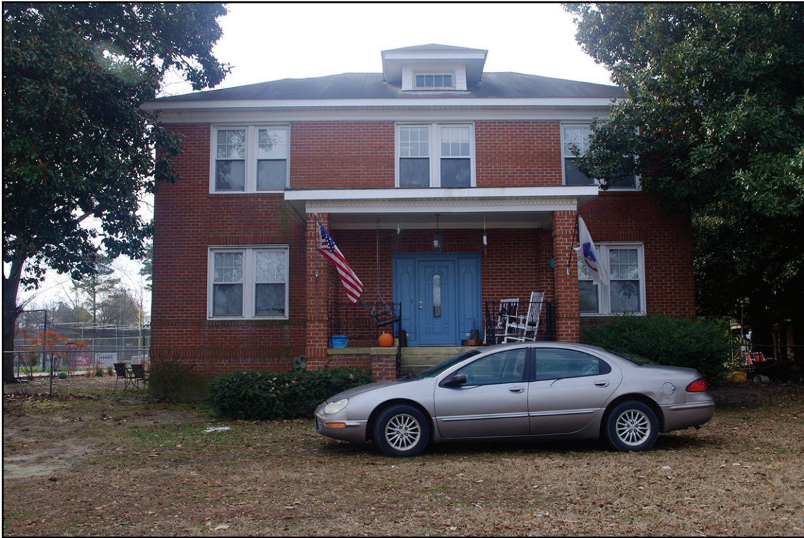
PLATE 34: East Elevation, Former Archer Lodge School Teacherage (JT1995), Johnston County, North Carolina
