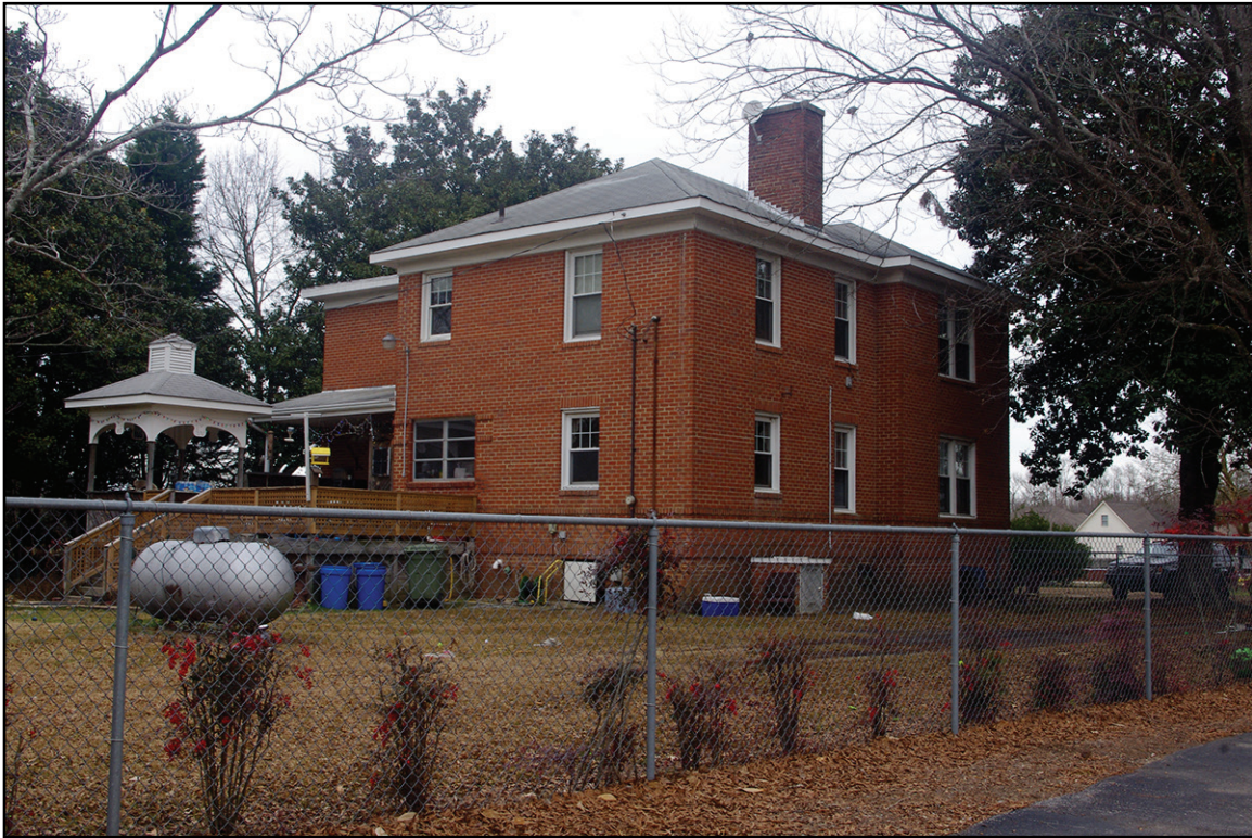
PLATE 36: Oblique View of West Elevation, Former Archer Lodge School Teacherage (JT1995), Johnston County, North Carolina
