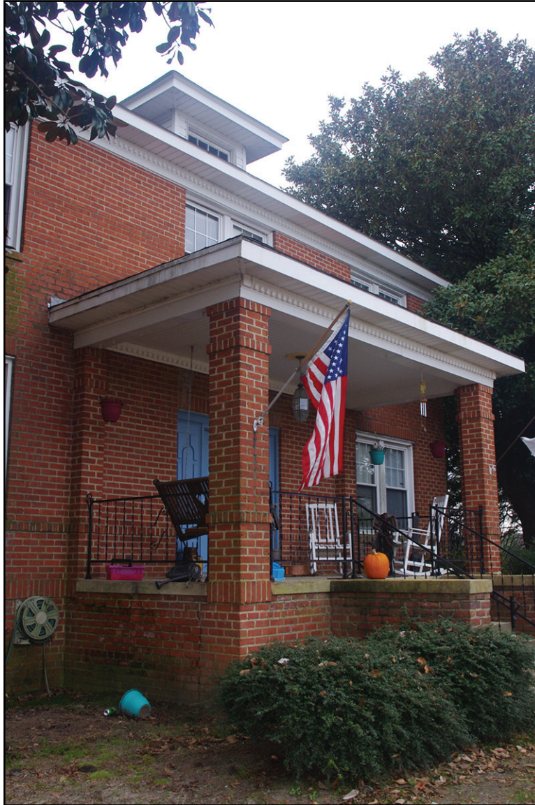
PLATE 33: Detail of Entrance Porch, East Elevation, Former Archer Lodge School Teacherage (JT1995), Johnston County, North Carolina
