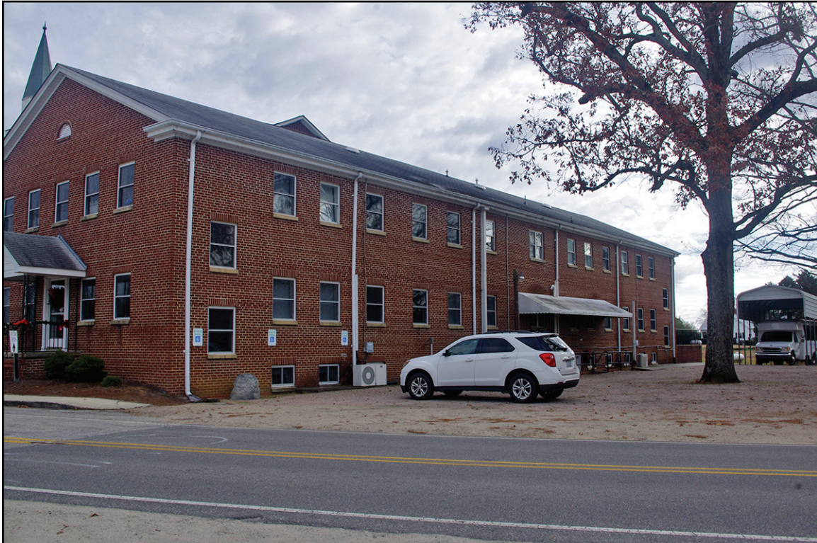
PLATE 5: West Elevation, White Oak Baptist Church (JT1994), Johnston County, North Carolina
