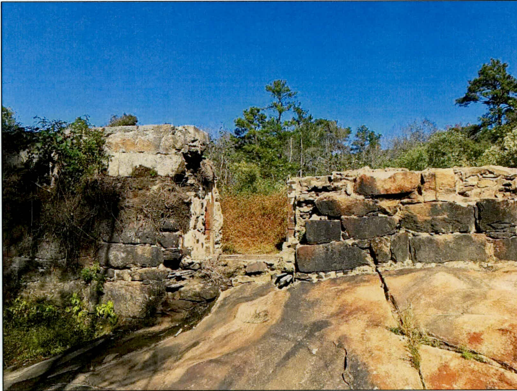
Photo 10: Western side of Moore's Mill Dam, facing north.
