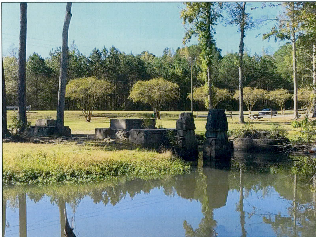
Photo 17: Foundation of Moore's Mill, facing southwest.
