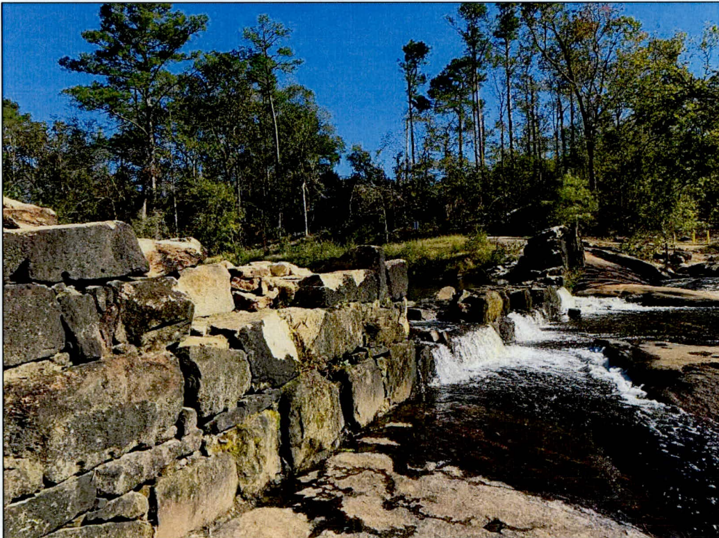
Photo 7: Moore's Mill Dam, facing east.
