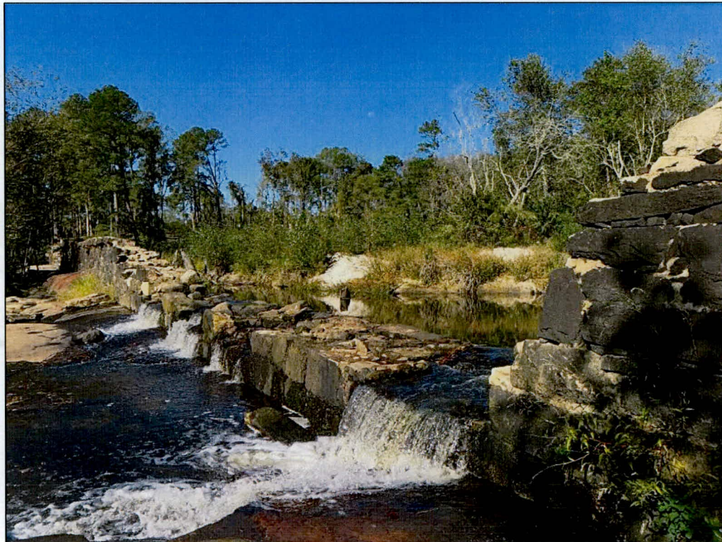
Photo 3: Moore's Mill Dam, facing west.
