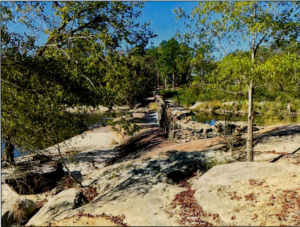
Photo 4: Moore's Mill Dam, facing southwest.
