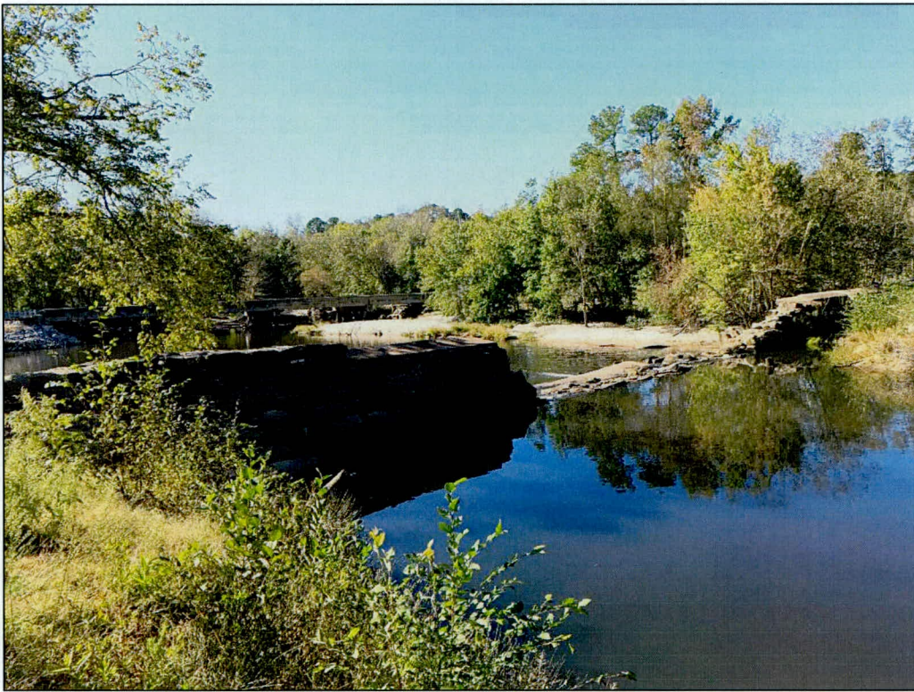
Photo 5: Moore's Mill Dam, facing south.
