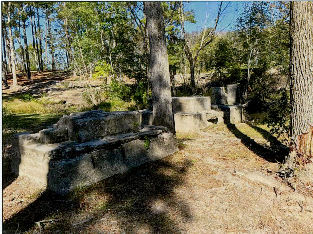
Photo 15: Foundation of Moore's Mill, facing northwest.
