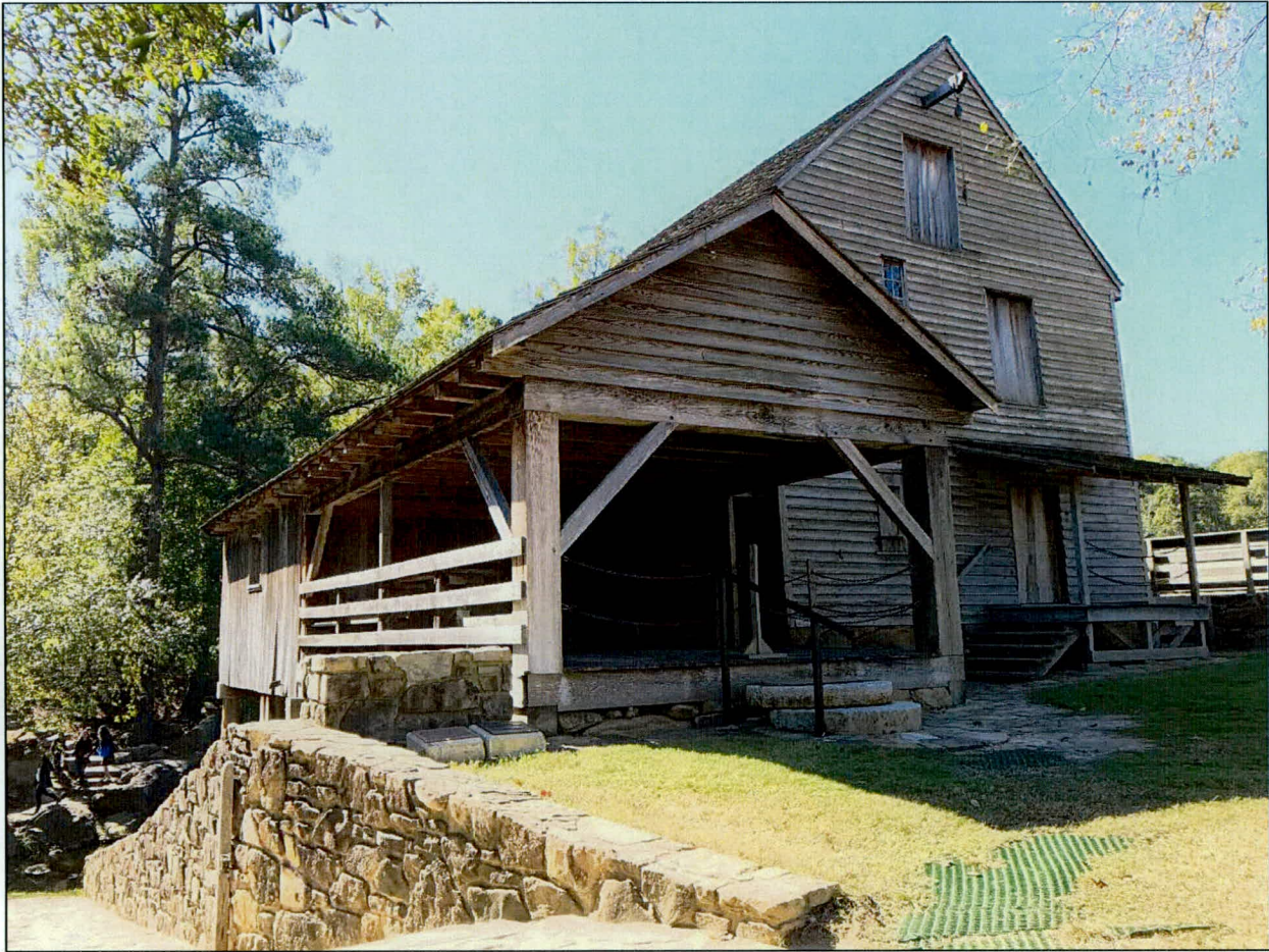
View of north and east elevations of Yates Mill, facing southwest.
