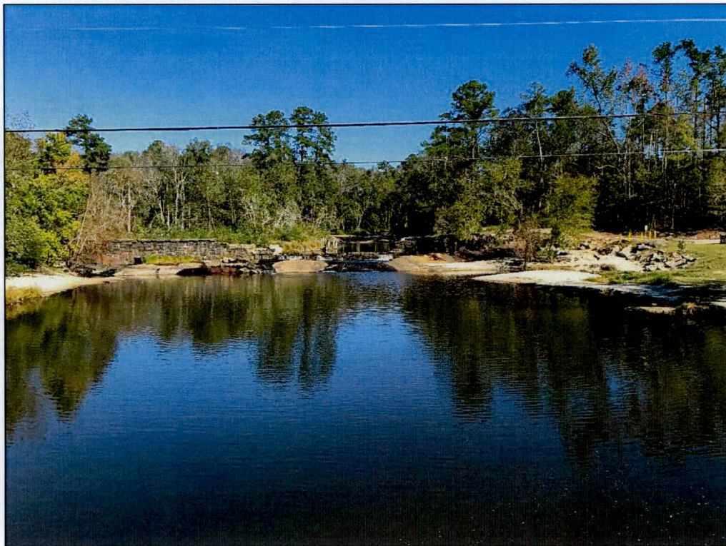
Photo 1: Moore's Mill Dam from NC 97, facing north.
