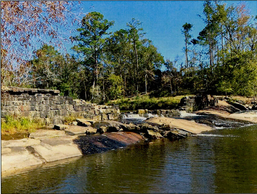
Photo 6: Moore's Mill Dam, facing northeast.
