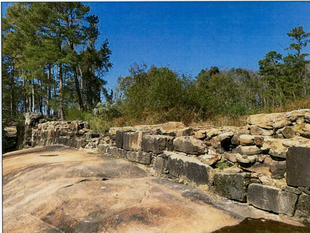
Photo 9: Western side of Moore's Mill Dam, facing west.
