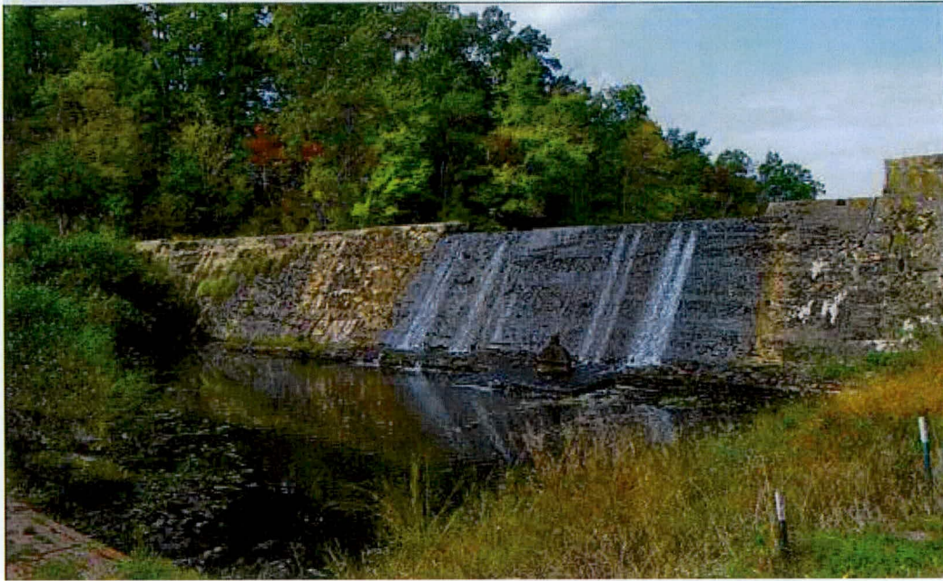
View of Myatt's Mill dam,
