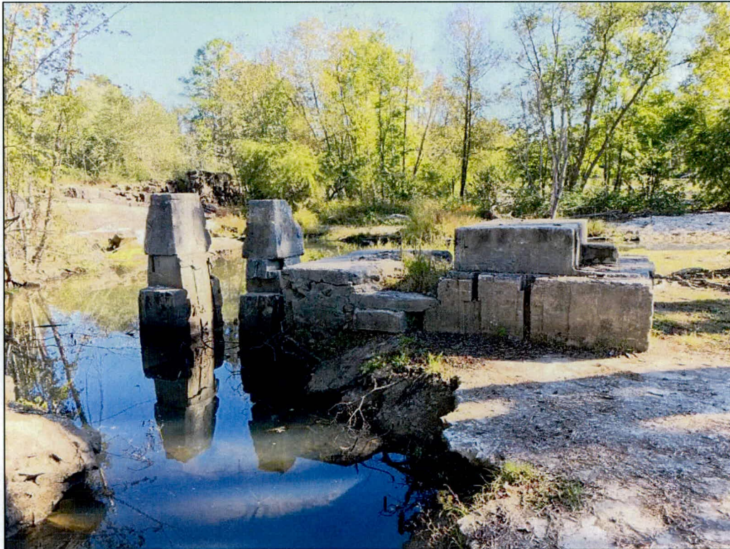
Photo 13: Foundation of Moore's Mill, facing east.
