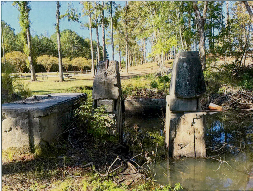
Photo 16: Foundation of Moore's Mill, facing west.
