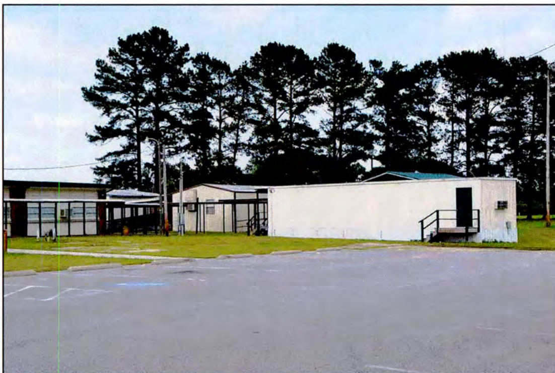
Figure 39. RB0701, Oxendine Elementary School, Portable Classroom 3, northwest and southwest elevations, view to the east.
