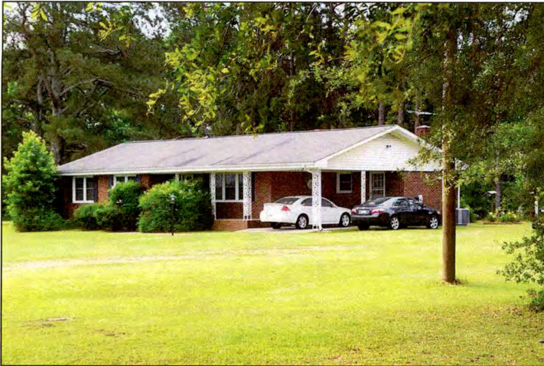
Figure 76. RB0708, dwelling carport, north and west elevations, view to the southeast.
