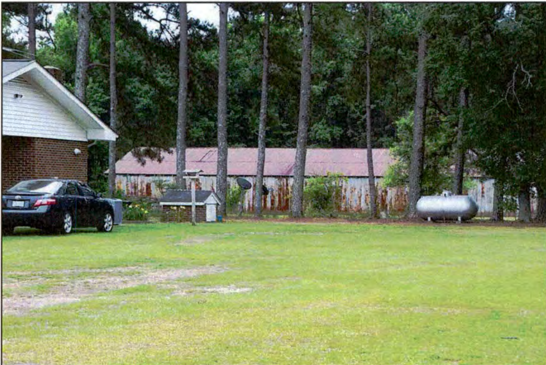
Figure 88. RB0709, barn, north elevation, view to the south-southeast.
