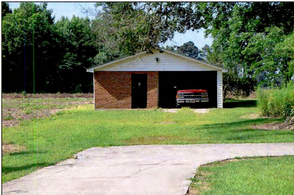
Figure 72. RB0707, garage, north elevation, view to the south.
