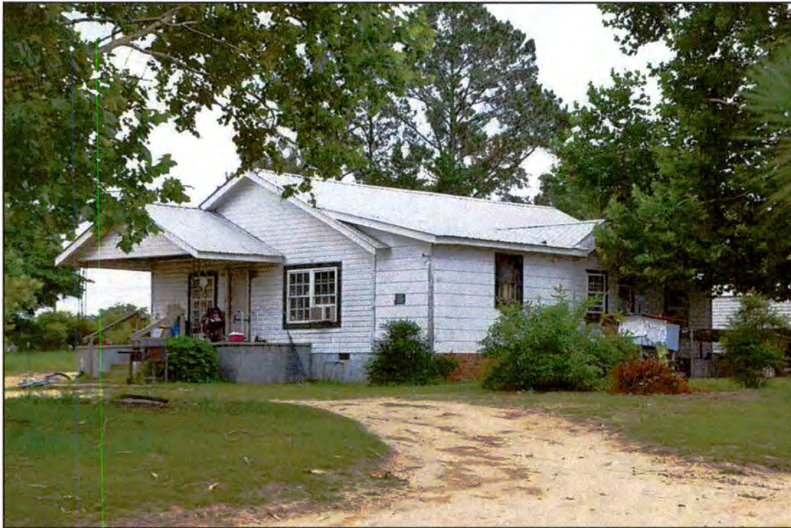
Figure 100. RB0713, dwelling addition, northwest and southwest elevations, view to the east.
