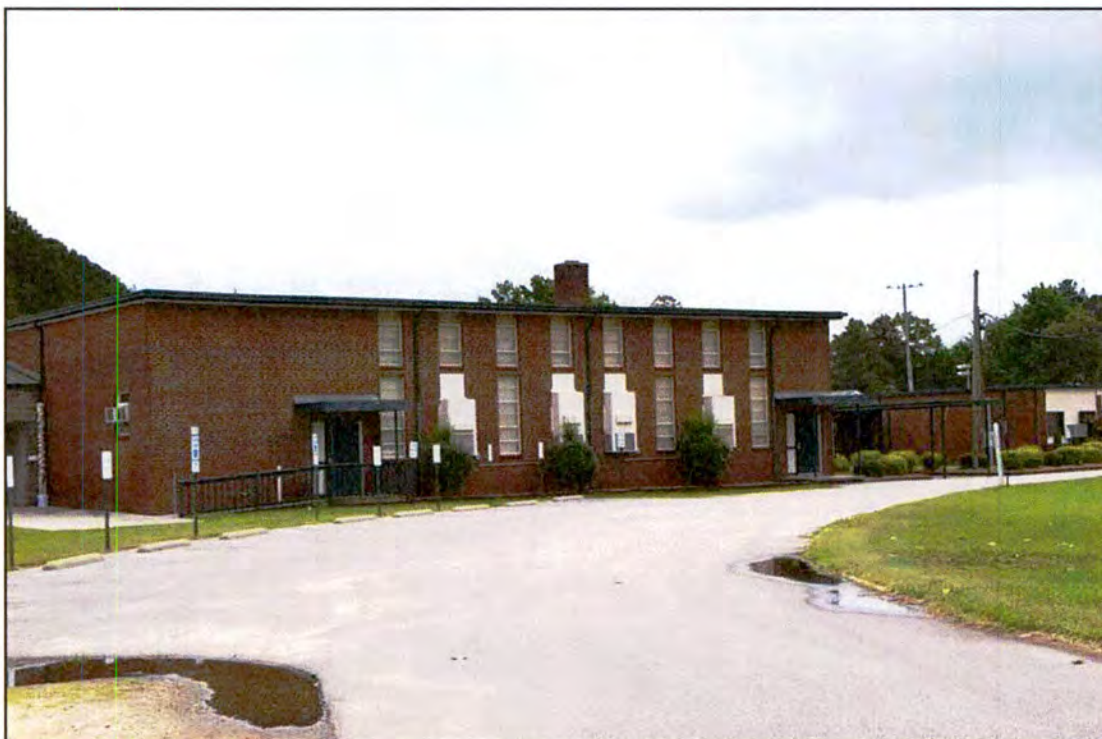
Figure 31. RB0701, Oxendine Elementary School, Addition 2, west and north elevations, view to the southeast.
