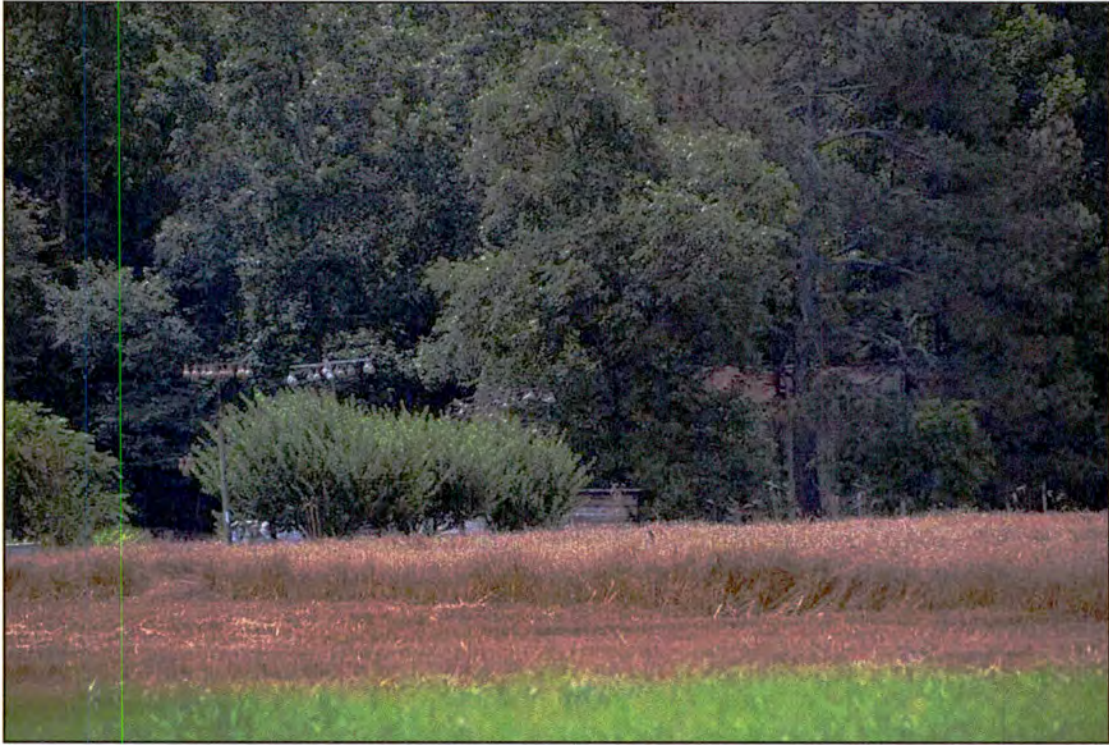
Figure 48. RB0702, outbuilding and shed, northwest and southwest elevations, view to the southeast.
