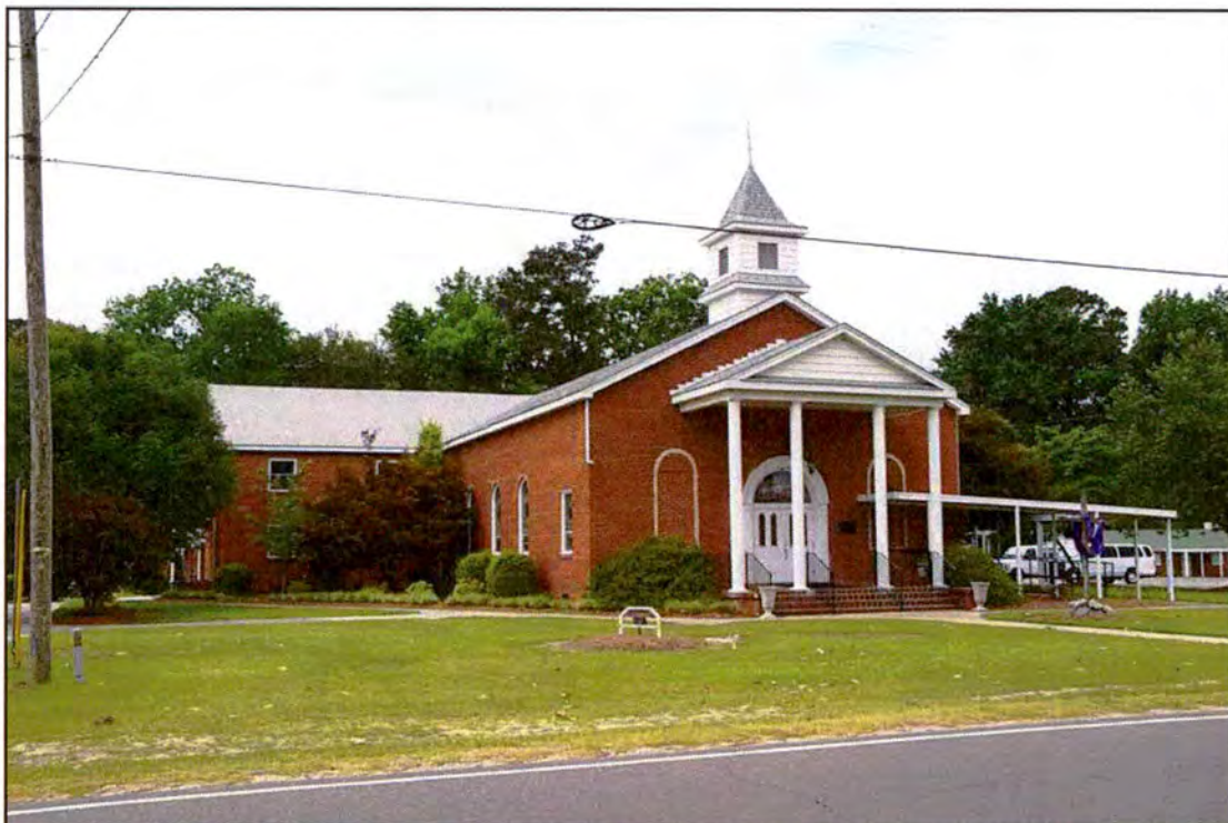
Figure 19. RB0700, Cherokee Chapel Holiness Methodist Church, oblique of east and south elevations, view to the northwest.
