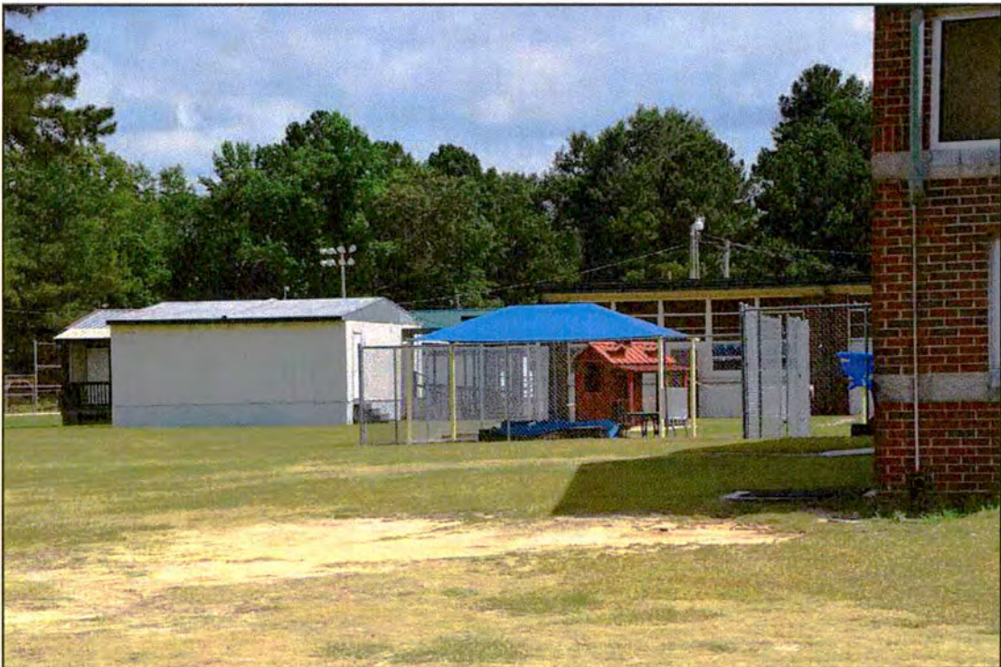
Figure 29. RB0701, Oxendine Elementary School, Addition 1, north elevation, view to the southeast.
