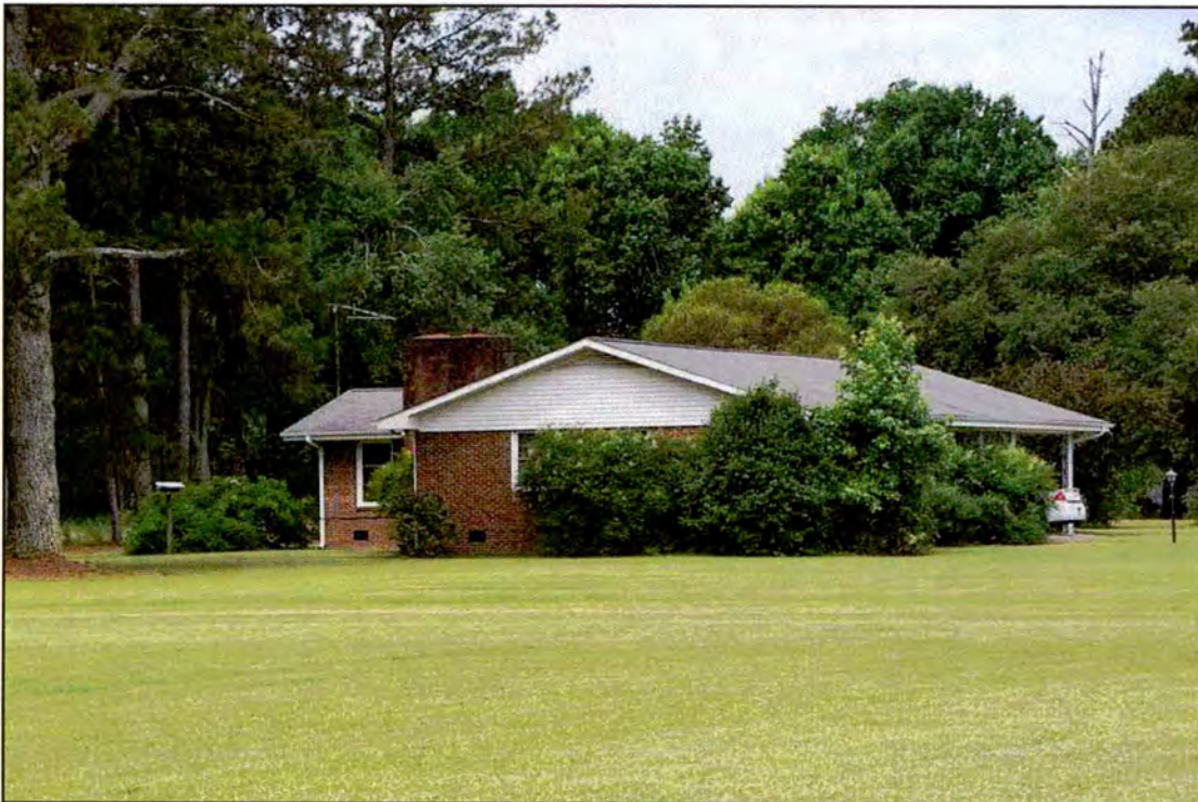
Figure 77. RB0708, dwelling addition, east elevation, view to the west-southwest.
