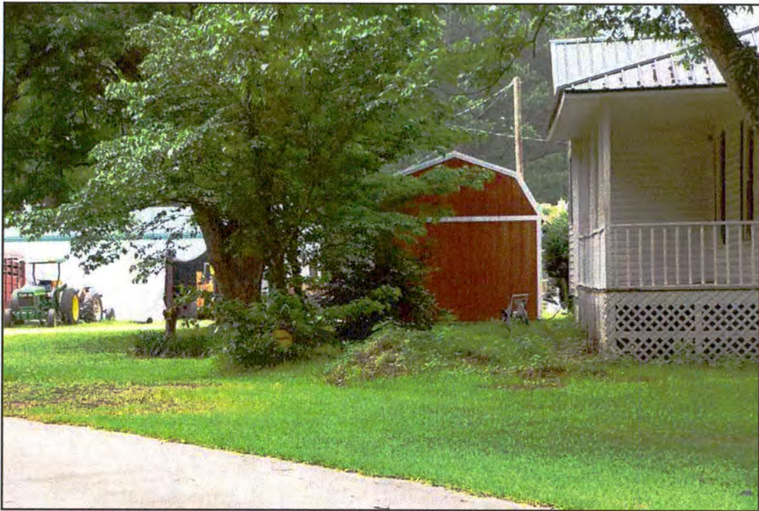
Figure 15. RB0699, Shed 1, north elevation, view to the south.
