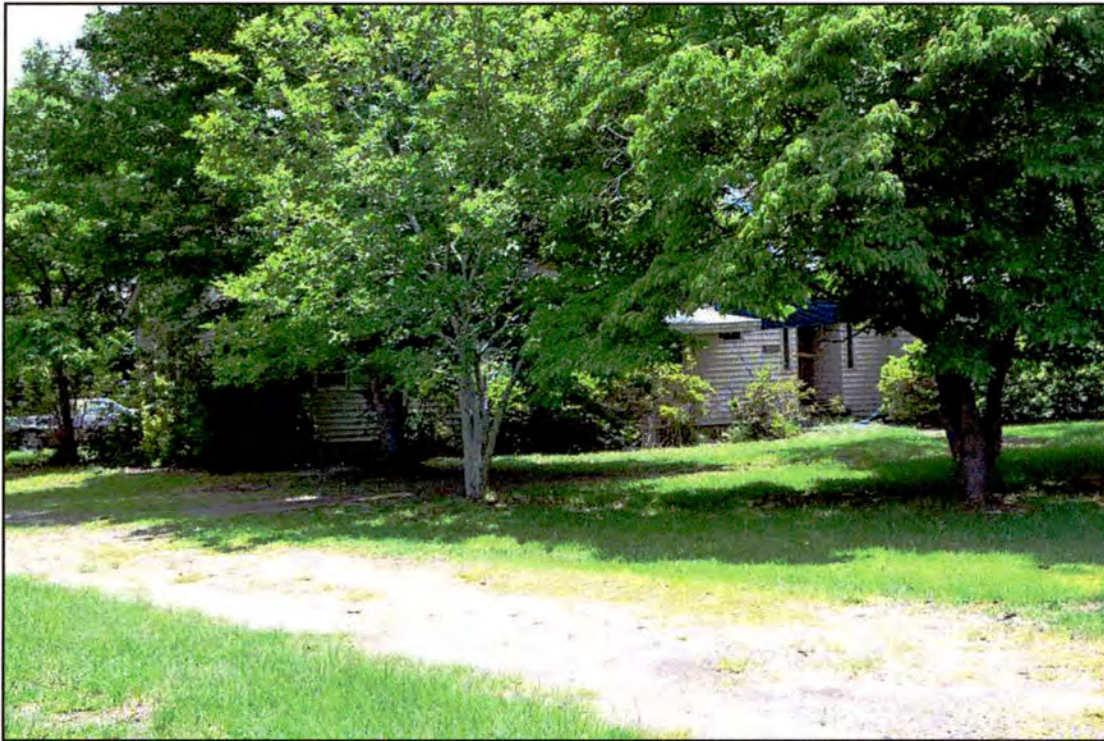
Figure 55. RB0704, dwelling, north and east elevations, view to the southwest.
