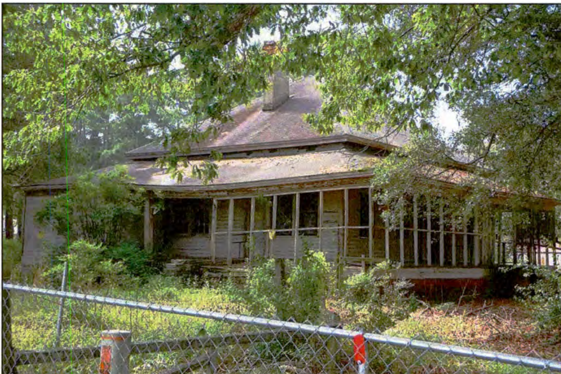
Figure 82. RB0709, dwelling, north and west elevations, view to the southeast.
