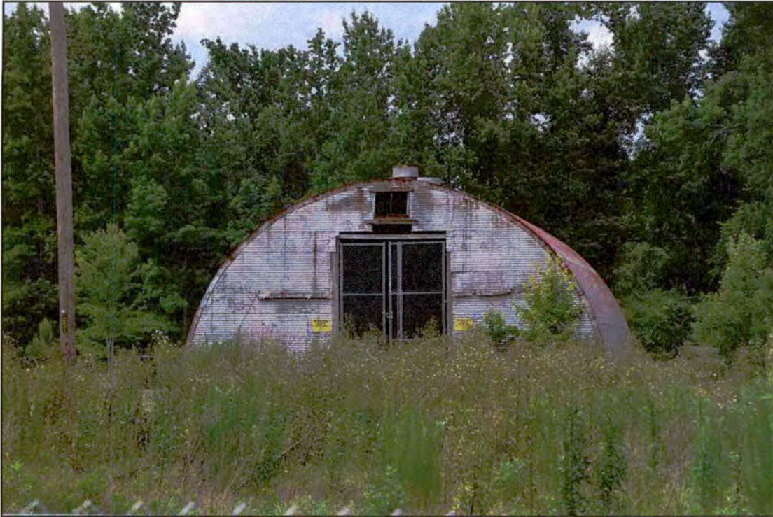
Figure 87. RB0709, pesticide storage structure, north elevation, view to the south.
