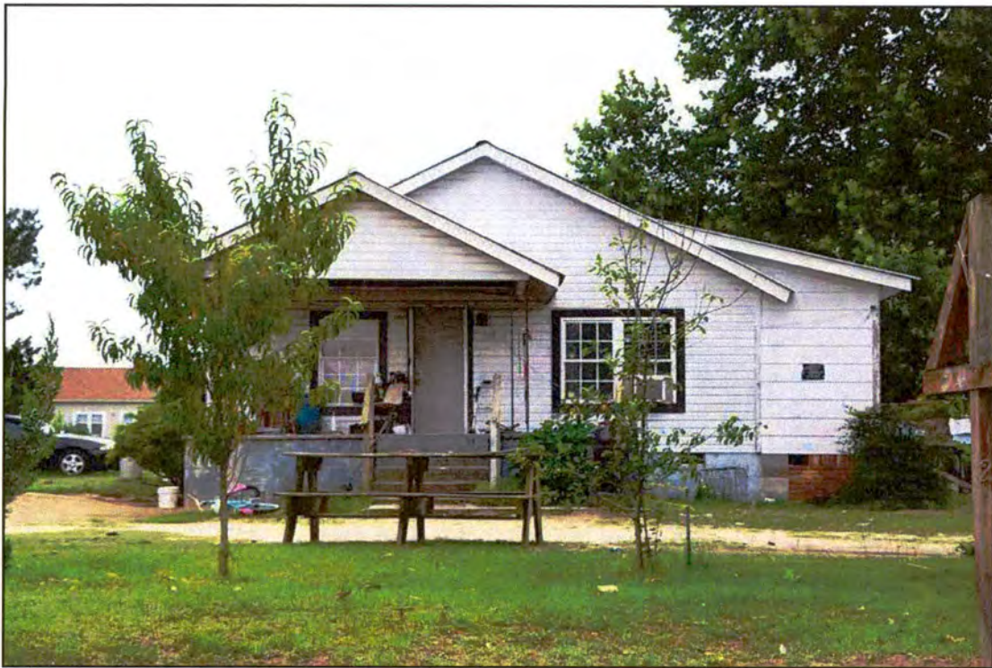
Figure 98. RB0713, dwelling, northwest elevation, view to the southeast.
