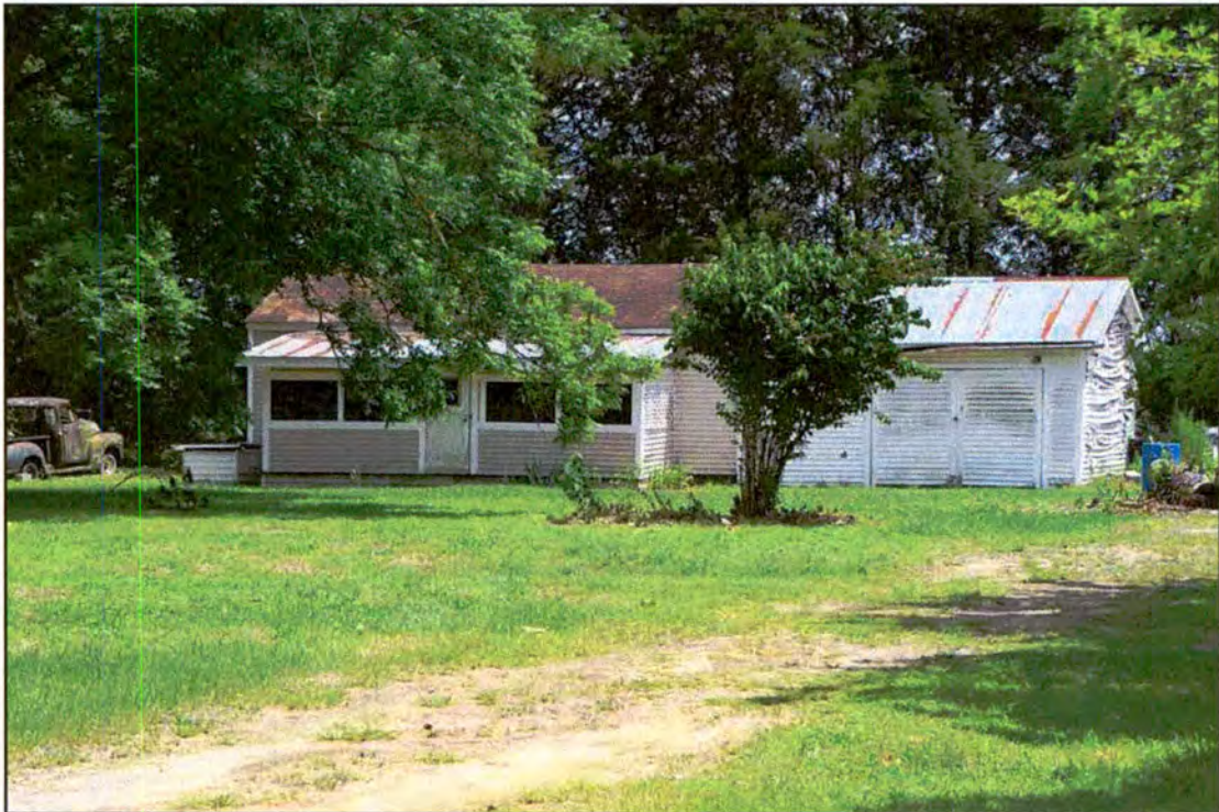
Figure 58. RB0704, outbuilding, north and west elevations, view to the southeast.
