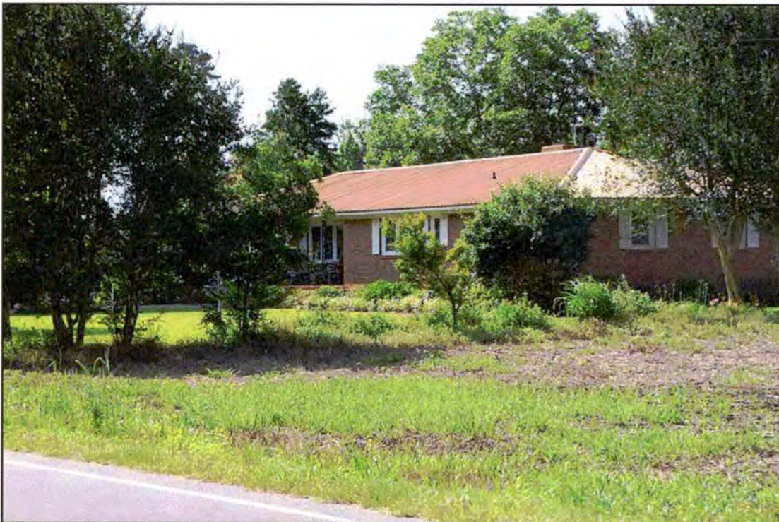
Figure 70. RB0707, dwelling, north and west elevations, view to the southeast.
