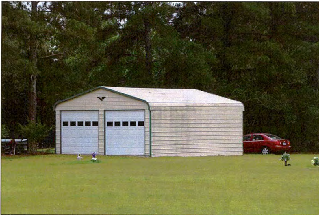
Figure 22. RB0700, garage, oblique of east and north elevations, view to the southwest.
