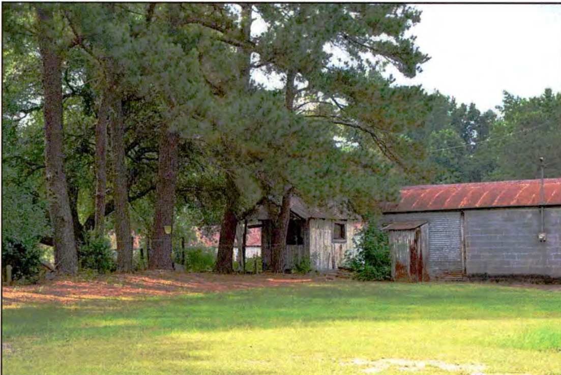
Figure 84. RB0709, shed, north and west elevations, view to the southeast.
