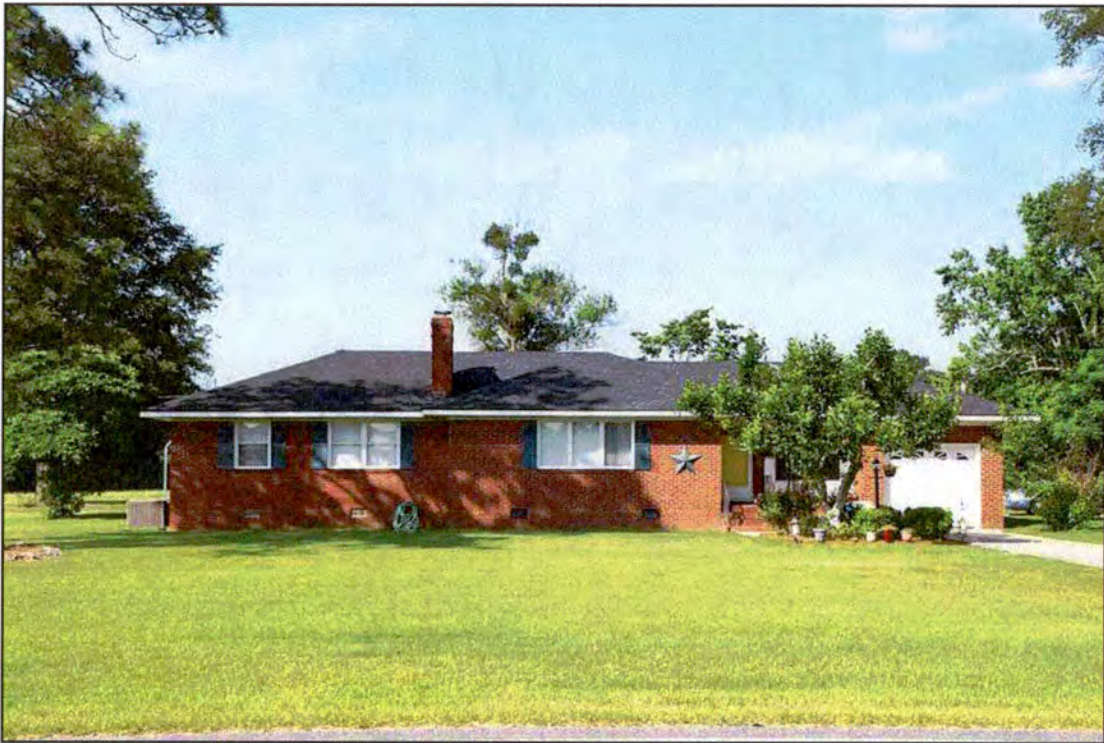
Figure 63. RB0706, dwelling, northeast elevation, view to the southwest.
