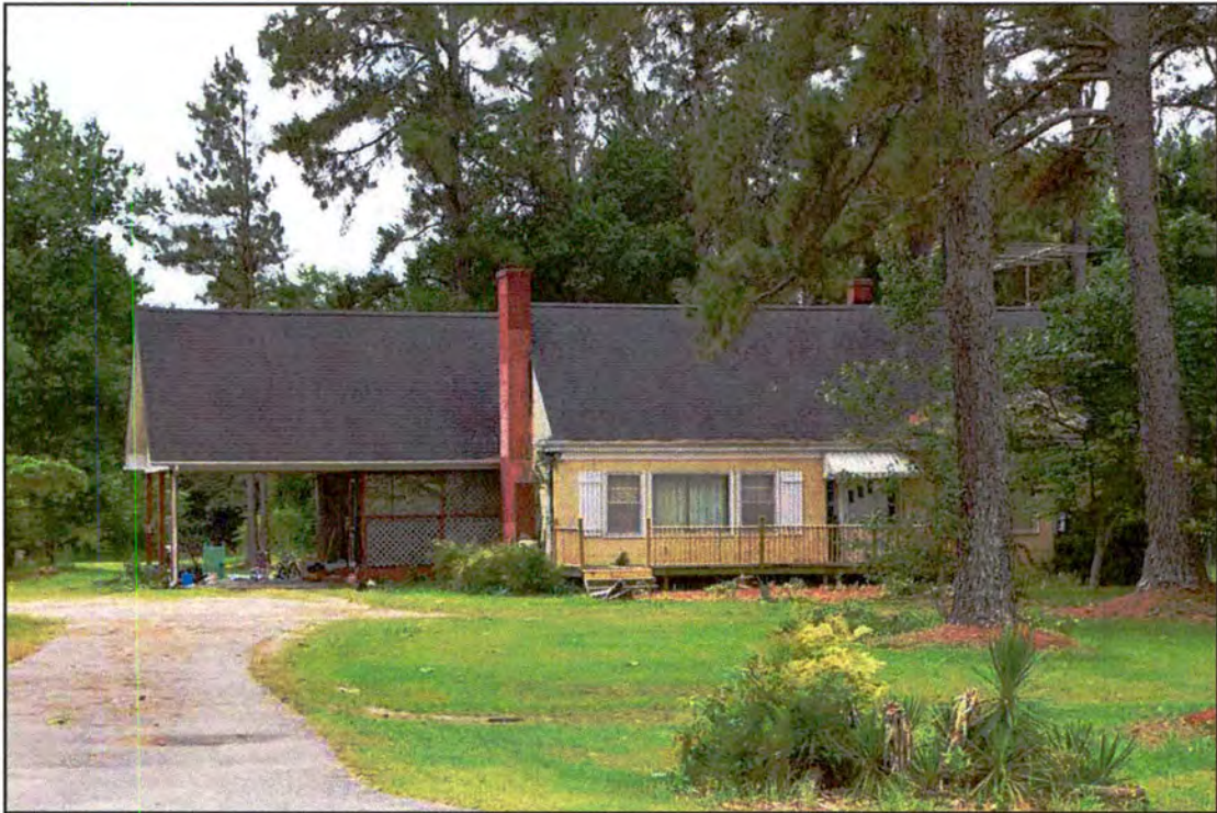
Figure 51. RB0703, dwelling, north and east elevations, view to the south-southeast.
