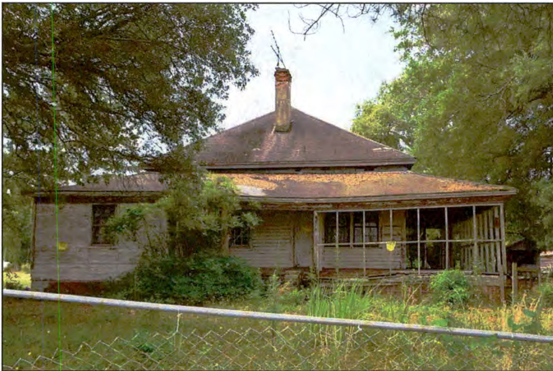
Figure 81. RB0709, dwelling, north elevation, view to the south.
