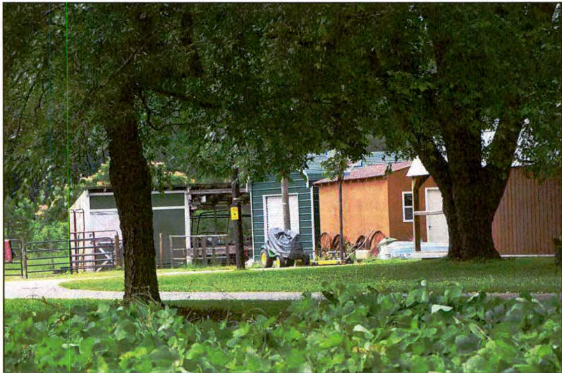
Figure 14. RB0699, Equipment Shelter, Garage 2, Shed 2, north and east elevations, view to the southwest.
