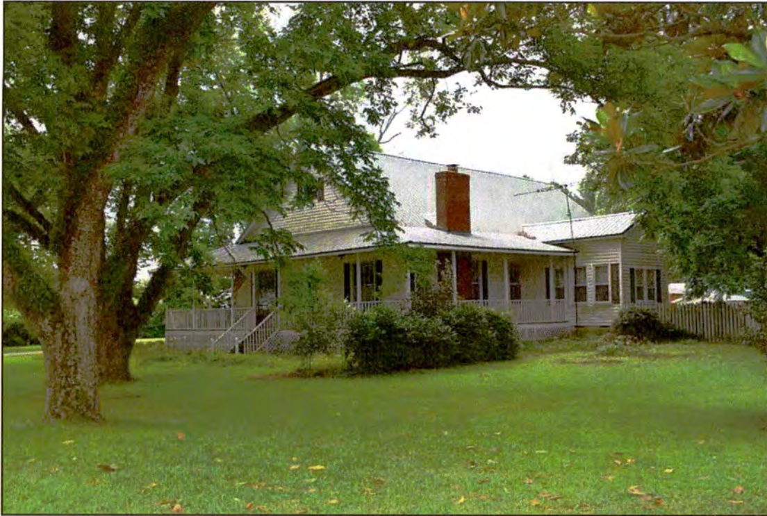
Figure 11. RB0699, dwelling addition, north and west elevations, view to the southeast.
