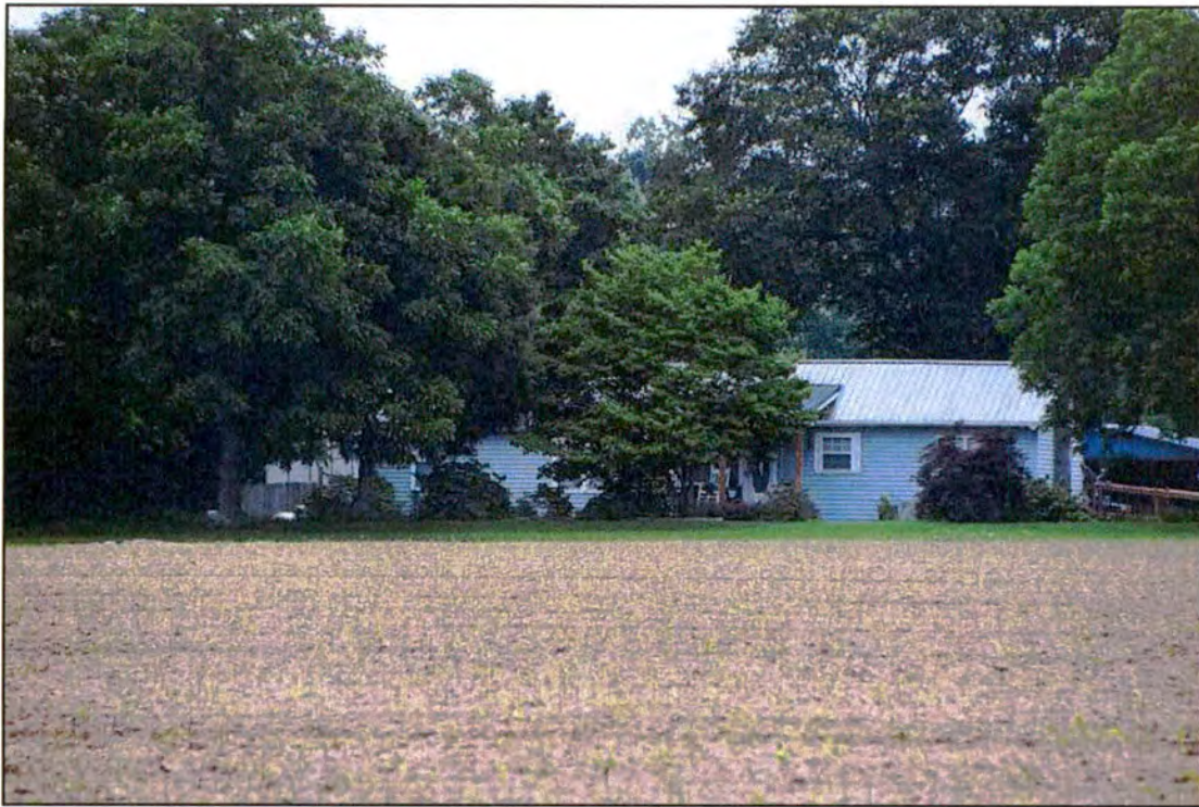
Figure 92. RB0711, dwelling, north elevation, view to the south.
