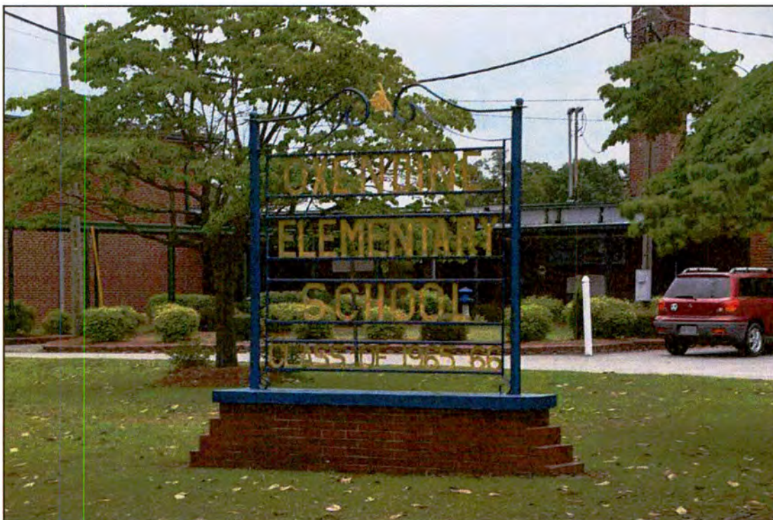
Figure 30. RB0701, Oxendine Elementary School, porch addition, west elevation, view to the east-northeast.
