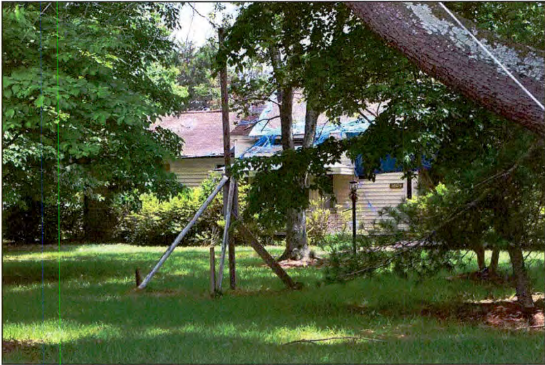
Figure 57. RB0704, dwelling (original blocks), north elevation, view to the southeast.
