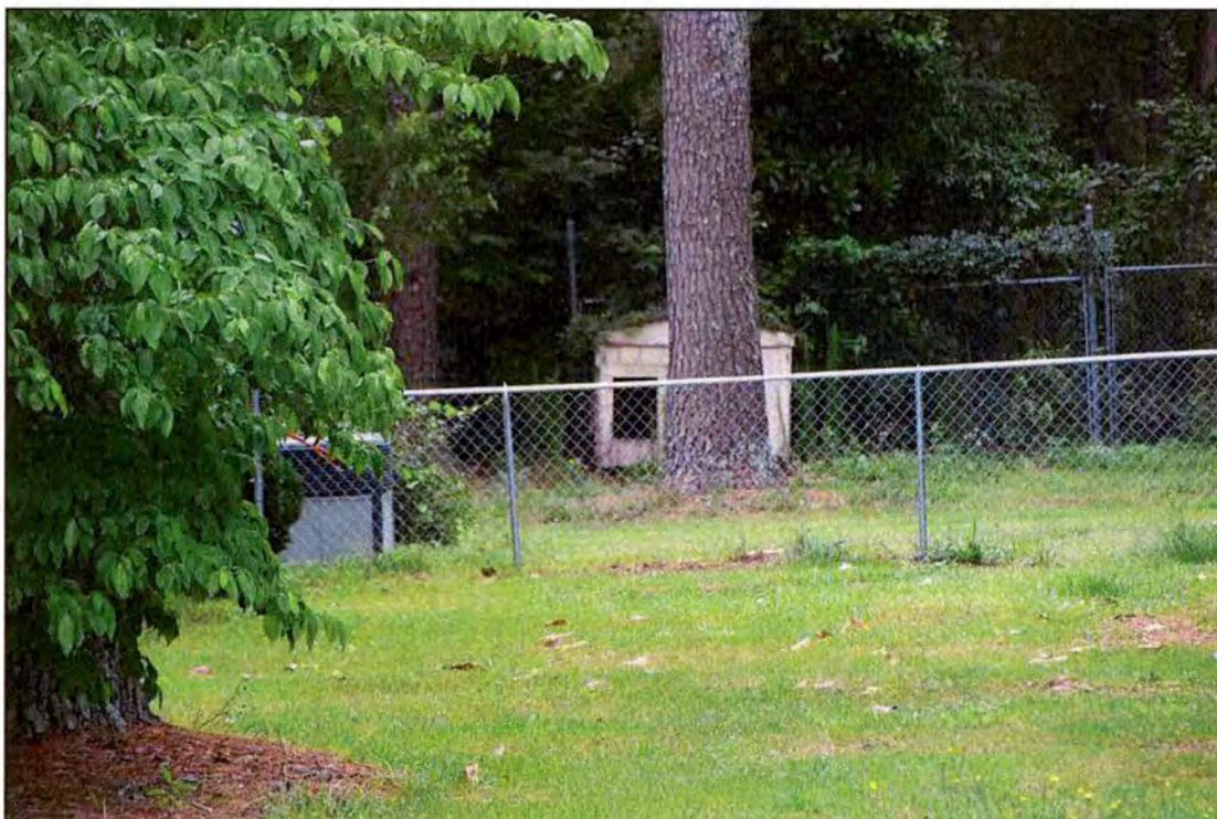
Figure 53. RB0703, outbuilding, north elevation, view to the south.
