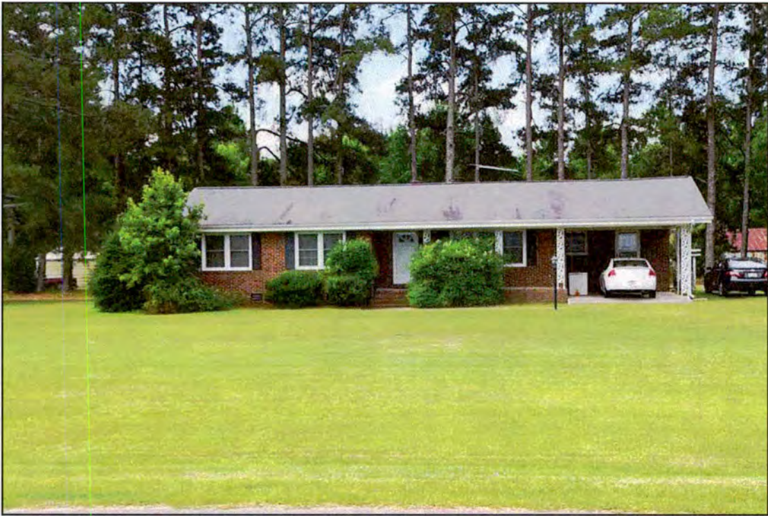
Figure 74. RB0708, dwelling, north elevation, view to the south.
