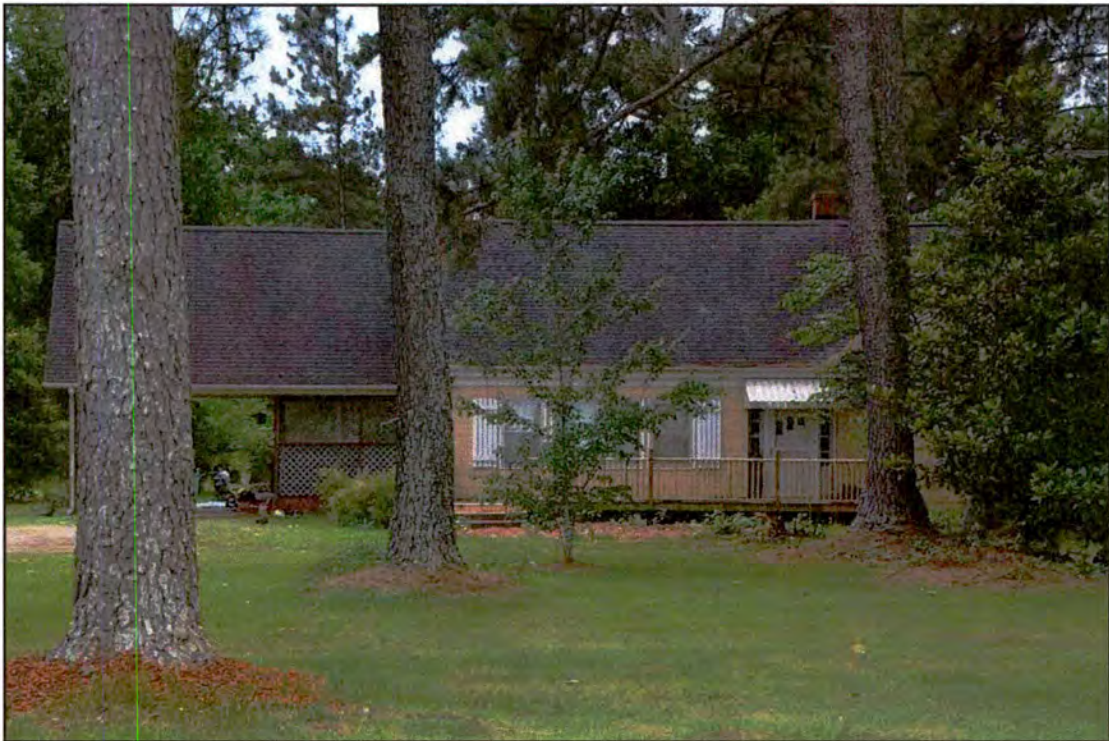
Figure 52. RB0703, dwelling, north elevation, view to the south.
