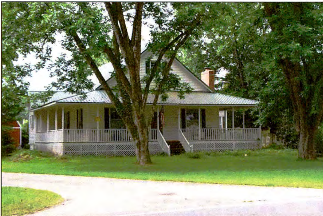
Figure 12. RB0699, dwelling addition, north and east elevations, view to the south-southwest.
