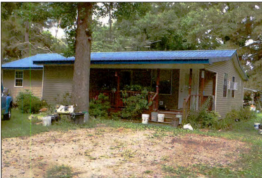
Figure 6. RB0698, dwelling, north and east elevations, view to the southwest.
