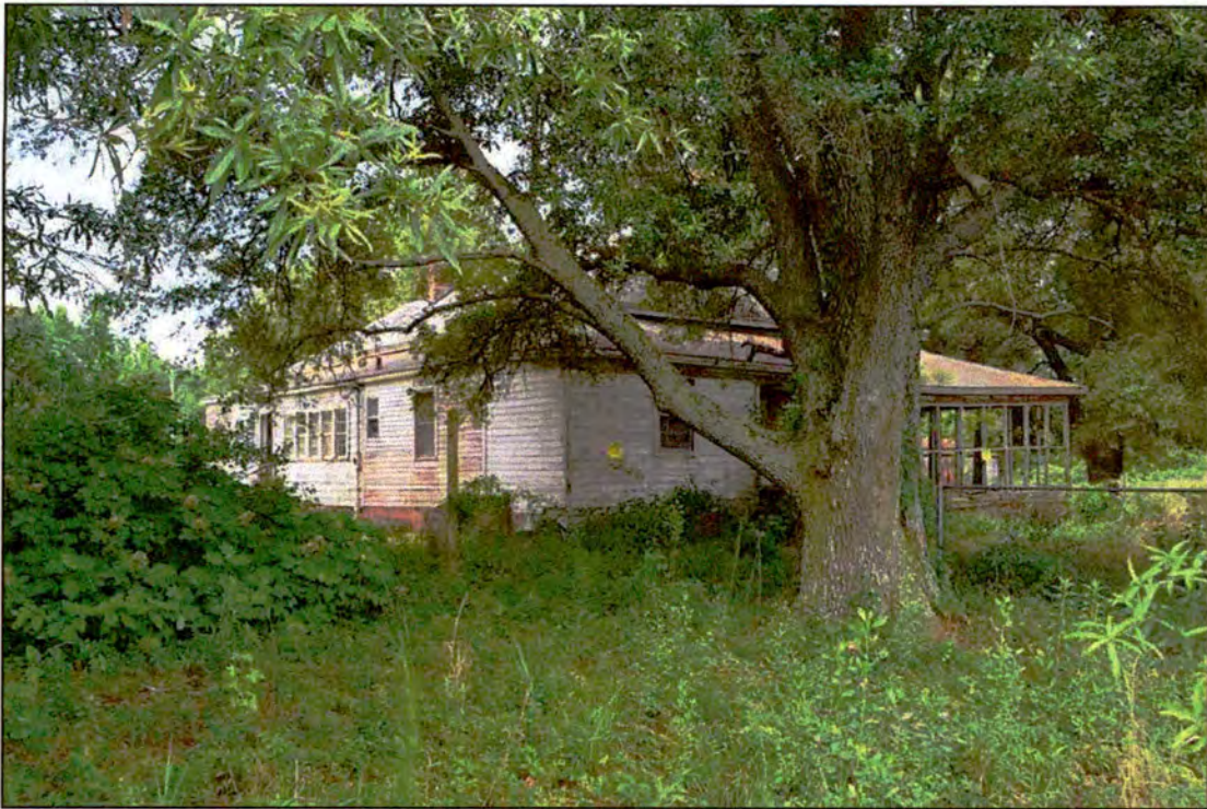
Figure 83. RB0709, dwelling, north and east elevations, view to the southwest.
