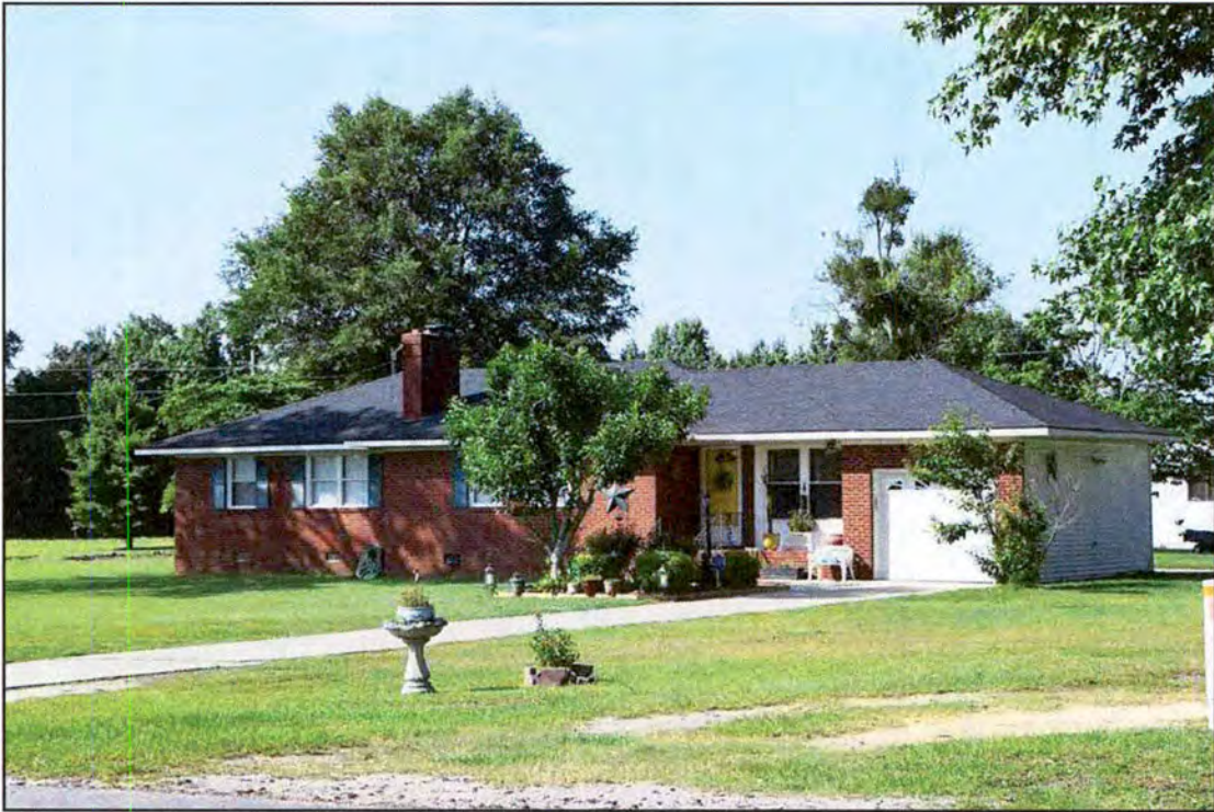
Figure 65. RB0706, dwelling addition, northeast and northwest elevations, view to the south.
