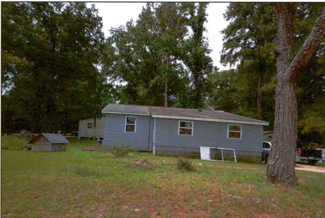
Figure 3. RB0697, dwelling addition, north elevation, view to the south.
