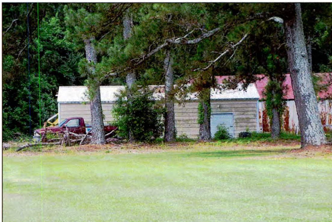
Figure 79. RB0708, garage, north elevation, view to the south.
