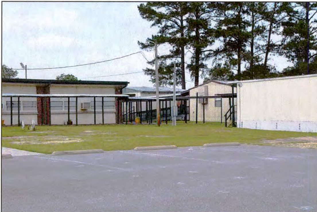
Figure 41. RB0701, Oxendine Elementary School, Portable Classroom 5, west elevation, view to the northeast.
