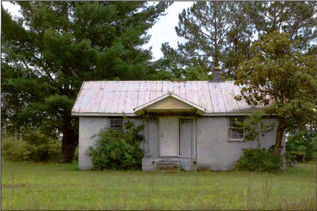
Figure 95. RB0712, dwelling, northwest elevation, view to the southeast.
