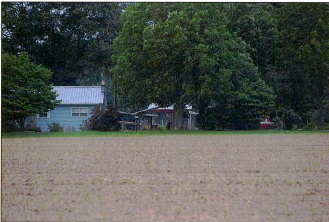
Figure 93. RB0711, Outbuildings 1, 2, and 3 from NC-17, view to the south.
