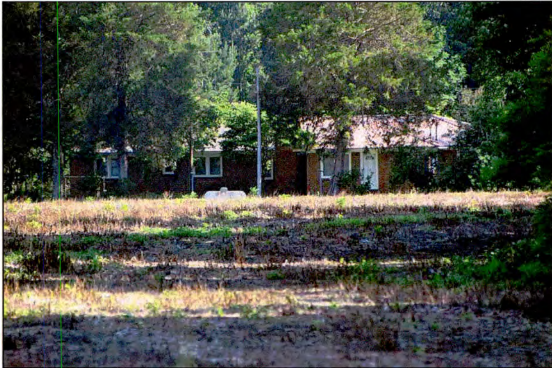
Figure 71. RB0707, dwelling rear addition, south elevation, view to the north.
