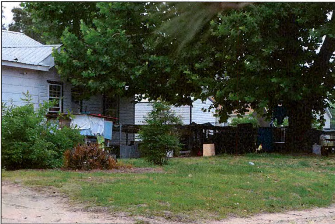
Figure 102. RB0713, shed and chicken coop, northwest and southwest elevations, view to the east.
