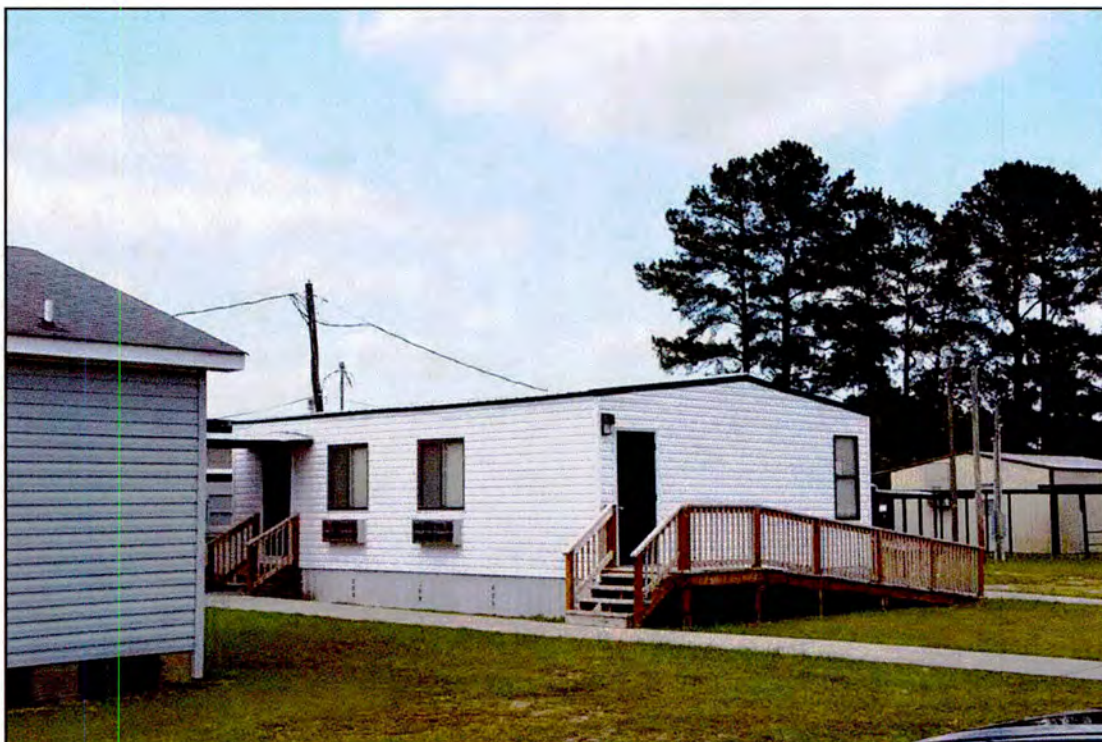
Figure 38. RB0701, Oxendine Elementary School, Portable Classroom 2, south and west elevations, view to the northeast.
