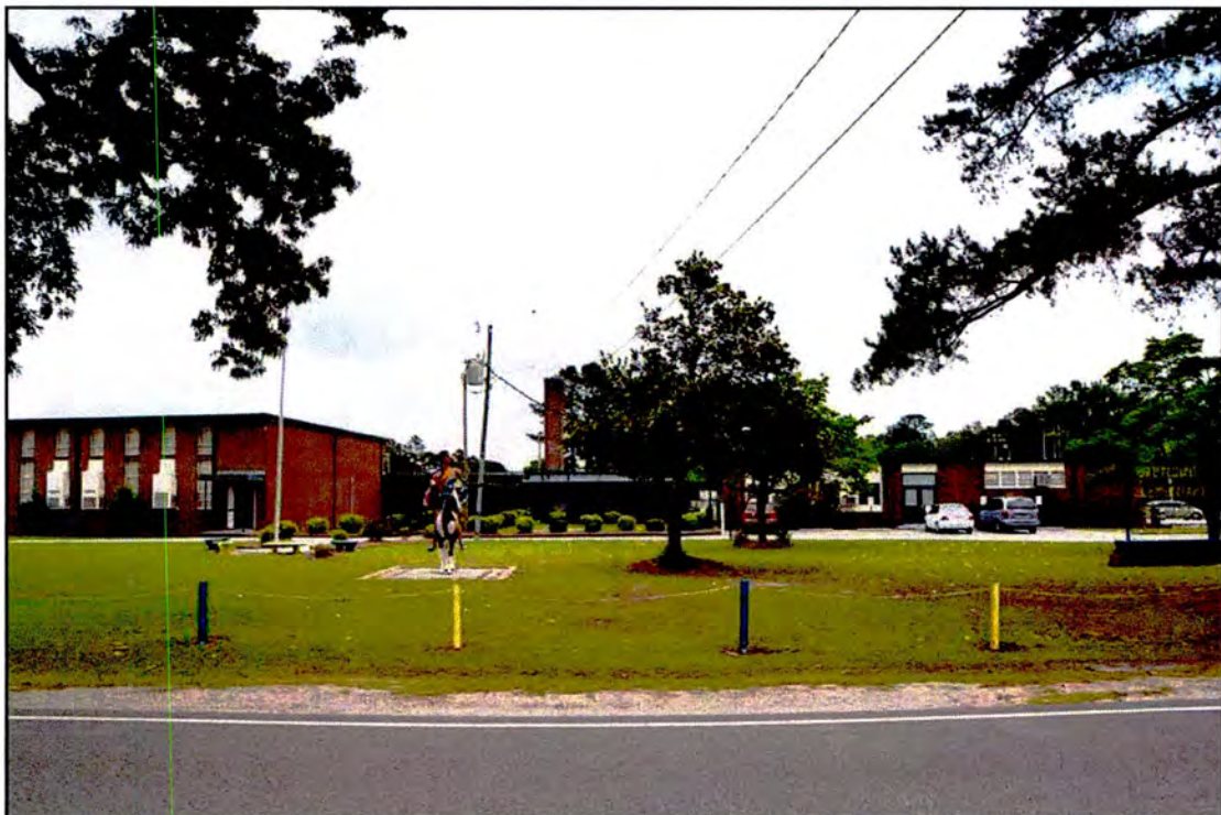
Figure 27. RB0701, Oxendine Elementary School, original block with chimney stack, west elevation, view to the east.
