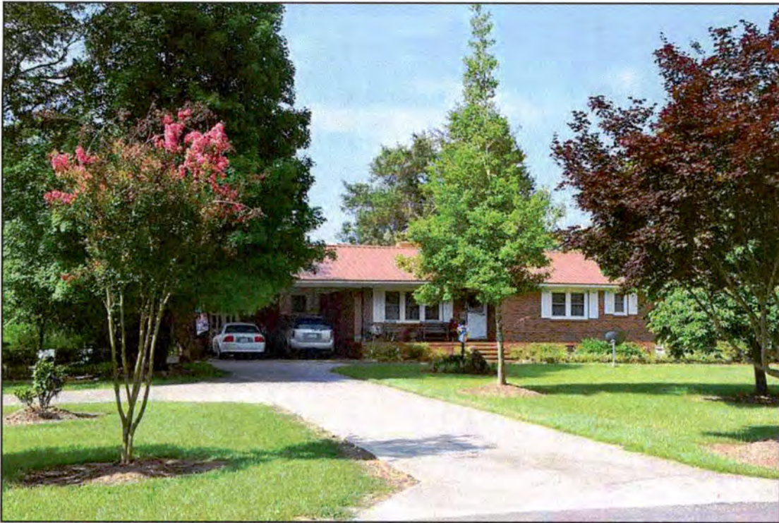
Figure 69. RB0707, dwelling, north elevation, view to the south-southwest.
