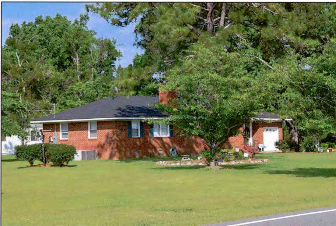
Figure 64. RB0706, dwelling, northeast and southeast elevations, view to the west.
