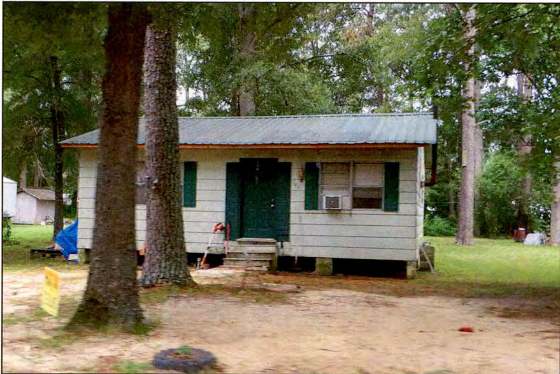
Figure 61. RB0705, dwelling, north and east elevations, view to the southwest.
