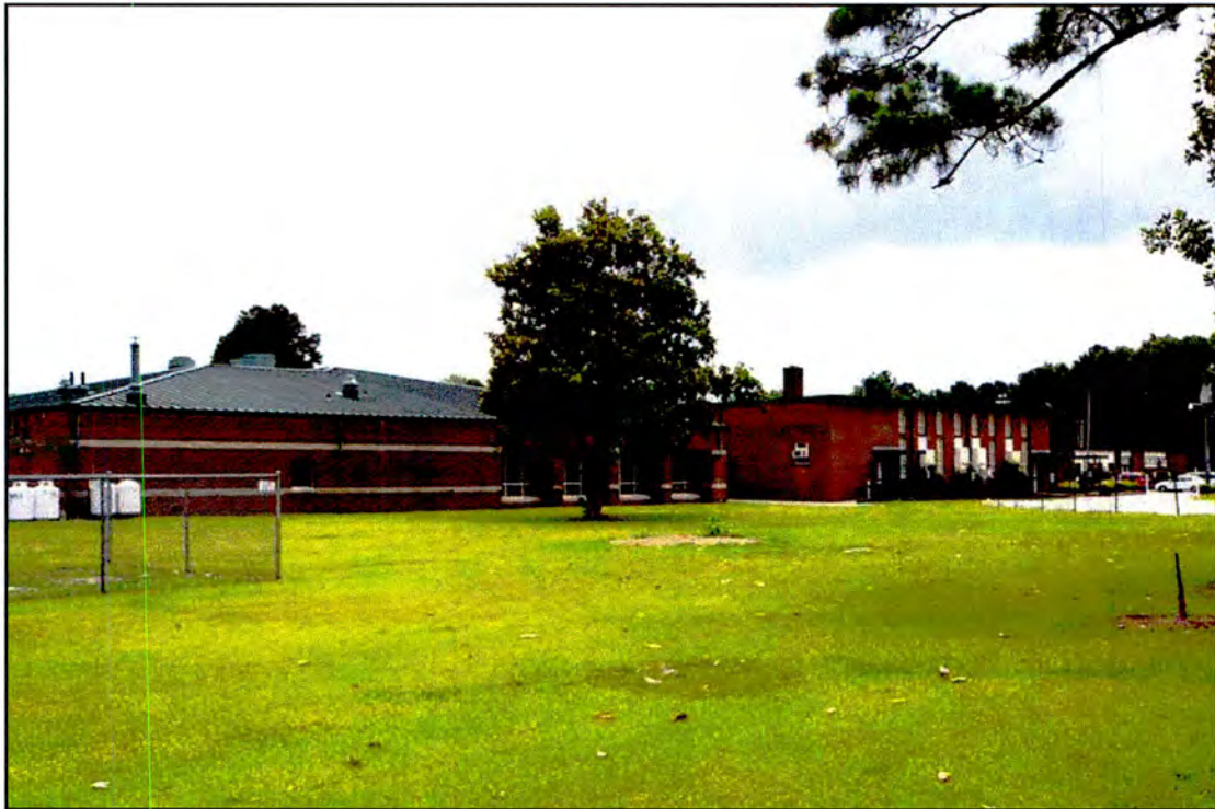
Figure 26. RB0701, Oxendine Elementary School, overview, west and north elevations, view to the southeast.
