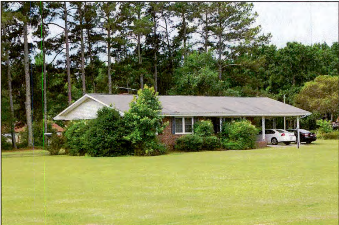
Figure 75. RB0708, dwelling, north and east elevations, view to the southwest.
