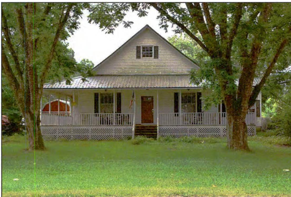
Figure 9. RB0699, dwelling, north elevation, view to the south.
