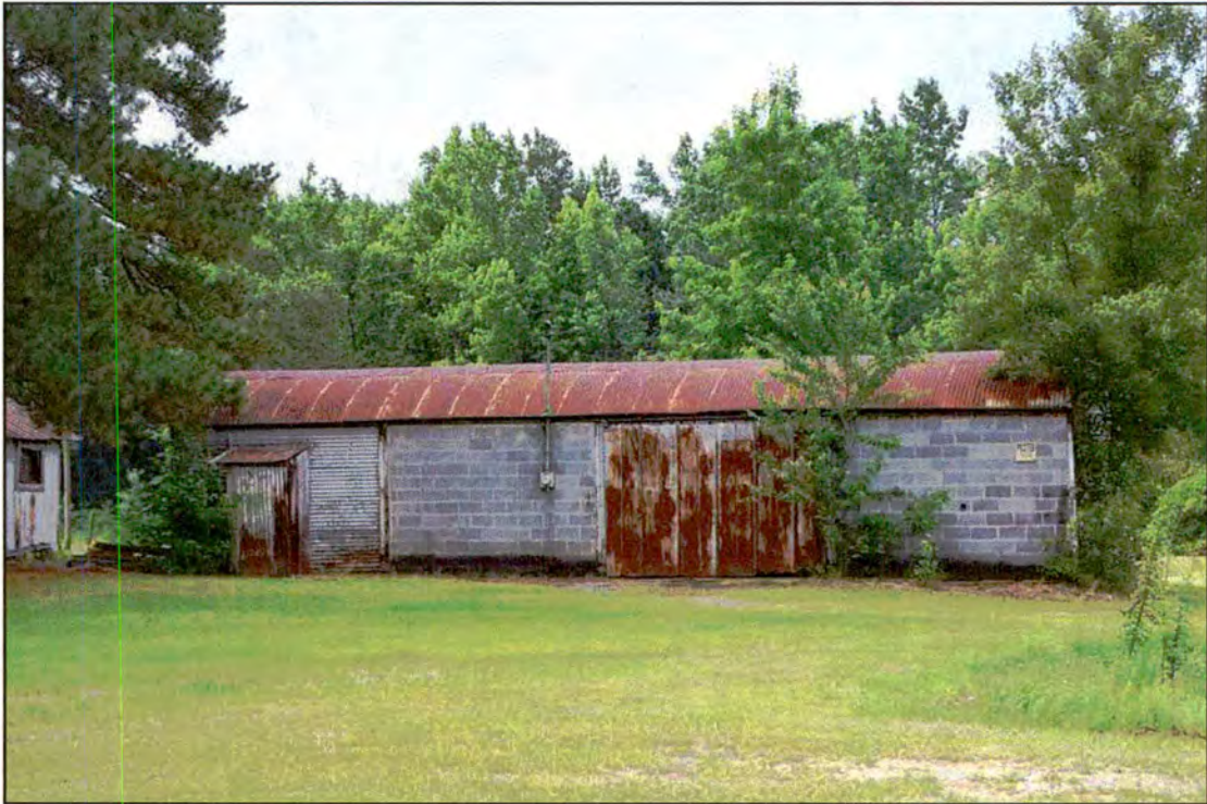
Figure 85. RB0709, bunker silo, north elevation, view to the south.
