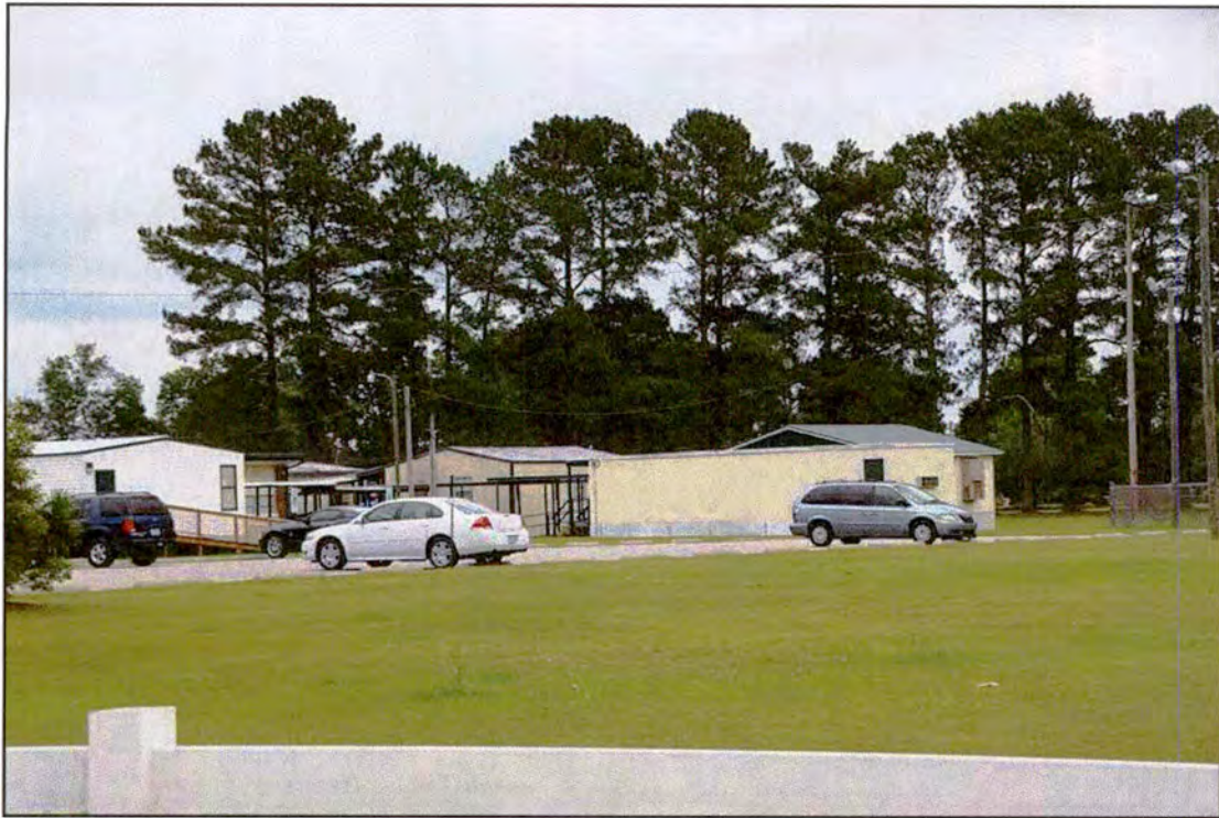
Figure 40. RB0701, Oxendine Elementary School, partial view of Portable Classroom 4, northwest and southwest elevations, view to the east.
