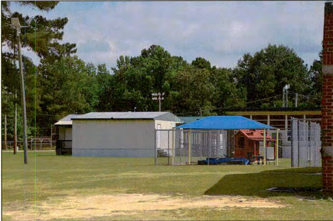
Figure 42. RB0701, Oxendine Elementary School, Portable Classroom 6, north and west elevations, view to the southeast.
