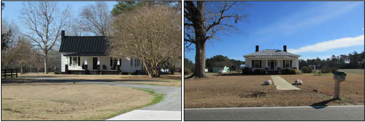
Photo 18: View of 849 Nor-Am Road (Left) and 194 Nor-Am Road (Right).
