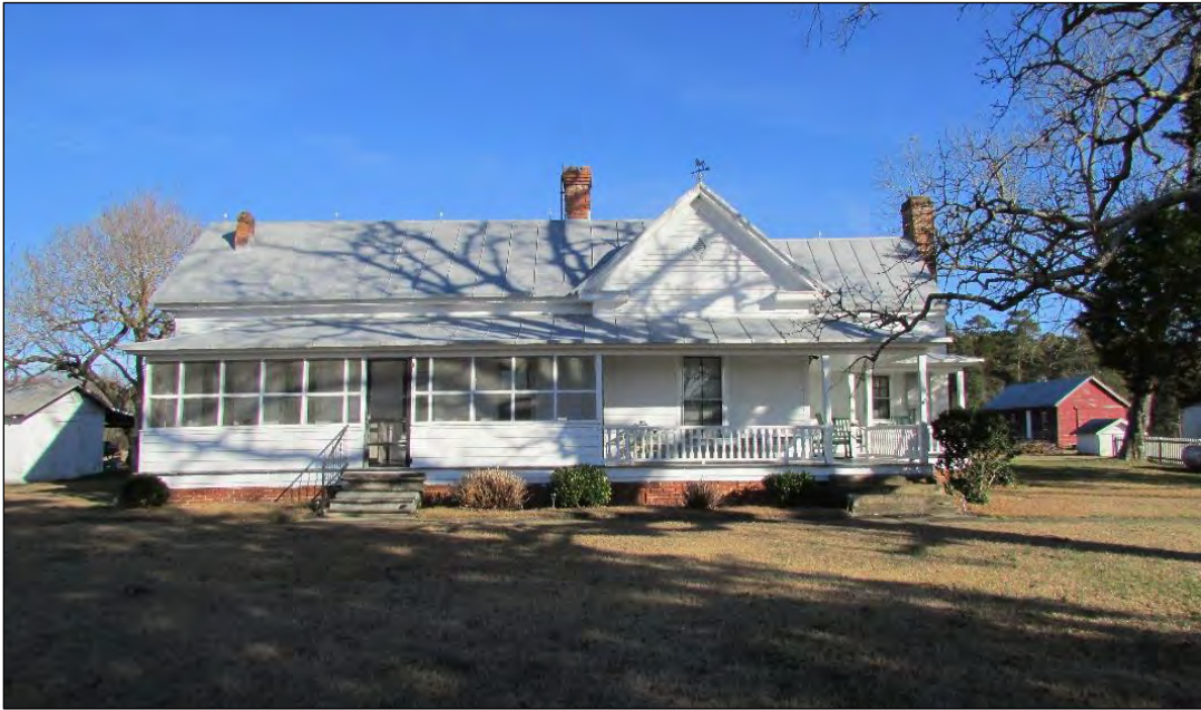
Photo 1: Primary (South) Elevation of Deans House.
