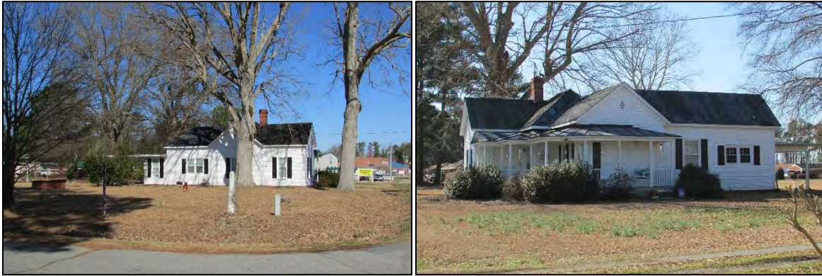
Photo 20: View of 617 NC 581 Road from the south side (Left) and the north side (Right).
