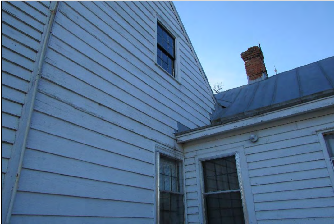
Photo 7: View of Original Core Attached to Additions, Looking Southeast.
