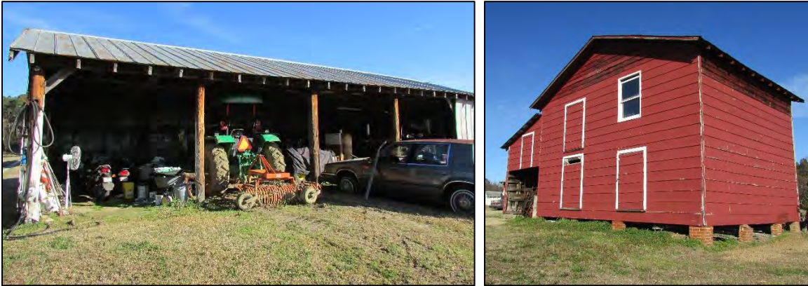
Photo 12: Primary (South) Elevation of Open Garage, Looking North (Left) and Northwest Oblique of Barn, Looking Northwest (Right).
