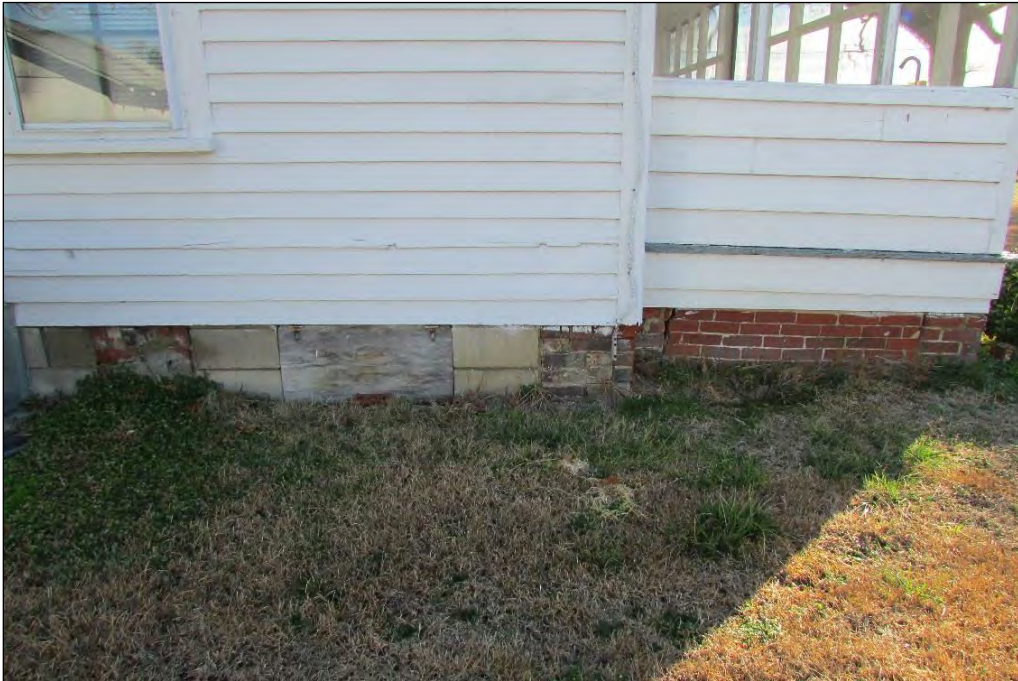
Photo 3: Detail of Concrete, Wood, and Brick Foundation, Looking West.
