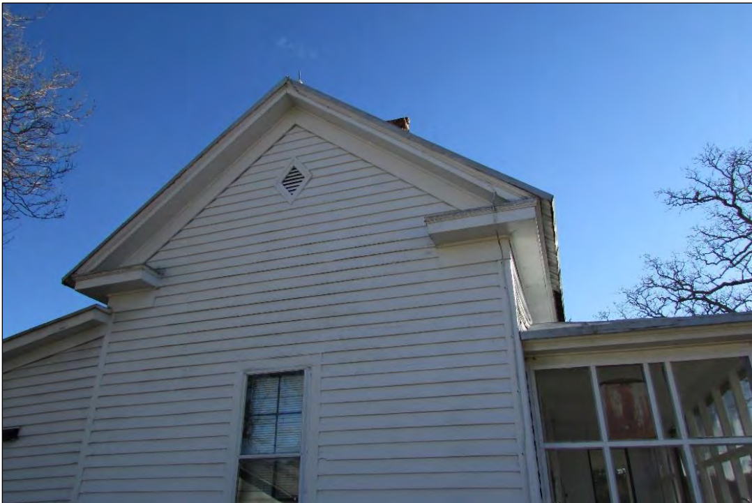
Photo 2: Detail of Vent in Gable End, Looking East.
