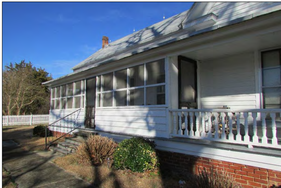
Photo 6: View of Doors on the Screened-in-Porch, Looking Northwest.
