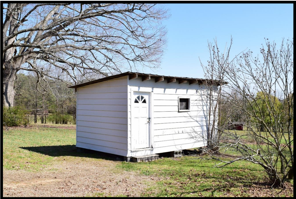
Figure 16: Storage Shelter, Looking East.
