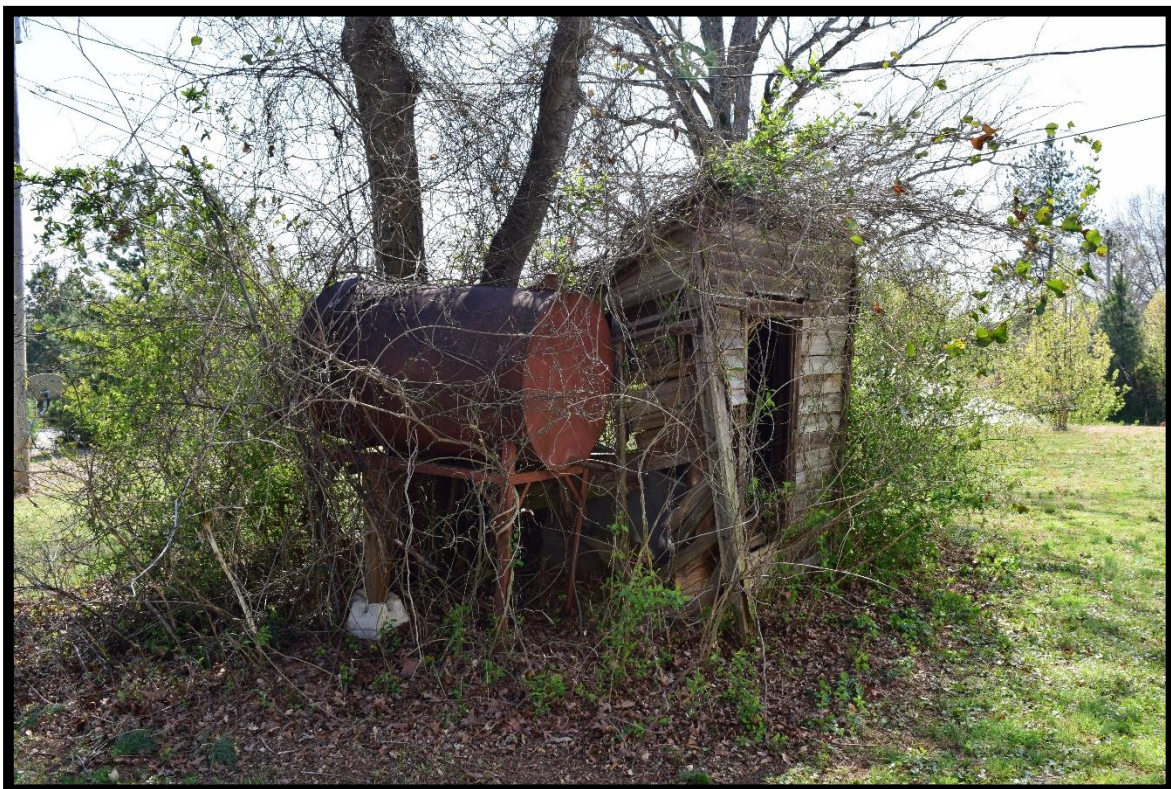
Figure 14: Shed and Tank, Looking South.
