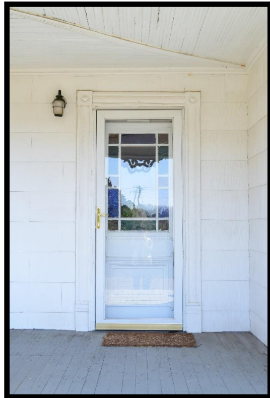
Figure 6: Sustar House, Entry Door.
