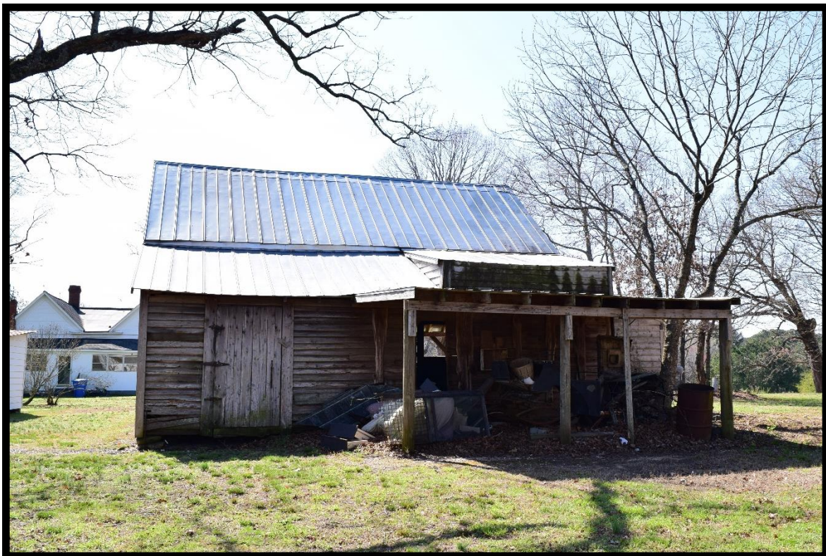
Figure 18: Storage Shelter, Looking Southwest.
