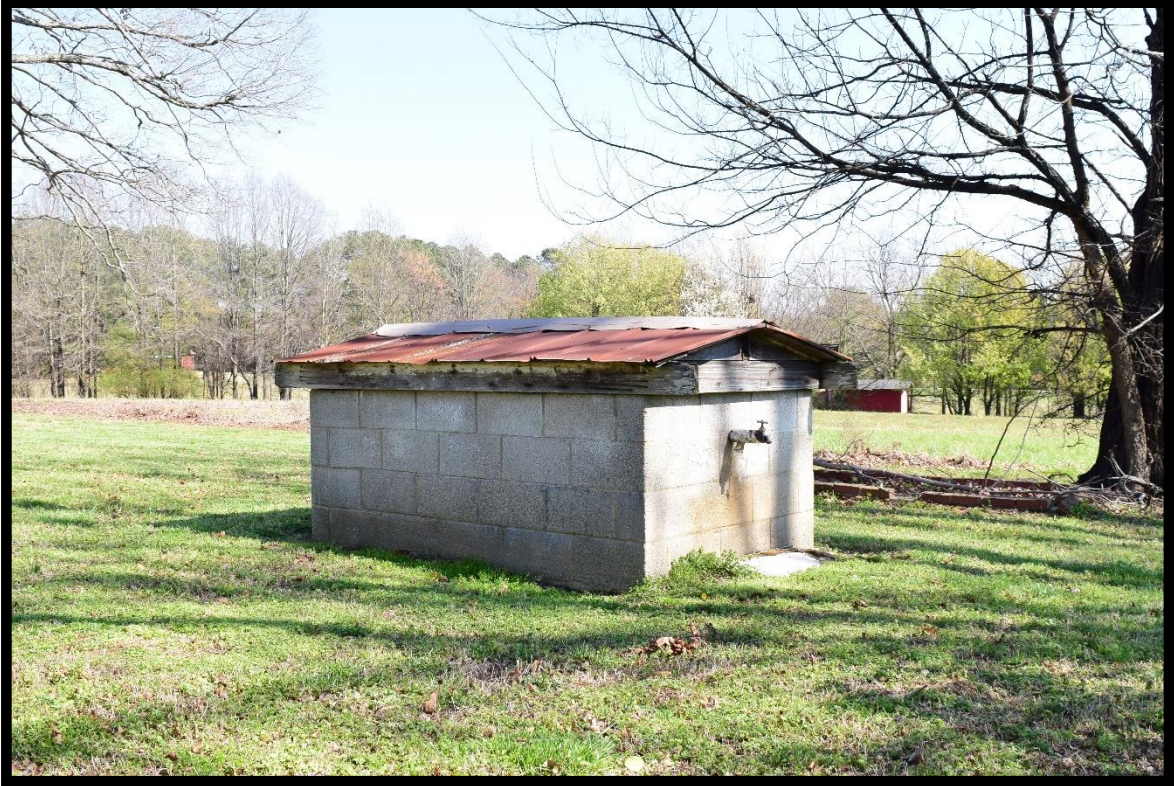
Figure 15: Well-shelter, Looking East.
