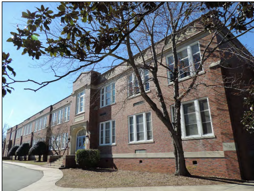
Figure 12: Facing southwest to façade
