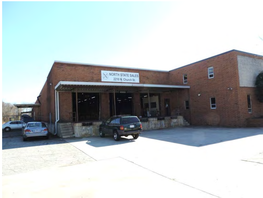
Figure 85. Facing southeast to loading dock and office block's north elevation
