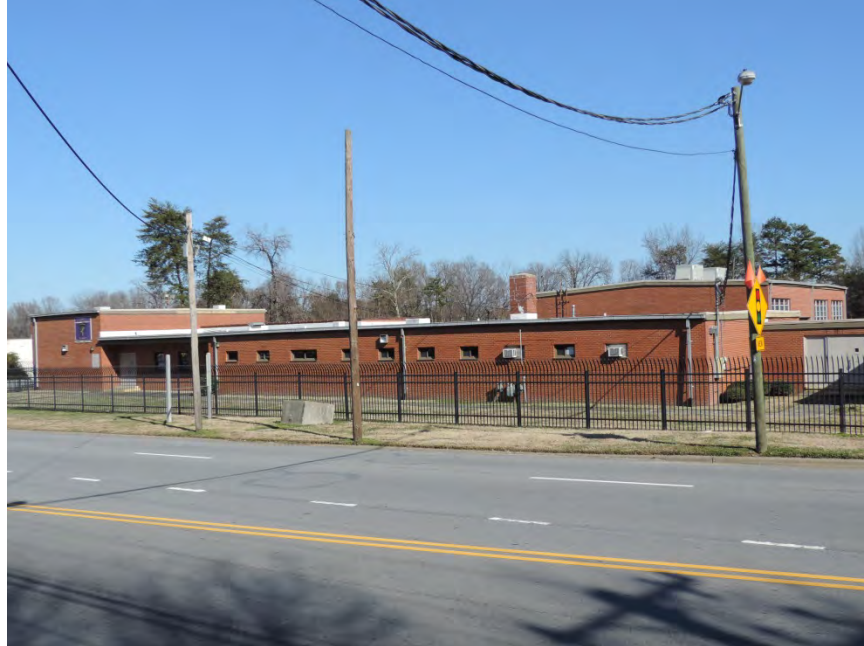
Figure 101. Facing northeast from North Church Street to main building; assembly hall visible to rear
