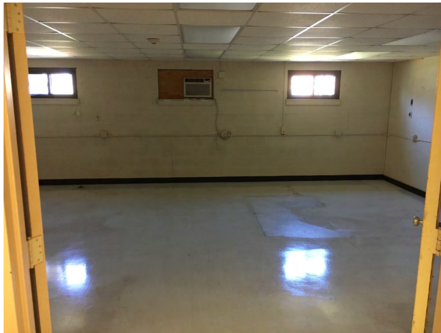
Figure 108. Main building representative classroom (Source: ALPHA Facilities Solutions)
