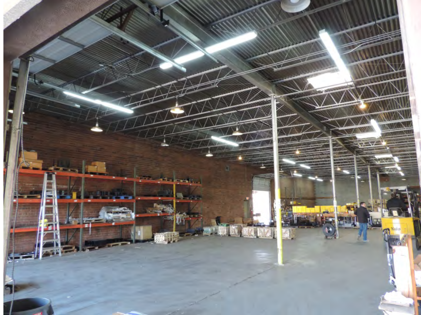
Figure 90. Representative interior view
