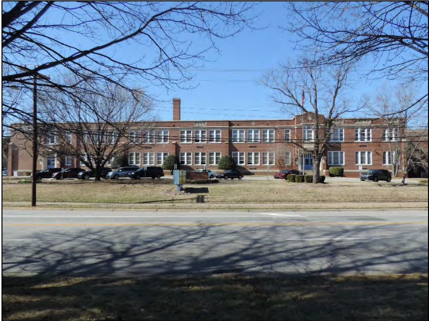
Figure 14: Facing northwest from North Church Street to main block’s façade
