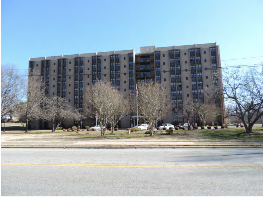
Figure 54. Facing east to Hall Towers from North Church Street
