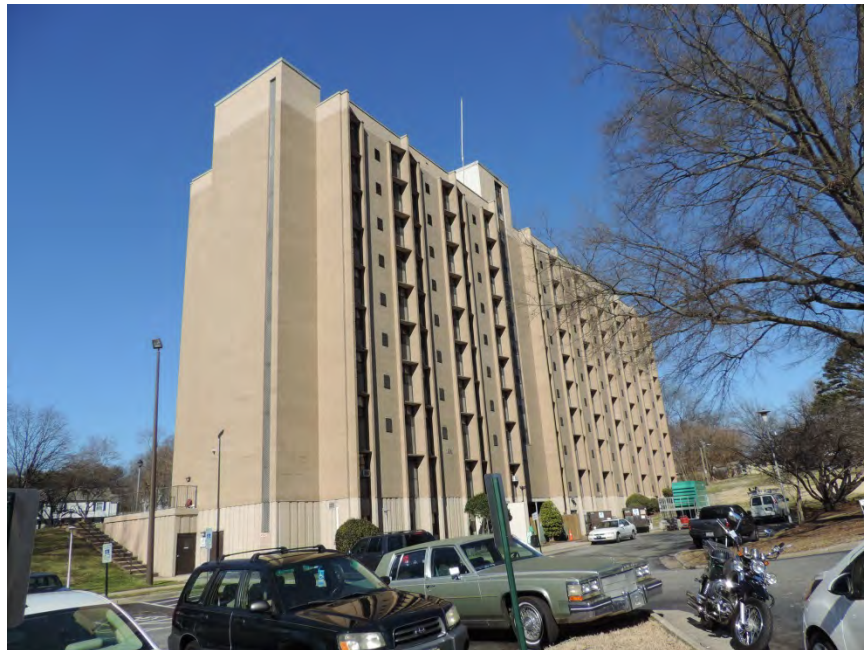
Figure 59. Facing northwest to rear or east elevation
