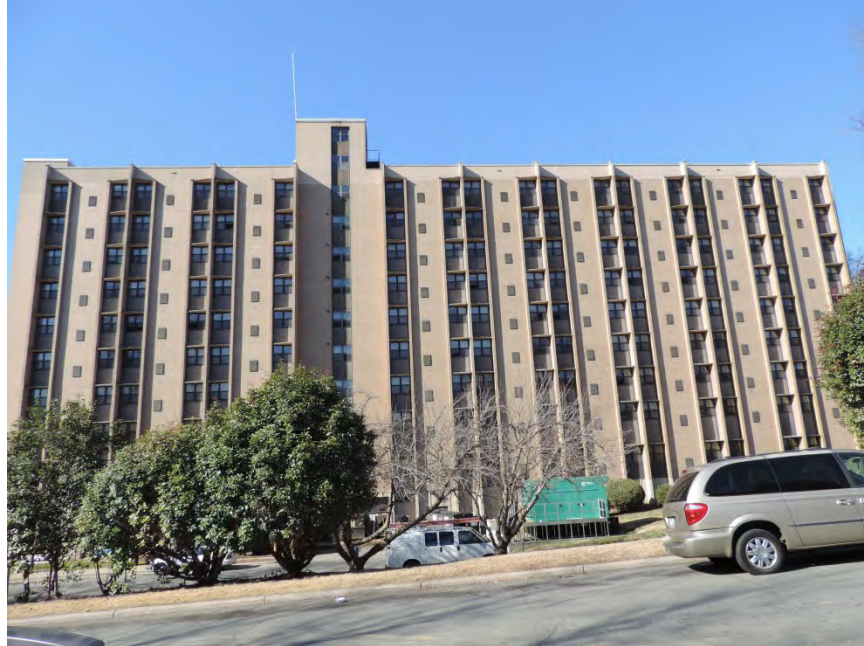
Figure 60. Facing west to rear elevation
