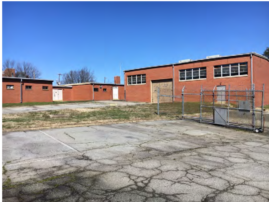
Figure 106. Facing northwest to main building's east elevation (off-center to south), assembly hall's south elevation (to north), and south building (Source: ALPHA Facilities Solutions)
