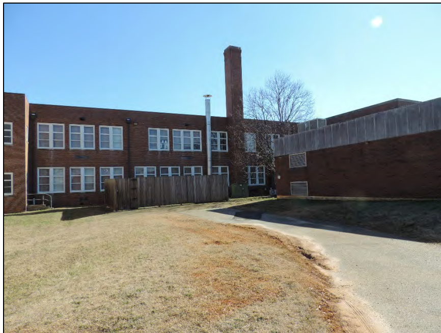
Figure 21: Facing southeast to main block's rear elevation
