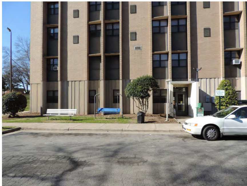
Figure 61. Rear entrance detail
