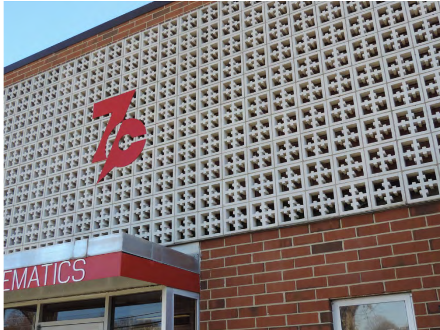
Figure 84. Second story concrete screen detail
