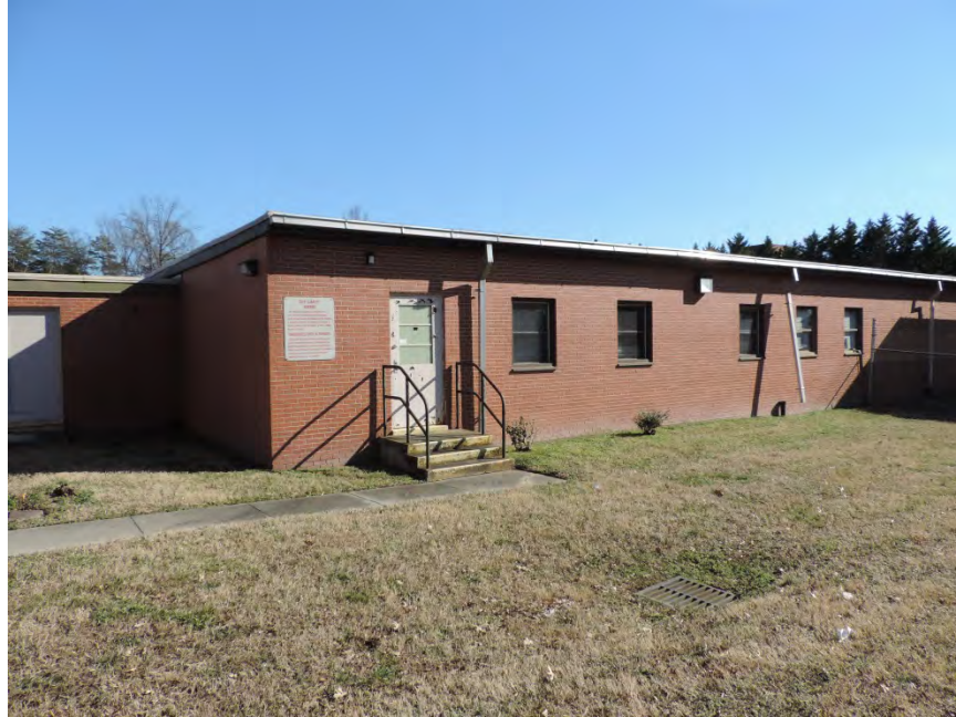
Figure 109. Facing southeast to south building's west elevation
