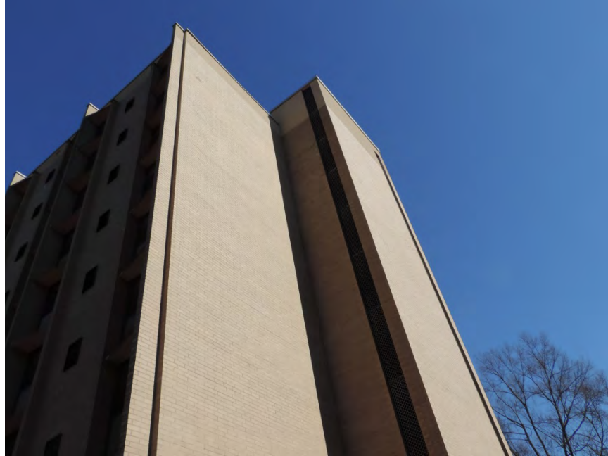
Figure 64. South side elevation detail
