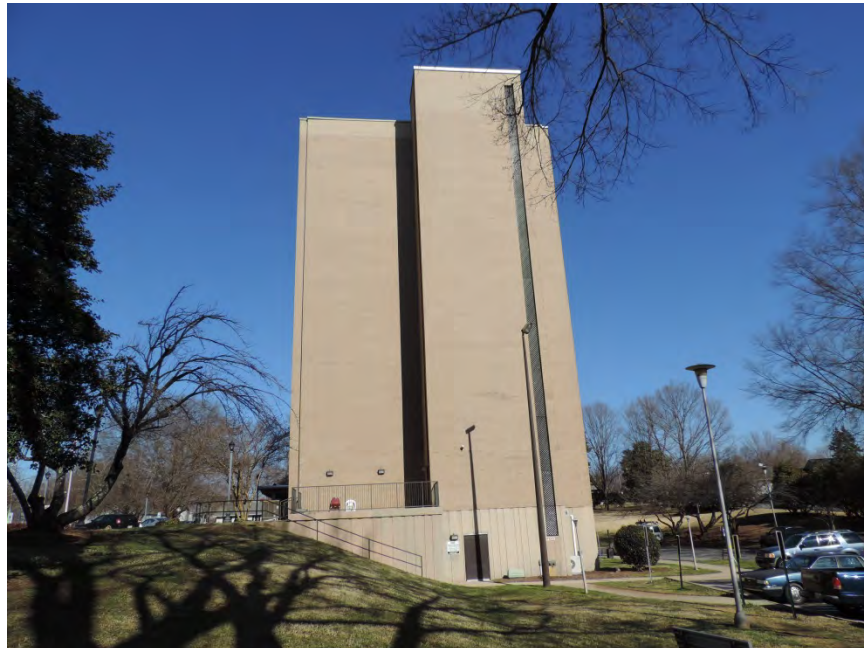
Figure 63. Facing north to south side elevation
