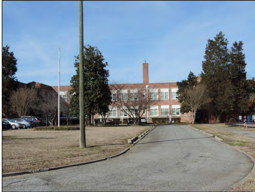
Figure 43: John Van Lindley Elementary School (GF 1451)
