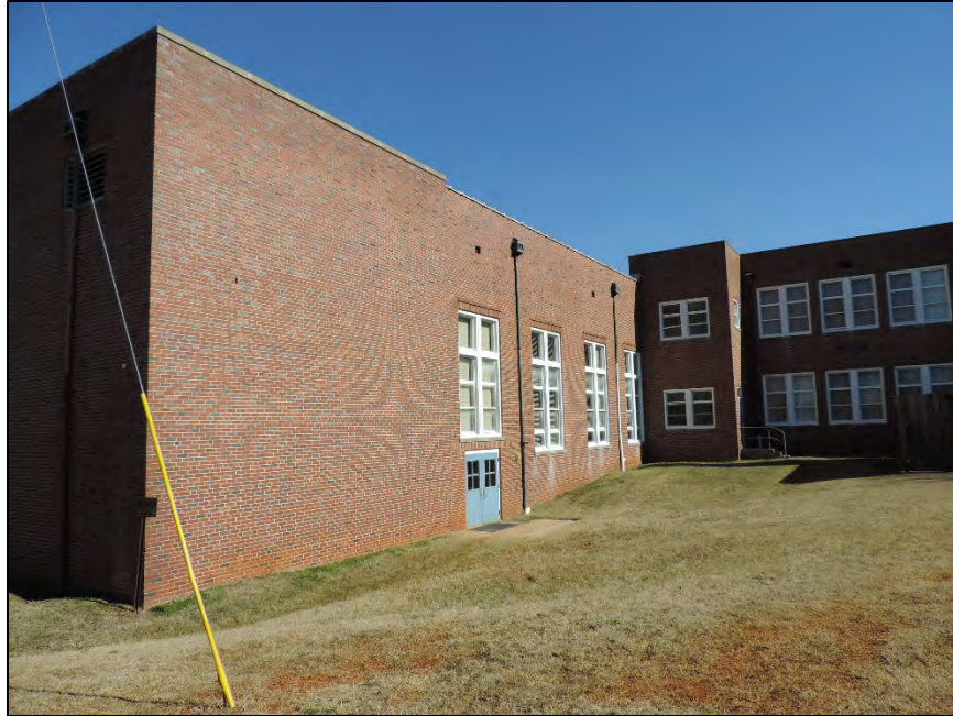
Figure 20: Facing northeast to the auditorium's southwest side elevation
