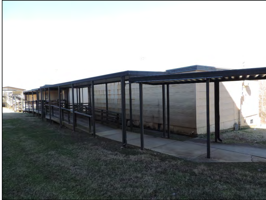
Figure 30: Facing northwest to modular classroom buildings and covered walkway
