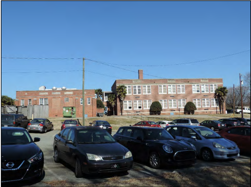
Figure 23: Facing northeast to southwest side elevation and cafeteria building
