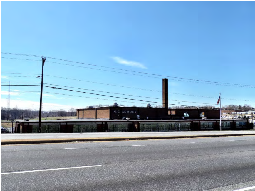
Figure 121. Winston-Salem National Guard Armory (FY 3915)
