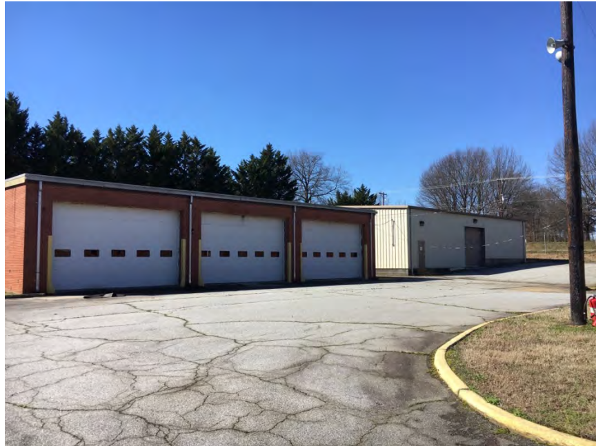
Figure 113. Facing southwest to OMS (Source: ALPHA Facilities Solutions)
