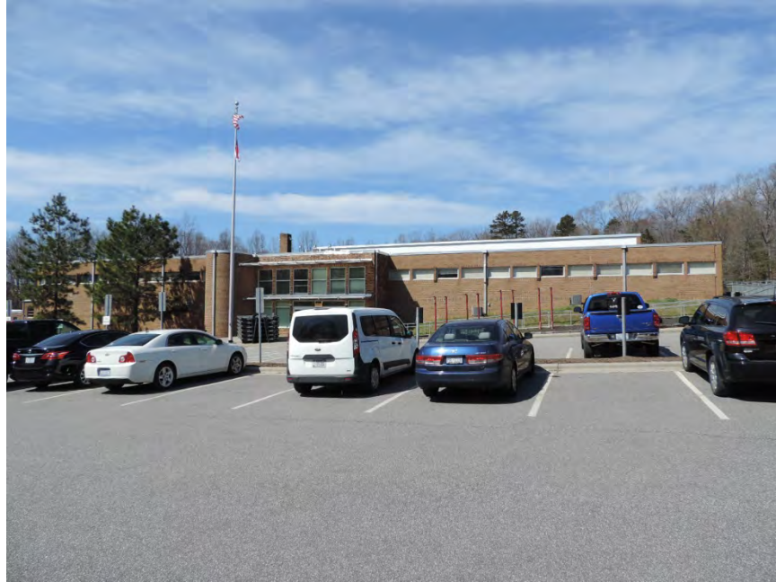
Figure 122. High Point National Guard Armory
