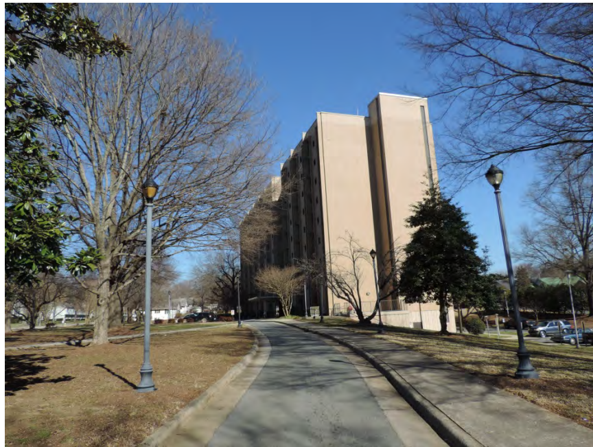
Figure 73. Facing north along driveway to building
