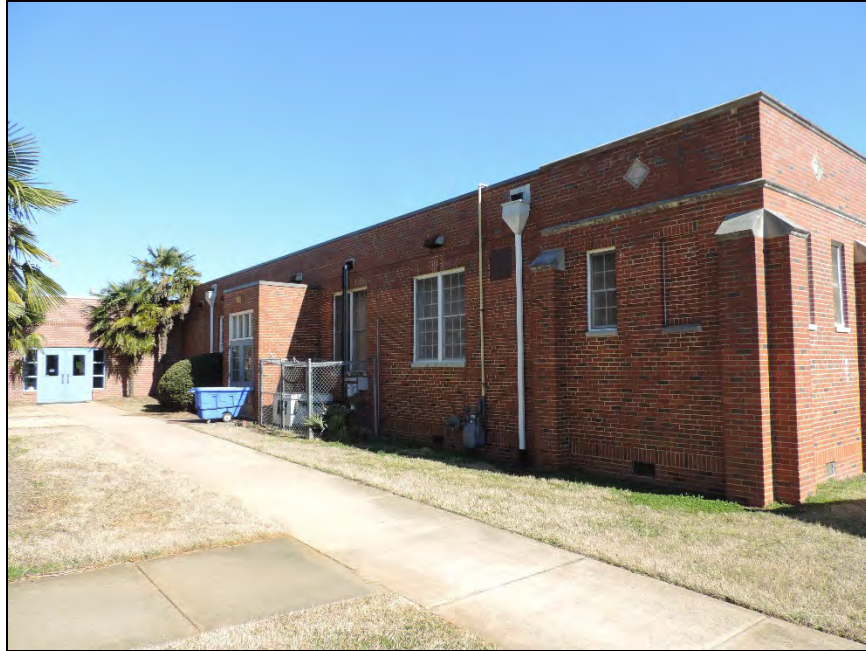
Figure 26: Facing northeast to cafeteria building
