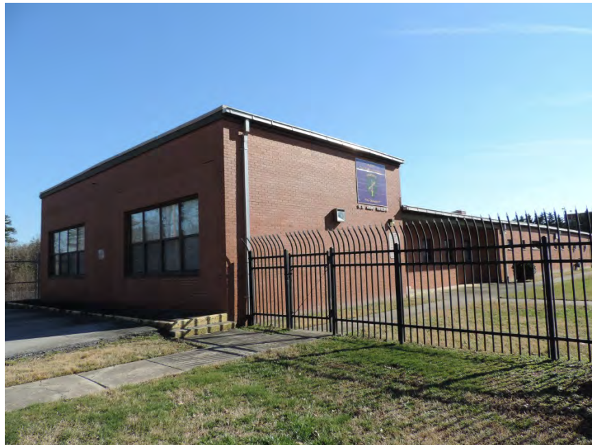
Figure 102. Facing southeast to main building's west and north elevations
