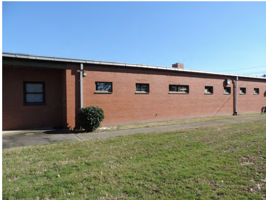
Figure 104. Facing east to main building's west window bays
