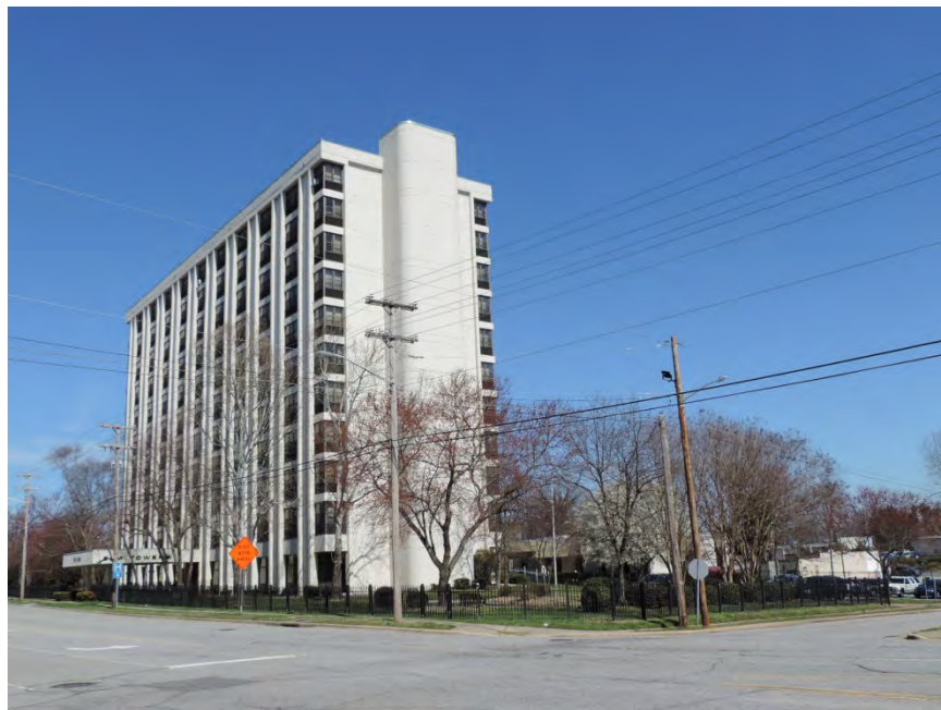
Figure 76. Elm Towers, High Point
