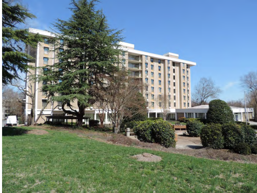
Figure 77. Astor Dowdy Towers, High Point
