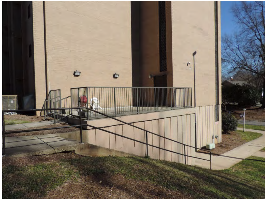
Figure 65. South side elevation detail
