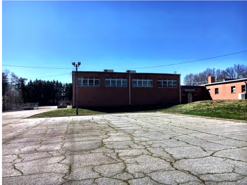
Figure 111. Facing south to assembly hall's north elevation (Source: ALPHA Facilities Solutions)
