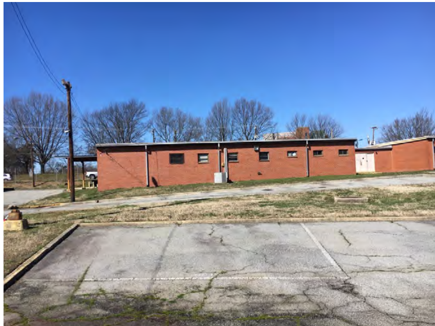
Figure 110. Facing west to south building's east elevation (Source: ALPHA Facilities Solutions)
