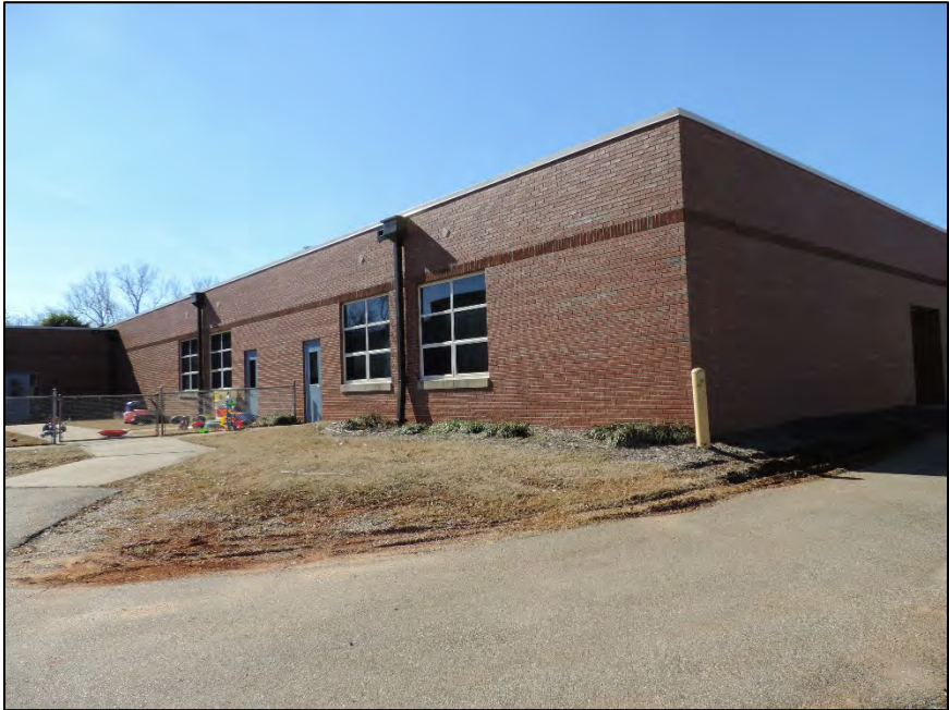
Figure 29: Facing southwest from behind main school building to kindergarten wing
