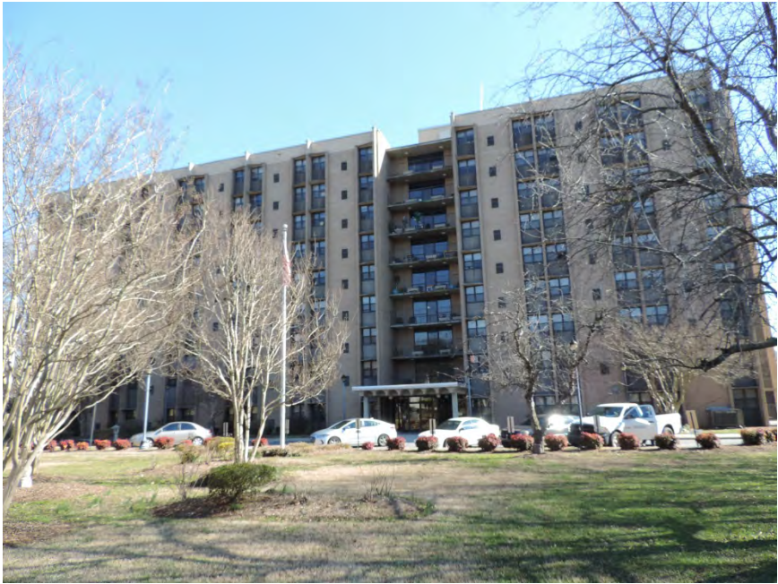
Figure 55. Facing east to Hall Towers
