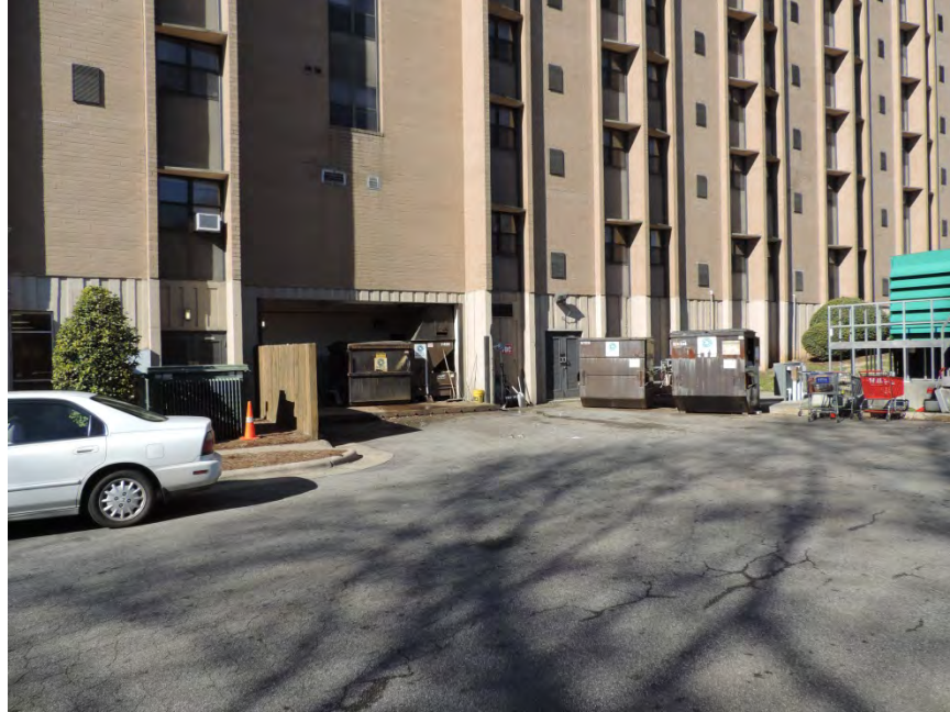
Figure 62. Rear service bays detail
