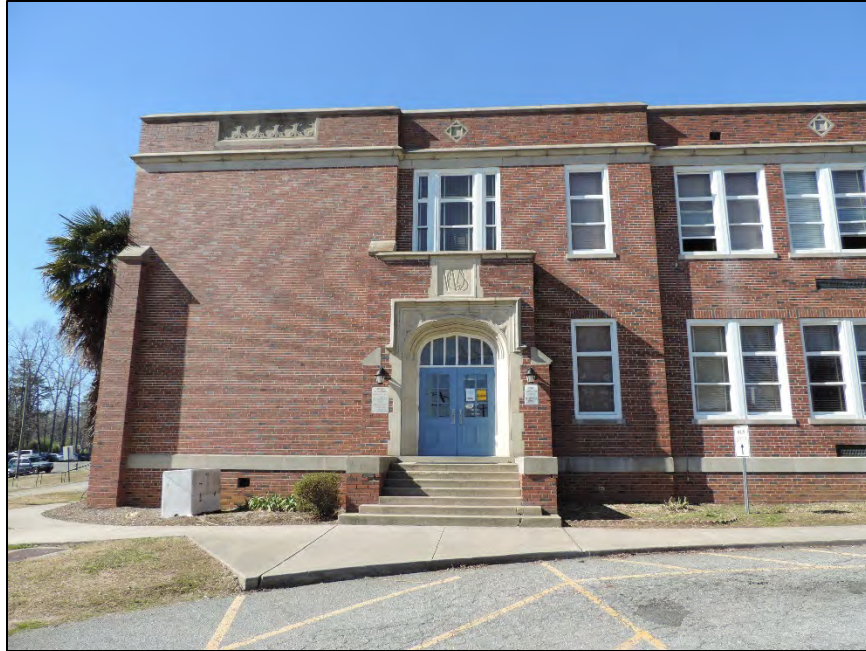
Figure 15: Facing northwest to façade's southwest corner
