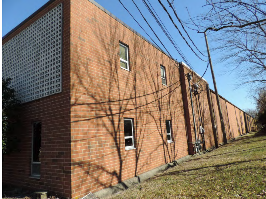
Figure 88. Facing northeast along south side elevation
