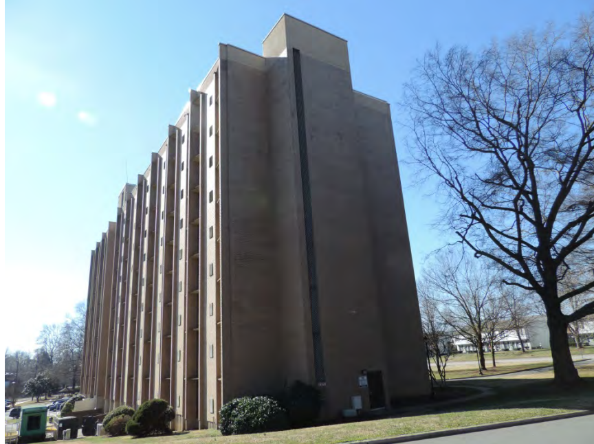
Figure 66. Facing southwest to north side elevation
