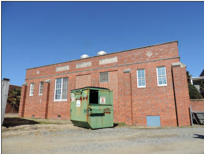
Figure 25: Facing northeast to cafeteria building
