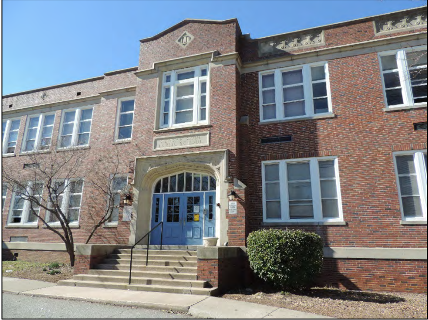
Figure 13: Facing northwest to façade and north entrance
