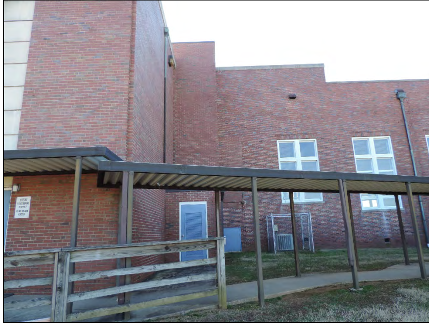
Figure 17: Facing southwest to northwest side elevation
