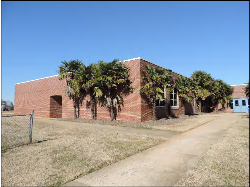
Figure 28: Facing north to kindergarten wing
