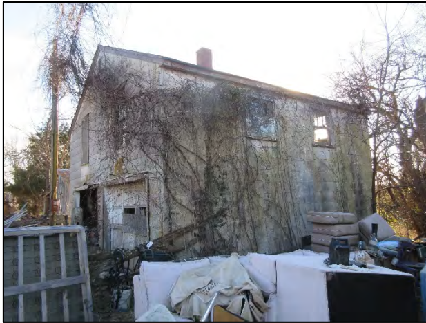
Garage oblique view of façade, view to southwest
