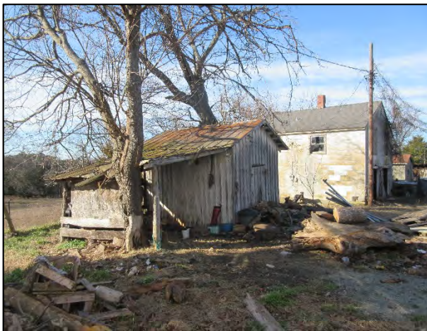
Shed 1 (foreground), view to northwest. Garage in background.
