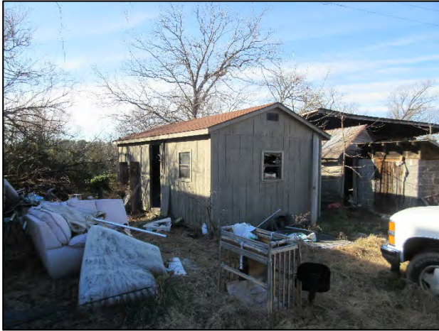
Shed 2, view to northwest
