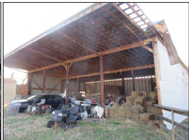
Equipment shed 2, view to southwest
