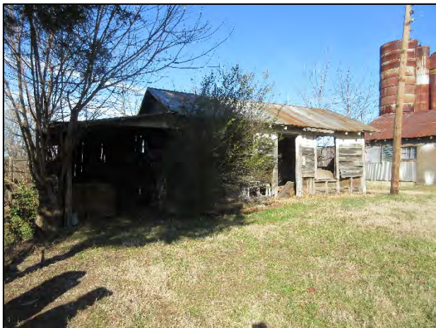
Milk House, view to northeast
