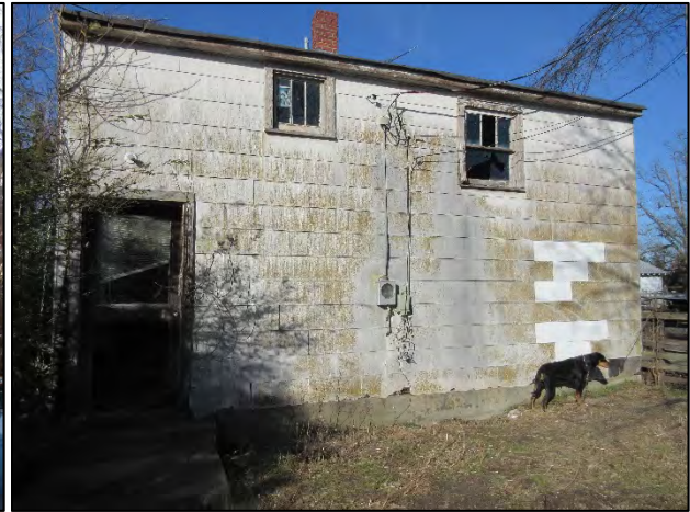
South elevation of Garage, view to northeast
