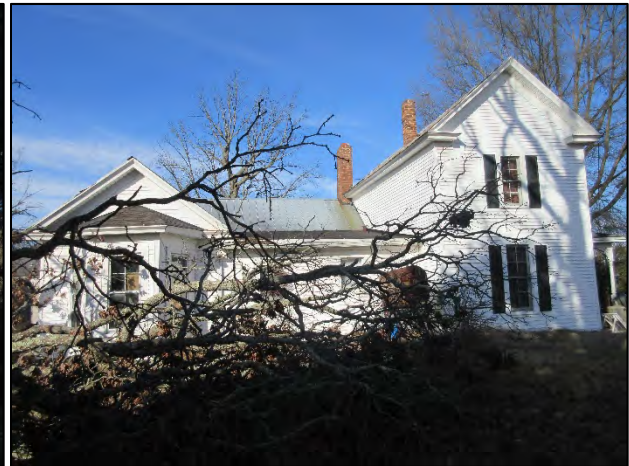
Jordan House south elevation, view to north
