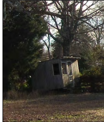
Shed 3, view to south
