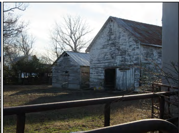
Double crib barn (right), equipment shed 3 (left) view to southwest
