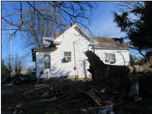
Jordan House rear elevation, view to east
