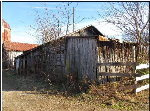
Milk House, view to southeast
