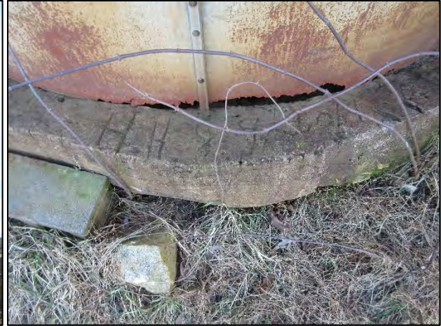
Silo foundation (east) detail, "H.H.J. 9/20/1930"
