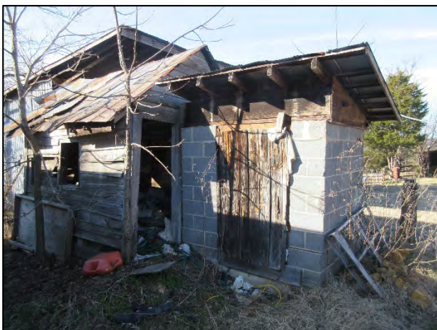
Well house (right) and tack room (left), view to northwest
