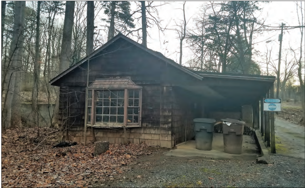
Figure 3.13. Garage Located at 3521 Battleground Avenue, Looking Northeast
