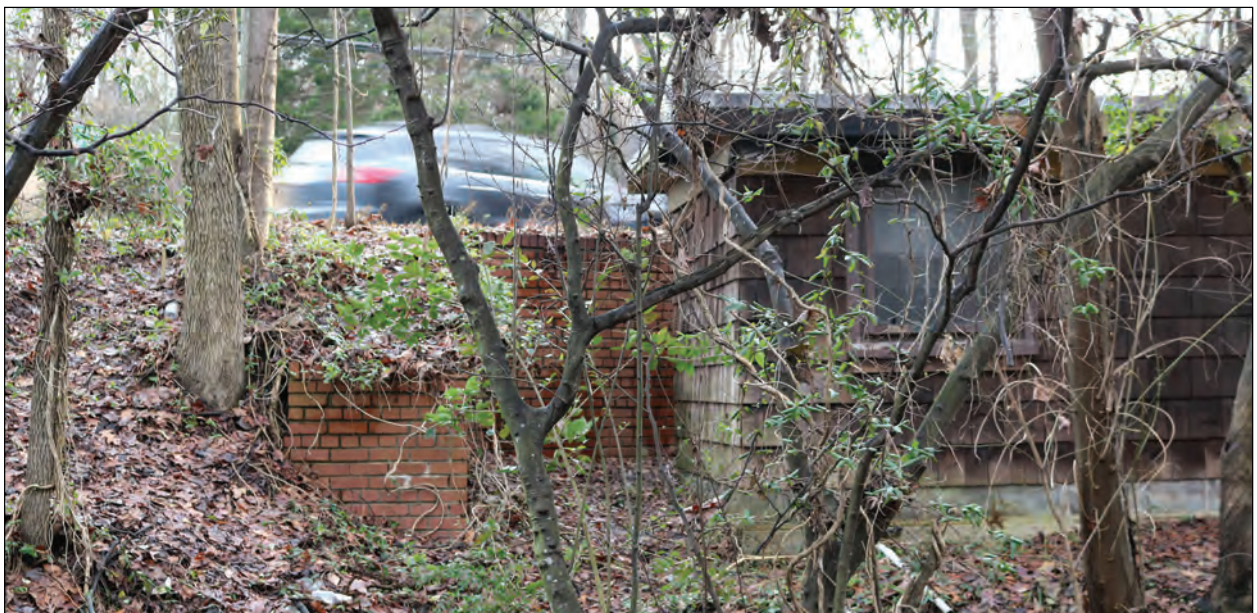
Figure 3.6. West Elevation and Retaining Wall, Looking East
