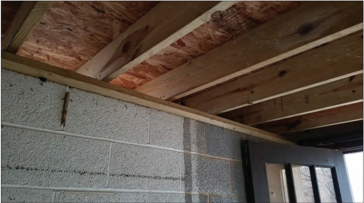
Figure 3.5. Interior, Looking Southeast
