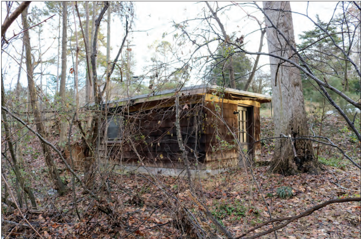
Figure 3.2. Fitzgerald-Schlanger Pumphouse, Looking Northeast
