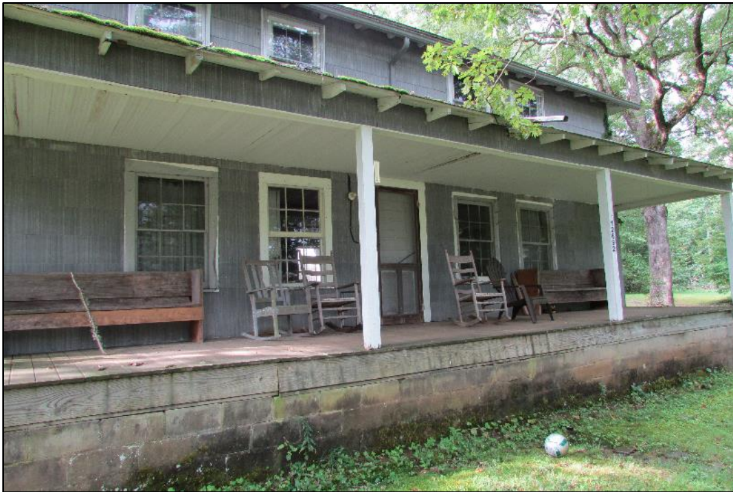
Figure 11. Charlie Slagle Lodge (Black Place), ca. 1923 house, porch deail, looking southwest.
