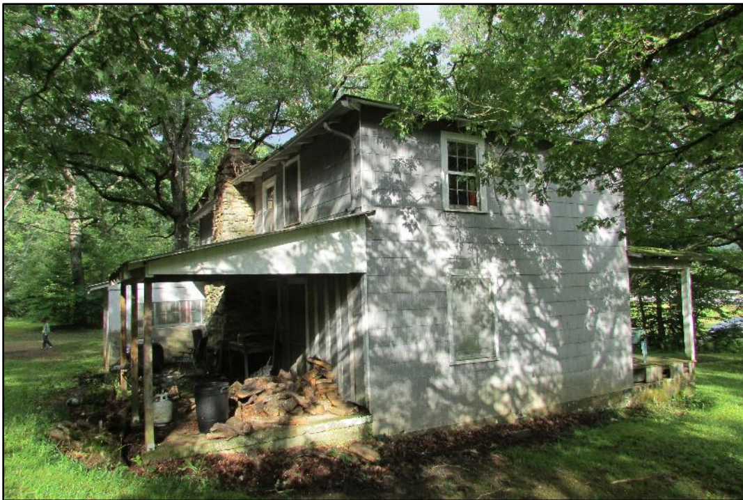
Figure 12. Charlie Slagle Lodge (Black Place), ca. 1923 house, southeast corner, looking northwest.
