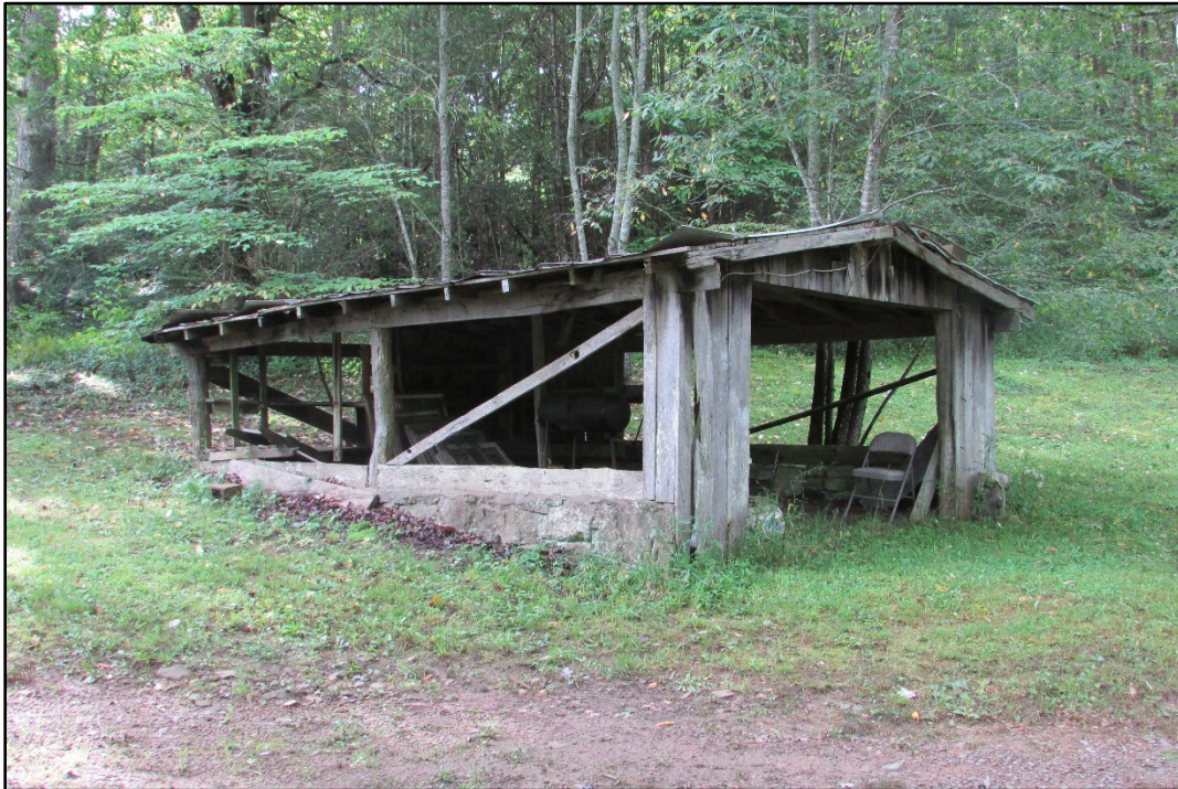
Figure 16. Shed, looking south.
