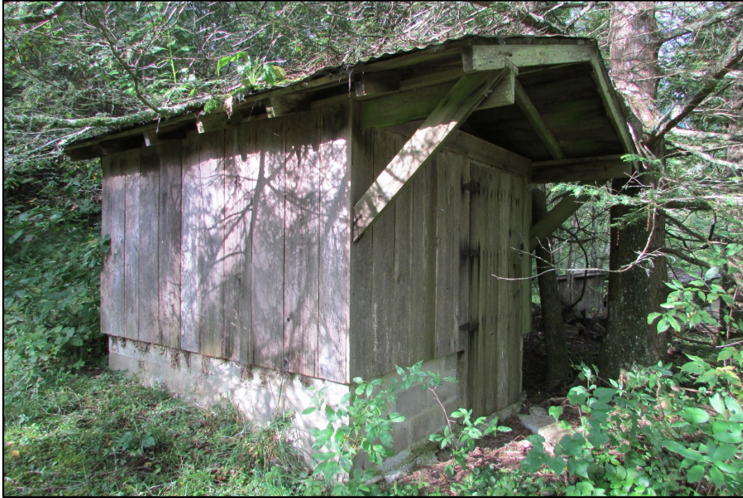
Figure 15. Smokehouse, looking southwest.
