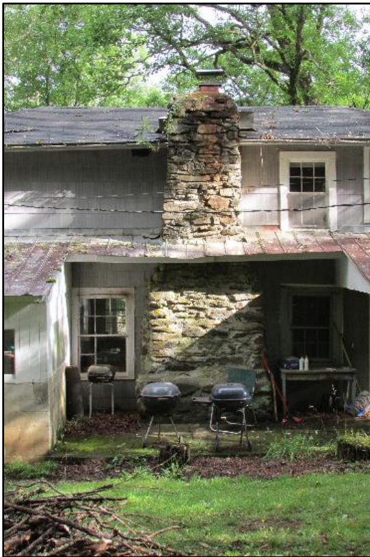
Figure 14. Chimney detail, south elevation, looking north.
