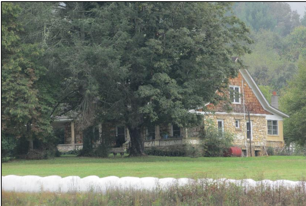
Figure 25. A.B. Slagle Dairy Farm (MA210), 760 Wayah Road, Franklin, looking southeast.
