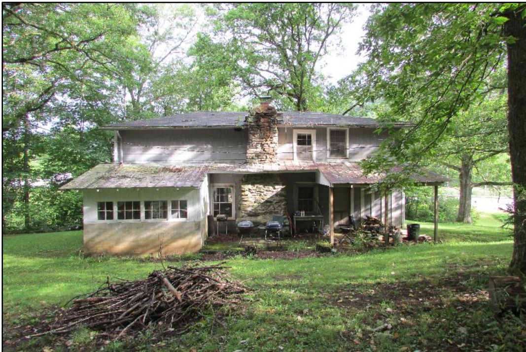
Figure 10 Charlie Slagle Lodge (Black Place), ca. 1923 house, south elevation, looking north.
