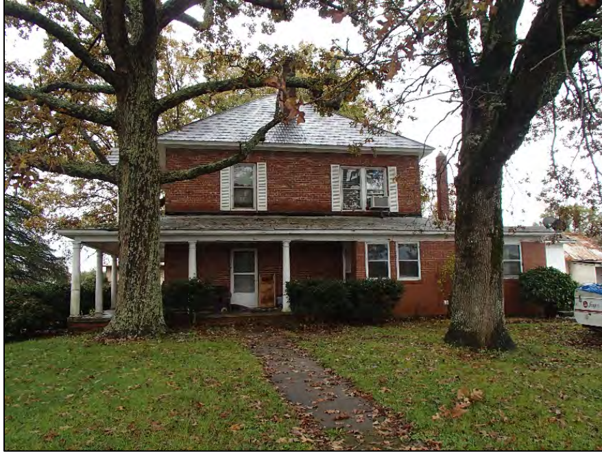
Figure 6: Teague House, facing southwest to northeast side elevation
