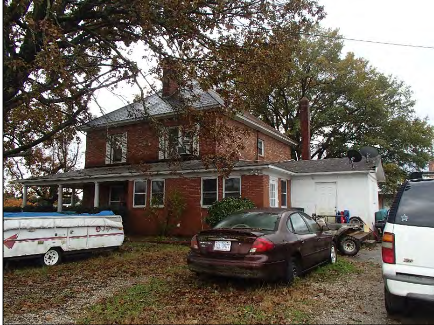
Figure 7: Teague House, facing southwest to northeast side and rear elevations
