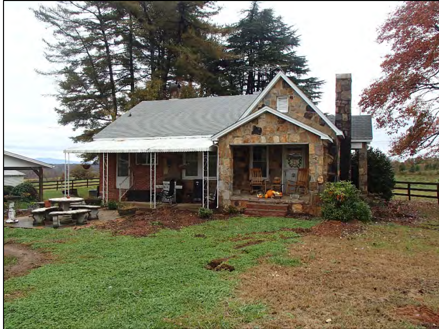
Figure 23: Deal House, facing north to south side elevation
