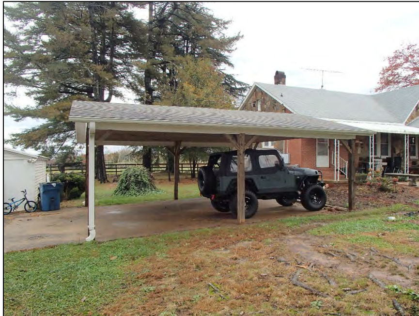
Figure 27: Deal House, north to non-historic carport
