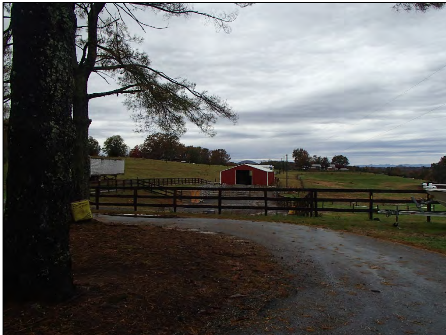
Figure 29: Deal House, facing west to non-historic barn
