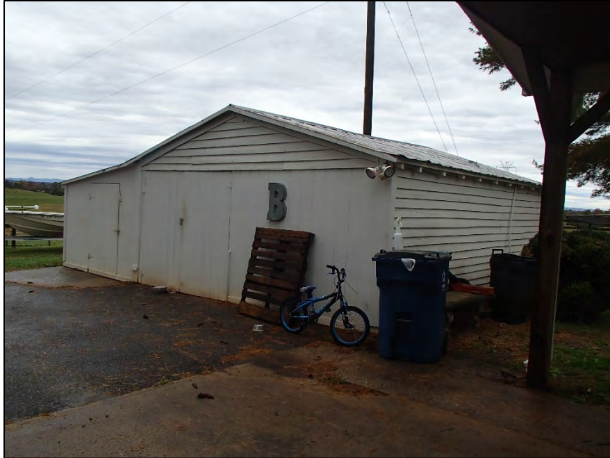
Figure 28: Deal House, facing northwest to historic outbuilding
