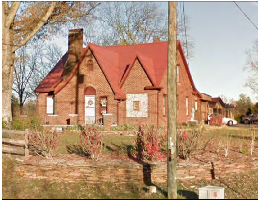
Figure 31: 4184 S NC 127 Hwy, Hickory
