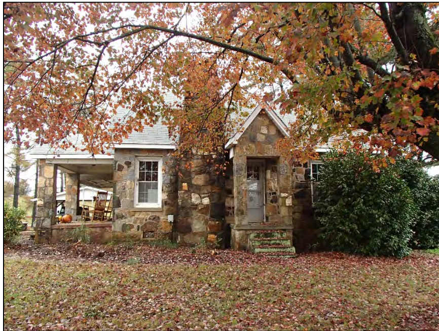
Figure 22: Deal House, facing west to façade
