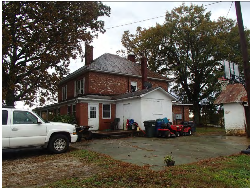
Figure 8: Teague House, facing southeast to rear elevation
