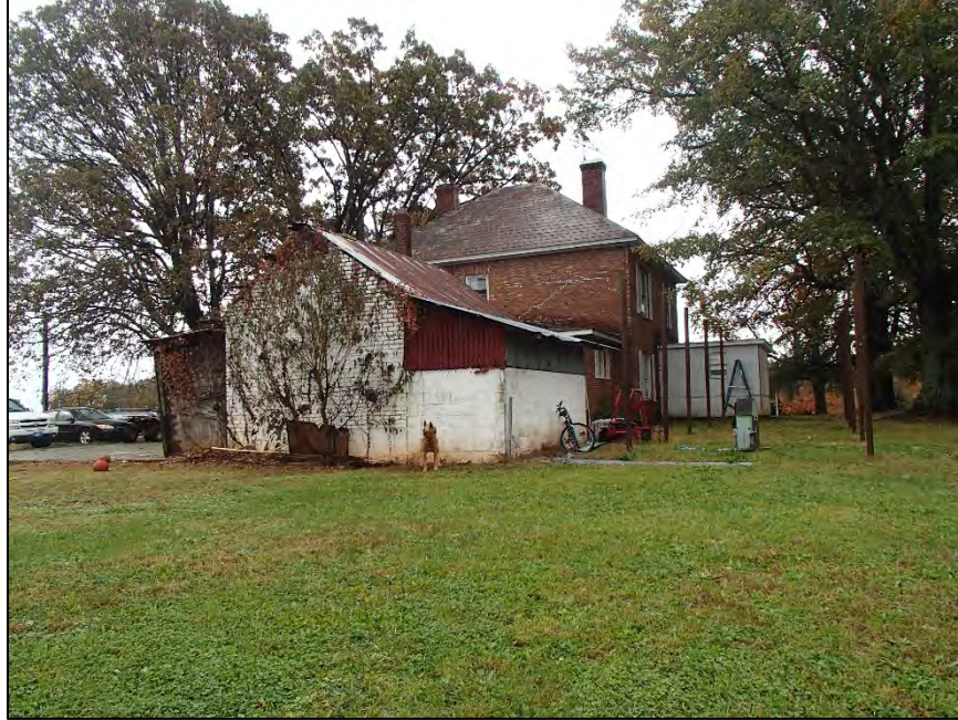
Figure 9: Teague House, facing southeast to rear elevation
