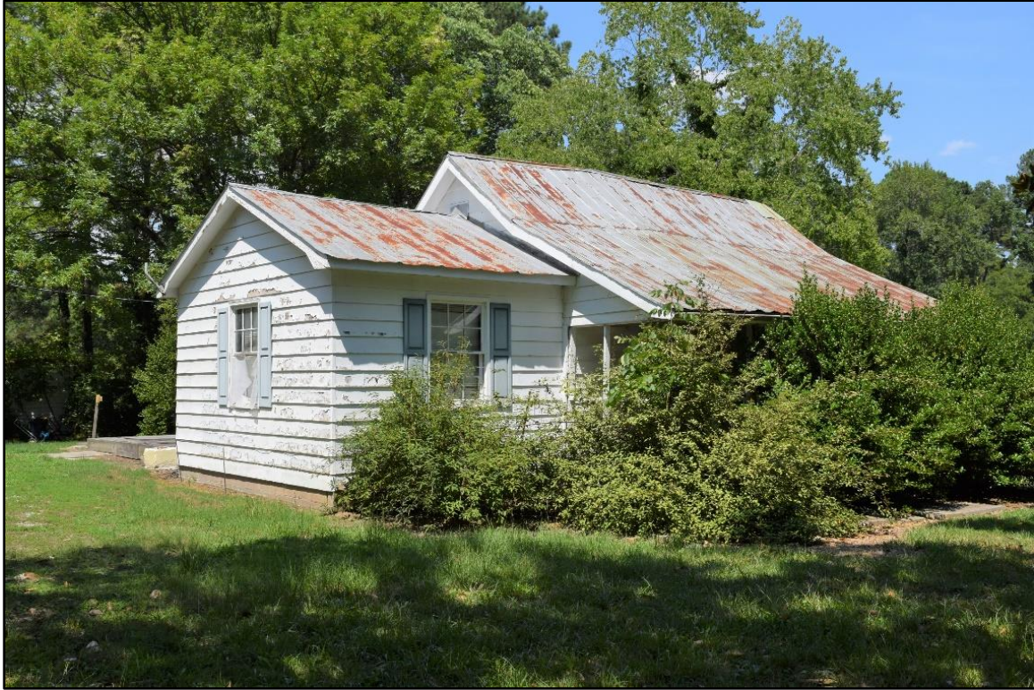
Fig. 1 The south elevation of the Lemuel Morgan Farm
