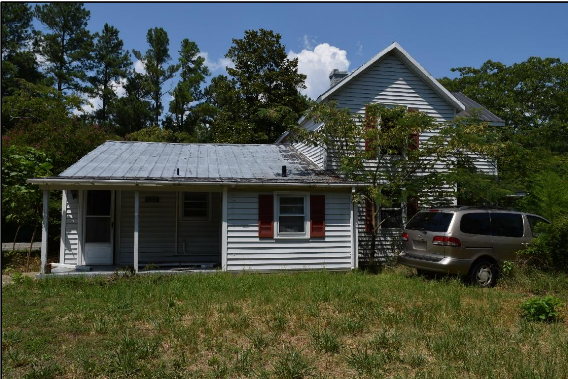
Fig. 2 The south elevation of the Lorenzo Morgan House
