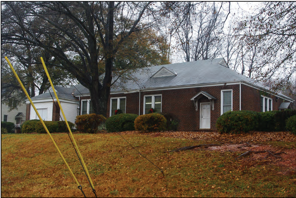
PLATE 28: J. Paul Ford Community Center (GS0145), North Elevation, Belmont, North Carolina
