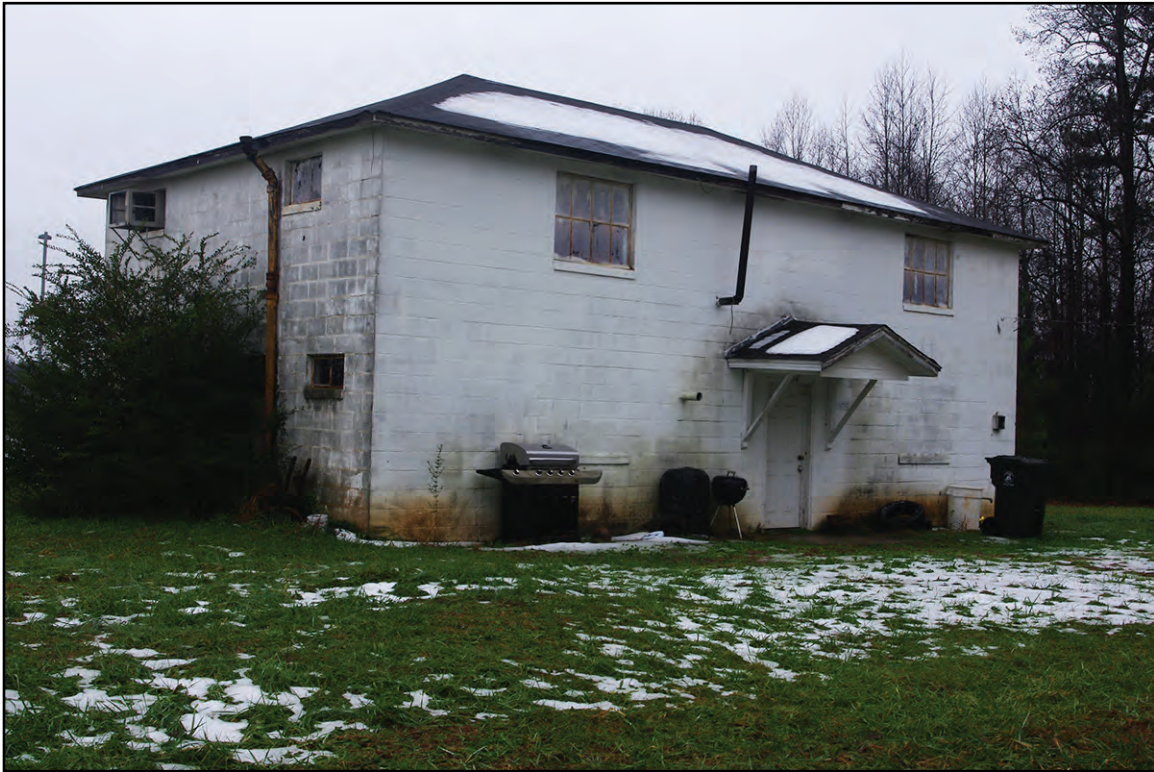
PLATE 13: Hiram Mason Lodge No. 22 (GS1711), Oblique View of North and East Elevations, Lowell, North Carolina
