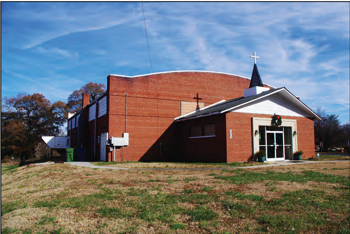
PLATE 19: South Elevation, Former Junior Chamber of Commerce Community Building (GS2423), Mount Holly, North Carolina
