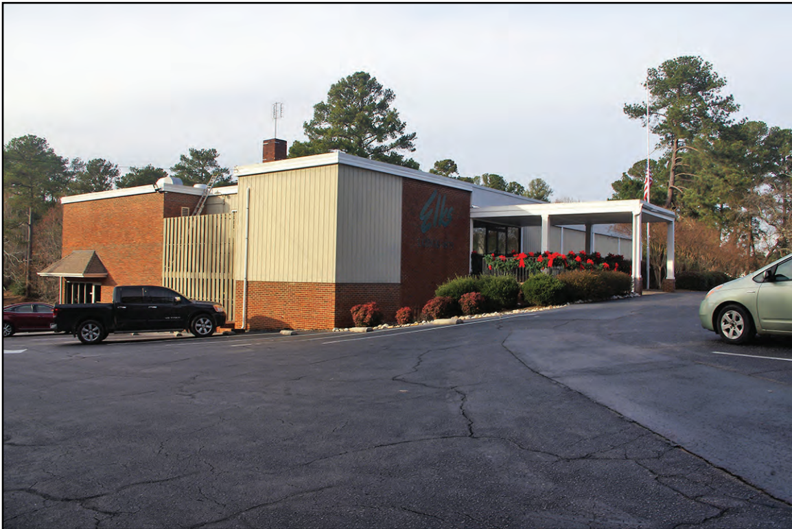
PLATE 16: Elks Lodge No. 1679 (LE0854), Oblique View of East and South Elevations, Sanford, North Carolina
