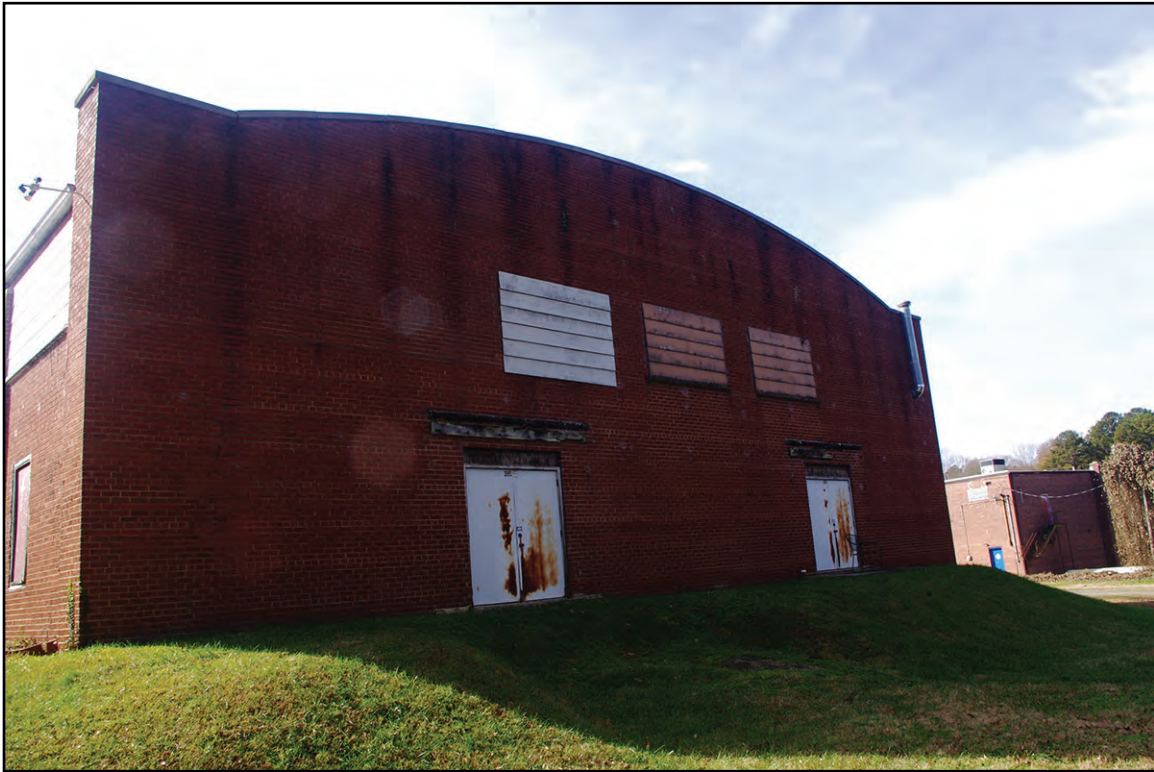
PLATE 23: North Elevation, Former Junior Chamber of Commerce Community Building (GS2423), Mount Holly, North Carolina
