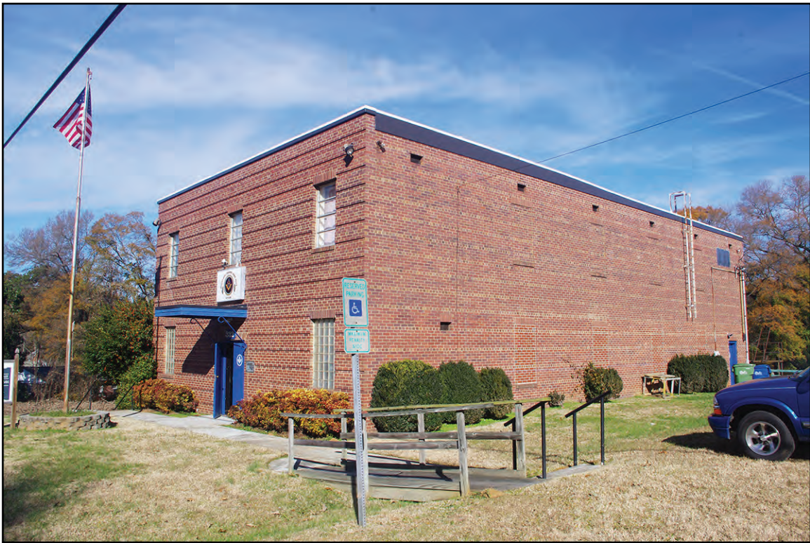
PLATE 1: Oblique View of South and East Elevations, Mount Holly Lodge 544 AF & AM (GS2422), Mount Holly, North Carolina
