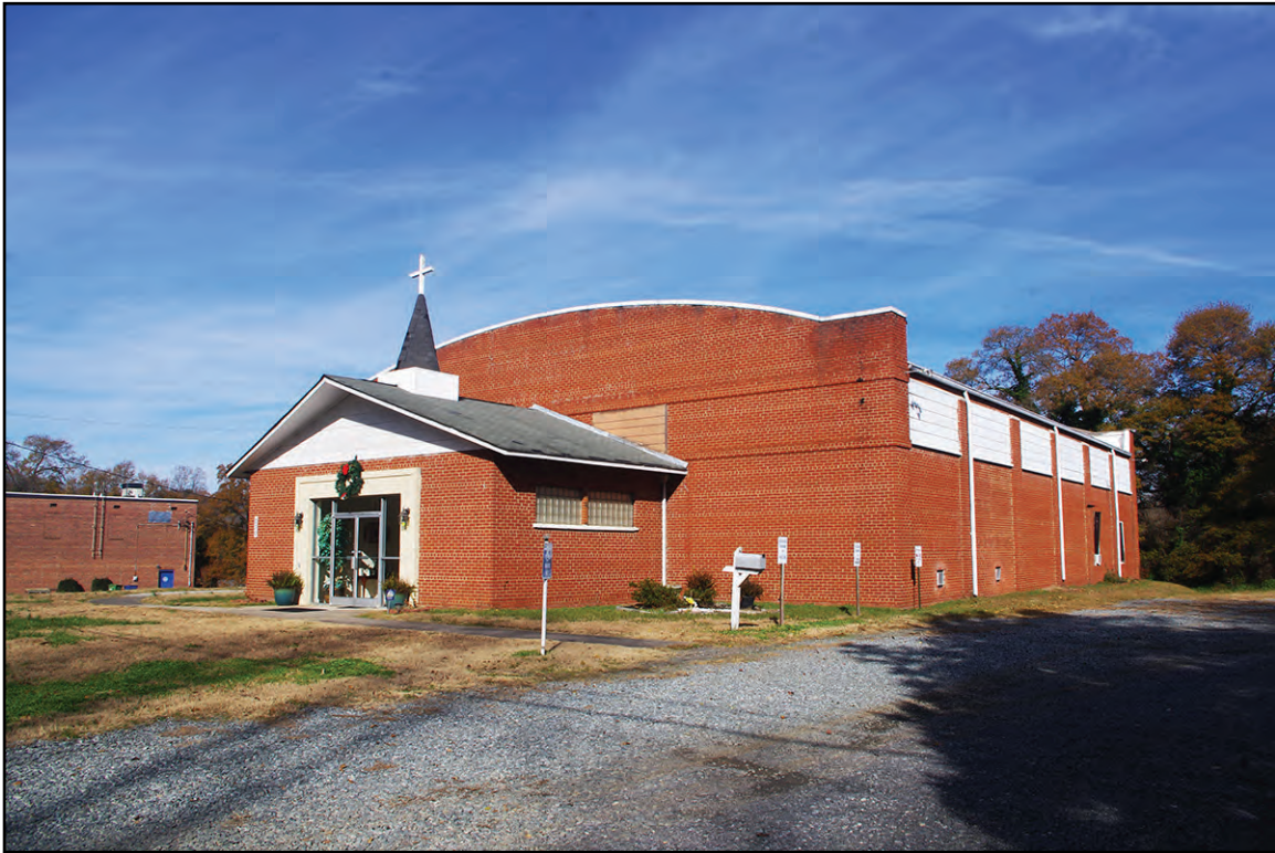
PLATE 18: Oblique View of South and East Elevations, Former Junior Chamber of Commerce Community Building (GS2423), Mount Holly, North Carolina
