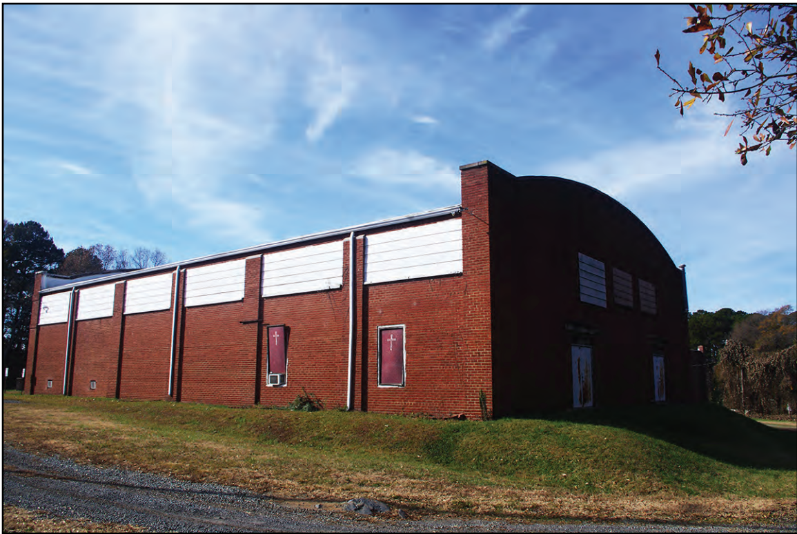
PLATE 26: Oblique View of East and North Elevations, Former Junior Chamber of Commerce Community Building (GS2423), Mount Holly, North Carolina
