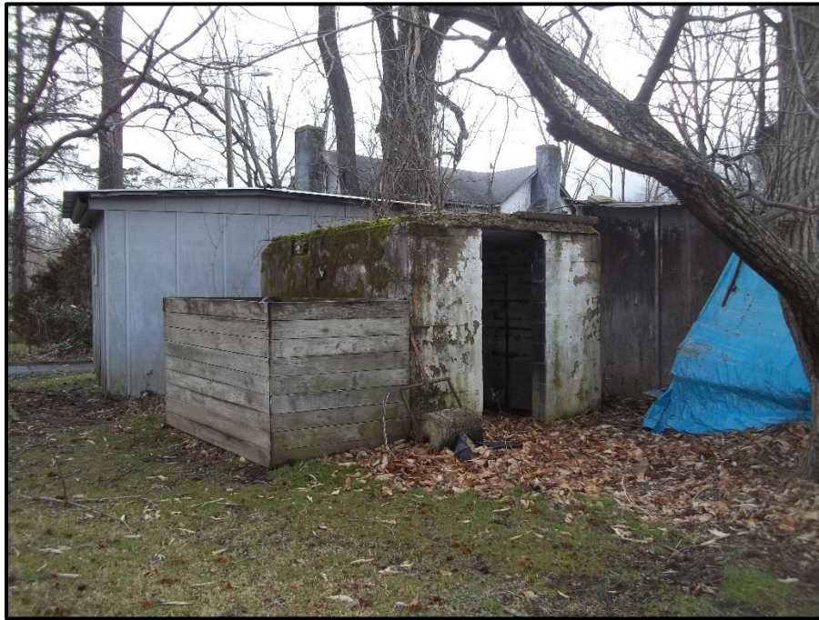
Figure 25. Shed, Looking West.
