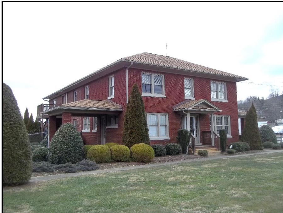
Figure 36. Allison House, Looking Northwest.
