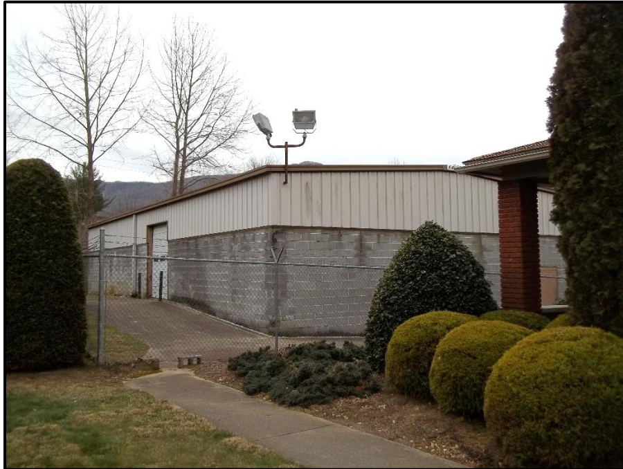
Figure 54. Commercial Storage Building, Looking Southwest.
