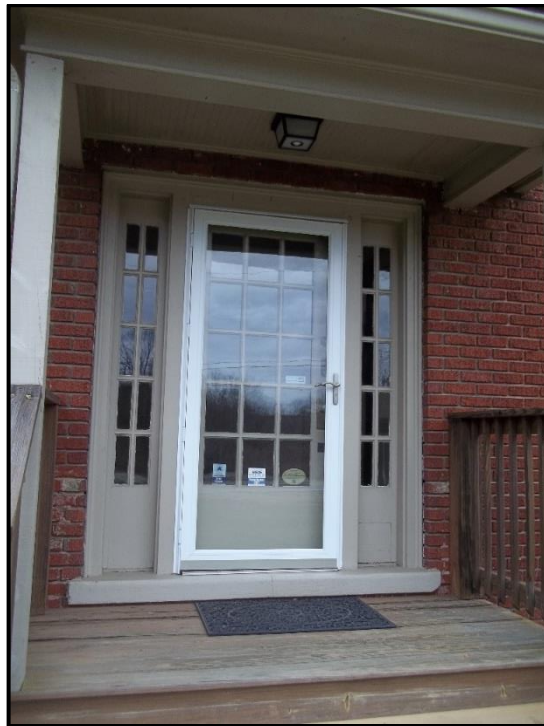
Figure 40. Detail of Front Entry Door, Looking West.
