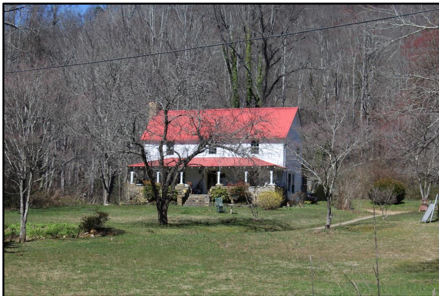
Figure 28. Millard Jones House (BN0487), Cragmont Road, Black Mountain, NC, View Looking Northwest.
