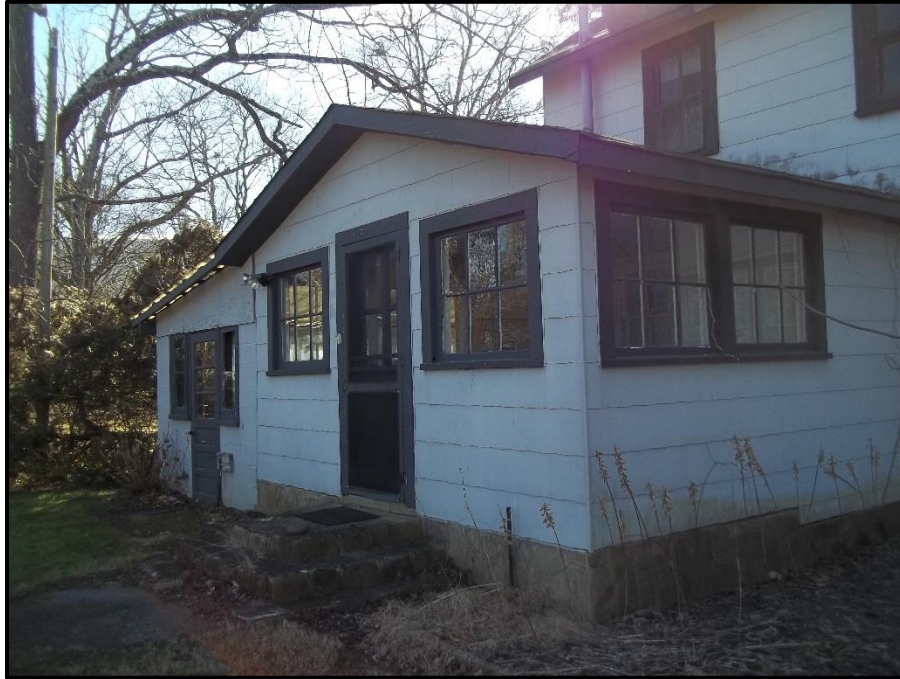
Figure 14. Detail of One-Story Greenhouse with Shed-Roofed EII, Looking Southwest.
