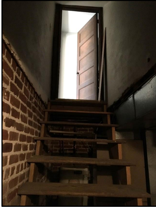
Figure 42. Basement Stairs, Looking West.
