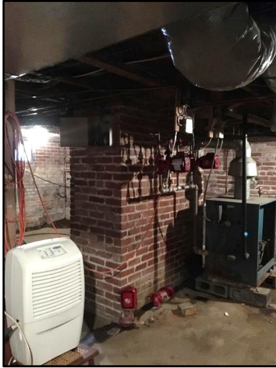
Figure 41. Overview of Basement, Looking Northwest.
