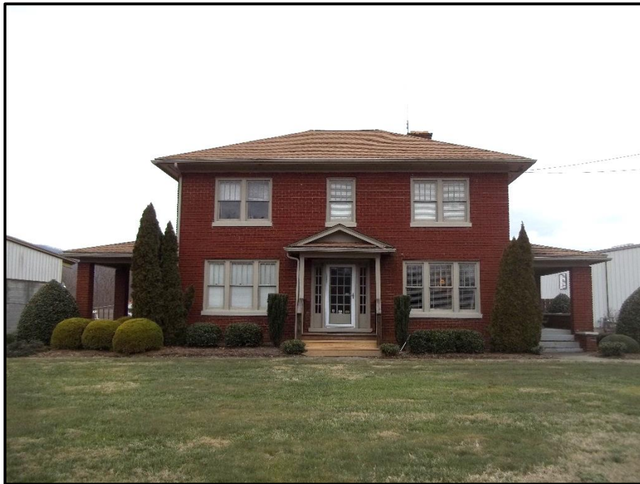
Figure 34. Allison House, Looking West.
