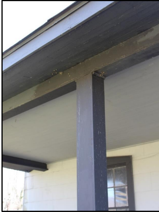
Figure 16. Detail of Front Porch, Looking East.
