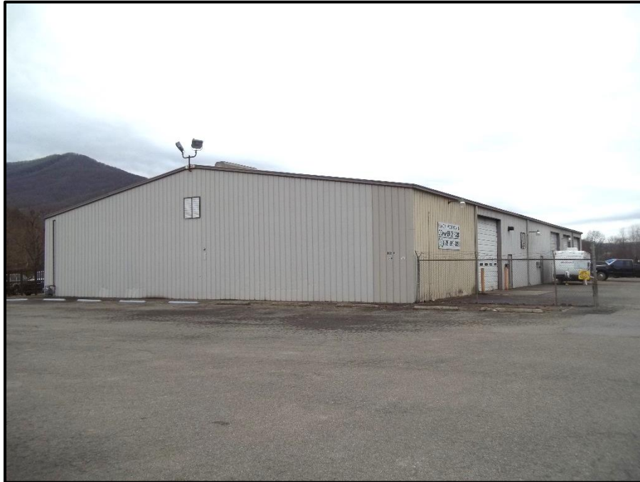
Figure 53. Commercial Storage Building, Looking Southwest.
