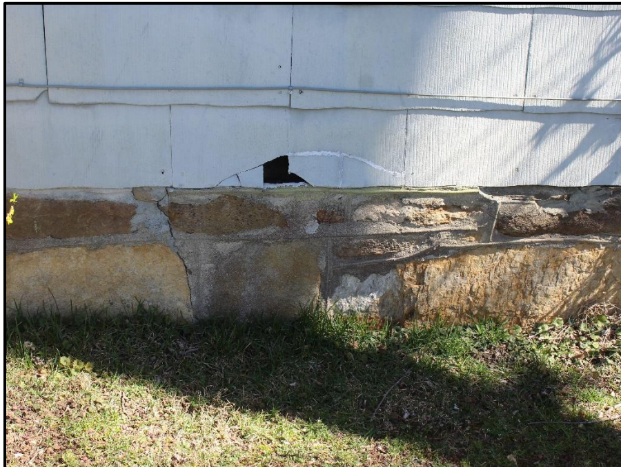
Figure 15. Detail of Foundation, Looking Northeast.
