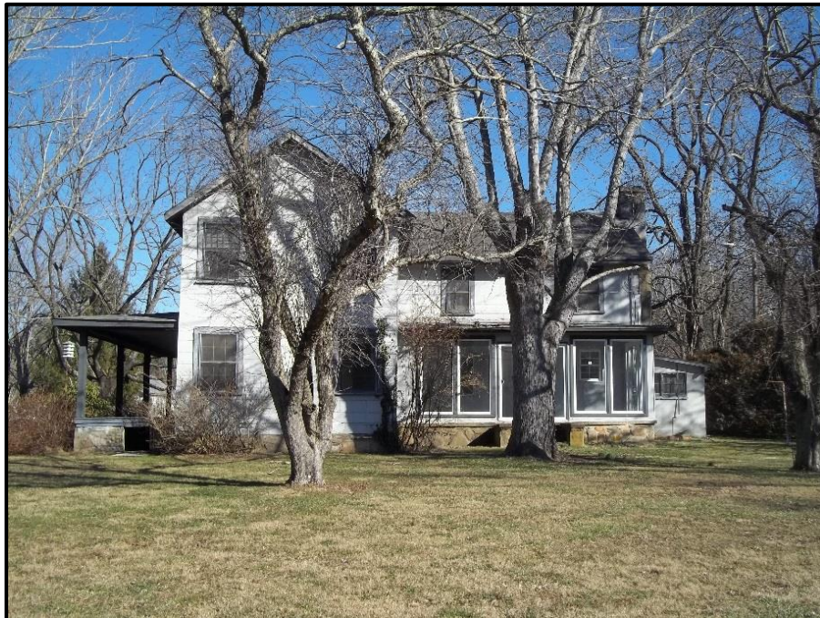
Figure 9. John Runion House, Looking East.
