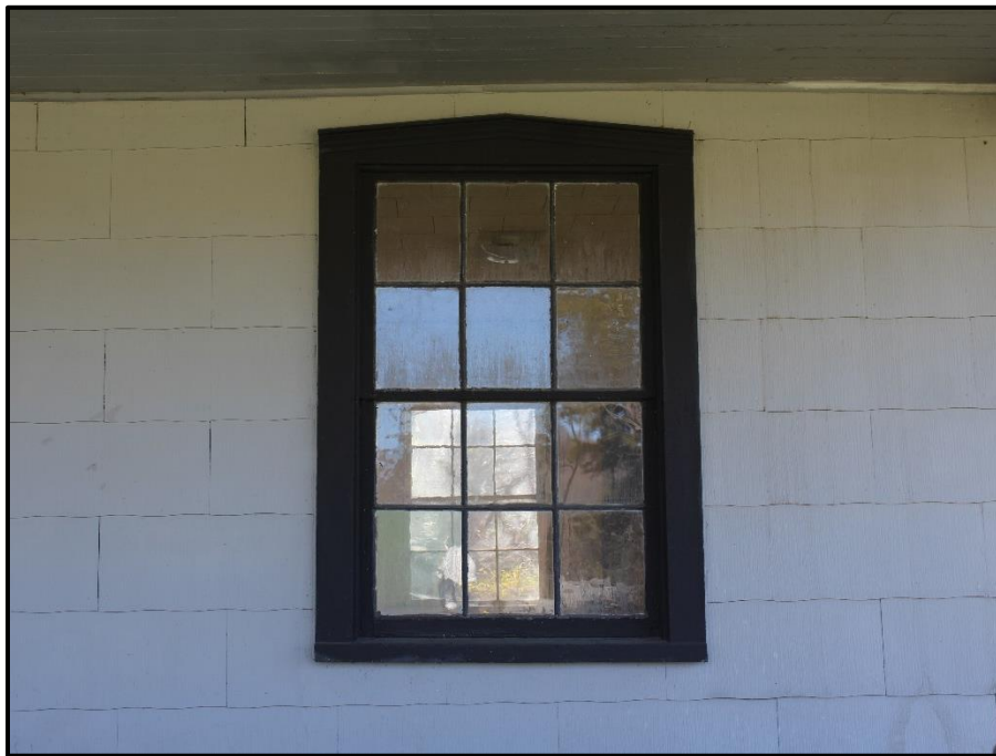
Figure 17. Detail of Window on Facade, Looking Southeast.
