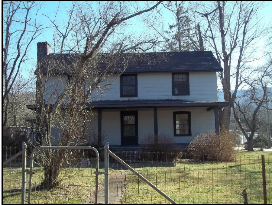
Figure 8. John Runion House, Looking South.
