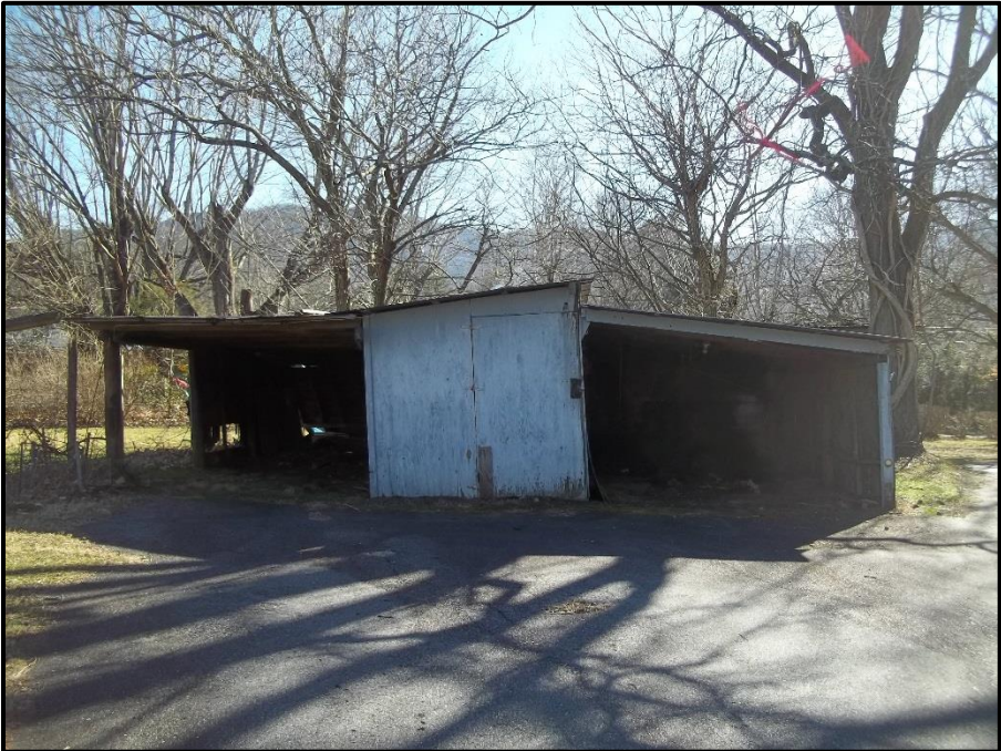
Figure 24. Vehicle Shed, Looking South.
