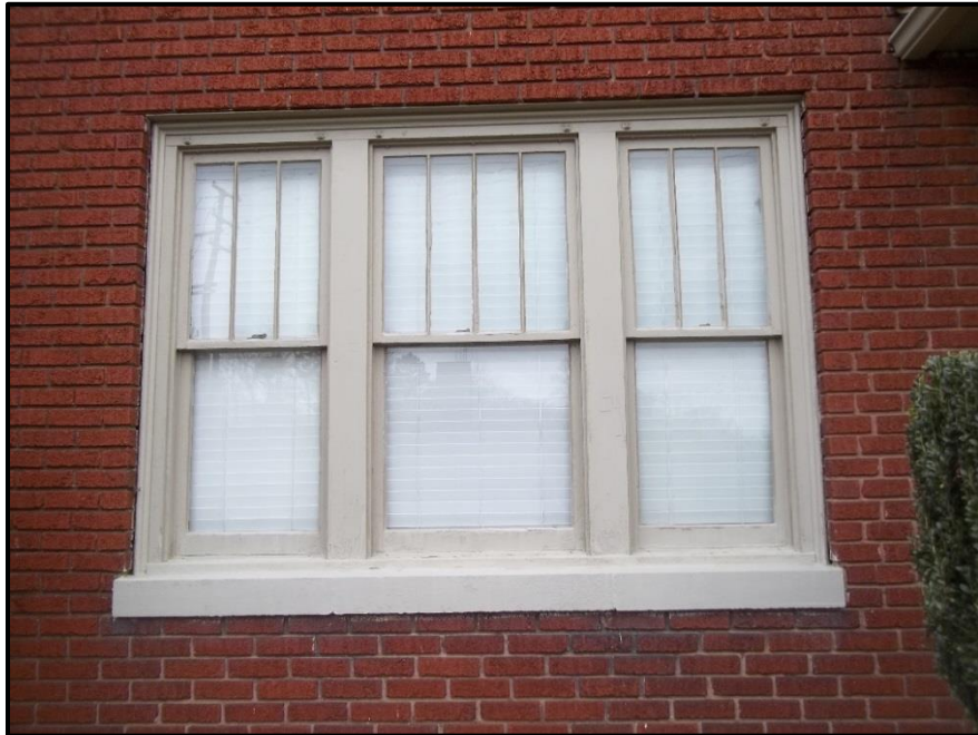
Figure 39. Detail of Triple Window on Facade, Looking West.
