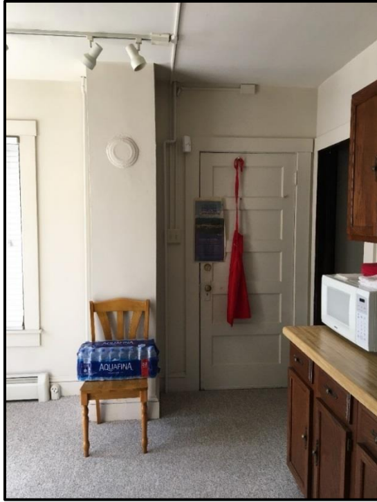
Figure 47. Kitchen Rear Wall (Southwest Room), Looking West.
