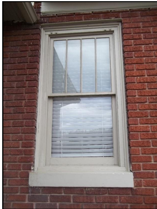
Figure 38. Detail of Window on Facade, Looking West.
