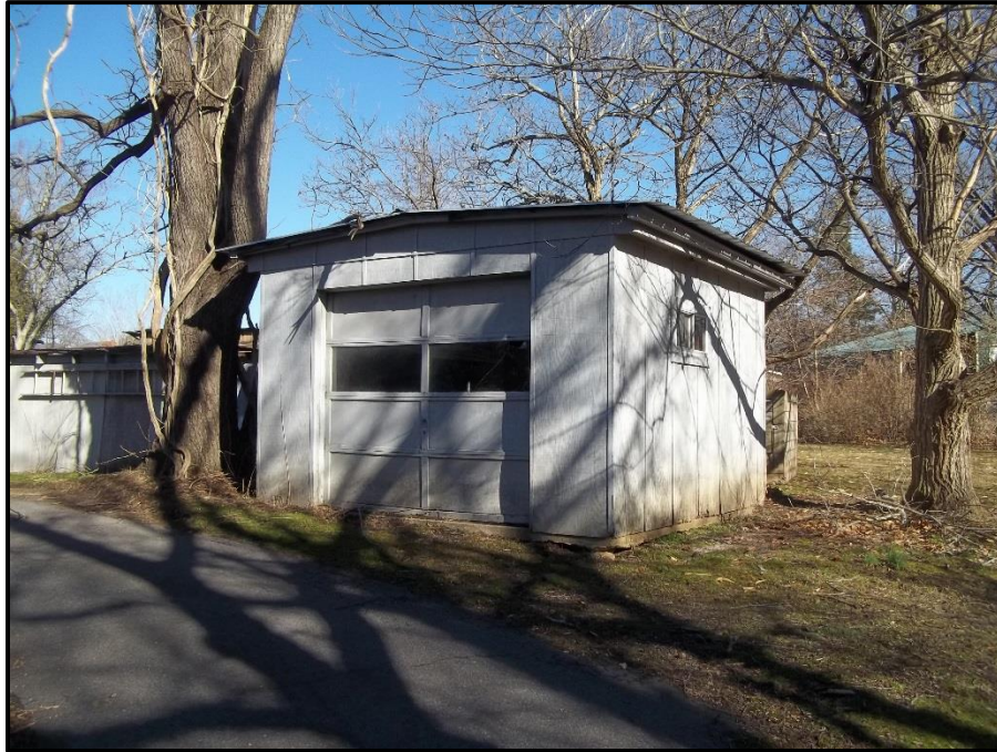
Figure 23. Garage, Looking Northeast.
