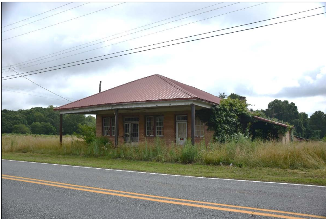
Figure 4.2. T. C. Falls Store Crossroads (LN0131), store, facing northeast.
