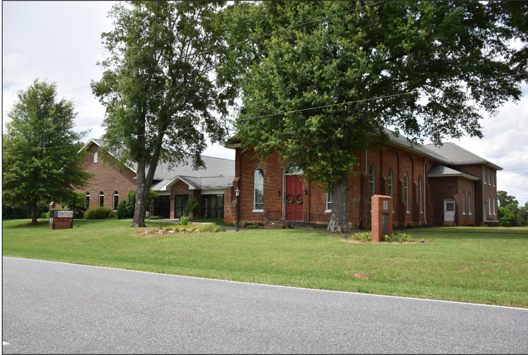
Figure 4.50. Daniels Lutheran Church (LN0159), facing northwest.
