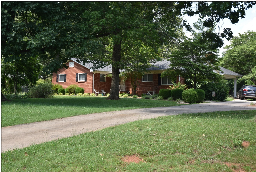
Figure 4.72. Carpenter House (LN0840), facing northeast.
