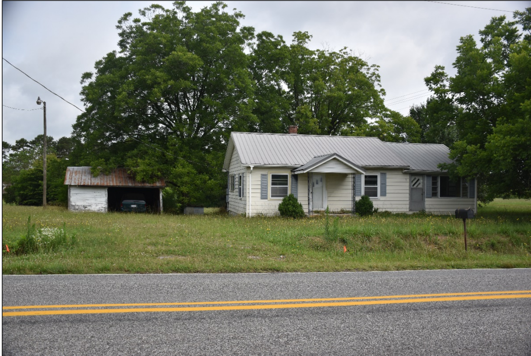
Figure 4.8. Elmore House (LN0809), facing southwest.
