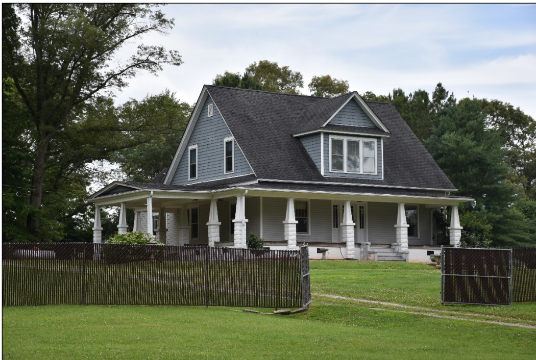
Figure 4.44. Baxter House (LN0830), facing south.
