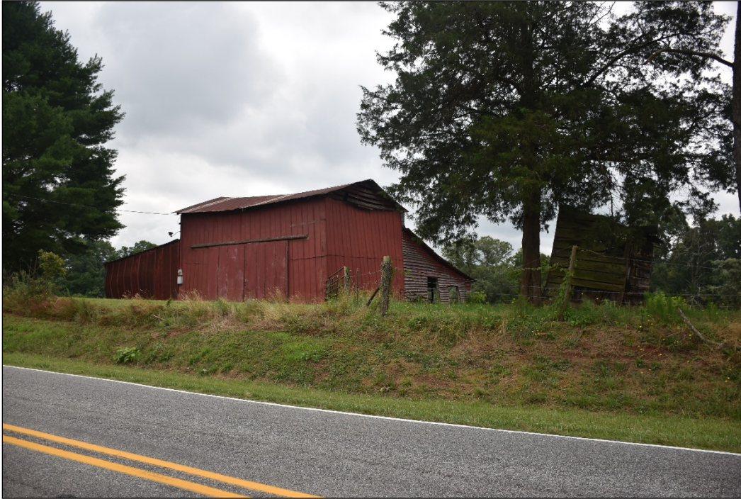
Figure 4.15. Hoover Barn (LN0812), facing southeast.
