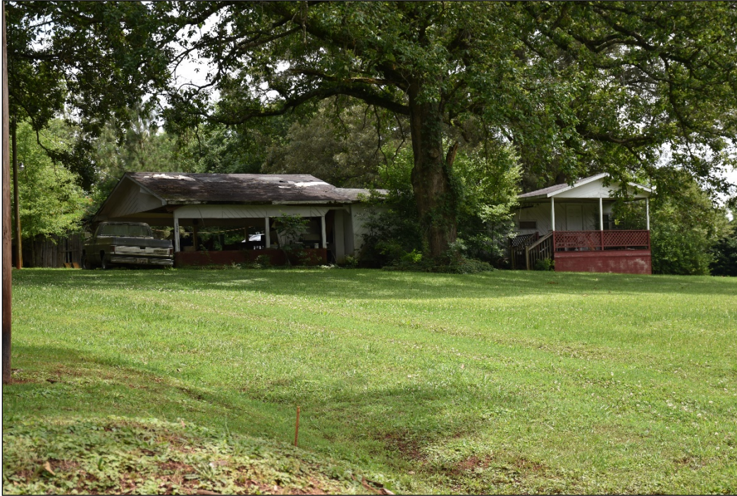
Figure 4.42. Wood House (LN0829), facing southeast.
