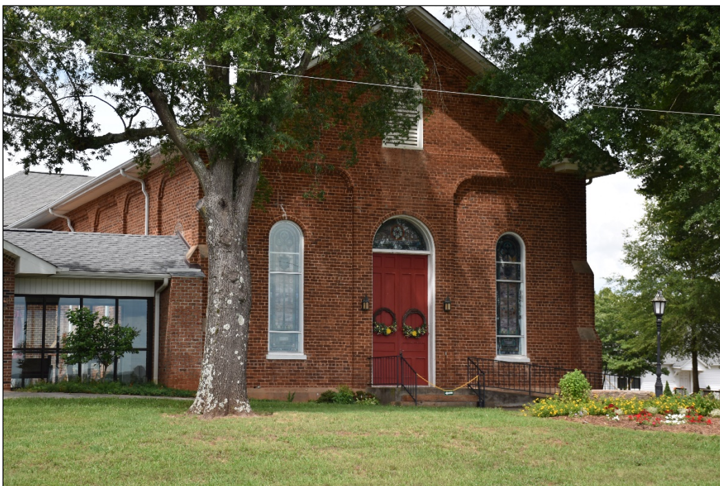
Figure 4.49. Daniels Lutheran Church (LN0159), facing north.
