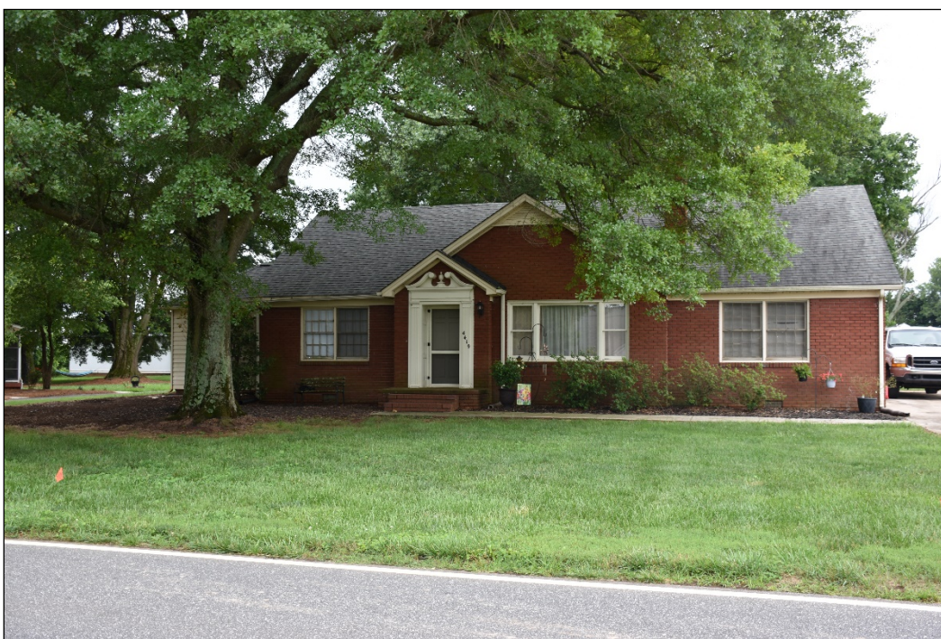
Figure 4.24. Moore House (LN0819), facing south.
