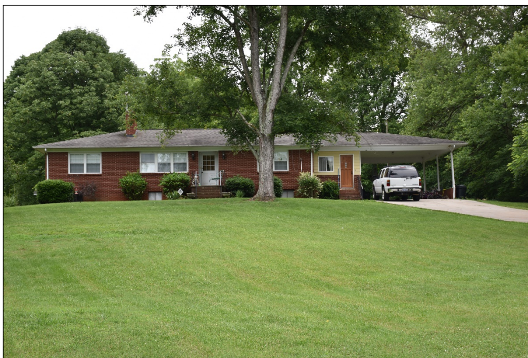
Figure 4.37. Springs House (LN0824), facing south.
