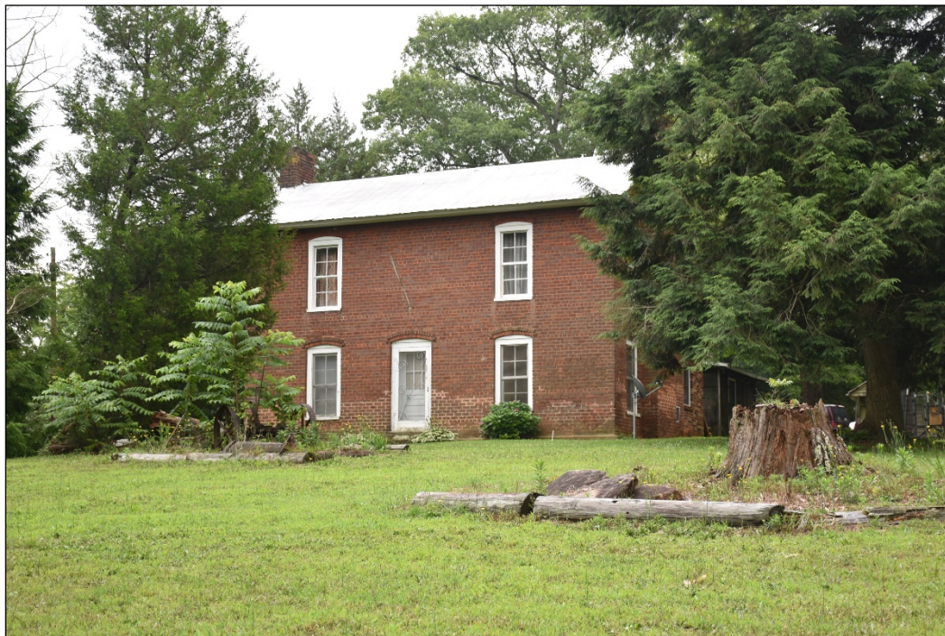
Figure 4.11. Eddney Hoover House (LN0087), facing southwest.
