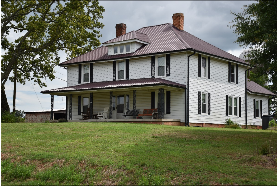
Figure 4.65. Leonard House (LN0835), facing south.
