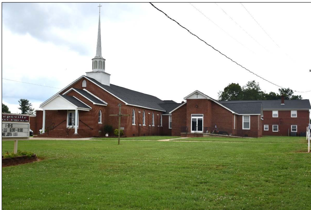
Figure 4.31. Reepsville Baptist Church (LN0822), facing southeast.
