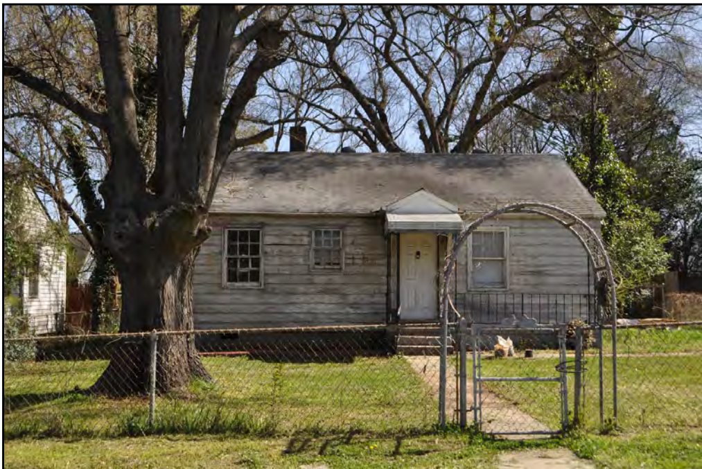
Plate 9.8: House with original wood siding and windows in Douglas Terrace (2308 Vanderbilt Road).
