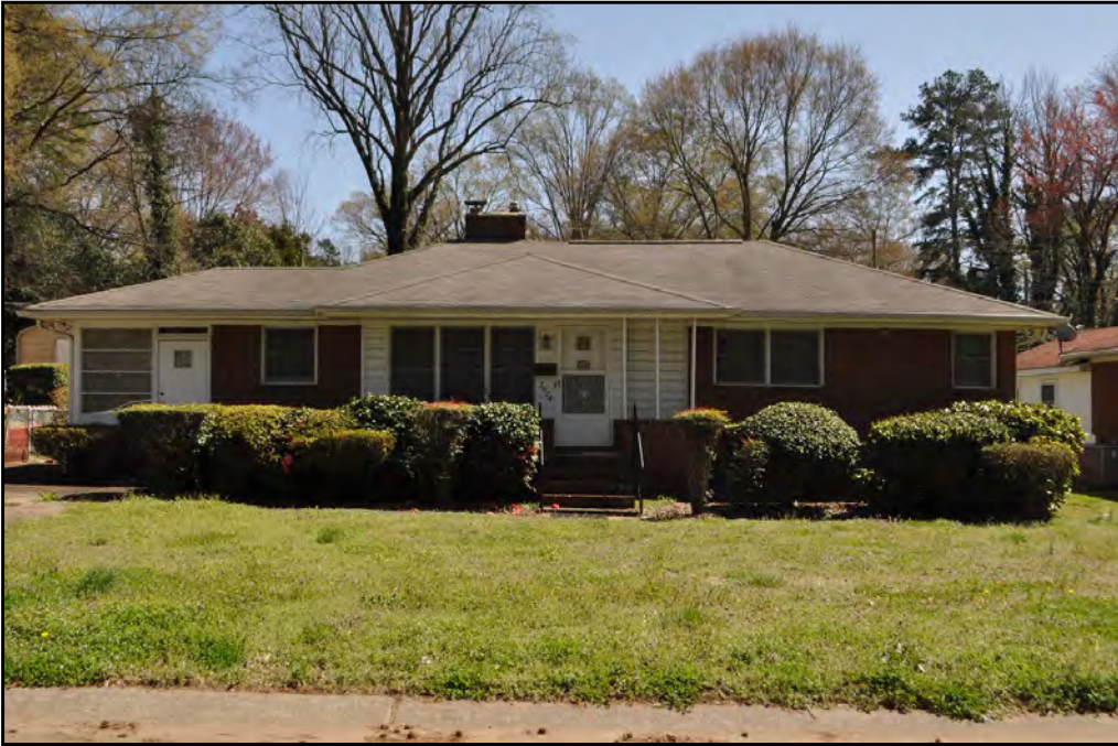
Plate 5.8: Linear Ranch in Graham Heights West (2624 Jefferson Davis Street).
