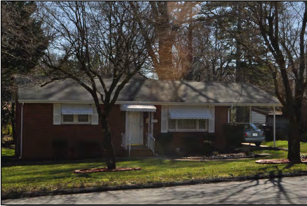
Plate 3.8: Compact Ranch house with metal porch posts and awnings in Graham Heights (2714 Dogwood Avenue).
