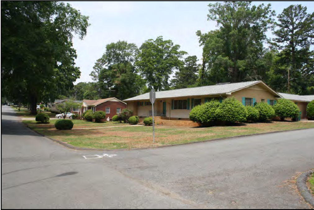
Plate 3.11: Typical Ranch house in McCrorey Heights (1624 Madison Avenue).
