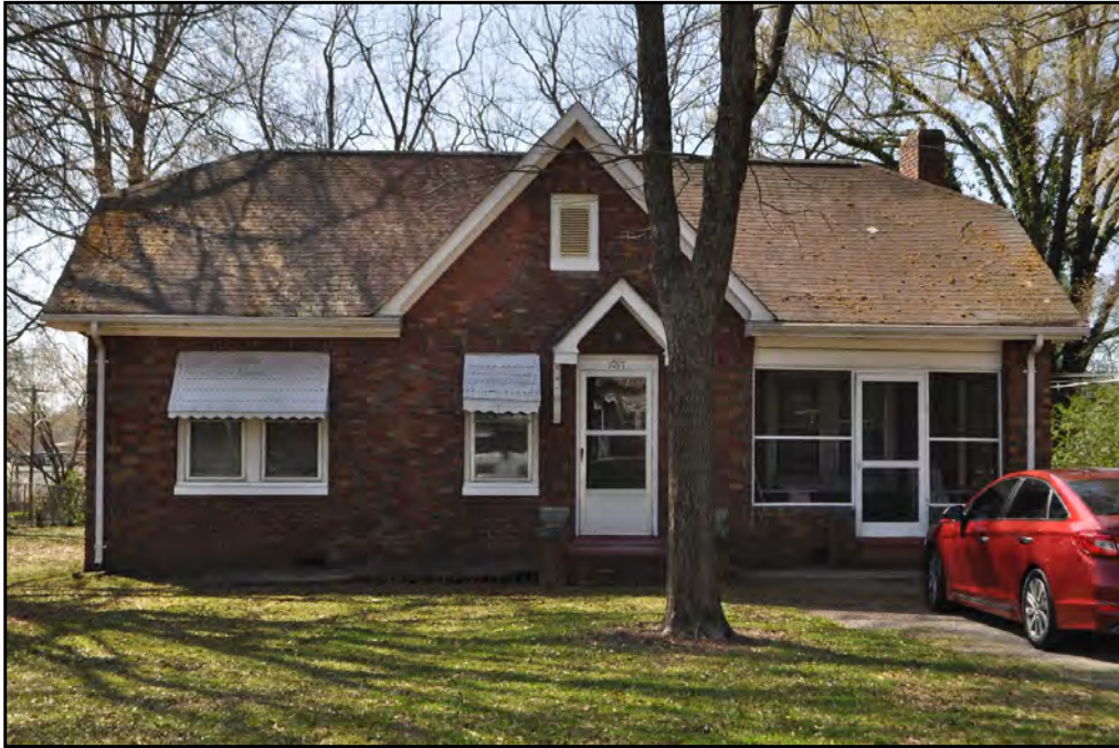
Plate 9.5: Minimal Traditional/Tudor Revival house in Douglas Terrace (1017 Kohler Avenue).
