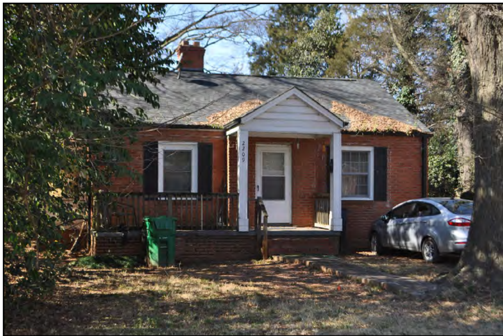
Plate 11.4: Typical brick-veneered Minimal Traditional house in Graham Heights (2209 Bancroft Street).
