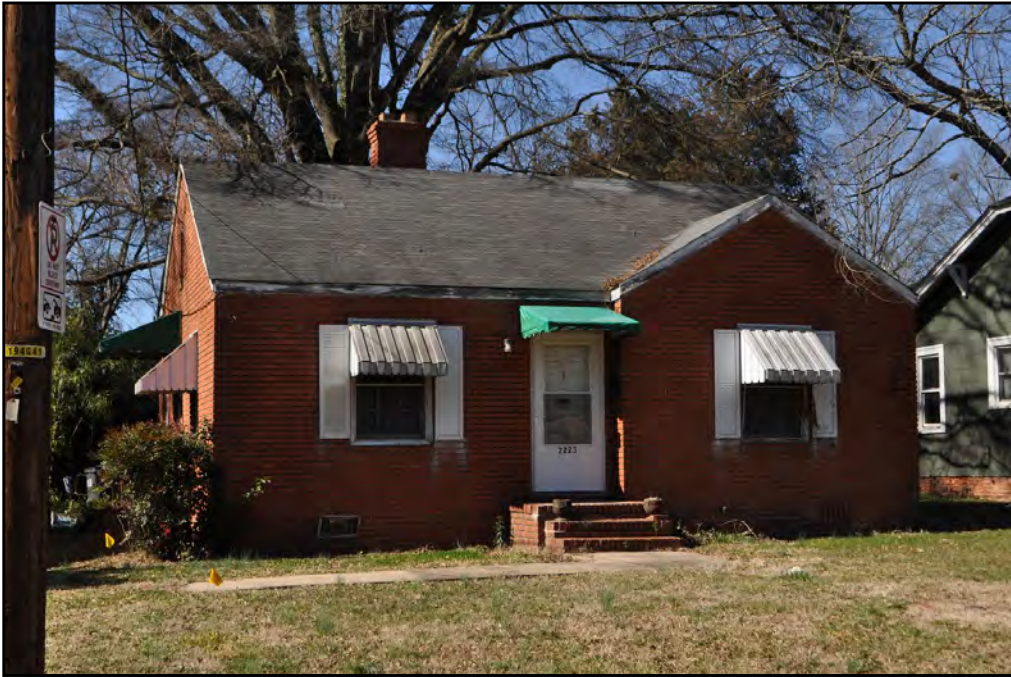
Plate 3.1: Typical brick-veneered Minimal Traditional house in Graham Heights (2223 Bancroft Street).
