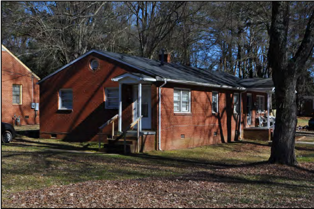
Plate 3.4: Minimal Traditional duplex in Graham Heights (2802 Grimes Street).
