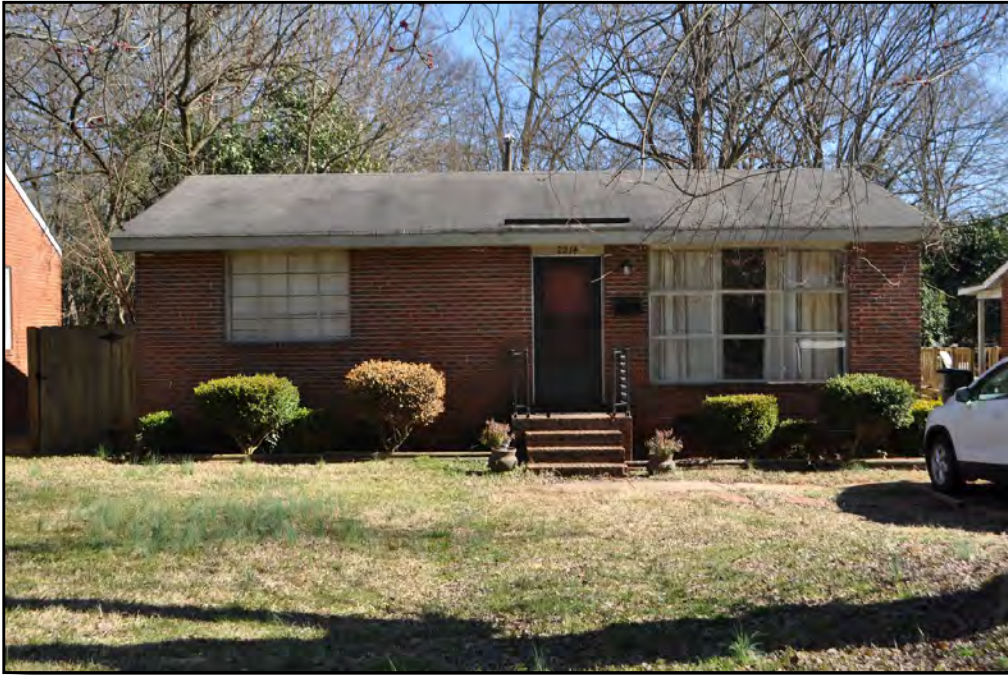
Plate 11.8: Compact Ranch with metal casement and picture windows in Graham Heights (2214 Bancroft Street).
