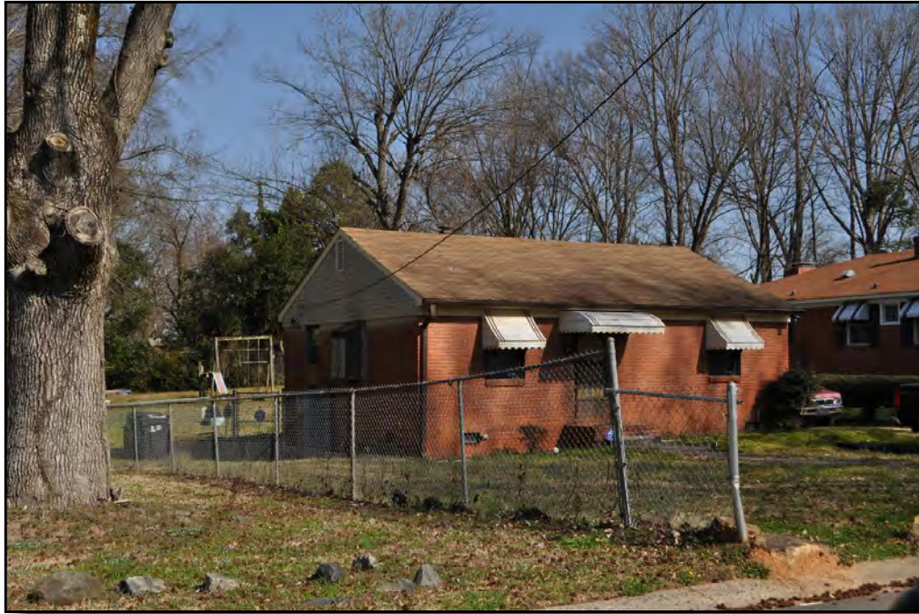
Plate 7.3: Typical Minimal Traditional house in Druid Hills South (1012 Druid Circle).
