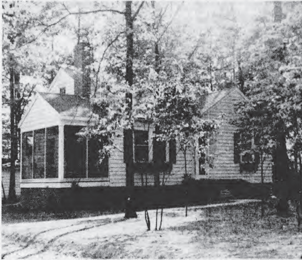
New Home of H. G. Propst, 3101 Dogwood Avenue
