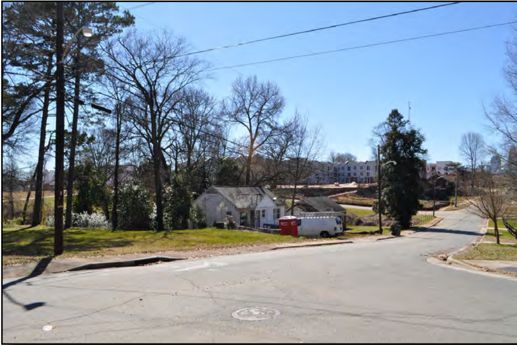
Plate 11.2: View of vacant lots on Catalina Avenue in Graham Heights where multiple houses have been demolished.
