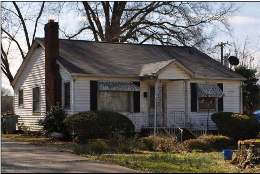
Plate 10.3: Minimal Traditional house in Mona Drive with replacement siding and windows (1133 Mona Drive).
