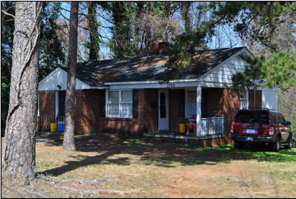
Plate 3.6: Compact Ranch house with Colonial Revival details in Graham Heights West (1200 Moretz Avenue).
