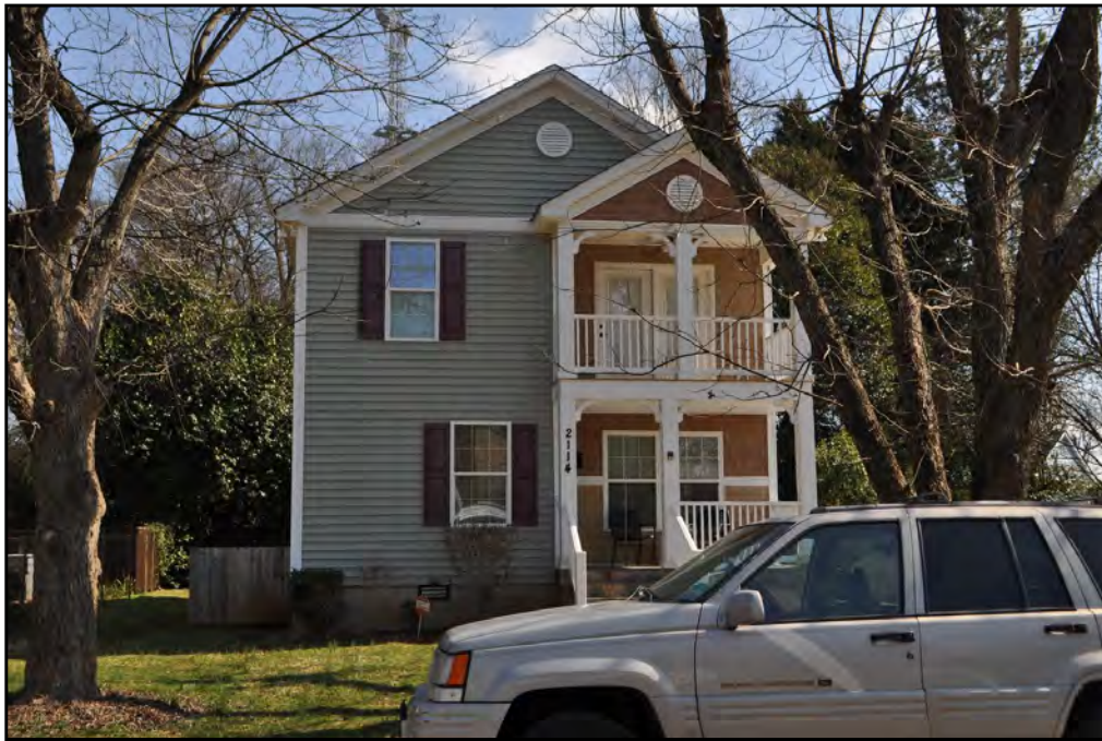
Plate 8.6: New construction in Edison Heights (2114 Edison Street).
