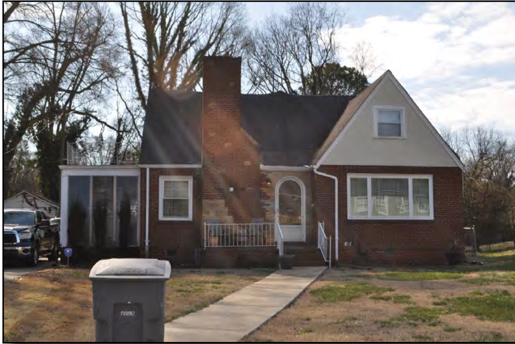
Plate 7.7: Tudor Revival style house in Druid Hills South (1017 Druid Circle).
