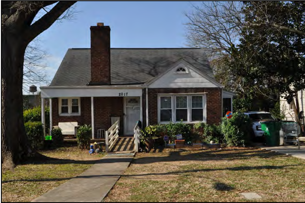
Plate 8.3: Minimal Traditional house with gable-front wing and façade chimney in Edison Heights (2017 Edison Street).
