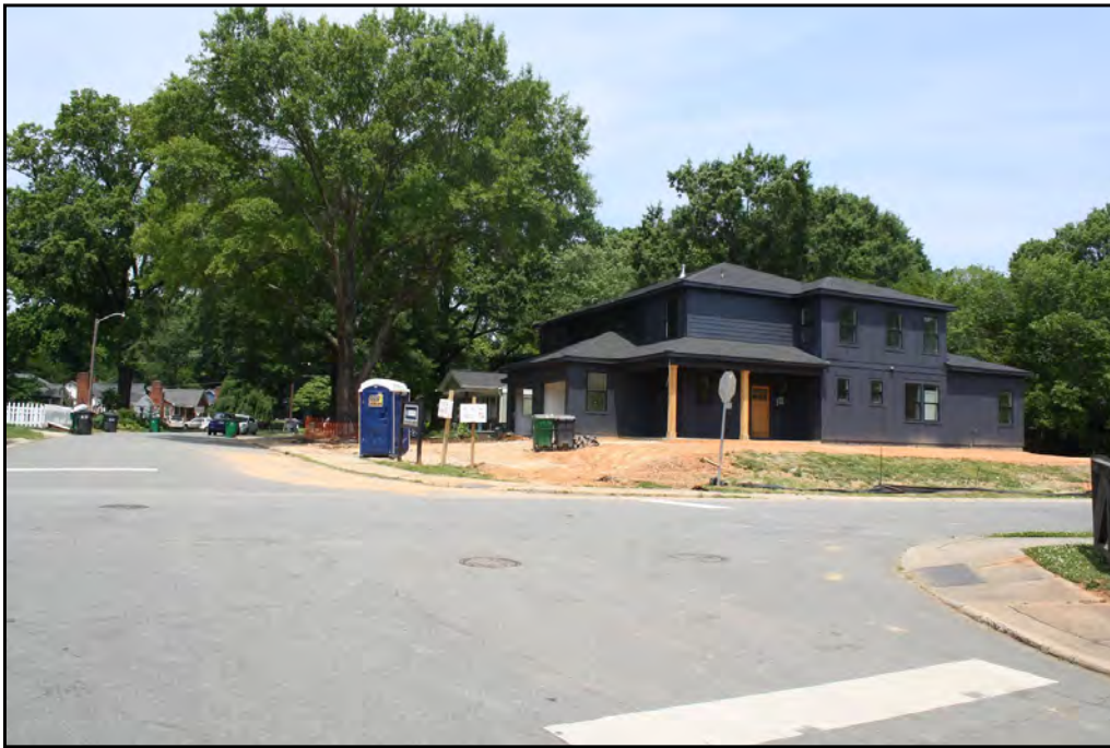
Plate 3.13: New construction in Plaza Acres (1255 Meadow Lane).
