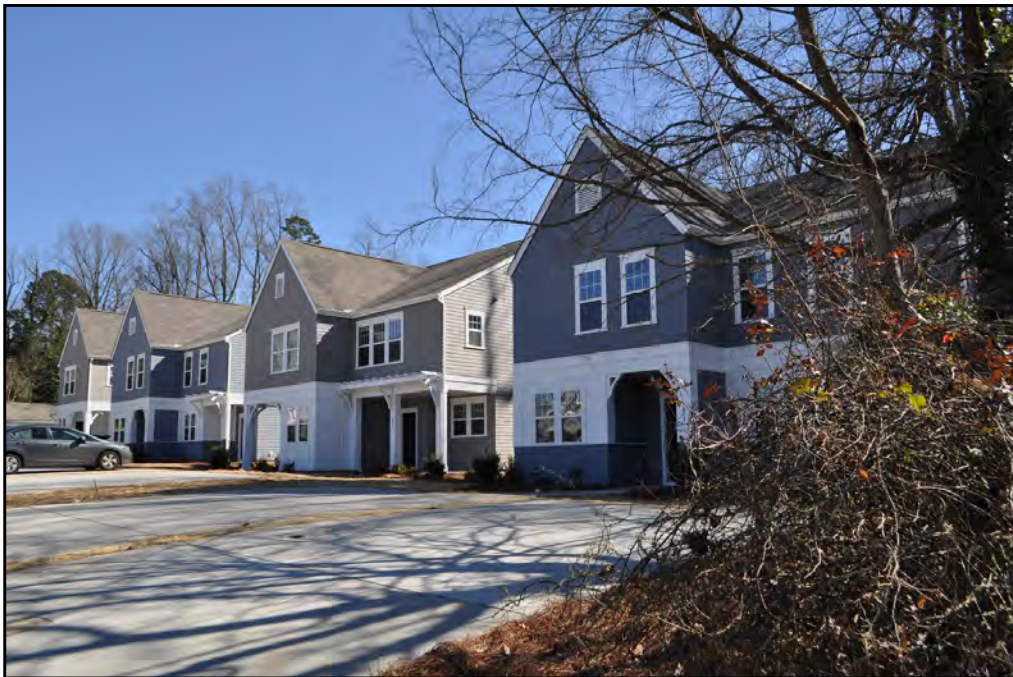
Plate 6.6: New construction in Statesville Avenue Terrace/Druid Hills North (805-817 McArthur Avenue).
