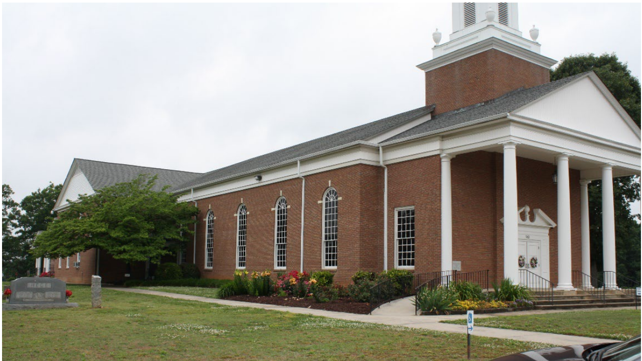
Figure 10: South elevation of sanctuary
