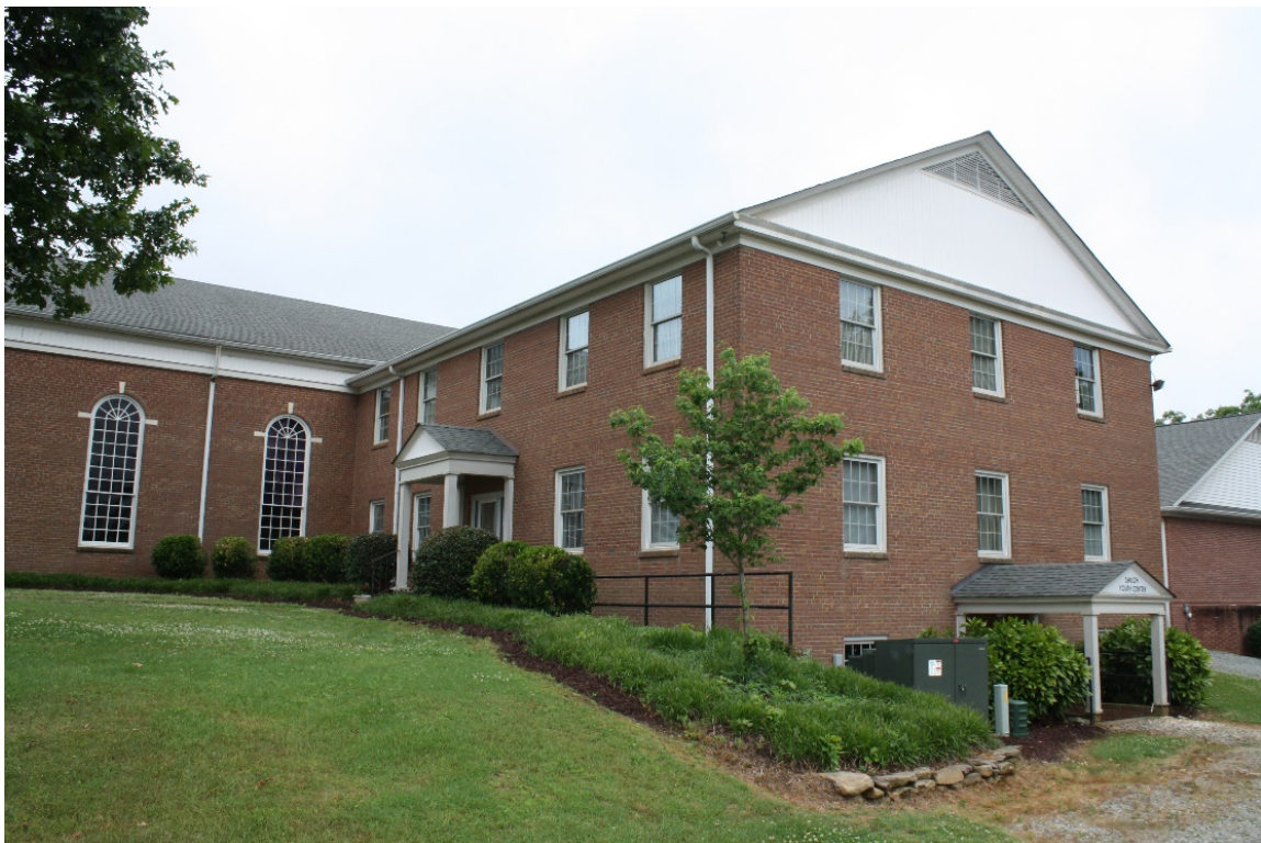
Figure 22: Facing south to the east elevations of education wing, sanctuary to the east
