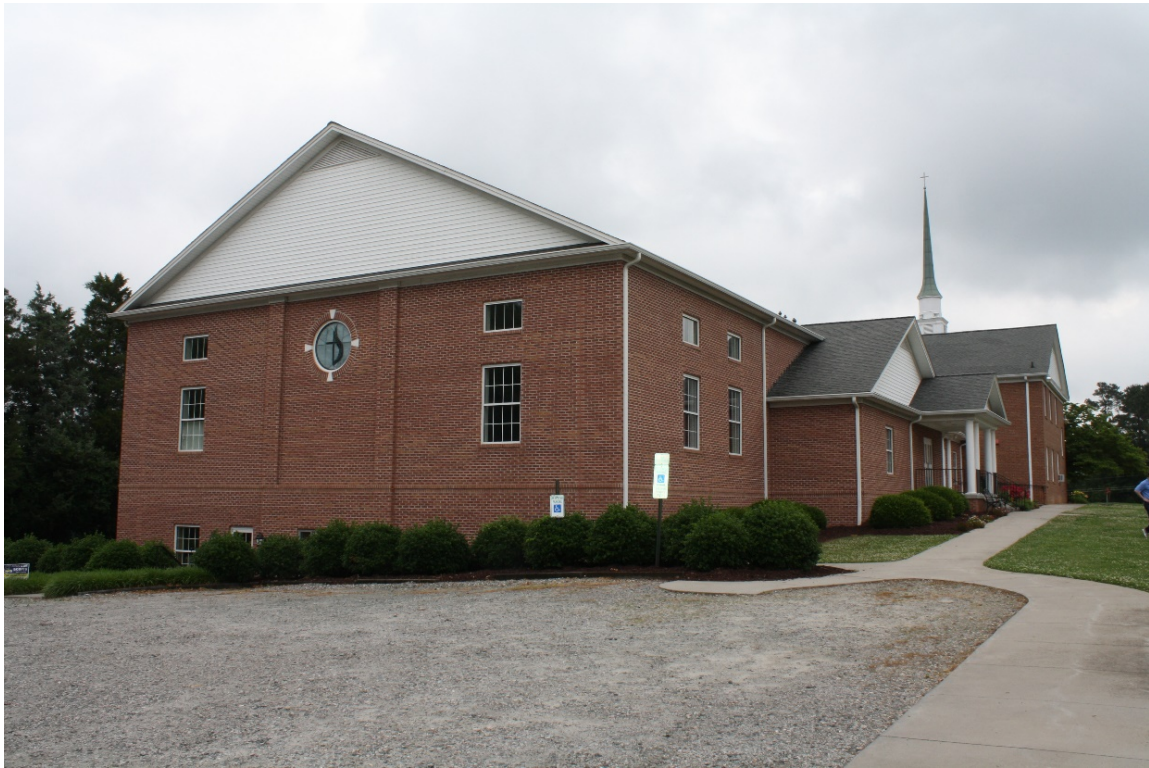
Figure 17: Looking east to west and south elevations of 2008 fellowship hall wing
