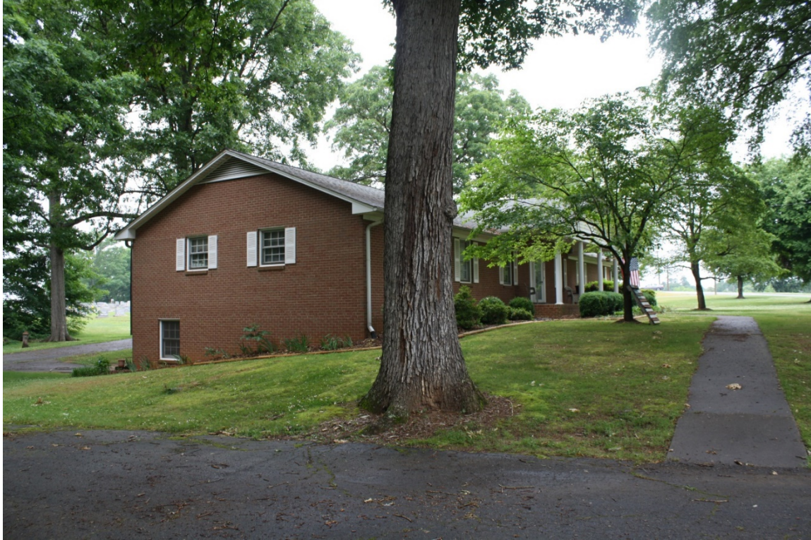
Figure 35: South and east elevations of 1967 parsonage
