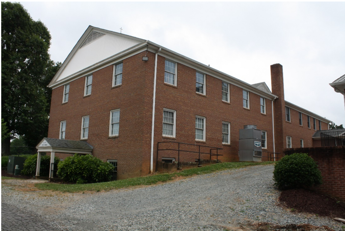
Figure 21: North and west (rear) elevations of 1960 office and classroom wing
