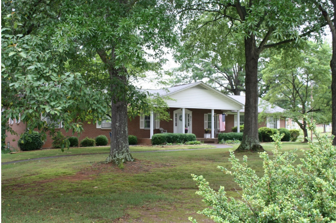
Figure 31: Front façade of 1967 parsonage
