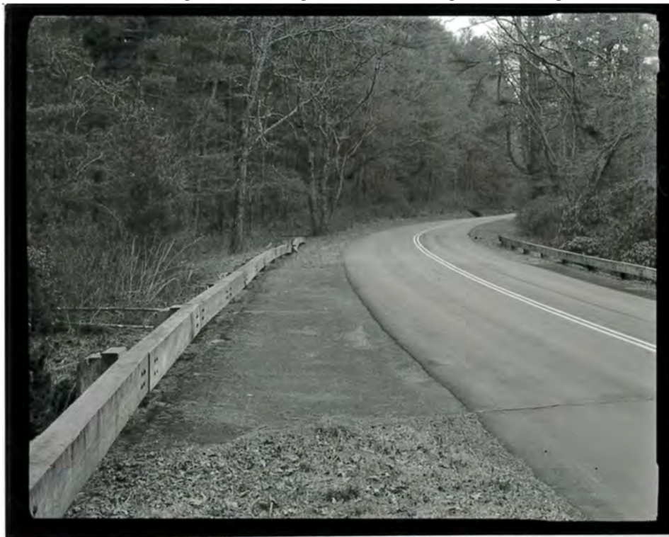
Photograph 18. View of Big Pine Creek Bridge #3, showing the bridge and asphalt shoulder, looking southeast (NC-42-C-8).
