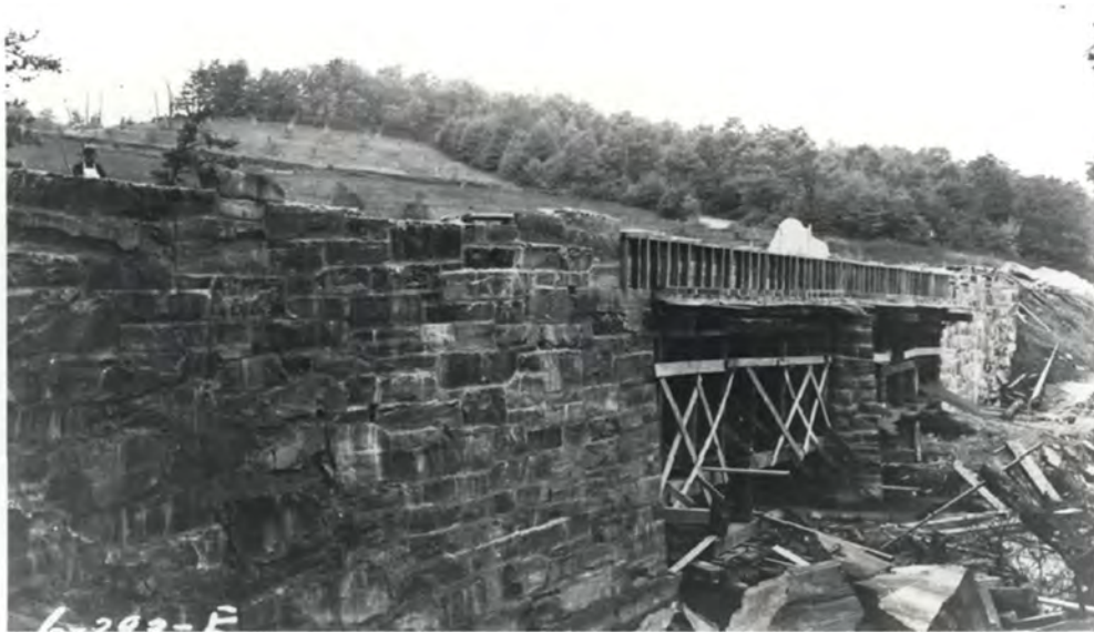
Figure 14. Photograph, ca. 1937, showing the construction of Brush Creek Bridge #1 (USDA BPR 1937).
