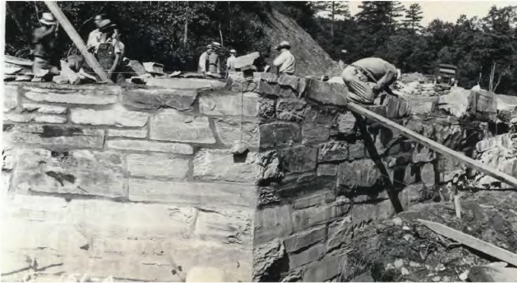
Figure 9. Photograph, ca. 1937, showing the construction of the abutment wings of Big Pine Creek Bridge #3 (USDA BPR 1937).
