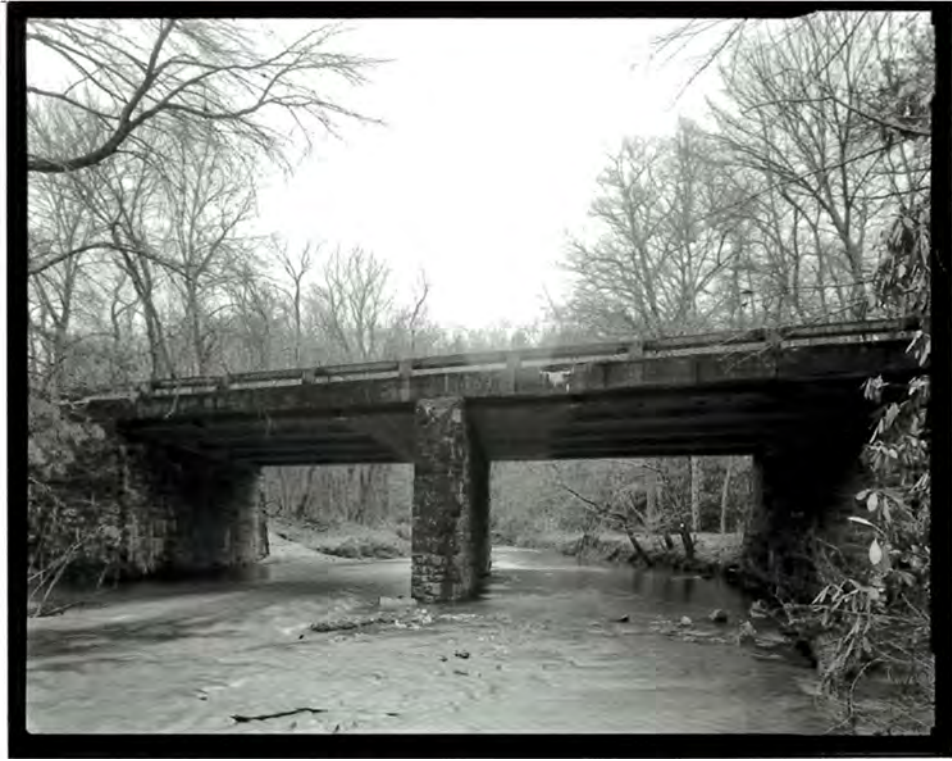
Photograph 32. View of Brush Creek Bridge #1, looking north-northeast (NC-42-E-7).
