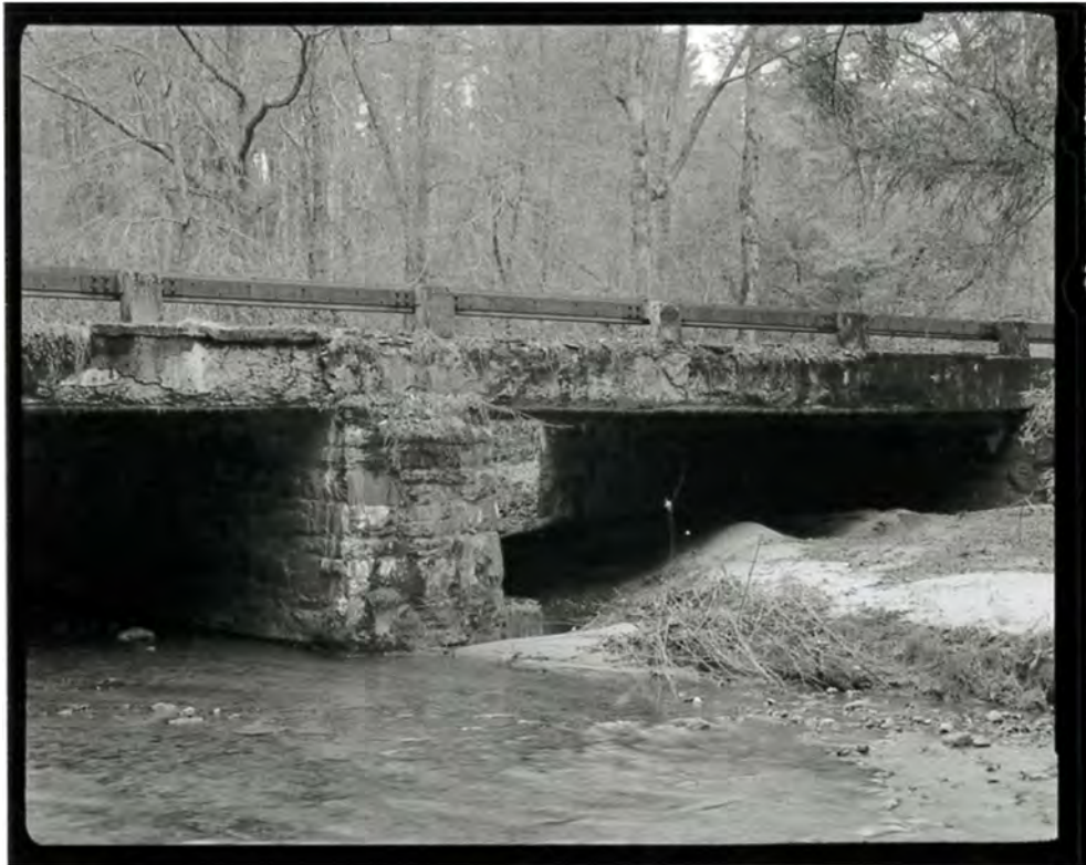
Photograph 20. View of Big Pine Creek Bridge #6, looking north-northwest (NC-42-D-2).
