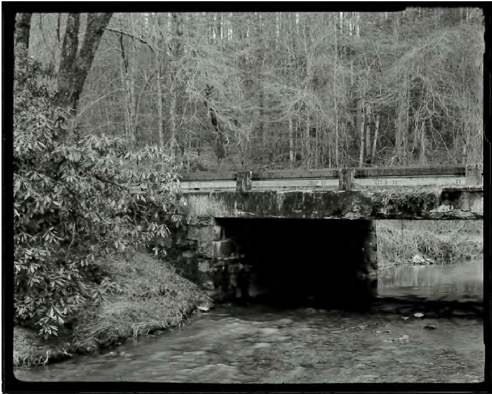
Photograph 21. View of Big Pine Creek Bridge #6, looking northwest (NC-42-D-3).
