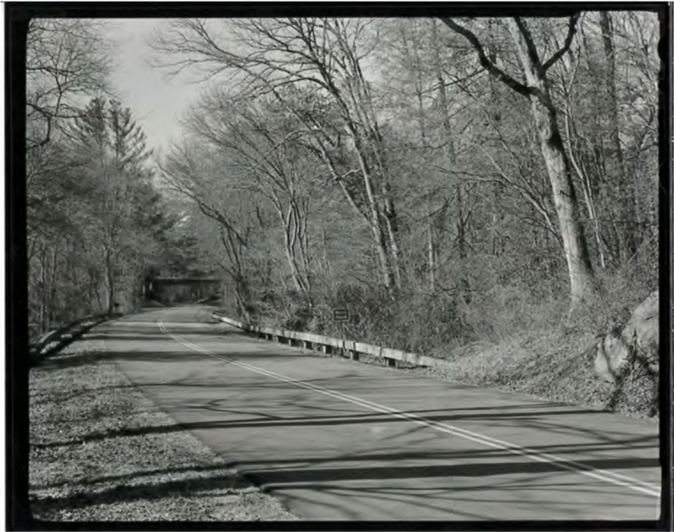
Photograph 26. View of Brush Creek Bridge #1, showing the deck, looking northwest (NC-42-E-1).
