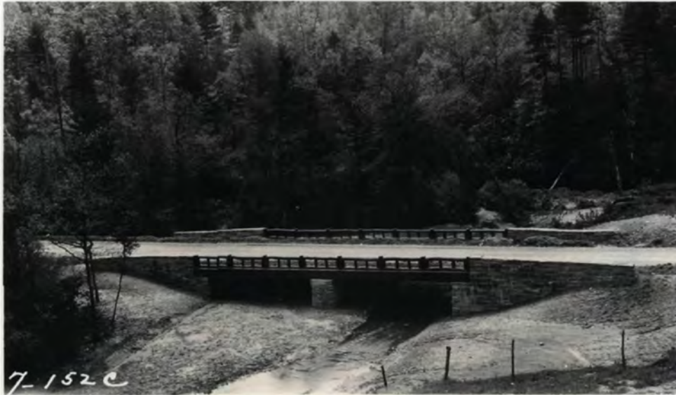
Figure 12. Photograph, ca. 1937, showing the newly completed Big Pine Creek Bridge #6 (USDA BPR 1937).
