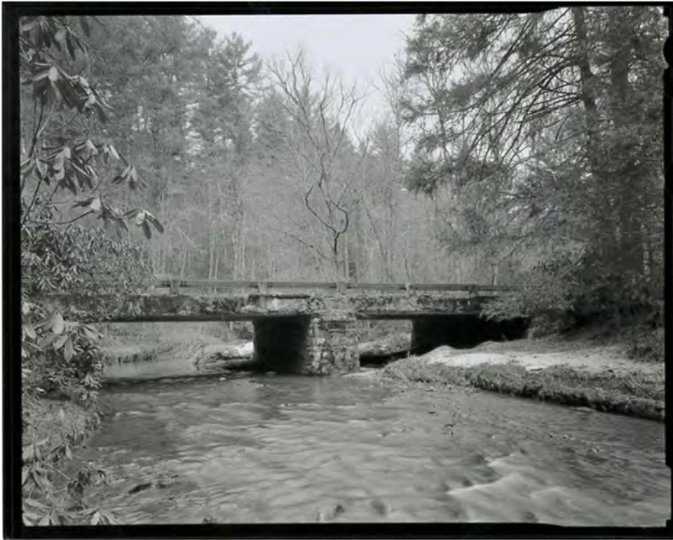
Photograph 19. View of Big Pine Creek Bridge #6, looking north-northeast (NC-42-D-1).
