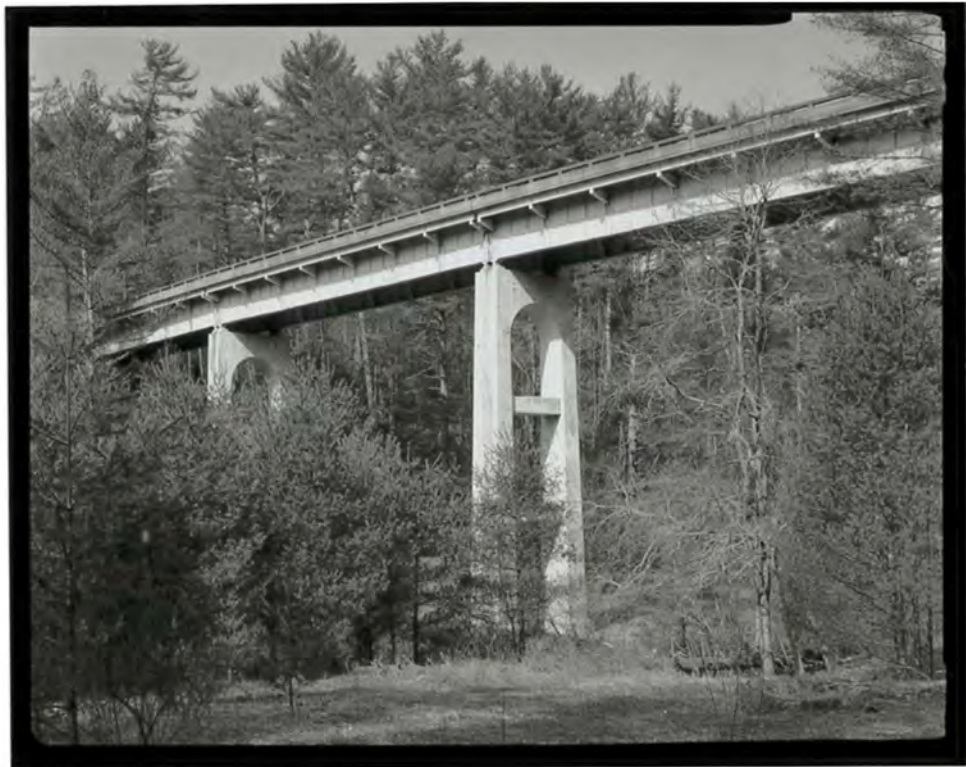
Photograph 4. South elevation of the Laurel Fork Viaduct, looking northwest (NC-42-B-4).
