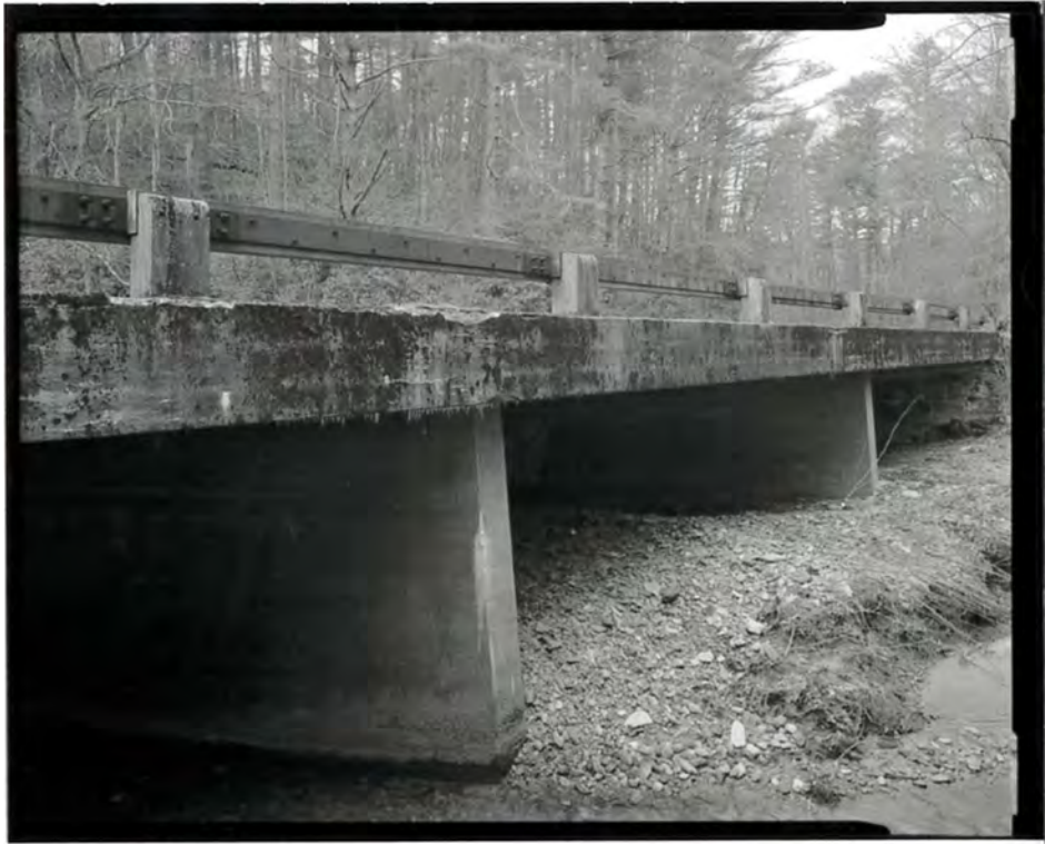
Photograph 11. Three-quarter view of Big Pine Creek Bridge #3, looking west-southwest (NC-42-C-1).
