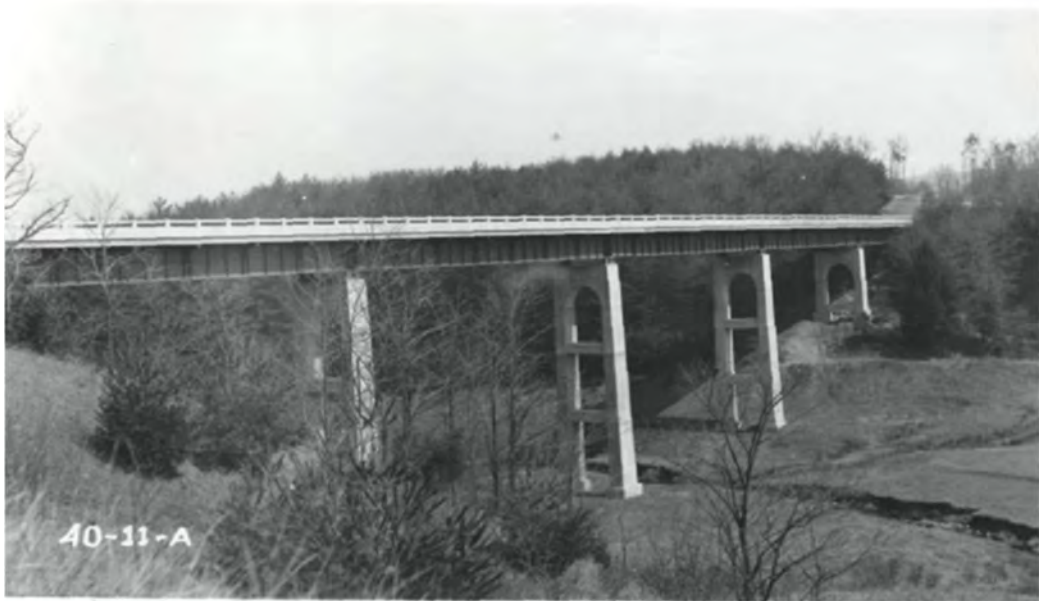
Figure 7. Photograph, ca. 1938, showing the newly completed Laurel Fork Viaduct (USDA BPR 1938).
