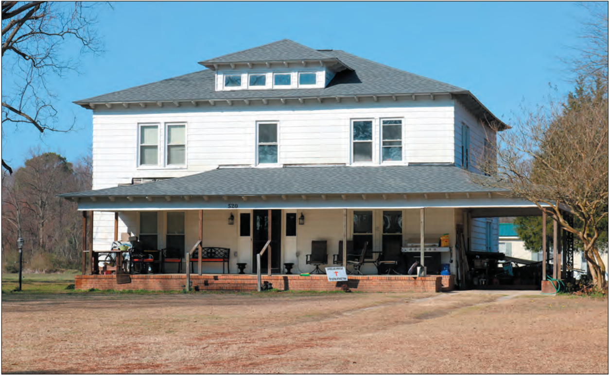
A. Dwelling, Looking West
