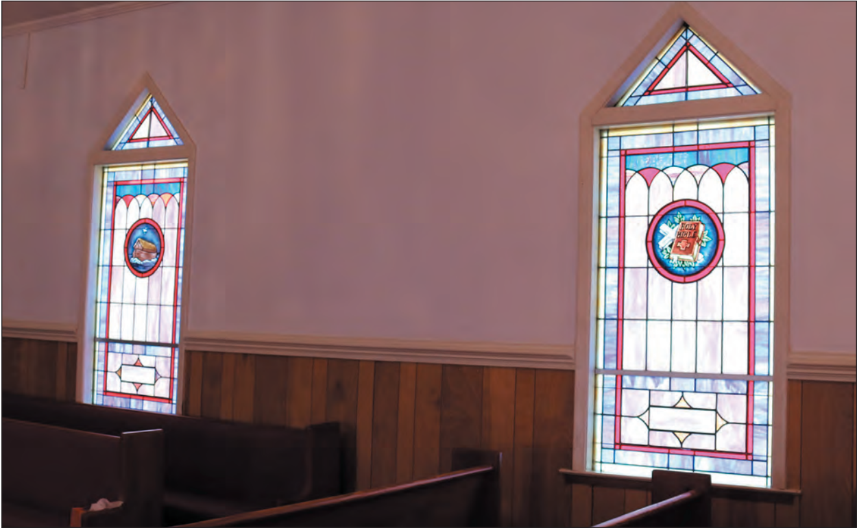
B. Original Windows, Looking Northeast
