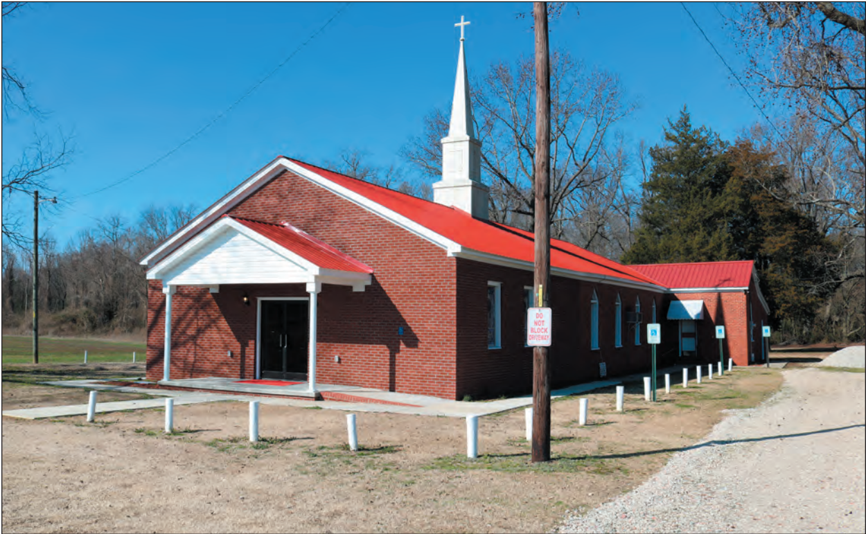
B. Looking Northwest
