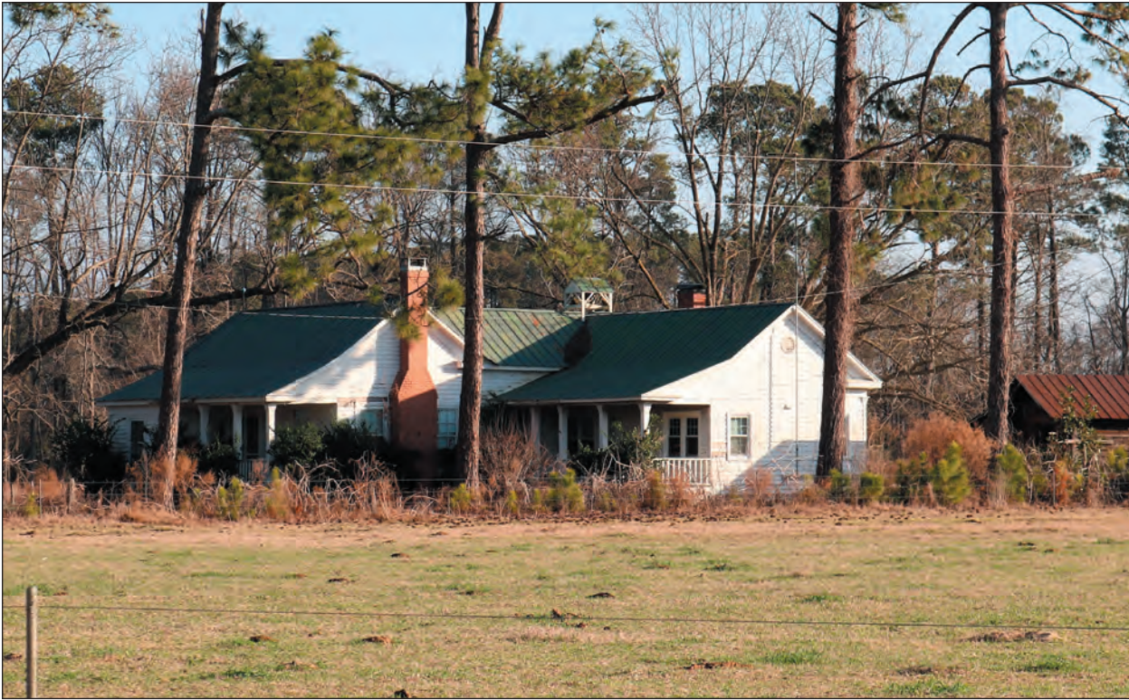
A. Dwelling, Looking Northeast
