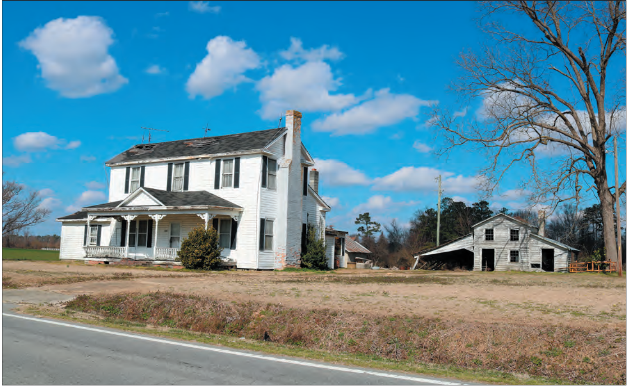
Figure 62. Photograph of Resource SP0380, Dwelling and Garage, Looking North
