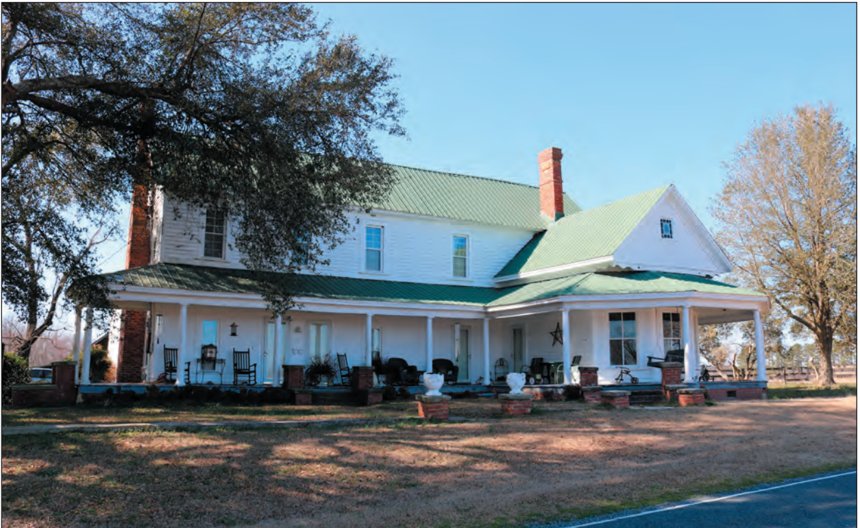
B. Looking Northwest
