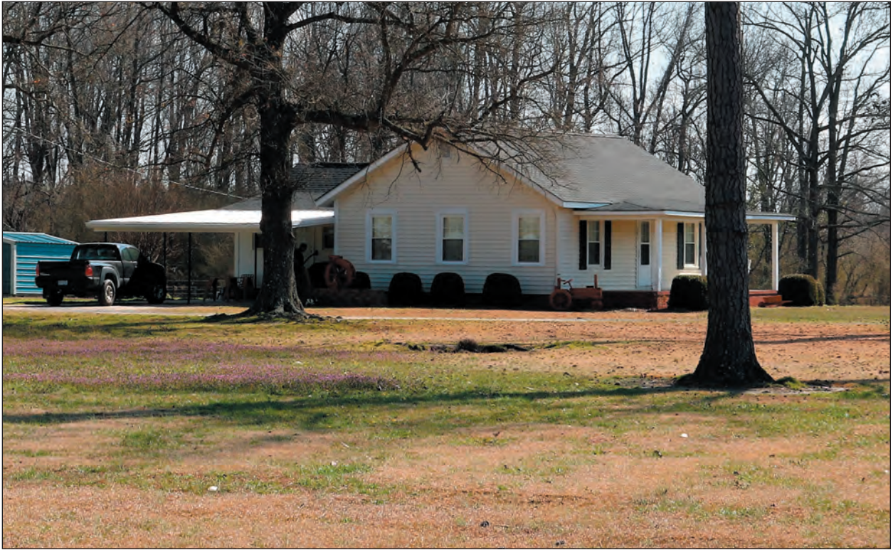
A. Looking Southeast
