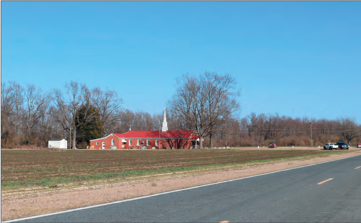
A. Looking Northeast
