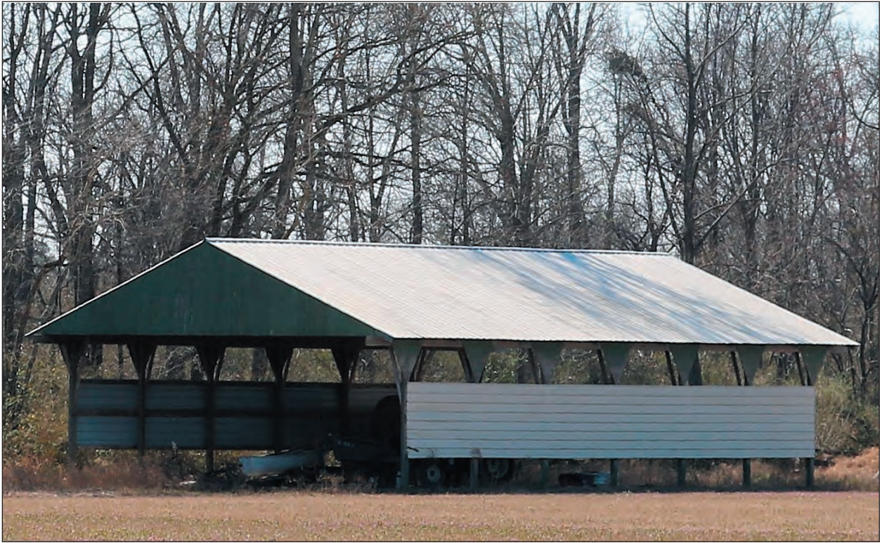
Figure 50. Photograph of the pole barn at SP0188, Looking Southwest, Looking Southwest
