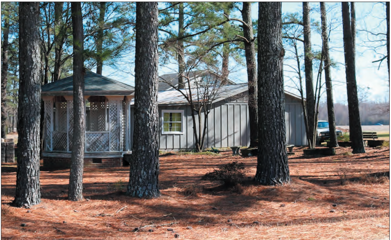
B. Multi-bay Garage and Gazebo, Looking Northeast
