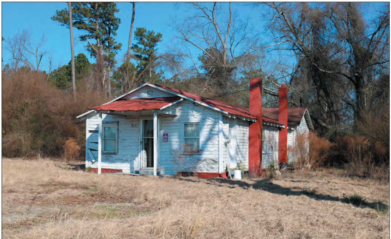
B. Looking Northwest
