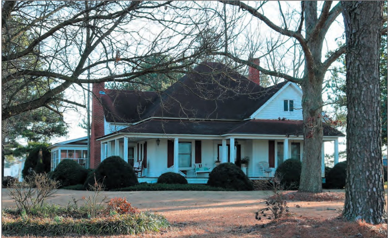
Figure 26. Photographs of Resource SP0753, Looking West
