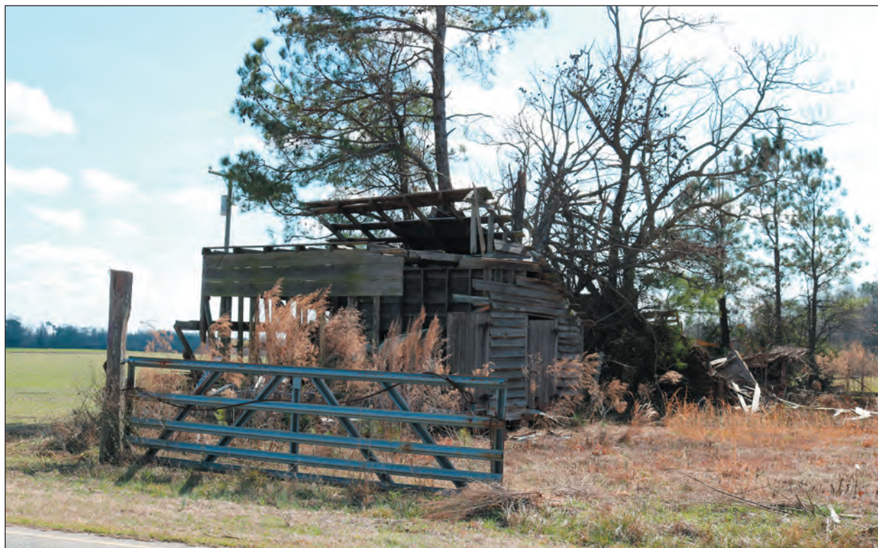
Figure 57. Photograph of Resource, Barn, SP0377, Looking Southeast
