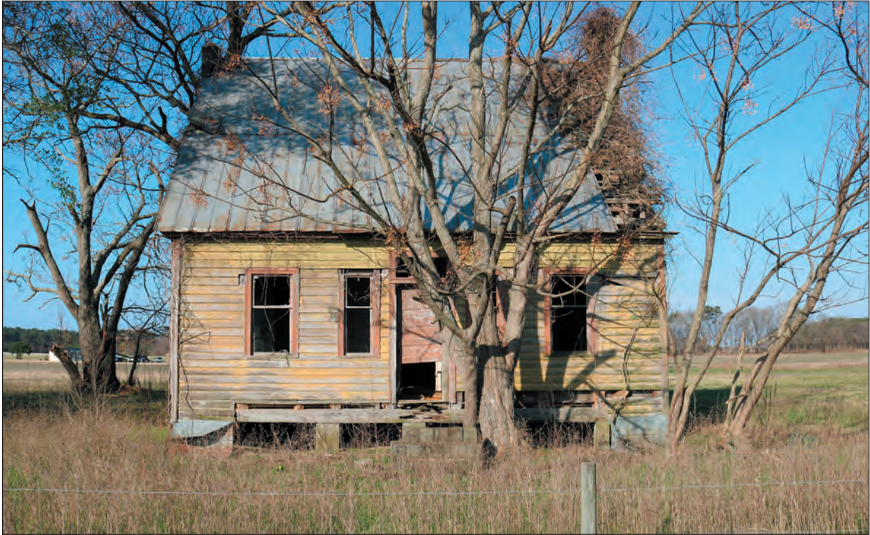
A. Looking West
