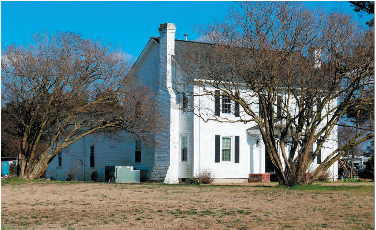
B. Main Dwelling, Looking Southeast
