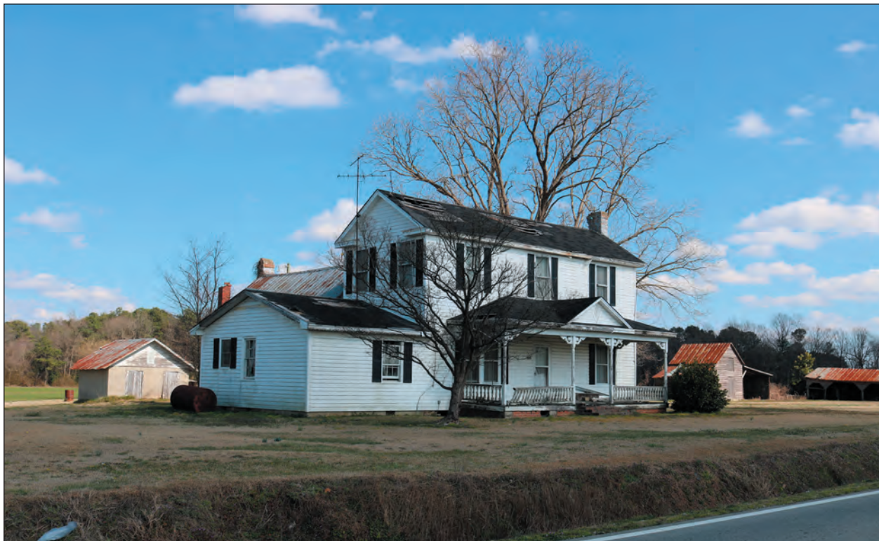
B. Dwelling, Looking Northeast
