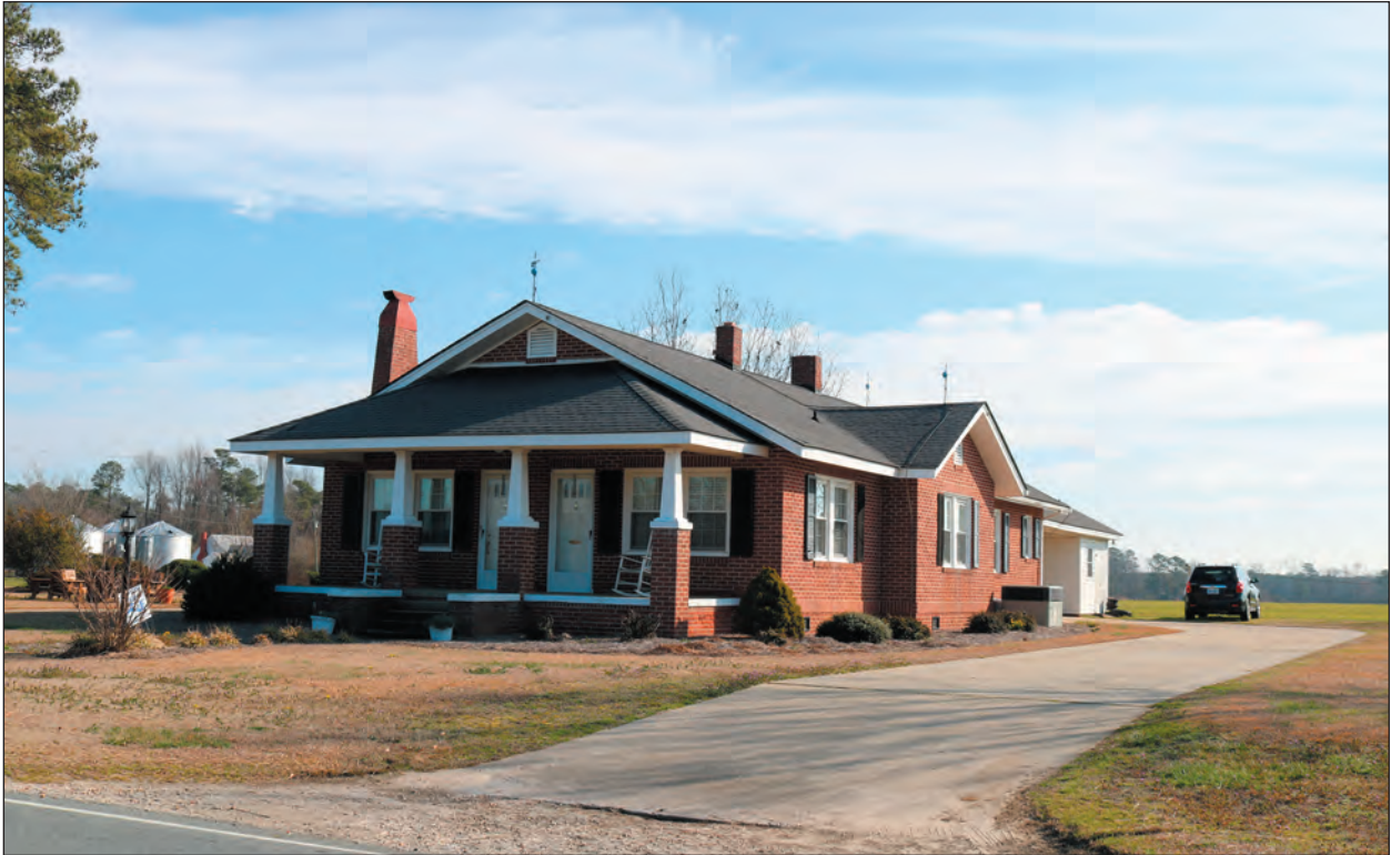
A. Looking Northeast
