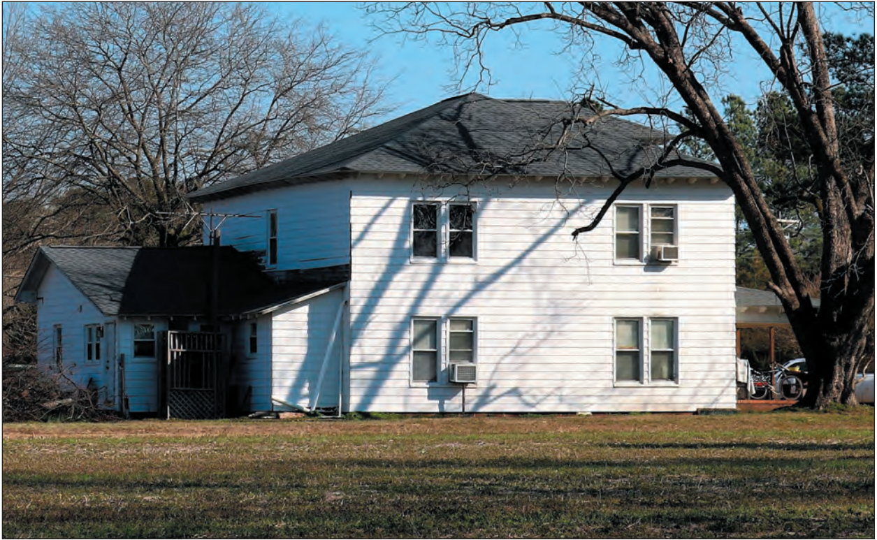
A. Dwelling, Looking Northeast
