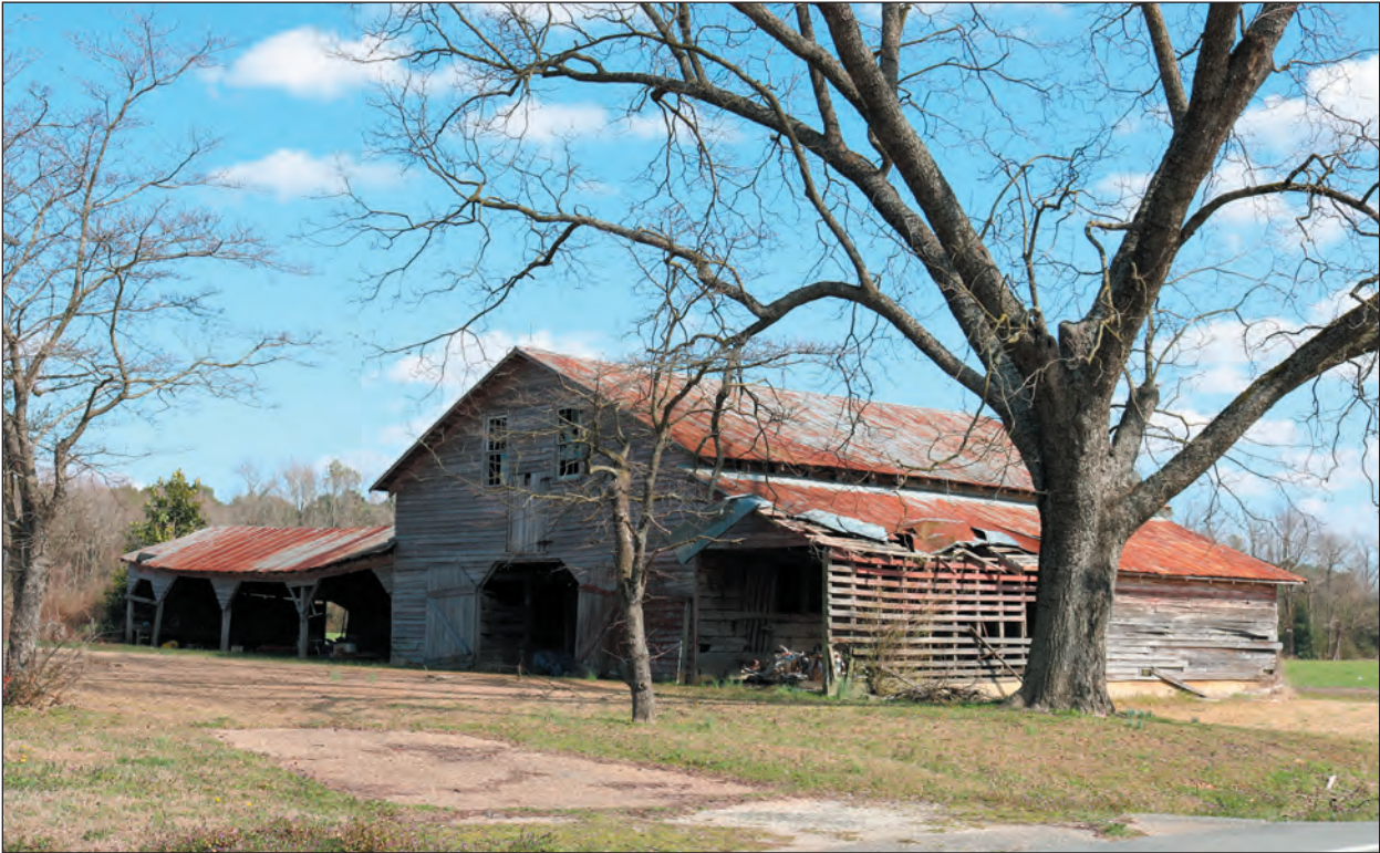
B. Outbuilding, Looking Northeast
