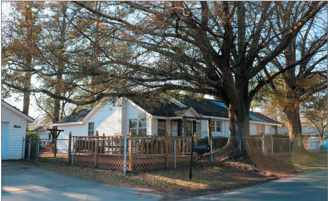
B. Looking Northwest
