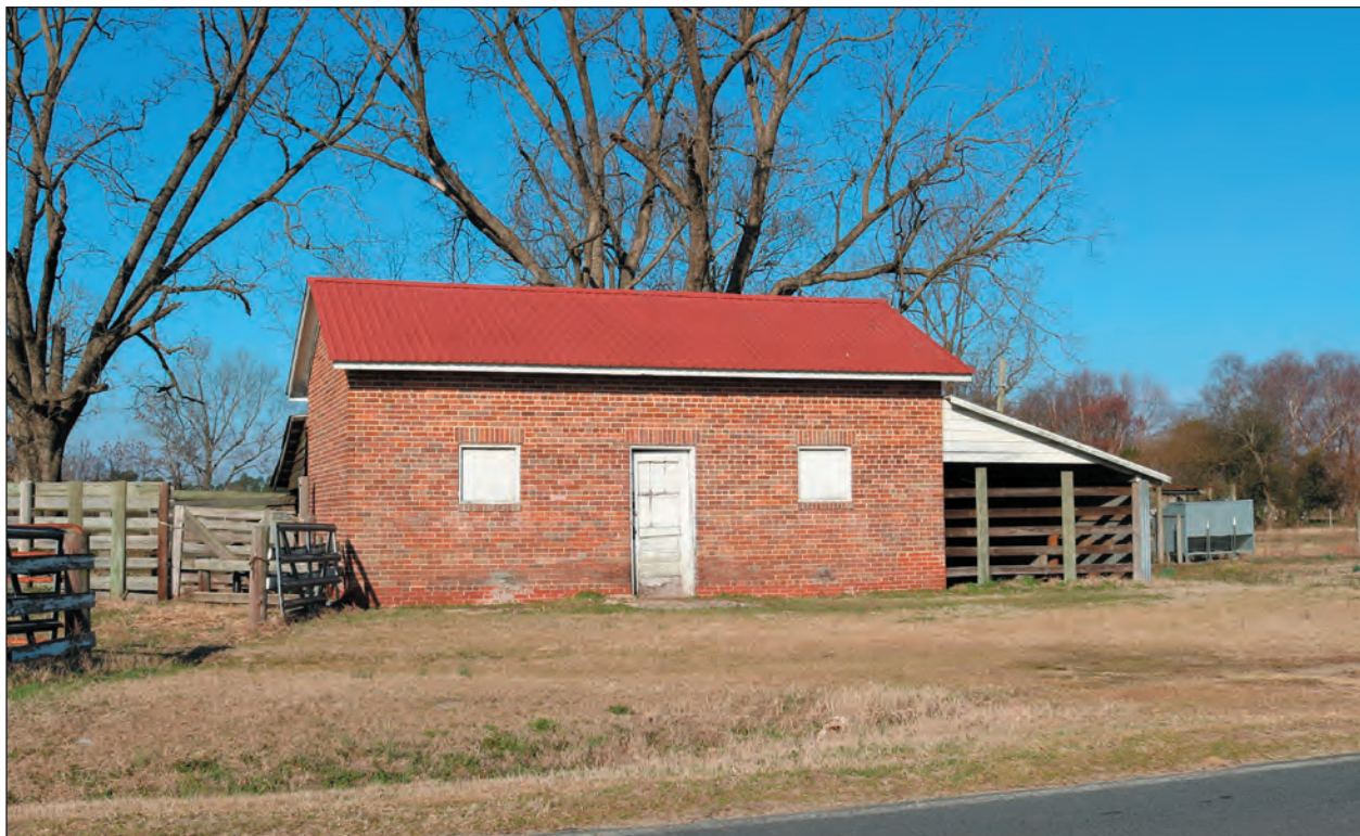
B. Former Commercial Building, Looking West
