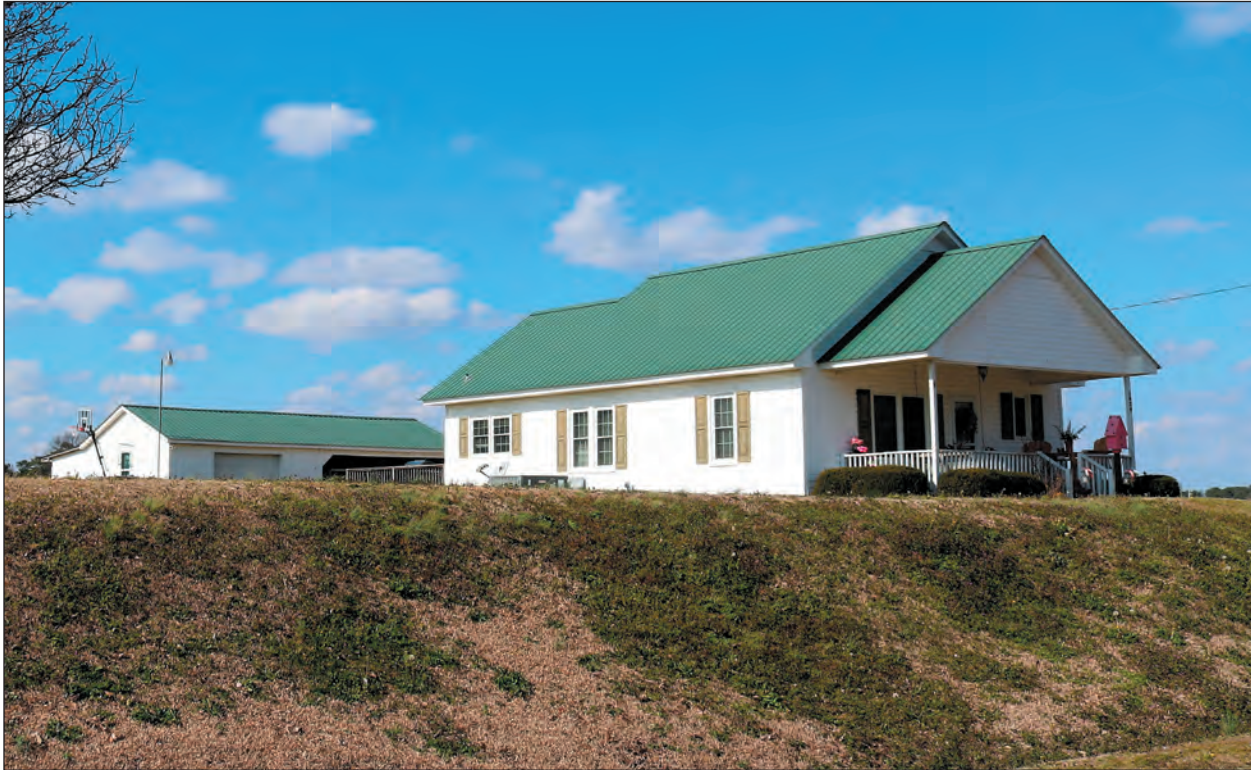
B. Looking Northwest
