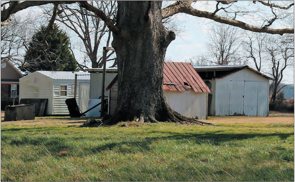
Figure 39. Photographs of Resource SP0763, Outbuildings, Looking Southeast
