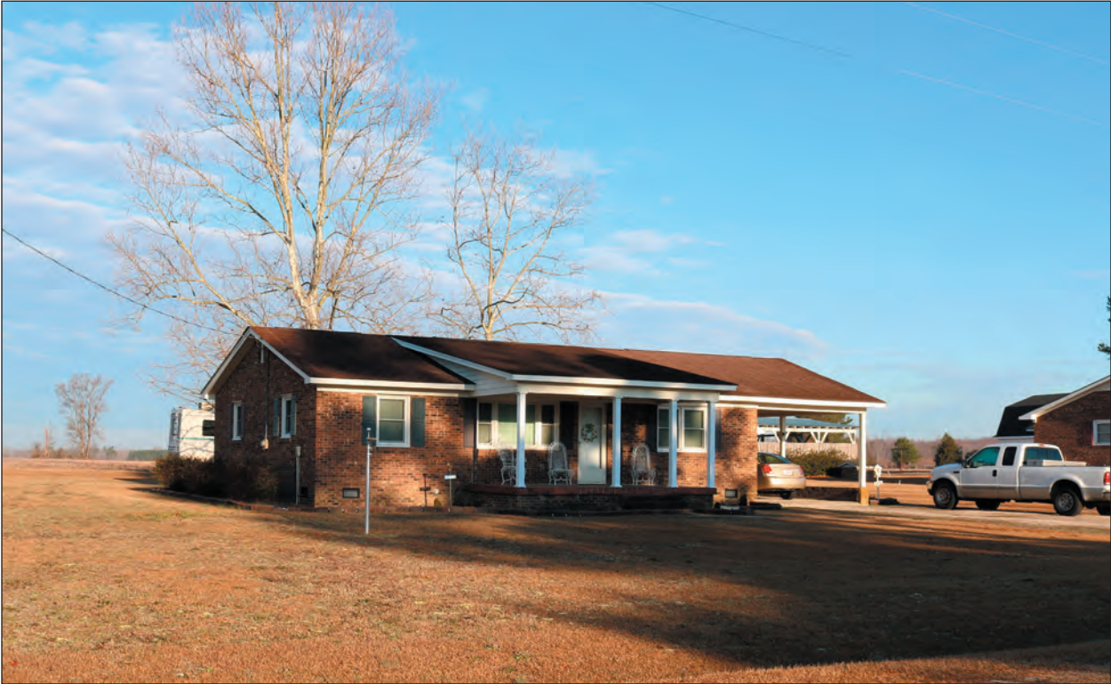
Figure 3. Photograph of Resource SP0739, Looking Northwest
