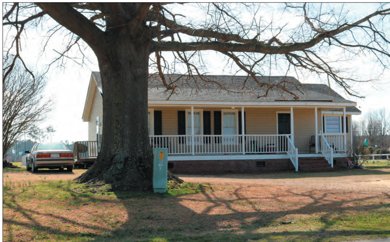
Figure 60. Photograph of Resource SP0379, Looking Southwest
