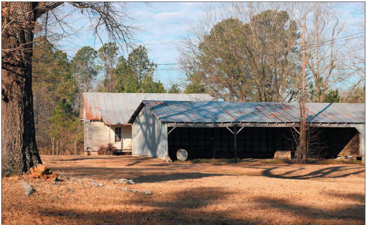
B. Equipment Shed, Looking West
