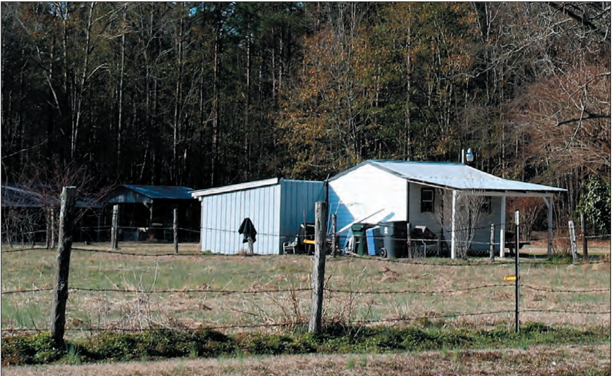
B. Outbuildings, Looking Southwest
