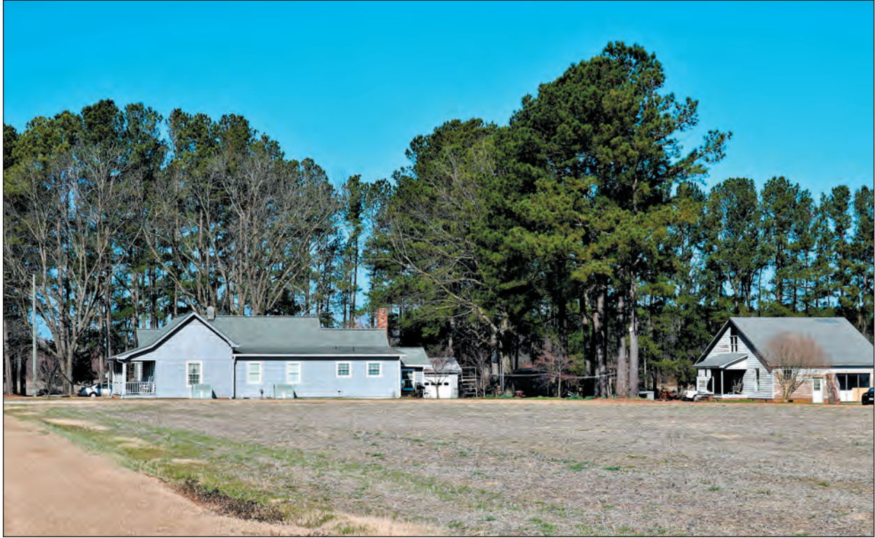
Figure 12. Photograph of Resource SP0745, Looking Northwest
