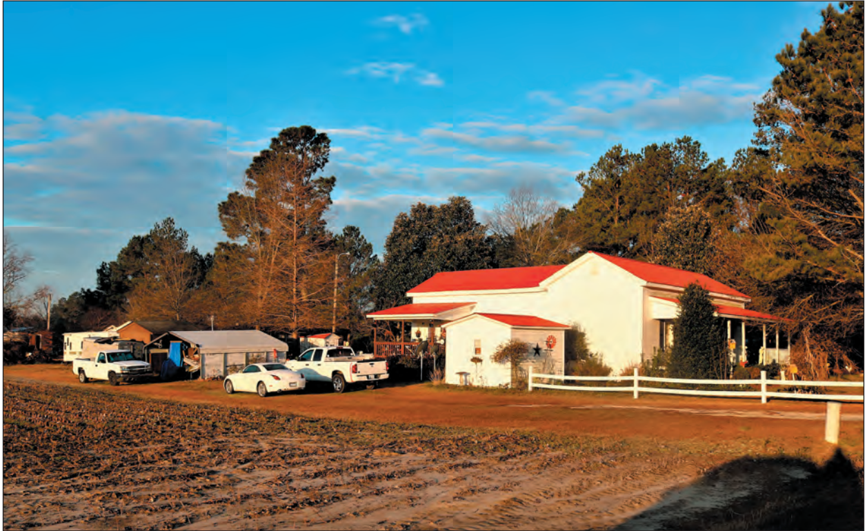
Figure 2. Photograph of Resource SP0738, Dwelling and Outbuildings, Looking West
