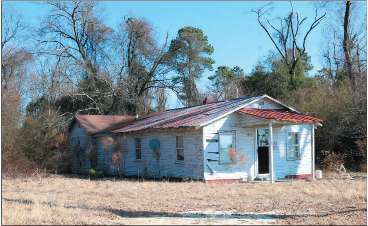
A. Looking Northeast
