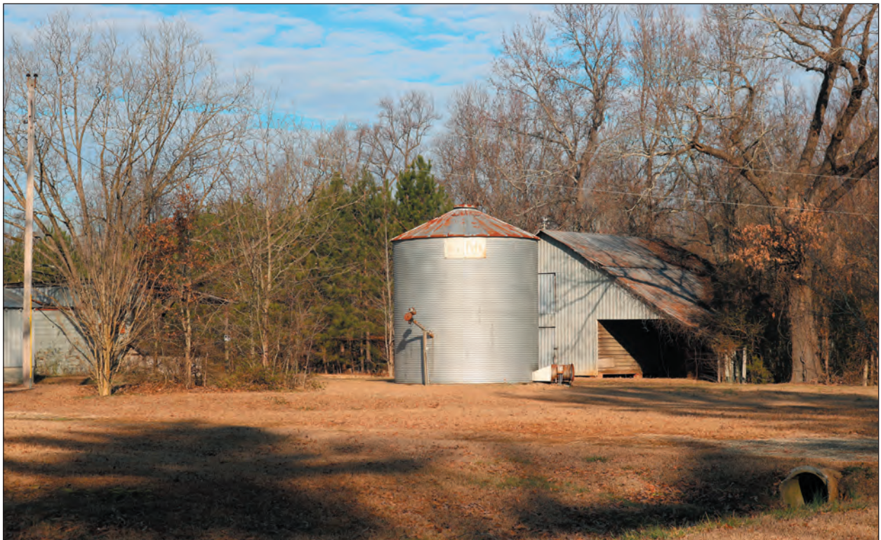
B. Metal Silo, Looking Northwest
