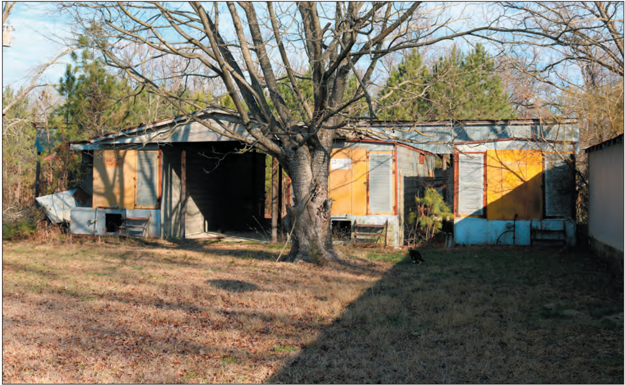
A. Modular Storage Building, Looking North
