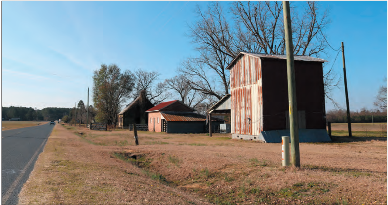
Figure 67. Photograph of Resource SP0523, Full Site, Looking Southwest
