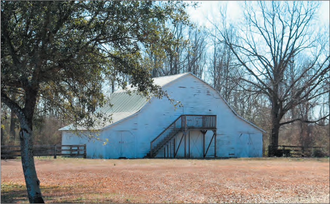
B. Center-aisle barn, Looking Southwest
