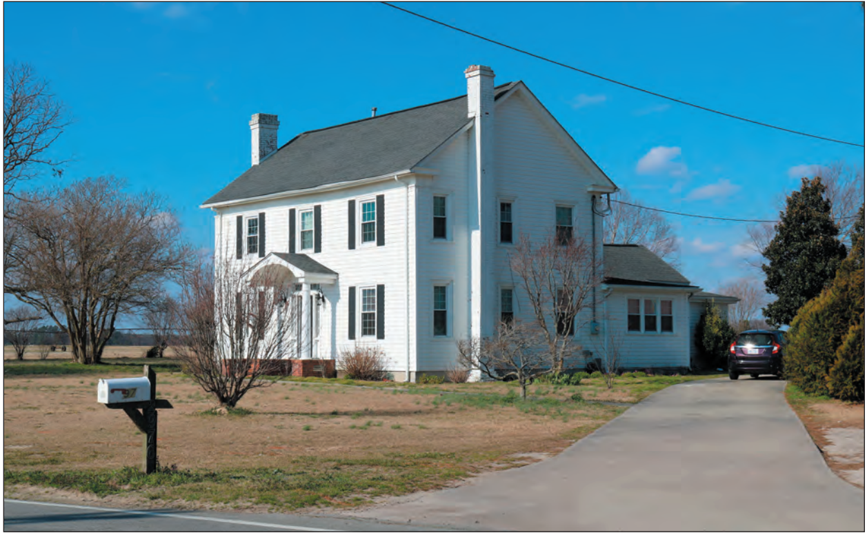
A. Main Dwelling, Looking Northwest
