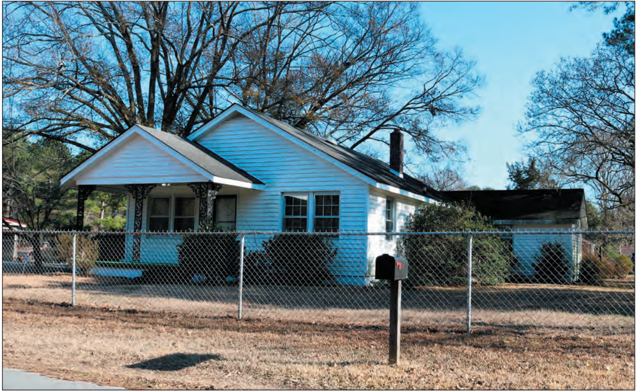
A. Looking Southeast
