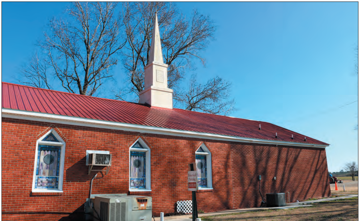
B. Vestibule Addition, Looking Southeast
