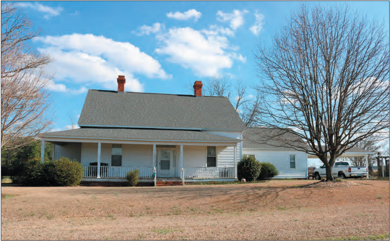
A. Looking East
