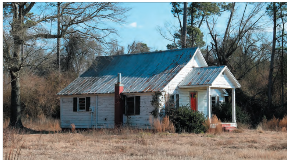
B. 201 Ryan Lane, Looking Northeast
