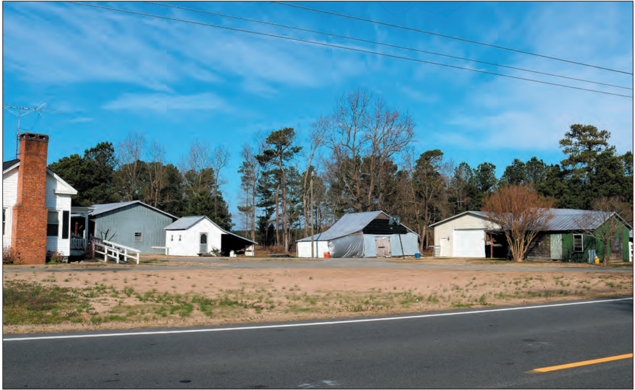
Figure 44. Photograph of Resource SP0766, Outbuildings, Looking Northwest
