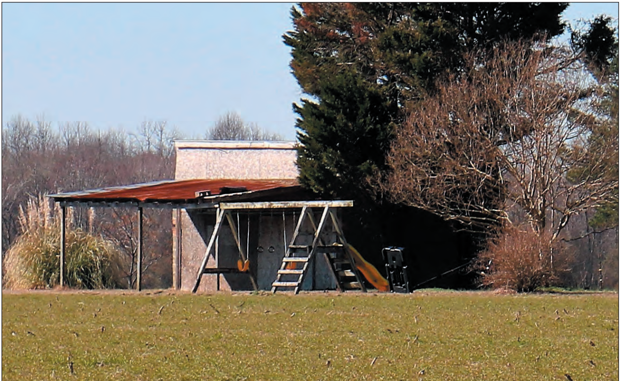
B. Outbuildings, Looking Northwest
