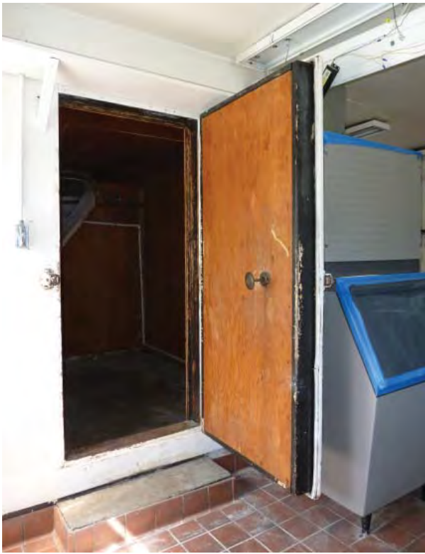
Figure C226. Doorway to walk-in cooler (Room 105B).
