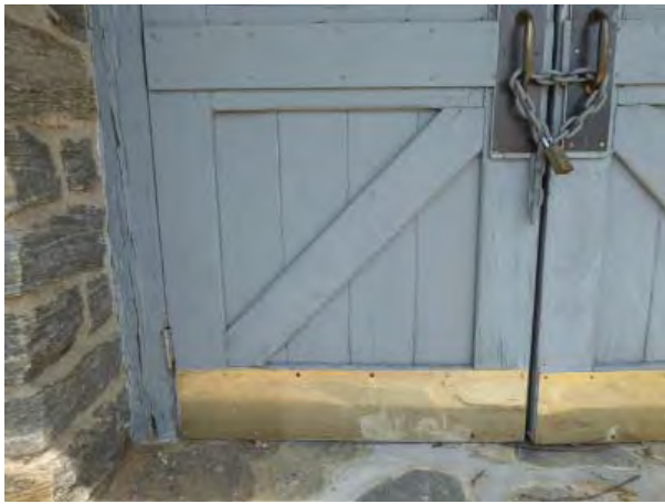
Figure C80. Detail of panels. Note added plywood at lock rails and handles.
