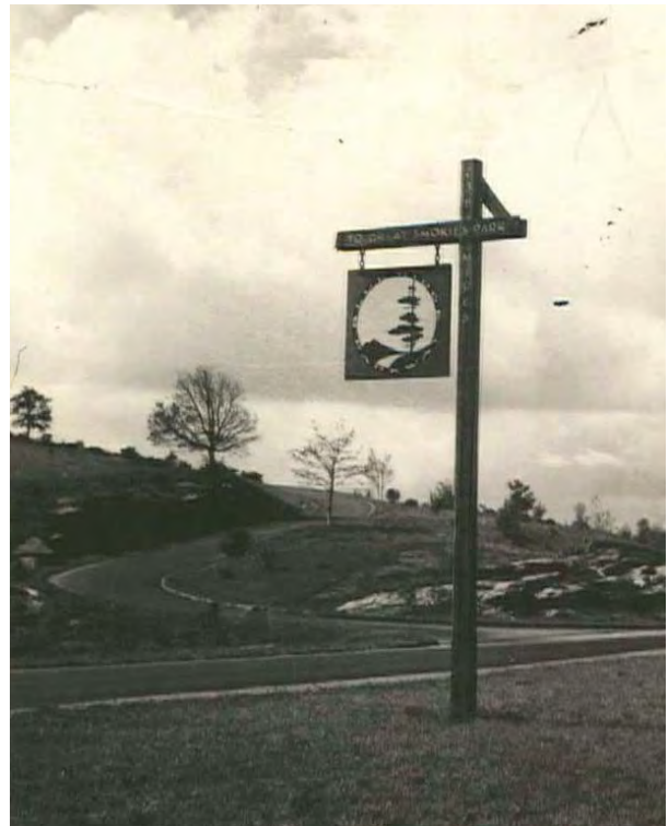
Figure A4. Undated photo of completed access road to Wildcat Rocks Overlook. Photograph taken from the grass median between the Parkway and future coffee shop. (BLRI Coll.)
