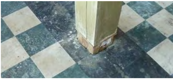
Figure C184. Concrete plinth at base of structural post.
