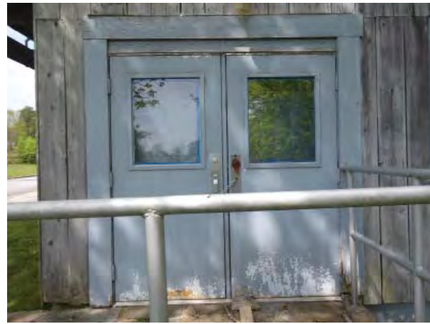
Figure C89. Replacement steel doors in added doorway on east elevation.
