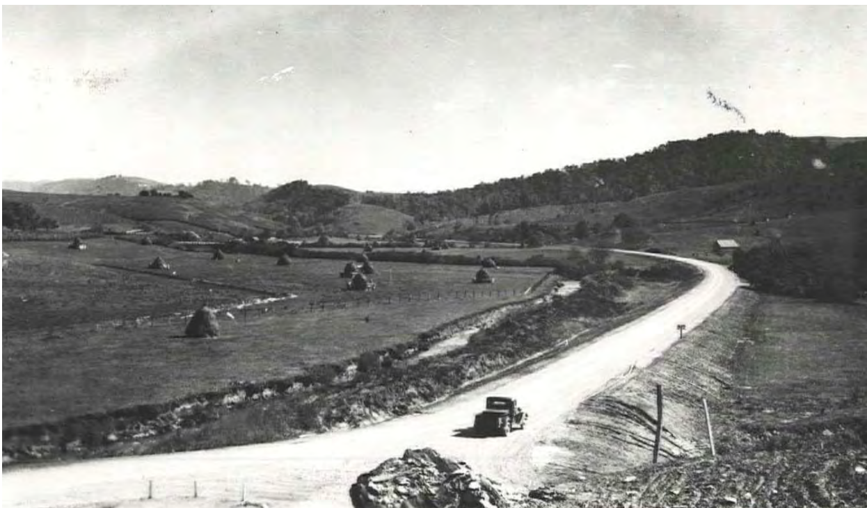
Figure A2. View of Parkway under construction at milepost 240, October 1937. (BLRI Coll.)
