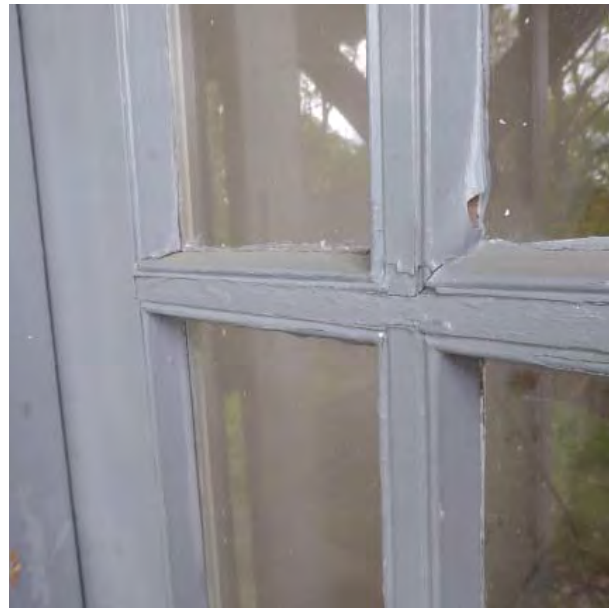
Figure C85. Detail of typical nine-light sash door muntins.
