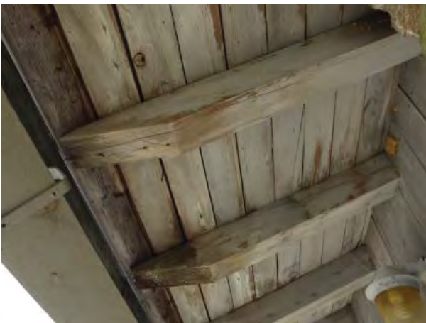
Figure C31. Typical roof decking at eave.
