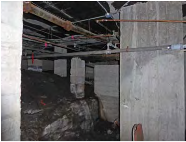
Figure C130. Room 000 looking southwest.
