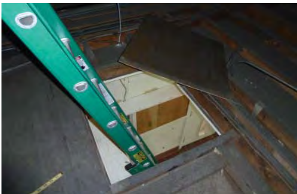
Figure C243. Hatch accessing attic from Room 105A.
