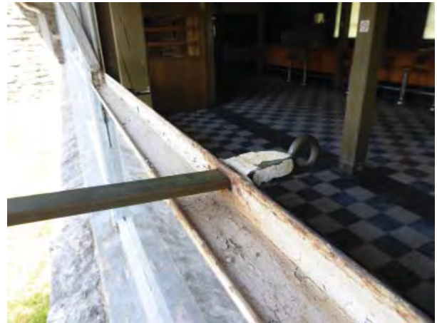
Figure C71. Typical prop-type awning operator.
