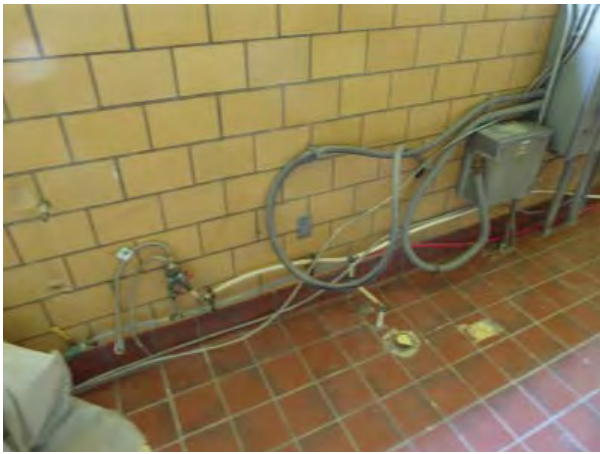
Figure C213. Terra cotta tile floor, base tile, and salt-glazed tile wainscoting.
