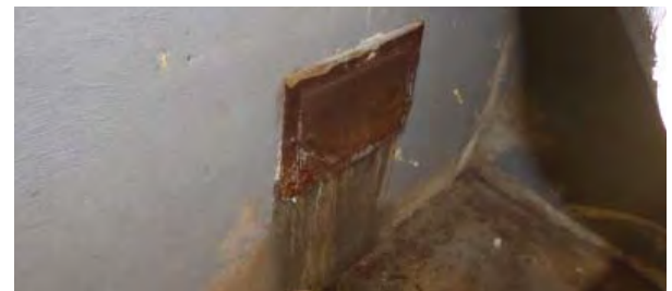
Figure C161. Chimney cleanout on east wall.
