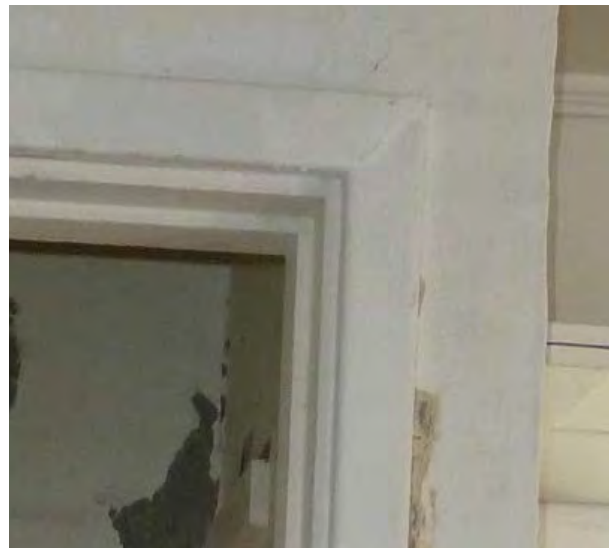
Figure C125. Typical rounded-corner door casing.
