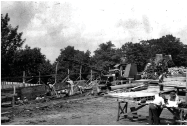
Figure B4. The coffee shop under construction in September 1948, looking northeast. Photograph by Construction photos by Superintendent Weems. (BLRI Coll.)
