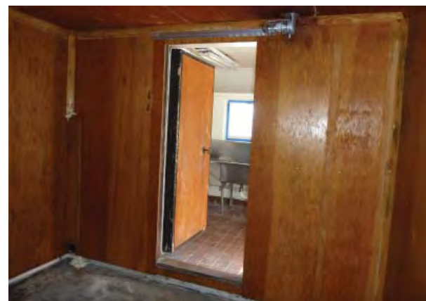
Figure C230. Room 105B - Oblique view looking southeast.
