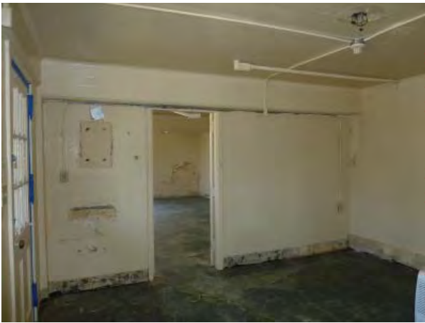
Figure C142. Room 002 - Oblique view looking southeast.
