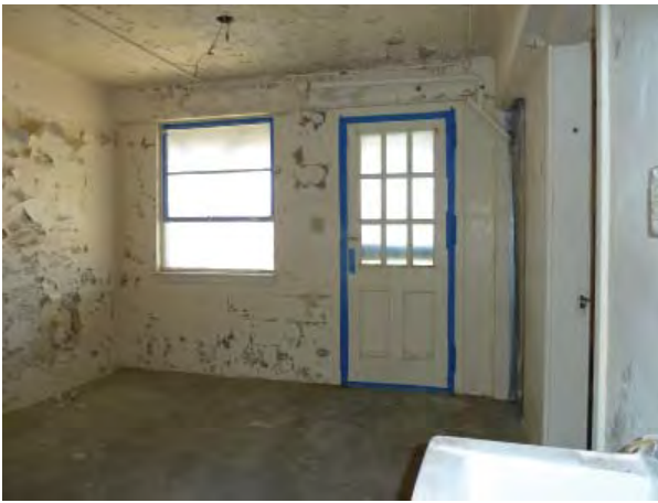
Figure C146. Room 004 - View looking north.
