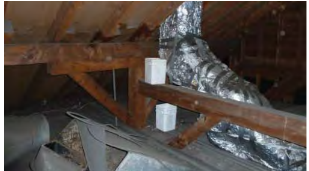
Figure C28. Timber frame extending into attic above Room 102.
