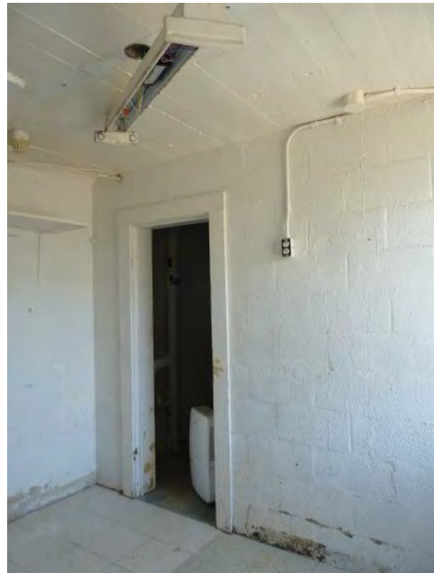
Figure C174. Room 010 - Oblique view looking southwest.
