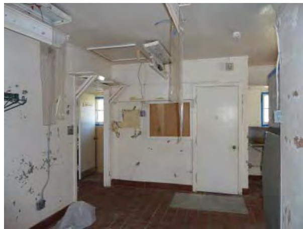
Figure C224. Room 105A - Oblique view looking southeast.
