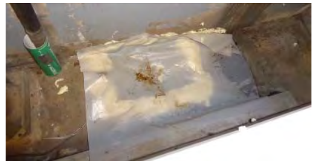
Figure C160. Floor drain along east wall, obscured by plastic.
