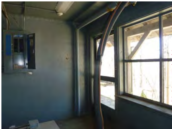
Figure C162. Room 007 - Oblique view looking northwest.
