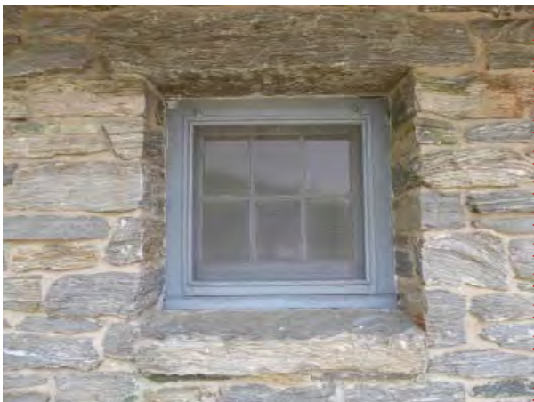
Figure C74. Typical six-light hopper-sash window.
