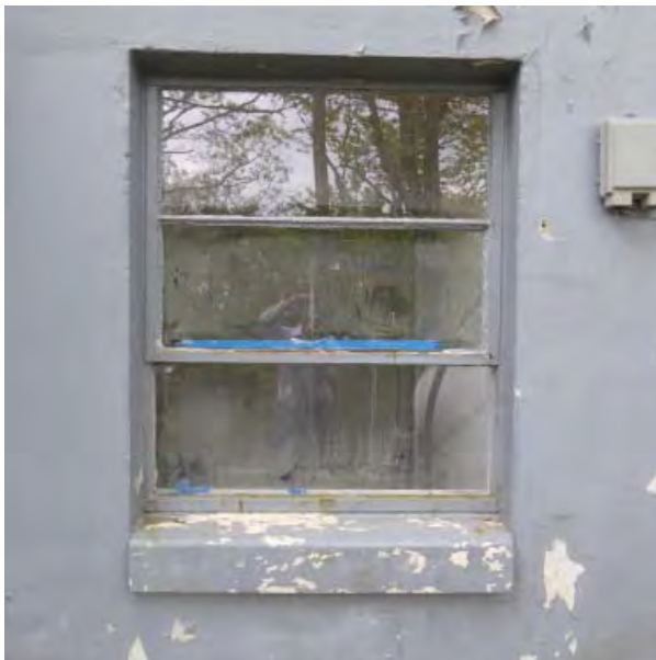
Figure C77. Typical two-over-one light awning-sash basement window.
