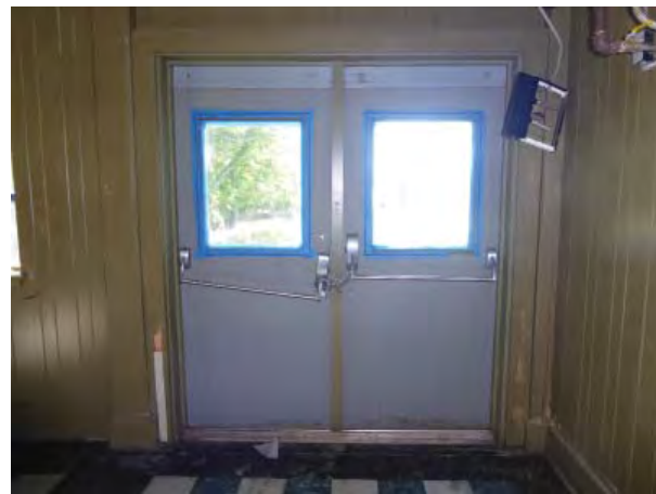
Figure C189. Interior view of east doorway.
