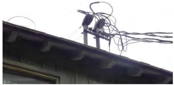
Figure C37. Weatherheads on north roof slope.
