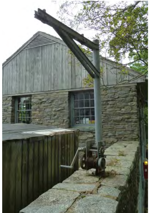
Figure C9. Hand-operated winch on north retaining wall.
