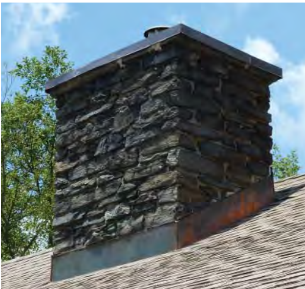
Figure C106. Exterior view of chimney. Note metal coping and copper flashing.
