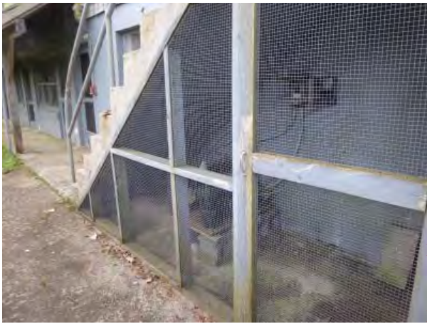
Figure C97. Screened area beneath exterior stair.
