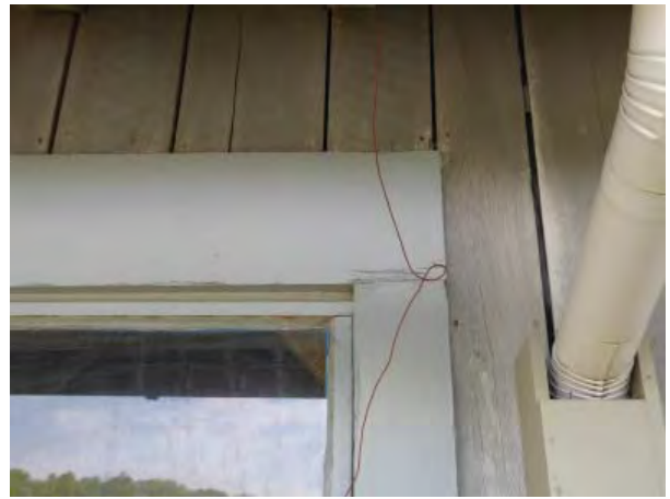
Figure C70. Plank board casing on ribbon window opening.
