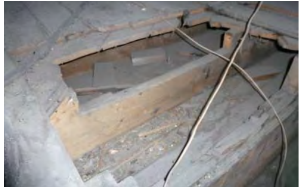
Figure C29. Roof framing above Room 102.
