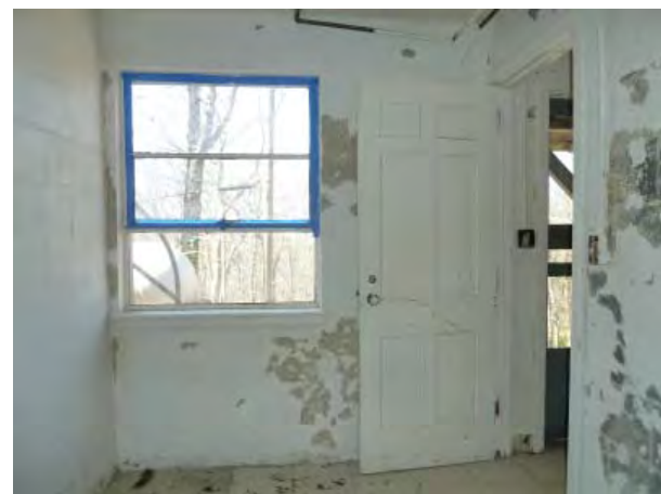
Figure C175. Room 010 - View looking north.
