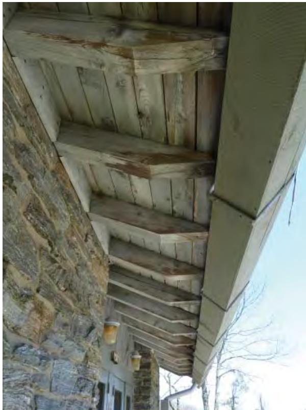
Figure C102. Exposed rafter tails and decking on south elevation.
