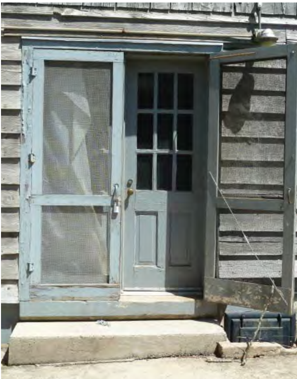
Figure C84. Overview of west doorway.
