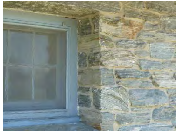
Figure C20. Stone exterior wall on south elevation, note depth at window opening.
