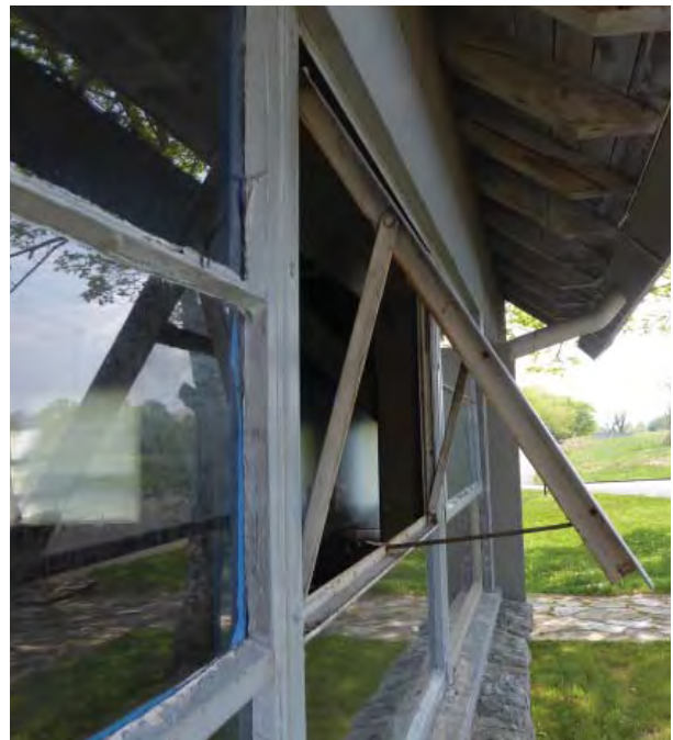
Figure C72. Detail of awning hinge and profile of sash frame.
