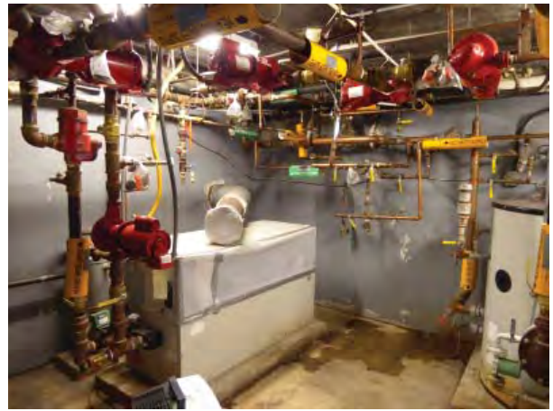
Figure C153. Room 006 - Oblique view looking southeast.
