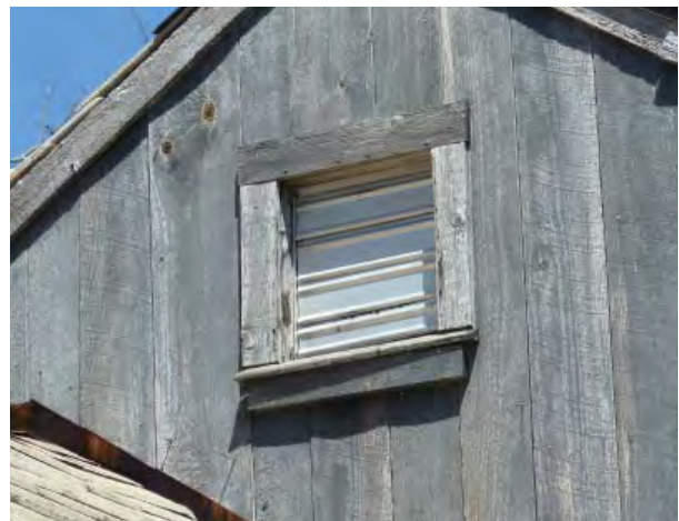
Figure C109. Metal louvered vent on west gable end of main body.
