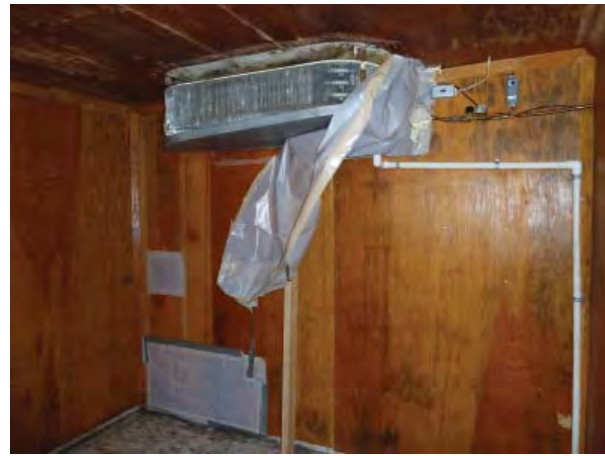
Figure C229. Room 105B - Oblique view looking northwest.
