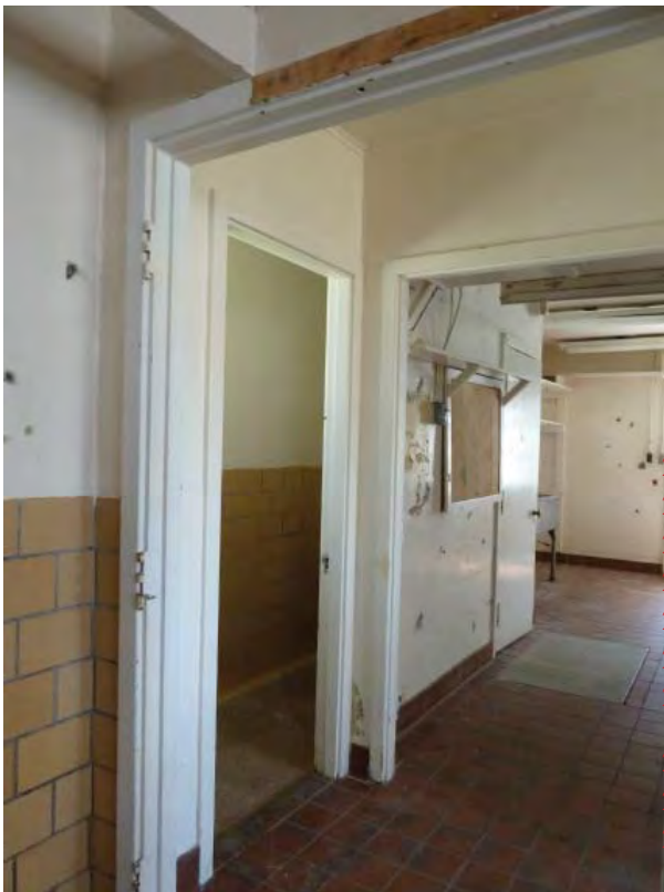
Figure C214. Doorway on west wall. Note remaining partial hinges.
