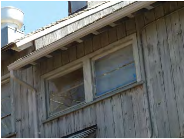
Figure C73. Paired two-light awning sash at west end of north elevation.
