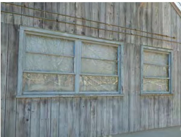
Figure C65. Examples of two-over-one-light awnings-sash windows on east elevation.
