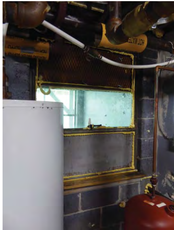
Figure C156. Window on north wall.
