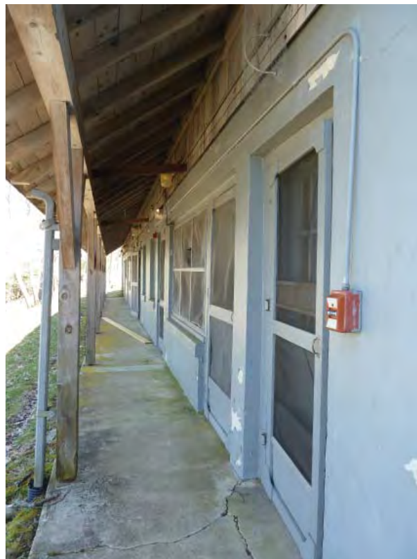
Figure C95. Concrete walkway along north elevation.
