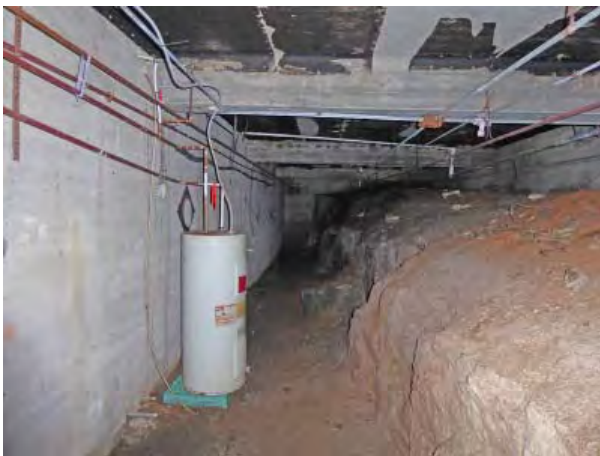
Figure C131. Room 000 looking east.
