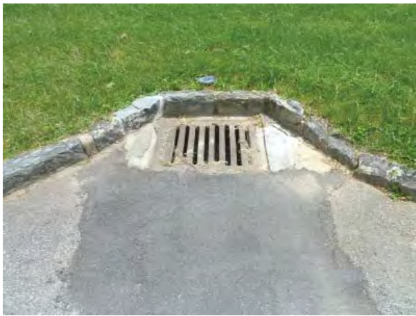
Figure C5. Storm water collection basin, note asphalt patch from recent drainage repair.
