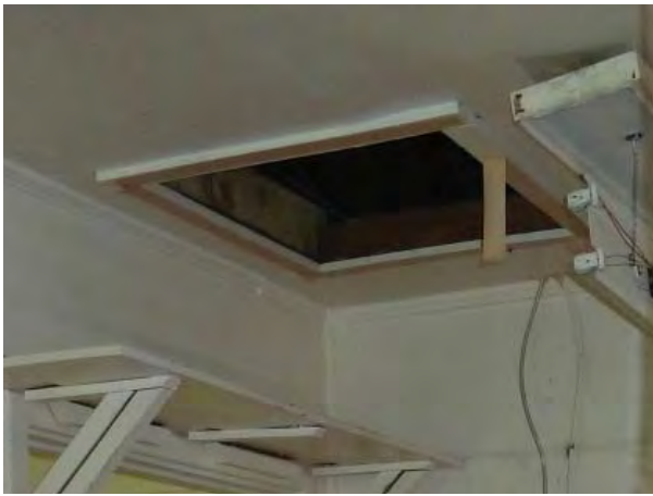
Figure C228. Attic access hatch in southeast corner of Room 105A.
