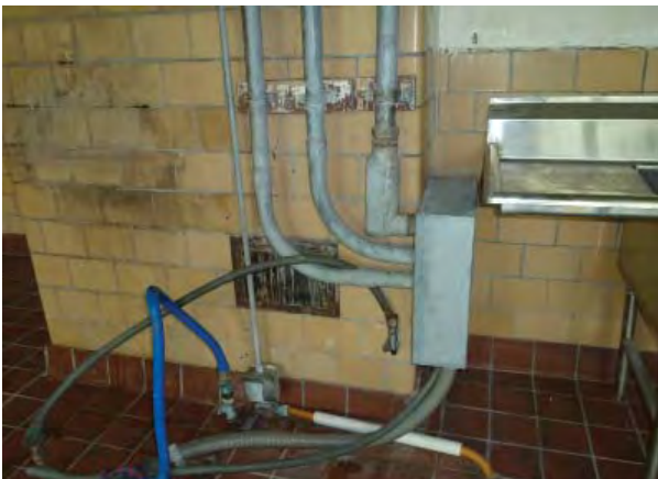
Figure C217. Electrical box and cleanout on north face of chimney.
