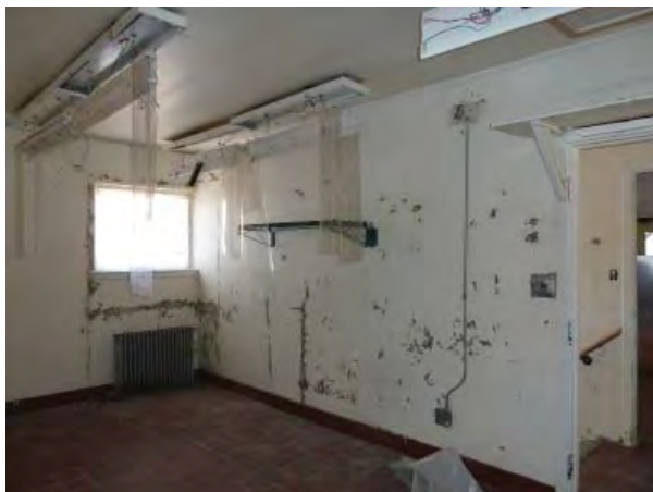
Figure C223. Room 105A - Oblique view looking northeast.
