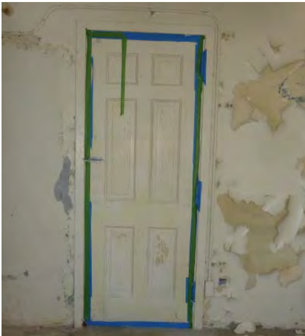
Figure C132. Doorway to crawl space viewed from Room 004.
