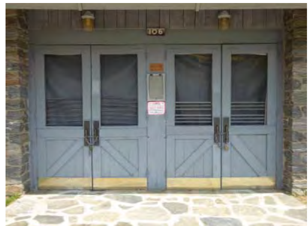
Figure C79. Overview of main entrance doorways. Note inconsistent size of lower panel at far right.
