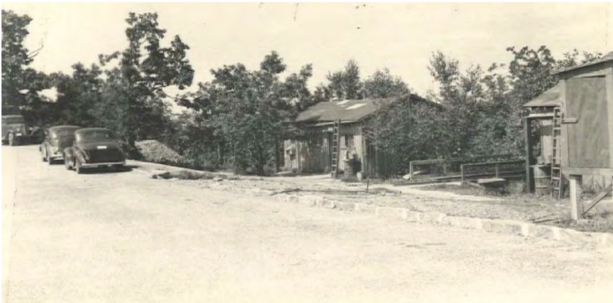
Figure A6. Work camp at future site of coffee shop and service station in 1941. Note roadway and stone curbs already in place. (BLRI Coll.)
