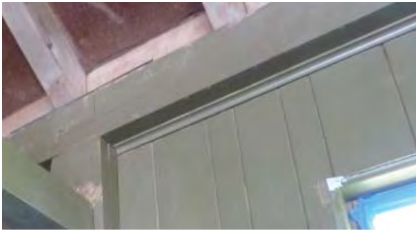
Figure C185. Typical cove molding at top of paneling.
