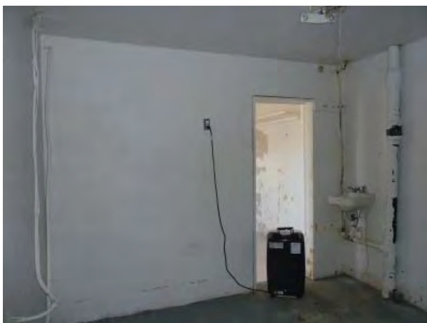
Figure C176. Room 011 - View looking east.
