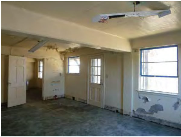
Figure C138. Room 001 - Oblique view looking northwest.
