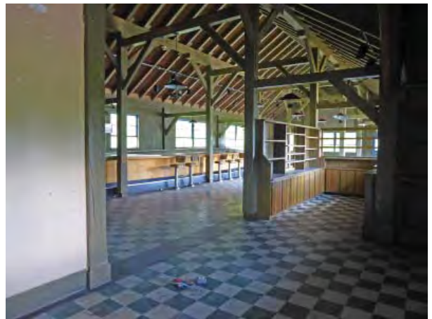
Figure C206. Room 101B - Oblique view looking northeast.
