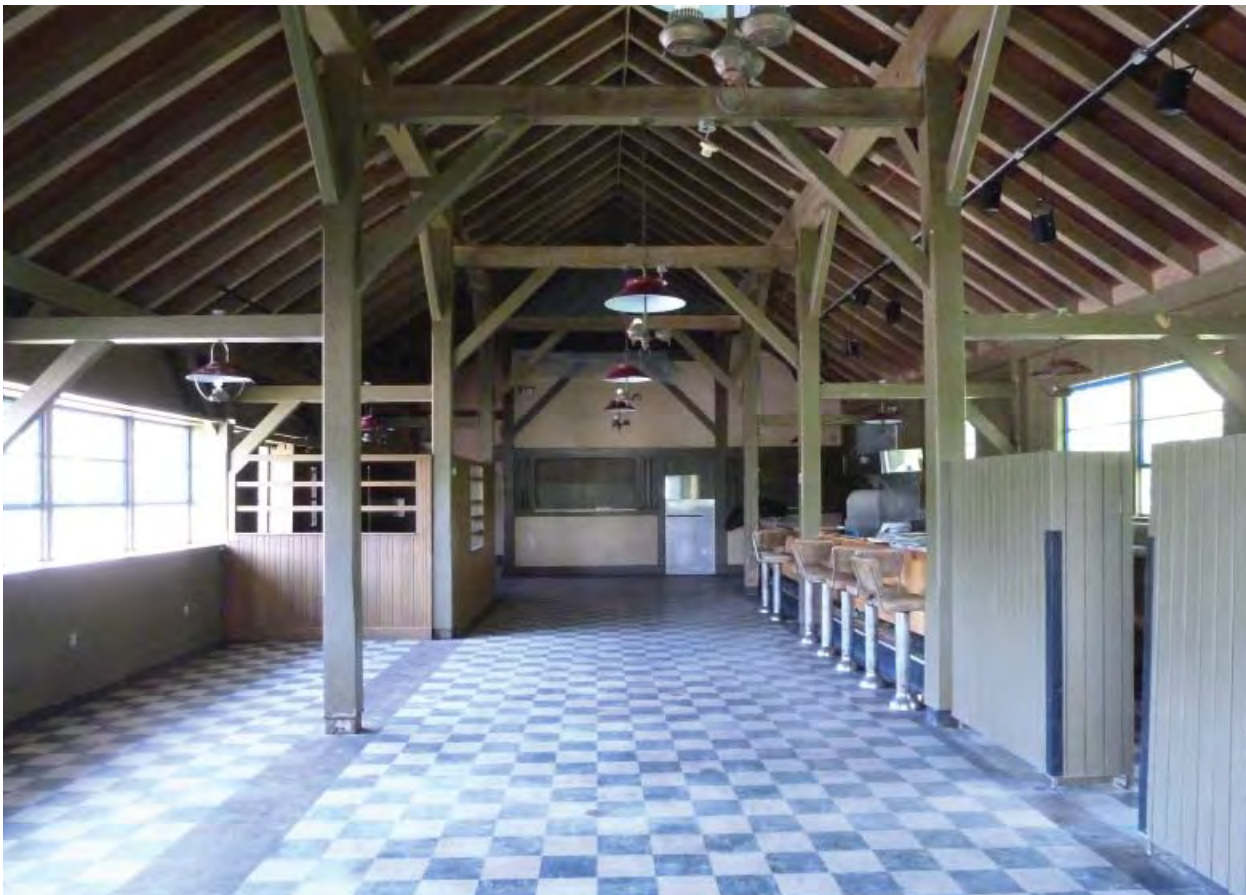
Figure C178. Room 101A - Overview looking west.
