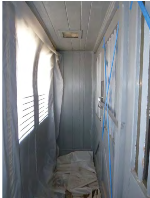
Figure C237. Room 108 - View looking west.
