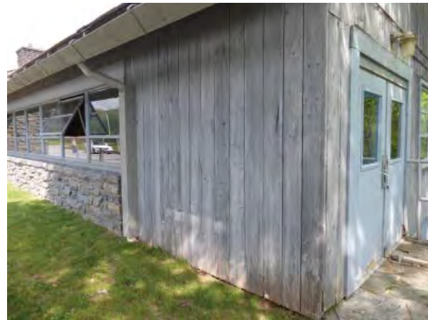
Figure C57. Vertical plank board siding at southeast corner.
