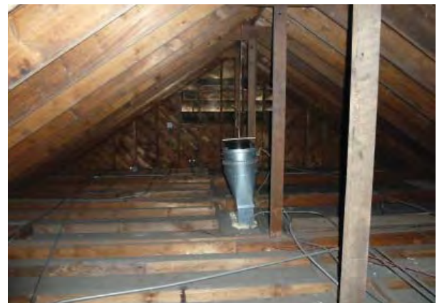
Figure C241. View of attic above west wing looking west.
