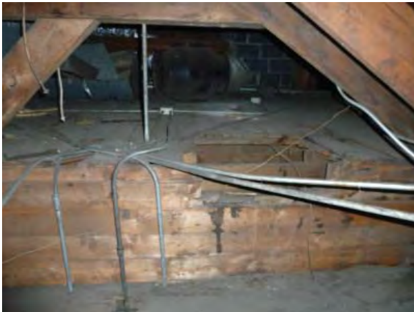
Figure C242. Tongue-and-groove flooring and ceiling height transition above kitchen.
