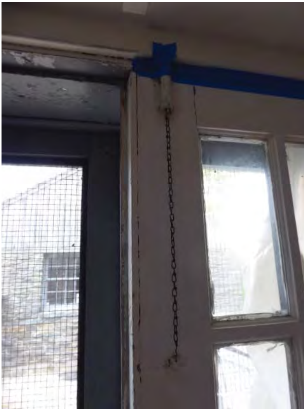
Figure C87. Likely-original interior head bolt with chain on west doorway.
