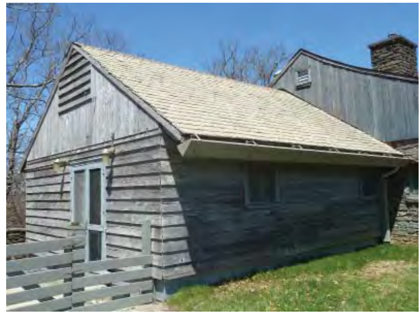
Figure C62. Horizontal weatherboard on west wing.
