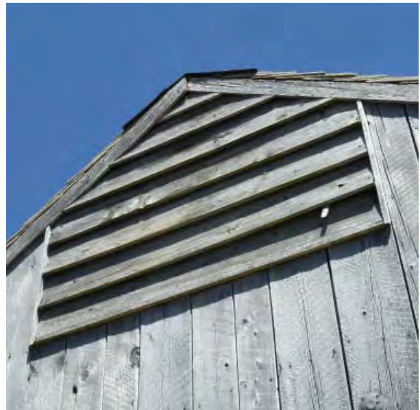
Figure C63. Louvered vent on west gable end of wing.
