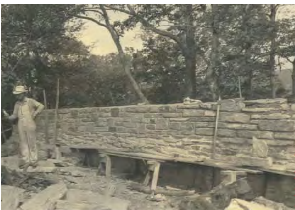
Figure A7. Construction of stone retaining wall of parking area for the Woods Picnic Area, east of future coffee shop site, July 1938. (BLRI Coll.)
