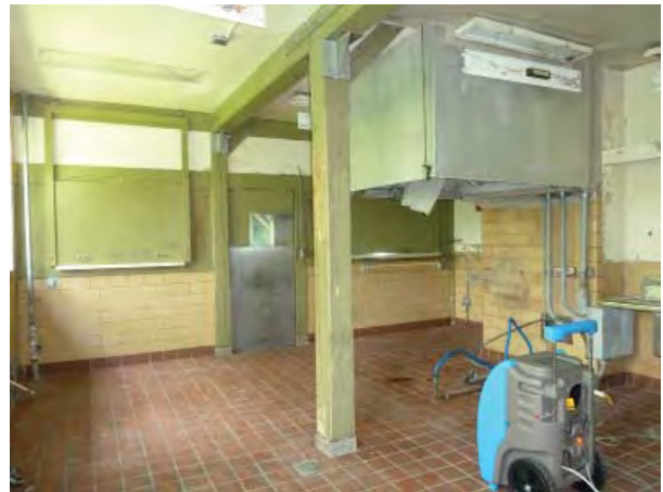
Figure C211. Room 102 - Oblique view looking southeast.
