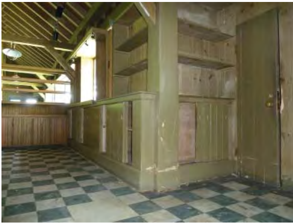
Figure C193. Original casework on south wall in gift shop area.
