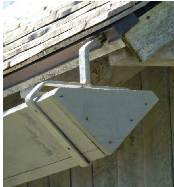
Figure C113. Original smaller gutter design on east end of south elevation.
