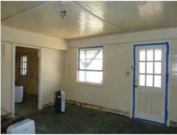
Figure C141. Room 002 - Oblique view looking northwest.
