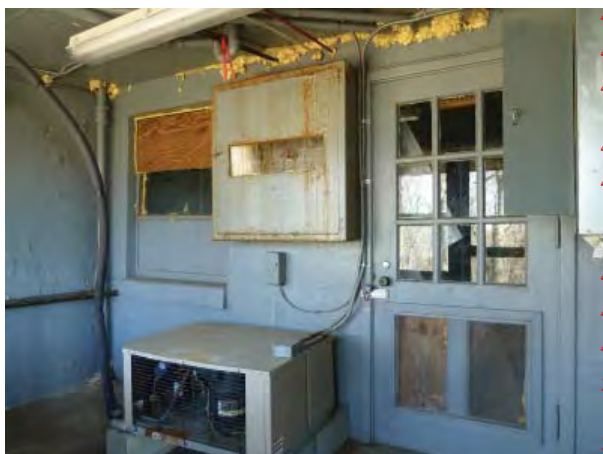
Figure C163. Room 007 - Oblique view looking southeast
