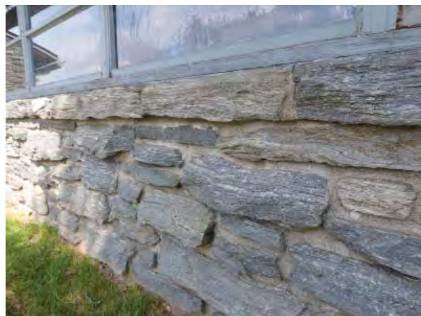
Figure C67. Projecting stone stubsill below south ribbon windows.
