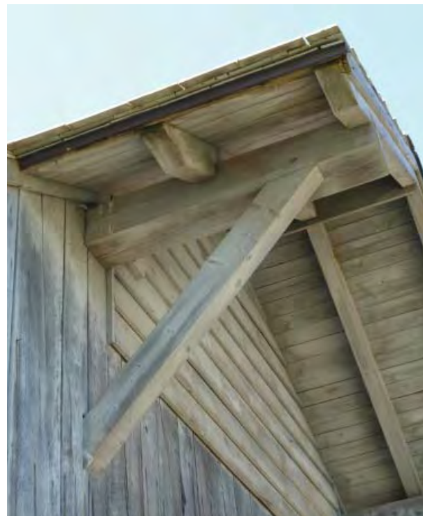
Figure C104. Detail of hood on east elevation.
