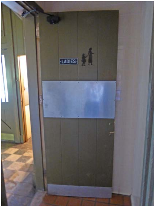
Figure C231. Room 106A - View looking south.
