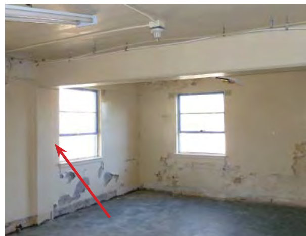
Figure C17. Engaged concrete column (left) and concrete beam in Room 001.
