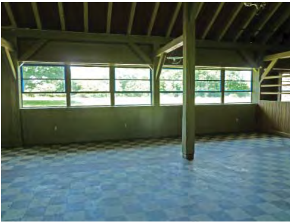
Figure C190. South ribbon windows viewed from interior.
