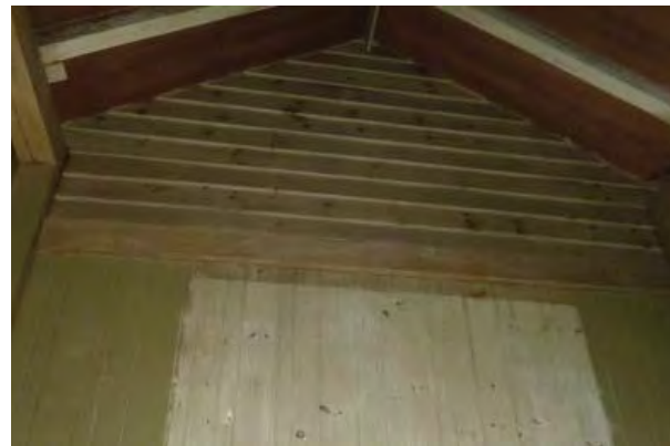
Figure C188. Weatherboard gable on east wall.
