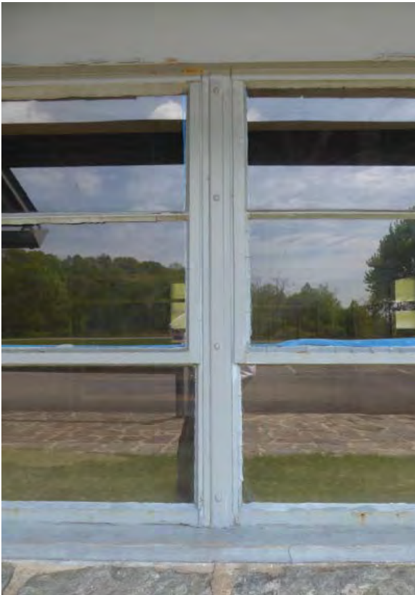
Figure C69. Typical window mullion.
