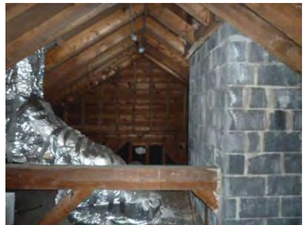
Figure C240. View of attic looking east.
