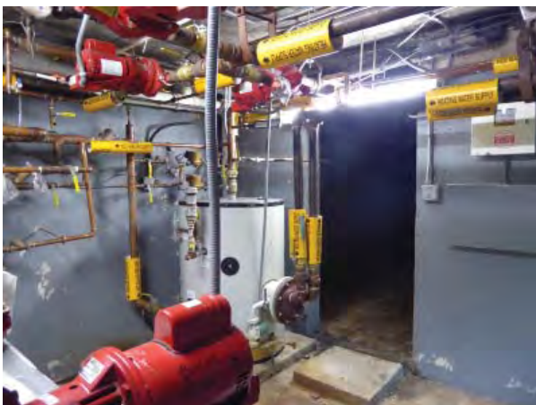
Figure C152. Room 006 - Oblique view looking southwest.
