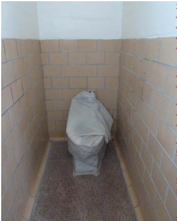
Figure C222. Room 104 - View looking west.
