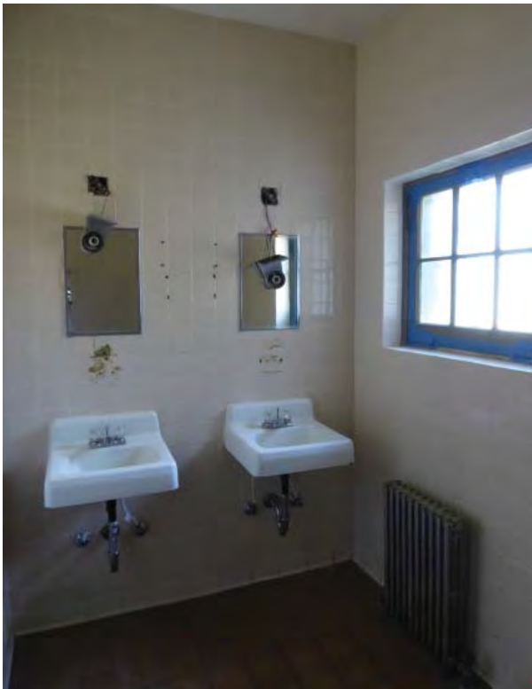
Figure C232. Room 106B - Oblique view looking southwest.
