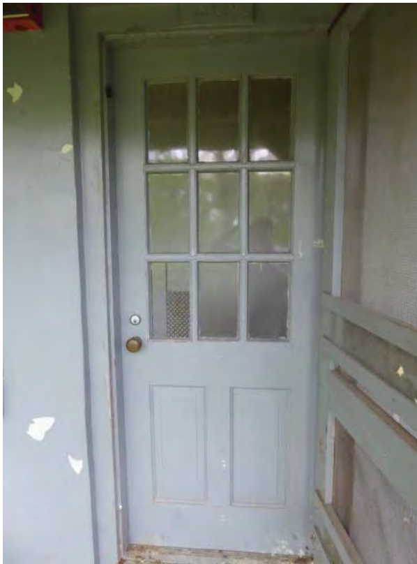
Figure C90. Typical exterior door at basement level.
