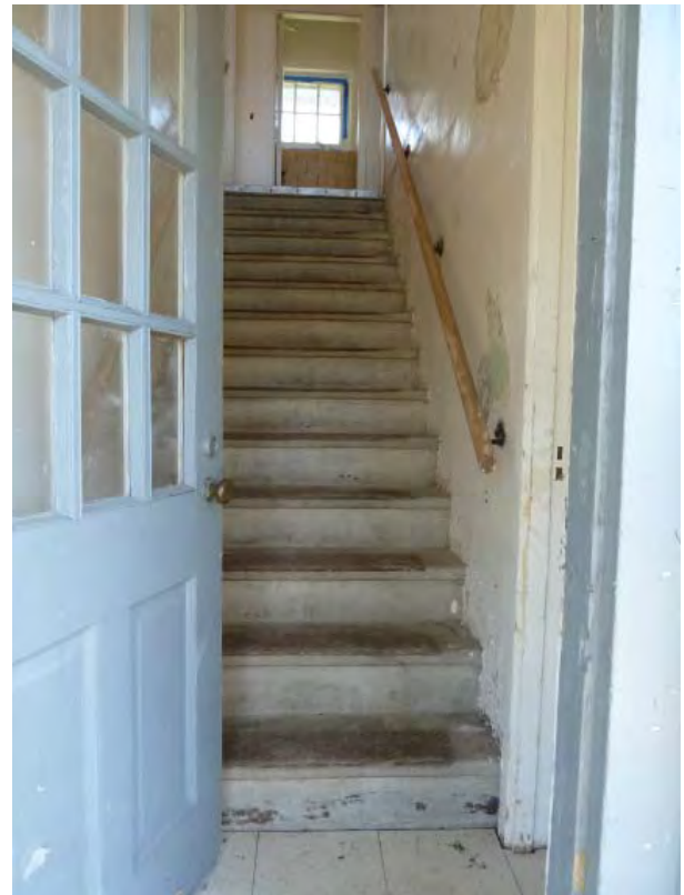
Figure C172. Stair to main level.
