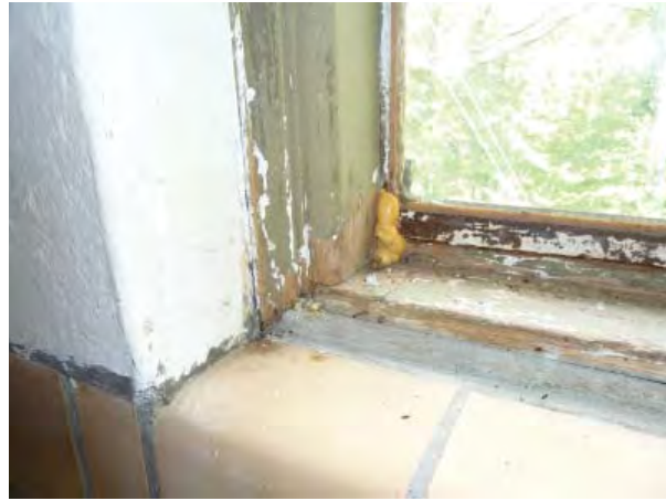
Figure C215. Detail of window and sill in Room 102.
