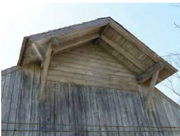
Figure C103. Projecting hood on east elevation.
