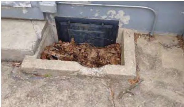
Figure C119. One of two coal hatches on west elevation.
