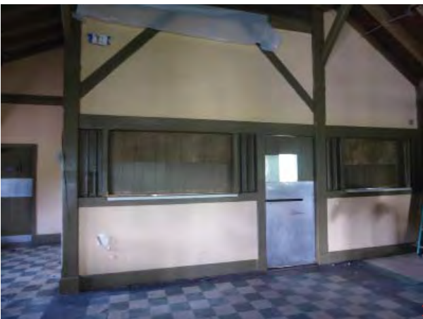
Figure C186. Plaster finish on west wall.
