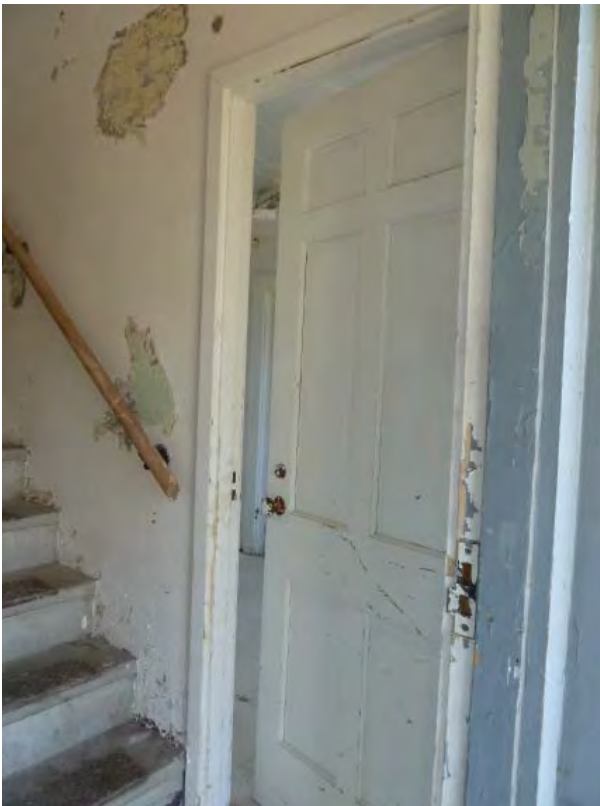
Figure C171. Doorway in west wall accessing Room 010.
