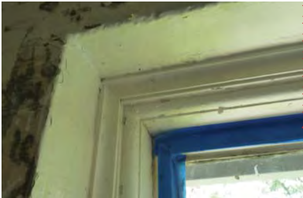
Figure C127. Trim at typical window opening in masonry wall.
