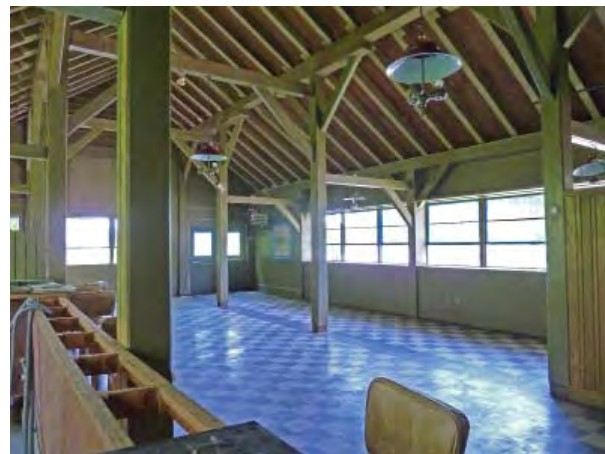
Figure C180. Room 101A - Oblique view looking southeast.
