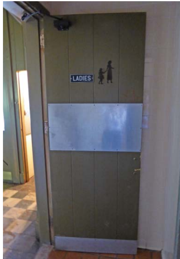
Figure C120. Typical flush-panel V-groove door.
