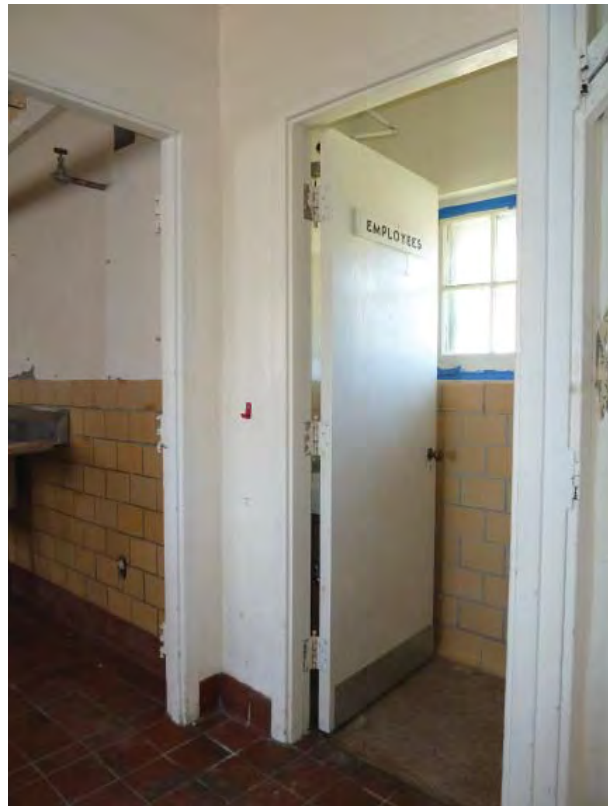
Figure C221. Room 103 - Oblique view looking southeast into Room 104.
