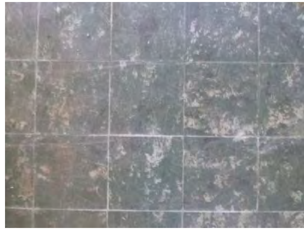
Figure C140. Typical 9x9 asphalt tile flooring.
