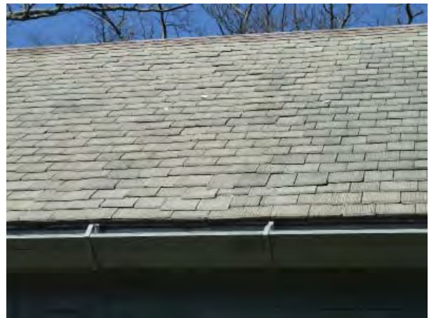
Figure C100. Cement shingle roof. Note several courses of composition shingle at ridge.
