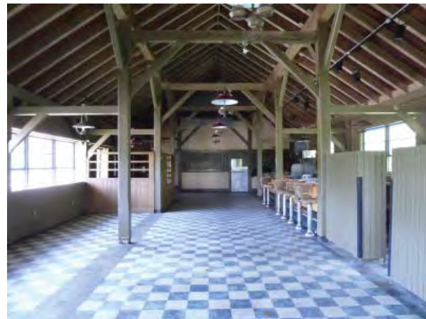
Figure C23. Overview of timber framing in Room 101A, looking west.
