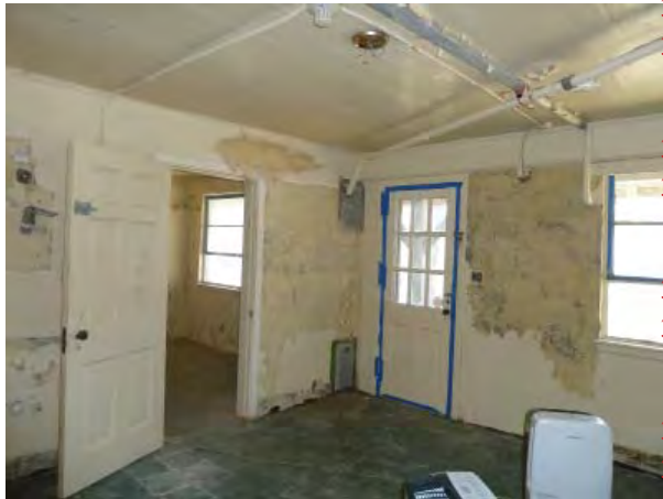
Figure C143. Room 003 - Oblique view looking northwest.
