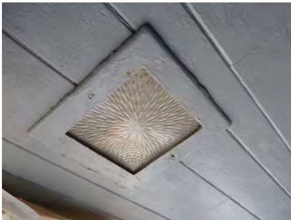
Figure C239. Original ceiling fixture in Room 108.
