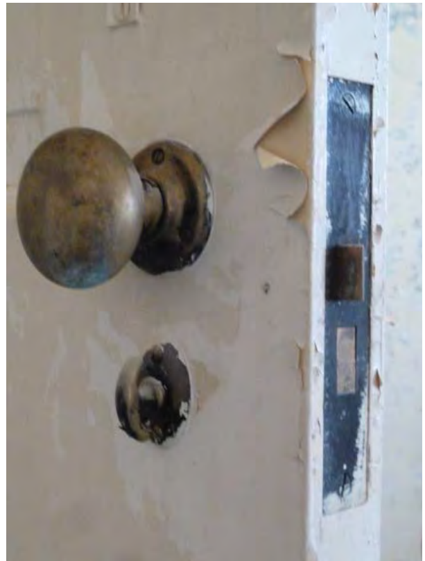
Figure C124. Example of mortised lockset with privacy lock at basement level.
