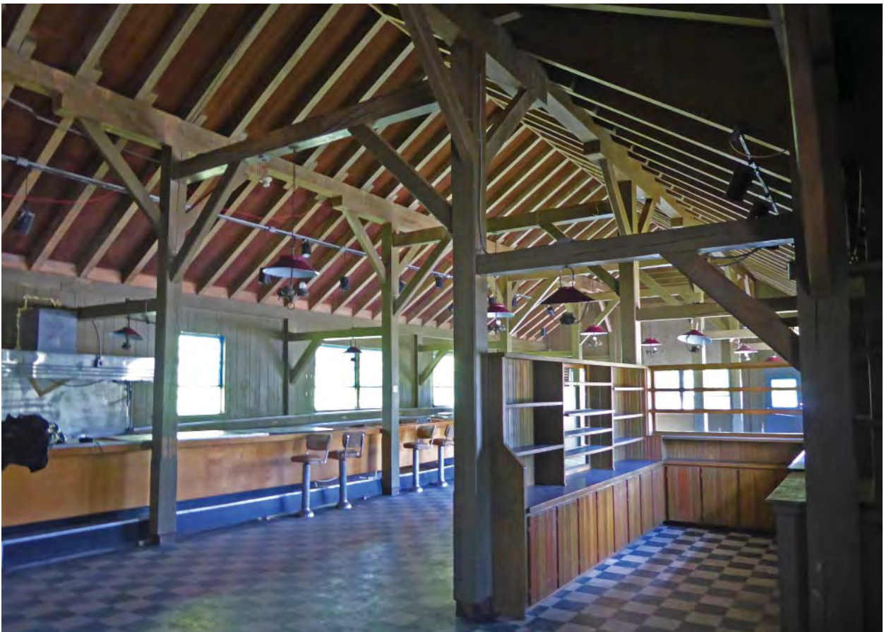
Figure C181. Room 101A - View looking northeast from entryway (Room 101B).
