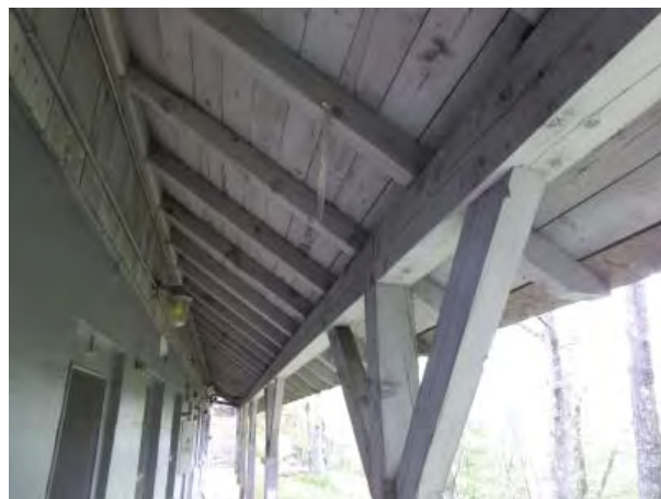
Figure C96. Porch roof framing.
