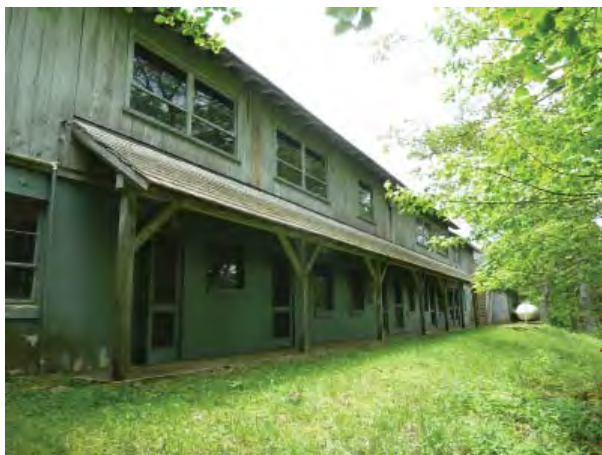
Figure C94. Shed-roofed open rear porch.
