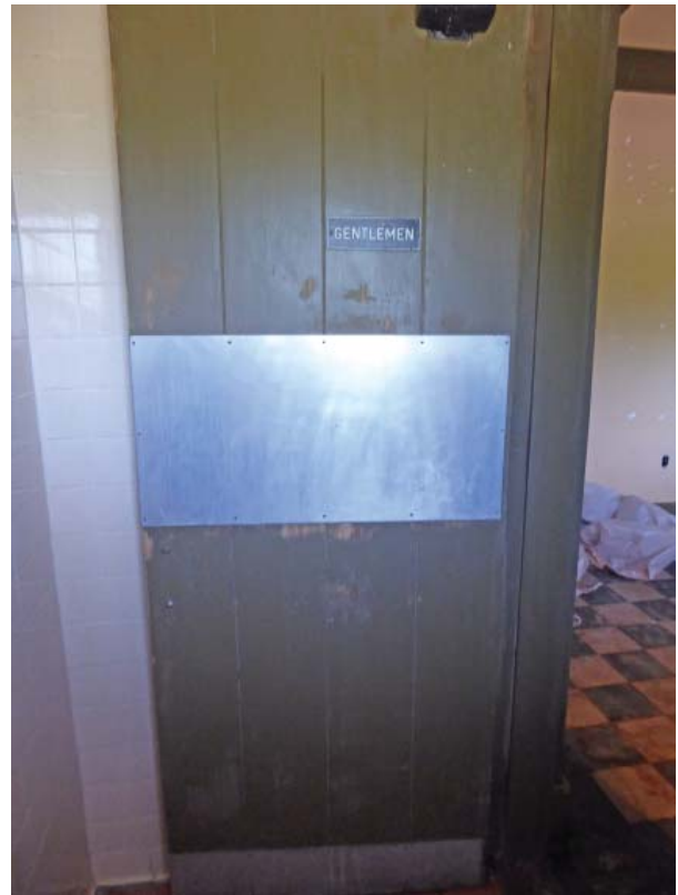
Figure C235. Room 107A - View looking north.
