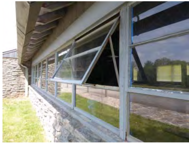
Figure C66. Ribbon windows on south elevation. Note awning sash operation.
