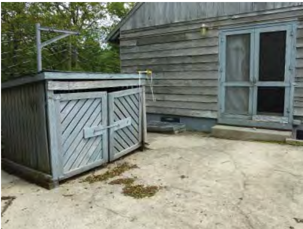
Figure C7. Service area looking northeast.
