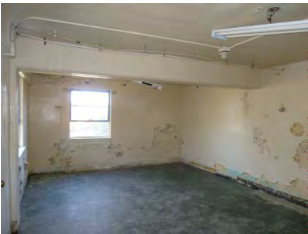
Figure C139. Room 001 - Oblique view looking southeast
