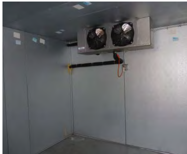
Figure C150. Interior of walk-in cooler looking southeast.
