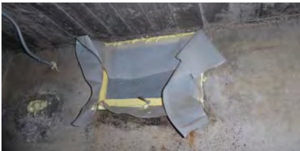
Figure C169. Secured coal door on west wall.
