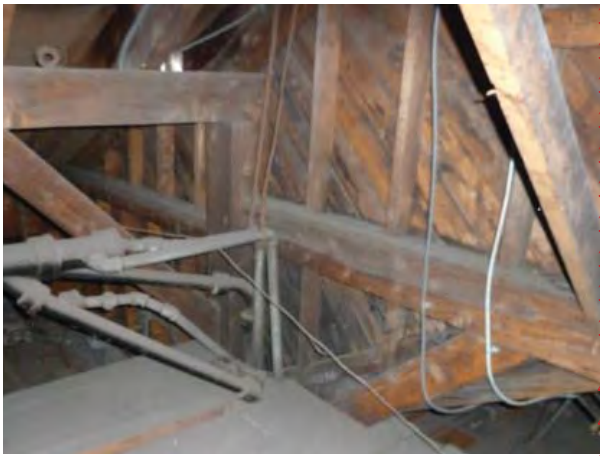
Figure C22. Exterior wall framing at west wall of extending southern bay.
