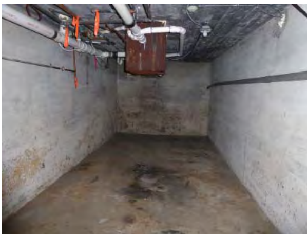
Figure C164. Room 008 - View looking west.
