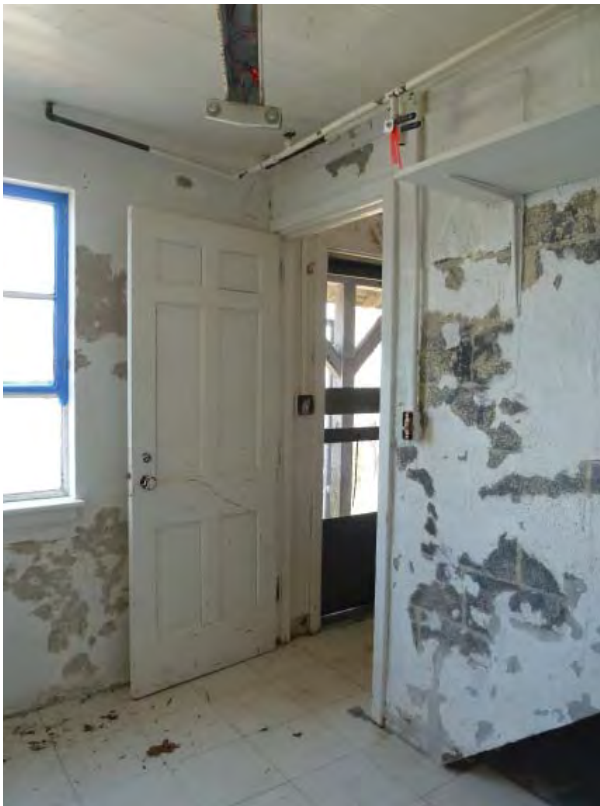
Figure C173. Room 010 - Oblique view looking northeast.
