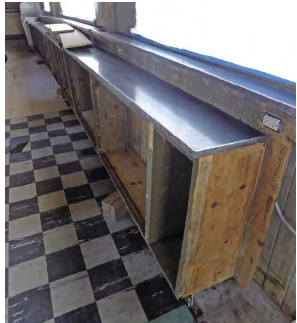
Figure C192. Rear counter. Note replacement tile.
