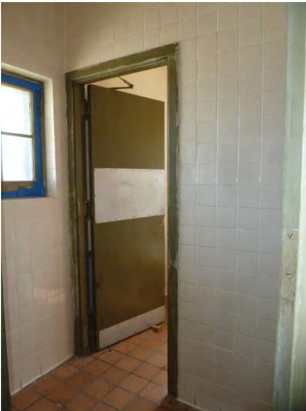
Figure C234. Room 107A - Oblique view looking southwest.
