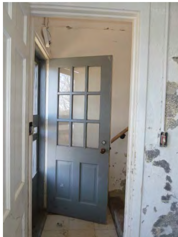
Figure C170. Room 009 - View looking east from Room 010.
