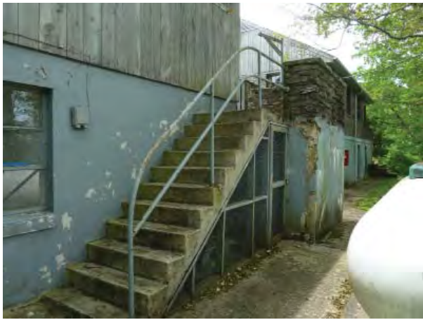
Figure C10. Concrete exterior stair.
