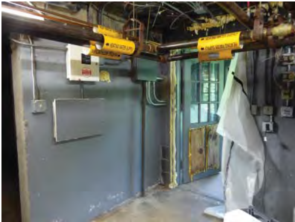
Figure C151. Room 006 - Oblique view looking northwest.
