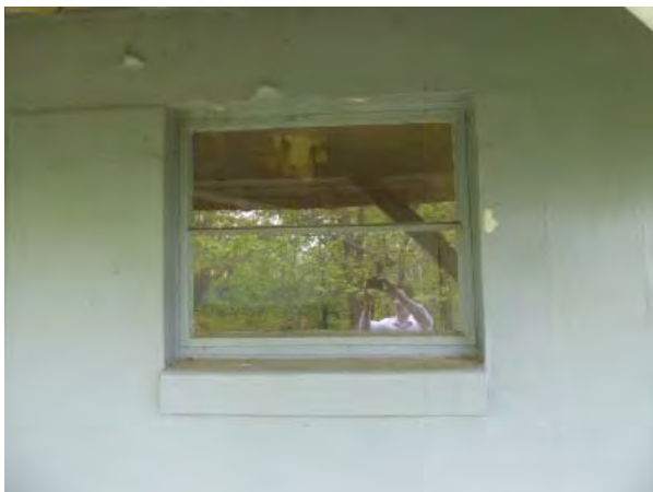
Figure C78. Two-light awning-sash basement window on north elevation.
