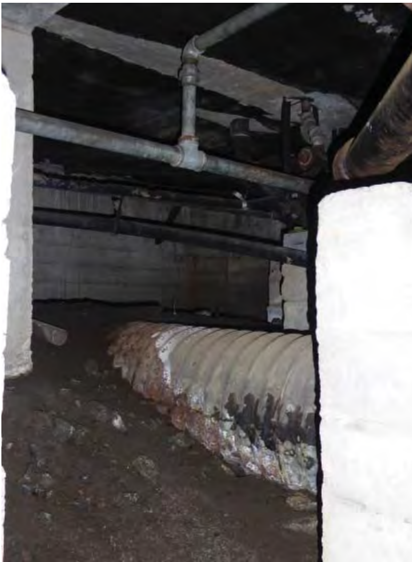
Figure C135. Corrugated storm water pipe leading to collection basin.
