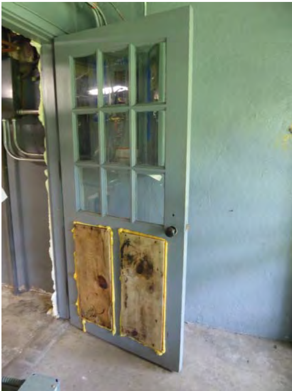
Figure C155. Nine-light sash door on north wall of Room 006.
