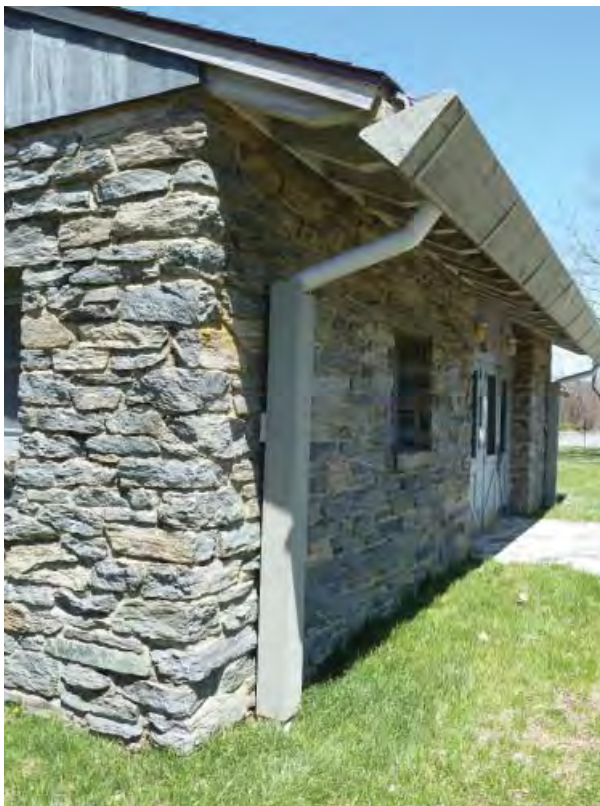
Figure C115. Typical round metal downspouts with wood wrapping on south elevation.
