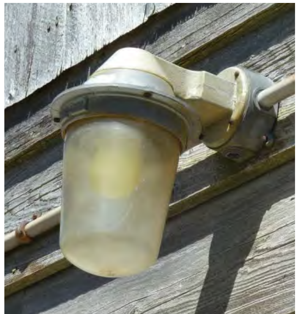
Figure C117. Typical wall-mounted replacement light fixture.
