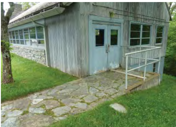
Figure C99. Ramp leading to east doorway.
