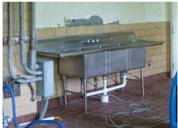
Figure C218. Stainless steel sink on south wall.
