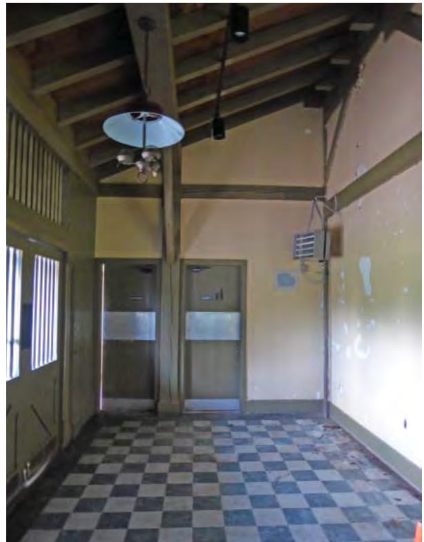
Figure C205. Room 101B - View looking west.
