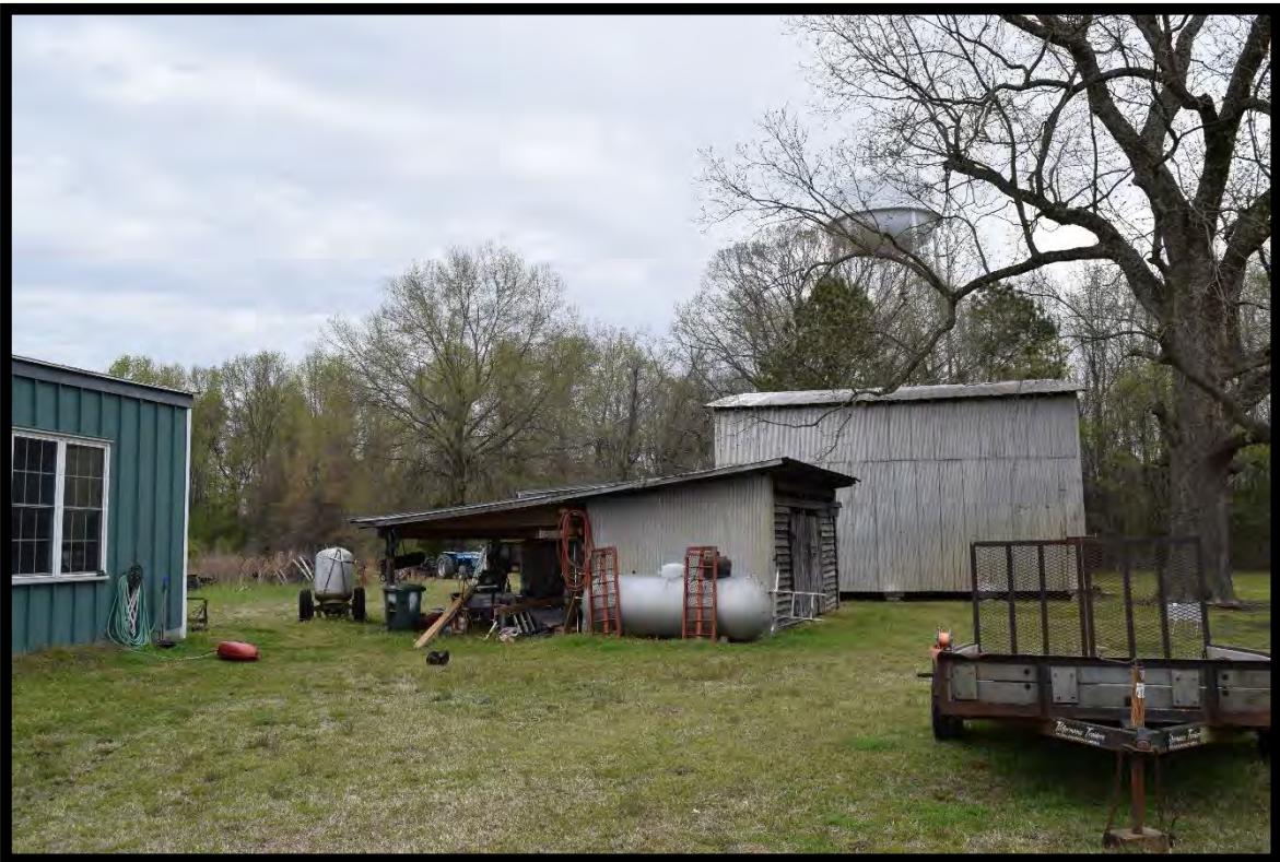
Figure 60: George Hinton House, Mule Stable, Looking East
