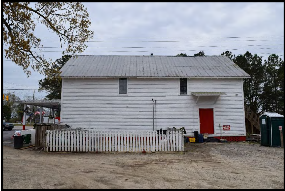
Figure 21: J. O. Barnes Store, Looking South.
