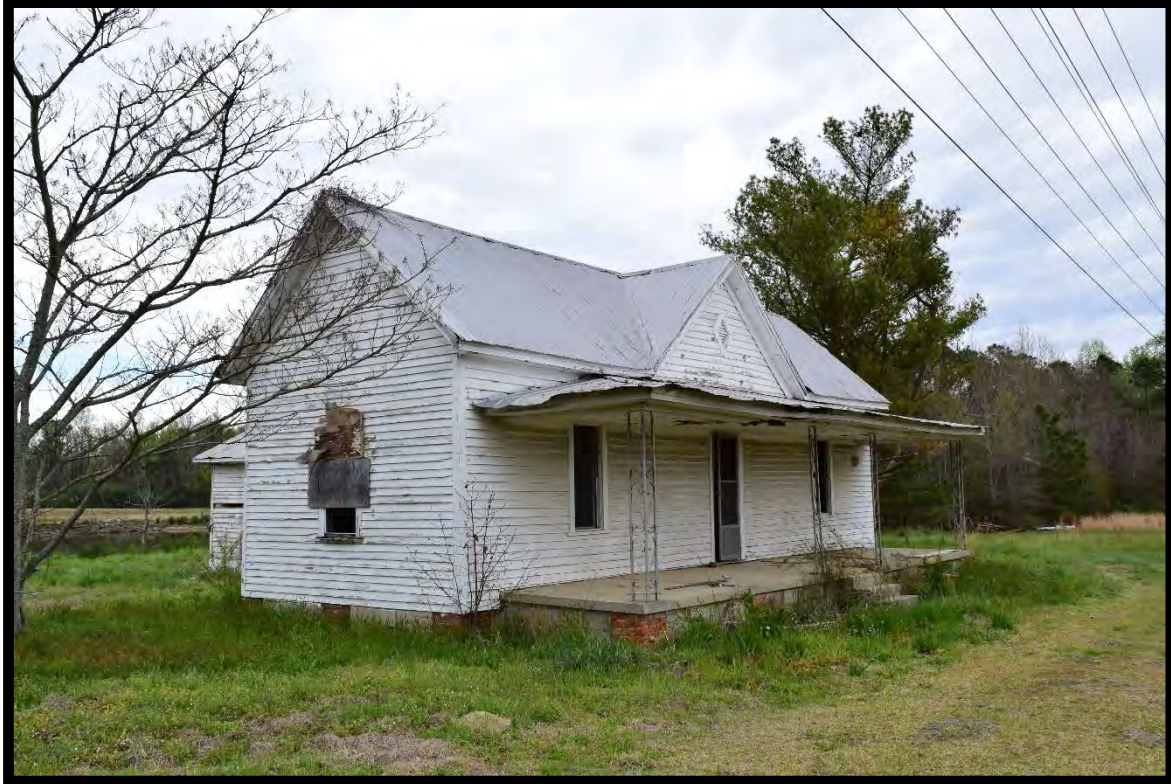
Figure 8: Barnes House, Looking Northeast.
