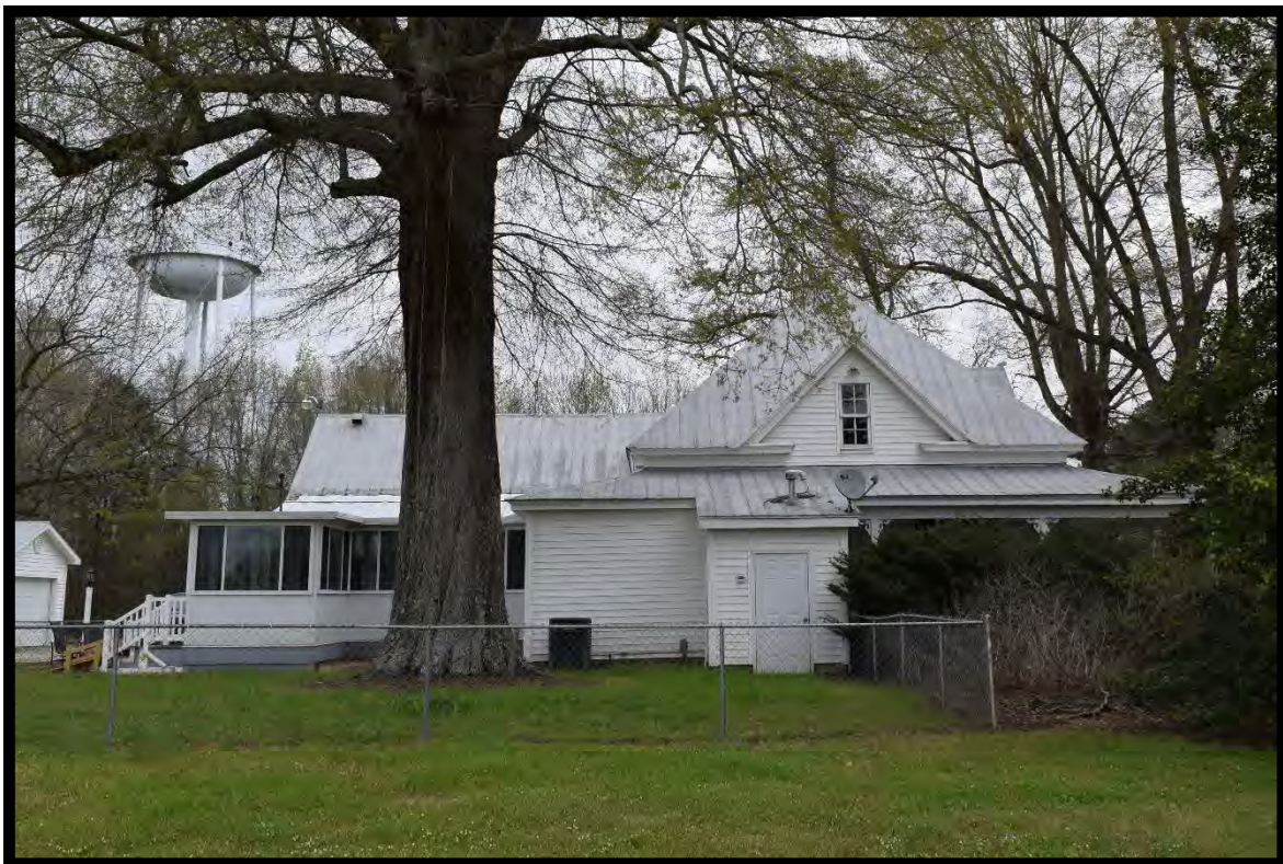
Figure 54: George Hinton House, Looking East.
