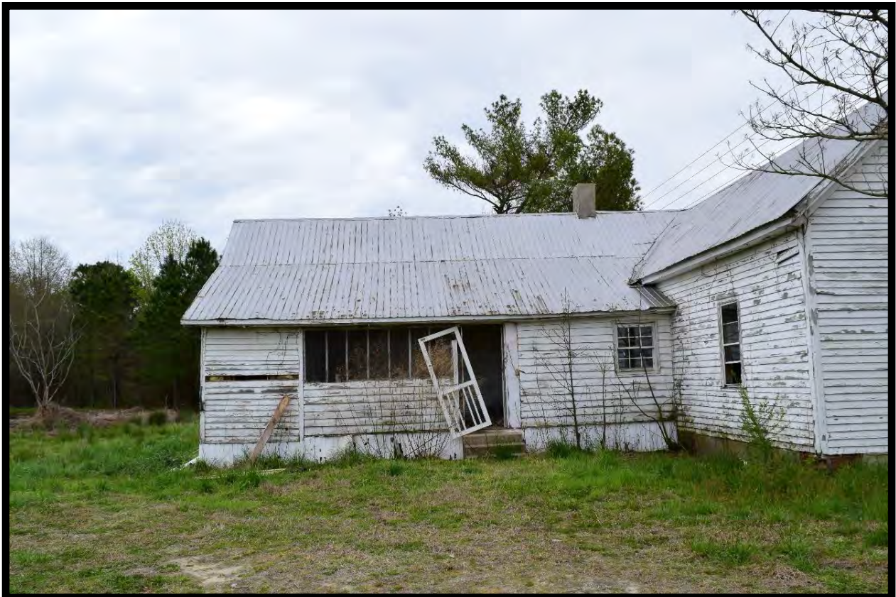
Figure 7: Barnes House, Looking East.
