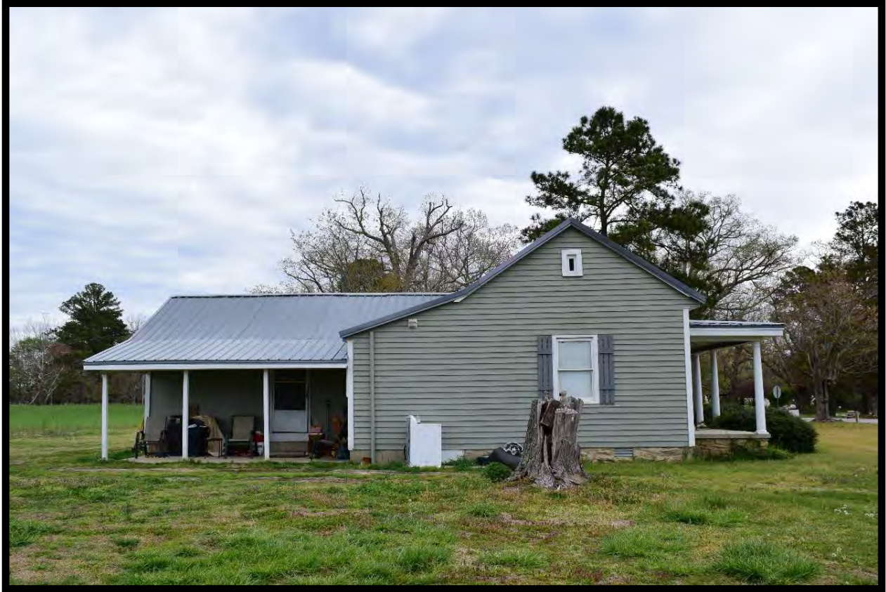
Figure 41: Wall House, Looking Northeast.
