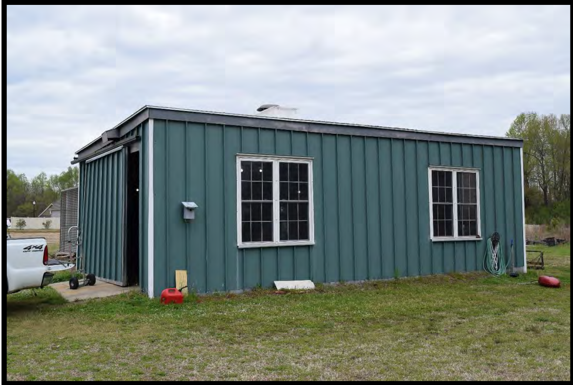
Figure 64: George Hinton House, Outbuilding, Looking North.
