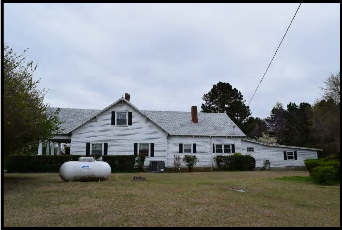
Figure 27: J. O. Barnes House, Looking South.
