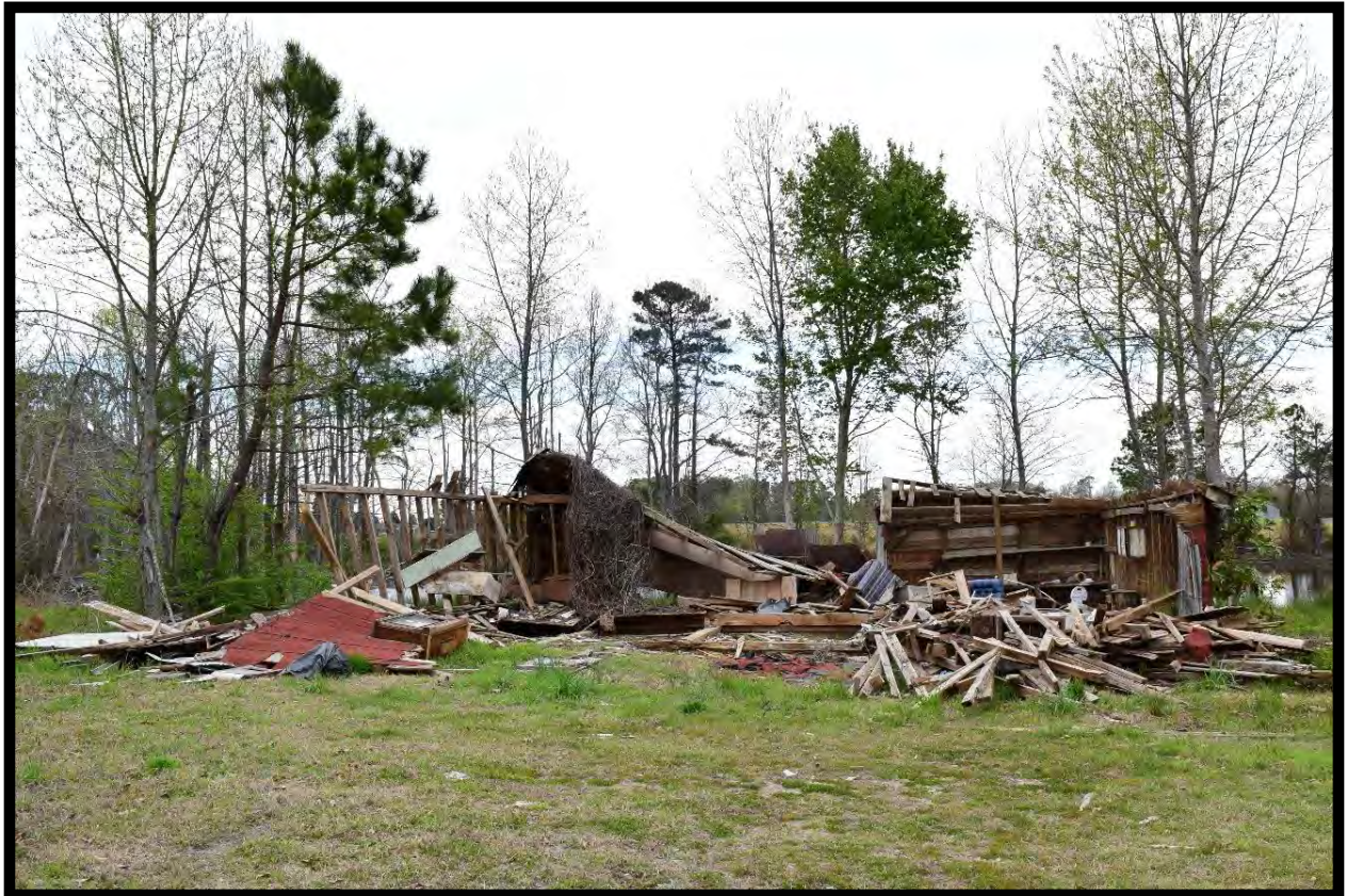
Figure 12: Barnes House, Ruins of Gambrel Roofed Barn.
