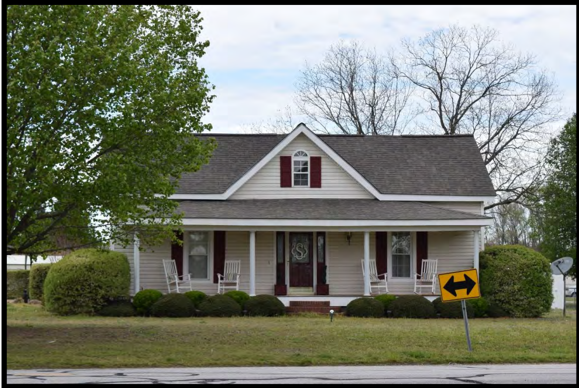
Figure 16: 6097 Covered Bridge Road, Archer Lodge, NC.
