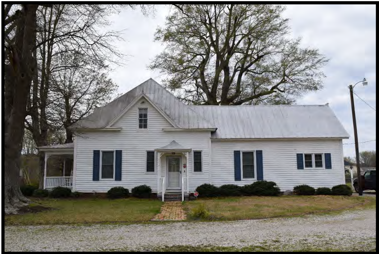
Figure 52: George Hinton House, Looking West.
