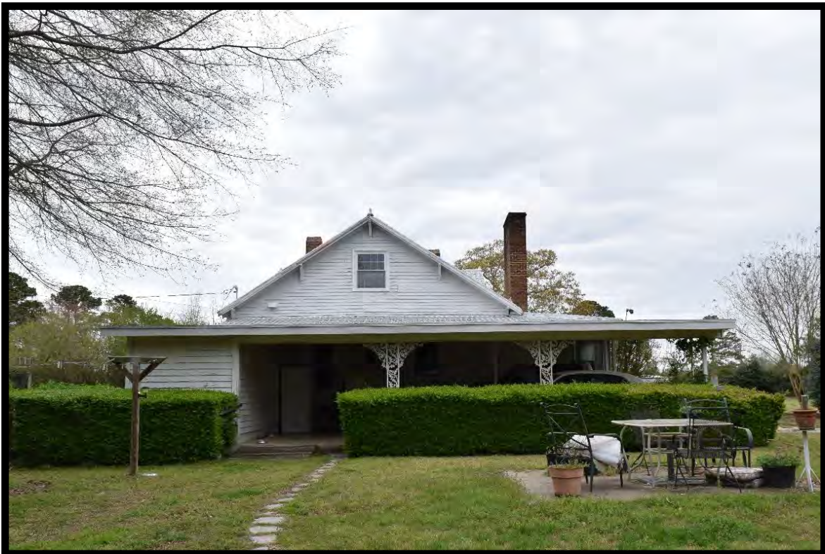
Figure 28: J. O. Barnes House, Looking East.
