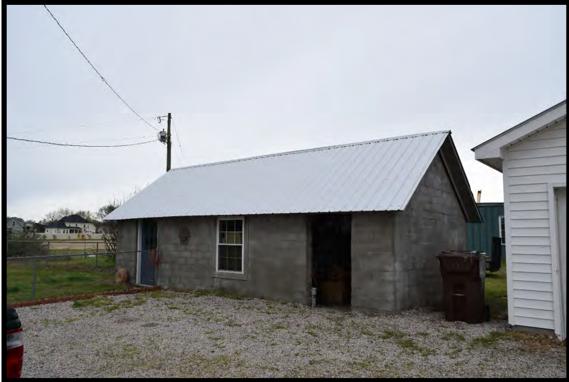
Figure 61: George Hinton House, Washhouse/Smokehouse, Looking Northwest.
