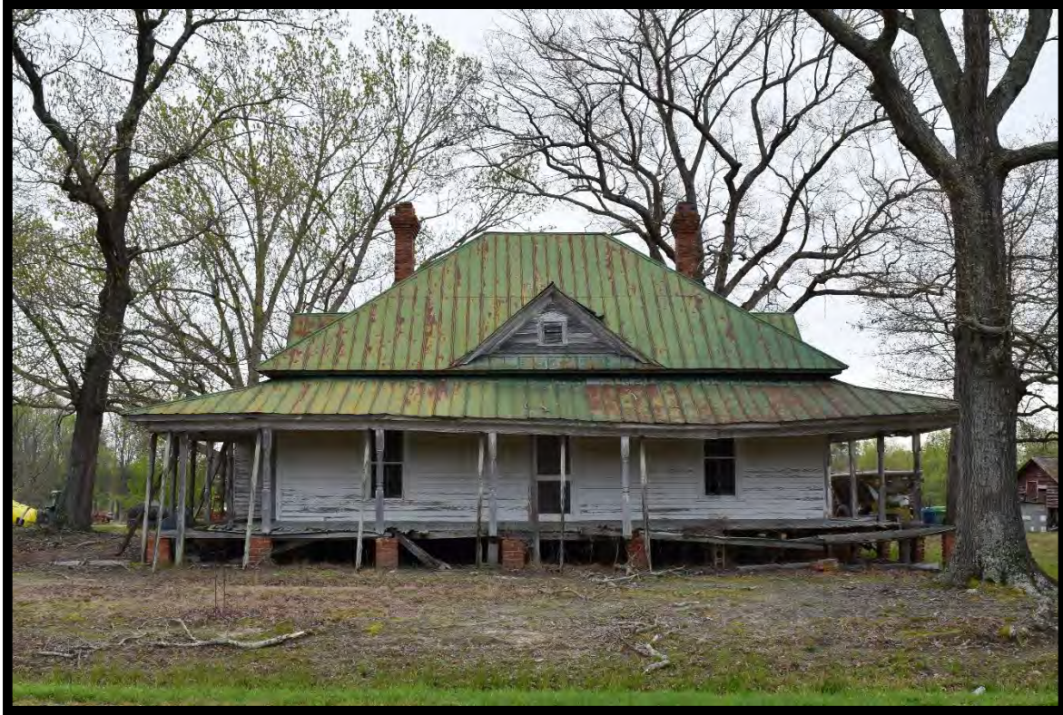
Figure 68: 106 Loop Road, Archer Lodge, North Carolina.
