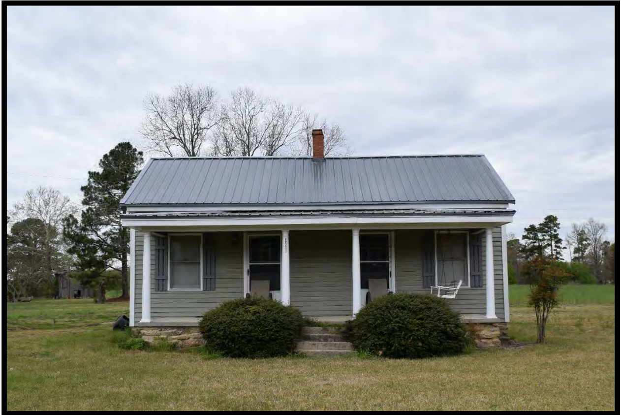
Figure 36: Wall House, Looking Northeast.
