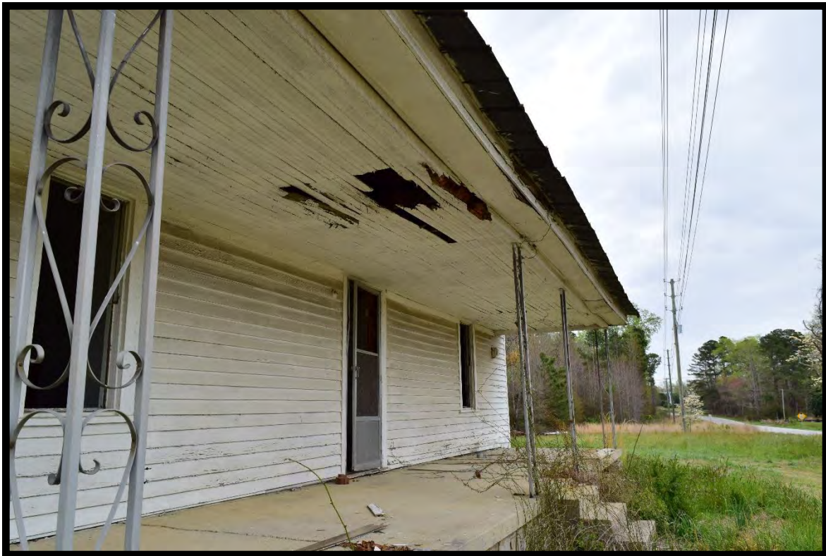
Figure 9: Barnes House, Ceiling of Porch.
