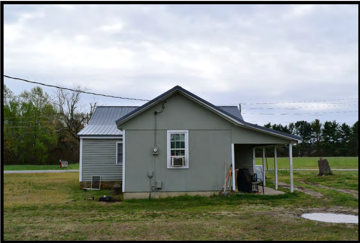
Figure 40: Wall House, Looking Southeast.
