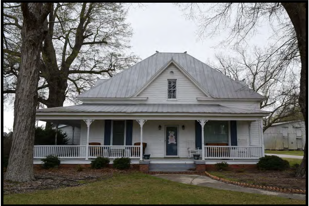
Figure 50: George Hinton House, Looking North.
