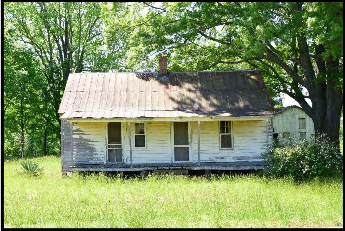
Figure 49: Farm Complex, 719 New Bethel Road (JT1702).
