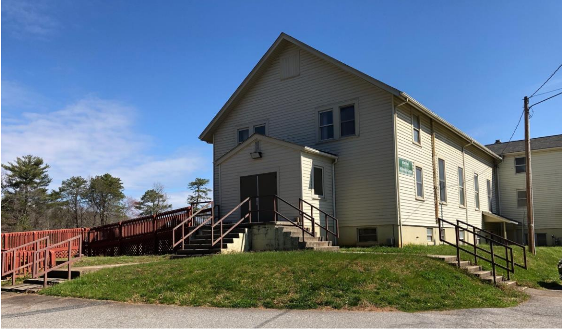
Bent Creek Baptist 1921 Church, front entrance, March 2019
