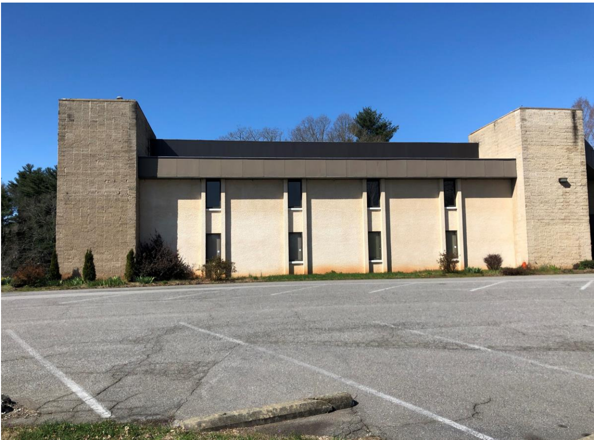
Bent Creek Baptist 1989 Church, east elevation, March 2019
