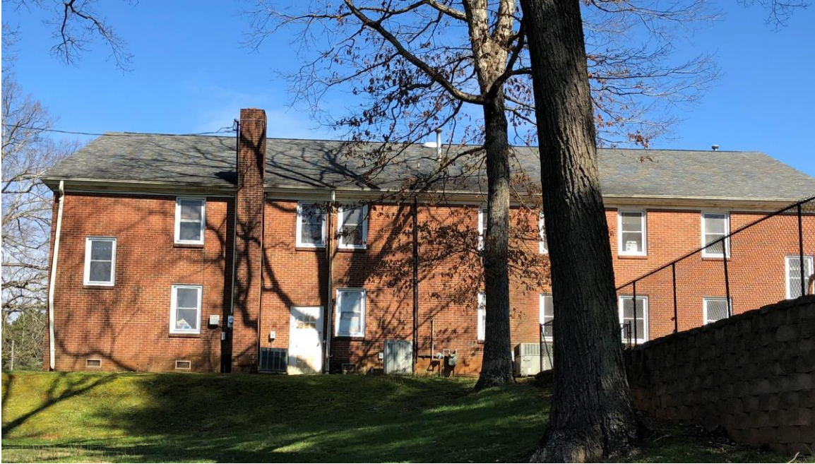
Bent Creek Baptist 1980s Fellowship Hall, south elevation, March 2019
