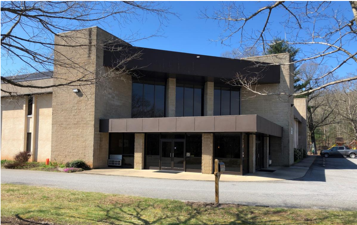
Bent Creek Baptist 1989 Church, front entrance, March 2019
