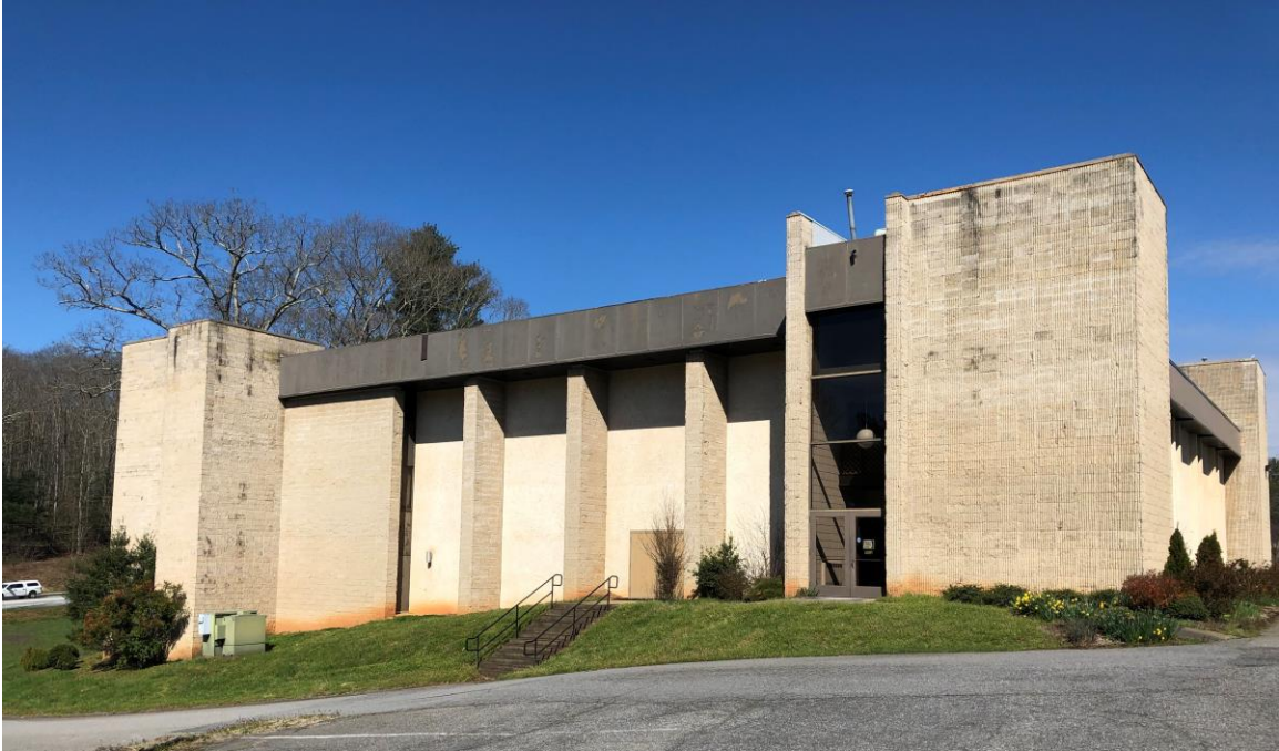
Bent Creek Baptist 1989 Church, south elevation, March 2019
