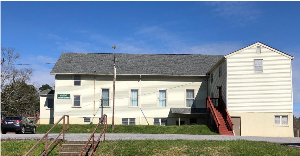
Bent Creek Baptist 1921 Church, south side elevation, March 2019
