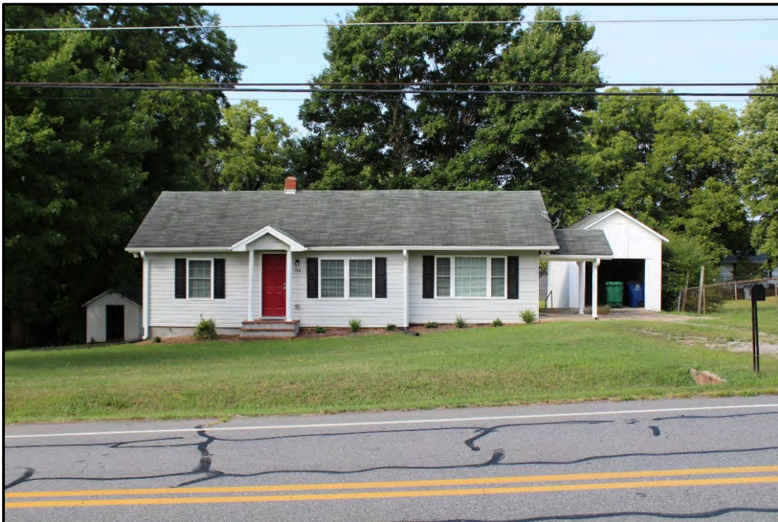
Figure 5.157. Architectural resource RK1705; view is southwest featuring the façade.
