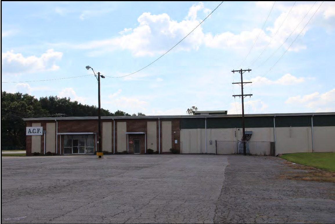
Figure 5.348. Architectural resource RK1780; view is west featuring the primary façade and main entrance of the 1960 plant building.
