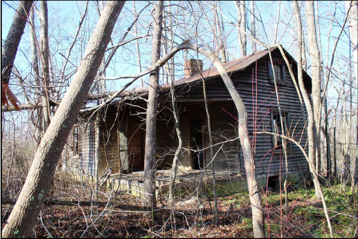
Figure 5.284. RK1758 tenant house; view is west featuring the façade and southeast elevation.
