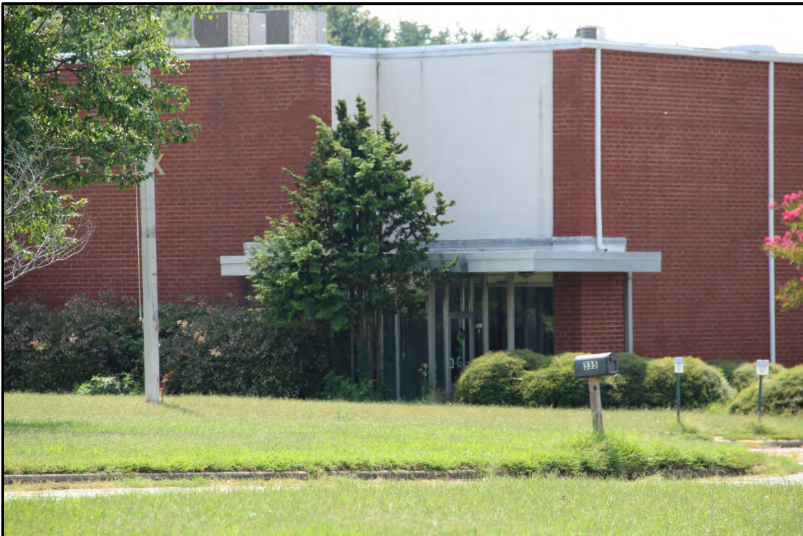
Figure 5.334. Architectural resource RK1776; view is southwest featuring the main entrance bay.
