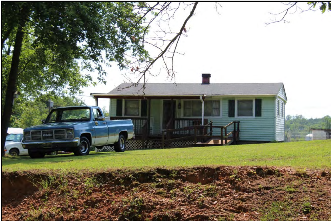
Figure 5.120. Architectural resource RK1690; view is southwest, featuring the façade and north elevation.
