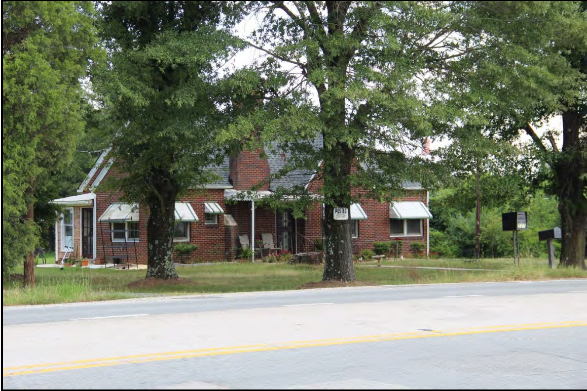
Figure 5.343. Architectural resource RK1779; view is southeast featuring the façade and north elevation.
