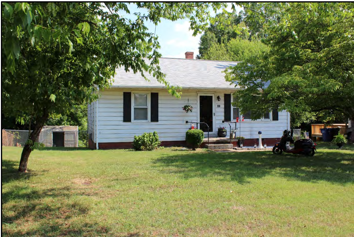
Figure 6.164. Architectural resource AM2560; view is southeast featuring the façade.
