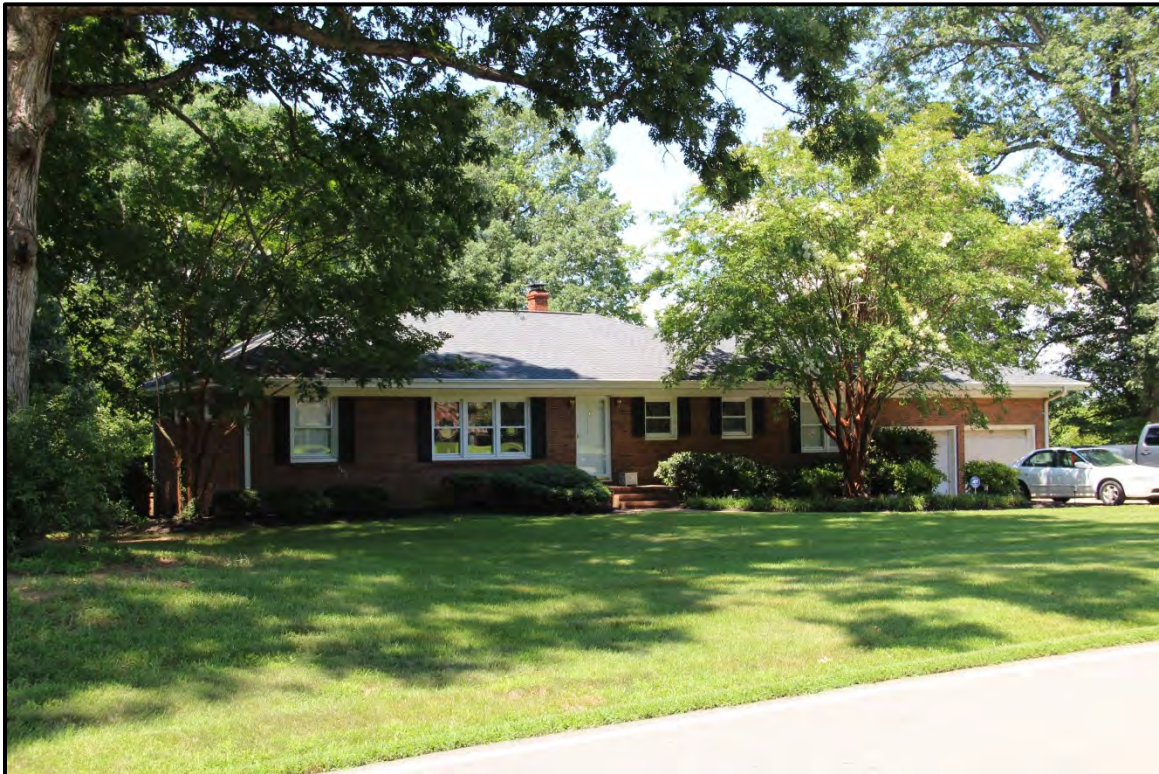
Figure 5.298. Architectural resource RK1761; view is northwest and features the façade and southwest elevation.
