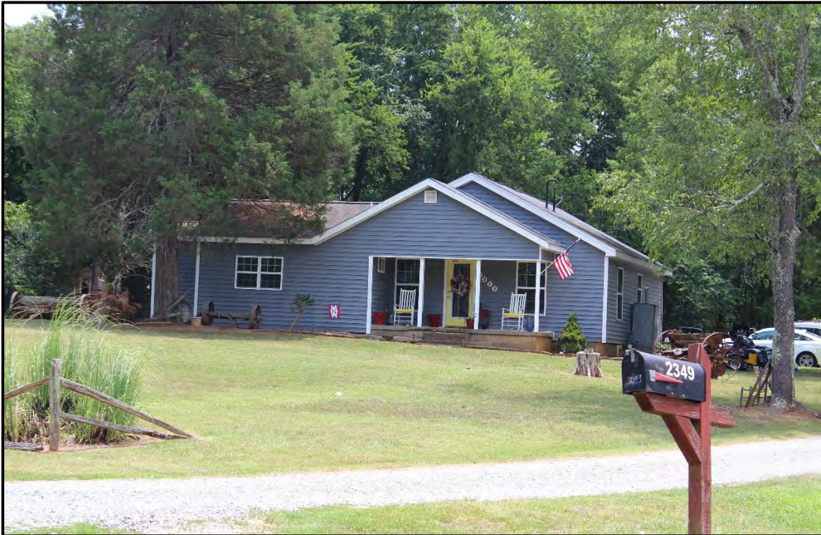
Figure 6.160. Architectural resource AM2556; view is southeast featuring the façade and southwest elevation.
