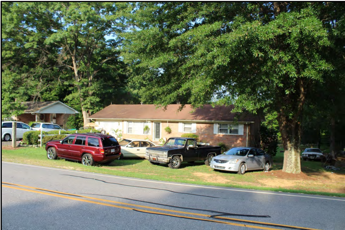
Figure 5.123. Architectural resource RK1691; view is southwest featuring the façade and north elevation.
