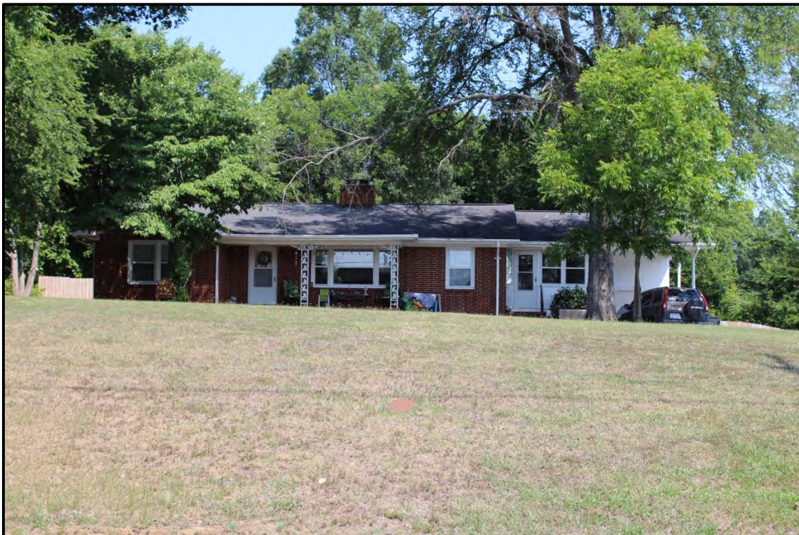
Figure 6.193. Architectural resource AM2587; view is northwest featuring the façade.
