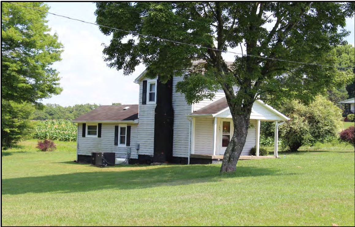
Figure 5.112. Architectural resource RK1685; view is southeast featuring façade, north elevation and rear gabled wing.
