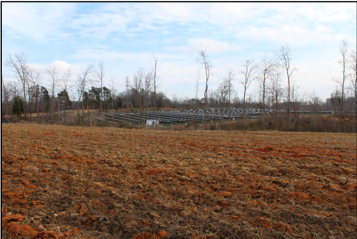
Figure 5.289. RK1758; view is southeast featuring the solar arrays on former agricultural fields.
