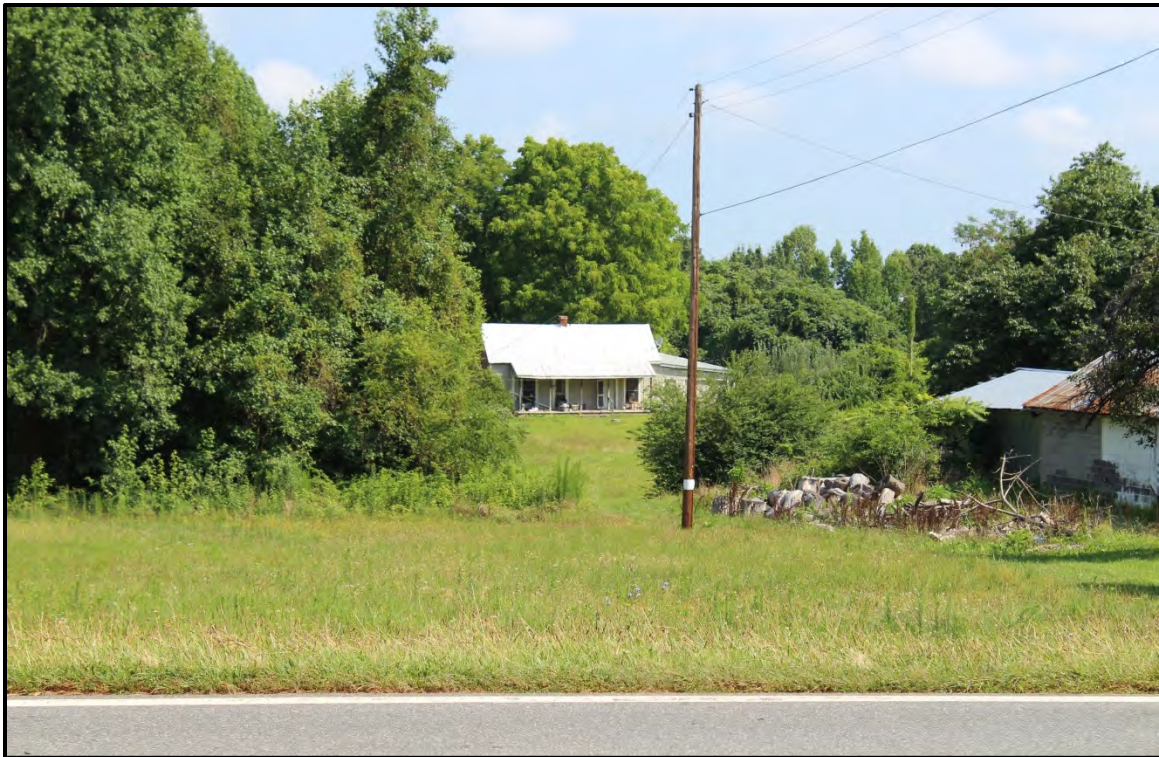
Figure 5.124. Architectural resource RK1693 (in background); view is northwest featuring the façade and hipped wing.
