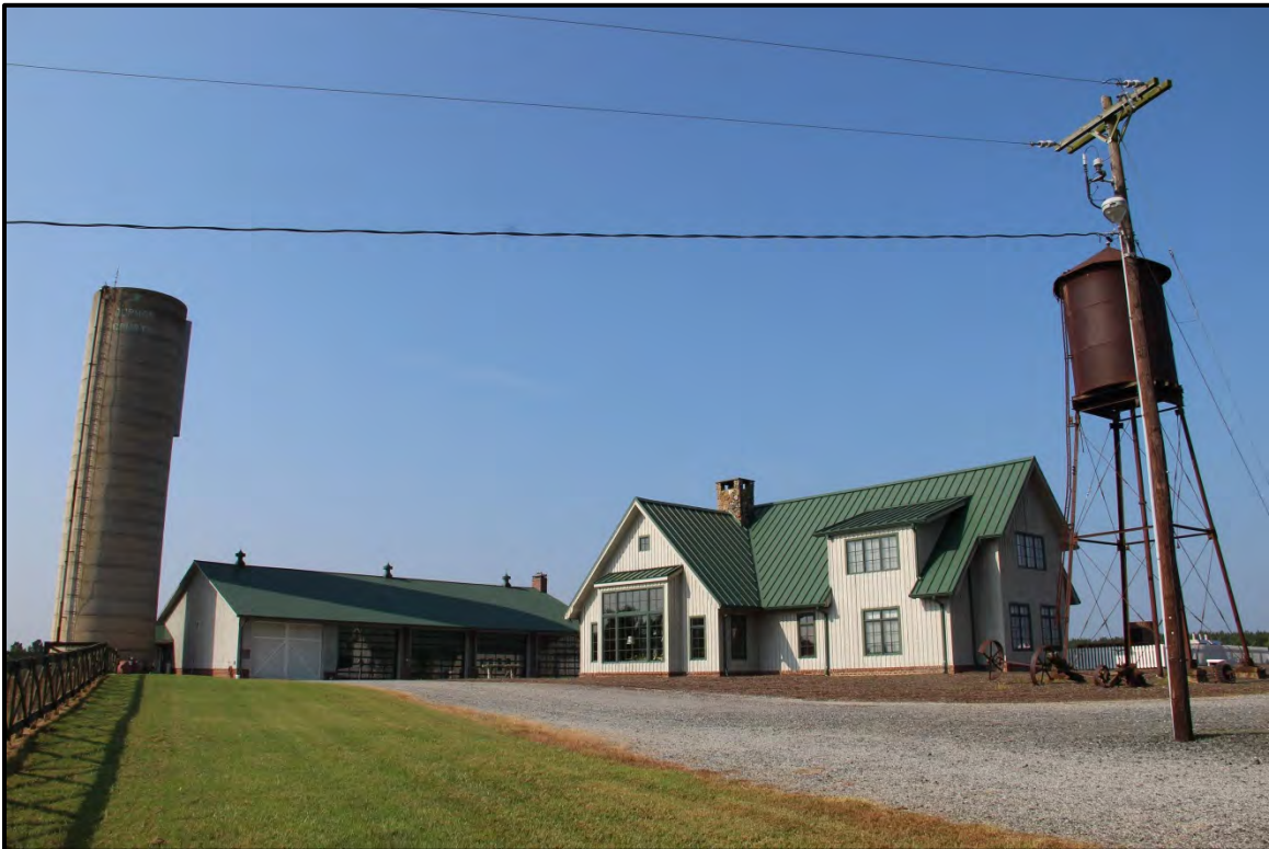
Figure 5.26. Willow Oaks Plantation House; view is southwest featuring the modern hunting lodge, ca. 1960 silo, ca. 2004 agricultural building, and ca. 1920 water tank.
