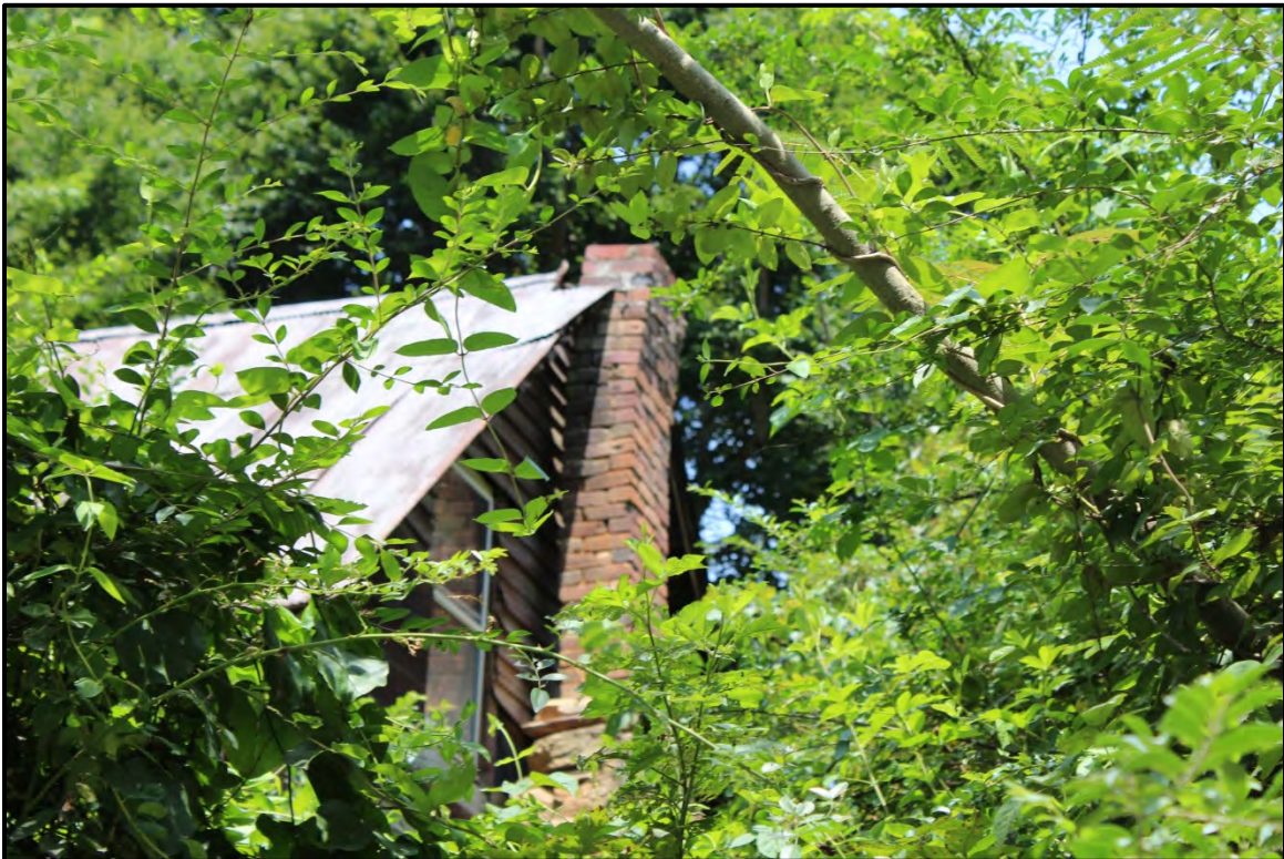
Figure 5.65. Architectural resource RK1670; photo features chimney (top) on the northeast elevation.
