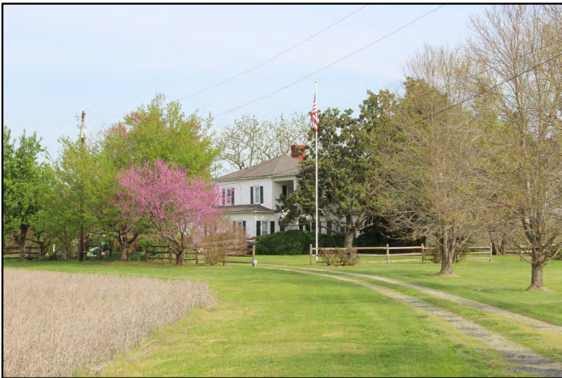
Figure 6.37. Architectural resource AM1529; view is southeast featuring the façade and north elevation.
