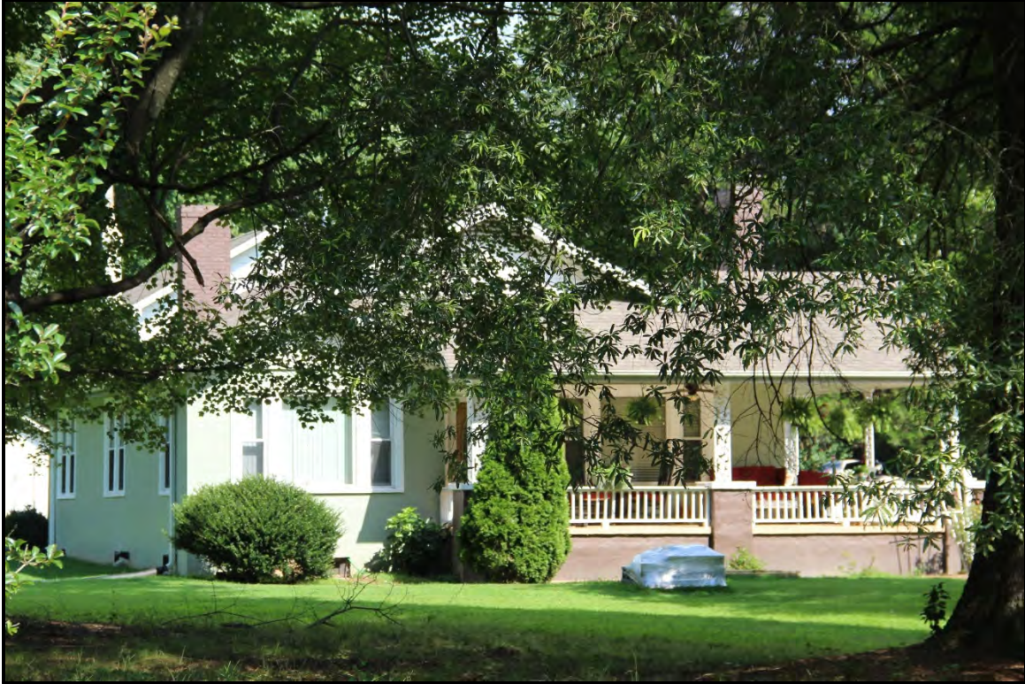
Figure 6.71. Architectural resource AM2505; zoomed-in view of the façade.
