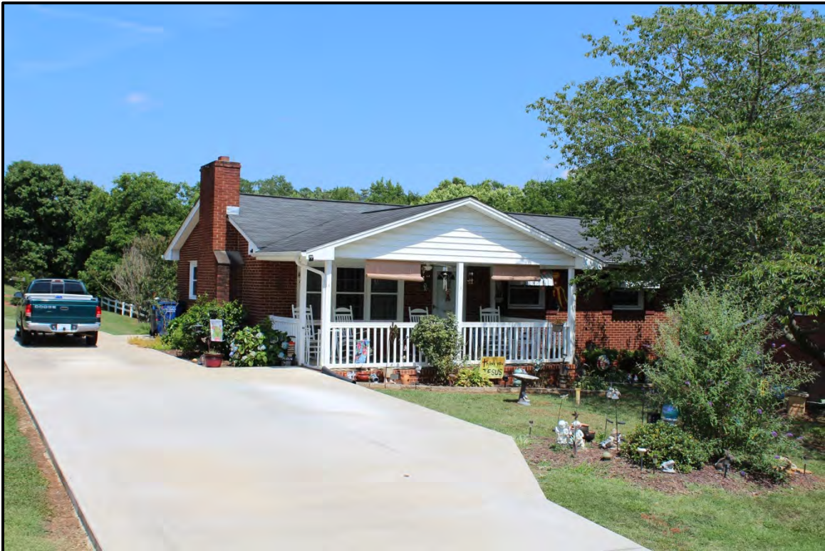
Figure 6.186. Architectural resource AM2582; view is east featuring the façade and northwest elevation.
