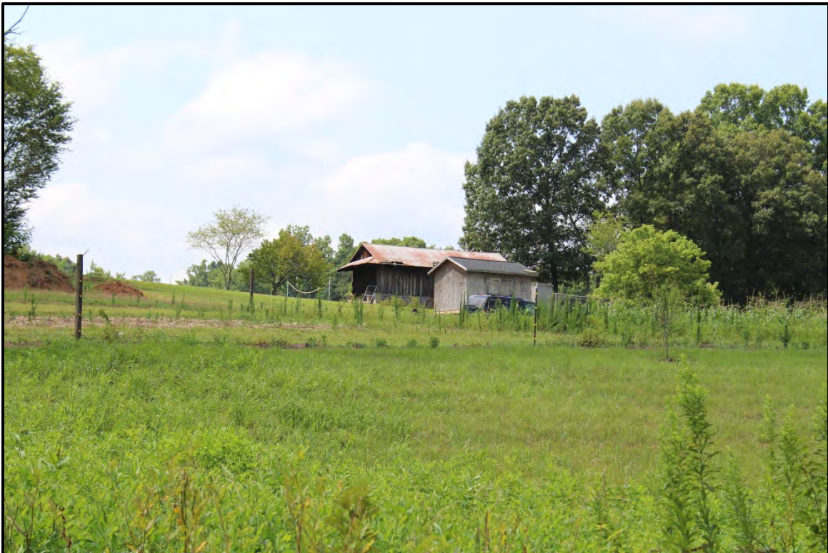
Figure 5.53. Architectural resource RK1663; frame shed and barn; view is southwest.
