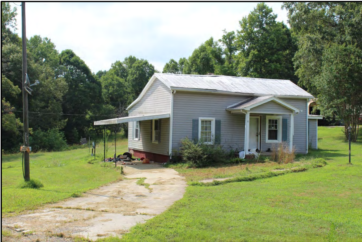
Figure 5.42. Architectural resource RK1659; view is south featuring the façade and northeast elevation.
