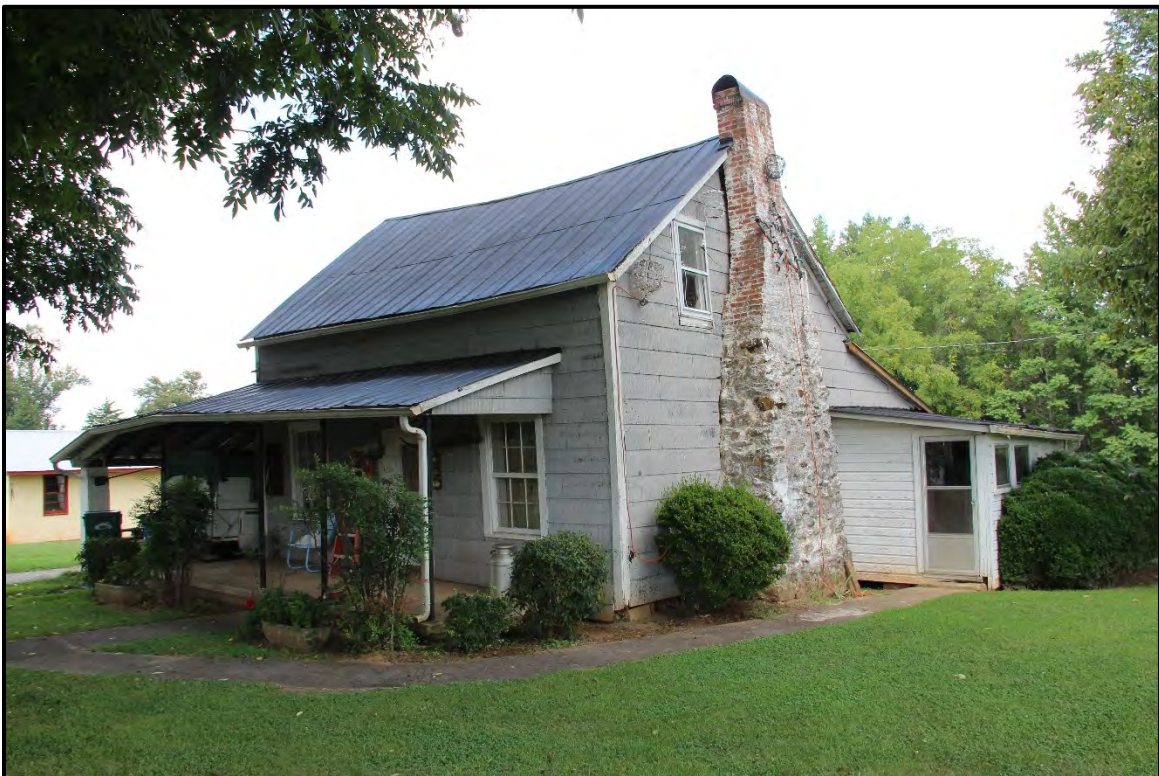
Figure 5.214. Architectural resource RK1741; view is northwest and features the façade and east elevation.
