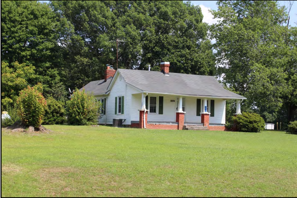
Figure 5.115. Architectural resource RK1686; view is southeast, featuring façade and north elevation.
