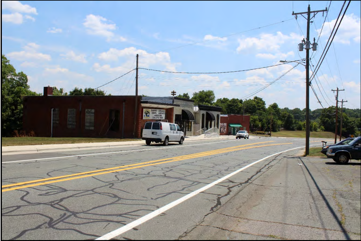
Figure 6.222. Architectural resource AM1595; East Main Street looking south.
