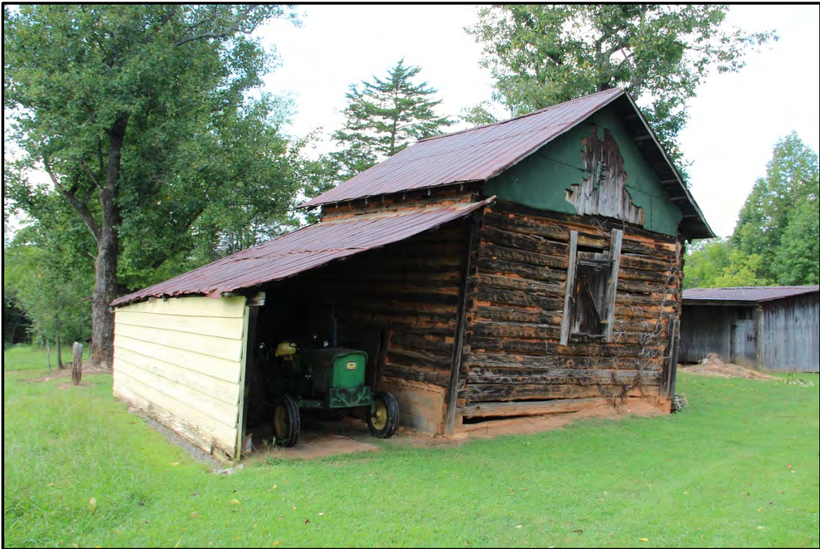
Figure 5.218. Architectural resource RK1741; view is northwest and features the log barn.
