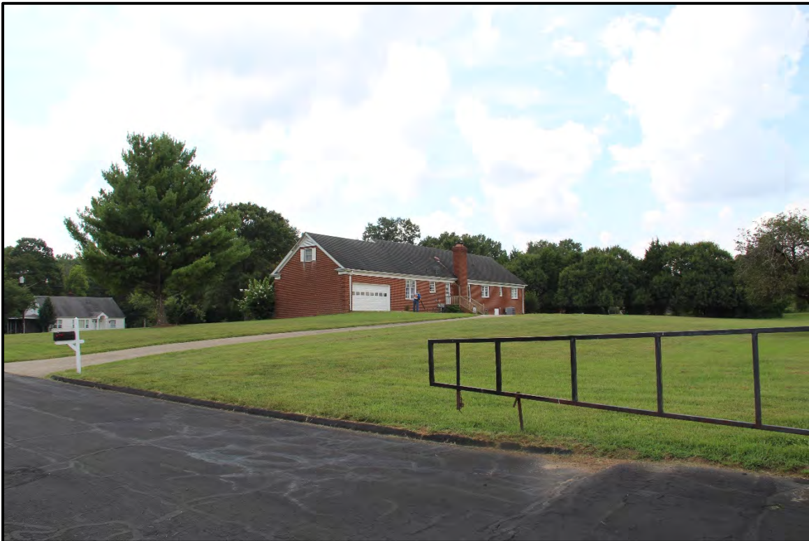
Figure 5.319. Architectural resource RK1770; view is southwest featuring the east and north (rear) elevations of the church manse.
