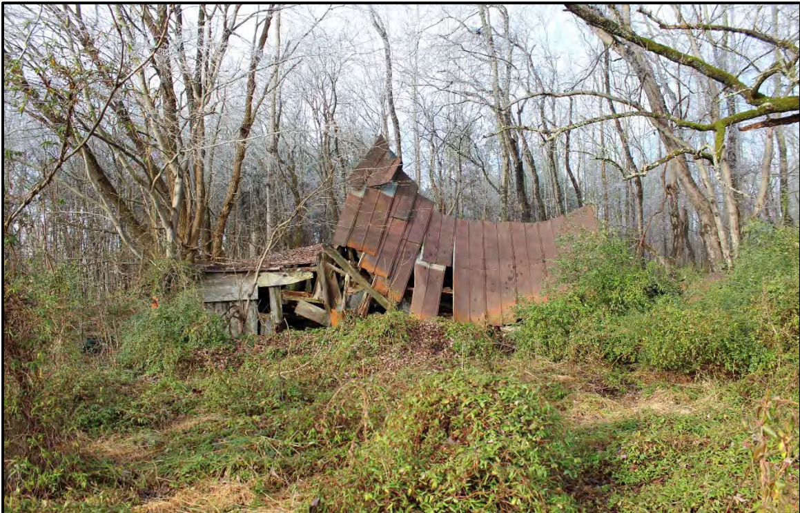
Figure 6.9. Architectural resource AM1520; view is north featuring one of three collapsed outbuildings.
