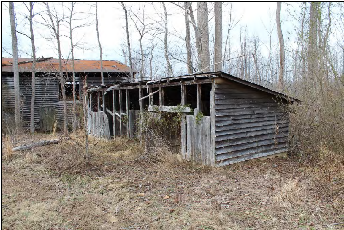
Figure 5.273. RK1758 stables; view is northwest featuring the façade and southeast elevation.
