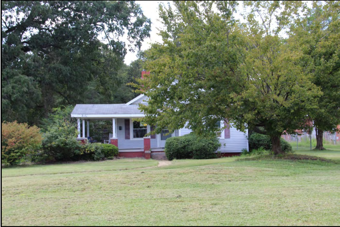
Figure 5.337. Architectural resource RK1777; view is west featuring the façade.
