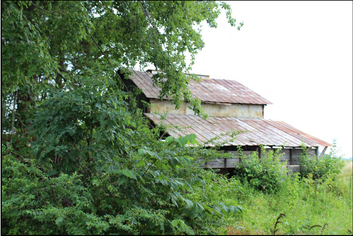
Figure 5.305. Architectural resource RK1764; view is northwest and features the tobacco barn.
