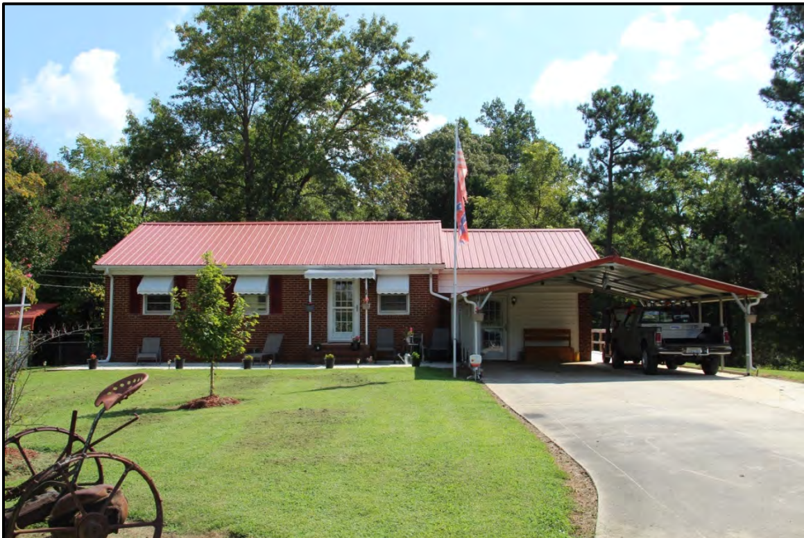
Figure 6.75. Architectural resource AM2508; view is east showing the façade and modern carport.
