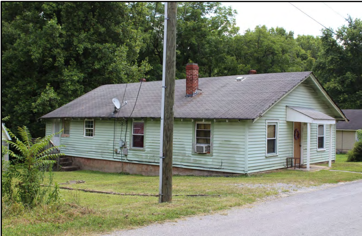
Figure 5.171. Architectural resource RK1717; view is east showing the façade and northwest elevation.
