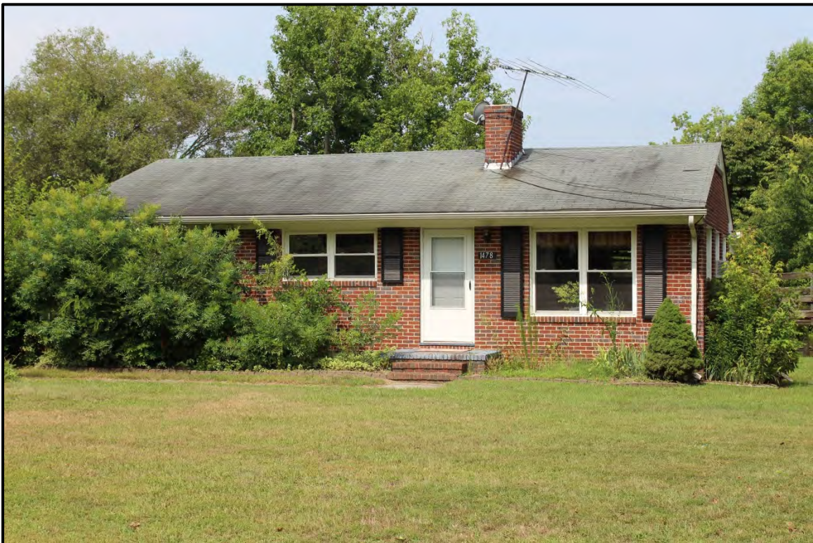
Figure 5.211. Architectural resource RK1739; view is west and features the façade.
