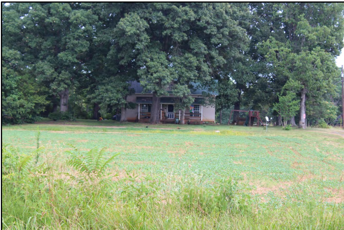
Figure 5.302. Architectural resource RK1763; view is east and features the façade.
