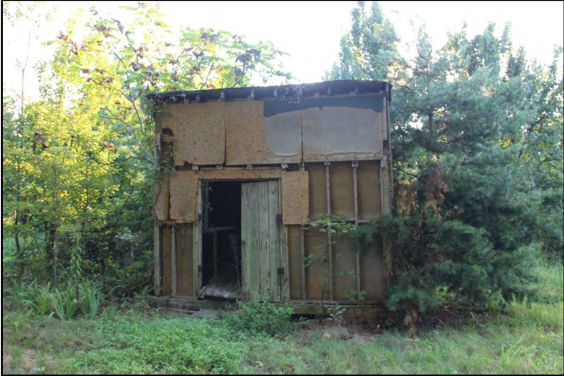
Figure 5.88. Architectural resource RK1768; view is east and features the shed.
