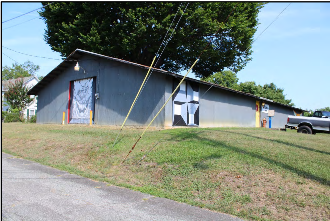
Figure 6.206. Architectural resource AM2595; view is northwest and features the south and east elevations.
