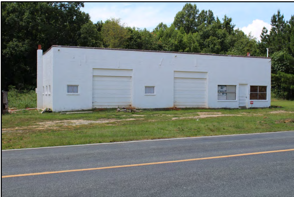
Figure 6.72. Architectural resource AM2507; view is northwest featuring the façade.
