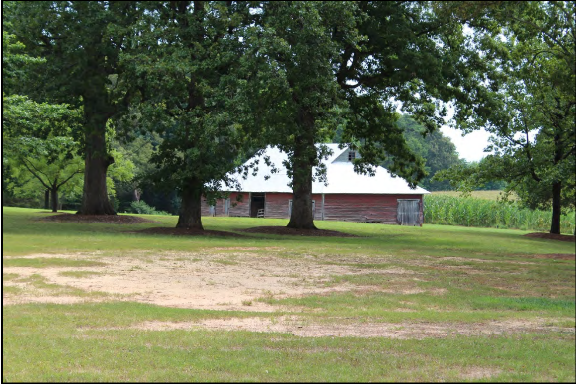
Figure 5.227. Architectural resource RK1534; view is southeast featuring the 1950 livestock barn.
