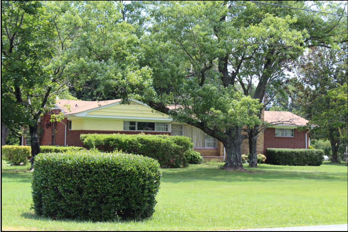
Figure 6.45. Architectural resource AM2497; view is southeast featuring the façade and north elevation.
