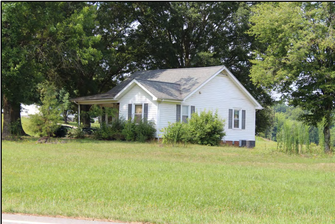
Figure 5.44. Architectural resource RK1661; view is southwest featuring the front-gabled wing and north elevation.
