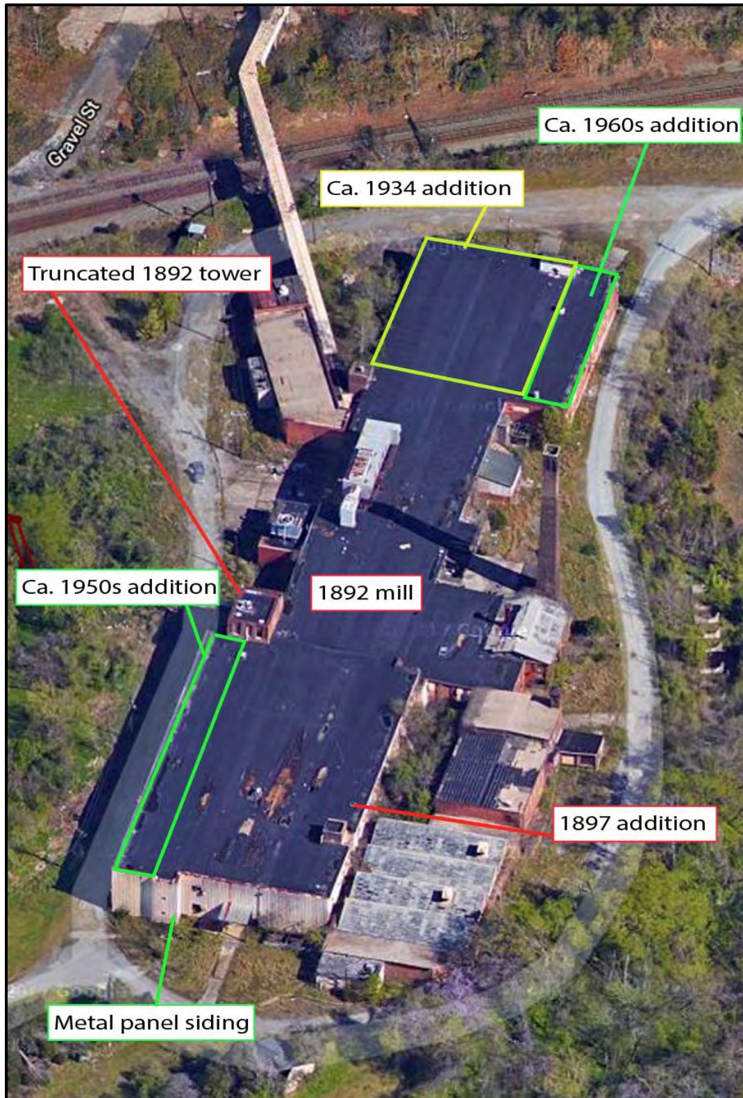
Figure 6.240. Current aerial view of the Holt-Tabardrey Mill depicting the metal panel siding applied to the south elevation and assorted alterations to the mill; view is north (image courtesy of Google Earth).
