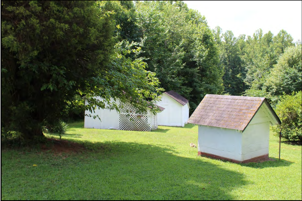
Figure 5.182. Architectural resource RK1723; view is south featuring the associated outbuildings.
