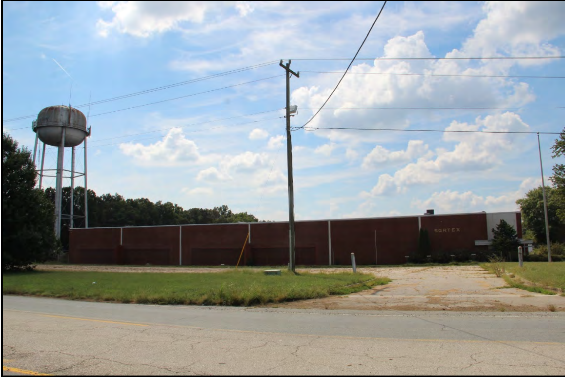
Figure 5.333. Architectural resource RK1776; view is west featuring the primary façade.
