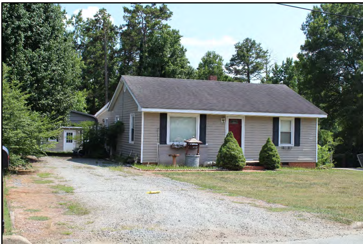
Figure 6.170. Architectural resource AM2566; view is south featuring the façade and northeast elevation.
