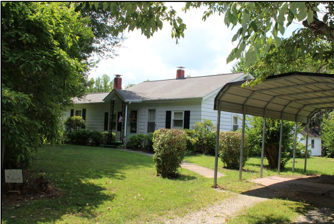
Figure 5.181. Architectural resource RK1723; view is south showing the façade and northwest elevation.
