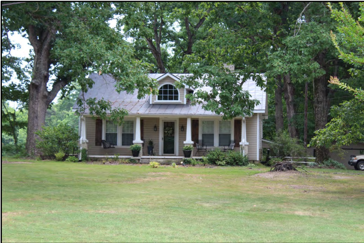
Figure 5.232. Architectural resource RK1746; view is southeast and features the façade.
