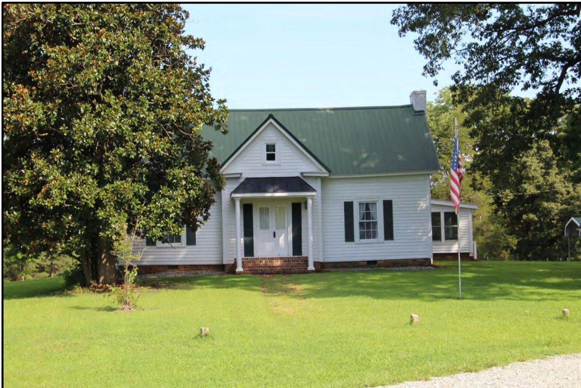
Figure 6.142. Architectural resource AM2542; view is northwest featuring the façade.
