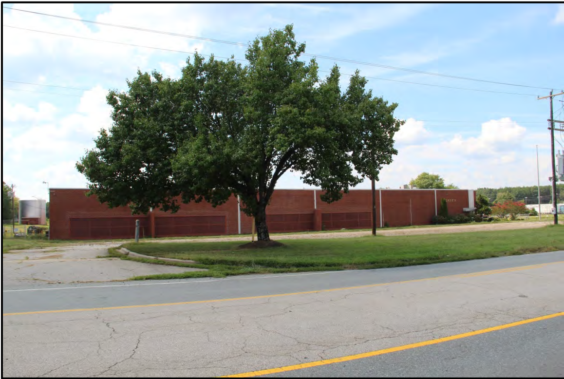
Figure 5.336. Architectural resource RK1776; view is northwest featuring the primary façade.
