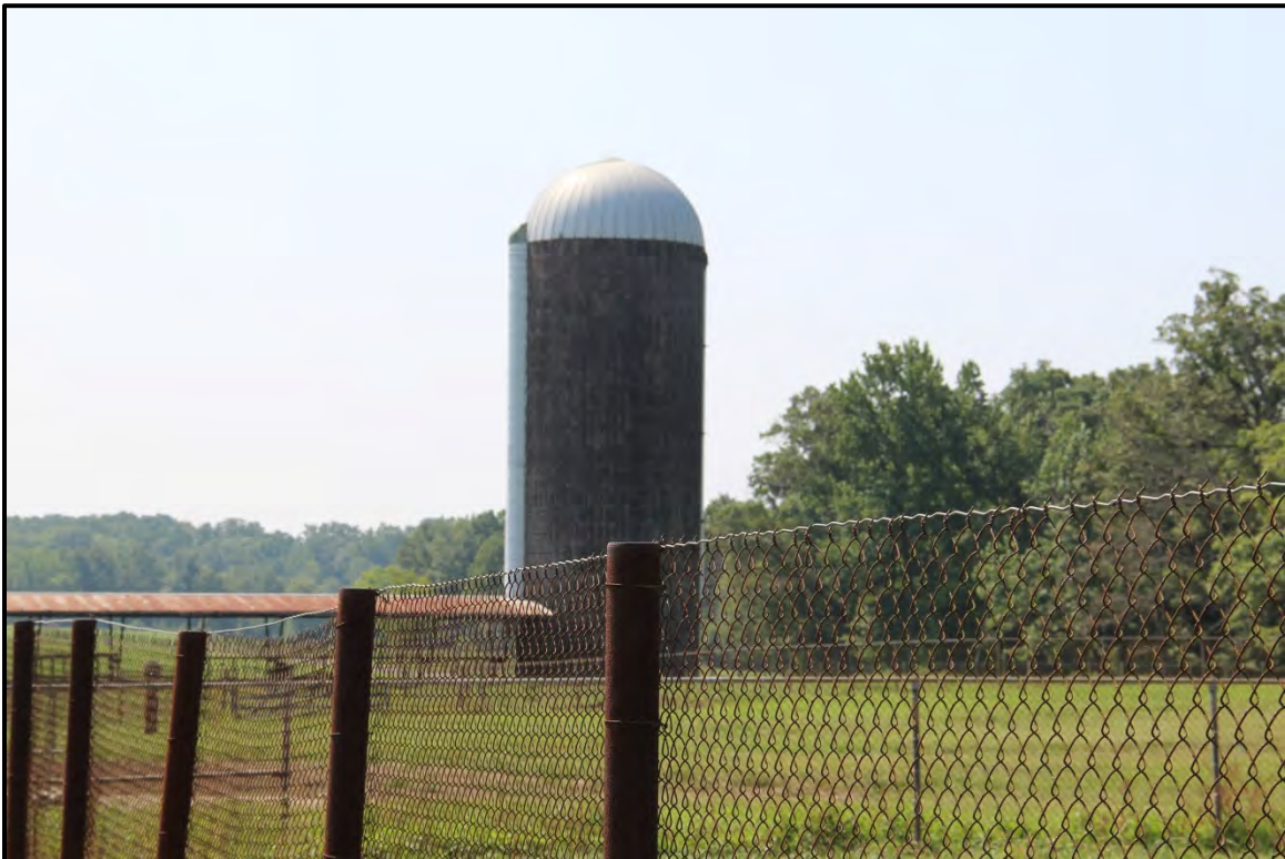
Figure 5.7. Architectural resource RK1655; view is south featuring the ca. 1940 silo and ca. 1970 livestock feeder.
