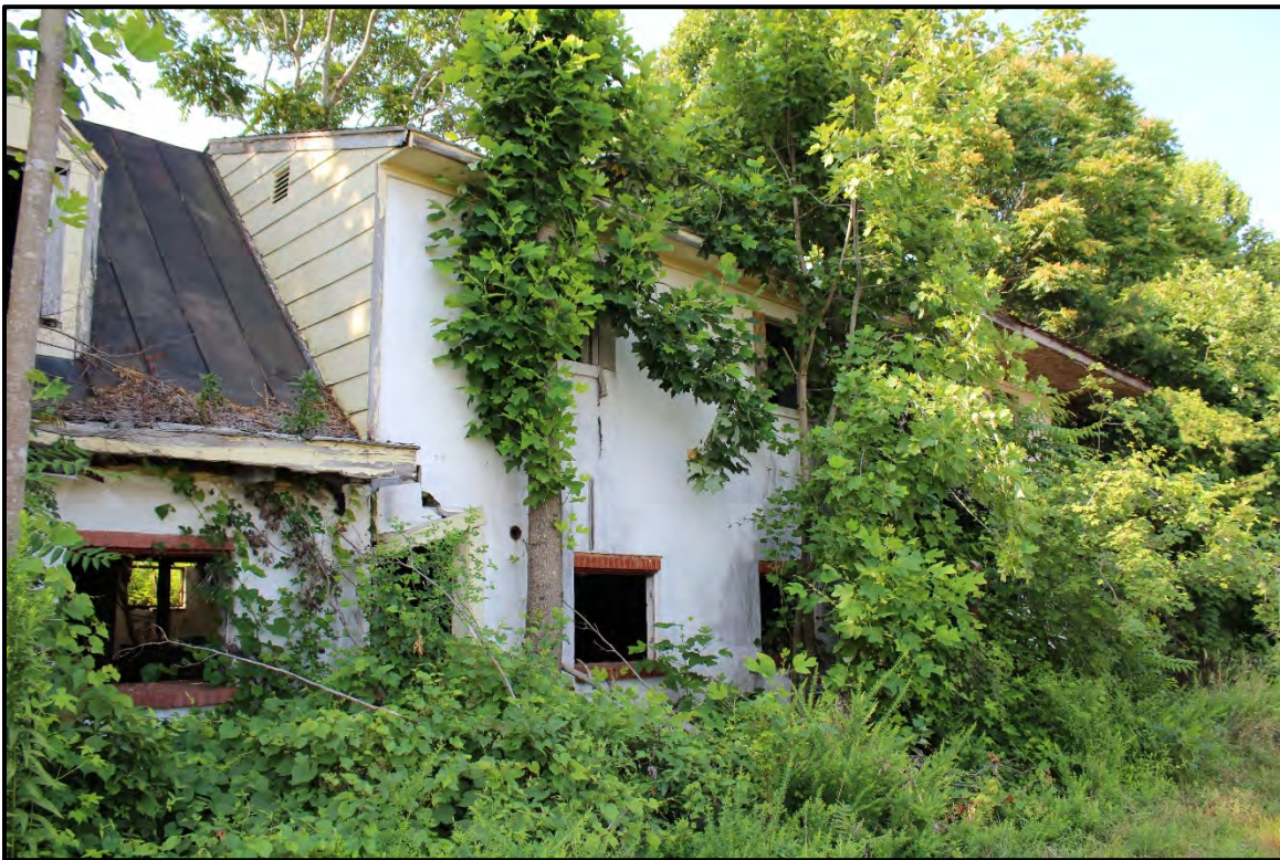
Figure 5.143. Architectural resource RK1702; detail view featuring the two-story masonry addition.
