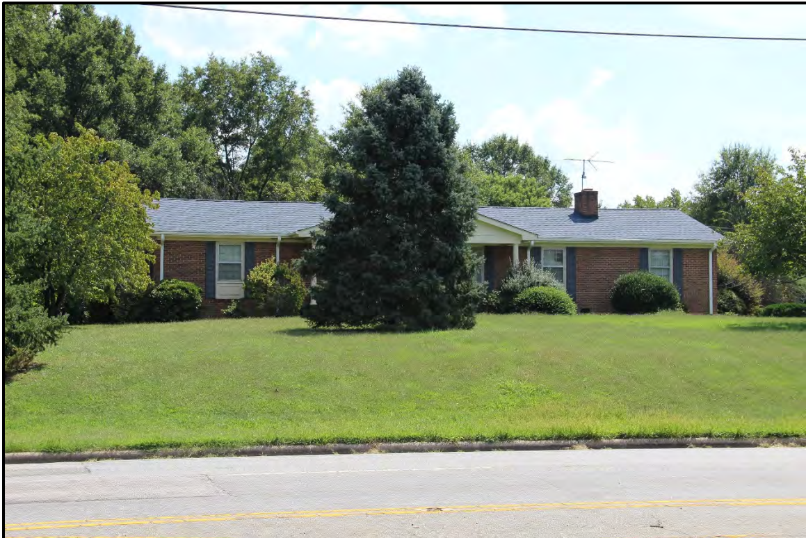
Figure 5.332. Architectural resource RK1775; view is south featuring the façade.
