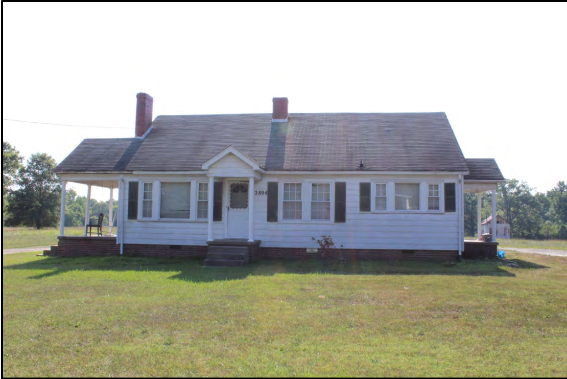
Figure 6.121. Architectural resource AM2527; view is west featuring the façade.
