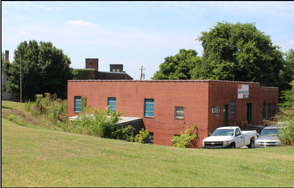
Figure 6.194. Architectural resource AM2588; view is south featuring the northeast corner of the commercial building.
