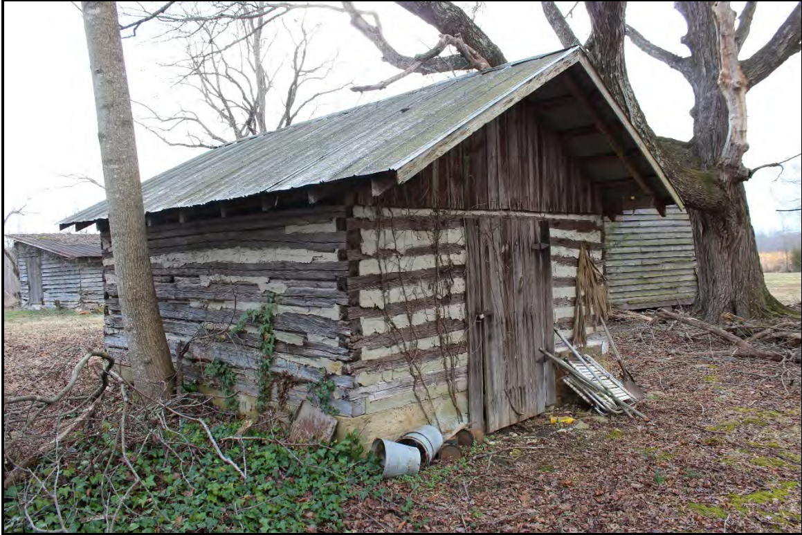
Figure 5.260. RK1758 smokehouse; view is southwest featuring the façade and east elevation.
