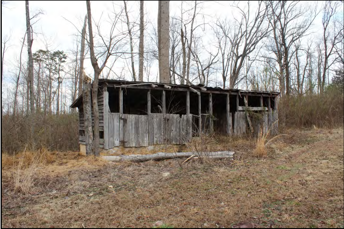
Figure 5.274. RK1758 stables; view is northeast featuring the façade and northwest elevation.
