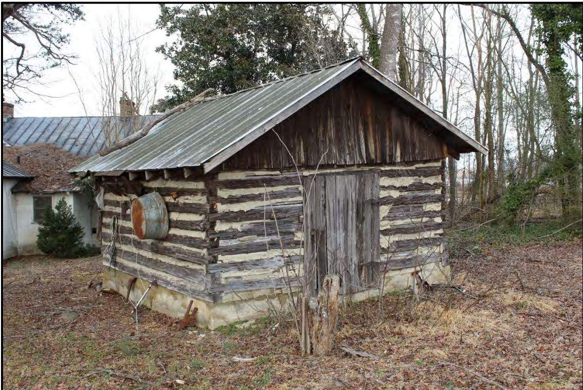
Figure 5.261. RK1758 smokehouse; view is northeast featuring the south (rear) and west elevations.
