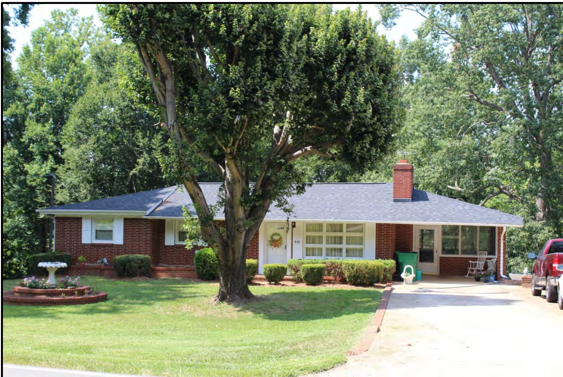
Figure 5.200. Architectural resource RK1735; view is north showing the façade.
