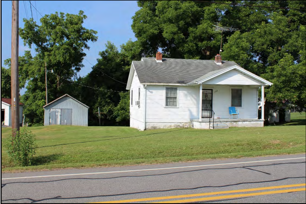
Figure 5.159. Architectural resource RK1706; view is northwest showing the façade and southwest elevation.
