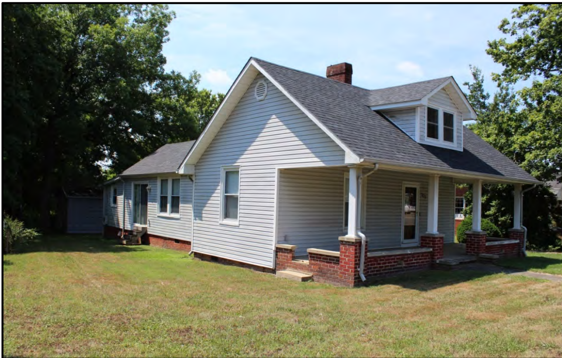
Figure 6.270. Architectural resource AM2602; view is southwest and features the façade and east elevation.
