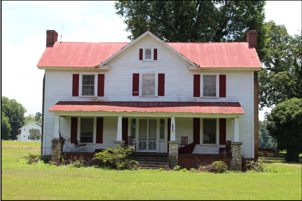
Figure 6.54. Architectural resource AM0160; view is south featuring the façade.
