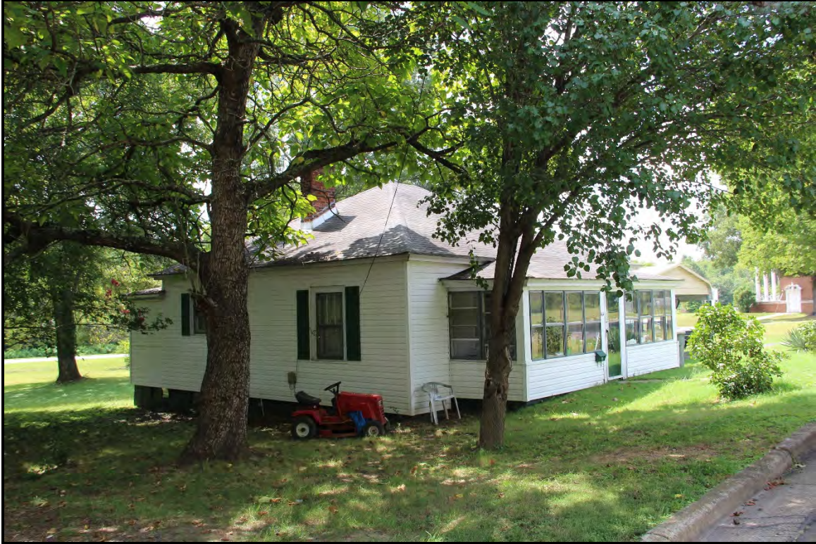
Figure 5.325. Architectural resource RK1772; view is southwest featuring the façade and east elevation.
