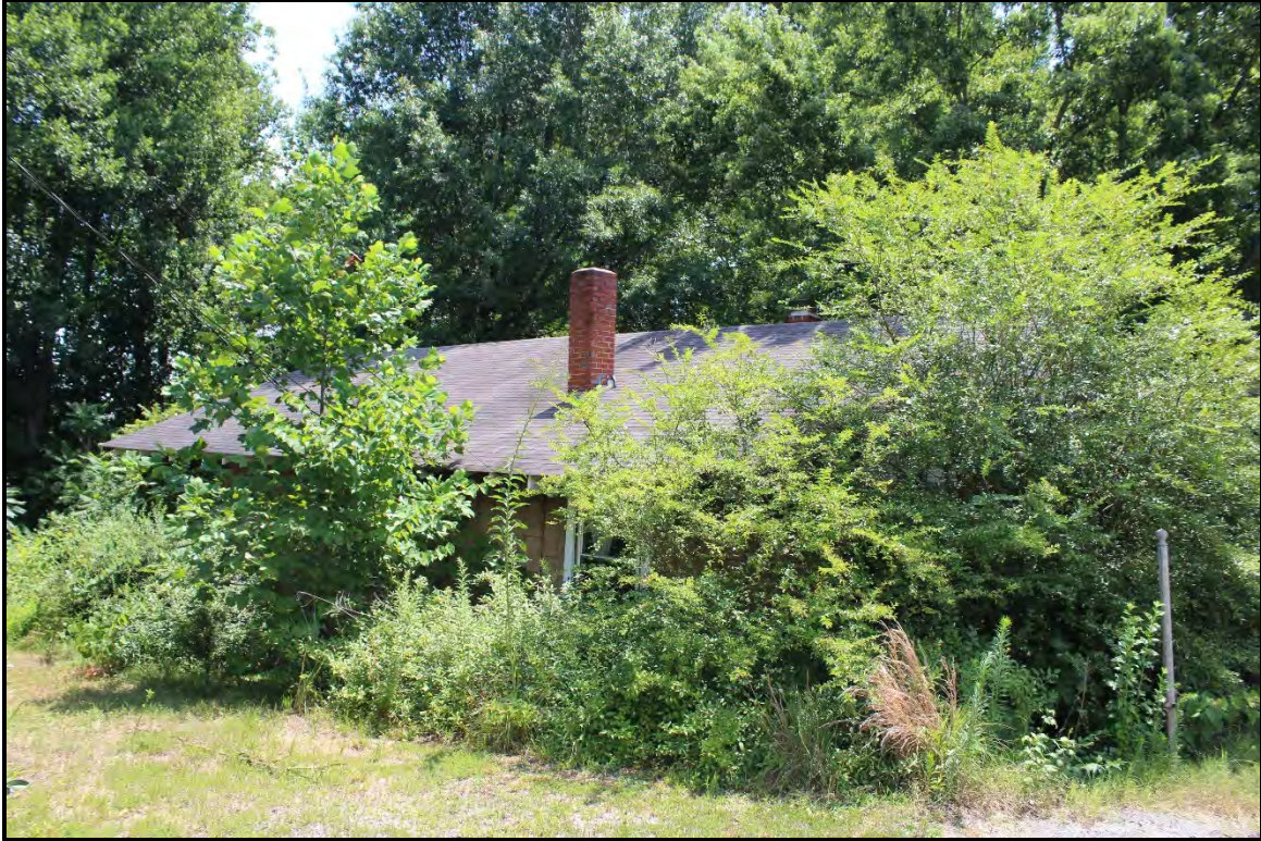
Figure 5.178. Architectural resource RK1721; view is south featuring the northwest elevation.
