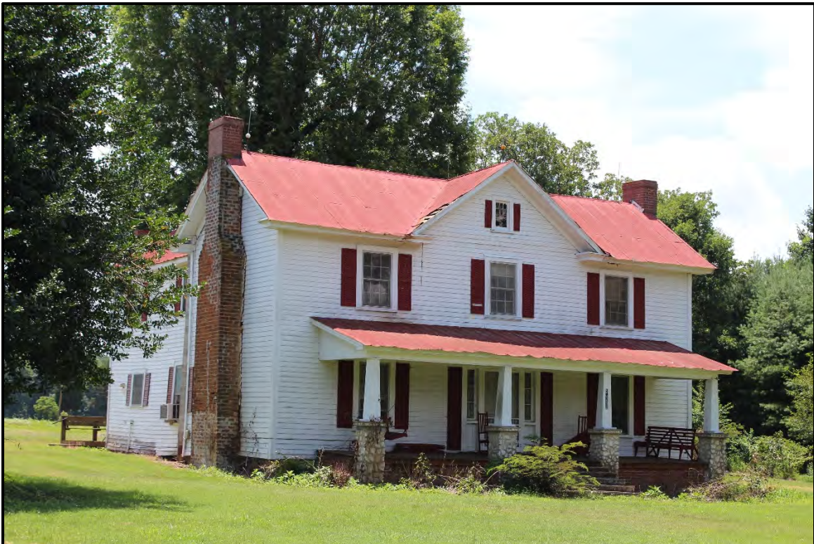
Figure 6.55. Architectural resource AM0160; view is southwest featuring the façade and the east elevation.
