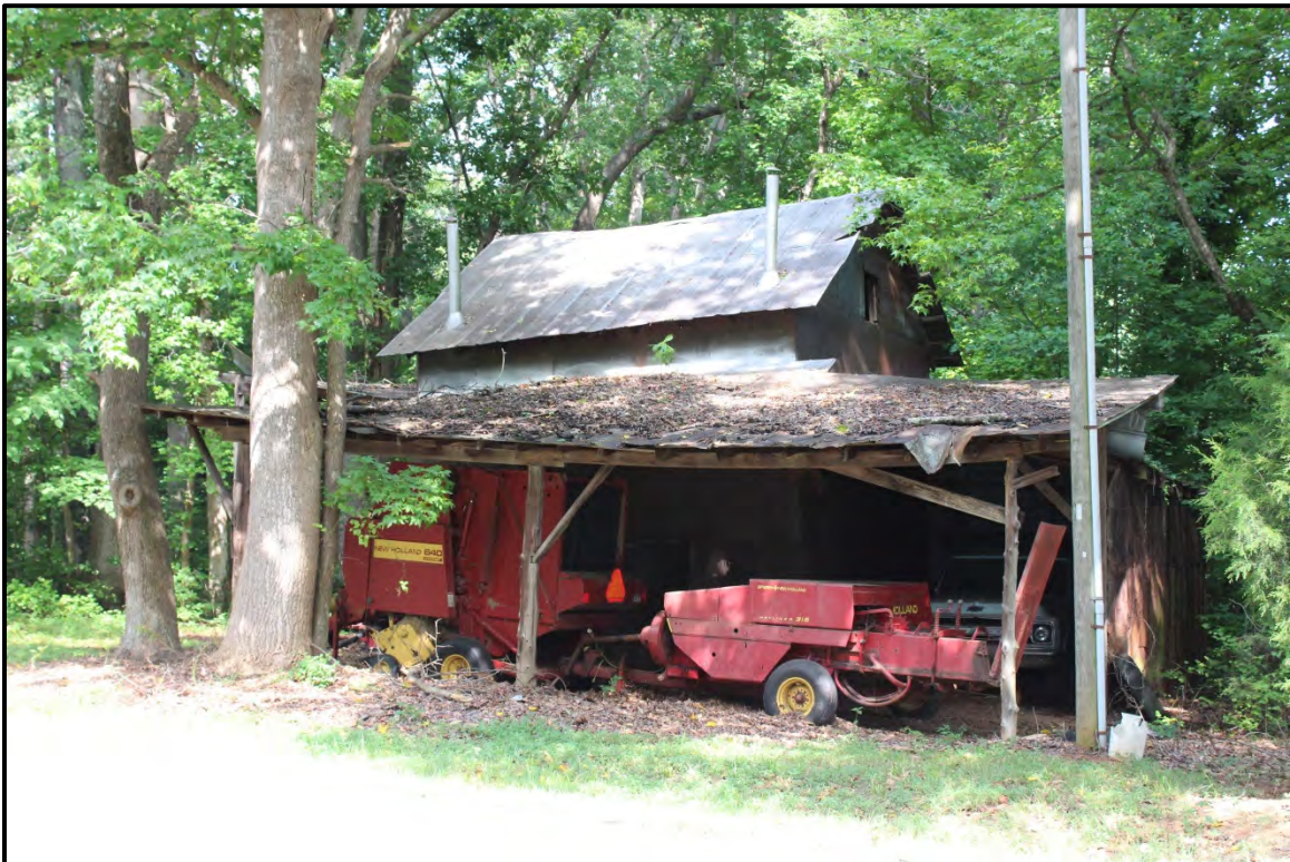
Figure 6.99. Architectural resource AM2516; view is southwest and features tobacco barn.
