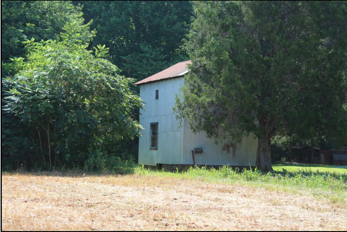
Figure 6.13. Architectural resource AM2490; view is southeast featuring the tobacco barn.
