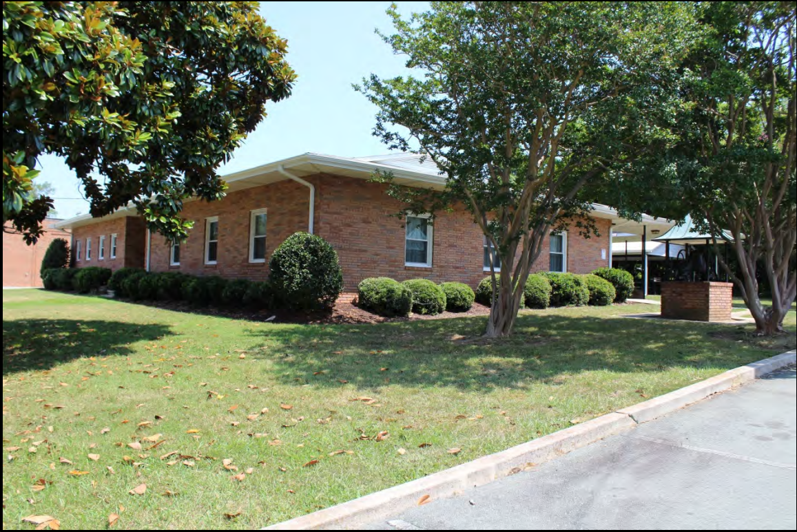
Figure 6.266. Architectural resource AM2599; view is northeast and features the façade and south elevation.
