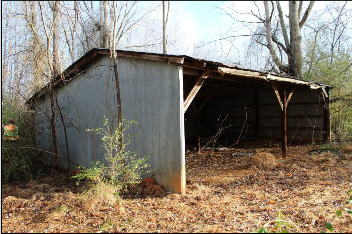
Figure 6.6. Architectural resource AM1520; view is northeast featuring the equipment shed.
