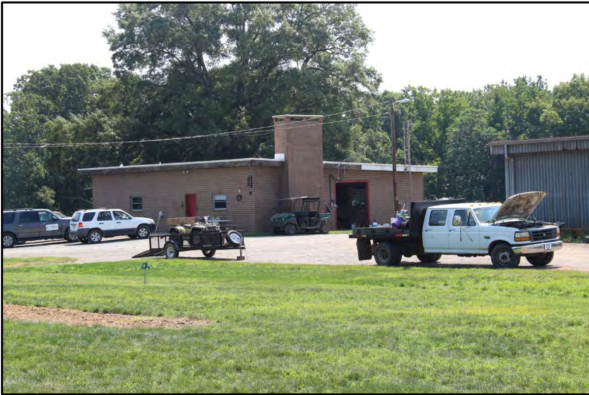
Figure 5.5. Architectural resource RK1655; view is southeast featuring the 1970 office building.
