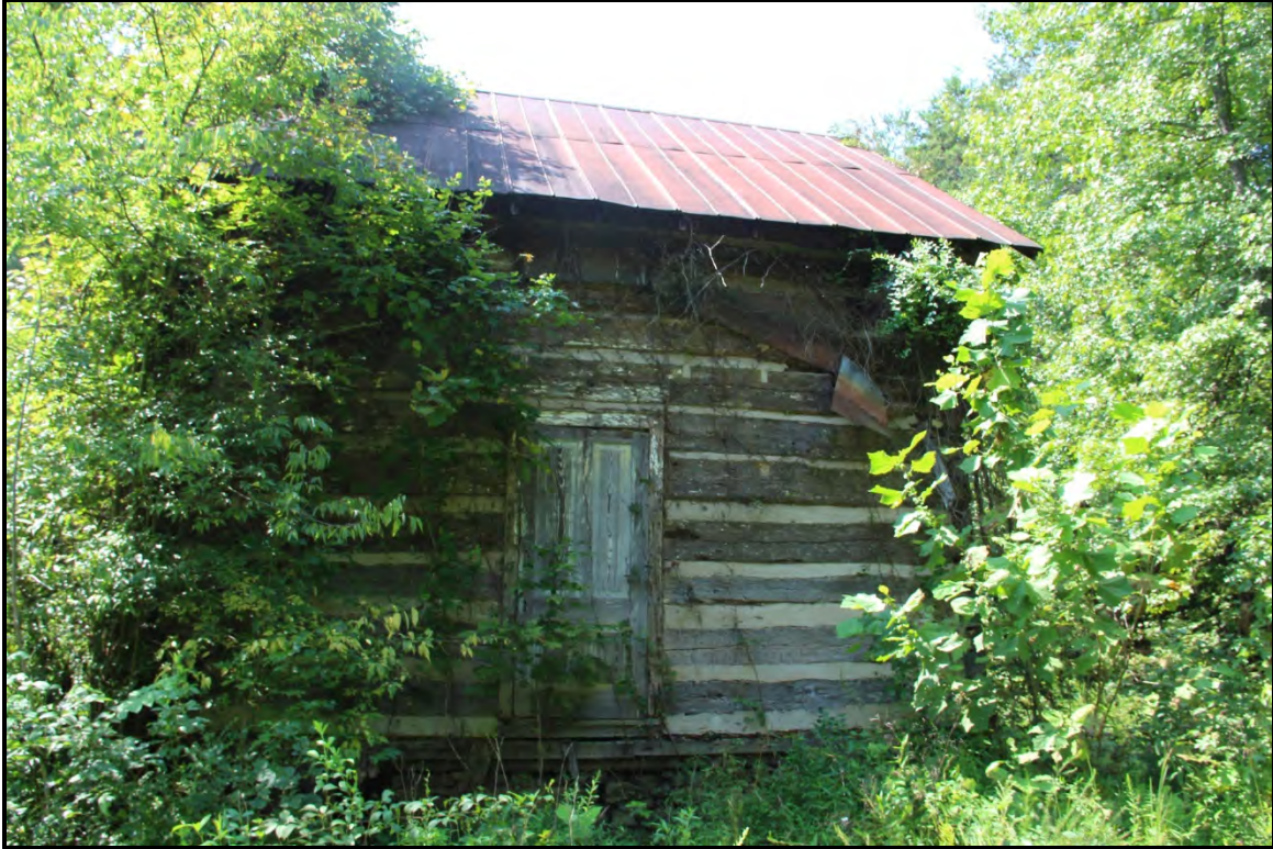
Figure 5.9. Architectural resource RK1656; view is southwest featuring the façade.
