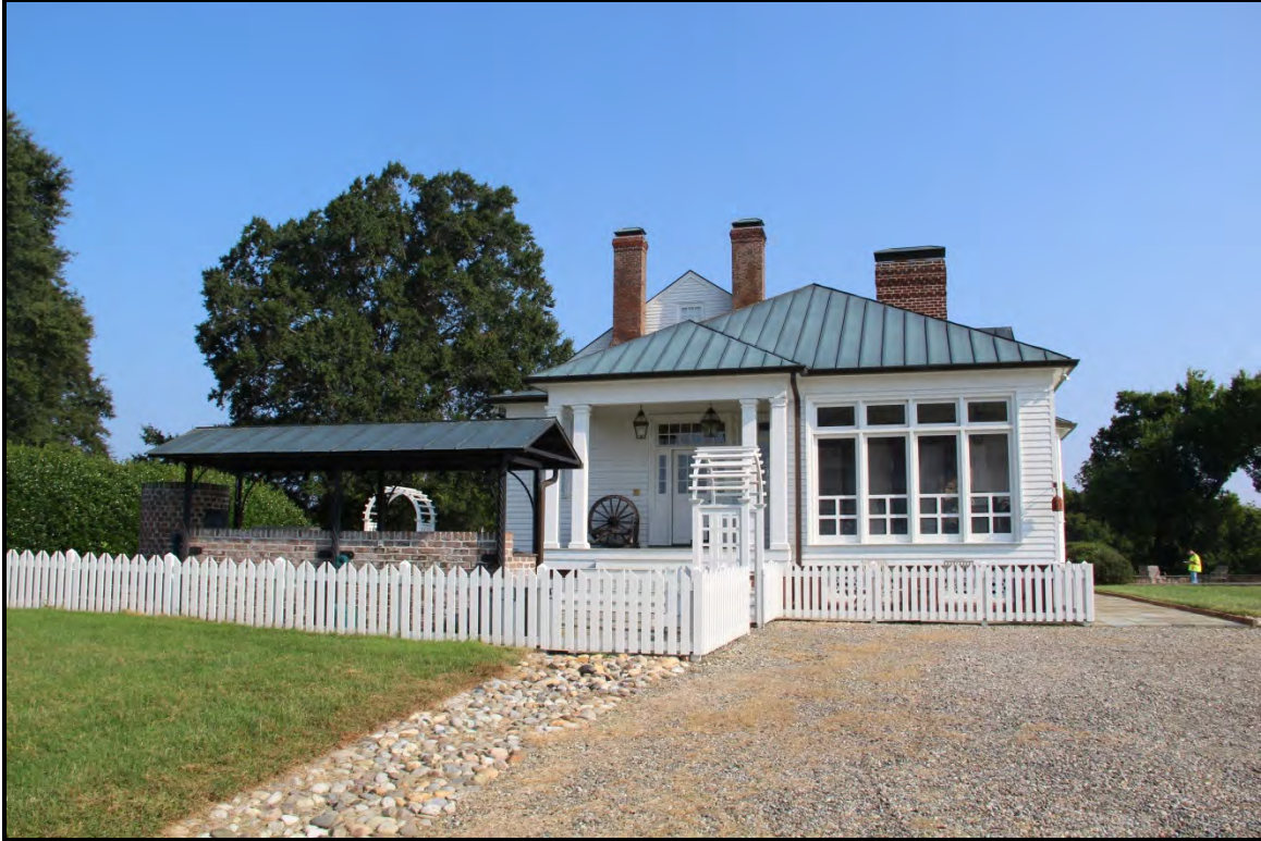
Figure 5.23. Willow Oaks Plantation House; view is north featuring the south elevation wing.
