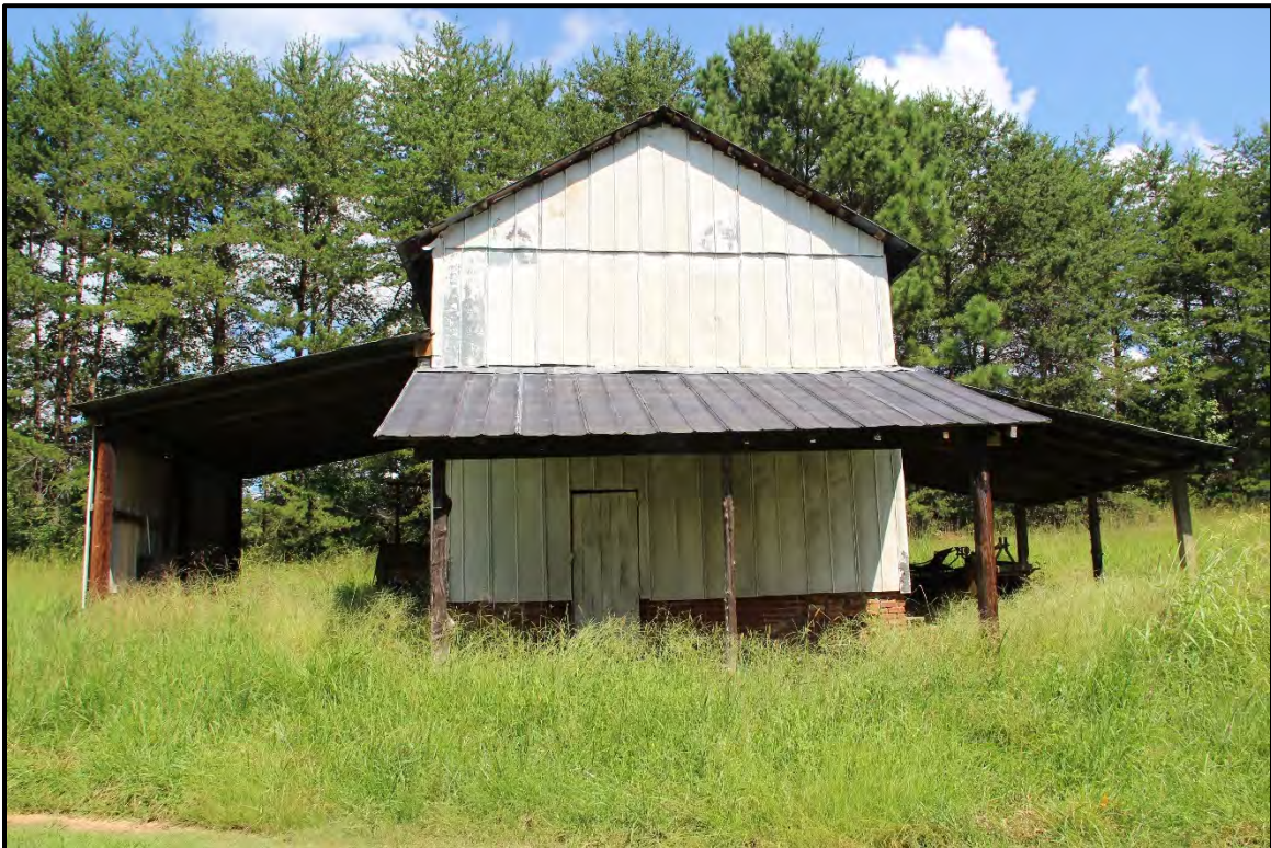
Figure 6.116. Architectural resource AM2523; view is north featuring “Tobacco Barn B”.
