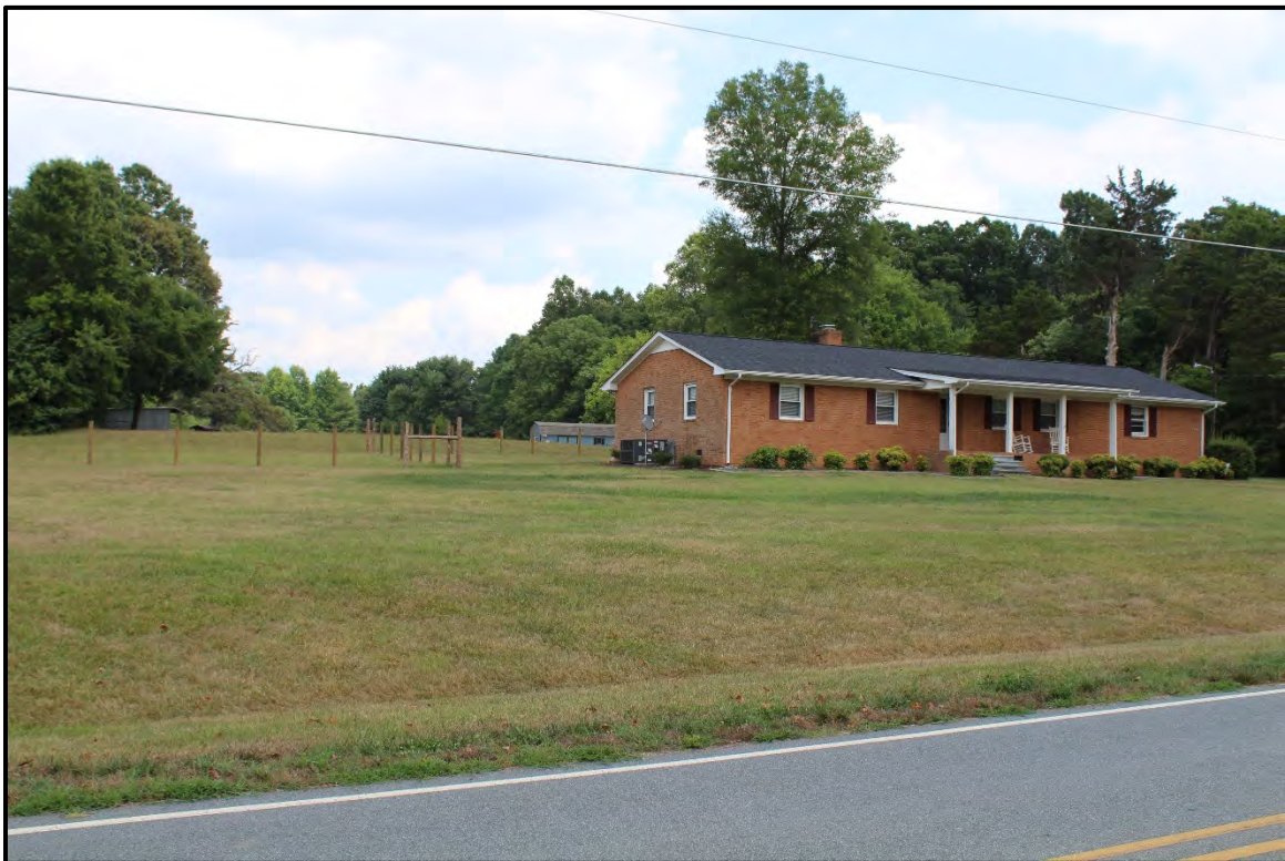
Figure 6.157. Architectural resource AM2553; view is southeast featuring the façade and northwest elevation.
