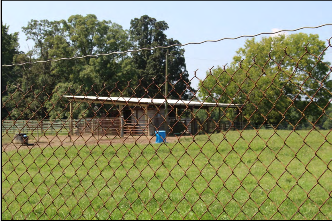
Figure 5.6. Architectural resource RK1655; view is southwest featuring the modern pole shed.
