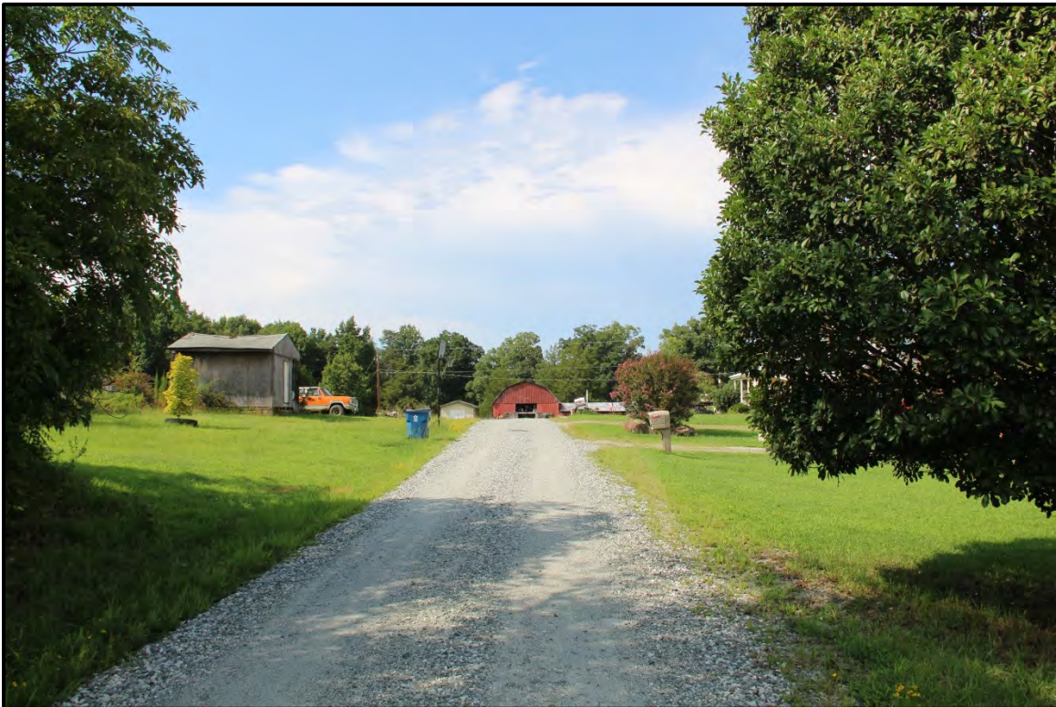
Figure 6.77. Architectural resource AM2509; view is north featuring the gambrel-roof barn and storage shed.
