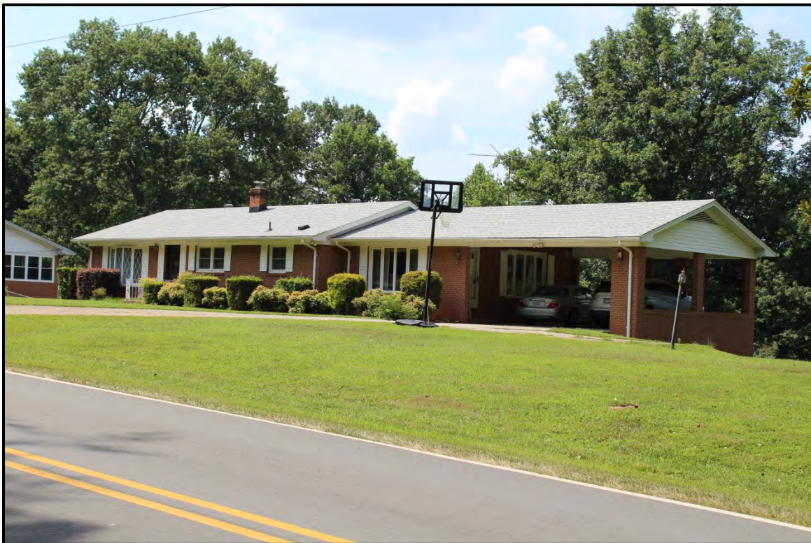
Figure 5.202. Architectural resource RK1737; view is northwest and features the façade and east elevation.
