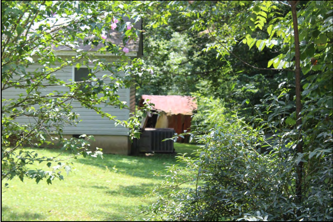
Figure 5.67. Architectural resource RK1671; view is southeast featuring the wood-frame outbuilding.
