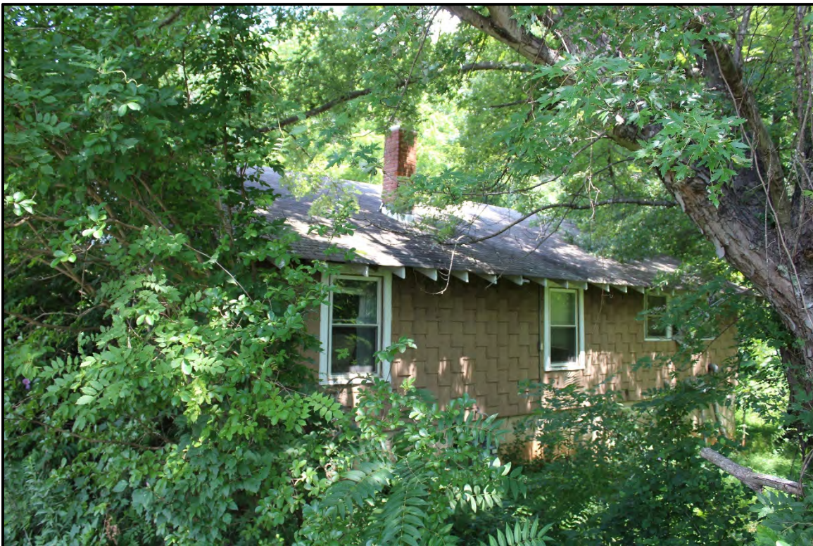
Figure 5.177. Architectural resource RK1721; view is north featuring the southeast elevation.
