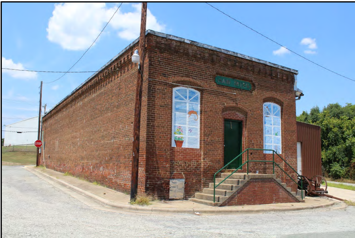
Figure 6.207. Architectural resource AM2596; view is northeast and features the south and west elevations.
