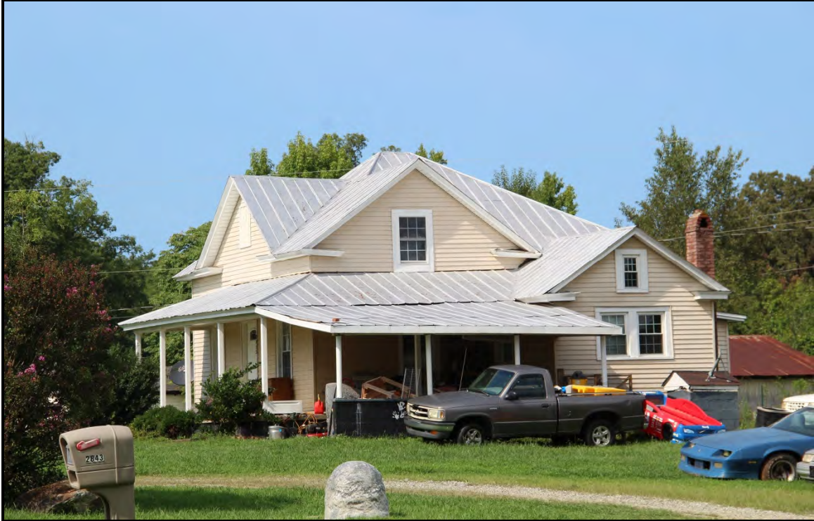
Figure 6.76. Architectural resource AM2509; view is southeast showing the façade and north elevation.
