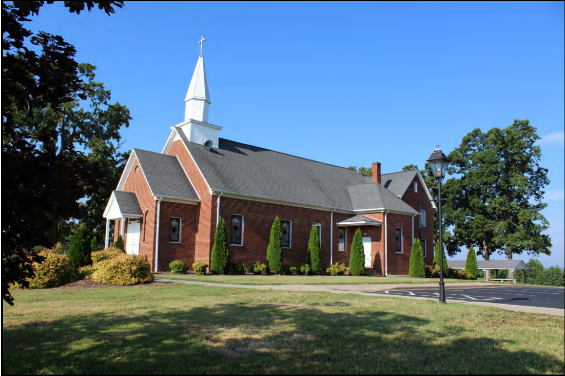
Figure 6.25. Architectural resource AM1523; oblique view showing east façade and north elevation.
