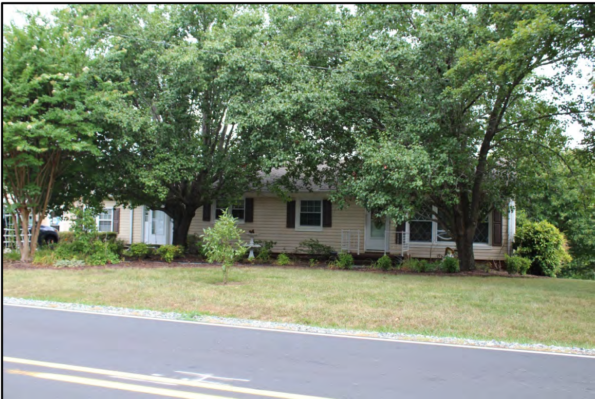
Figure 6.280. Architectural resource AM2608; view is northwest and features the façade.
