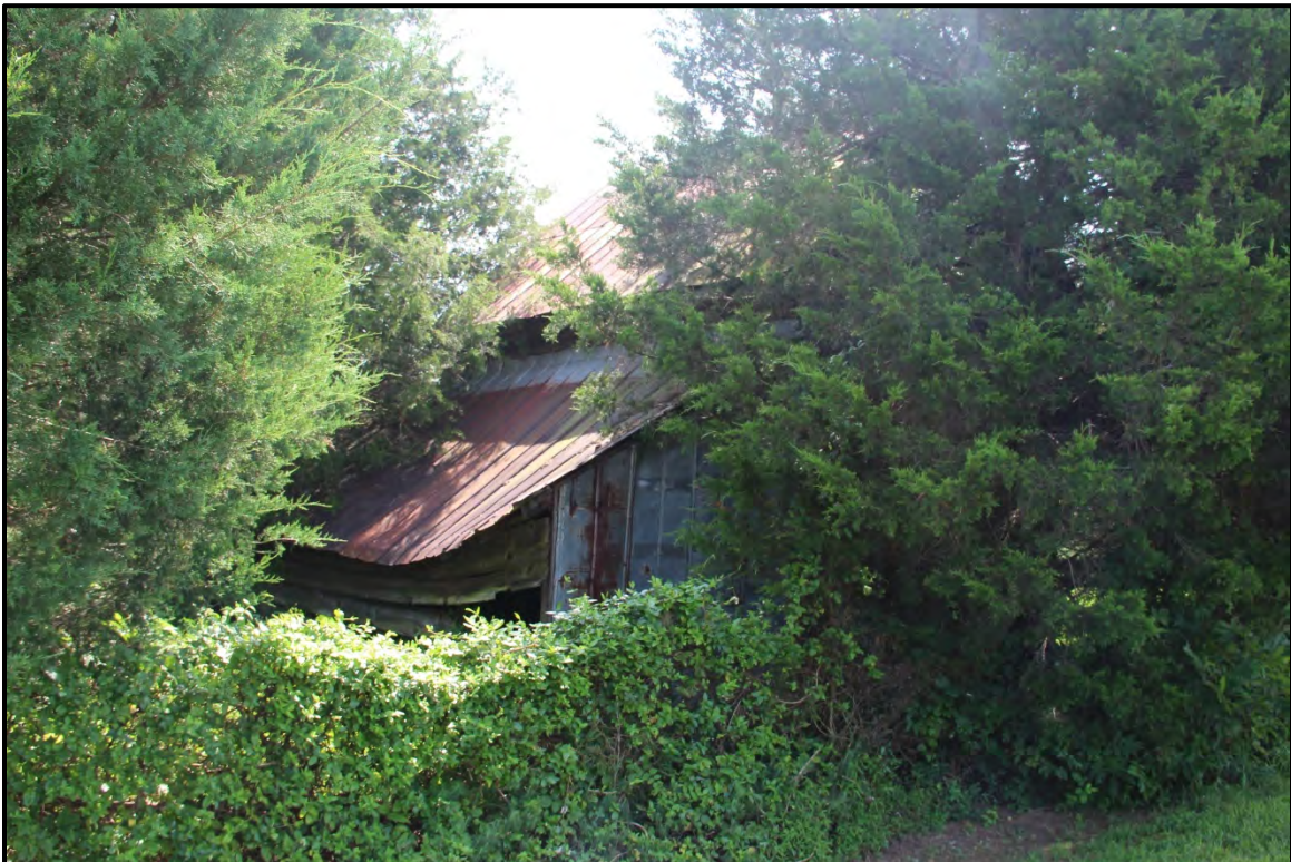
Figure 6.112. Architectural resource AM2520; view is southeast featuring the barn.
