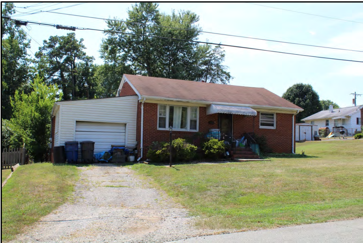
Figure 6.184. Architectural resource AM2580; view is northwest featuring the façade.
