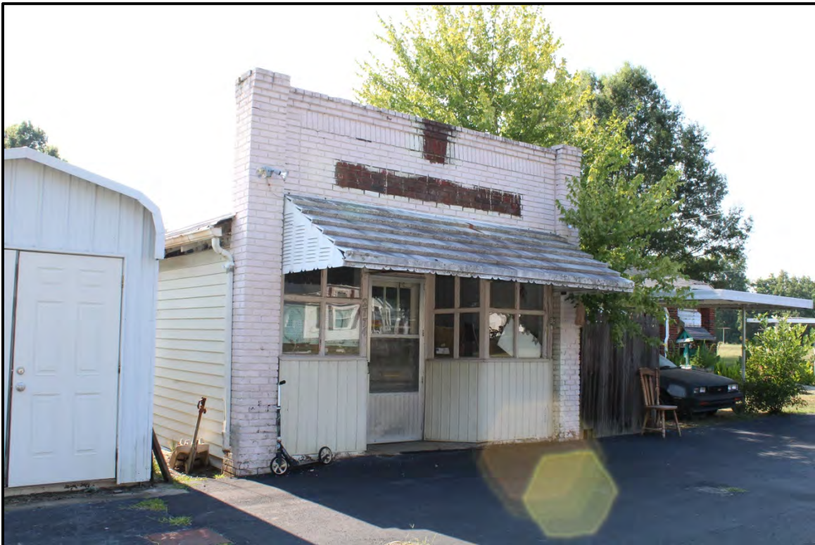
Figure 6.127. Architectural resource AM2532; view is northwest featuring the associated commercial building.
