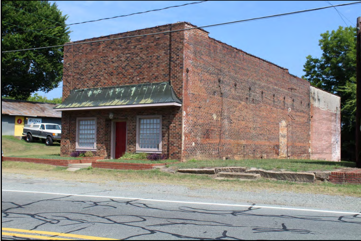
Figure 6.203. Architectural resource AM2592; oblique view featuring the façade and southeast elevation.
