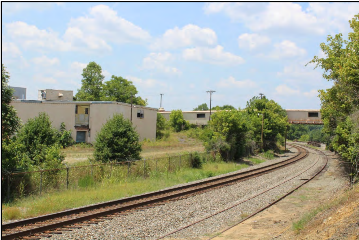
Figure 6.272. Architectural resource AM2603; view is west from architectural resource AM1516.
