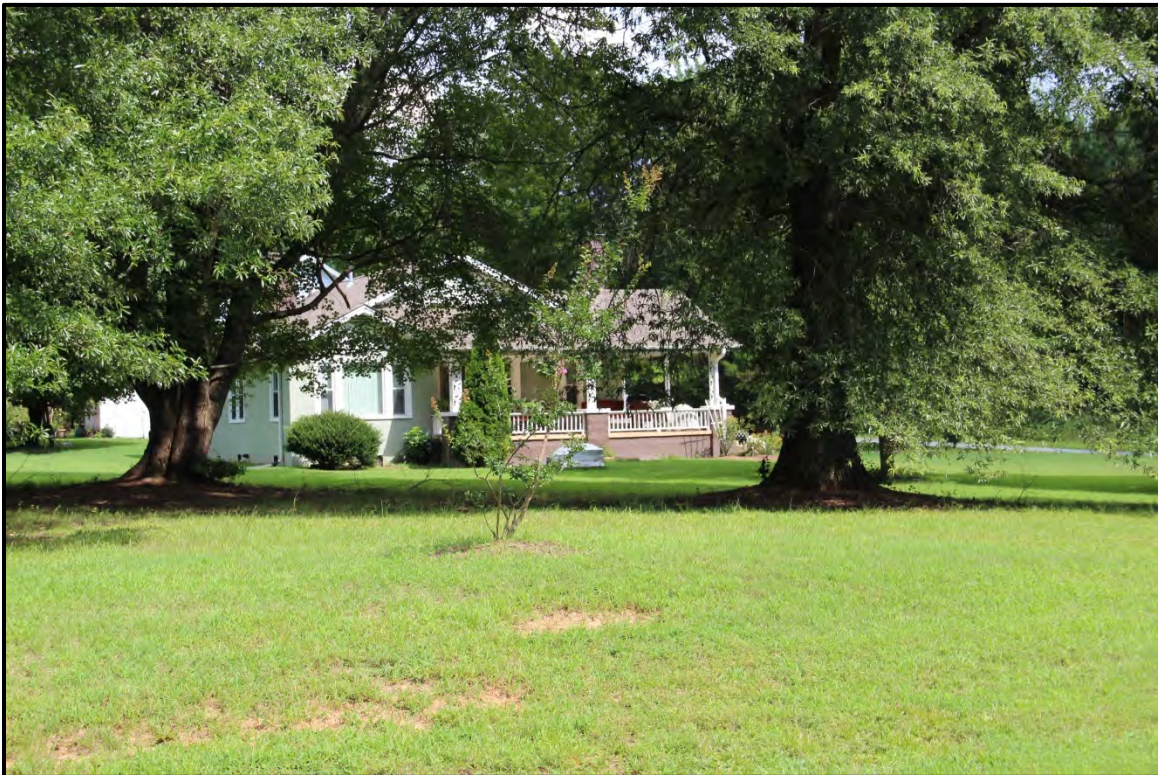
Figure 6.70. Architectural resource AM2505; view is east featuring the façade and north elevation.
