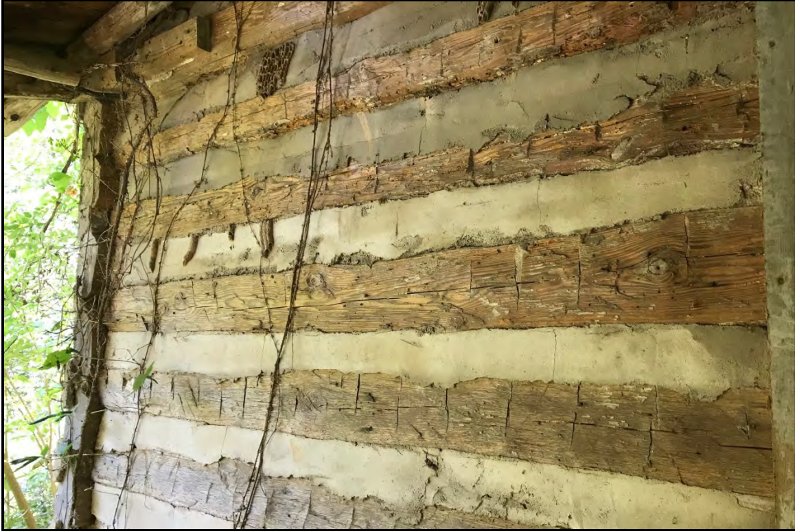
Figure 5.13. Architectural resource RK1656; hewn logs along the southwest (rear) elevation.
