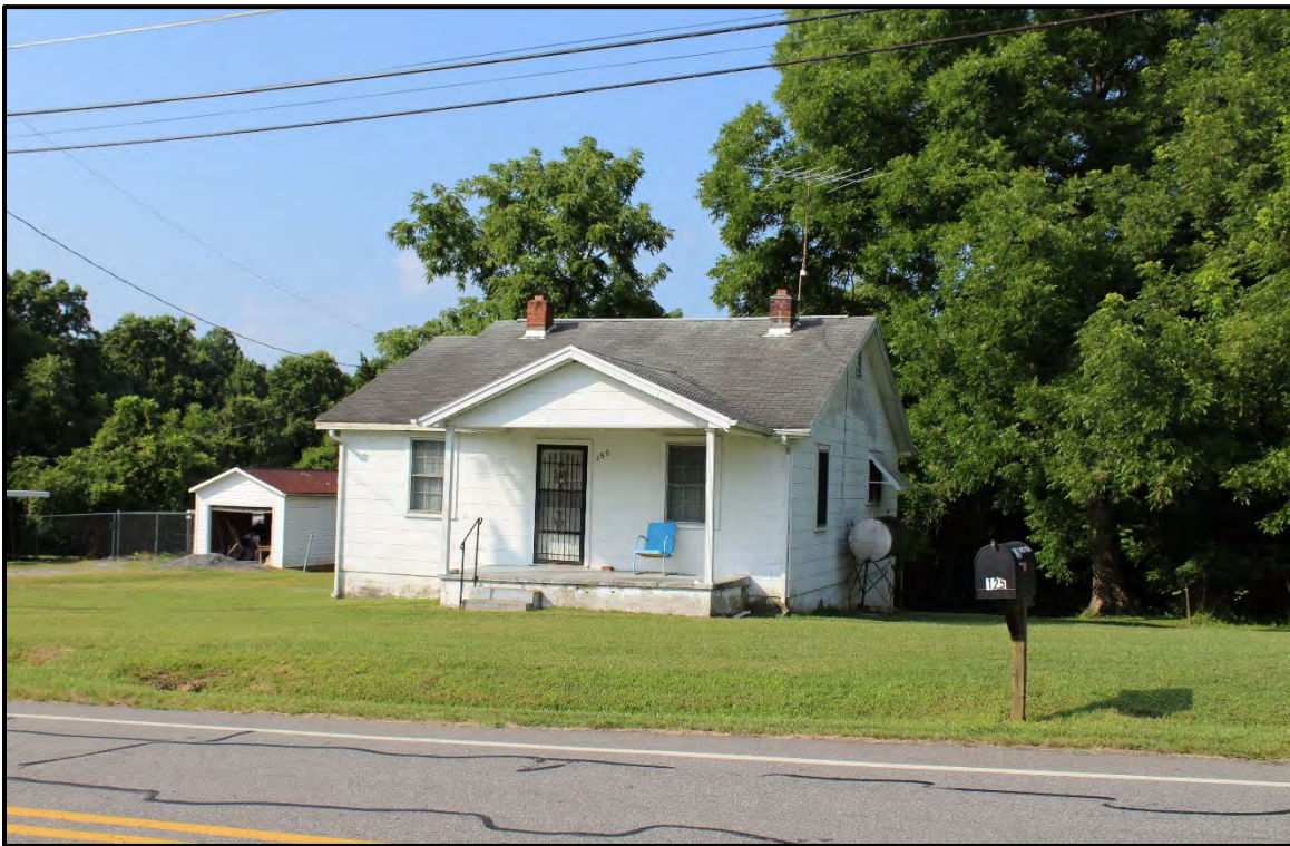
Figure 5.158. Architectural resource RK1706; view is southwest featuring the façade and northwest elevation.
