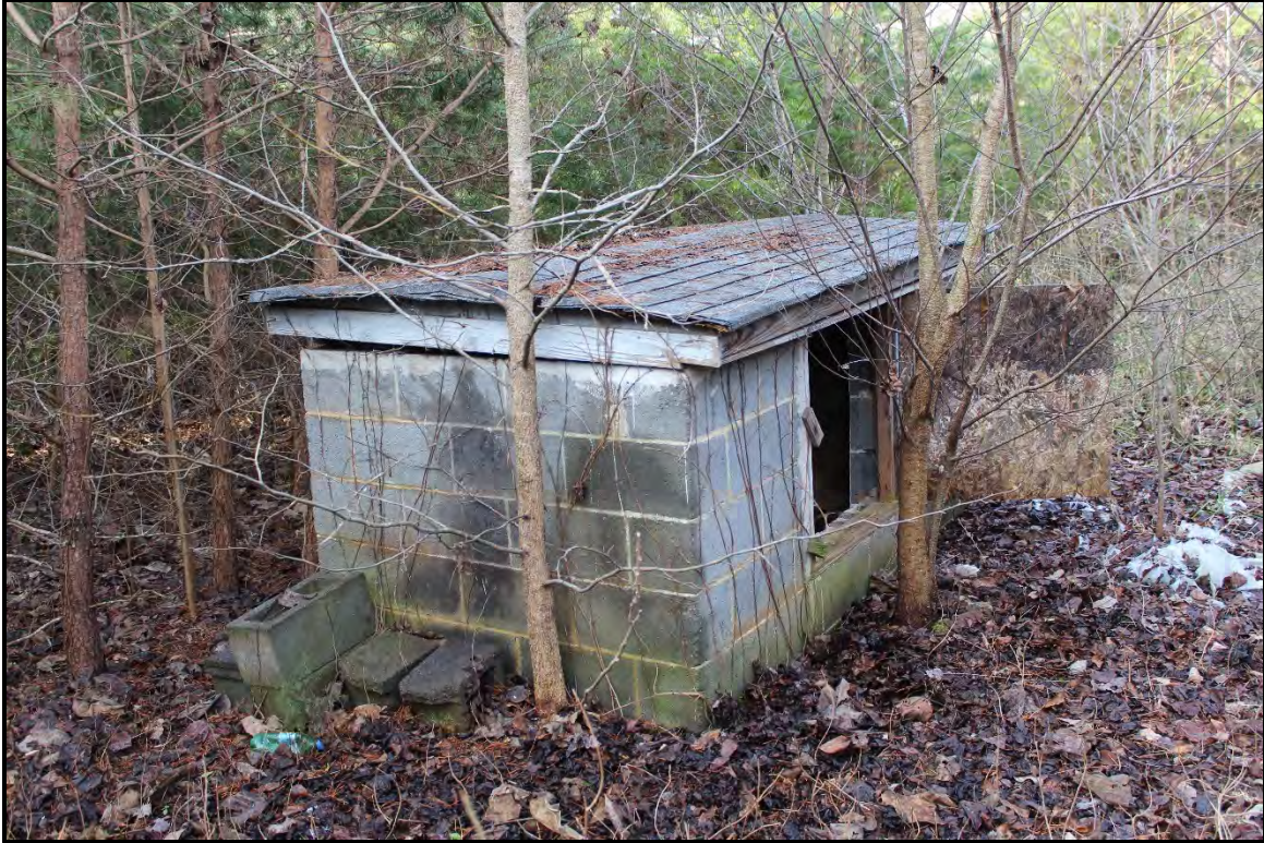
Figure 6.4. Architectural resource AM1520; view is southwest featuring the water pump shed.
