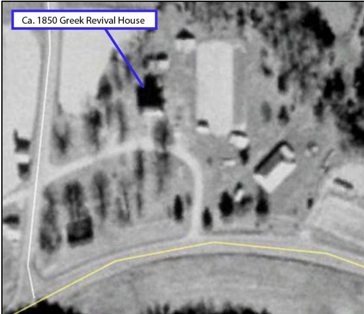
Figure 5.229. 1999 aerial imagery of RK1534 depicting the ca. 1850 Greek Revival residence and associated outbuildings.
