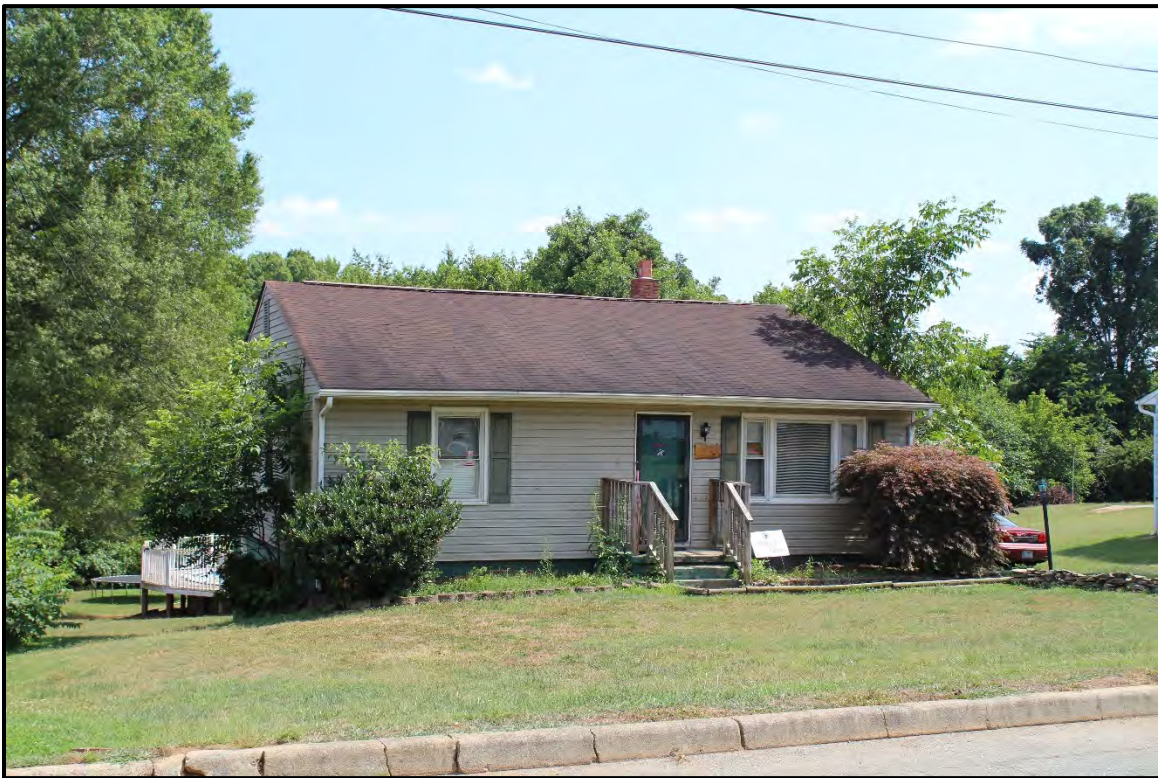
Figure 6.168. Architectural resource AM2564; view is south featuring the façade.
