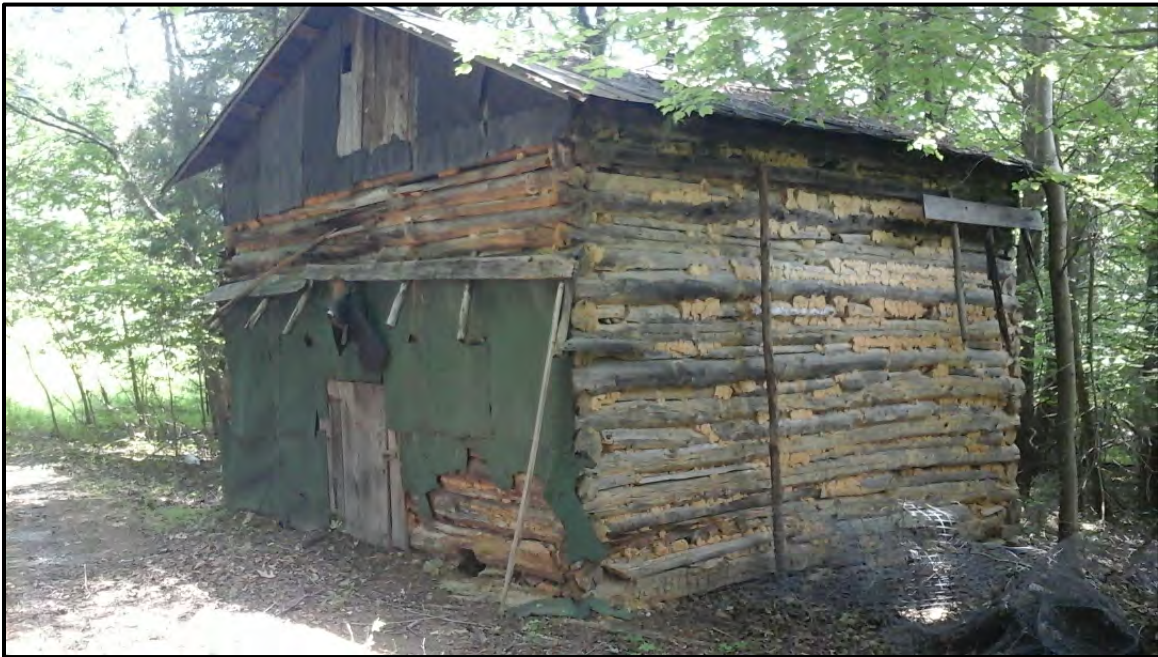
Figure 5.81. Architectural resource RK1676; view is of the primary and side elevations.
