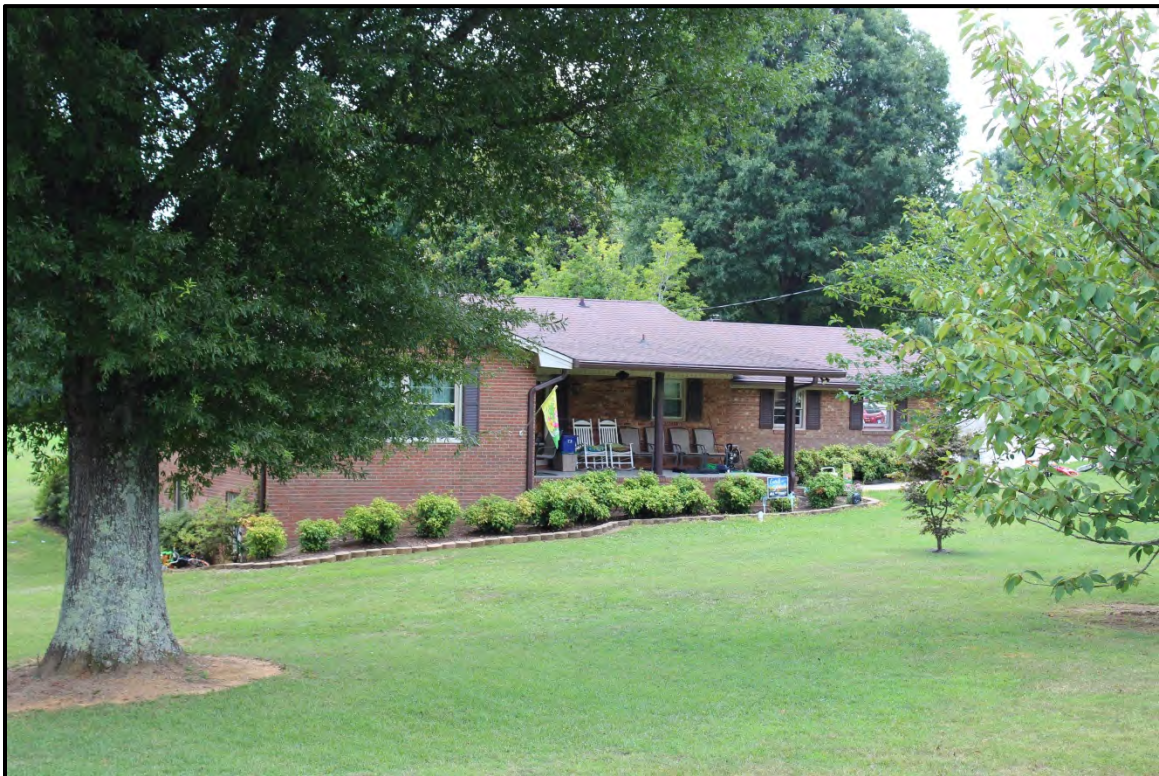
Figure 5.169. Architectural resource RK1716; view south featuring the façade.
