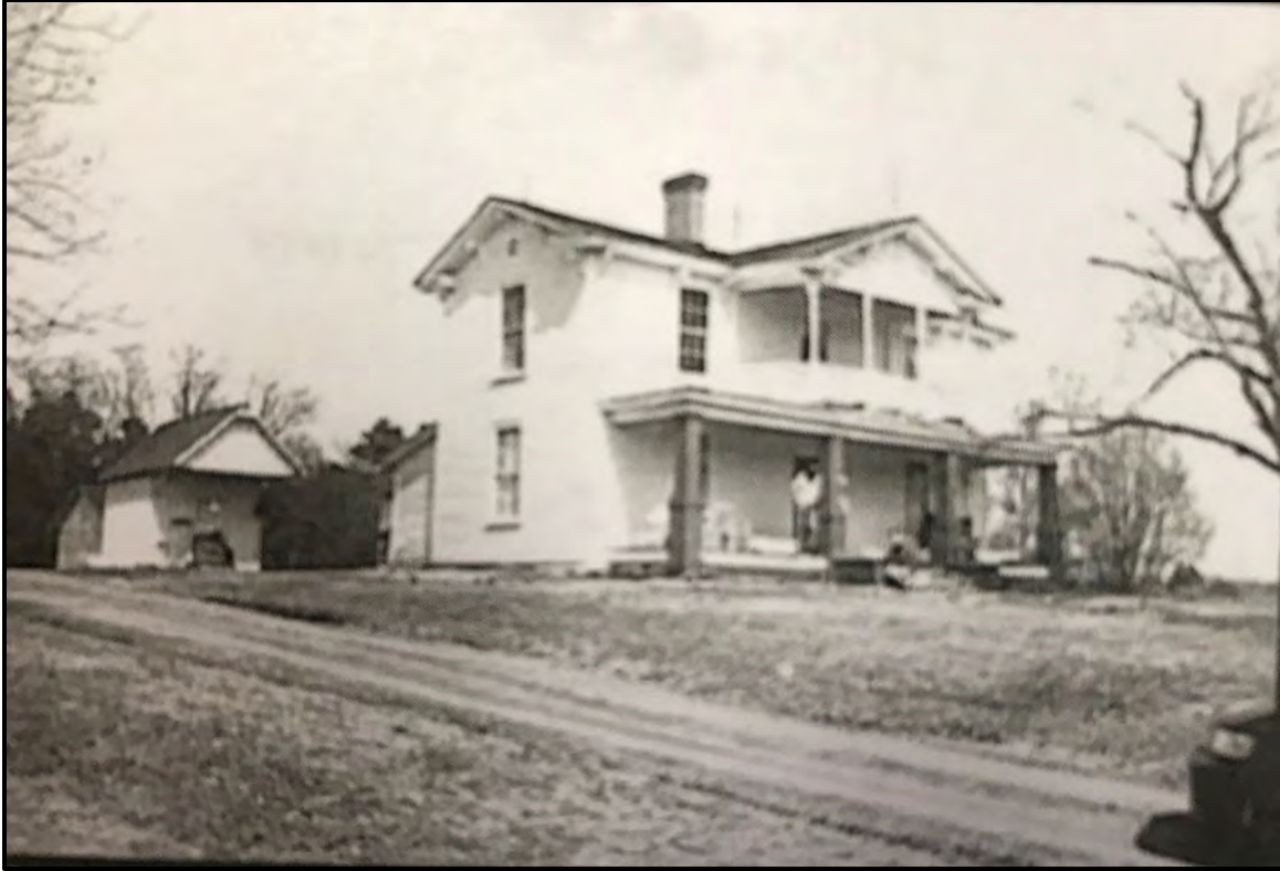
Figure 6.136. 2002 photo of AM0122 featuring the ca. 1885 Folk Victorian house (Barkhau 2002c).
