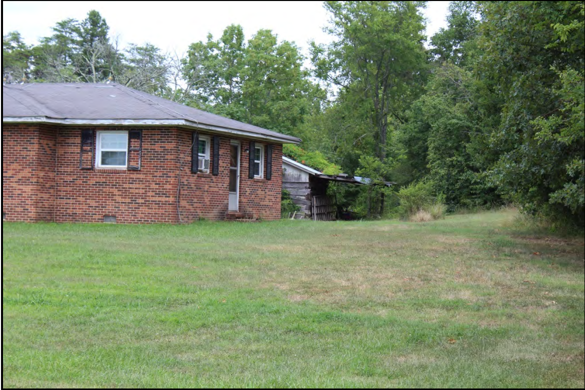
Figure 5.249. Architectural resource RK1754; view is north and features the log barn.
