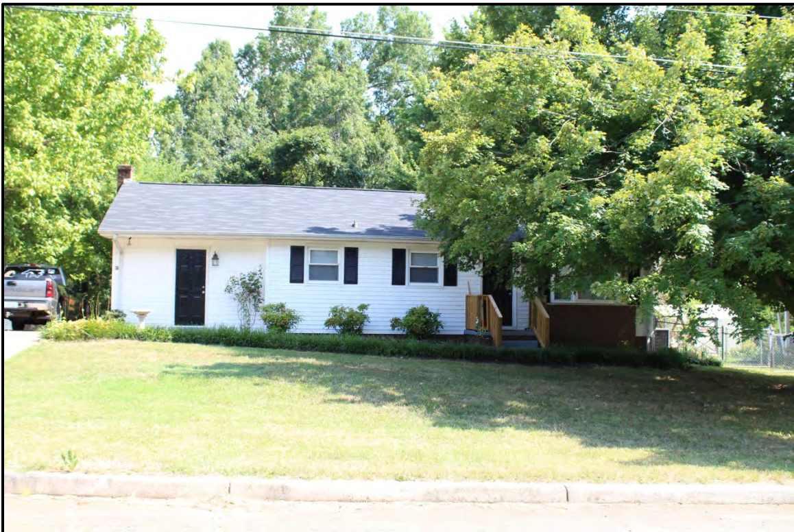
Figure 6.163. Architectural resource AM2559; view is southeast featuring the façade.
