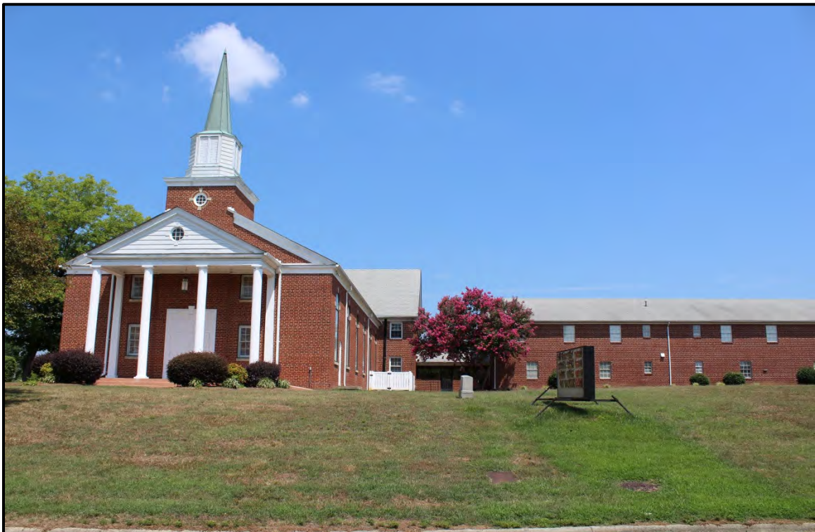
Figure 6.189. Architectural resource AM2585; view is northwest featuring the façade.
