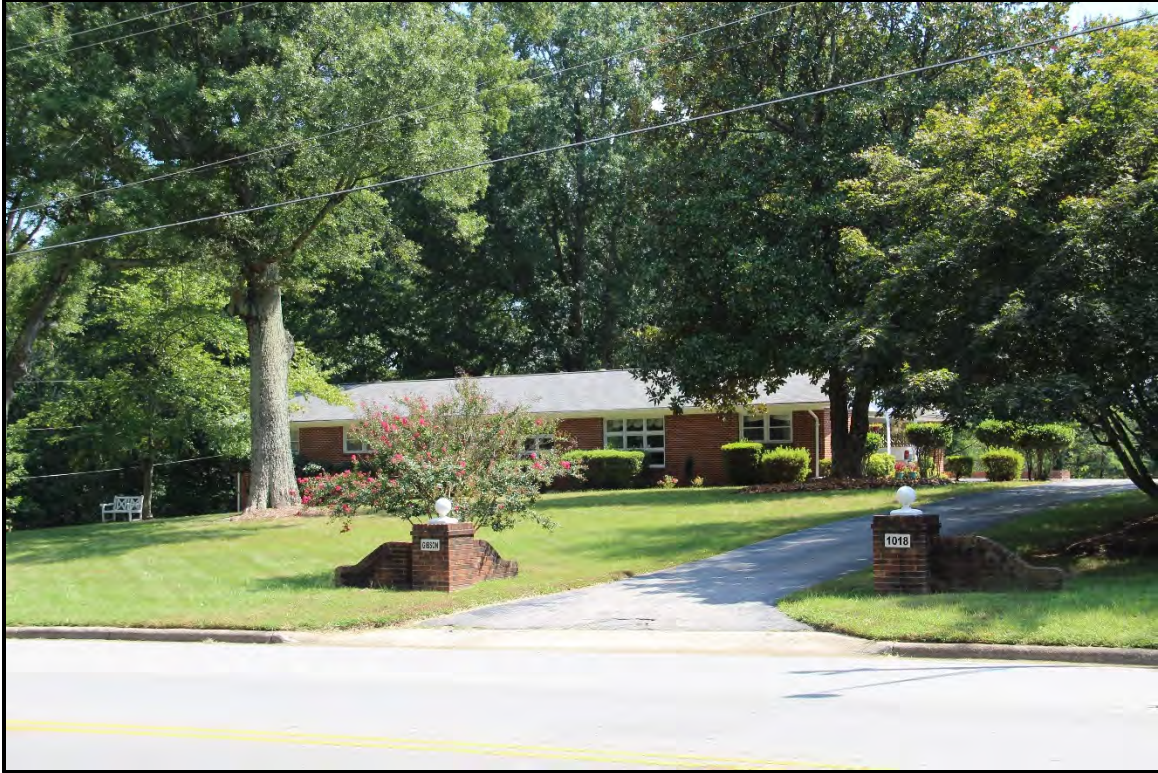
Figure 5.329. Architectural resource RK1773; view is southeast featuring the façade and west elevation.
