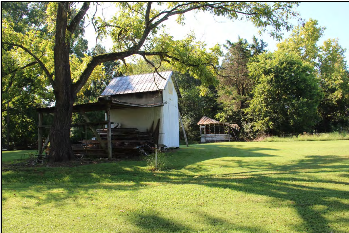
Figure 6.89. Architectural resource AM2514; view is southwest featuring the tobacco barn and partially collapsed chicken house in the background.
