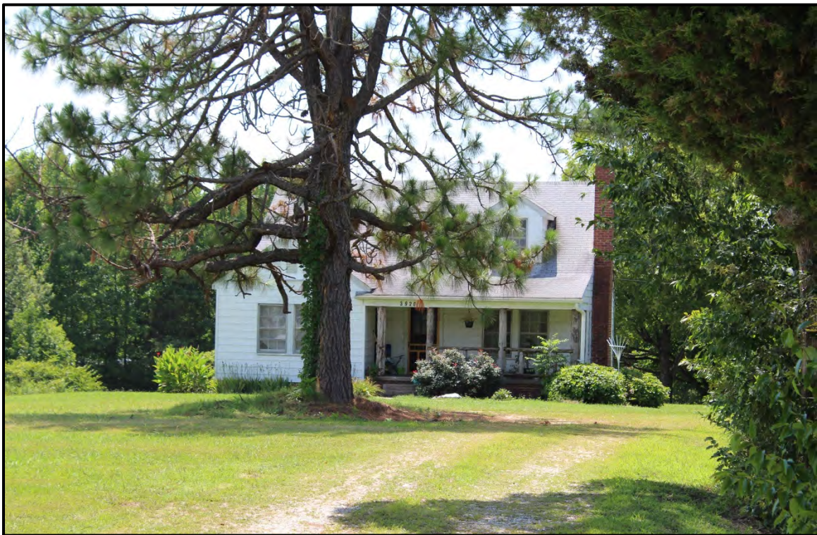
Figure 6.59. Architectural resource AM2502; view is west featuring the façade.
