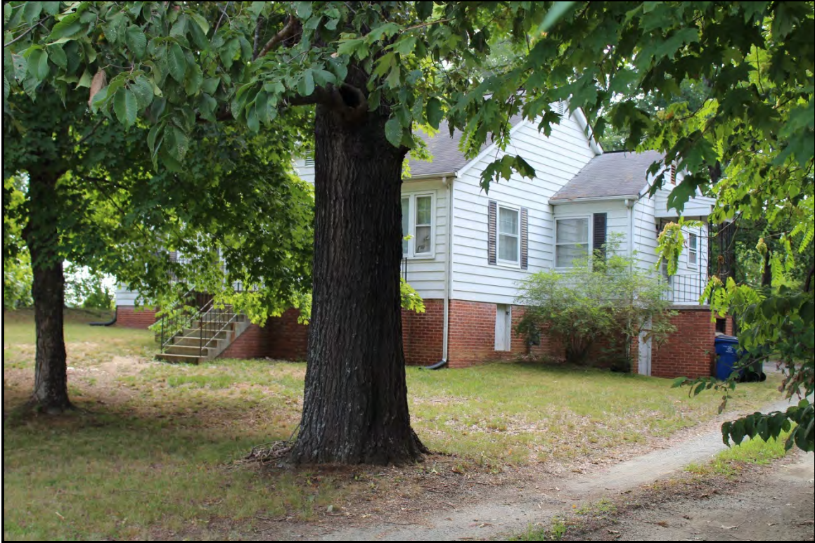
Figure 6.278. Architectural resource AM2605; view is northeast and features the façade and south elevation.
