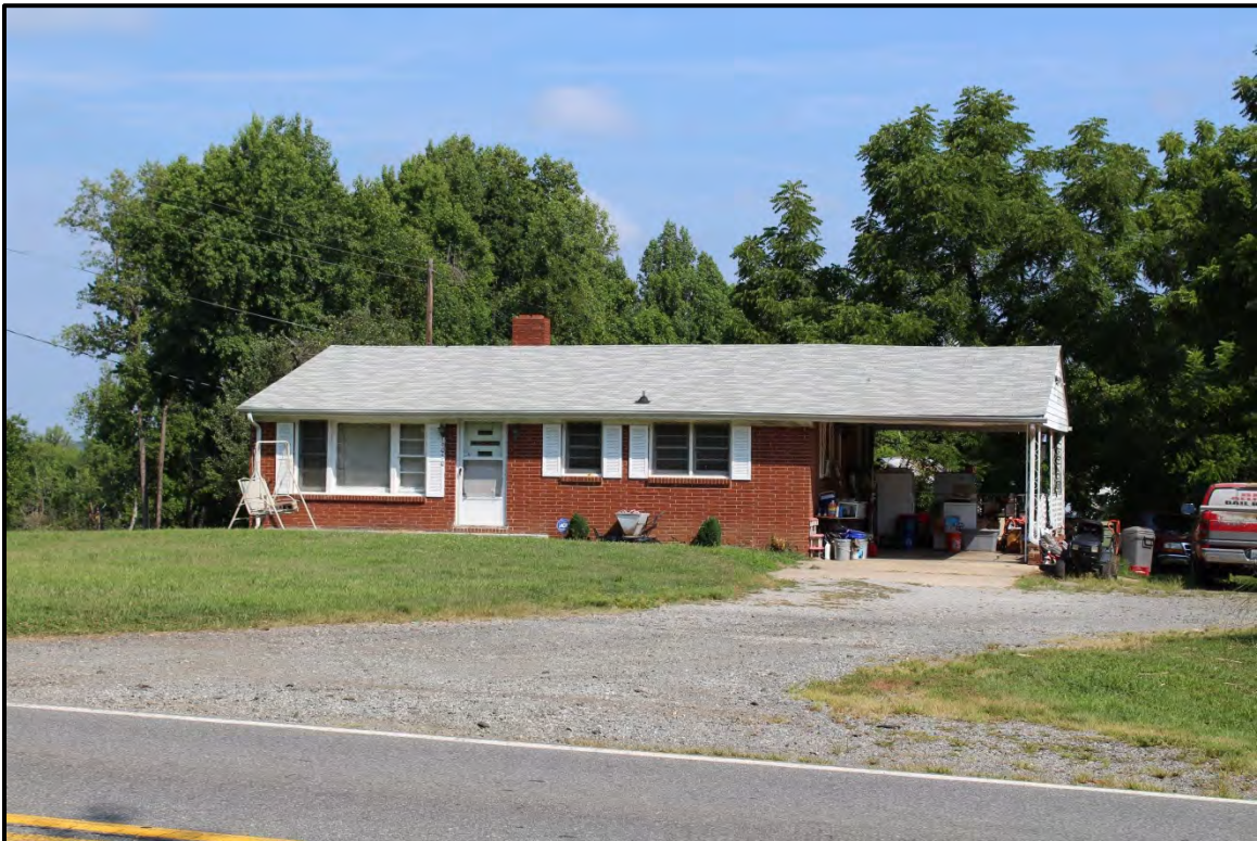
Figure 5.128. Architectural resource RK1696; view is northwest featuring the façade and carport.
