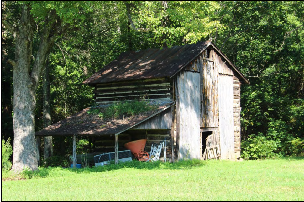
Figure 6.68. Architectural resource AM2504; view of log barn.
