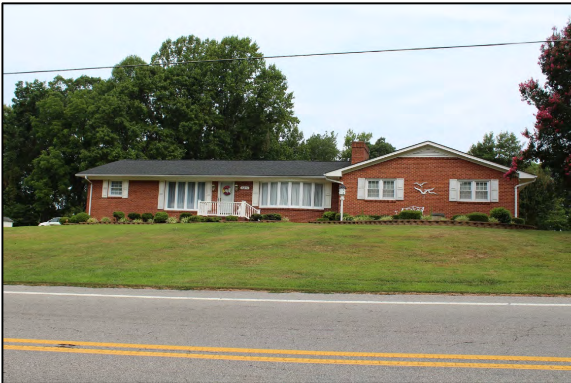
Figure 5.191. Architectural resource RK1729; view is northwest featuring the façade.
