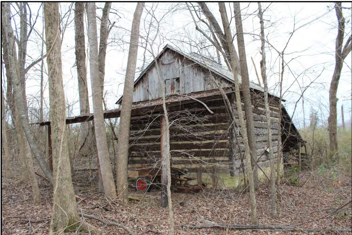
Figure 5.277. RK1758 tobacco barn #1; view is southwest featuring the façade and northeast elevation.
