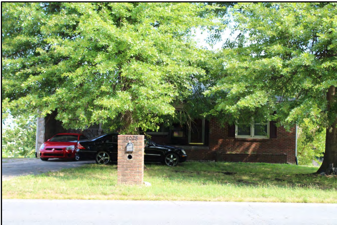
Figure 5.126. Architectural resource RK1695; view is northwest featuring the façade.
