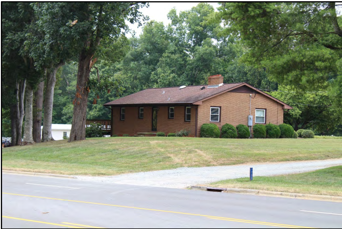
Figure 6.290. Architectural resource AM2615; view is southeast and features the façade and west elevation.
