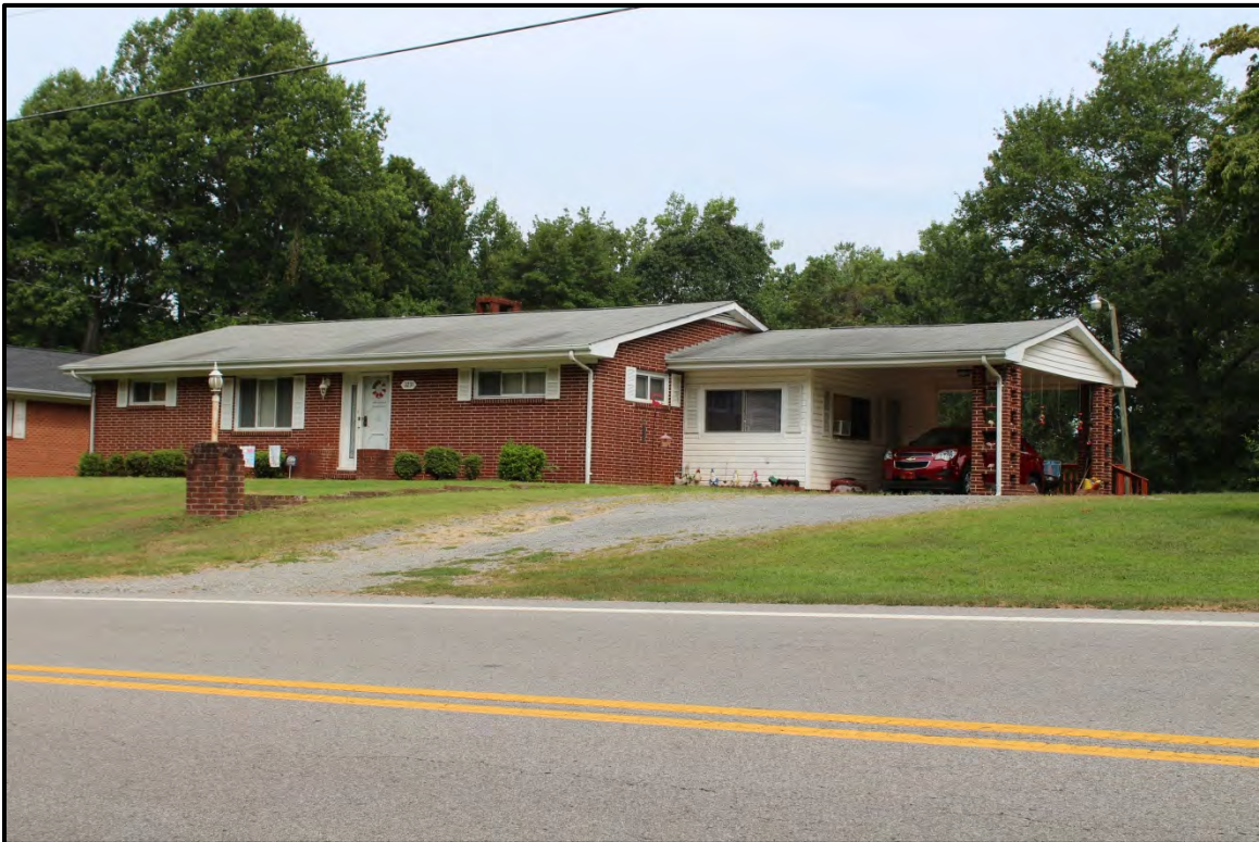
Figure 5.192. Architectural resource RK1730; view is northwest featuring the façade and attached carport on the northeast elevation.
