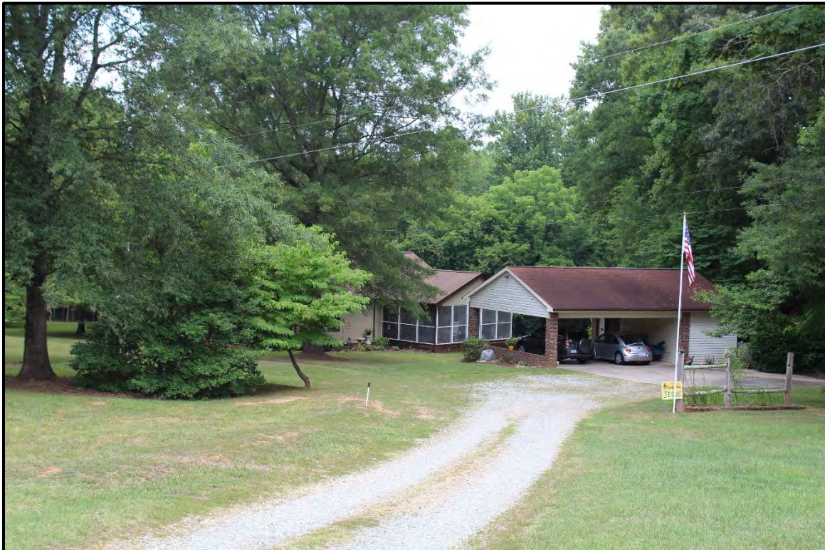
Figure 6.158. Architectural resource AM2554; view is northwest featuring the porch (southeast) elevation and the carport.
