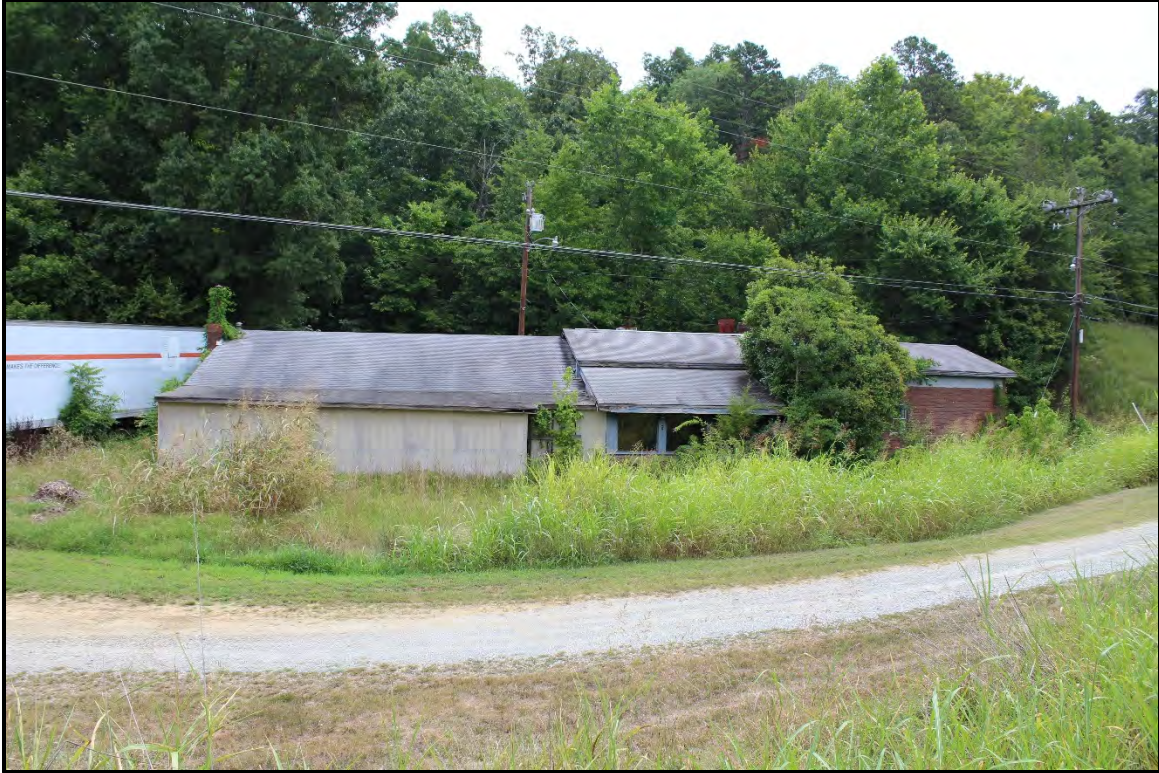
Figure 6.285. Architectural resource AM2611; view is northeast and features the west elevation.
