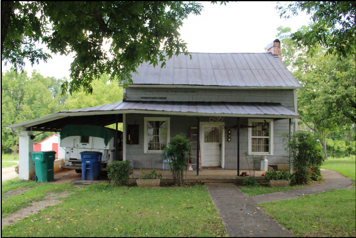
Figure 5.213. Architectural resource RK1741; view is north and features the façade.
