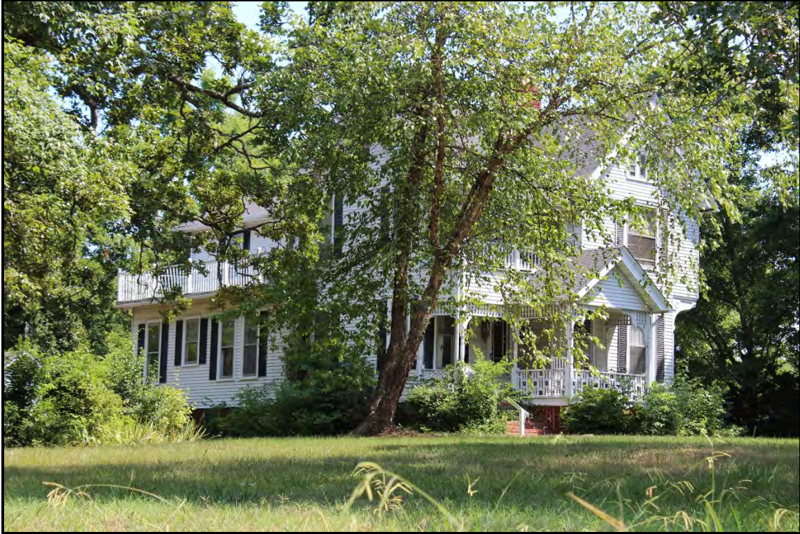
Figure 6.259. Architectural resource AM0350; view is northeast featuring the façade and the west northeast elevation.
