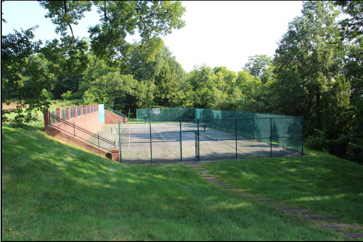
Figure 5.29. Willow Oaks Plantation House; view is north featuring the modern tennis courts.
