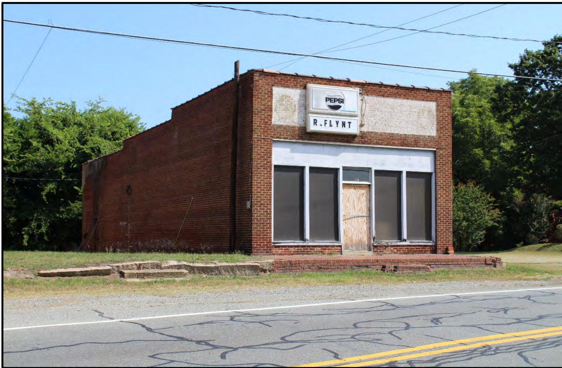
Figure 6.200. Architectural resource AM2590; view is northeast featuring the façade and southwest elevation.
