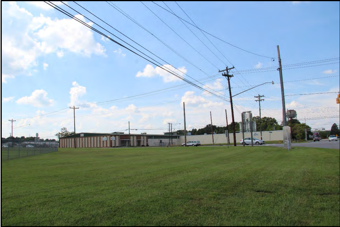
Figure 5.346. Architectural resource RK1780; view is northwest featuring the façade and south elevations of the 1960 plant building with the associated warehouse and loading bay additions.
