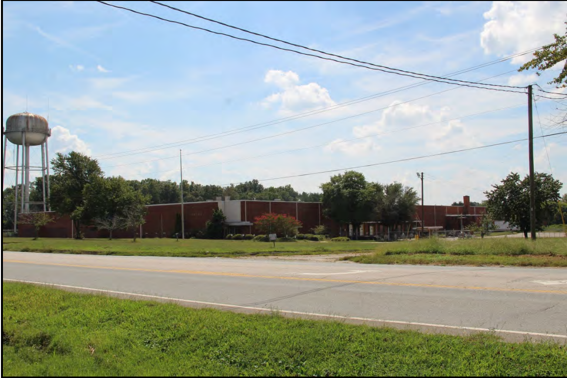
Figure 5.335. Architectural resource RK1776; view is southwest featuring the primary façade, the north elevation loading bays, and the water tank.
