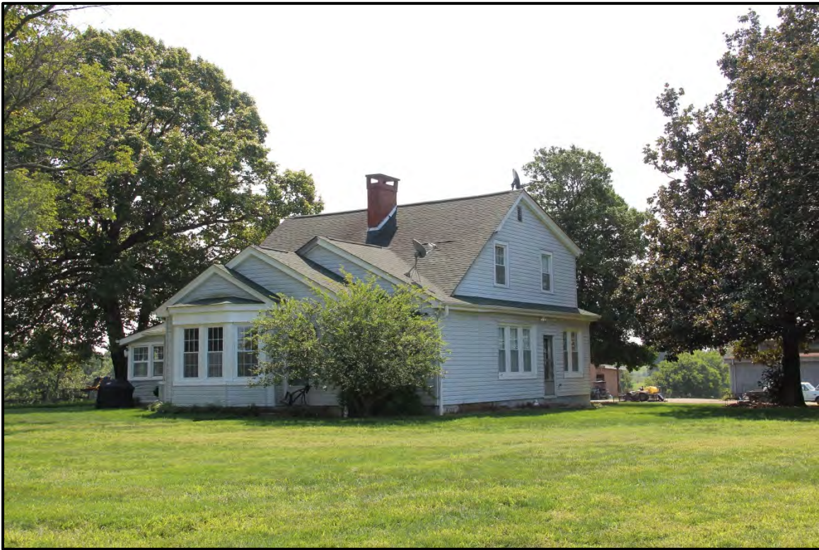
Figure 5.3. Architectural resource RK1655; view is southeast featuring the façade and west elevation.
