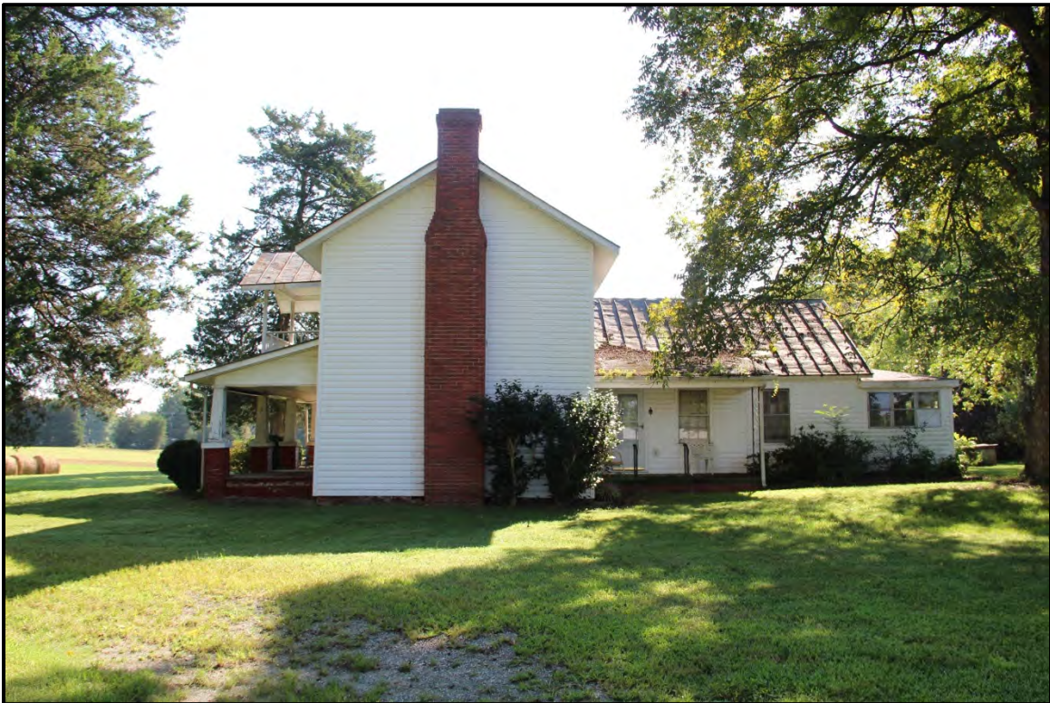
Figure 6.85. Architectural resource AM2514; view is east featuring the west elevation and rear ell.
