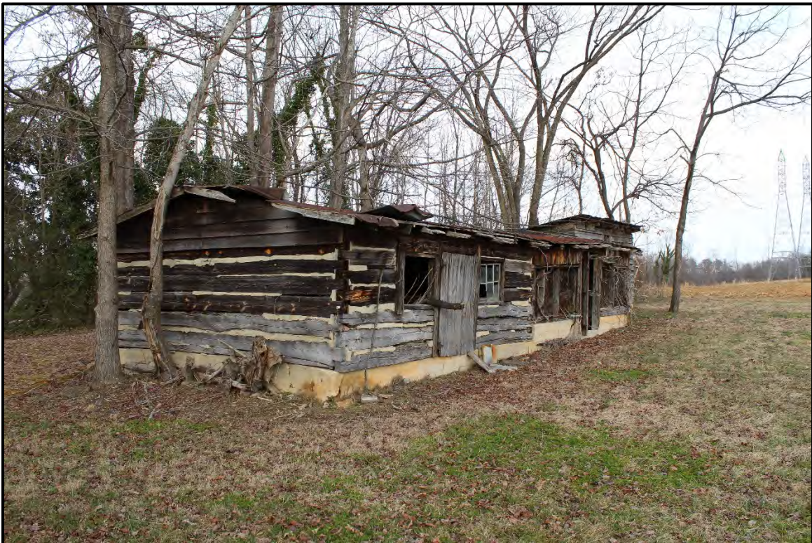
Figure 5.263. RK1758 chicken houses; view is northeast featuring the façade and southwest elevation.
