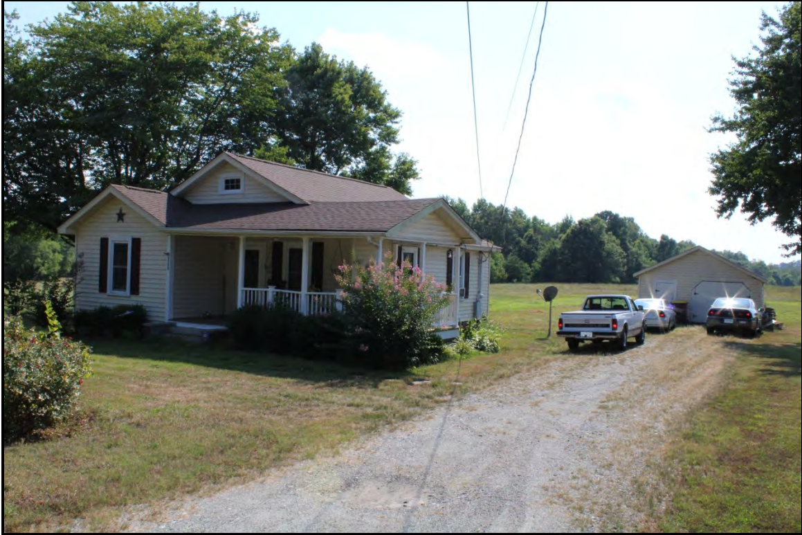
Figure 6.131. Architectural resource AM2616; view is southwest featuring the façade and north elevation.
