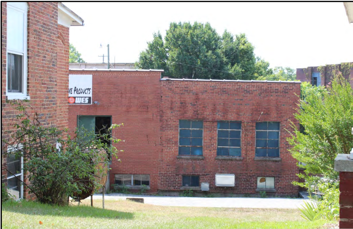
Figure 6.195. Architectural resource AM2588; view is southeast featuring a portion of the northwest elevation of the commercial building.
