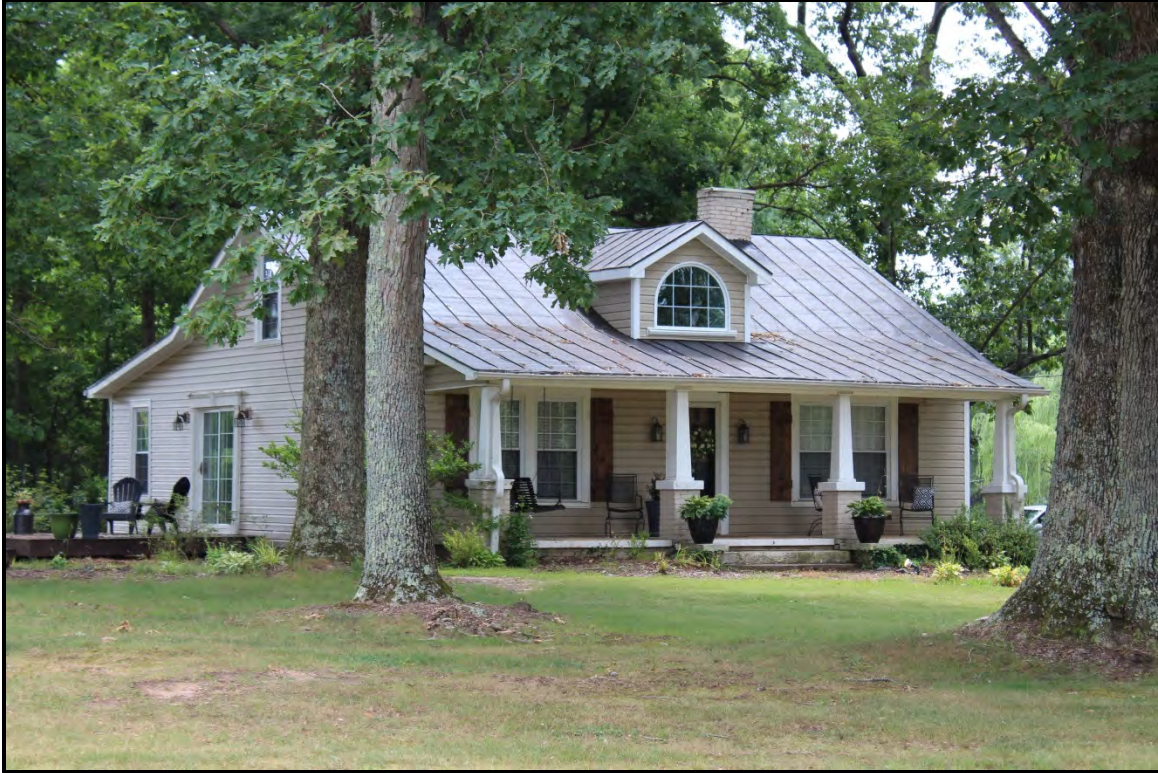
Figure 5.233. Architectural resource RK1746; view is south and features the façade and northeast elevation.
