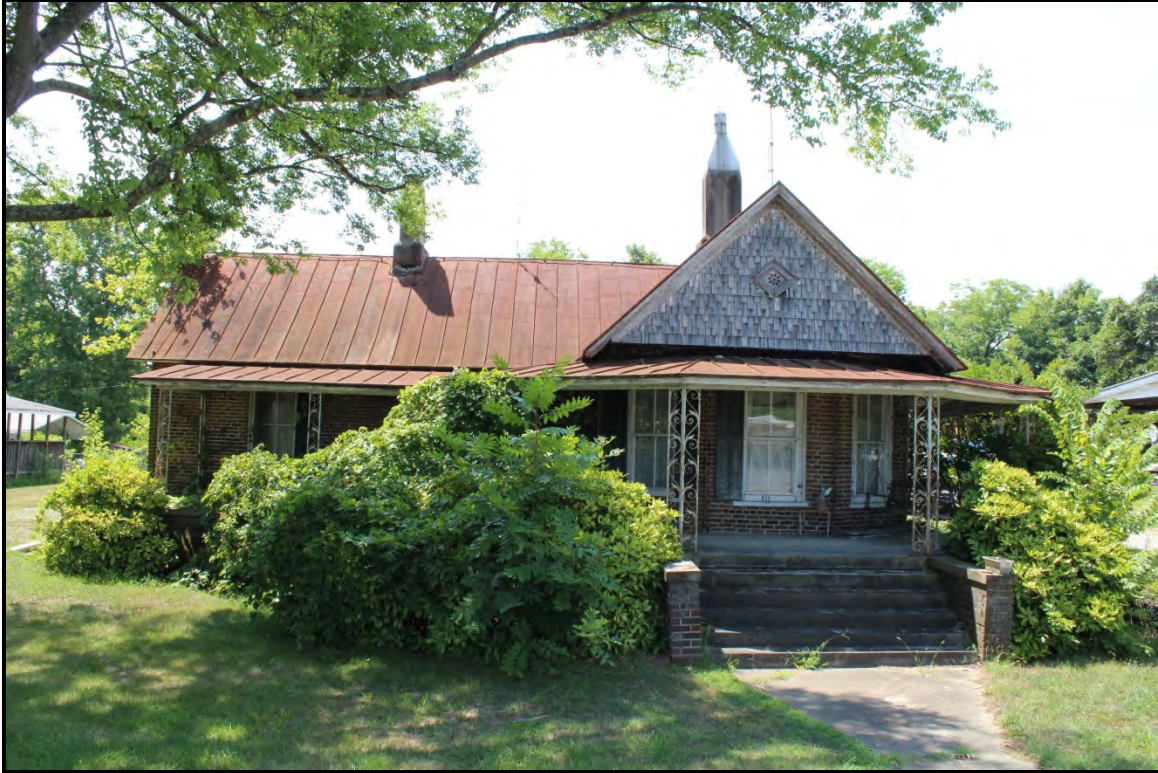
Figure 6.268. Architectural resource AM2601; view is south and features the façade.
