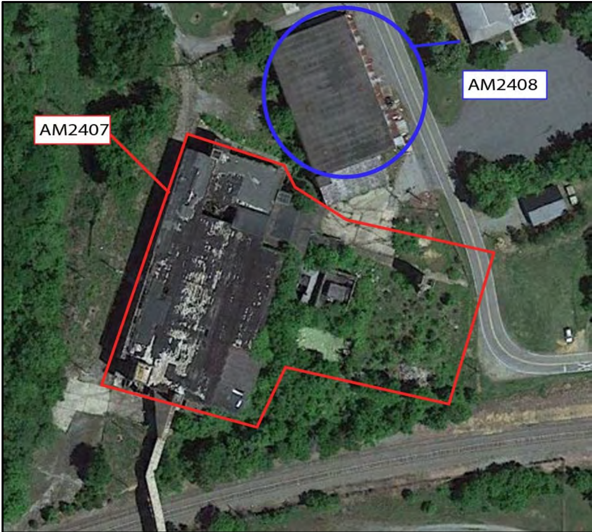
Figure 6.249. 2017 aerial image of Cora Mill showing the results of recent demolition of the associated warehouses (image courtesy of Google Earth).
