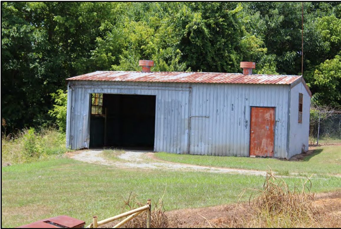
Figure 6.274. Architectural resource AM2604; view is southwest and features the maintenance garage.
