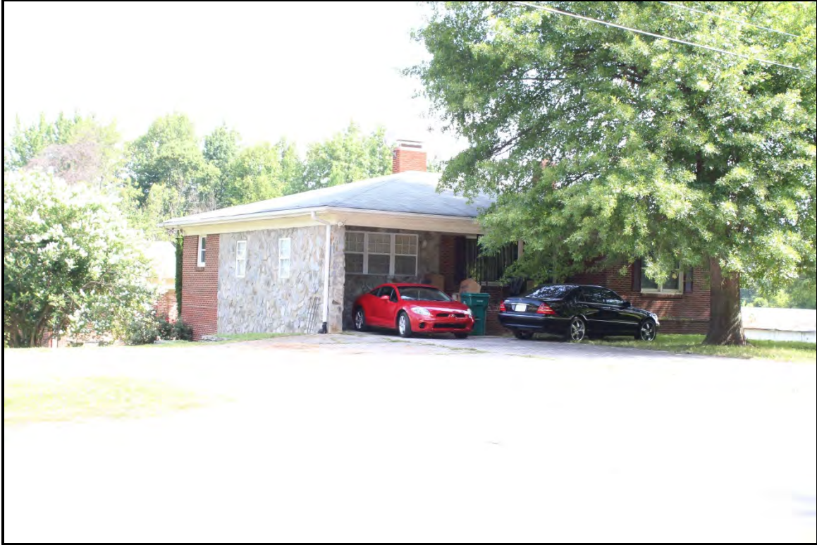
Figure 5.127. Architectural resource RK1695; view is northeast featuring the façade and southwest elevation.
