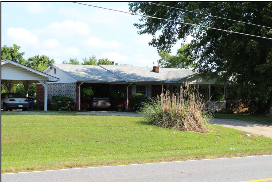
Figure 5.134. Architectural resource RK1697; view is northeast featuring the attached and detached carports.
