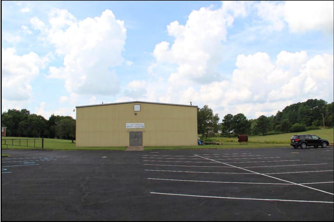
Figure 5.320. Architectural resource RK1770; view is west featuring the ca. 1970 activity building.
