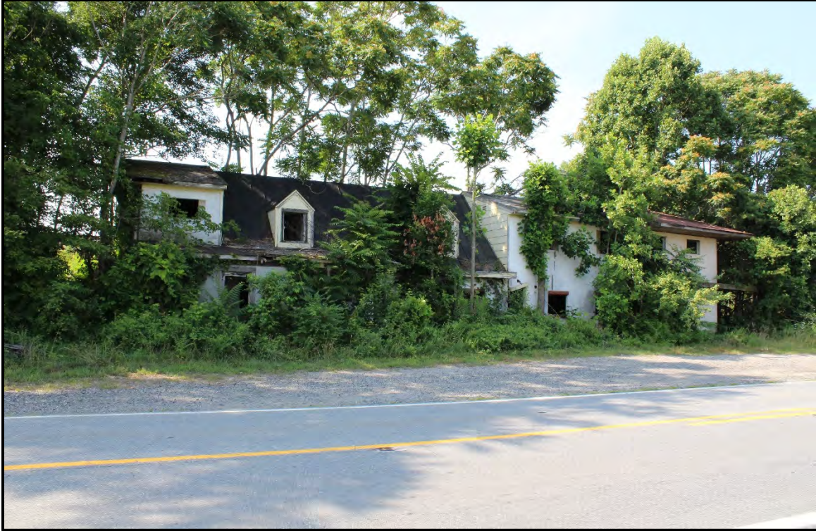
Figure 5.142. Architectural resource RK1702; view is southwest featuring the façade.
