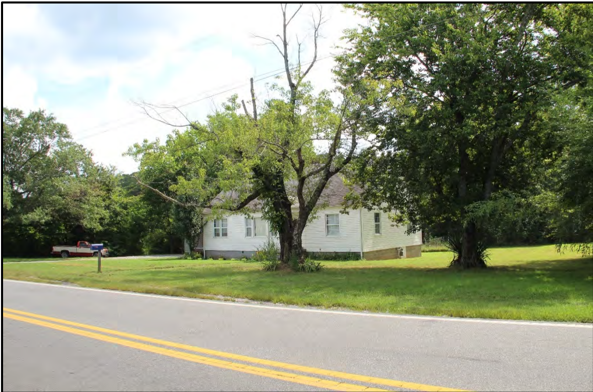
Figure 5.323. Architectural resource RK1771; view is southeast featuring the façade and west elevation.
