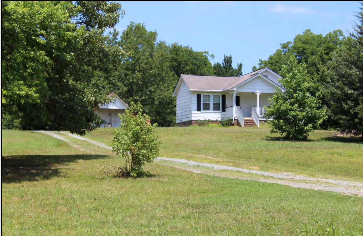
Figure 6.137. Architectural resource AM0122; view is north featuring the 1948 Minimal Traditional house and the early twentieth century well house.
