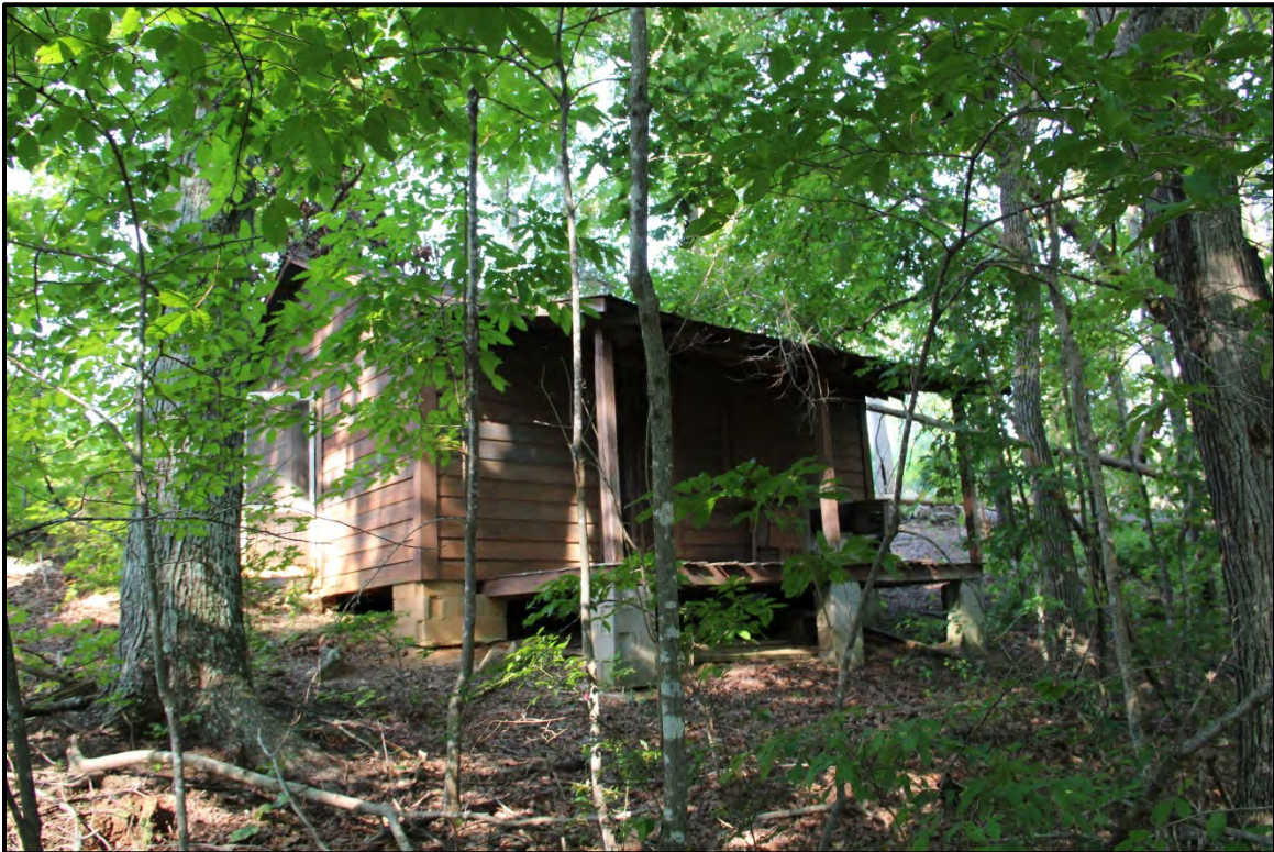
Figure 5.118. Architectural resource RK1688; view is northwest featuring the ca. 1960 cabin.
