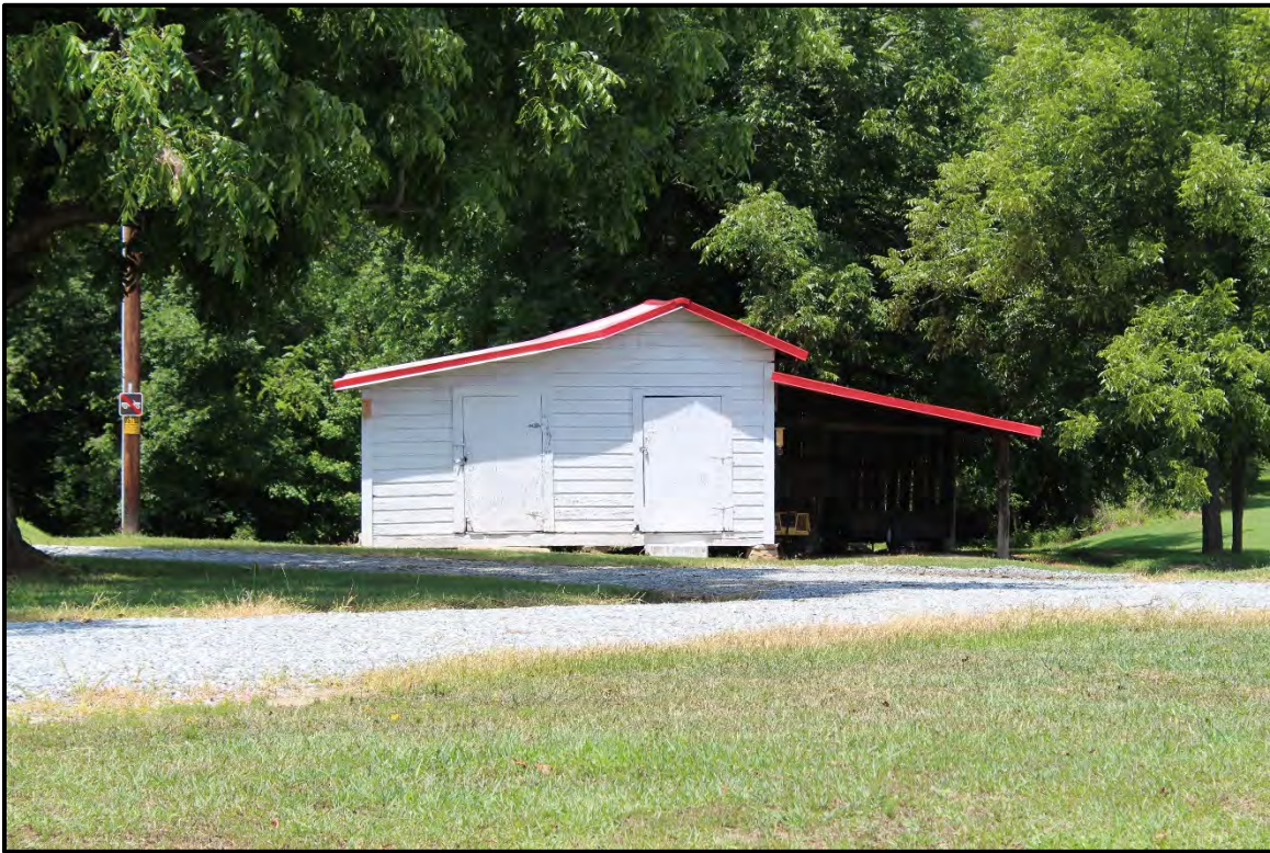
Figure 6.140. Architectural resource AM2540; view is north featuring the shed outbuilding.
