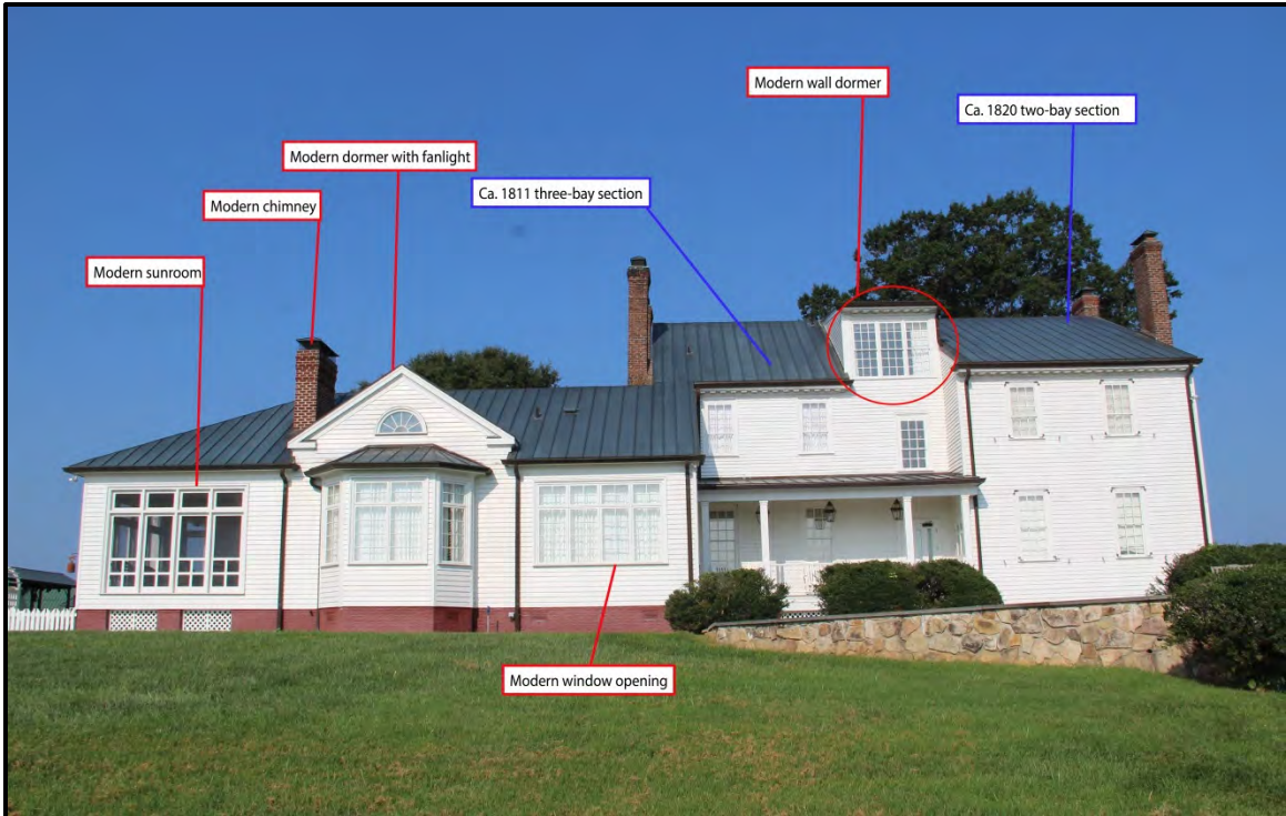
Figure 5.21. Willow Oaks Plantation House; view is west featuring the east (rear) elevation depicting the location of the house's building episodes and modern alterations.
