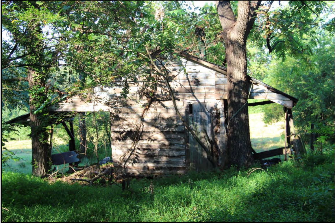
Figure 5.292. Architectural resource RK1759; view is southwest and features the utility building.
