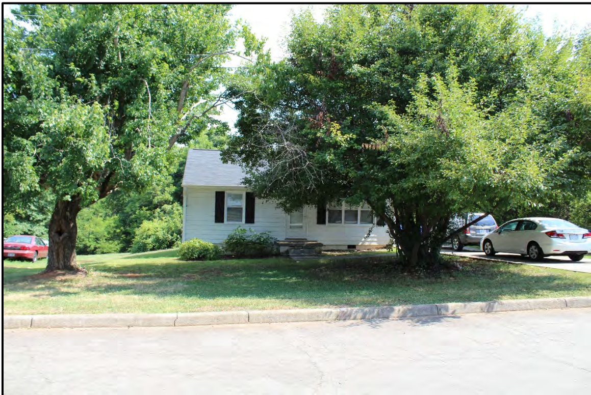
Figure 6.167. Architectural resource AM2563; view is southeast featuring the façade.
