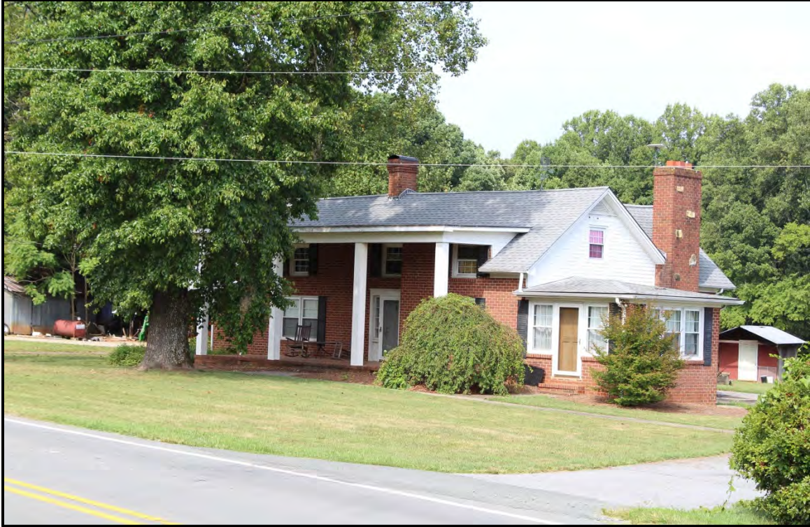
Figure 6.94. Architectural resource AM2516; view is southwest and features the façade and north elevation.
