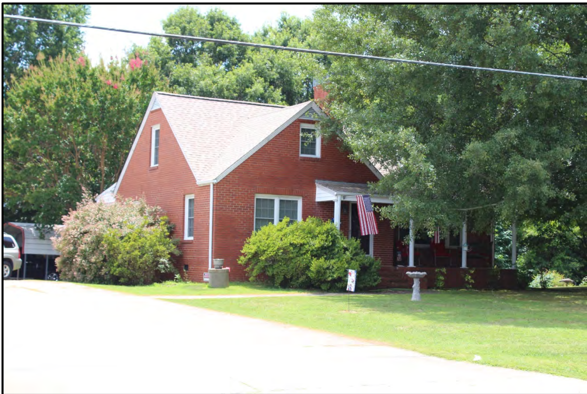
Figure 5.162. Architectural resource RK1710; view is southwest featuring the façade and east elevation.
