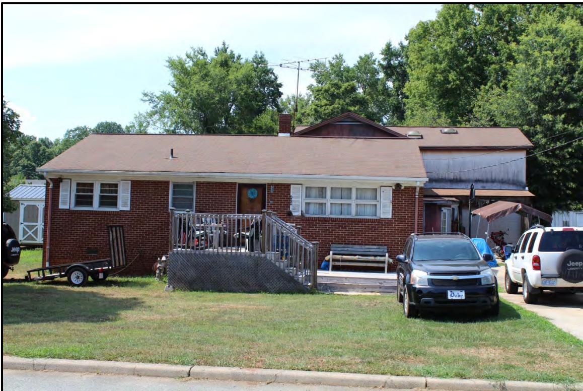
Figure 6.173. Architectural resource AM2569; view is northwest featuring the façade.
