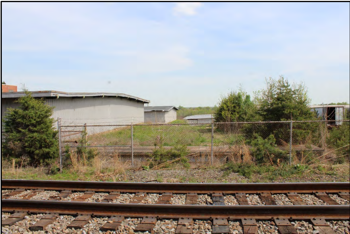
Figure 5.149. Architectural resource RK1704; view is south featuring intact warehouses.
