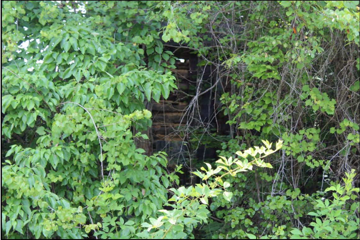
Figure 5.74. Architectural resource RK1674; view features an exterior log wall of a tobacco barn.
