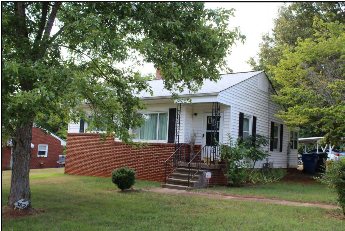
Figure 6.180. Architectural resource AM2576; view is northwest featuring the façade and northeast elevation.
