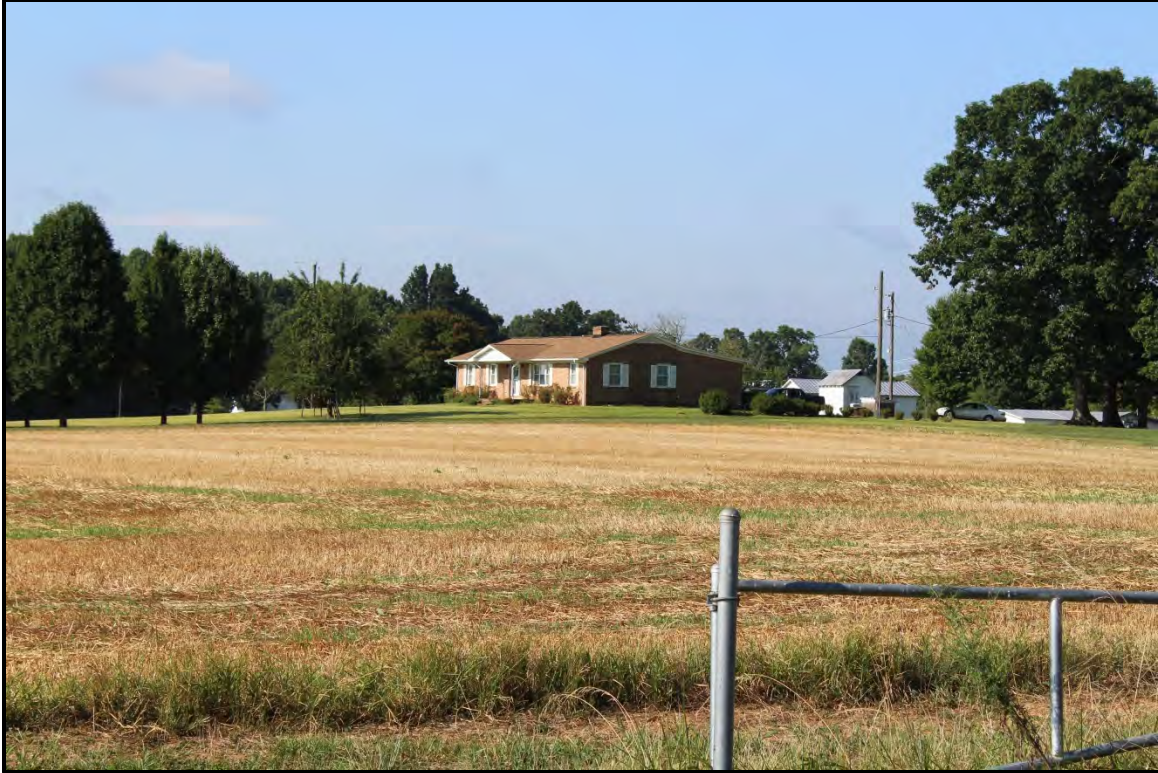
Figure 6.29. Architectural resource AM2493; view is southwest featuring the façade and north elevation.
