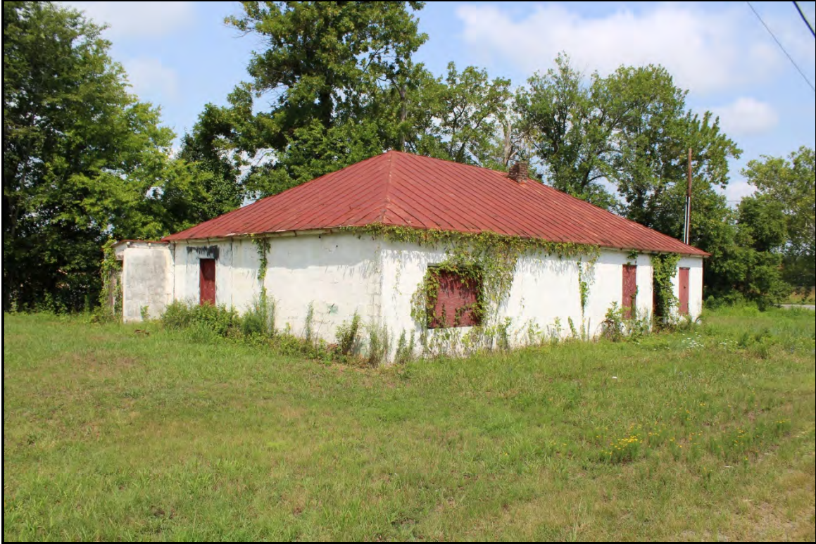
Figure 5.55. Architectural resource RK1664; view is northwest featuring the façade and southeast elevation.
