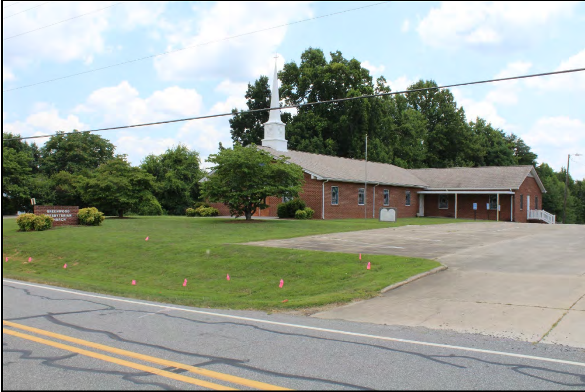
Figure 5.165. Architectural resource RK1712; view southeast featuring the façade and west elevation.
