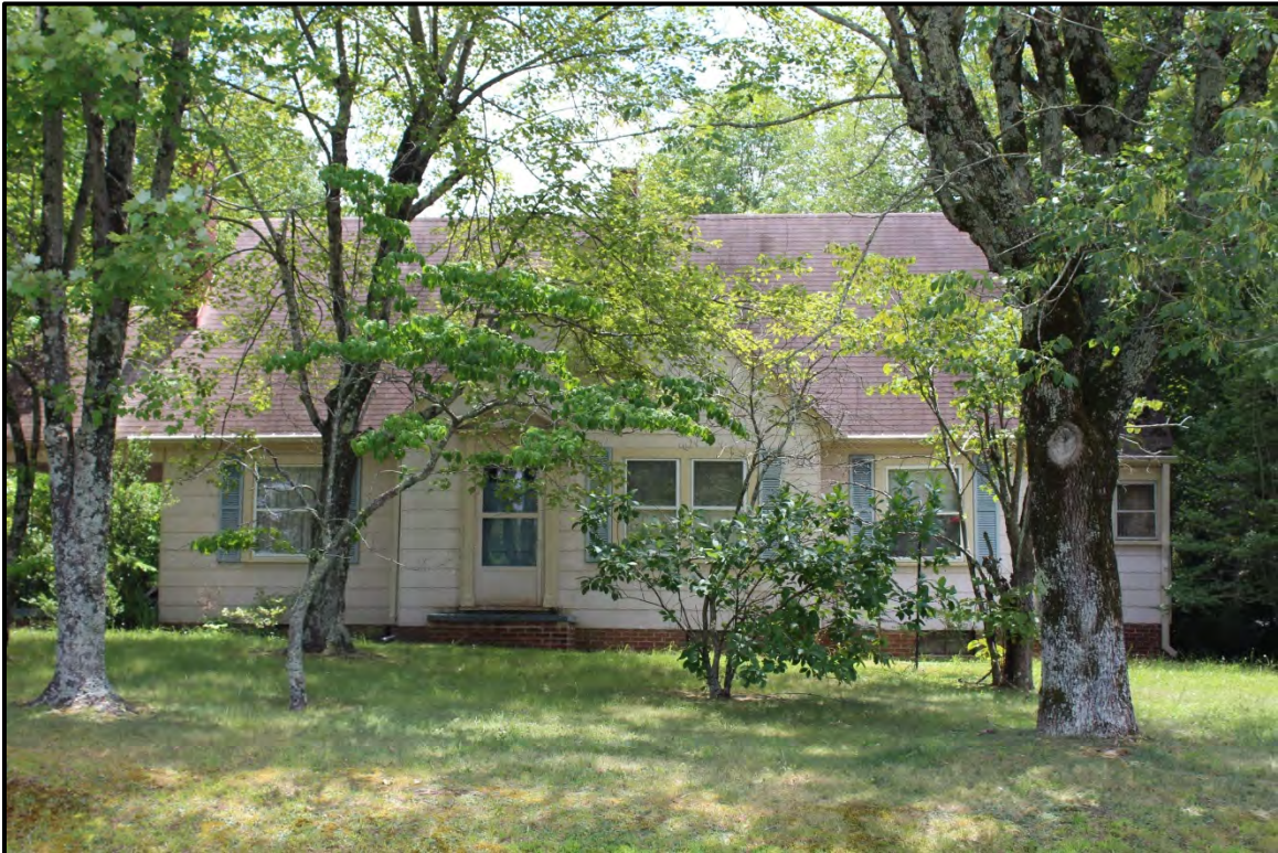
Figure 6.78. Architectural resource AM2510; view is south featuring the façade.
