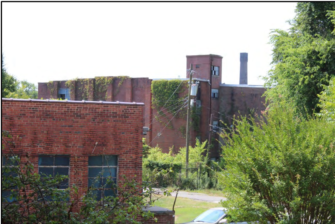
Figure 6.242. Architectural resource AM2407; view south toward northwest corner of the mill building.
