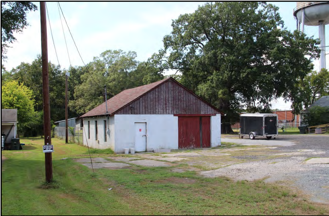
Figure 5.340. Architectural resource RK1777; view is northwest featuring the ca. 1939 garage and the ca. 1995 shed in the background.
