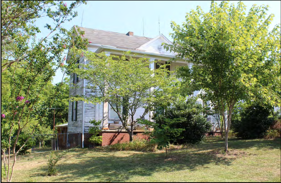
Figure 6.255. Architectural resource AM0266; view is northeast featuring the façade and west elevation.
