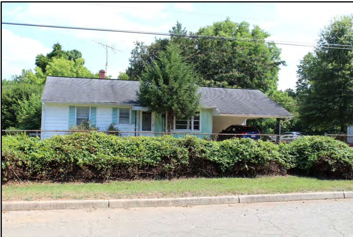
Figure 6.165. Architectural resource AM2561; view is southeast featuring the façade.
