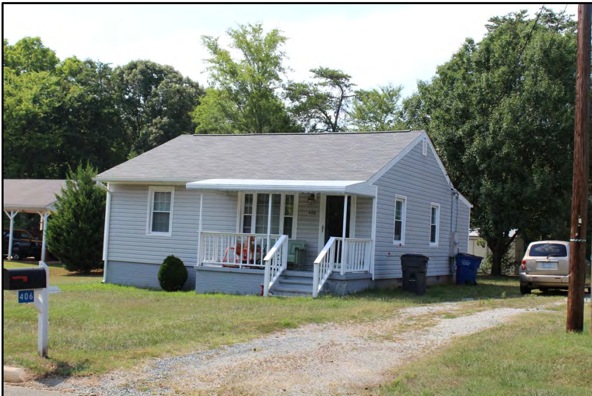
Figure 6.178. Architectural resource AM2574; view is northwest featuring the façade and northeast elevation.
