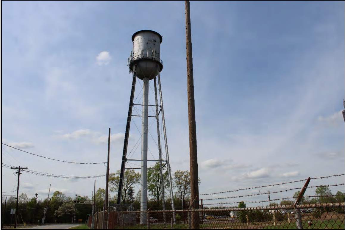
Figure 5.152. Architectural resource RK1704; view north featuring the water tower at the northwest corner of the parcel.
