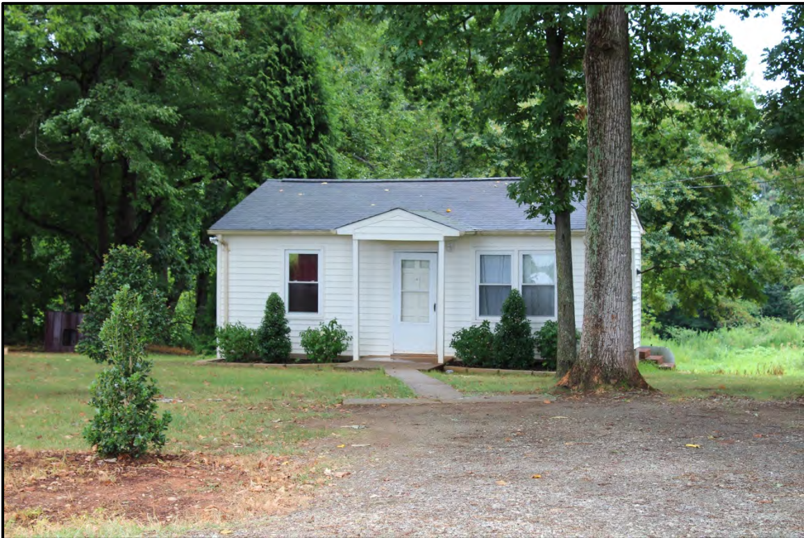
Figure 5.306. Architectural resource RK1765; view is northwest and features the façade.
