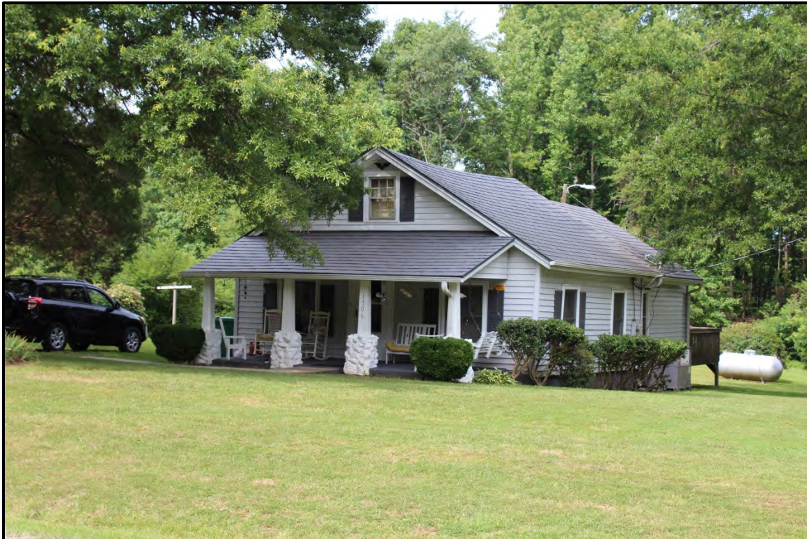
Figure 5.212. Architectural resource RK1740; view is southwest and features the façade and north elevation.
