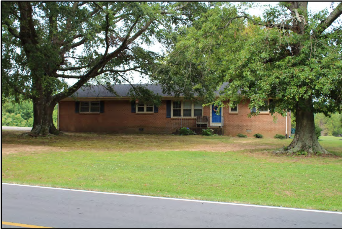
Figure 5.219. Architectural resource RK1742; view is southwest and features the façade.
