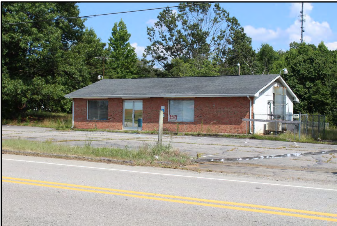
Figure 5.197. Architectural resource RK1734; view is southeast showing the façade and southwest elevation.
