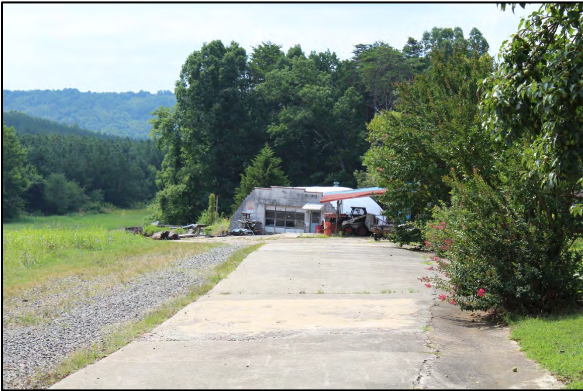
Figure 5.41. Architectural resource RK1658; view is south featuring the machine shop.
