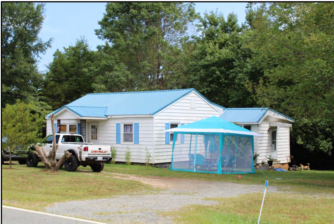
Figure 6.113. Architectural resource AM2521; view is northeast featuring the façade and southeast elevation.
