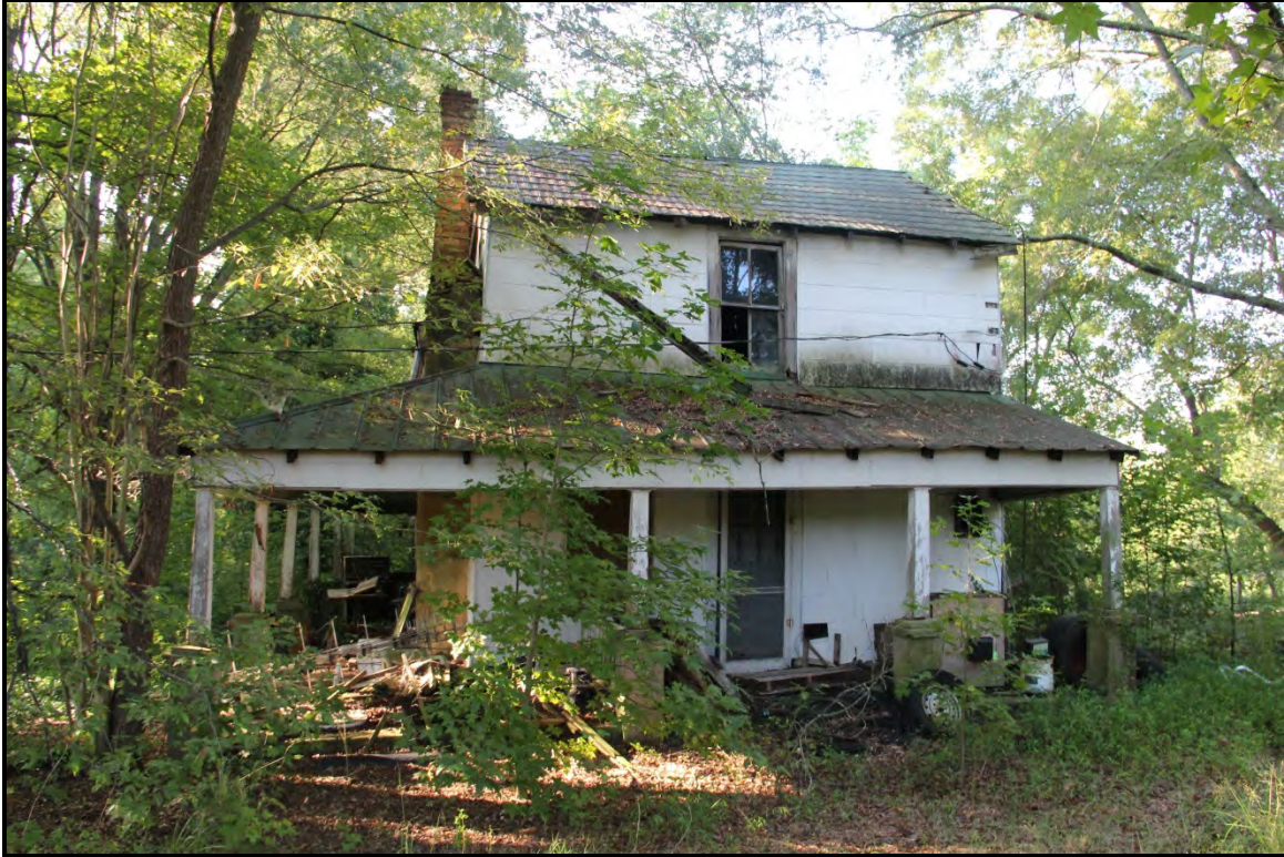
Figure 5.290. Architectural resource RK1759; view is south and features the façade.
