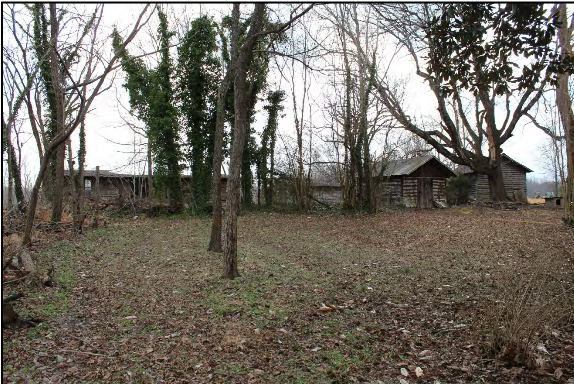
Figure 5.285. Overview of RK1758 outbuildings; view is southeast from the farmhouse.
