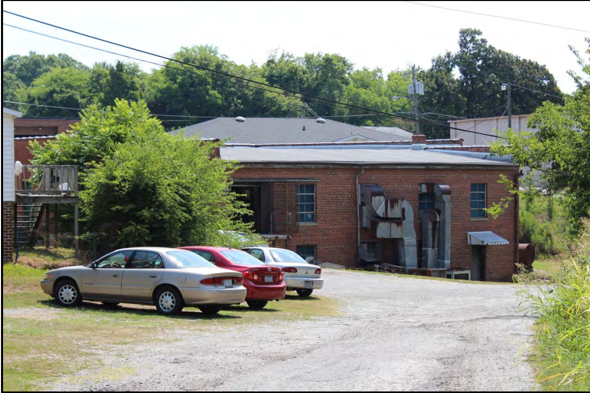
Figure 6.196. Architectural resource AM2588; view is east featuring the southwest (rear) elevation of the commercial building.
