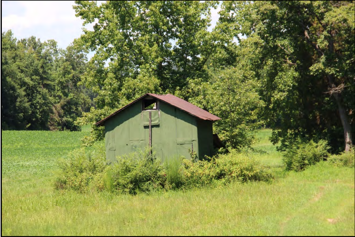
Figure 5.297. Architectural resource RK1760; view is north and features the late twentieth century shed.
