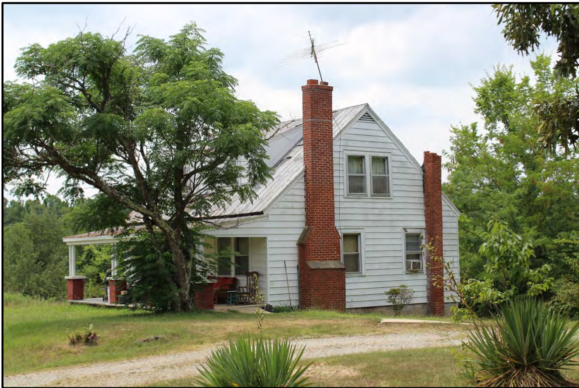
Figure 5.250. Architectural resource RK1755; view is southwest and features the façade and north elevation.
