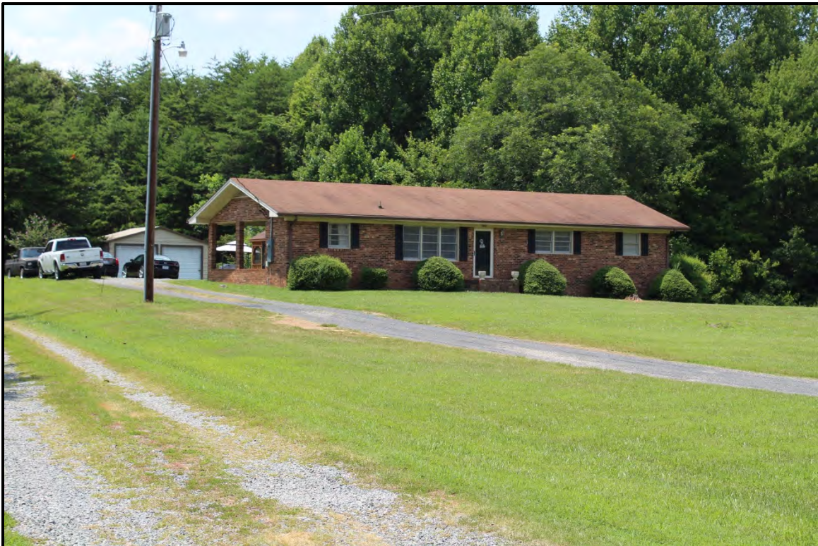
Figure 5.83. Architectural resource RK1677; view is northwest featuring the façade and south elevation.
