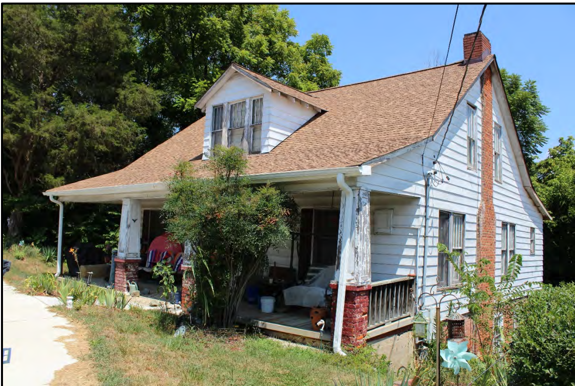
Figure 6.215. Architectural resource AM1595; view is northeast featuring 247 East Main Street.
