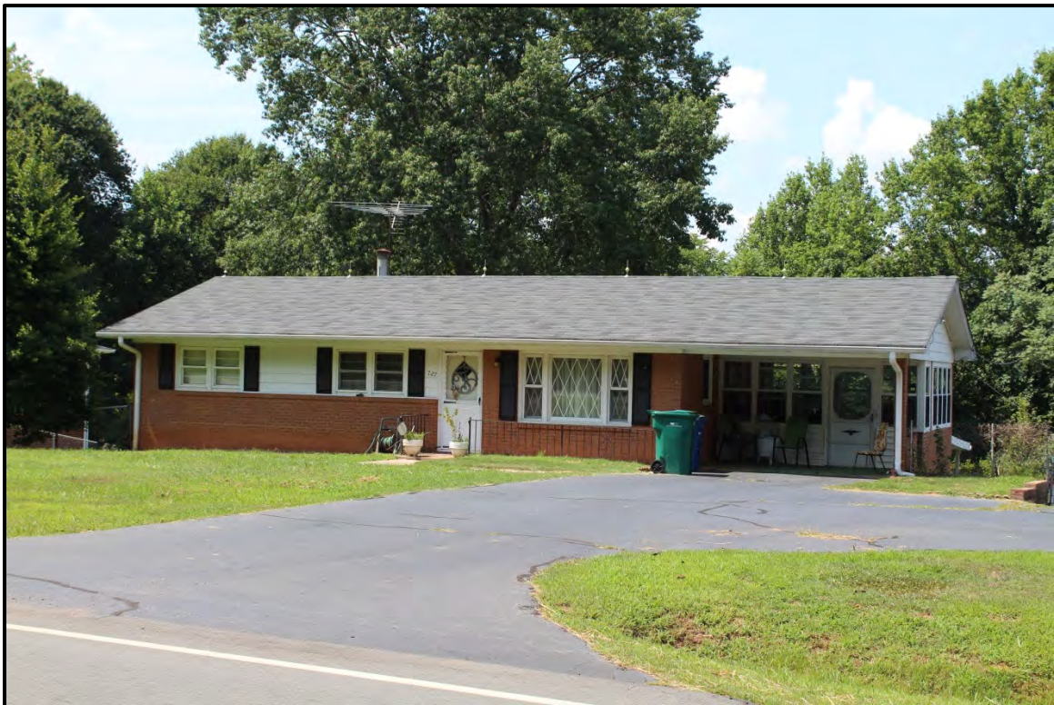
Figure 5.201. Architectural resource RK1736; view is northwest and features the façade and east elevation.
