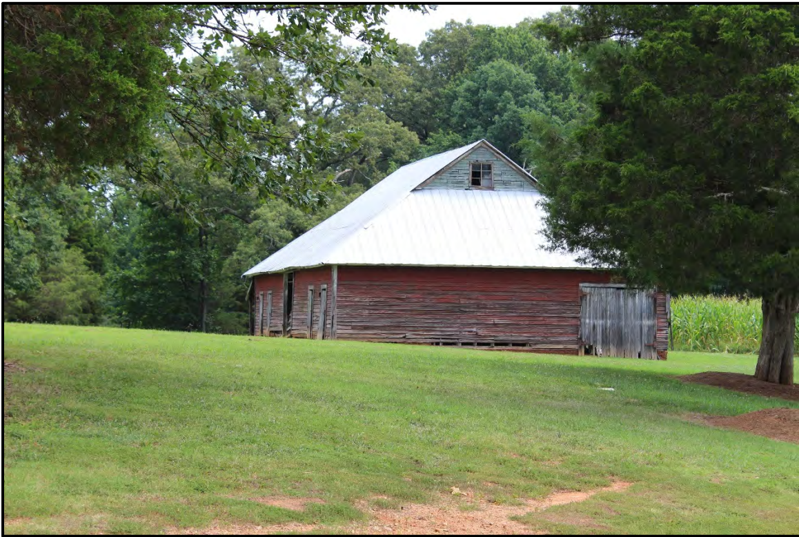
Figure 5.226. Architectural resource RK1534; view is northeast featuring the 1950 livestock barn.
