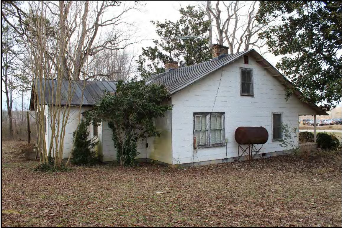
Figure 5.256. RK1758 1926 farmhouse; view is northwest and features the southeast elevation.
