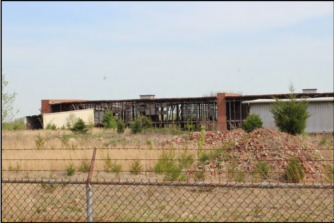
Figure 5.150. Architectural resource RK1704; view is southeast featuring warehouse ruins.
