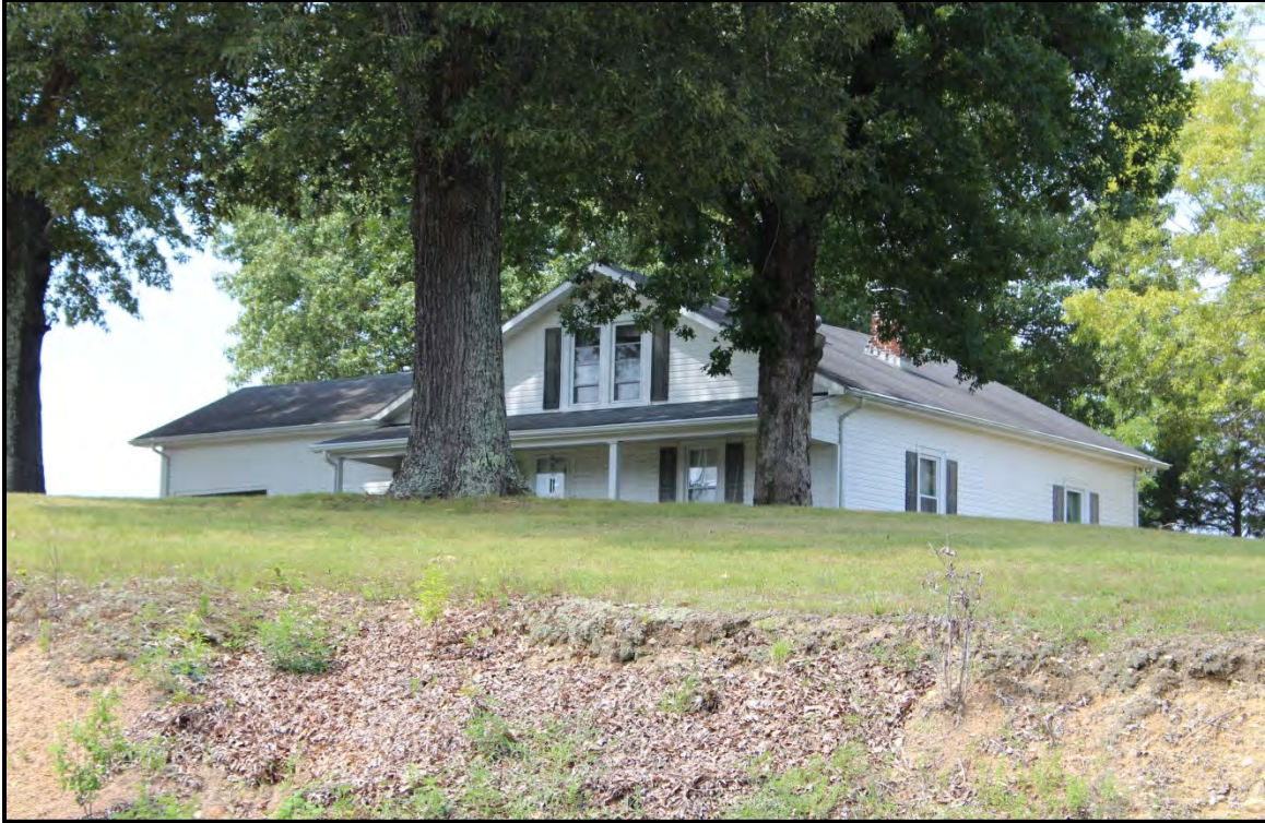
Figure 5.50. Architectural resource RK1663; view is southwest featuring the façade and north elevation.
