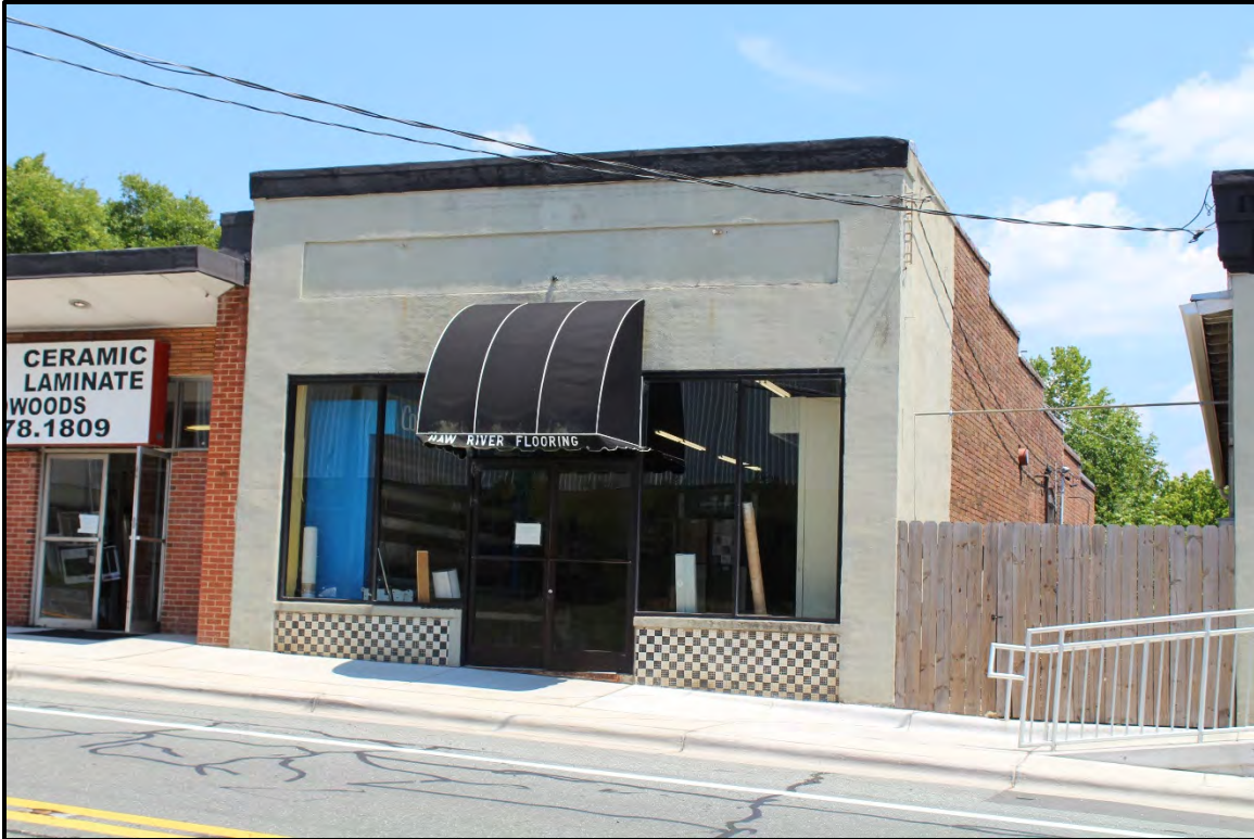
Figure 6.218. Architectural resource AM1595; view is northeast featuring 207 East Main Street.
