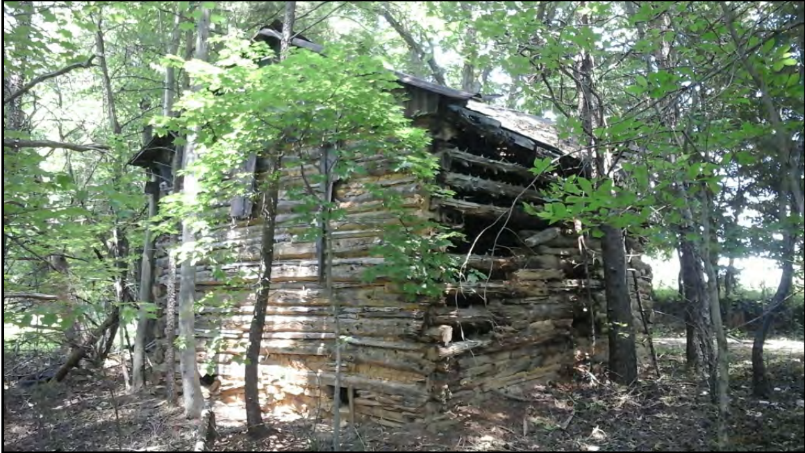
Figure 5.82. Architectural resource RK1676; view is of the rear and side elevations.
