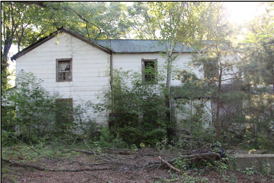
Figure 5.291. Architectural resource RK1759; view is east and features the west elevation.
