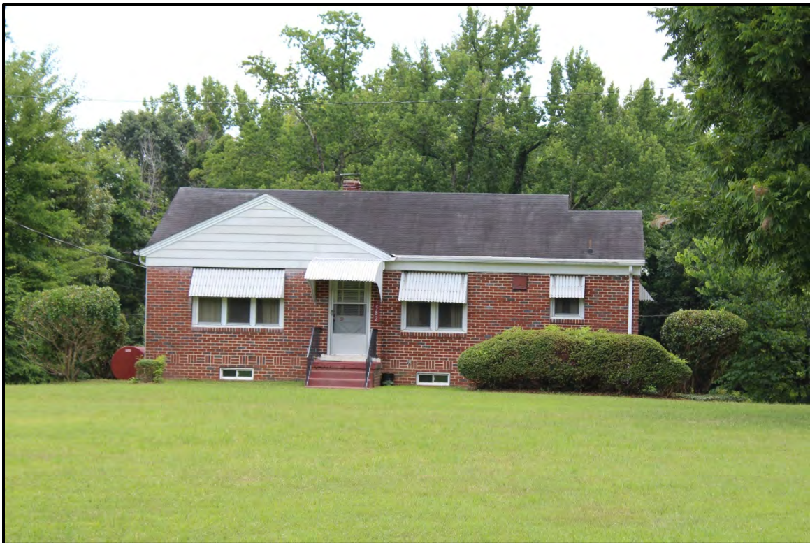
Figure 5.163. Architectural resource RK1711; view is south featuring the façade.
