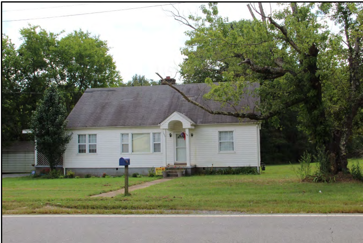
Figure 5.321. Architectural resource RK1771; view is south featuring the façade.
