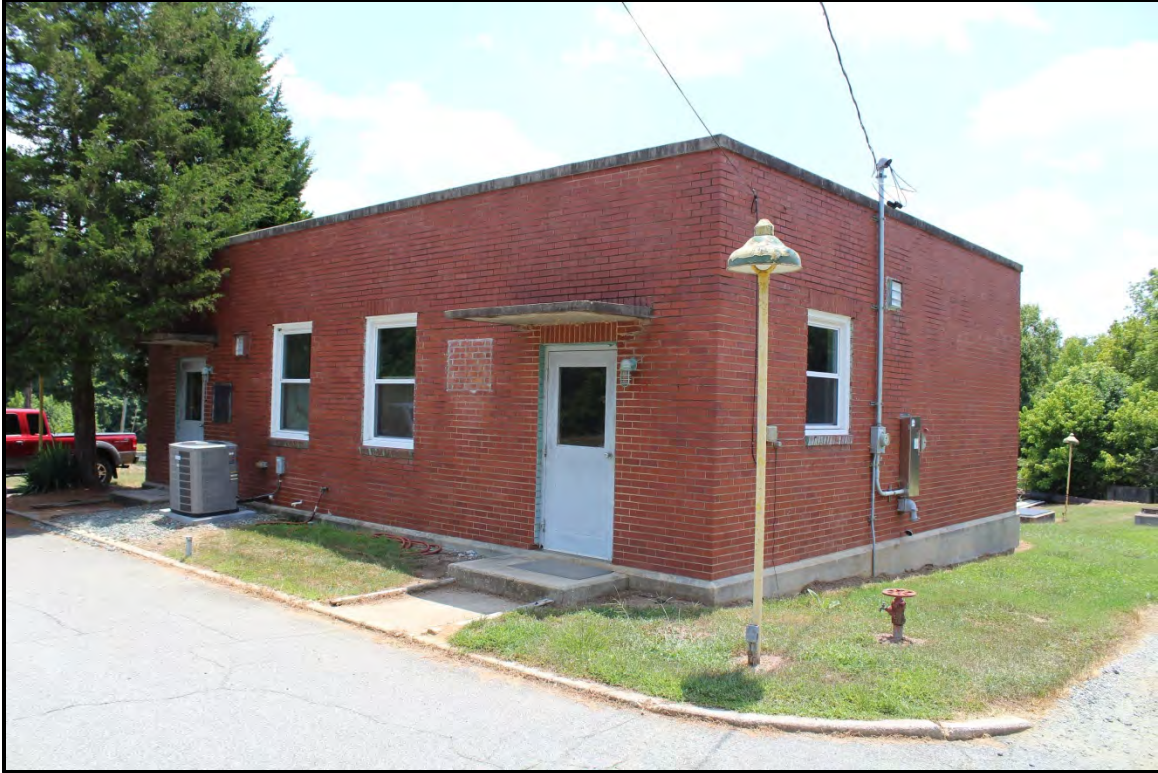
Figure 6.273. Architectural resource AM2604 control building; view is southeast and features the façade and west elevation.
