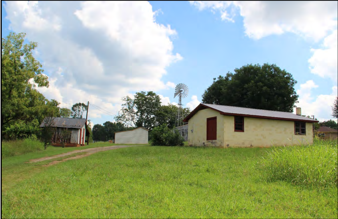
Figure 5.216. Architectural resource RK1741; view is southeast and features the associated outbuildings.
