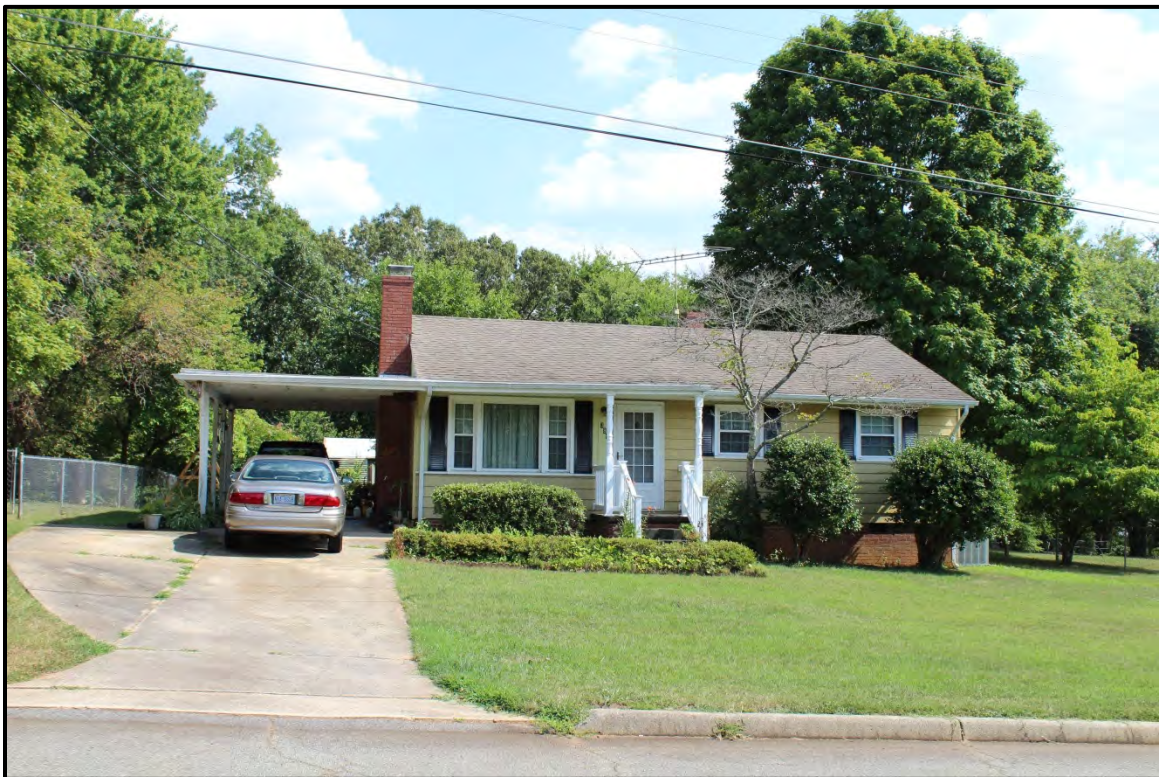
Figure 6.162. Architectural resource AM2558; view is southeast featuring the façade.
