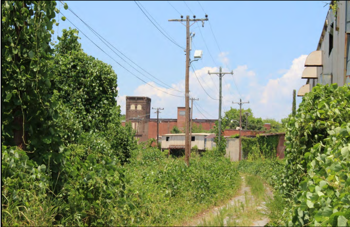
Figure 6.233. T.M. Holt Manufacturing Company; view is north featuring the elevated walkway to Tabardrey Mill (AM2407) in the background.
