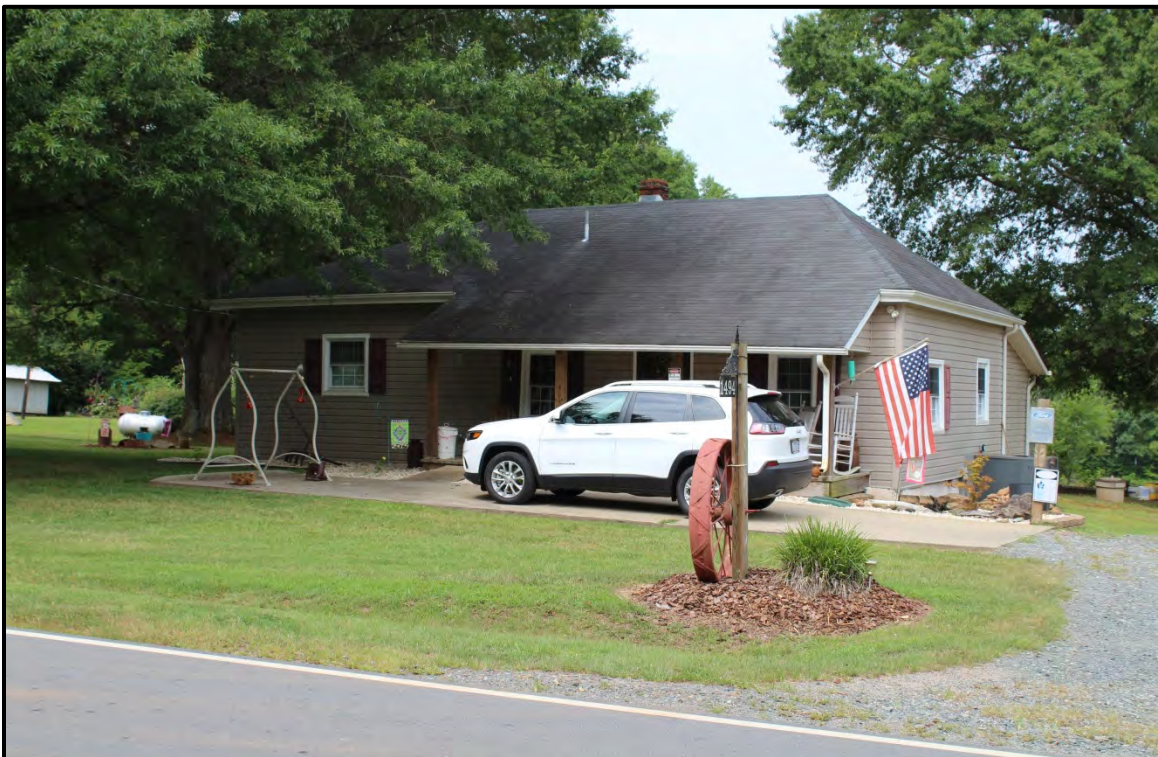
Figure 5.208. Architectural resource RK1738; oblique view featuring the façade and north elevation.
