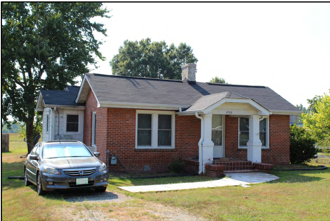
Figure 6.93. Architectural resource AM2515; view is northwest featuring the façade.
