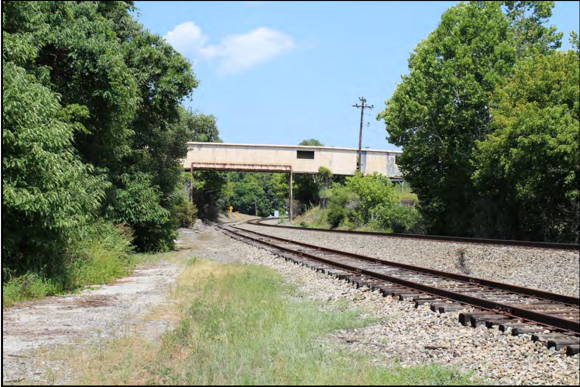
Figure 6.271. Architectural resource AM2603; view is east from architectural resource AM1516.
