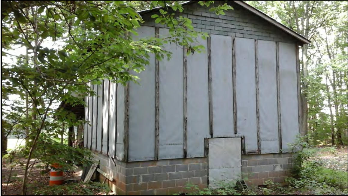
Figure 5.100. Architectural resource RK1682; view is northwest featuring the 1960 tobacco barn.
