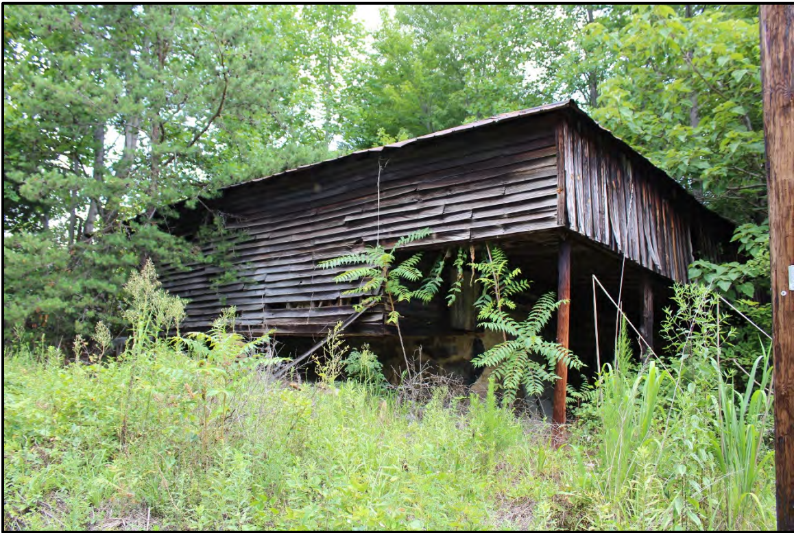
Figure 5.141. Architectural resource RK1701; view is southeast featuring the tobacco barn.
