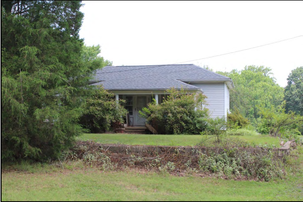
Figure 5.57. Architectural resource RK1665; view is northwest, featuring the façade.
