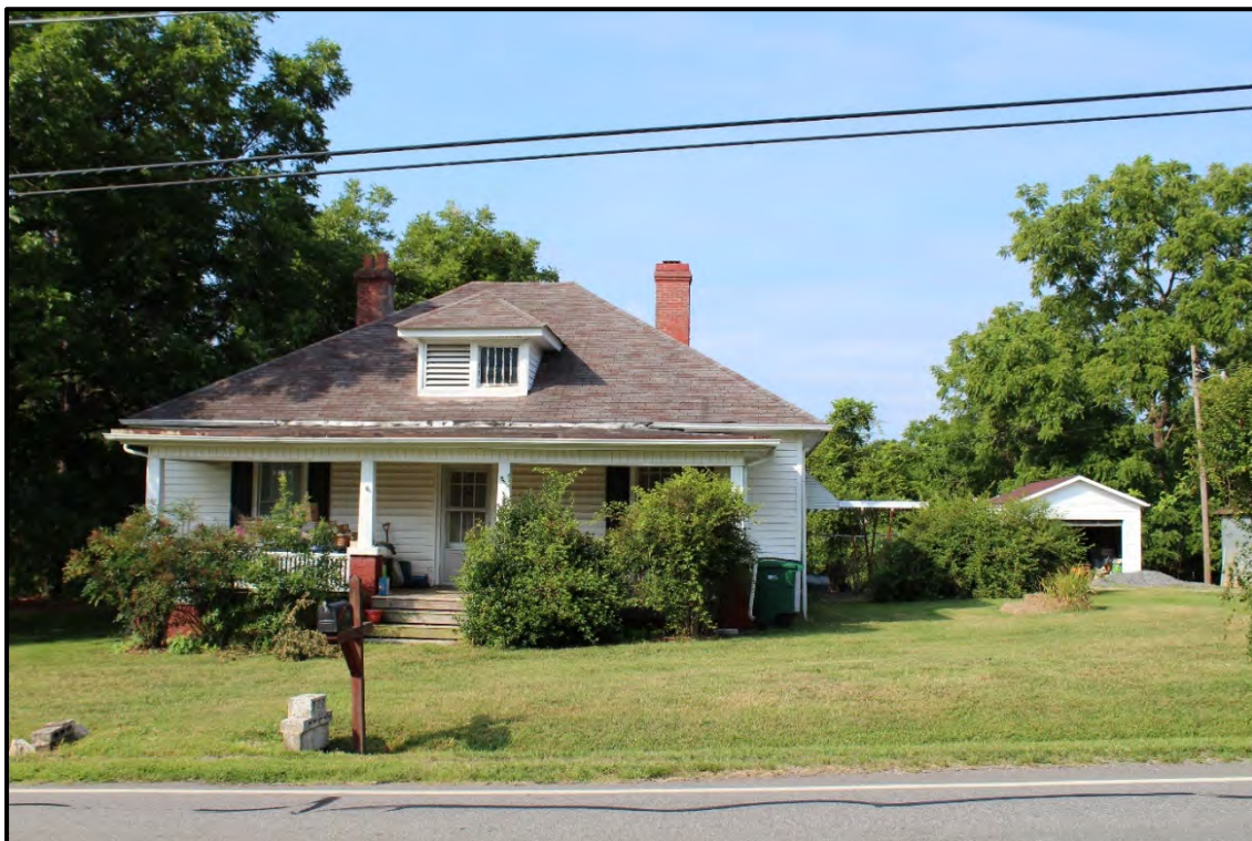
Figure 5.160. Architectural resource RK1707; view is southwest featuring the façade.
