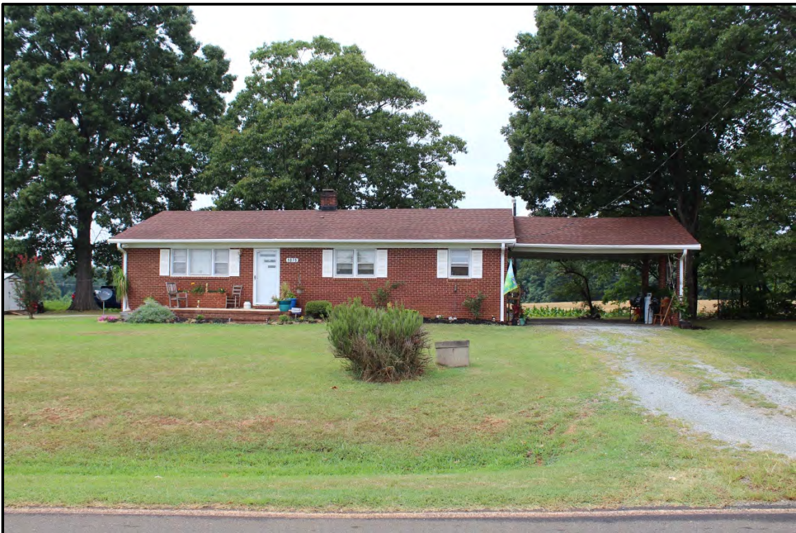
Figure 5.308. Architectural resource RK1767; view is north and features the façade.
