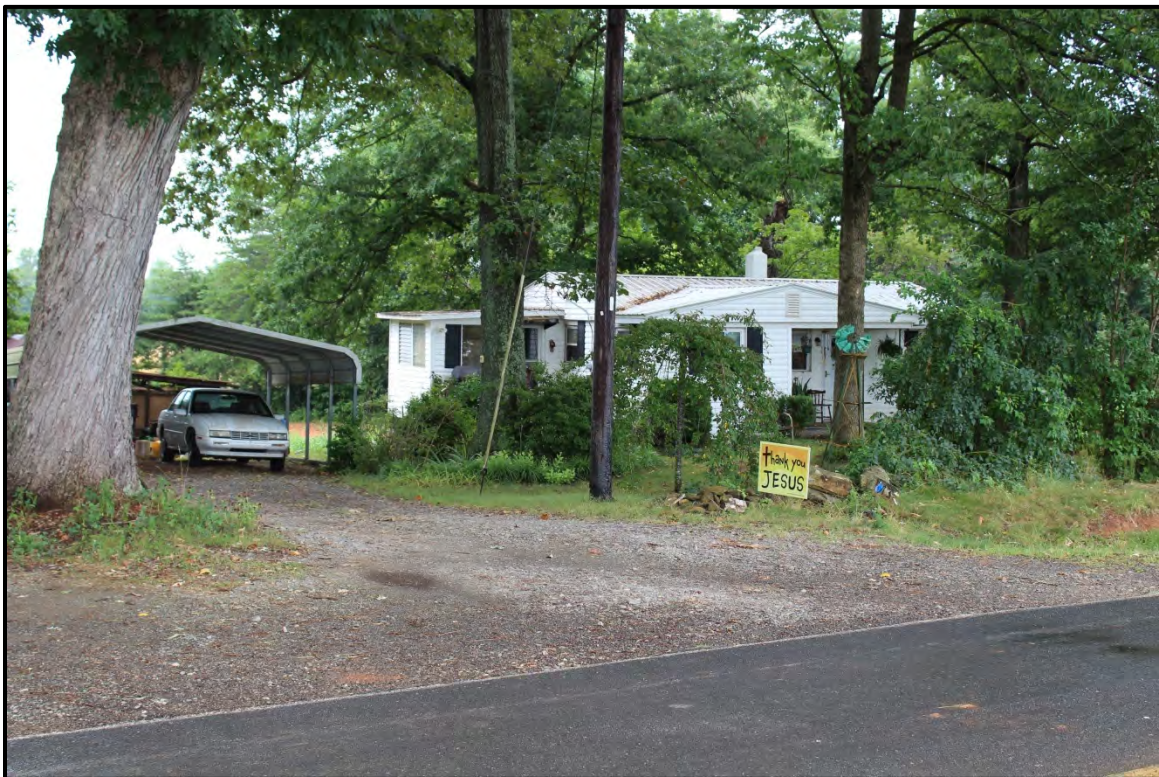
Figure 5.307. Architectural resource RK1766; view is northeast and features the façade and west elevation.
