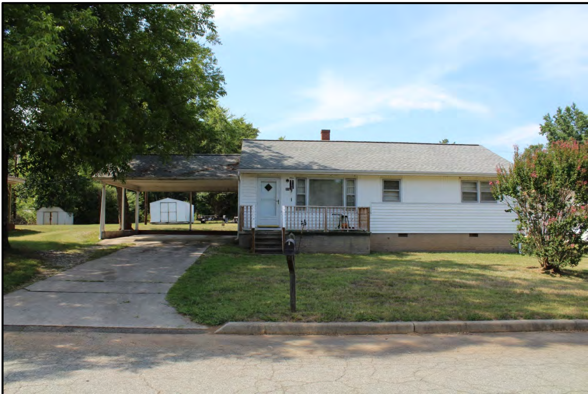
Figure 6.175. Architectural resource AM2571; view is northwest featuring the façade.
