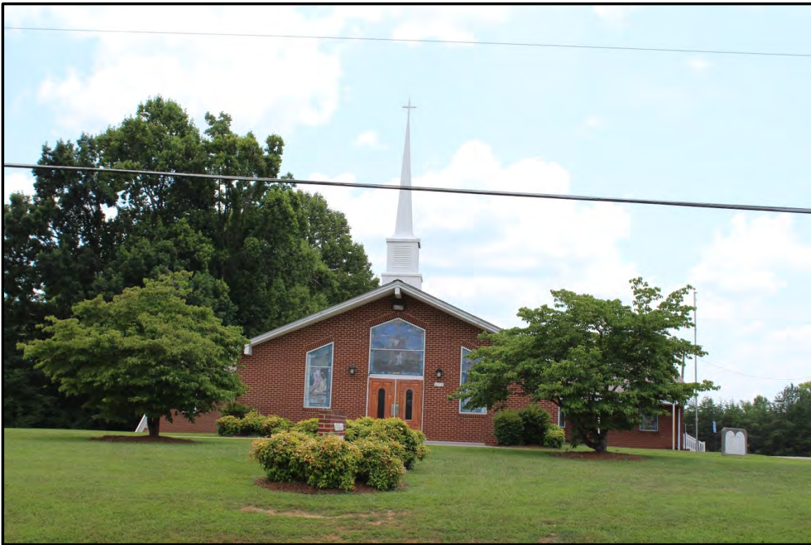
Figure 5.164. Architectural resource RK1712; view is south and features the façade.
