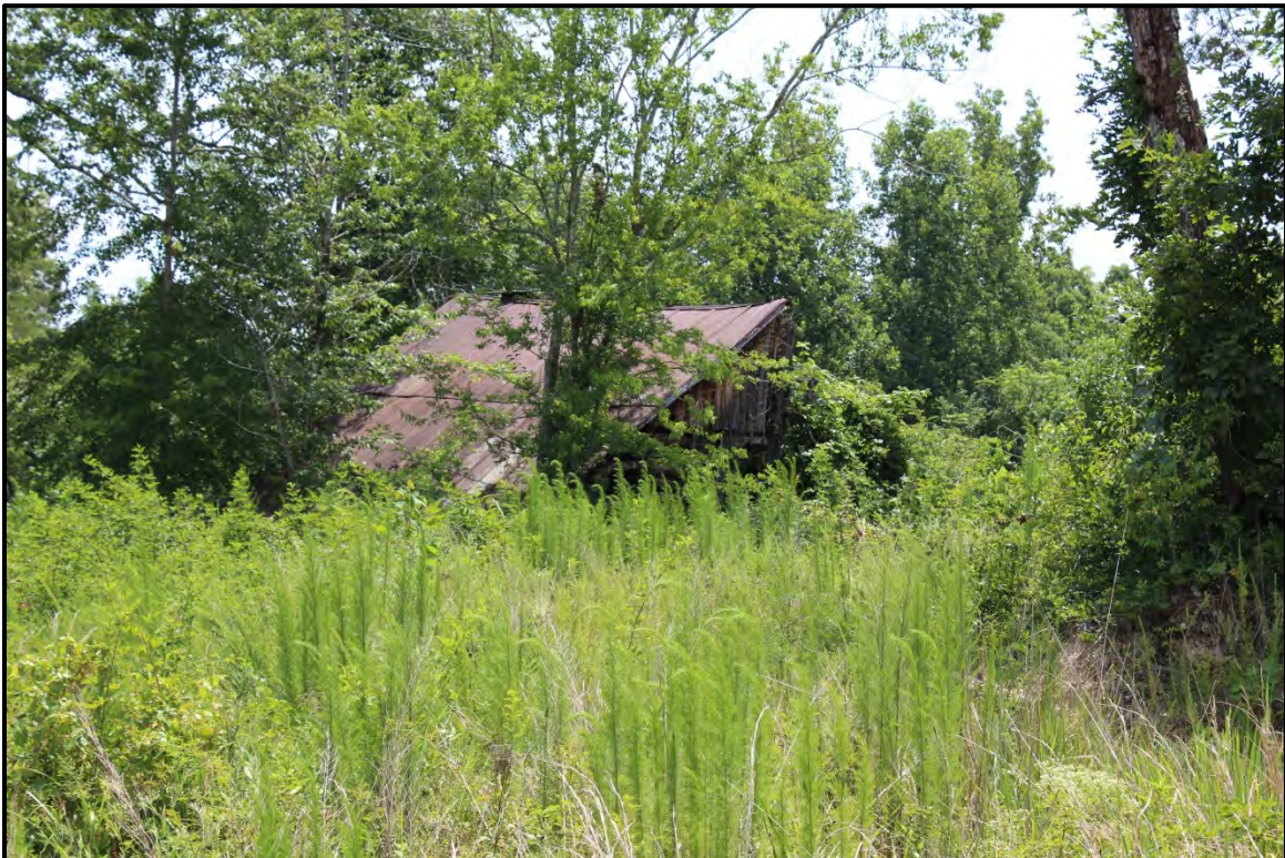
Figure 5.75. Architectural resource RK1674; view features the collapsed tobacco barn.
