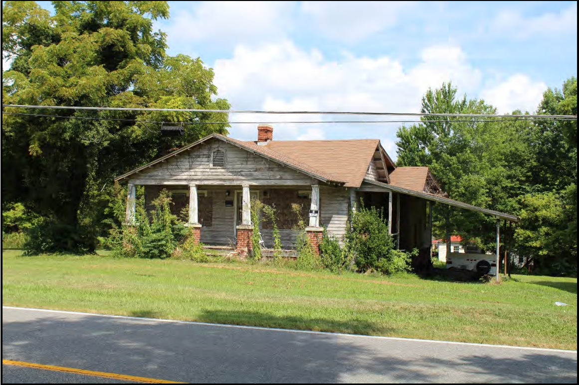
Figure 5.137. Architectural resource RK1700; view is north featuring the façade.
