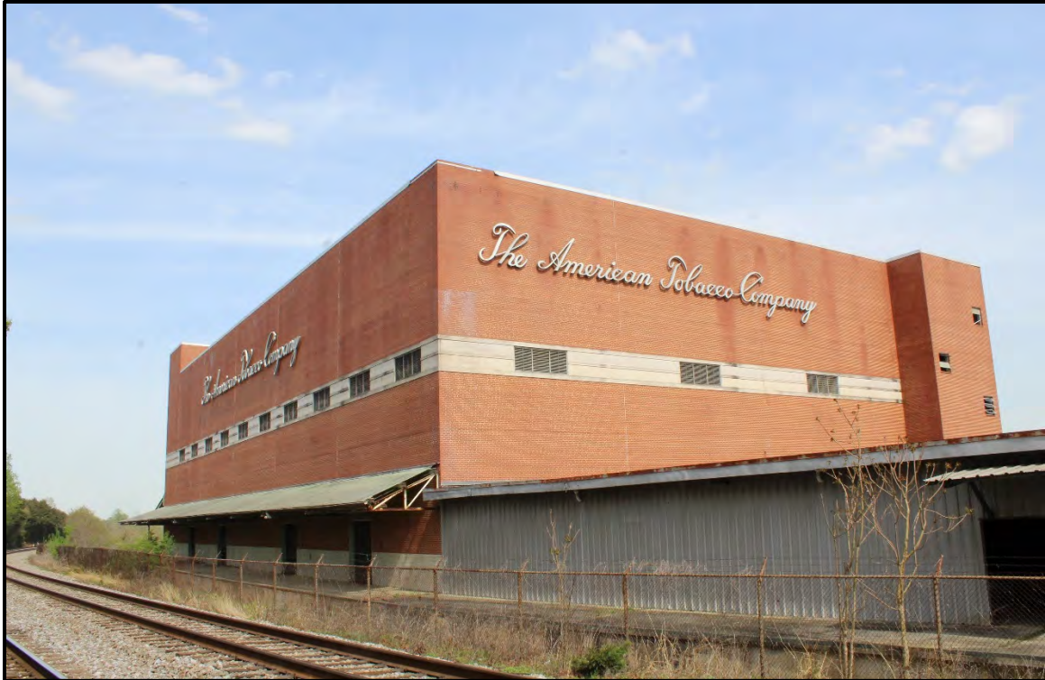
Figure 5.144. Architectural resource RK1704; view is east featuring the north and west elevations of the main manufacturing plant building.
