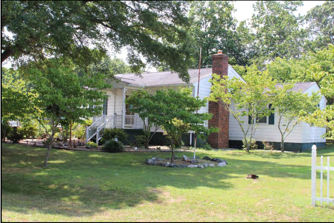
Figure 6.148. Architectural resource AM2546; view is south featuring the façade and northwest elevation.
