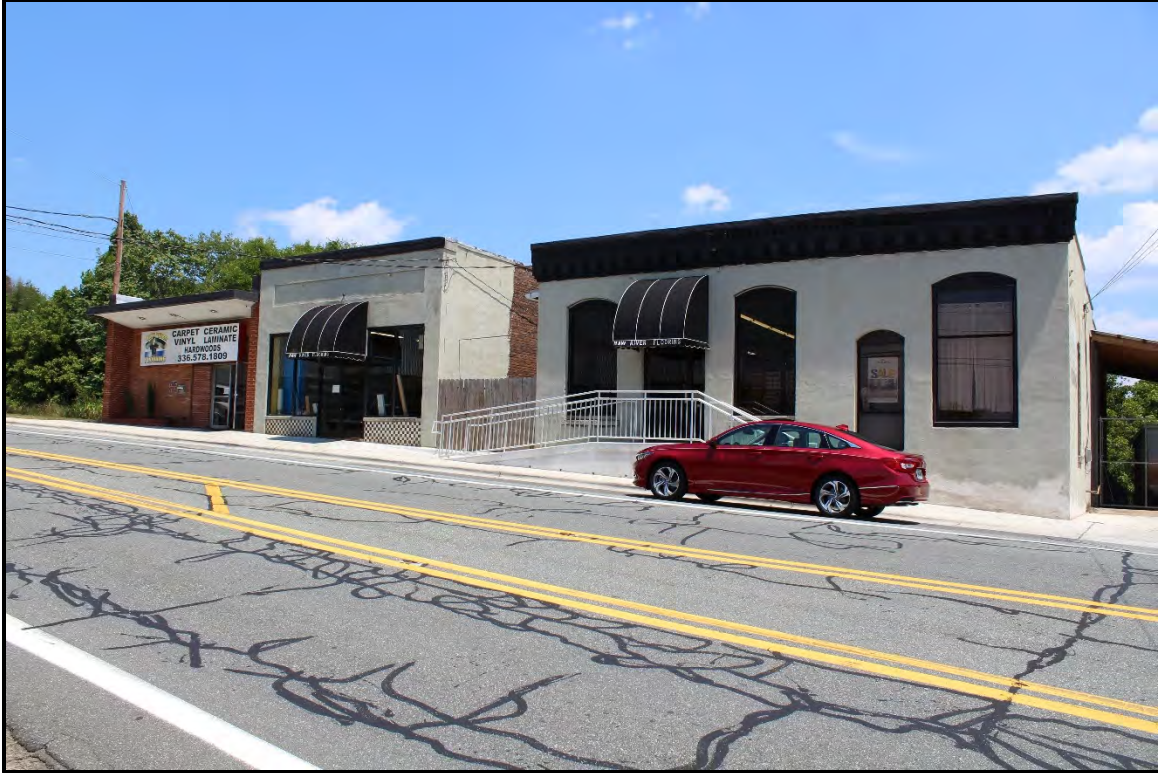
Figure 6.209. Architectural resource AM2597; view is northeast and features the west elevation.
