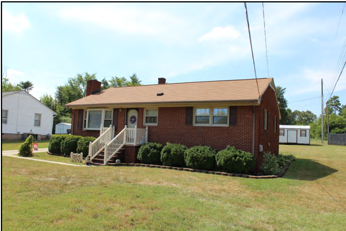
Figure 6.174. Architectural resource AM2570; view is northwest featuring the façade and northeast elevation.
