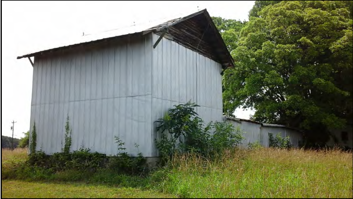
Figure 5.110. Architectural resource RK1684; view is southeast featuring tobacco barn.
