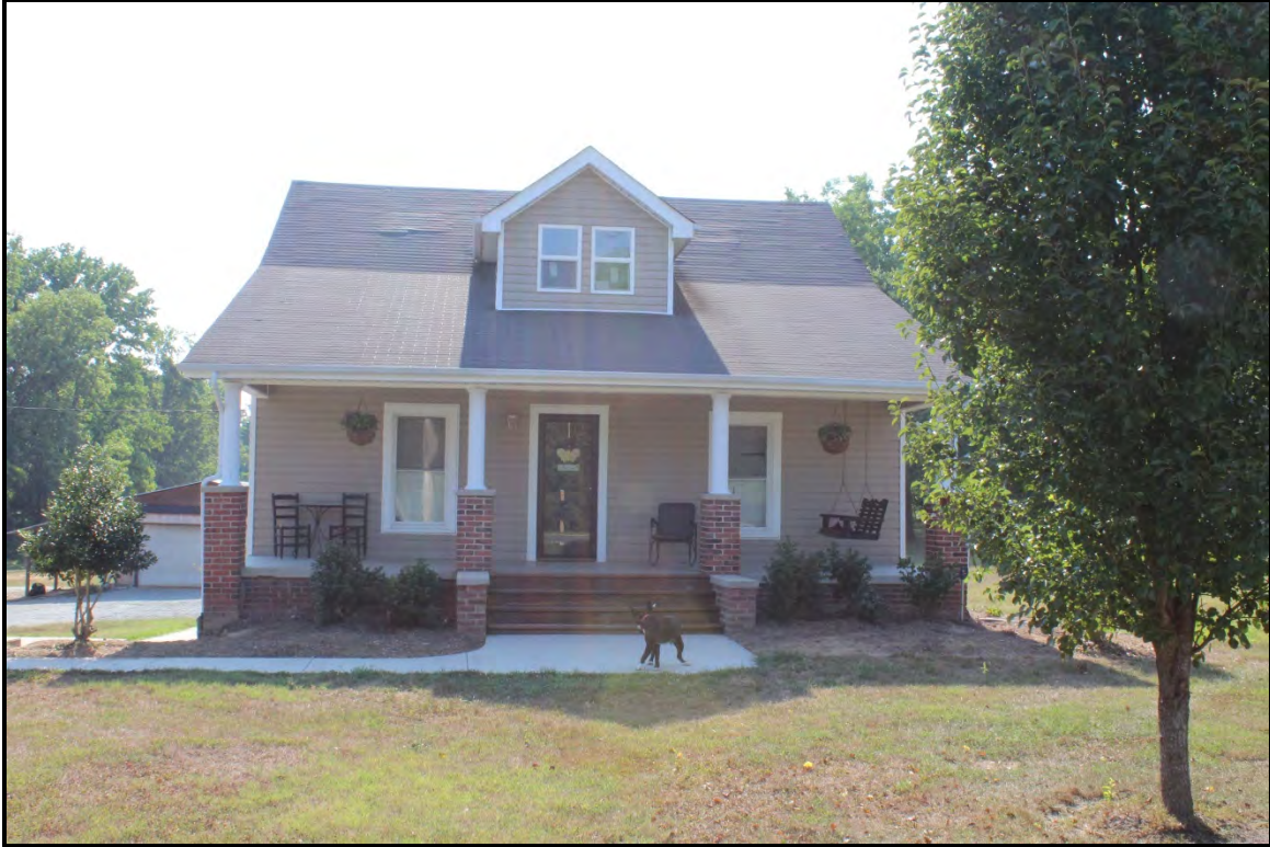
Figure 6.120. Architectural resource AM2526; view is west featuring the façade.
