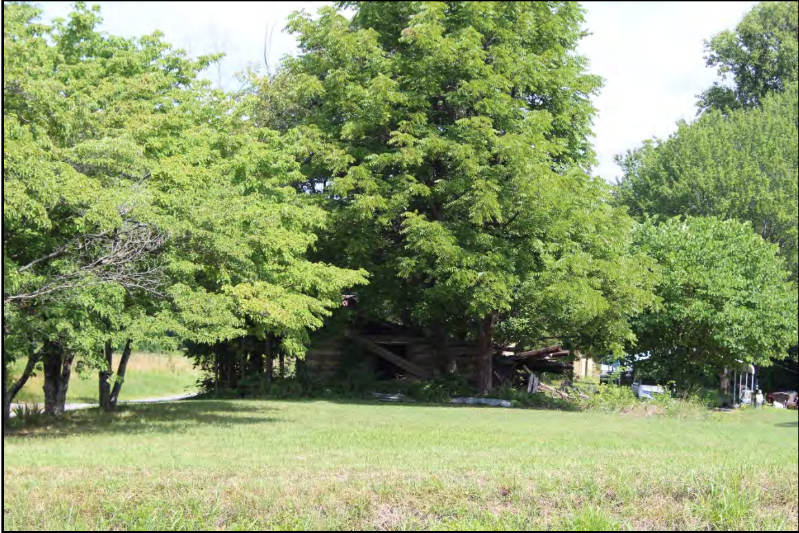
Figure 5.139. Collapsed and overgrown log tobacco barn at resource RK1700; view is north.
