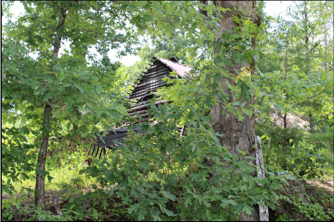
Figure 5.76. Architectural resource RK1674; view of partially collapsed tobacco barn.
