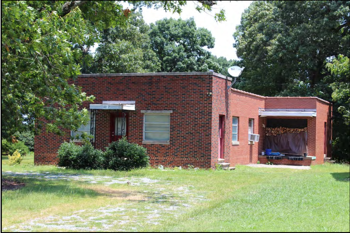
Figure 6.52. Architectural resource AM1527; view is northeast featuring the façade and south elevation of the book depository building.
