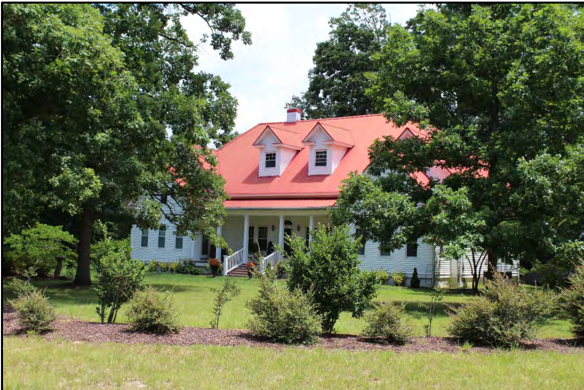
Figure 6.47. Architectural resource AM0157; view is north featuring the façade and a portion of the north elevation.
