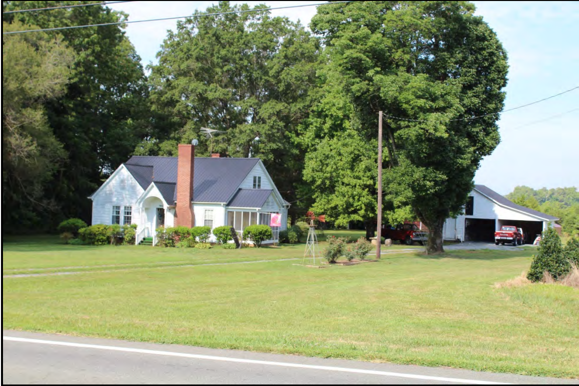
Figure 6.22. Architectural resource AM2492; view is southwest, featuring the house and barn/garage.
