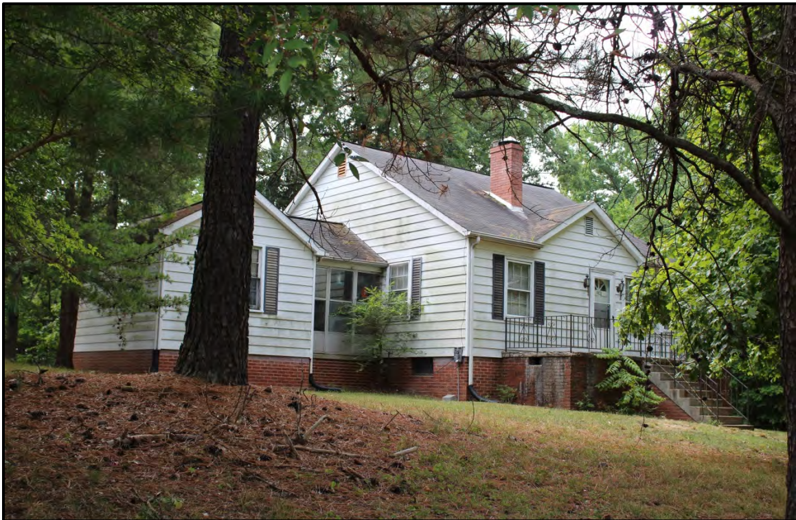
Figure 6.277. Architectural resource AM2605; view is southeast and features the façade and north elevation.
