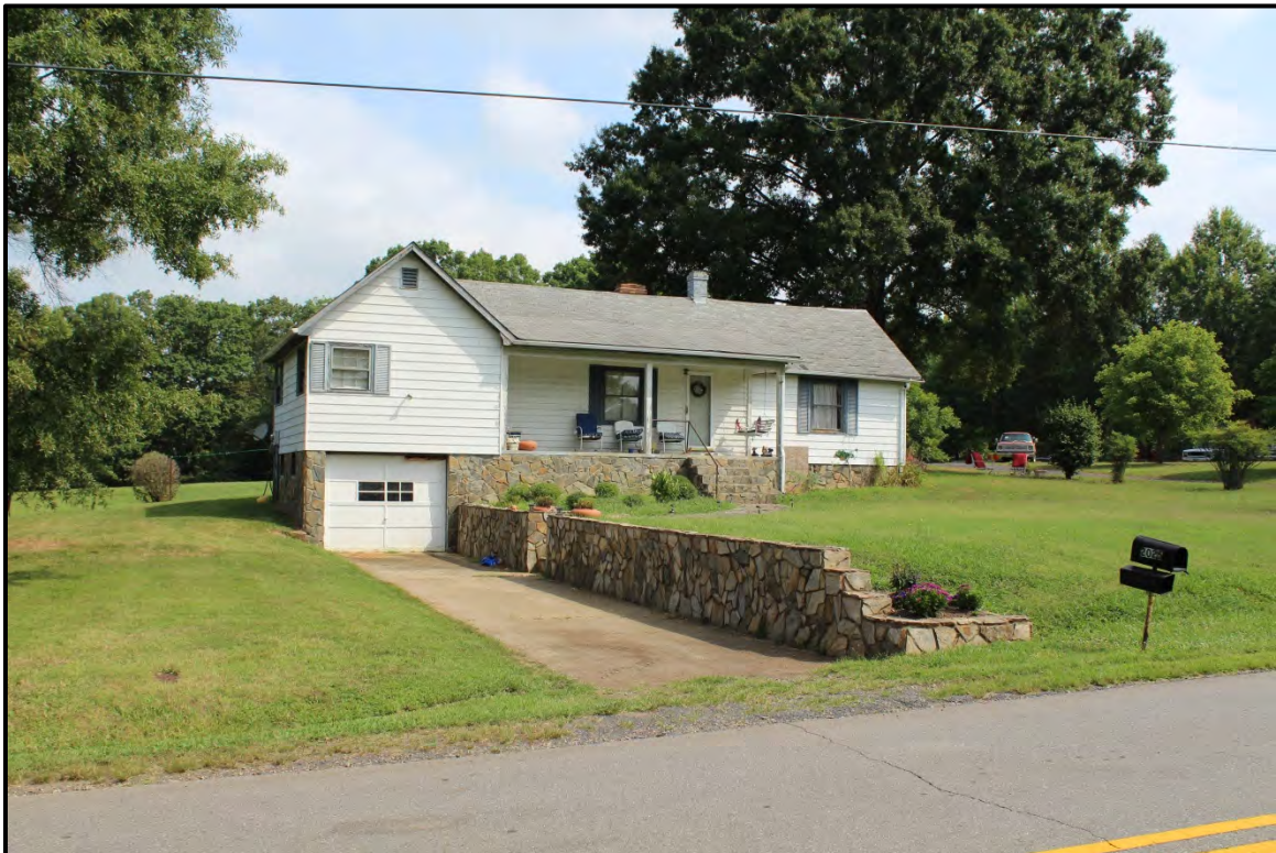
Figure 5.43. Architectural resource RK1660; view is north featuring the façade.
