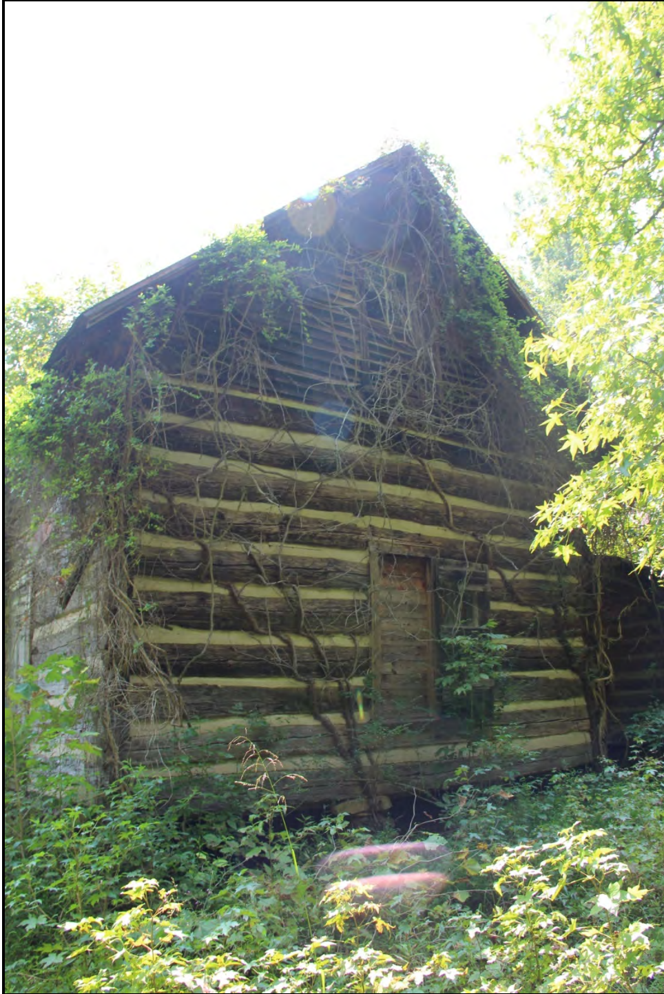
Figure 5.11. Architectural resource RK1656; view is south featuring the northwest elevation.
