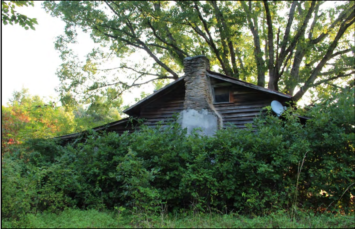
Figure 5.86. Architectural resource RK1768; view is east and features the west elevation.
