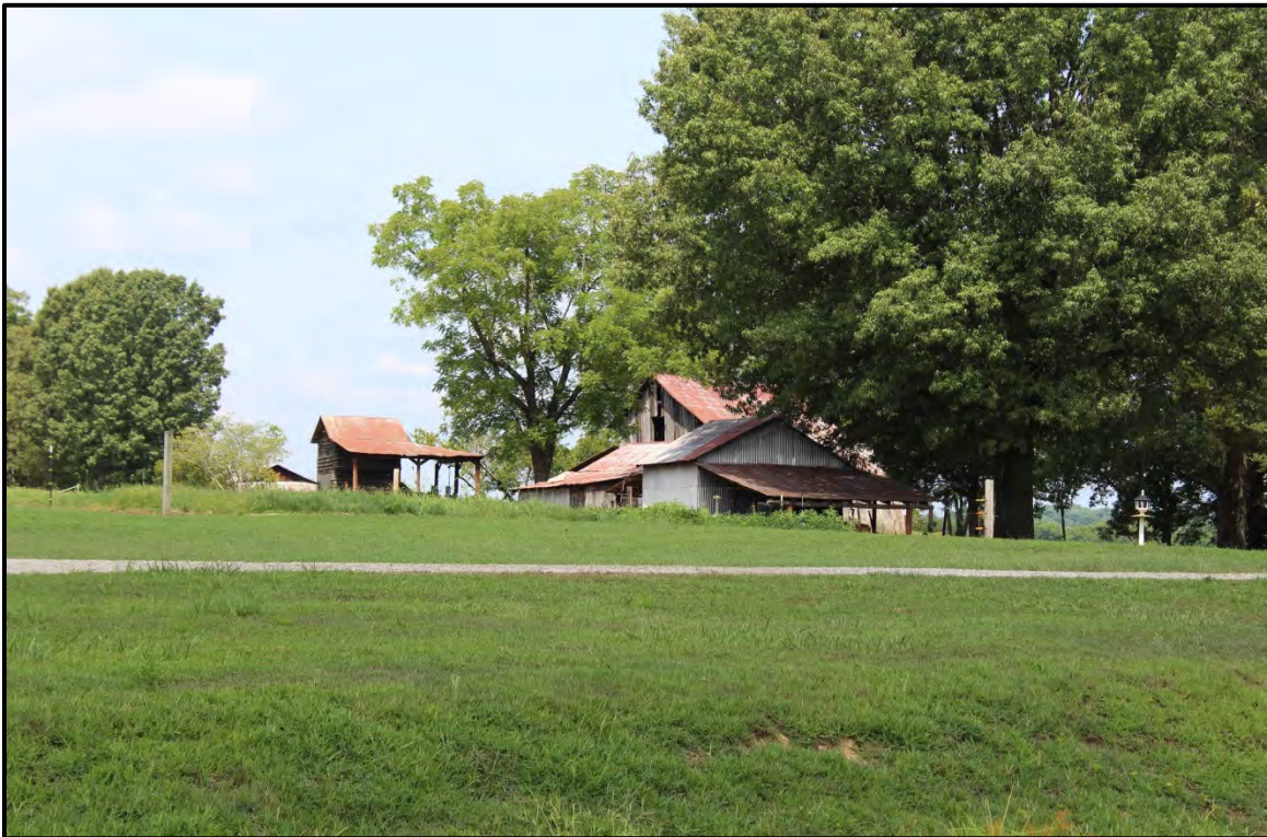
Figure 5.49. Architectural resource RK1663; view is northwest featuring associated outbuildings.
