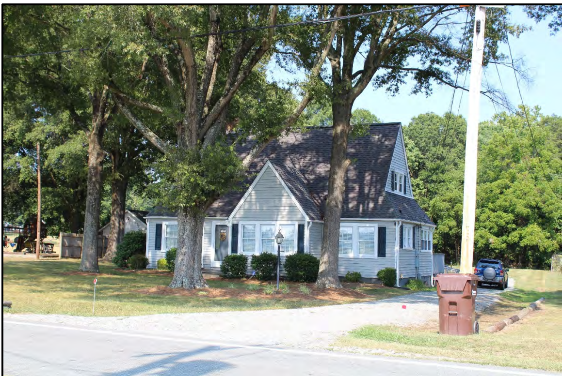
Figure 6.133. Architectural resource AM2537; view is northeast featuring the façade and south elevation.
