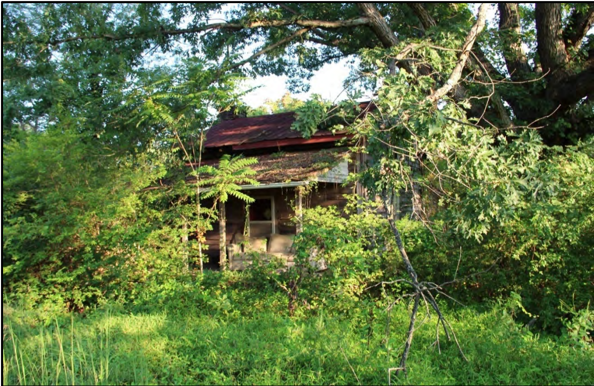
Figure 5.85. Architectural resource RK1768; view is northwest and features the façade and east elevation.
