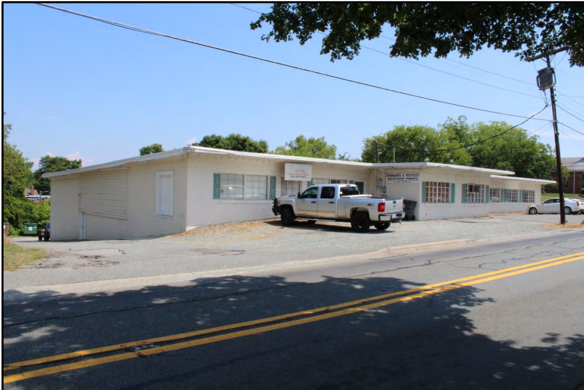
Figure 6.191. Architectural resource AM2586; view is northeast featuring the façade and southwest elevation.
