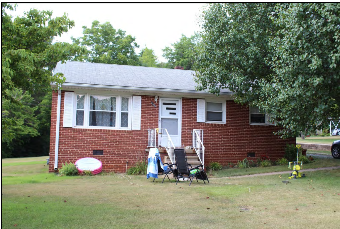
Figure 6.181. Architectural resource AM2577; view is northwest featuring the façade.
