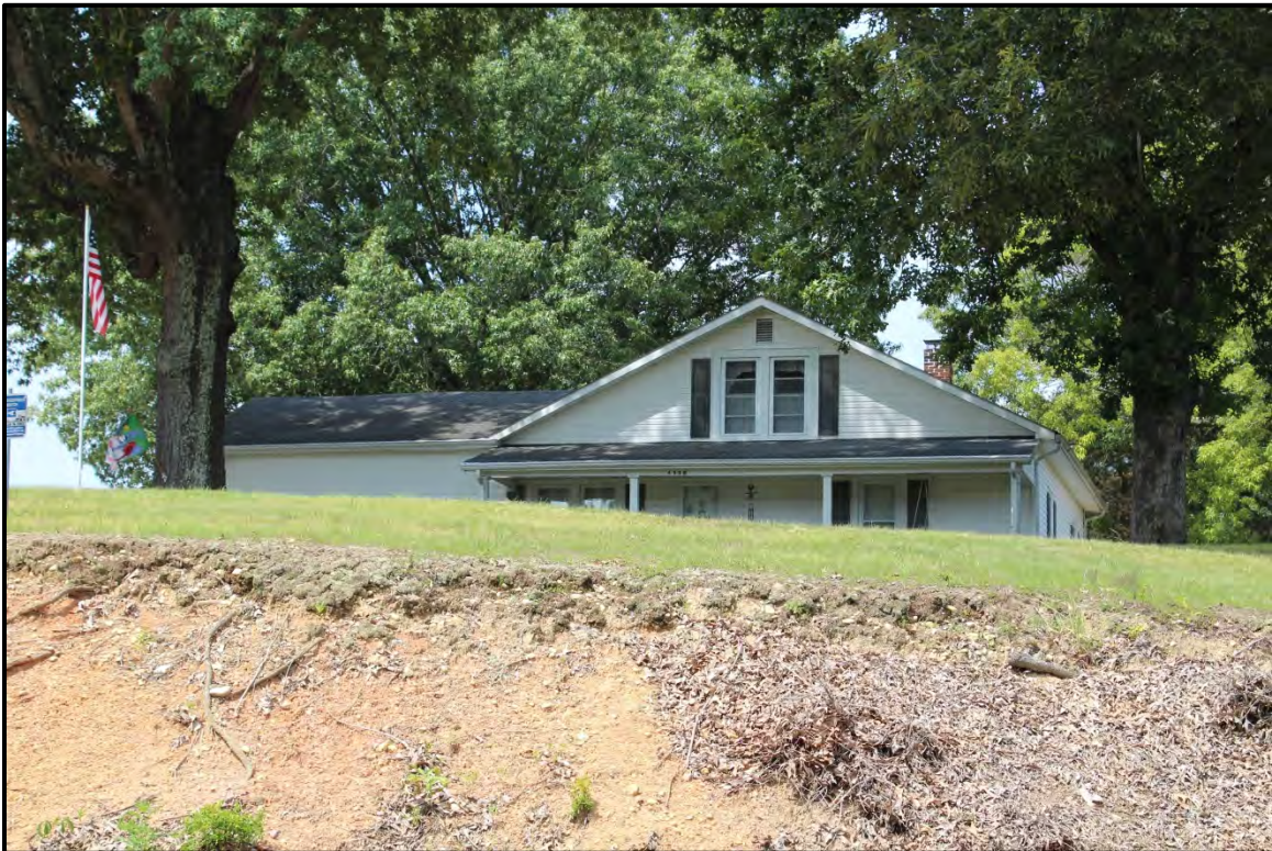
Figure 5.51. Architectural resource RK1663; view is west featuring the façade.
