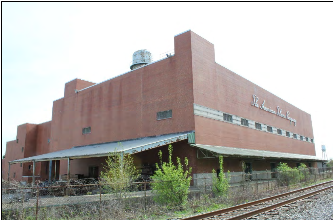
Figure 5.145. Architectural resource RK1704; view is west featuring the east and north elevations of the main manufacturing plant building.
