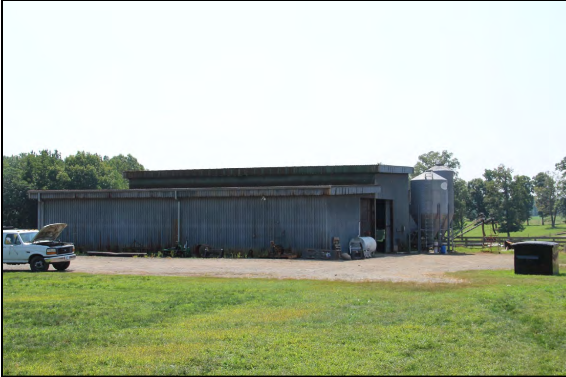
Figure 5.4. Architectural resource RK1655; view is south featuring the 1970 agricultural vehicle maintenance building.
