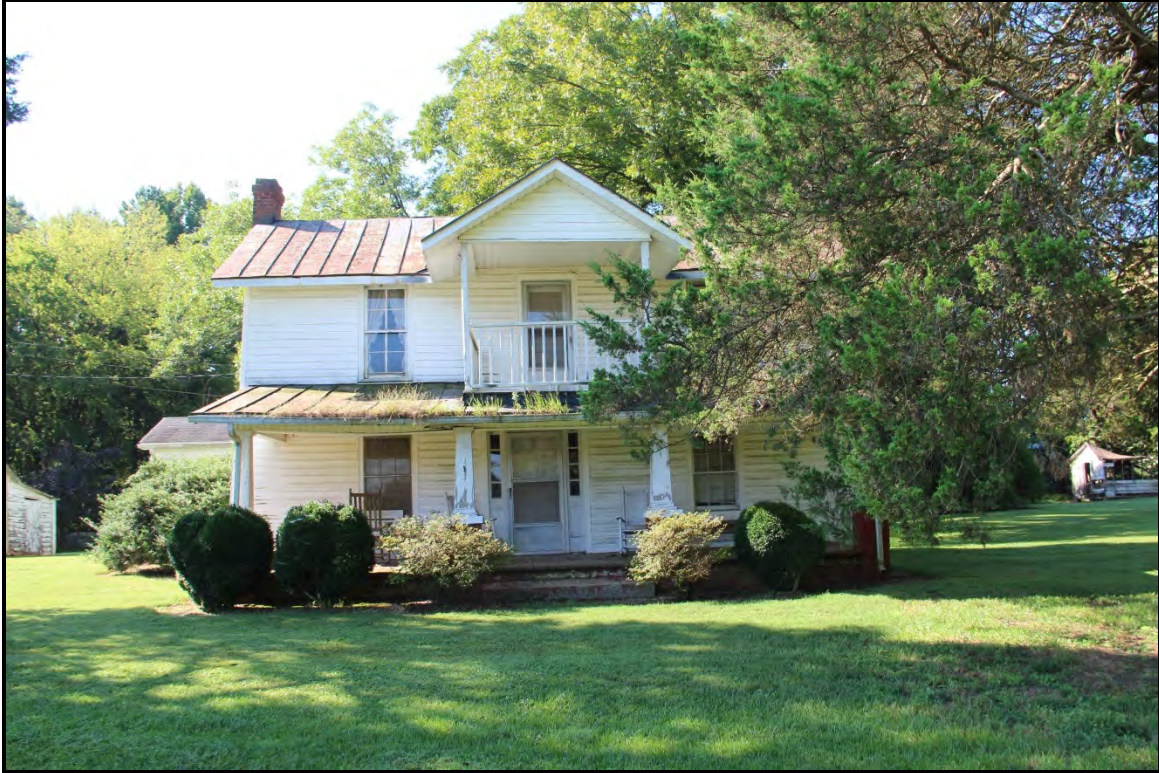
Figure 6.84. Architectural resource AM2514; view is south featuring the façade.
