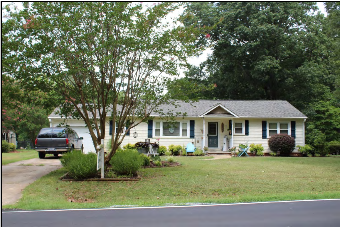
Figure 6.282. Architectural resource AM2610; view is northwest and features the façade.
