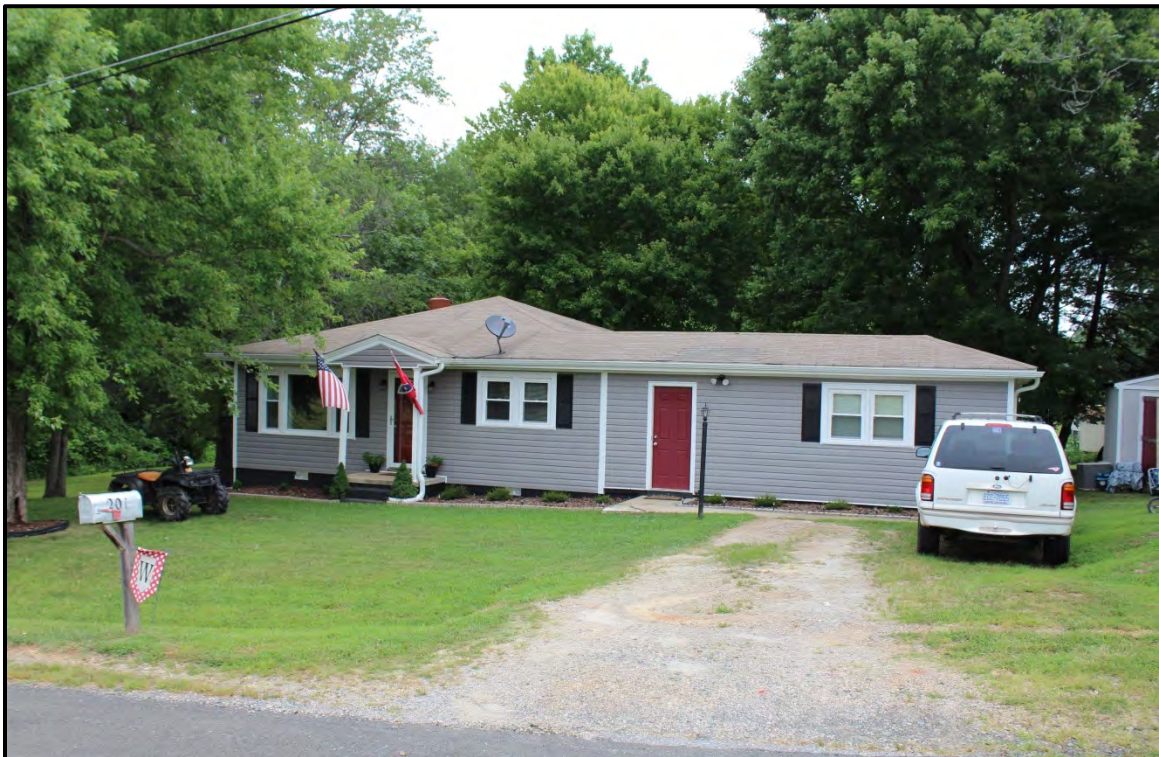
Figure 5.189. Architectural resource RK1727; view is northeast featuring the façade.
