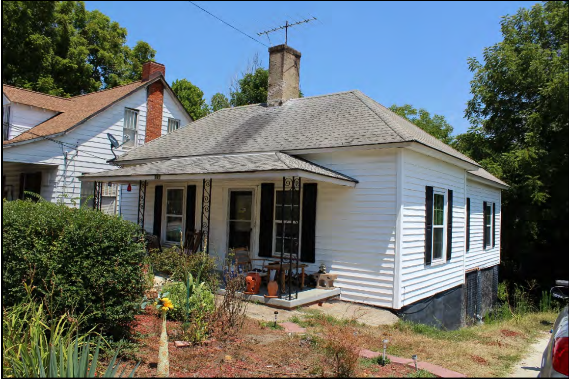
Figure 6.216. Architectural resource AM1595; view is northeast featuring 243 East Main Street.
