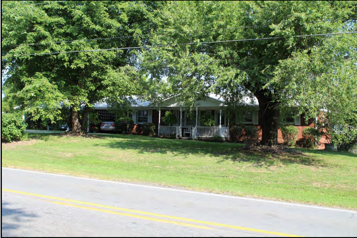
Figure 5.133. Architectural resource RK1697; view is northwest featuring the façade.
