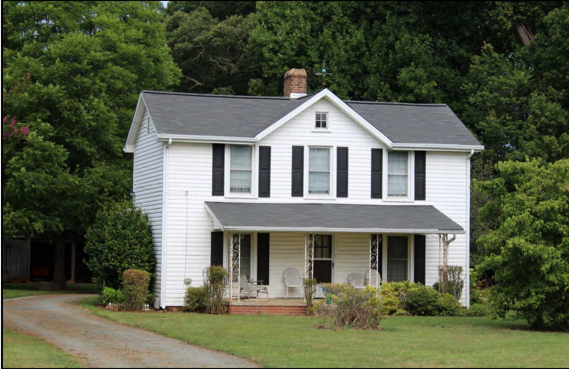
Figure 6.103. Architectural resource AM2518; view is northwest featuring the façade and south elevation.
