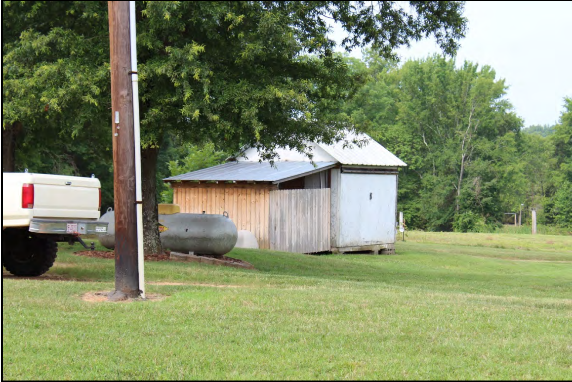
Figure 5.209. Architectural resource RK1738; oblique view featuring the late twentieth century shed.
