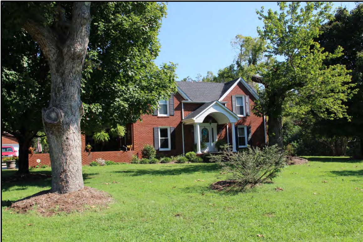
Figure 6.65. Architectural resource AM2504; view northwest featuring the façade.
