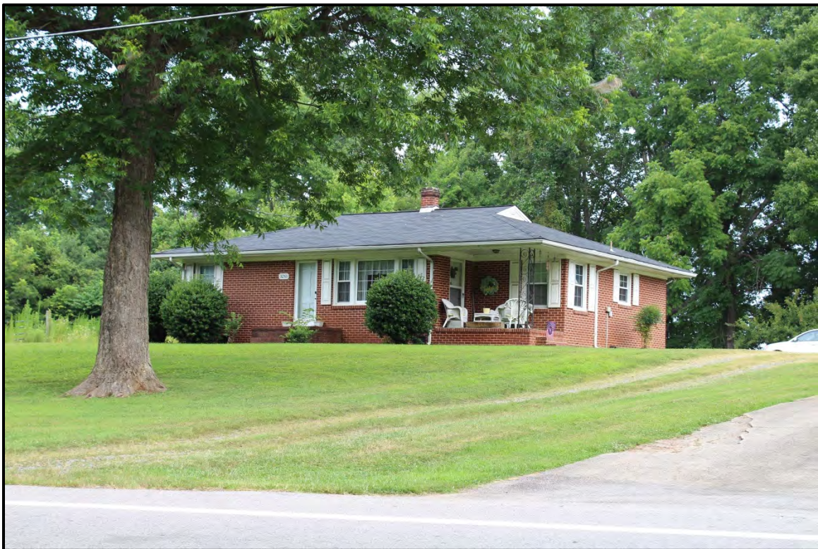
Figure 5.190. Architectural resource RK1728; view is northwest featuring the façade and northeast elevation.
