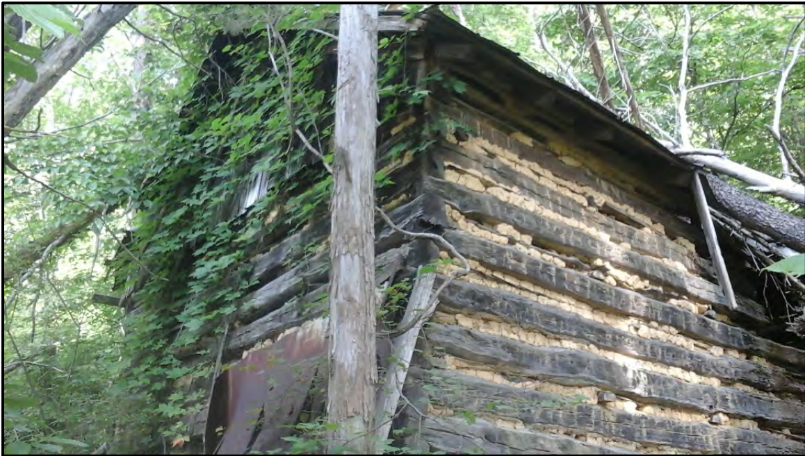
Figure 5.121. Architectural resource RK1689; view of upper wall and log detail.
