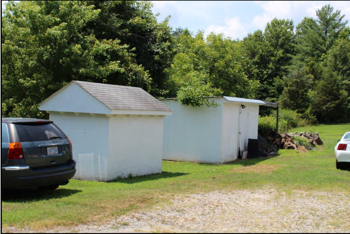
Figure 5.180. Architectural resource RK1722; view is southwest featuring the associated outbuildings.
