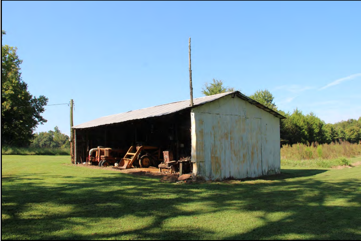
Figure 6.90. Architectural resource AM2514; view is southwest featuring the tractor shed.
