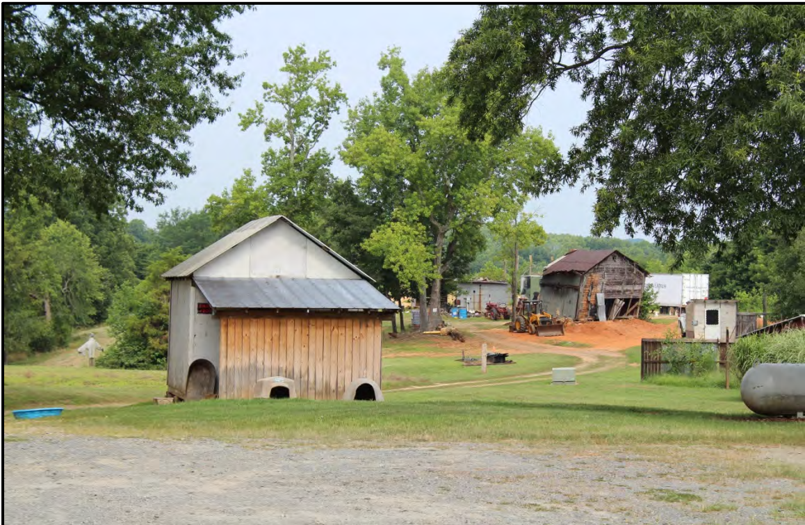
Figure 5.210. Architectural resource RK1738; view is northwest and features the late twentieth century shed and early twentieth century barn.
