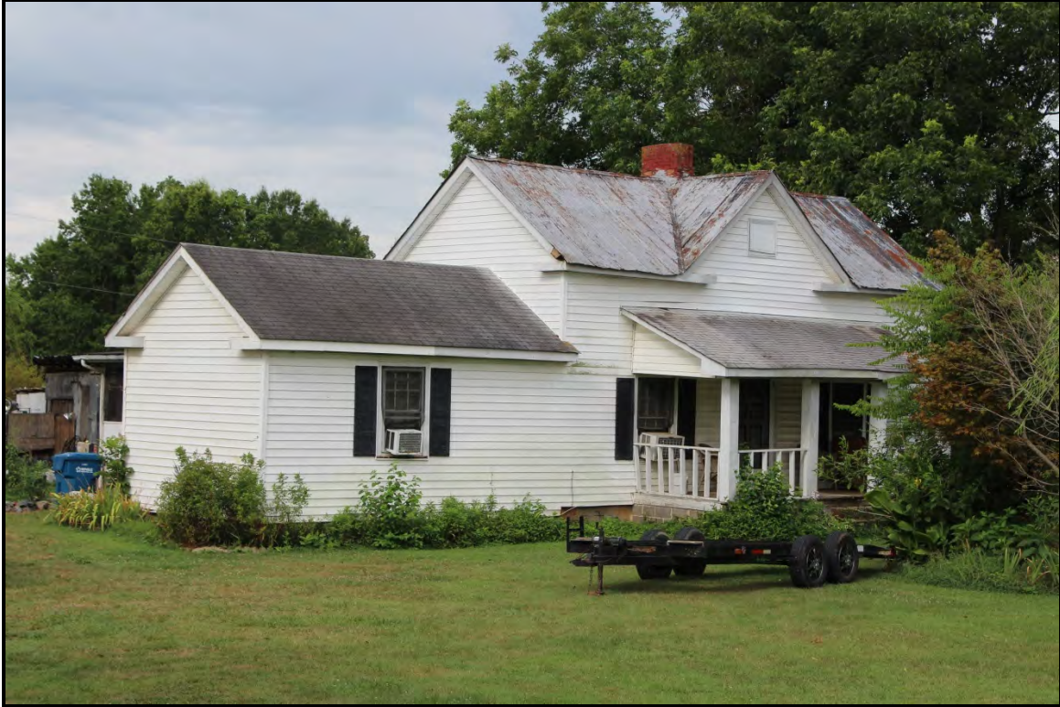
Figure 6.82. Architectural resource AM2512; view is west featuring the façade and east elevation.
