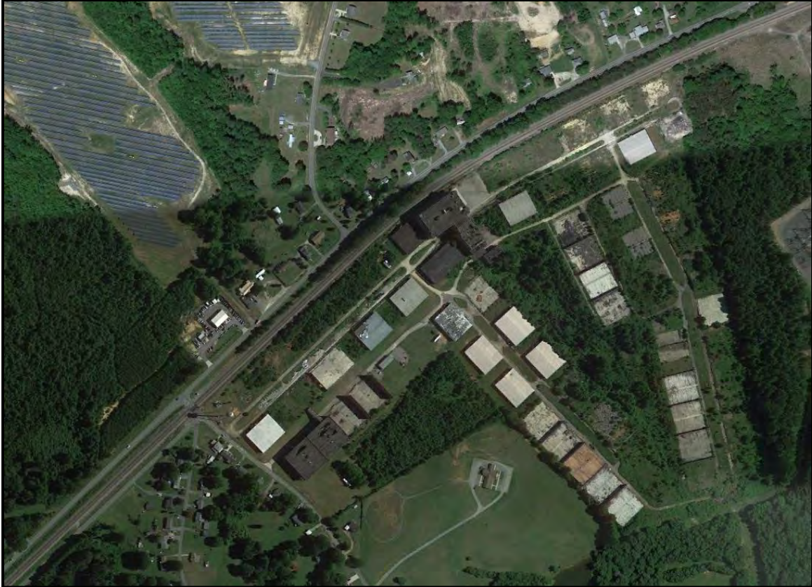
Figure 5.156. 2018 Google Earth aerial imagery depicting The American Tobacco Company manufacturing grounds after its closure and resulting demolition.
