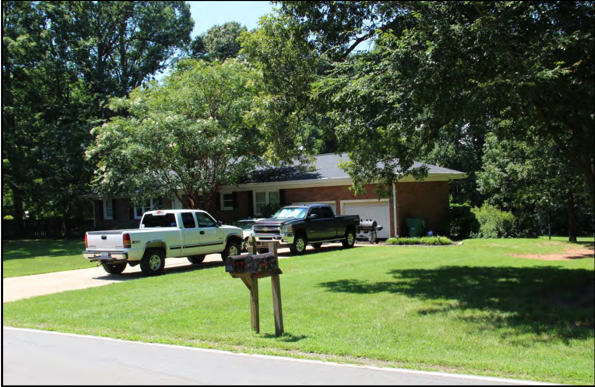
Figure 5.299. Architectural resource RK1761; view is southwest and features the façade and northeast elevation.
