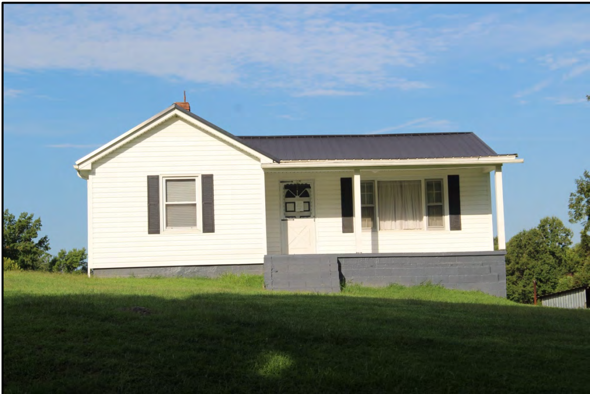
Figure 5.58. Architectural resource RK1666; view is southwest featuring the façade.
