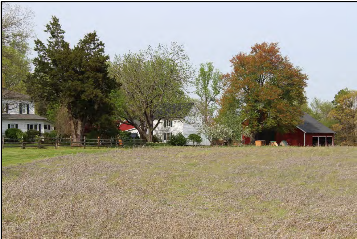
Figure 6.39. Architectural resource AM1529; view is northeast featuring the hay barn and potential seed storage building.
