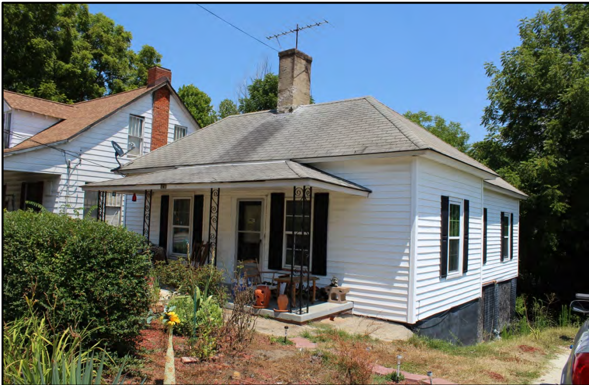
Figure 6.205. Architectural resource AM2594; view is northeast and features the façade and south elevation.
