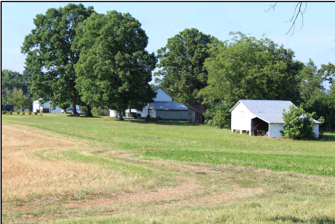
Figure 6.32. Architectural resource AM2493; view is southwest, featuring an overview of the property.
