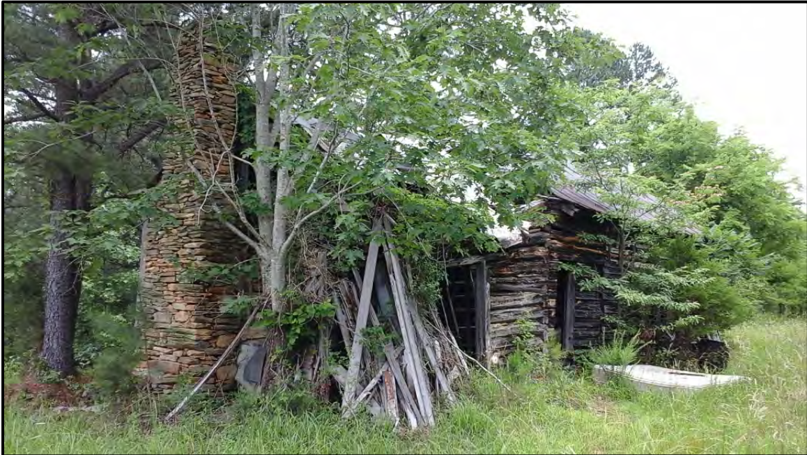
Figure 5.78. Architectural resource RK1678; view is southeast featuring the north and west (rear) elevations.
