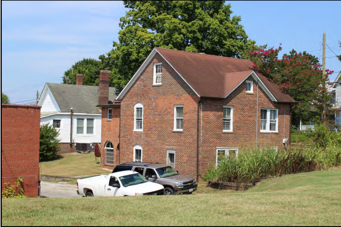
Figure 6.198. Architectural resource AM2588; view is northwest featuring the east and south (rear) elevations of the Folk Victorian-style house.
