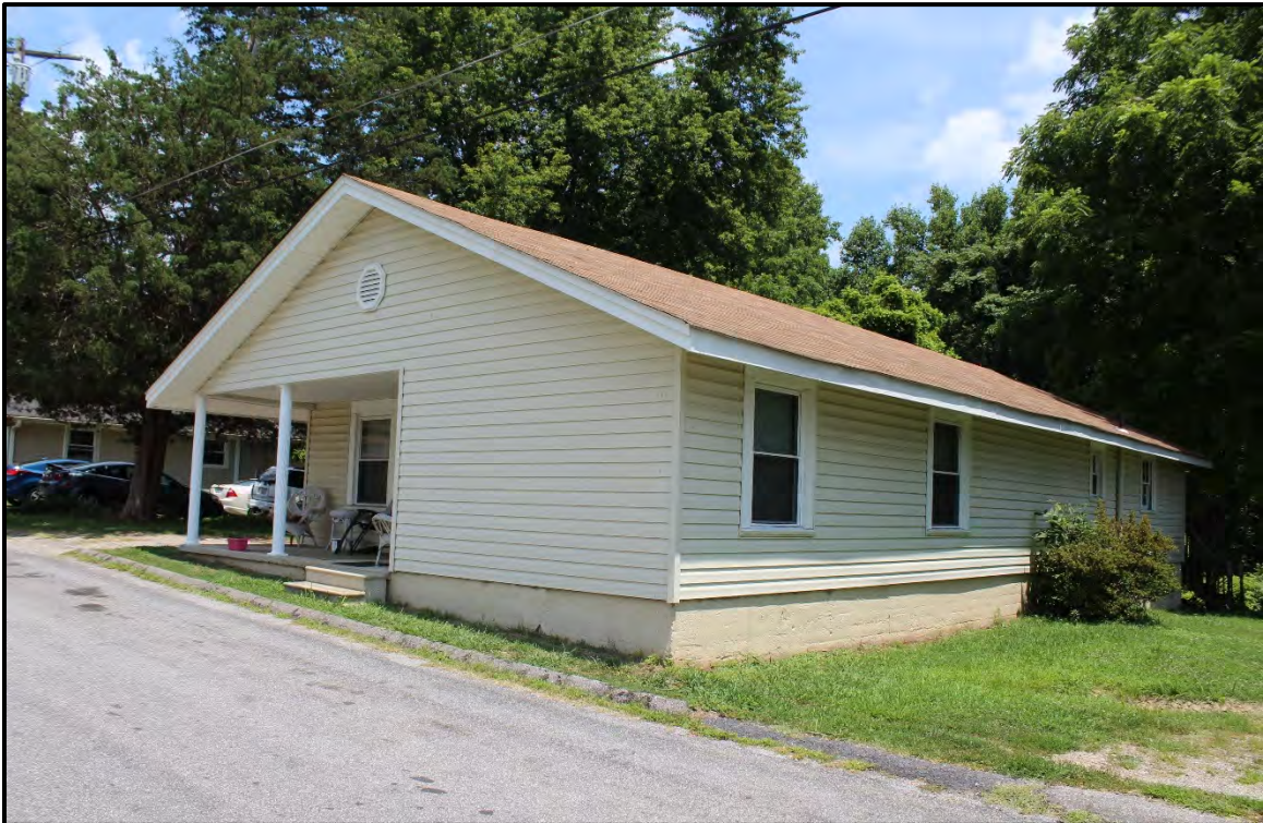
Figure 5.173. Architectural resource RK1719; view is north showing the façade and southeast elevation.
