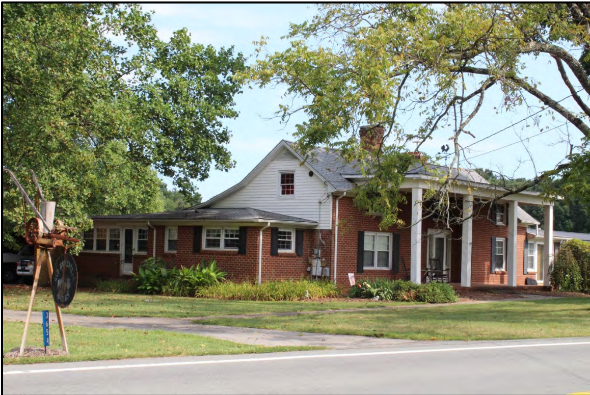
Figure 6.95. Architectural resource AM2516; view is northwest and features the façade and south elevation.
