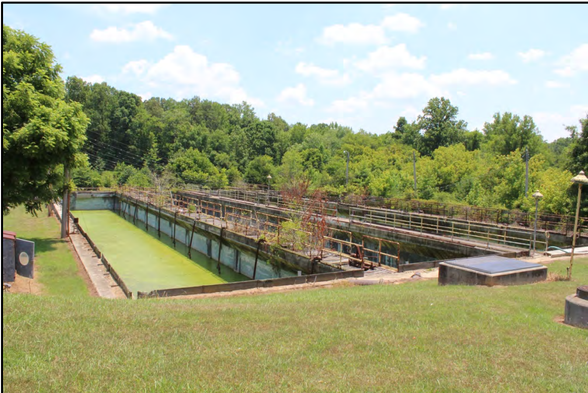
Figure 6.276. Architectural resource AM2604; view is southeast and features the sediment tanks.
