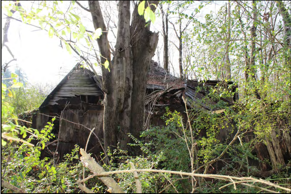
Figure 6.8. Architectural resource AM1520; view is west featuring one of three collapsed outbuildings.
