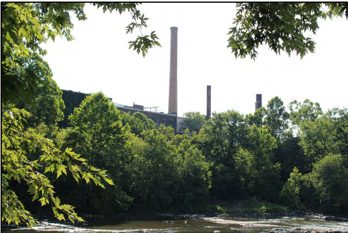
Figure 6.226. Granite Mill; view is southeast from across the Haw River featuring associated smokestacks and portions of the west elevation of Building 10.
