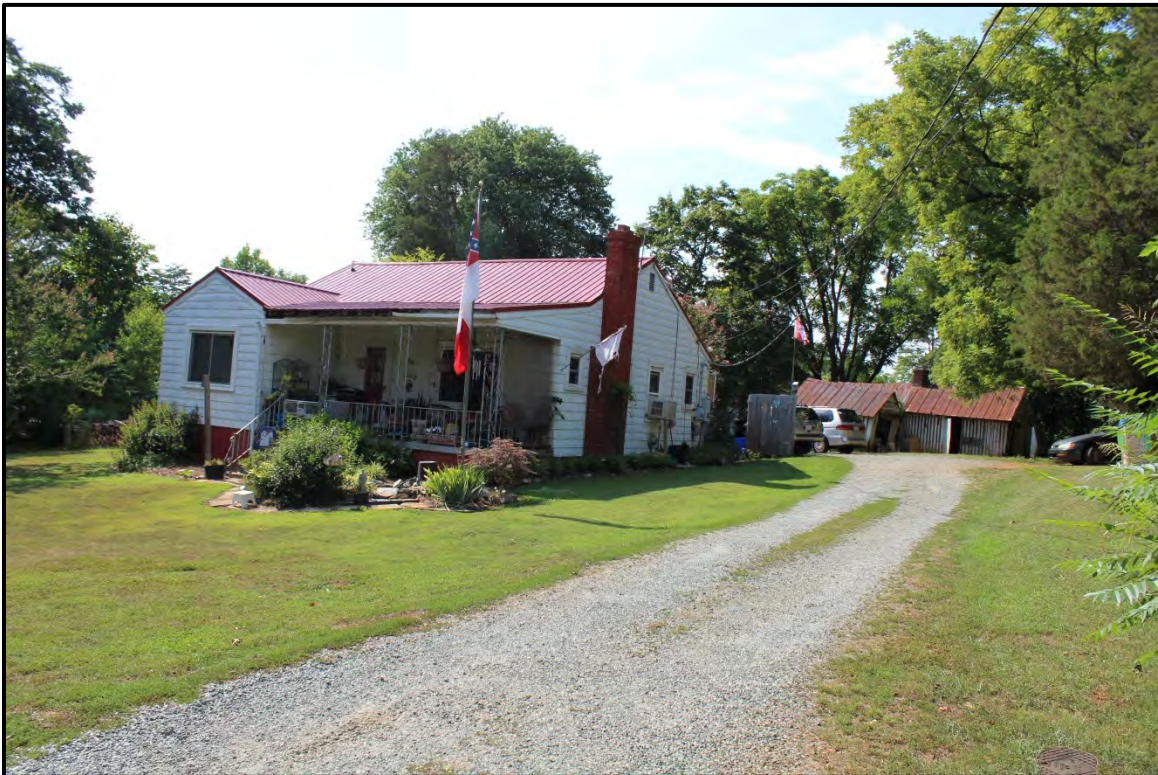
Figure 6.183. Architectural resource AM2579; view is northwest featuring the façade and northeast elevation.
