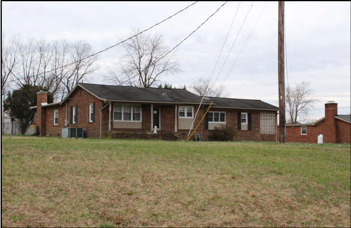
Figure 4.50. Architectural resource AM2640; view is southwest featuring the façade and east elevation.
