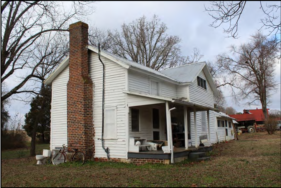
Figure 4.74. Architectural resource AM2631; view is north featuring the façade and southwest elevation of the ca. 1893 log-frame house.
