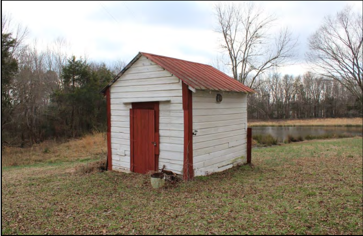
Figure 4.78. Architectural resource AM2631; view is southeast featuring the mid-twentieth century storage shed.
