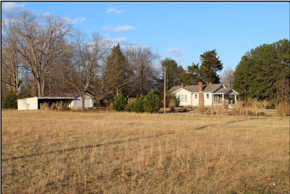
Figure 3.11. Architectural resource GF9109; view is northeast featuring the modern garage and attached vehicle shed.
