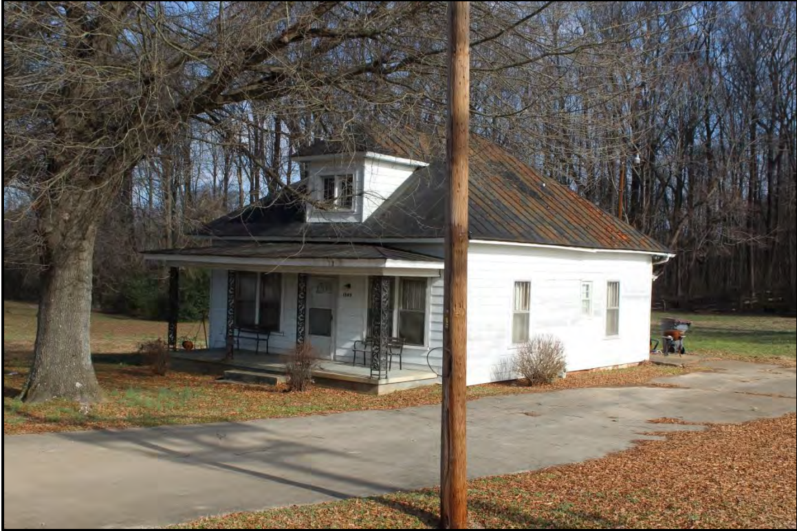
Figure 2.129. Architectural resource RK1808; view is northeast and features the façade and south elevation.
