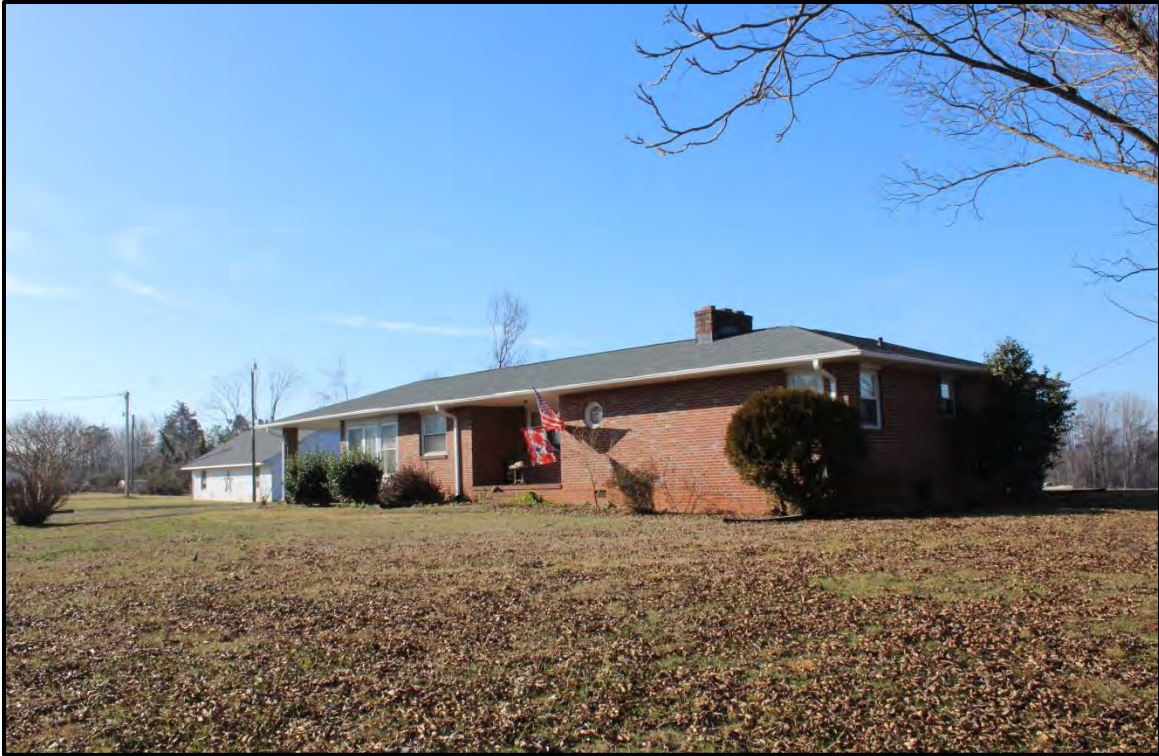
Figure 2.69. Architectural resource RK1799; view is northeast featuring the façade and south elevation.
