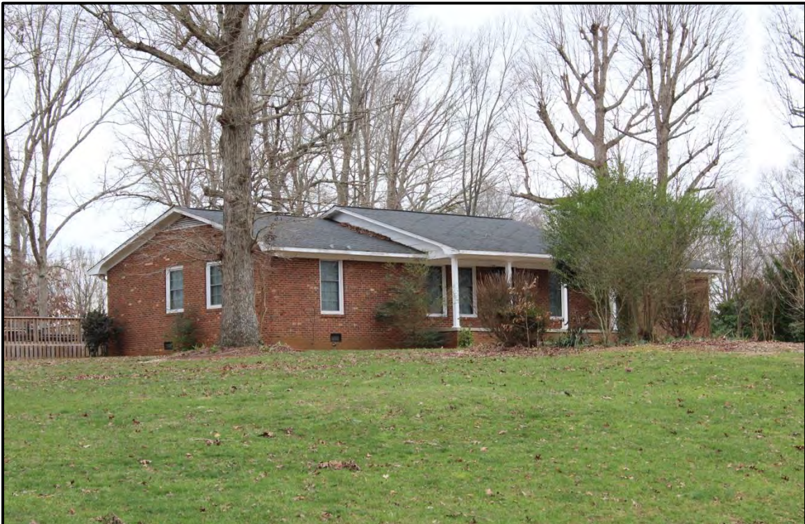
Figure 4.71. Architectural resource AM2637; view is southwest featuring the façade and east elevation.
