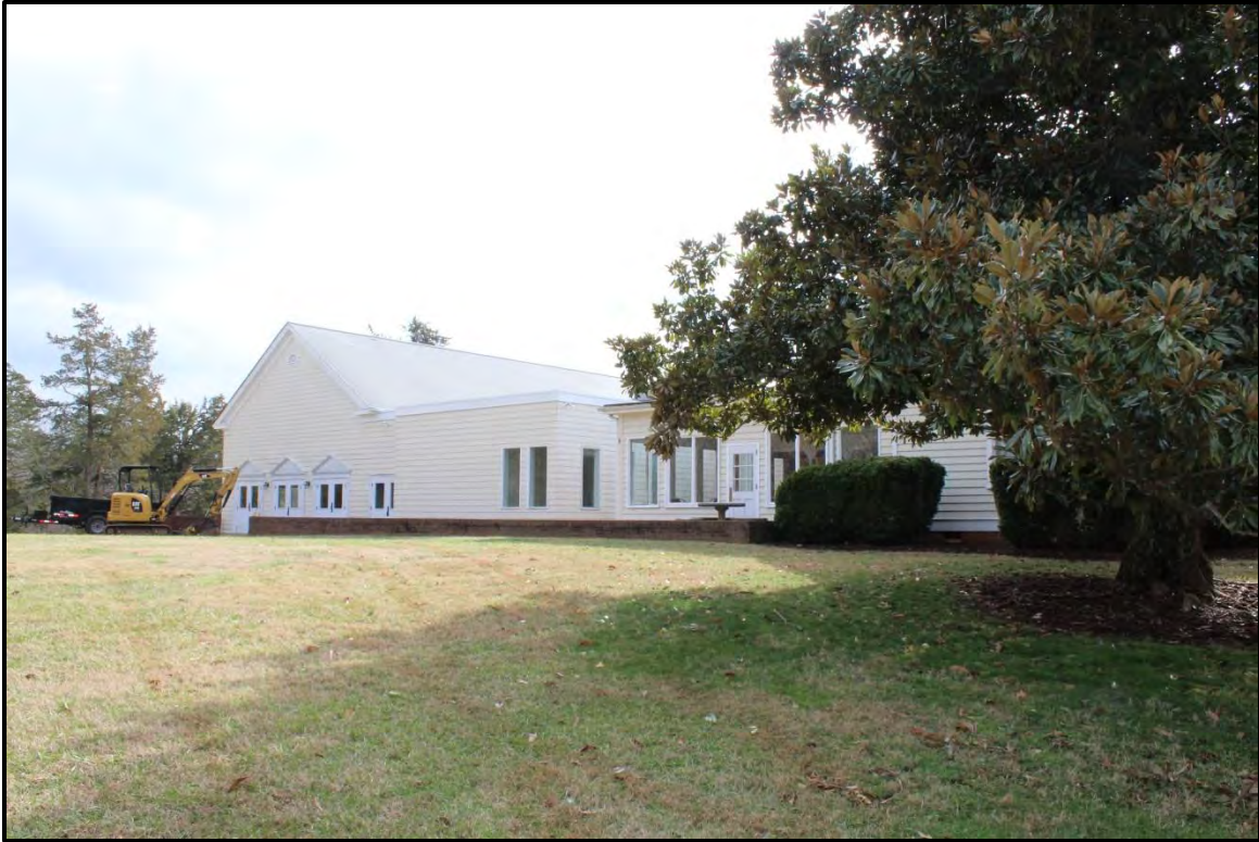
Figure 4.43. Architectural resource AM0360; view is southeast featuring the 1989 addition.
