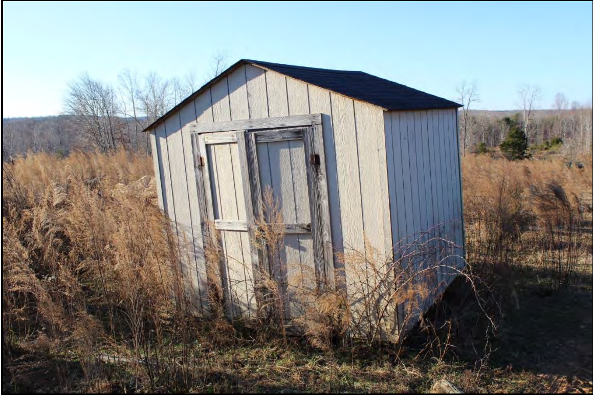
Figure 2.41. Architectural resource RK1792; view is southwest featuring the late twentieth century storage shed.
