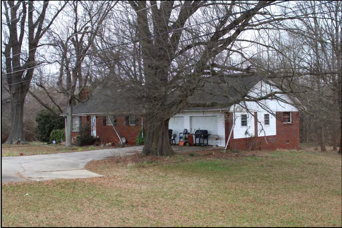
Figure 2.160. Architectural resource RK1817; view is northeast and features the façade and south elevation.
