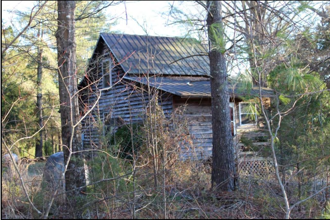
Figure 2.96. Architectural resource RK1800; view is southwest featuring the façade and east elevation.
