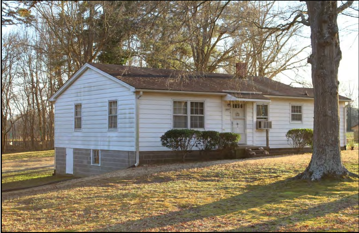
Figure 3.20. Architectural resource GF9114; view is southwest featuring the façade and east elevation.
