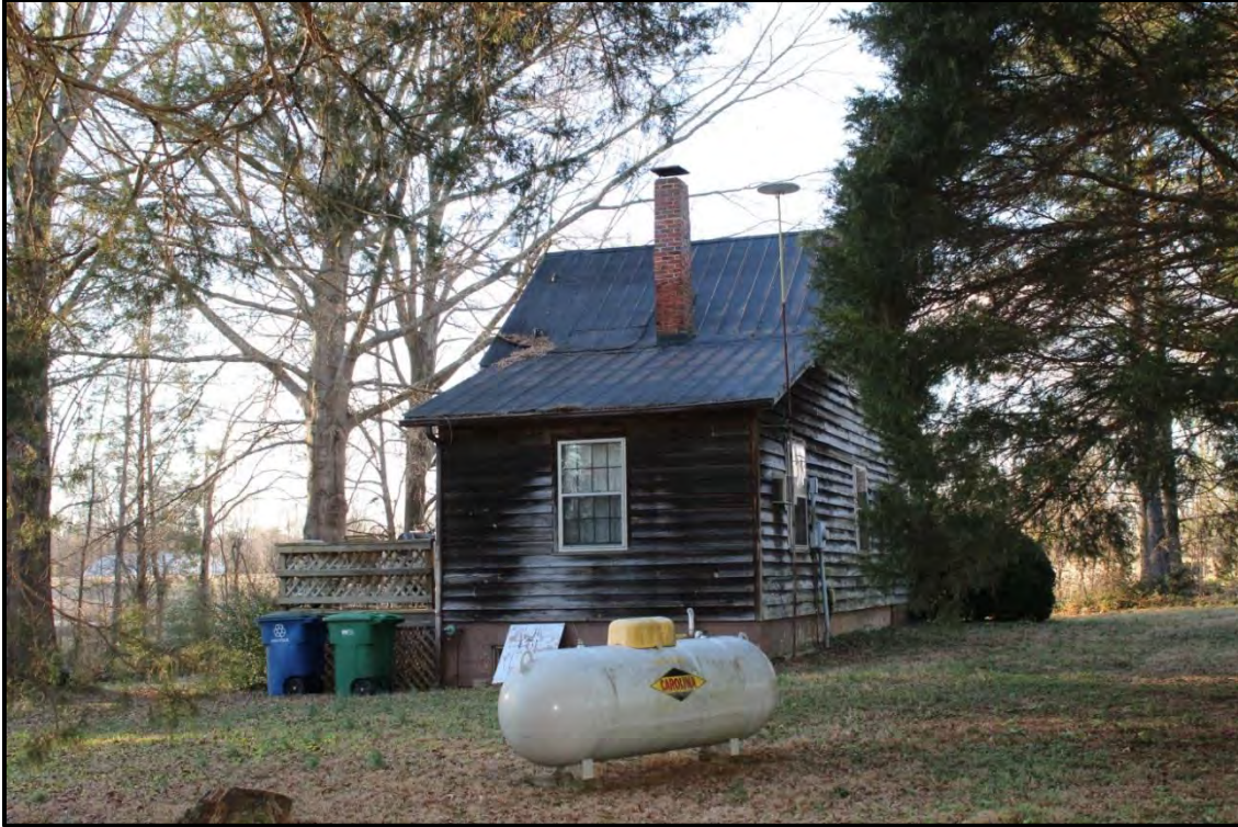
Figure 2.98. Architectural resource RK1800; view is northwest featuring the south (rear) and east elevations.
