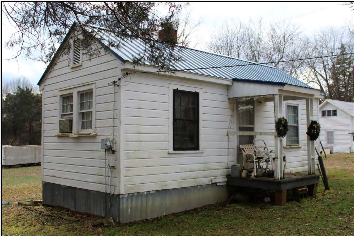
Figure 4.81. Architectural resource AM2631; view is southwest featuring the façade and east elevation of the ca. 1957 side-gabled house.
