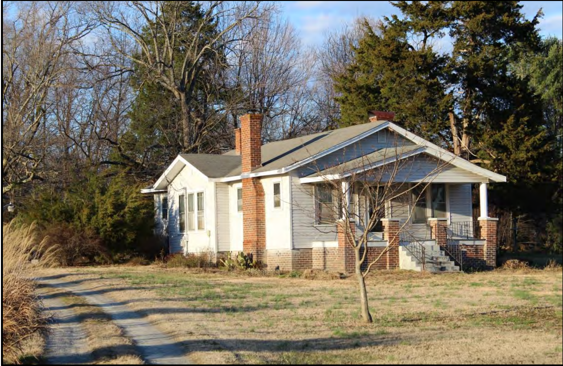
Figure 3.10. Architectural resource GF9109; view is northeast featuring the façade and west elevation.
