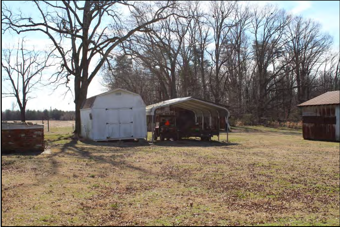
Figure 4.110. Architectural resource AM2635; view is west featuring a modern carport, a prefabricated storage shed, and the pump shed.
