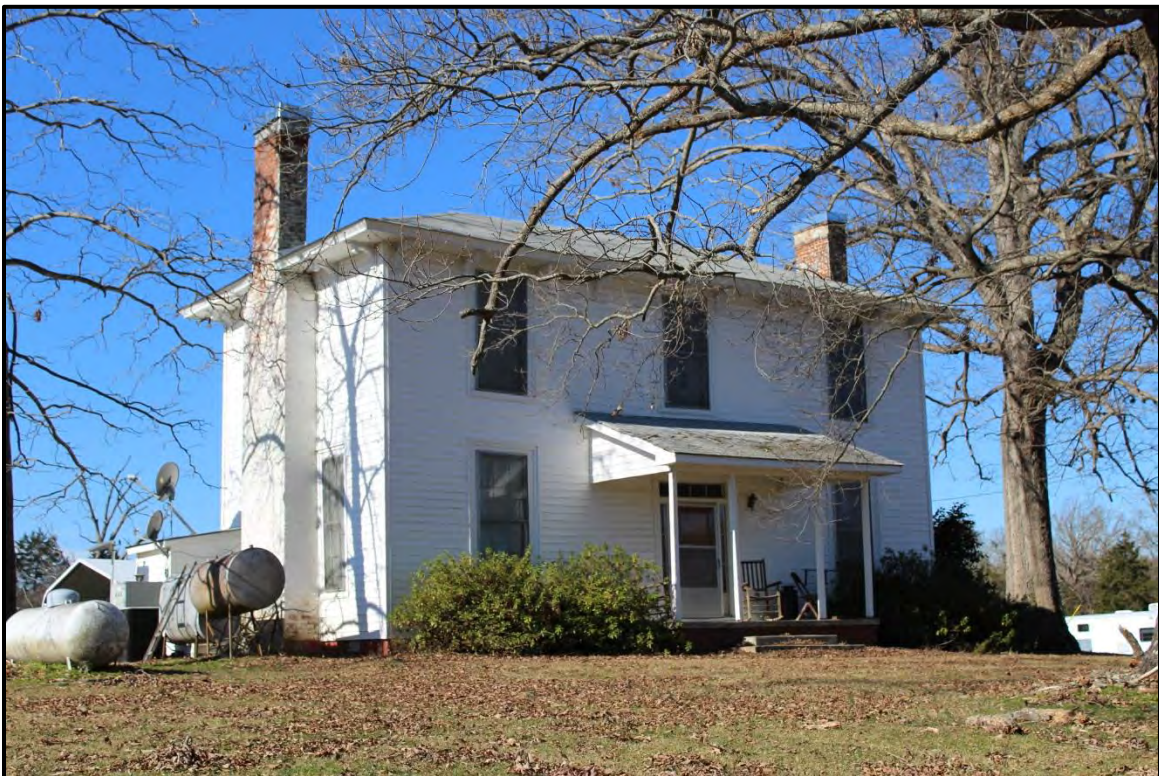
Figure 4.107. Architectural resource AM2635 farmhouse; view is northwest featuring the façade and south elevation.
