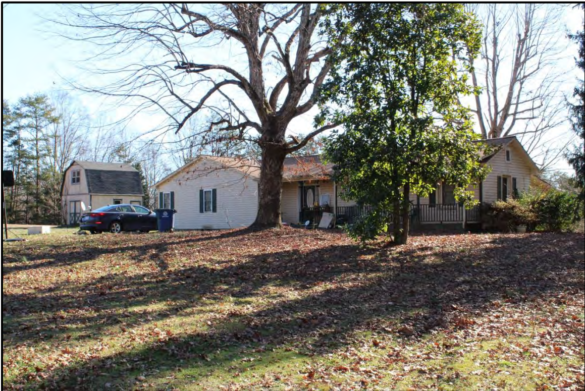
Figure 2.23. Architectural resource RK1789; view is southeast featuring the façade and the west elevation.
