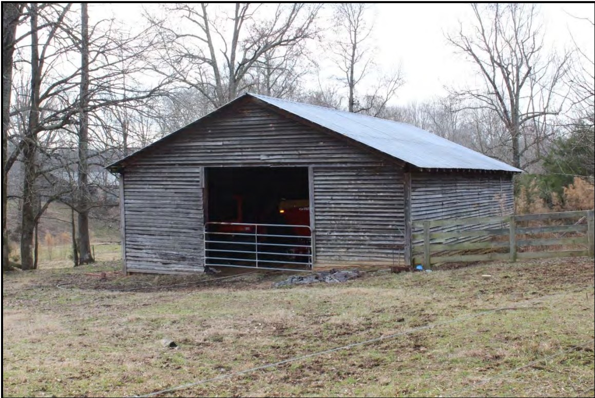
Figure 2.64. Architectural resource RK1820; view is south and features the ca. 1940 tractor barn.
