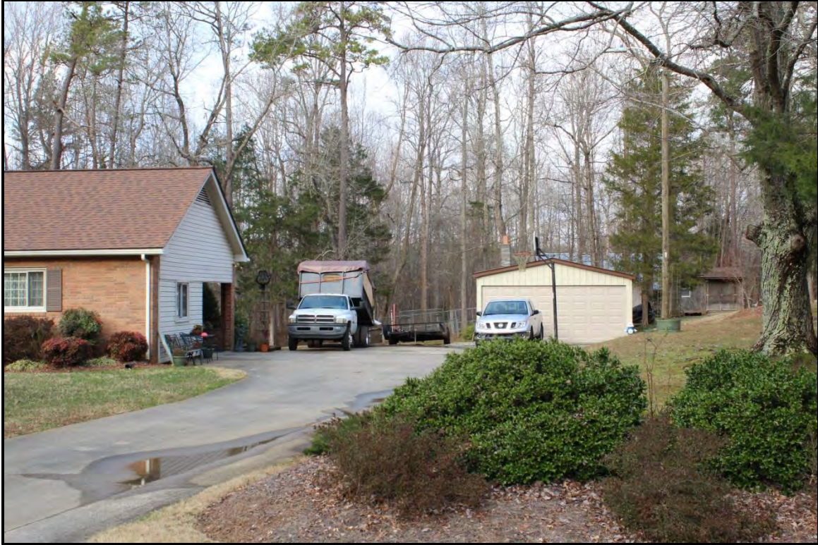
Figure 4.152. Architectural resource AM2651; view is north featuring the modern garage.
