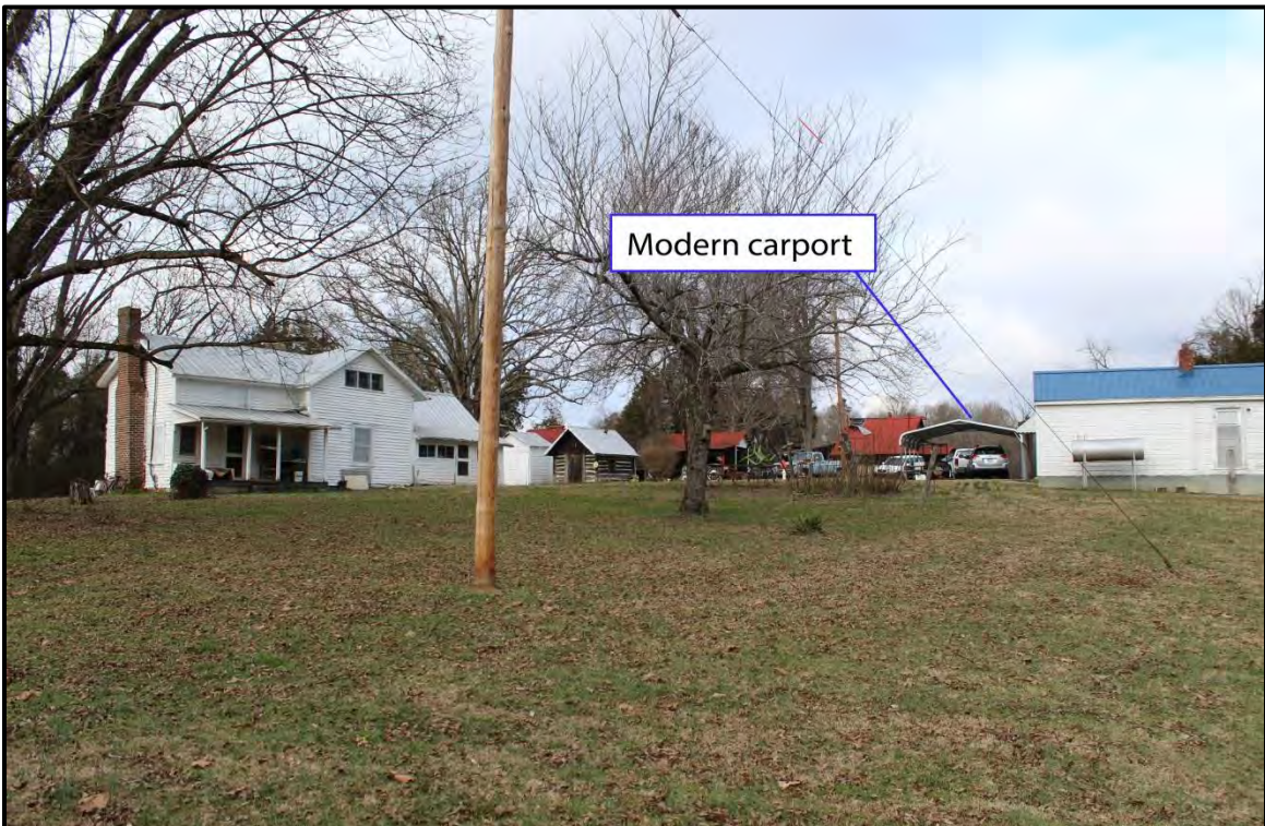
Figure 4.97. Overview of architectural resource AM2631; with the modern carport identified left of the ca. 1956 house.
