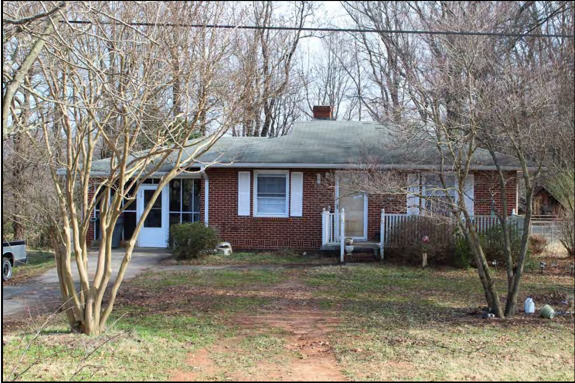
Figure 2.134. Architectural resource RK1810; view is east and features the façade.
