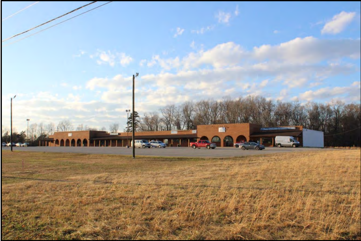
Figure 3.3. Architectural resource GF1536; view is northwest featuring the façade and east elevation wing.
