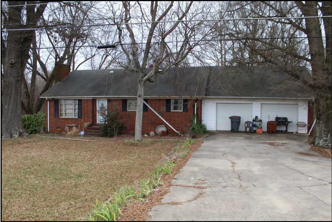
Figure 2.158. Architectural resource RK1817; view is east and features the façade.
