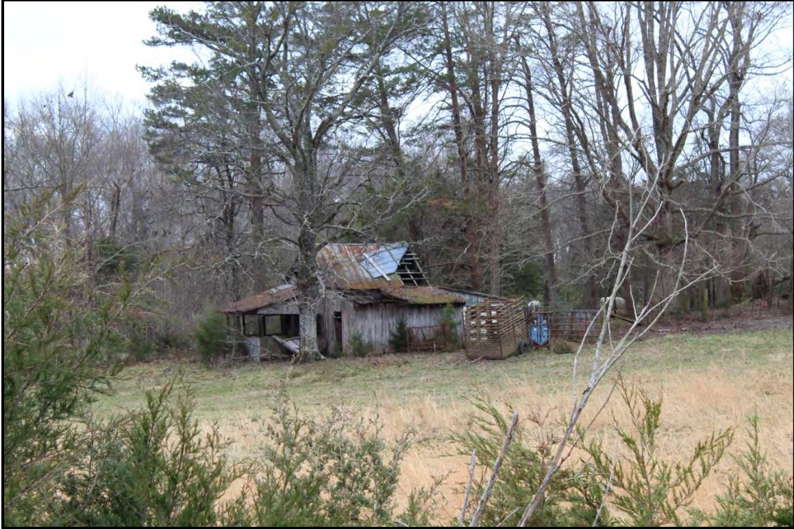
Figure 4.102. Architectural resource AM2652; view is south featuring the feed barn.
