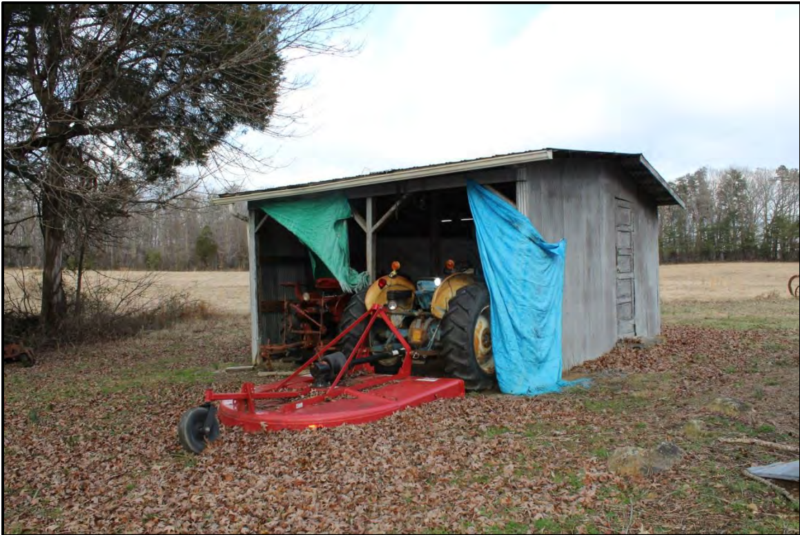
Figure 4.91. Architectural resource AM2631; view is northwest featuring the modern tractor shed.
