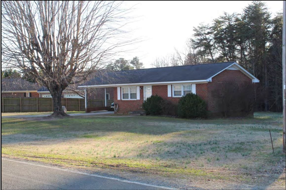
Figure 4.57. Architectural resource AM2643; view is southwest featuring the façade and north elevation.
