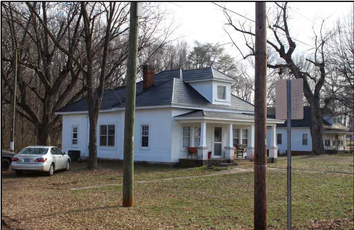
Figure 2.132. Architectural resource RK1809; view is southeast and features the façade and north elevation.
