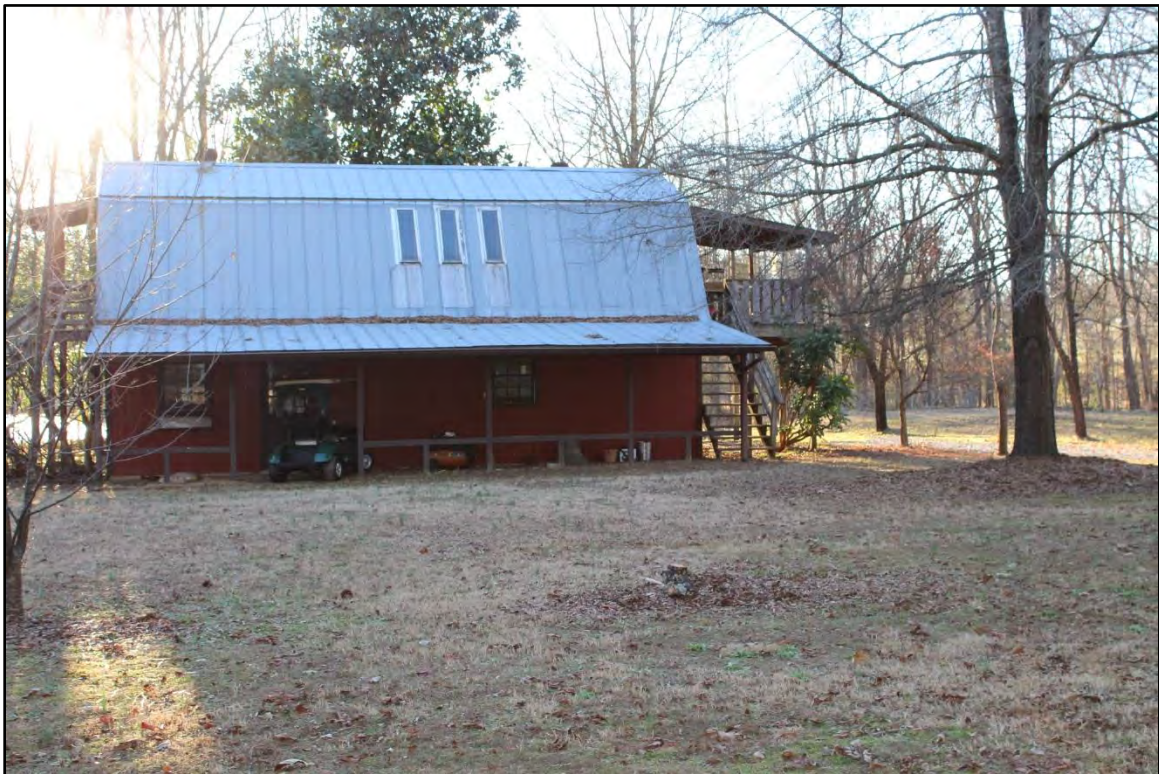
Figure 2.100. Architectural resource RK1801; view is west featuring the renovated barn.
