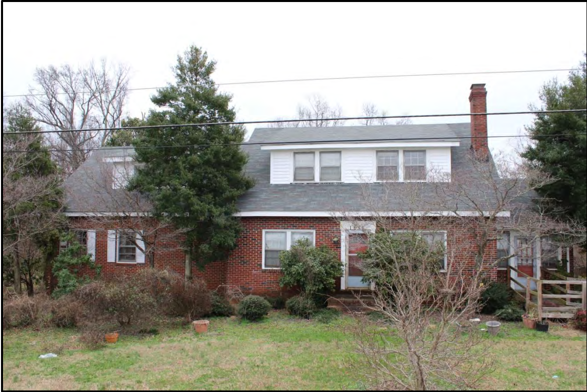
Figure 2.154. Architectural resource RK1816; view is east and features the façade.
