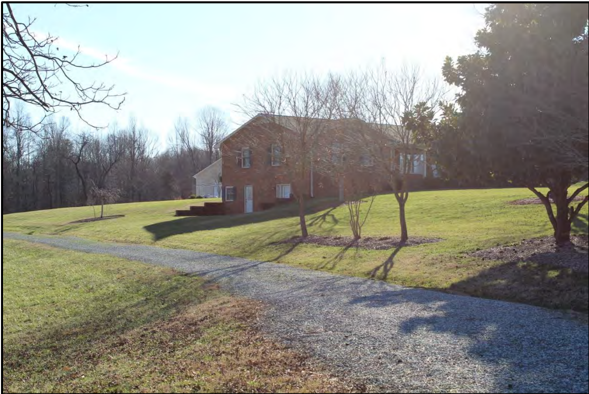
Figure 4.35. Architectural resource AM2626; view is southwest featuring the east elevation.
