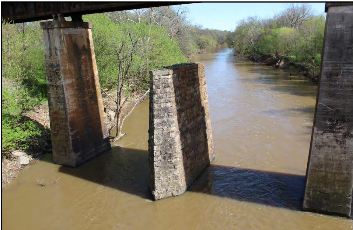
Figure 4.155. Architectural resource AM1324; view is southeast featuring the original polygon-shaped bridge pier (AM0184).
