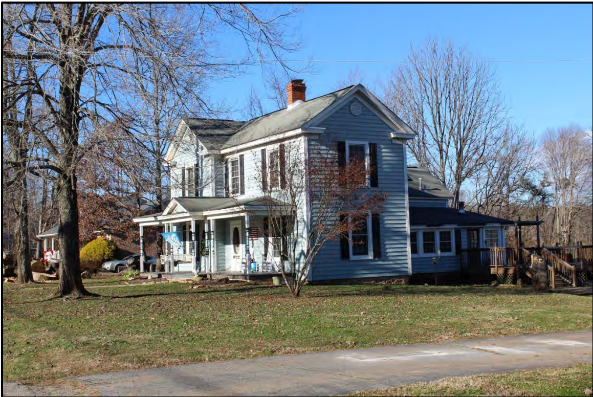
Figure 2.57. Architectural resource RK1796; view is northwest featuring the façade and east elevation.
