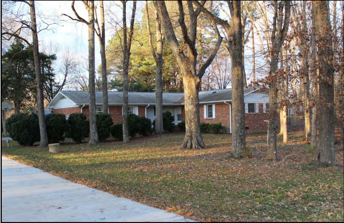
Figure 3.16. Architectural resource GF9112; view is northeast featuring the façade and west elevation.
