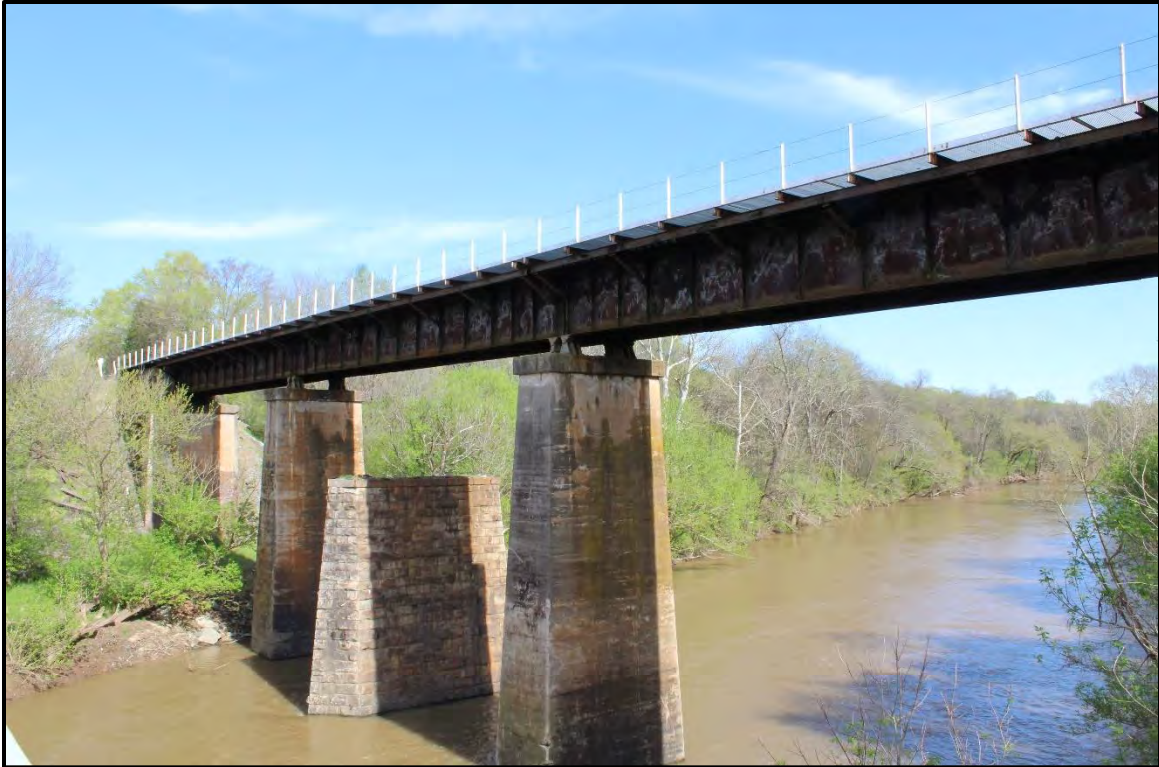
Figure 4.154. Architectural resource AM1324; view is east featuring the north elevation of the bridge.
