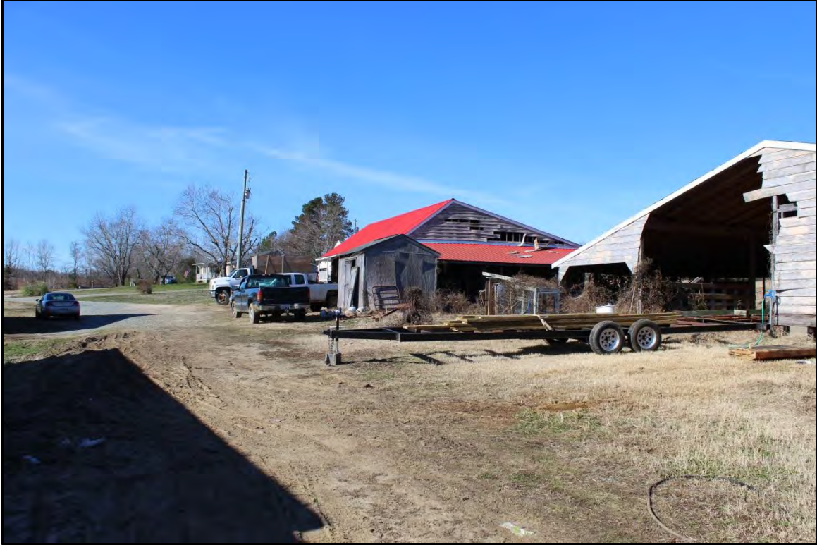
Figure 4.135. Architectural resource AM2634; view is west featuring the late twentieth century shed in the foreground.
