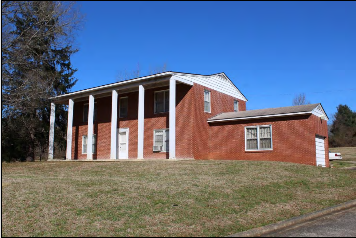
Figure 4.142. Architectural resource AM2644; view is north featuring the façade and southeast elevation garage wing.
