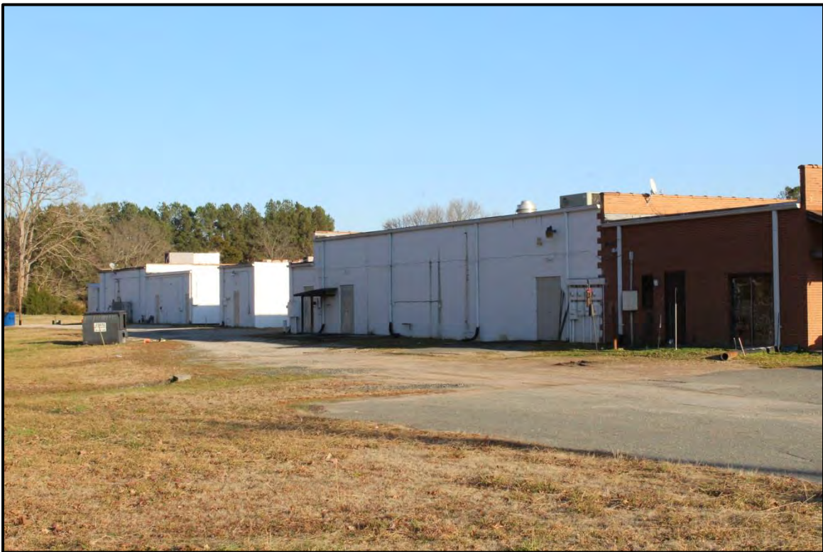
Figure 3.4. Architectural resource GF1536; view is southeast featuring the north (rear) elevation.
