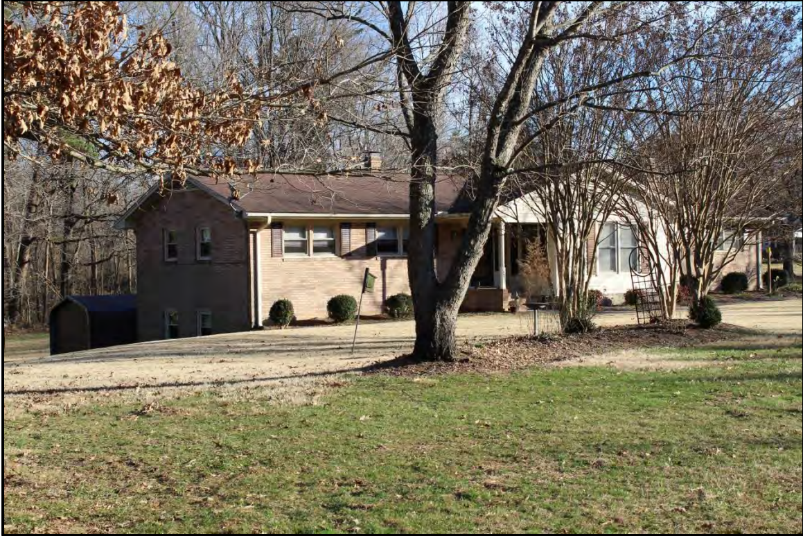
Figure 4.8. Architectural resource AM2619; view is northwest featuring the façade and south elevation.
