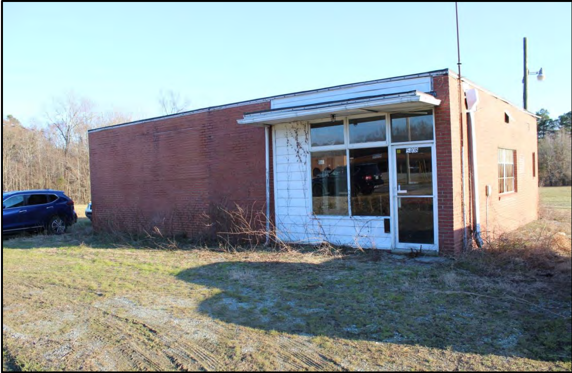
Figure 3.22. Architectural resource GF9115; view is southeast featuring the façade and west elevation.
