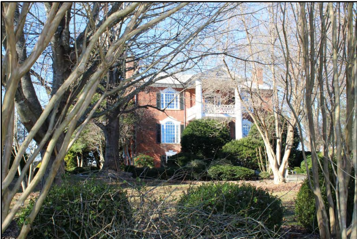
Figure 2.103. High Rock Farm; view is northwest featuring the façade and obscured south elevation.
