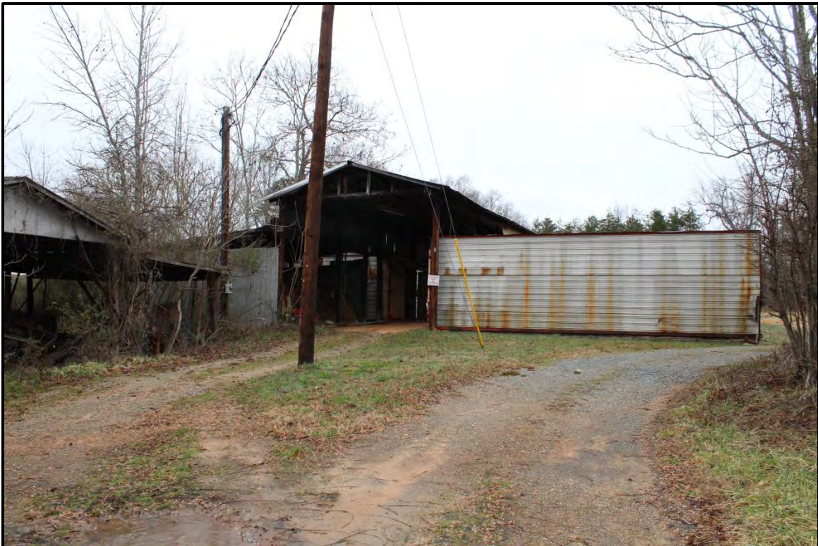
Figure 2.82. Architectural resource RK1818; view is north featuring the ca. 1965 pole shed.
