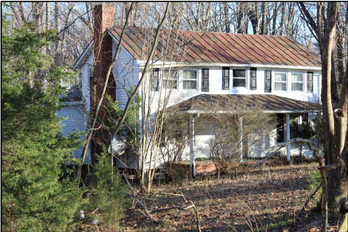
Figure 2.68. Architectural resource RK1798; view is southeast featuring the façade and north elevation.
