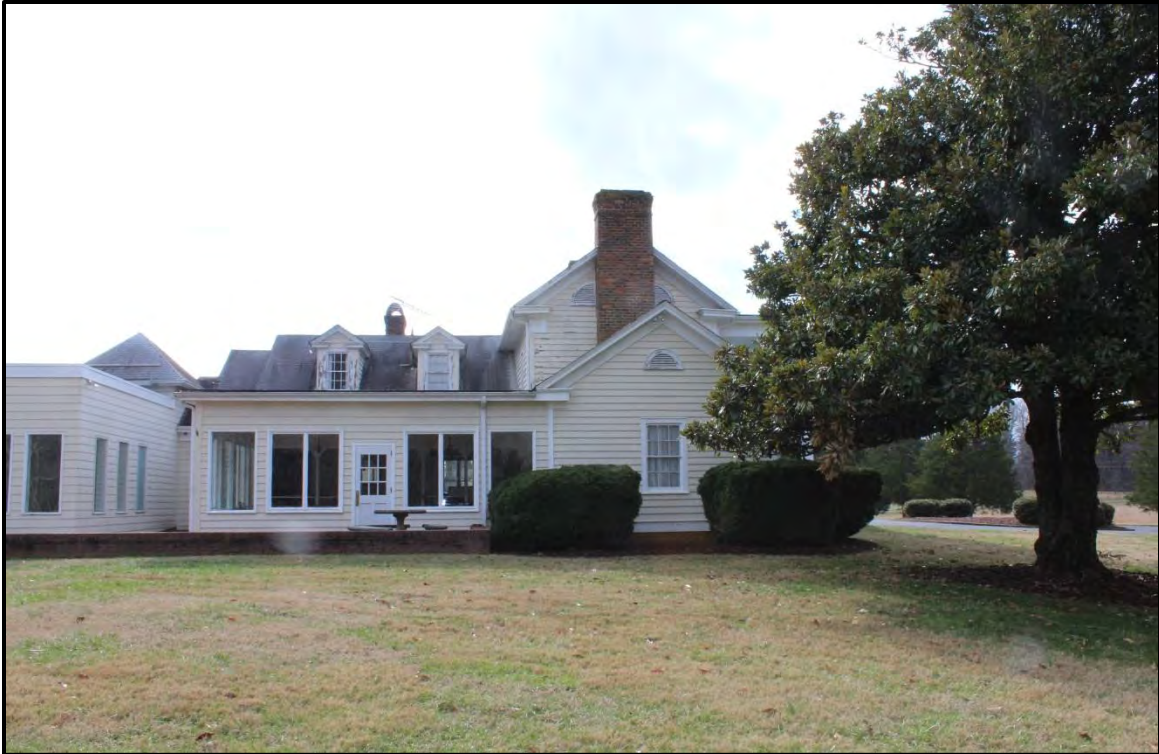
Figure 4.41. Architectural resource AM0360; view is south featuring the north elevation and rear ell with modern alterations.
