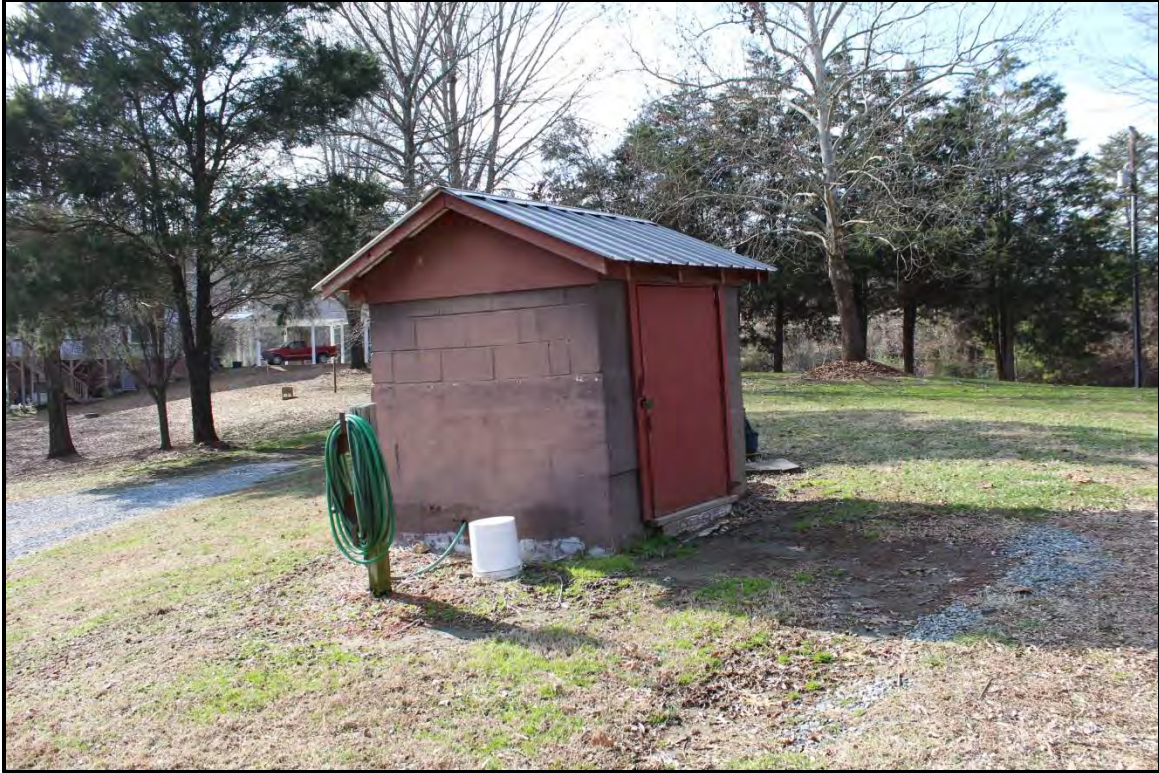
Figure 2.52. Architectural resource RK1794; view is northwest featuring the water pump shed.
