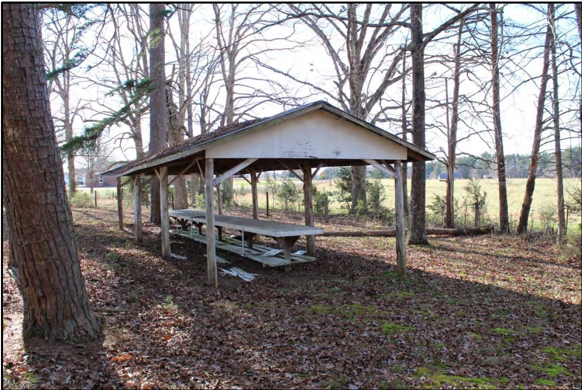
Figure 4.65. Architectural resource AM1603; view is west featuring the pavilion.
