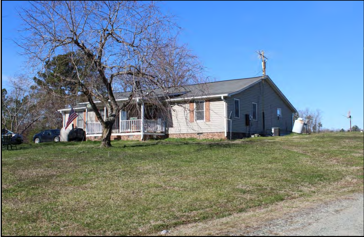
Figure 4.129. Architectural resource AM2634 farmhouse; view is northwest featuring the façade and east elevation.
