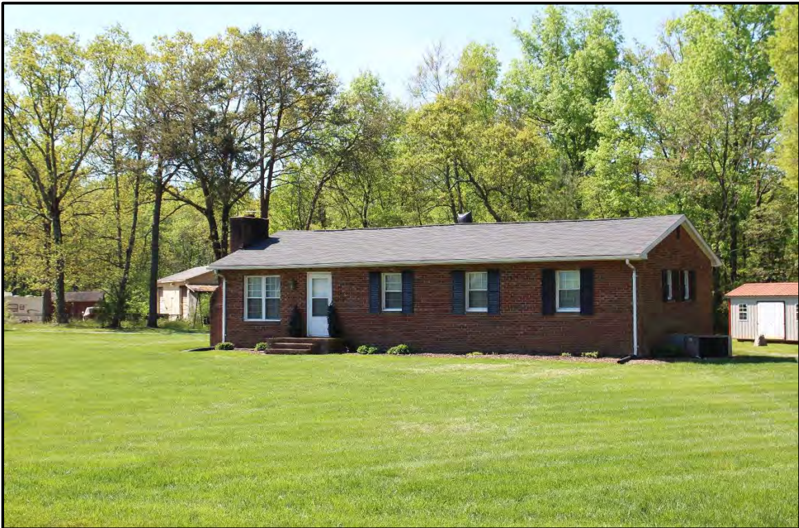
Figure 4.16. Architectural resource AM2654; view is south featuring the façade and northwest elevation.
