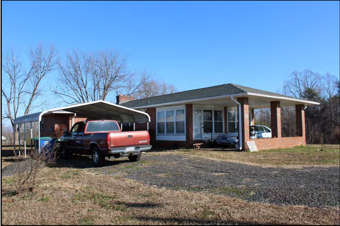
Figure 2.71. Architectural resource RK1799; view is northeast featuring the south and west (rear) elevations.
