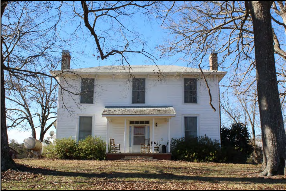
Figure 4.106. Architectural resource AM2635 farmhouse; view is west featuring the façade.
