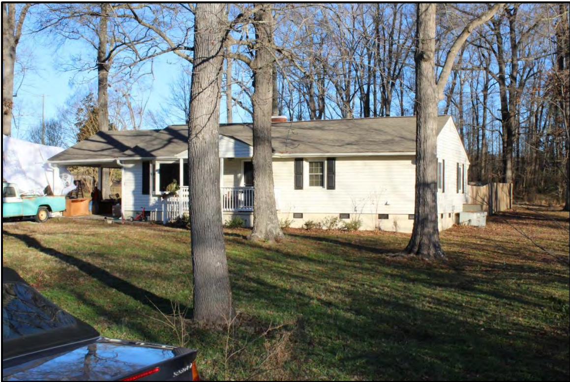
Figure 3.36. Architectural resource GF9119; view is northeast featuring the façade and west elevation.
