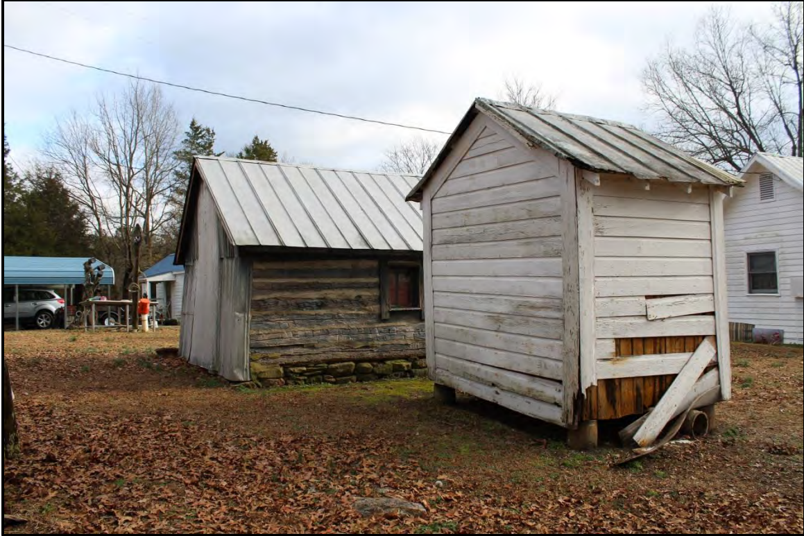
Figure 4.84. Architectural resource AM2631; view is southeast featuring the north (rear) and east elevations of the ca. 1900 log kitchen and adjacent mid-twentieth century shed.
