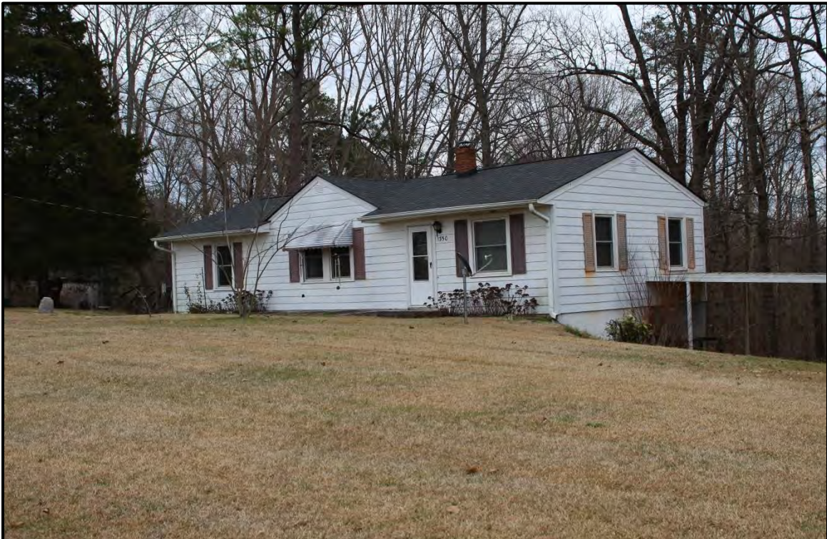
Figure 4.159. Architectural resource AM2647; view is northeast featuring the façade and south elevation.
