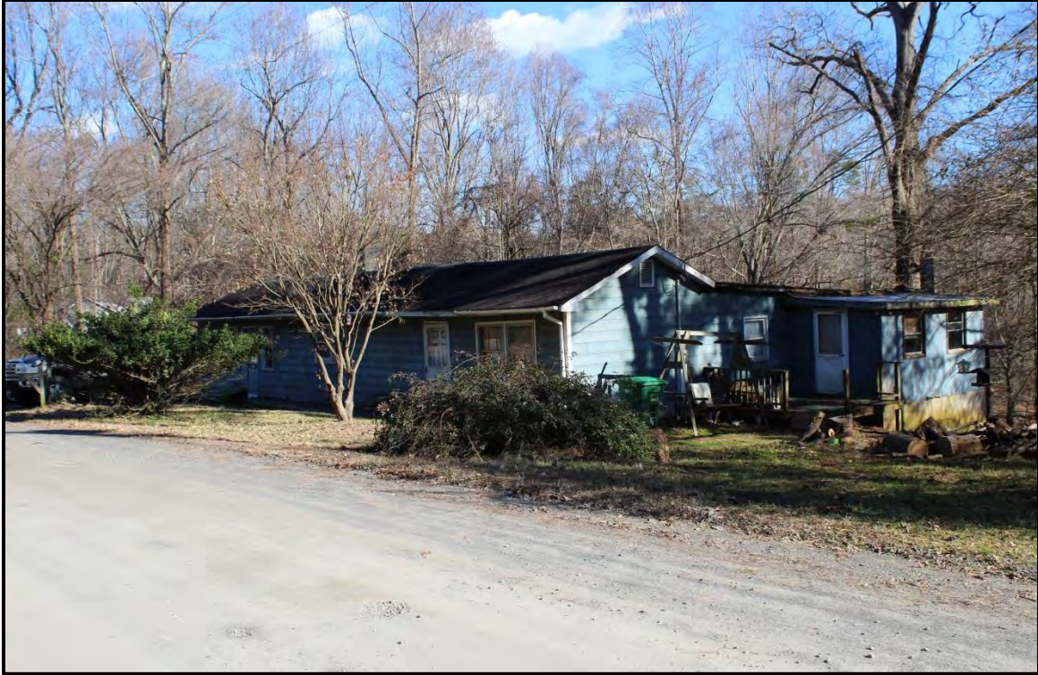
Figure 2.46. Architectural resource RK1793; view is northeast featuring the façade and southwest elevation.
