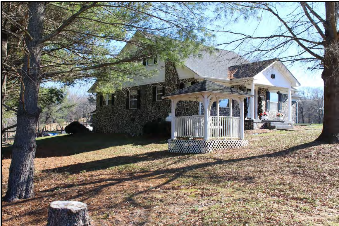
Figure 2.26. Architectural resource RK1790; view is southeast featuring the façade and the north elevation.
