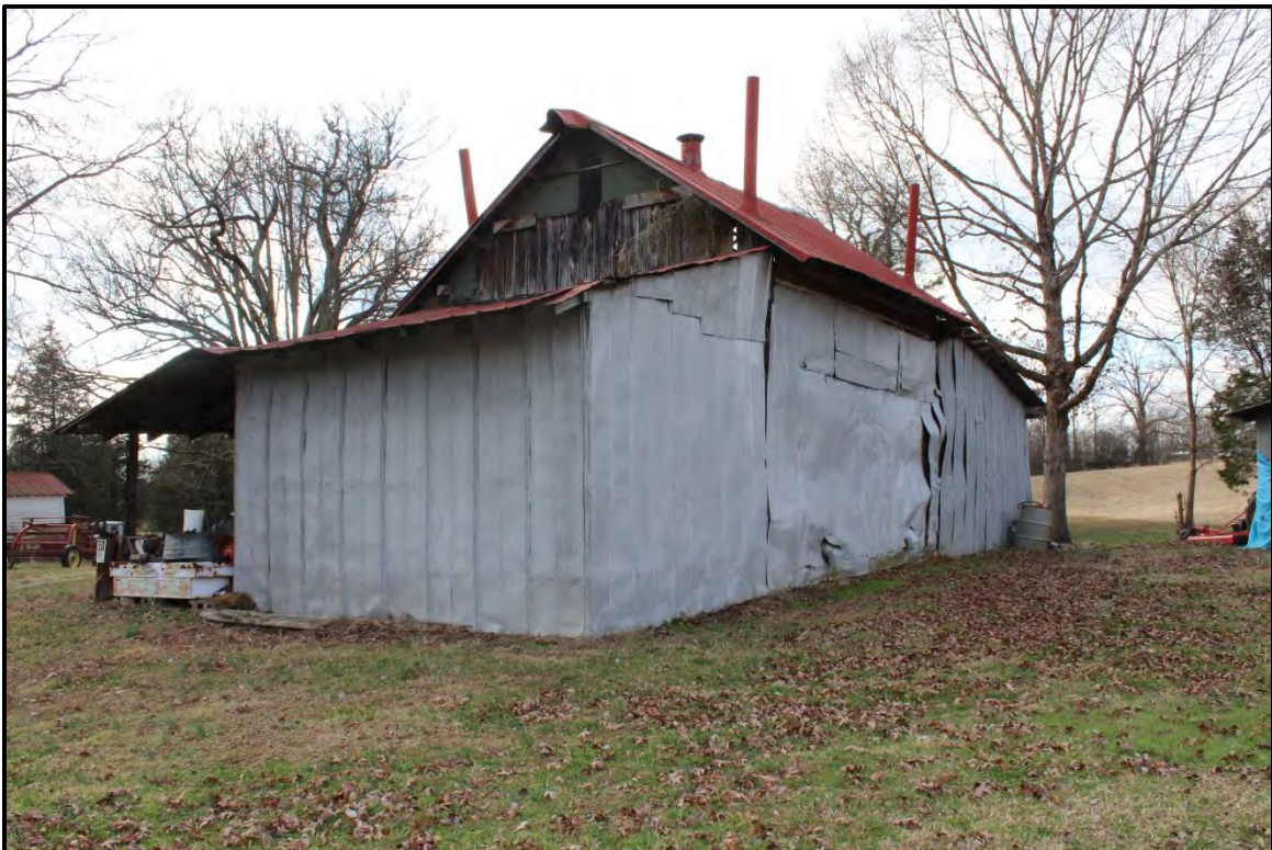
Figure 4.93. Architectural resource AM2631; view is southwest featuring the north (rear) and east elevations of the mid-twentieth century tobacco barn.
