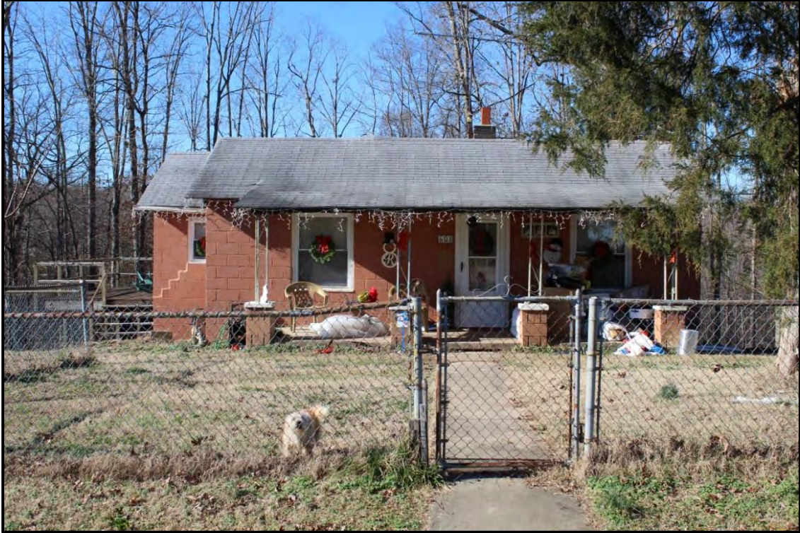
Figure 2.6. Architectural resource RK1784; view is west featuring the façade.
