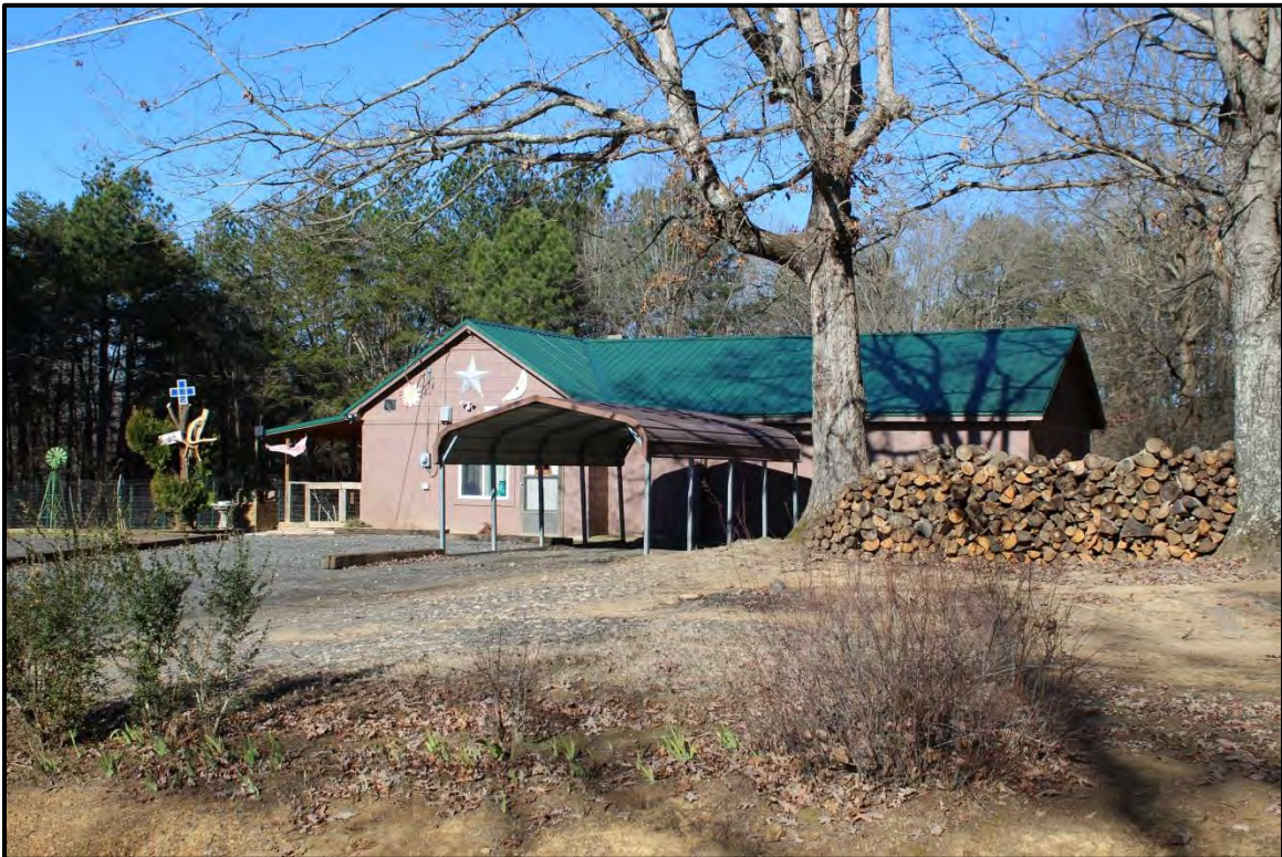
Figure 2.21. Architectural resource RK1788; view is northwest featuring the south elevation and rear addition to the house. Located in the foreground is the metal carport.
