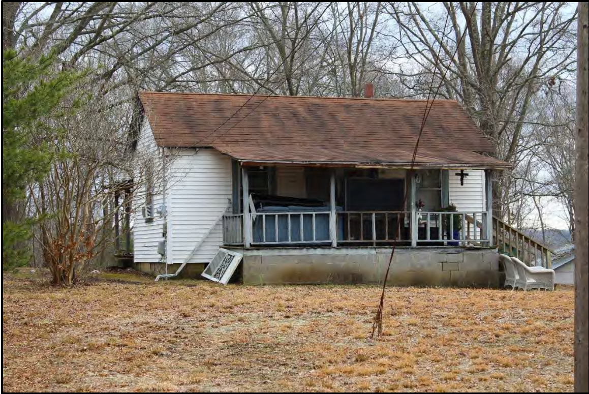
Figure 2.11. Architectural resource RK1821; view is southeast and features the façade and the northeast elevation.
