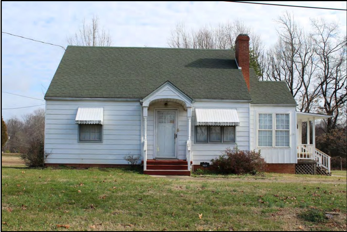
Figure 2.144. Architectural resource RK1813; view is east and features the façade.
