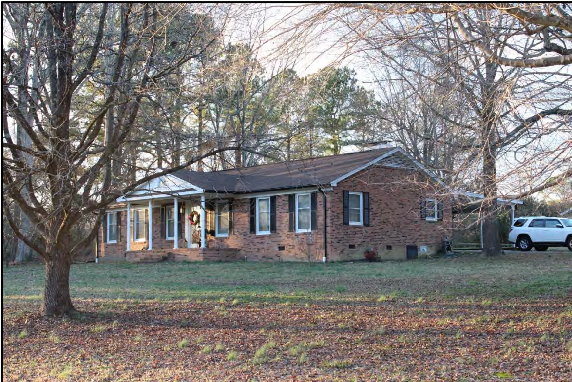
Figure 3.19. Architectural resource GF9113; view is northwest featuring the façade and east elevation.
