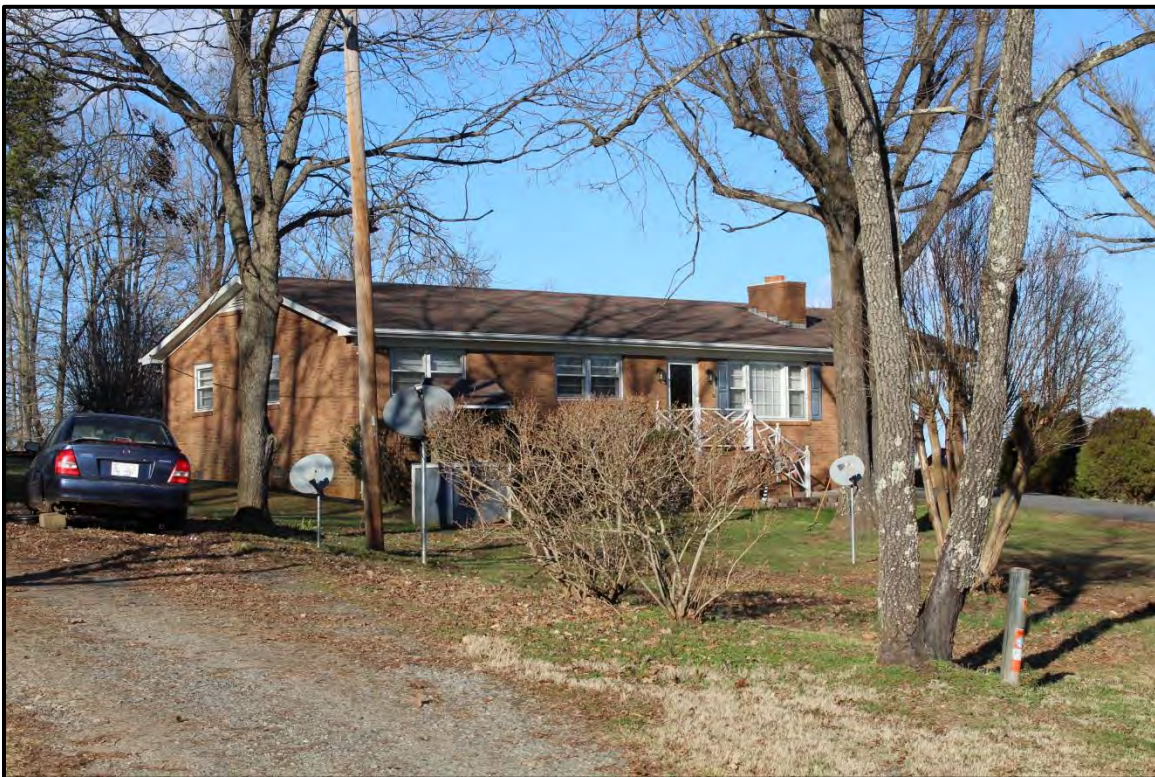
Figure 2.66. Architectural resource RK1797; view is northeast featuring the façade and west elevation.
