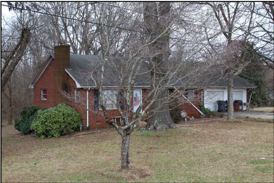
Figure 2.159. Architectural resource RK1817; view is southeast and features the façade and north elevation.
