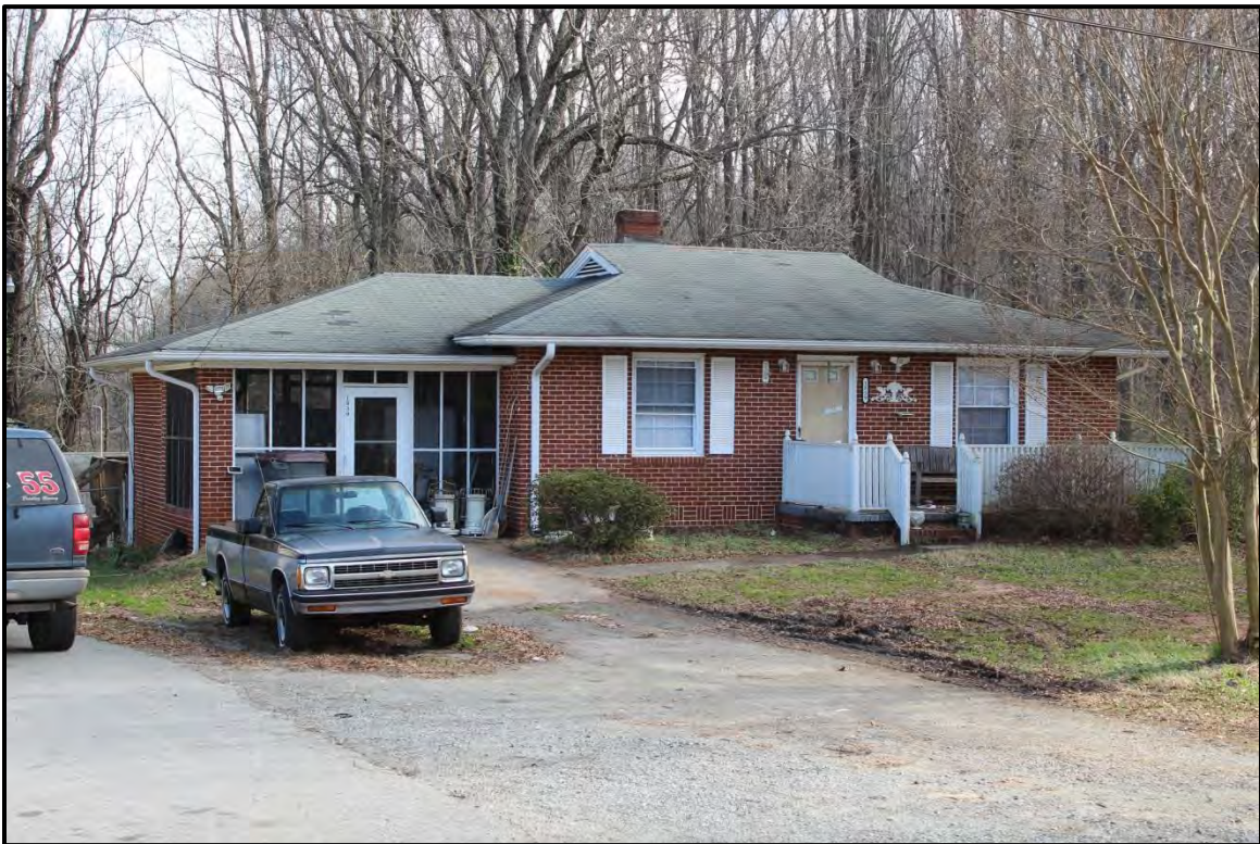
Figure 2.135. Architectural resource RK1810; view is southeast and features the façade and north elevation.
