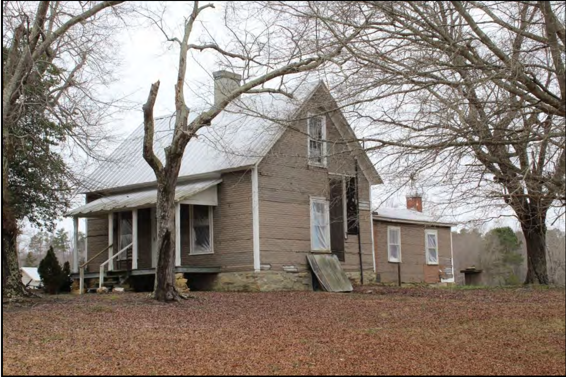
Figure 4.127. Architectural resource AM0362; view is northwest featuring the façade, east elevation, and rear ell.
