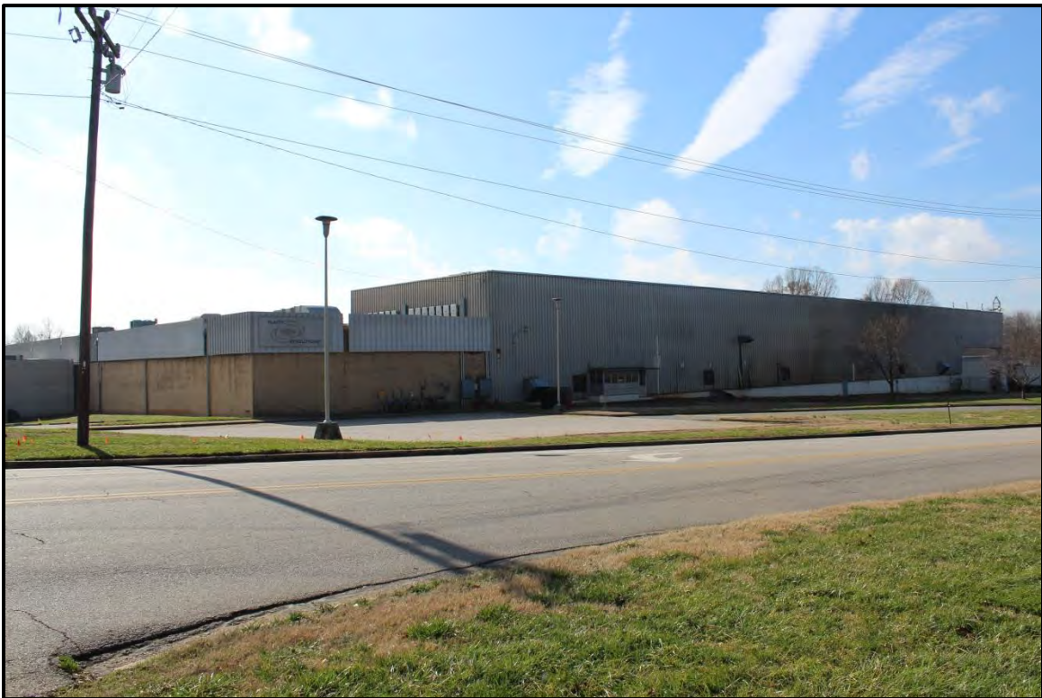
Figure 2.111. Architectural resource RK1803; view is southwest and features the north elevation of the manufacturing building.
