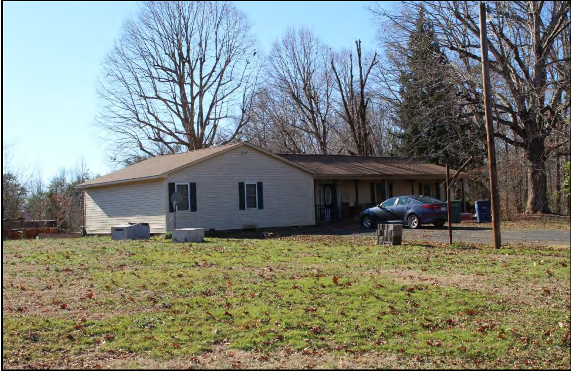
Figure 2.22. Architectural resource RK1789; view is southwest featuring the façade and the modern addition attached to the west elevation.
