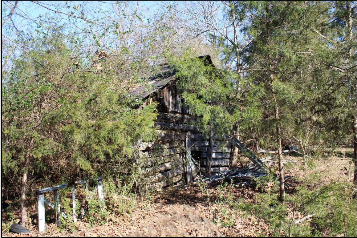
Figure 4.116. Architectural resource AM2635; view is southwest featuring the log storage crib.
