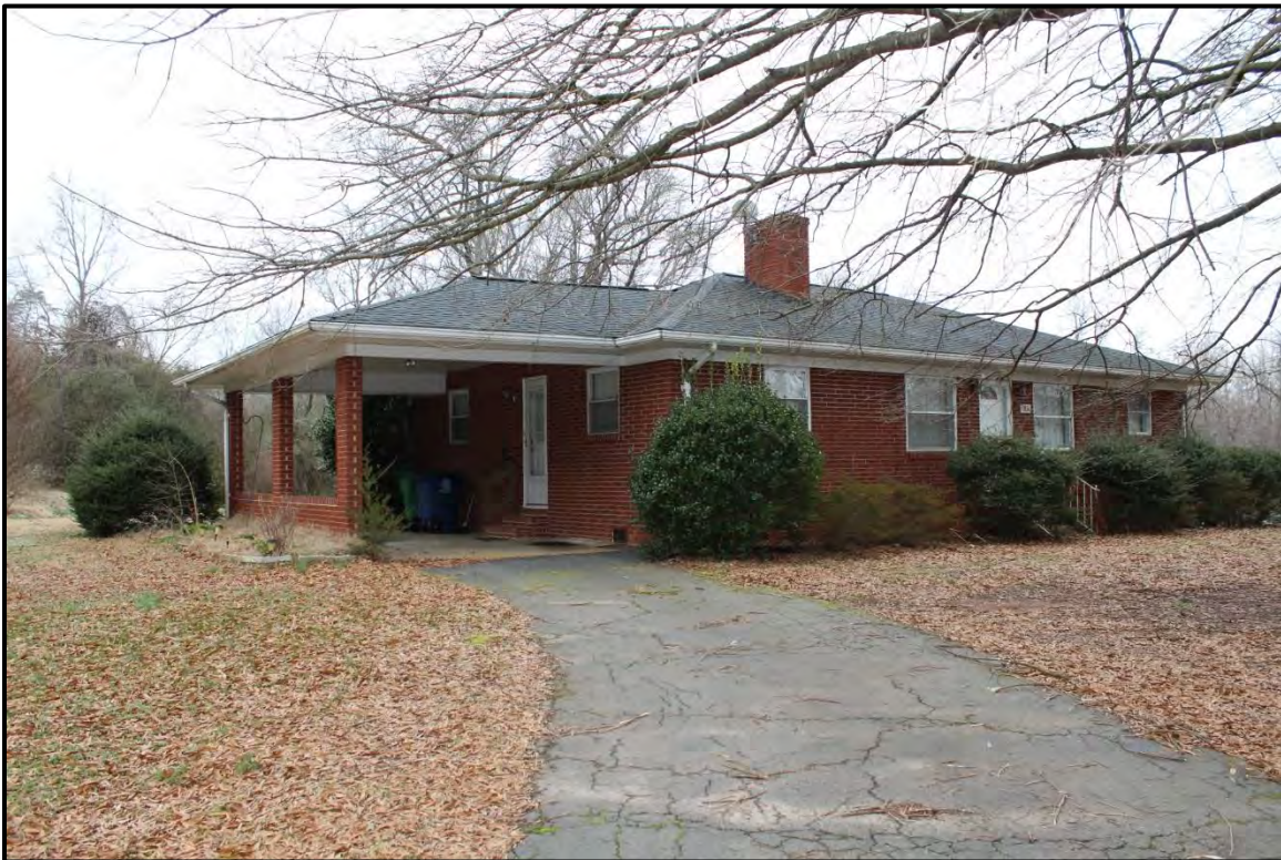
Figure 2.74. Architectural resource RK1818 farmhouse; view is northeast featuring the façade and west elevation.
