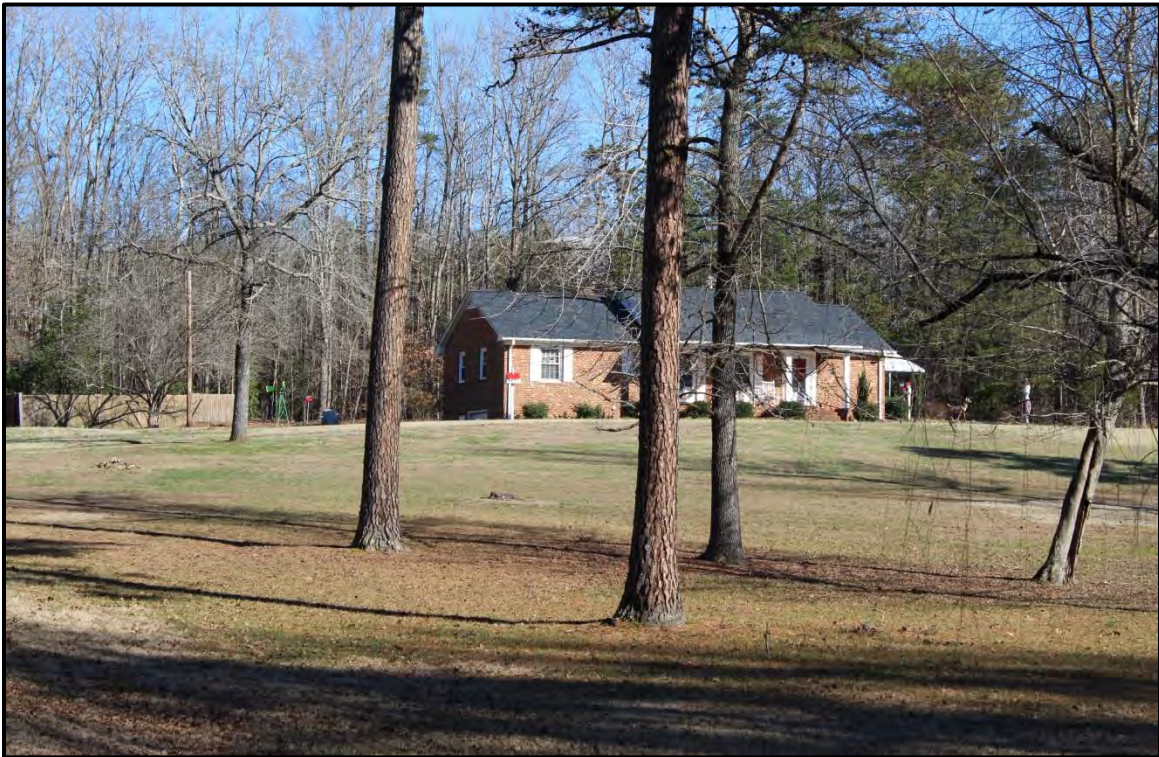
Figure 4.24. Architectural resource AM2624; view is northeast featuring the façade and west elevation.
