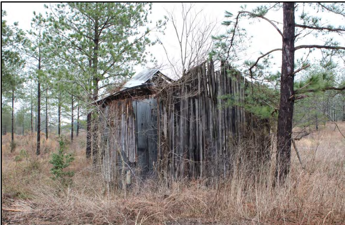
Figure 2.4. Architectural resource RK1086; view is southeast featuring the north (primary) and west elevations.
