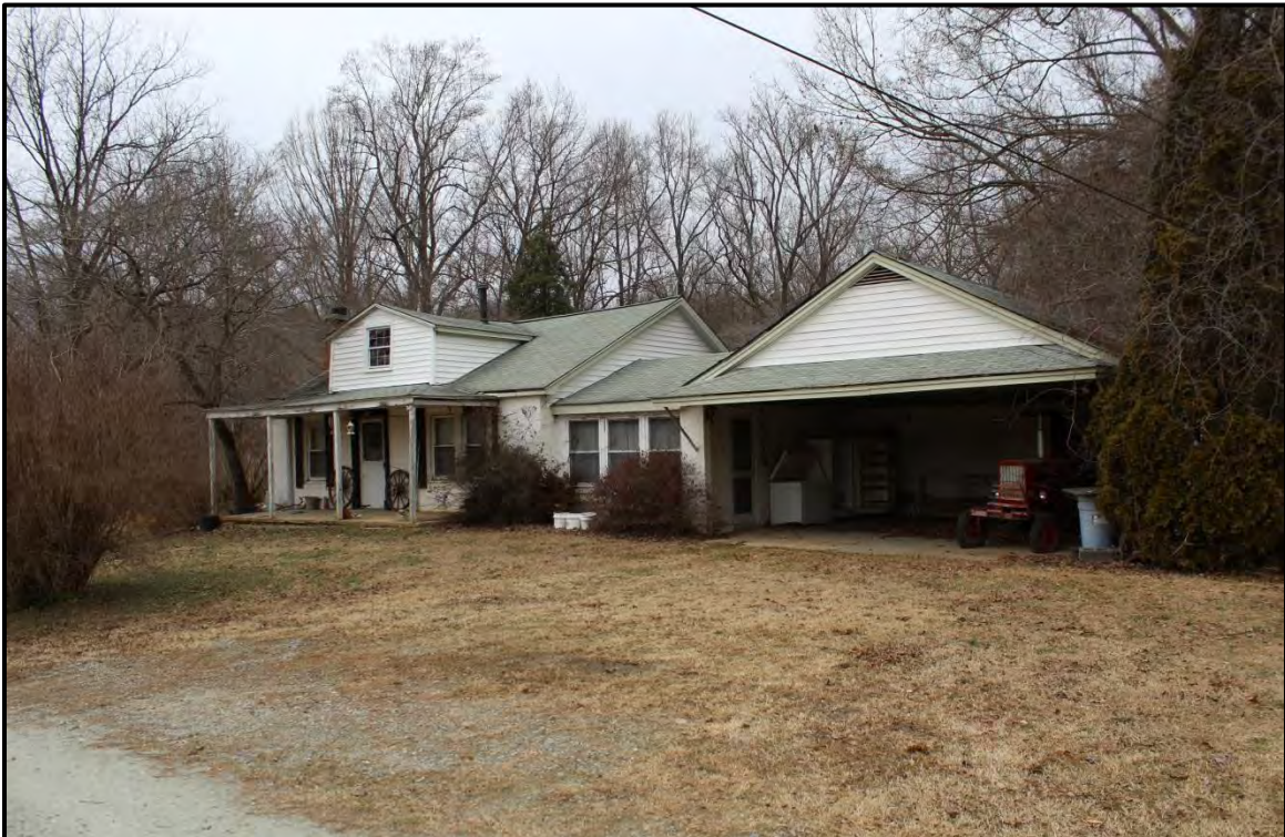
Figure 4.139. Architectural resource AM2645; view is northwest featuring the façade and east elevation garage wing.
