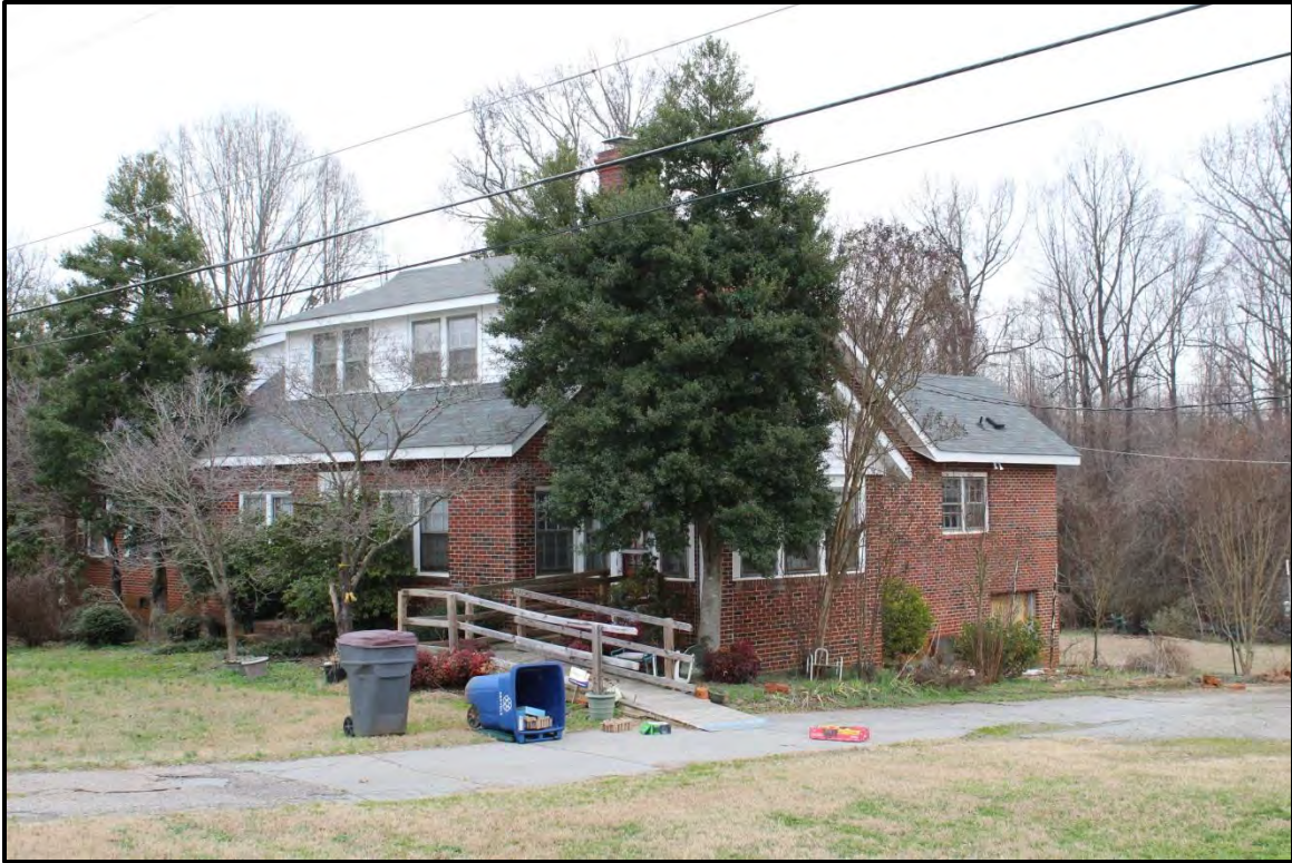
Figure 2.156. Architectural resource RK1816; view is northeast and features the façade and south elevation.
