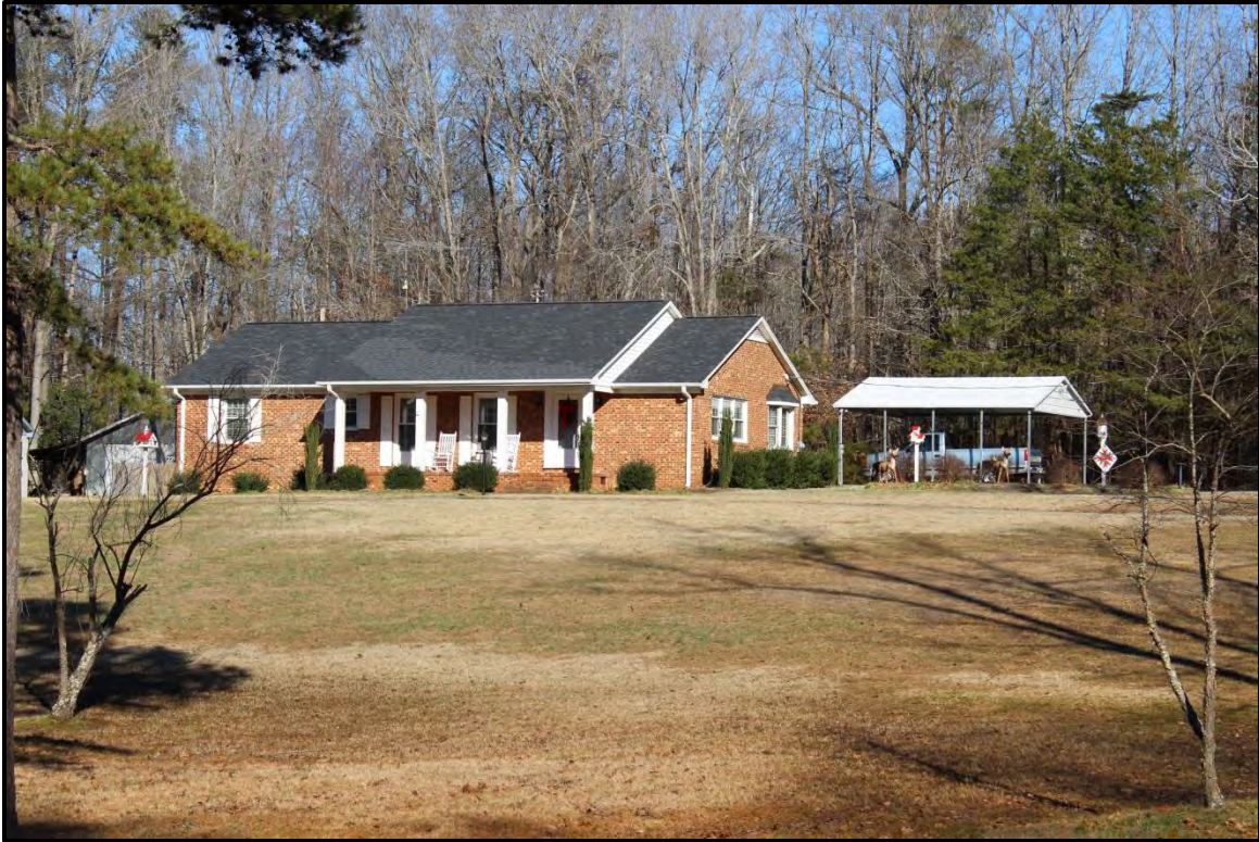
Figure 4.23. Architectural resource AM2624; view is northwest featuring the façade and east elevation of the primary residence with the modern carport to the right.
