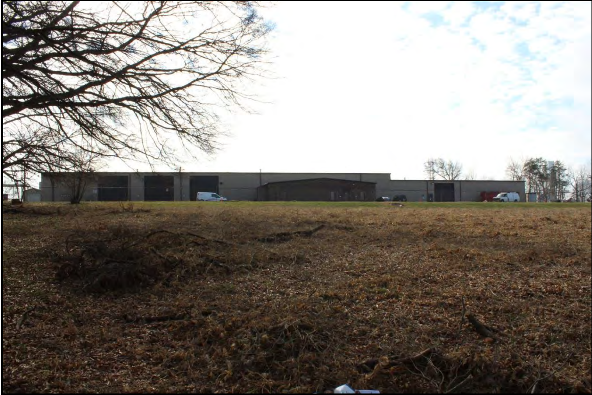
Figure 2.117. Architectural resource RK1804; view is south and features the north elevation of the warehouse building.
