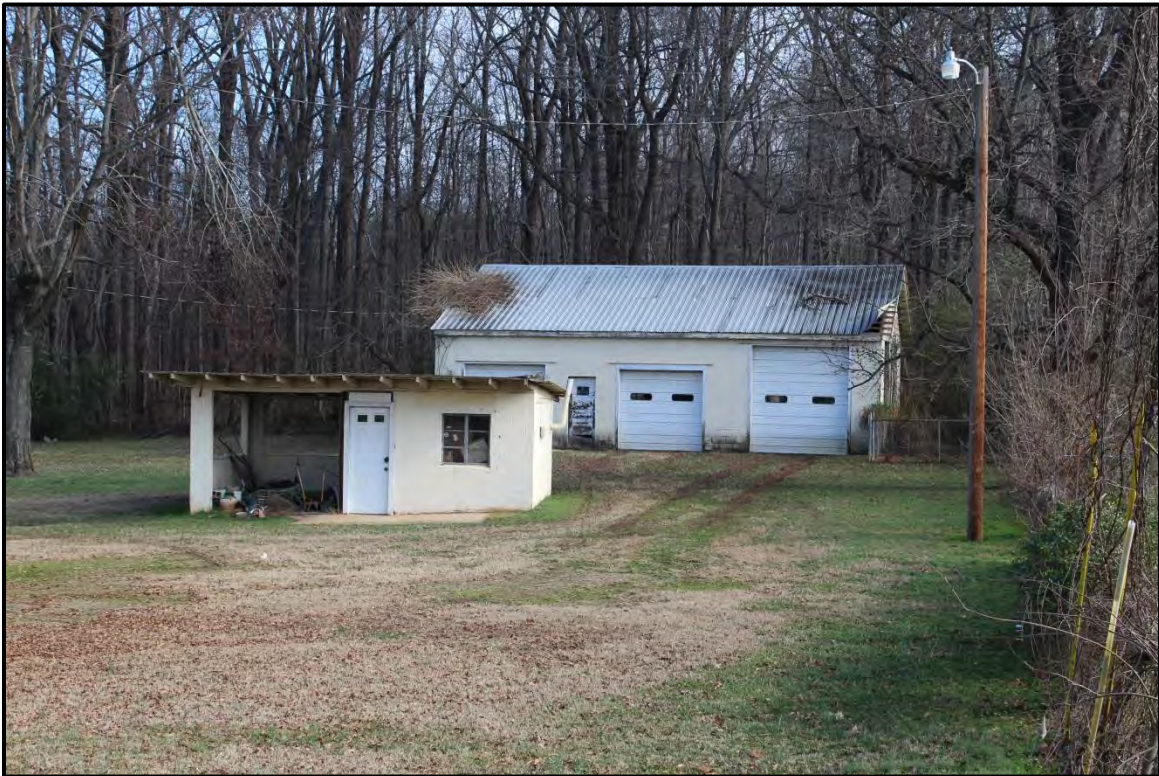
Figure 2.130. Architectural resource RK1808; view is east featuring the storage building and garage.
