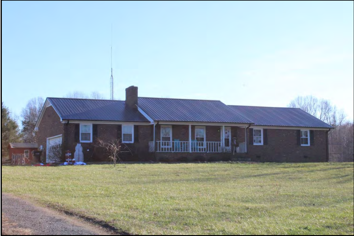
Figure 4.37. Architectural resource AM2627; view is southwest featuring the façade and east elevation garage. The modern shed is located in the background.
