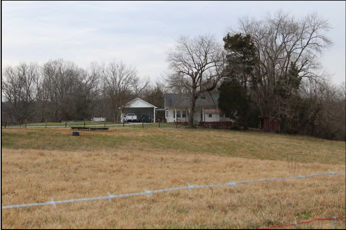
Figure 4.166. Architectural resource AM2650; view is west featuring the façade of the primary residence and the associated carport.
