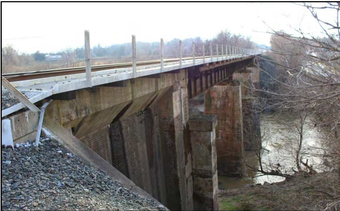
Figure 4.153. Architectural resource AM1324; view is northeast featuring the south elevation of the bridge with the attached walkway.
