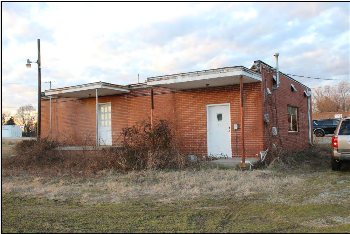
Figure 3.23. Architectural resource GF9115; view is northwest featuring the south (rear) and east elevations.
