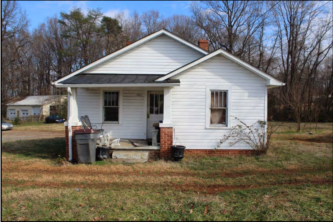
Figure 2.121. Architectural resource RK1806; view is east and features the façade.
