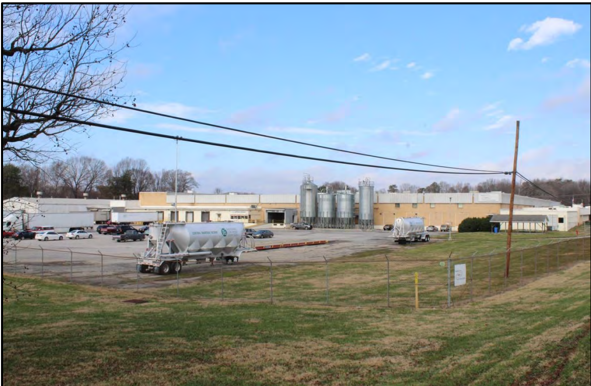
Figure 2.113. Architectural resource RK1803; view is northwest and features the south elevation of the manufacturing building, multiple docking bays, the storage silos, and the picnic shelter.
