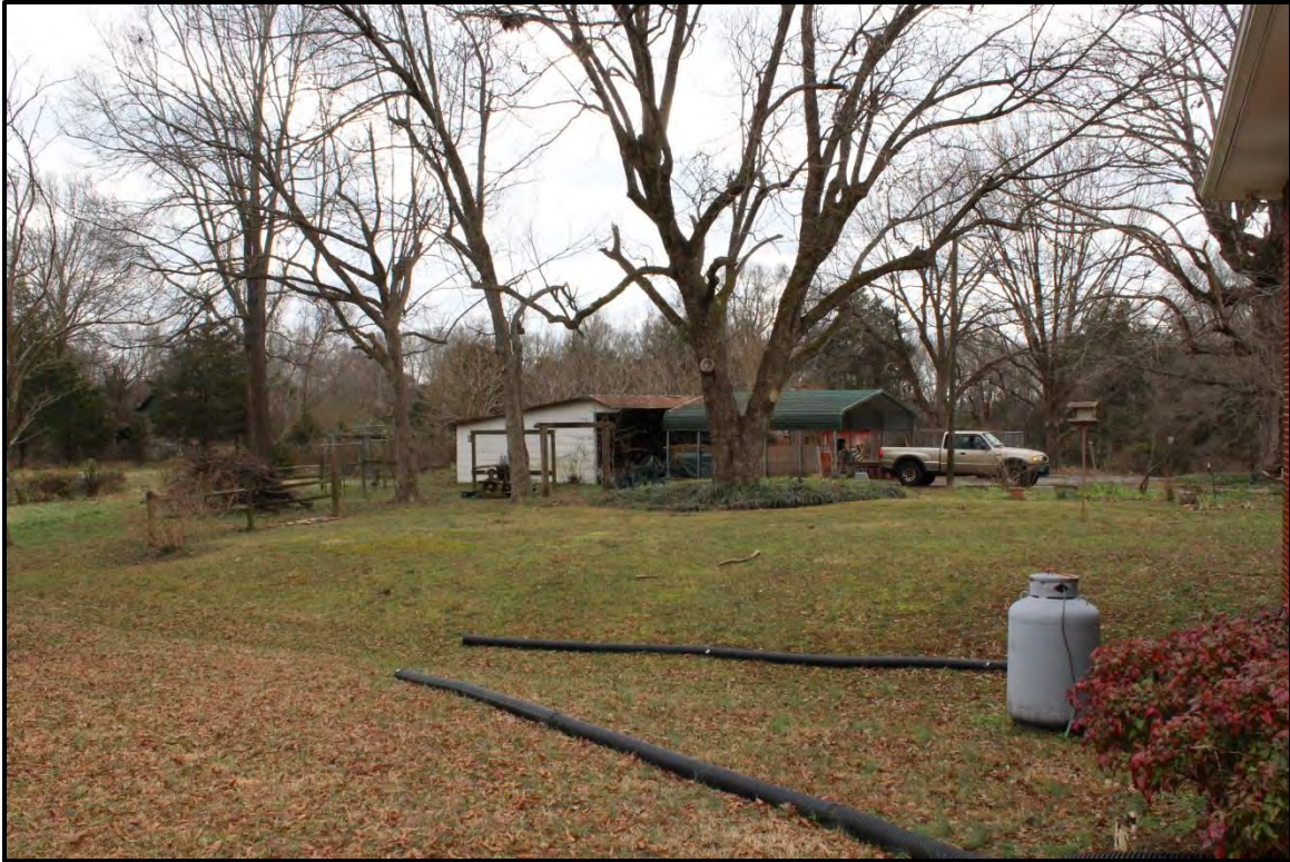
Figure 4.100. Architectural resource AM2652; view is south featuring the equipment shed and modern carport.
