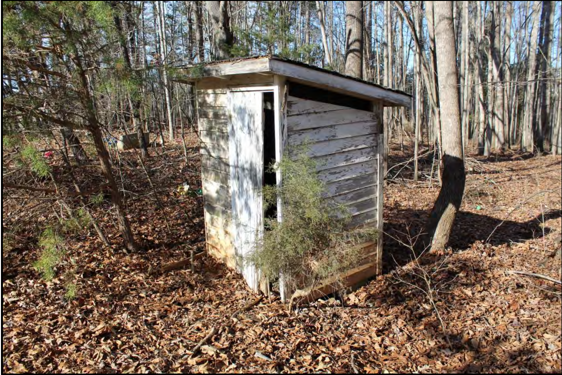
Figure 4.64. Architectural resource AM1603; view is northwest featuring the “North Privy.”
