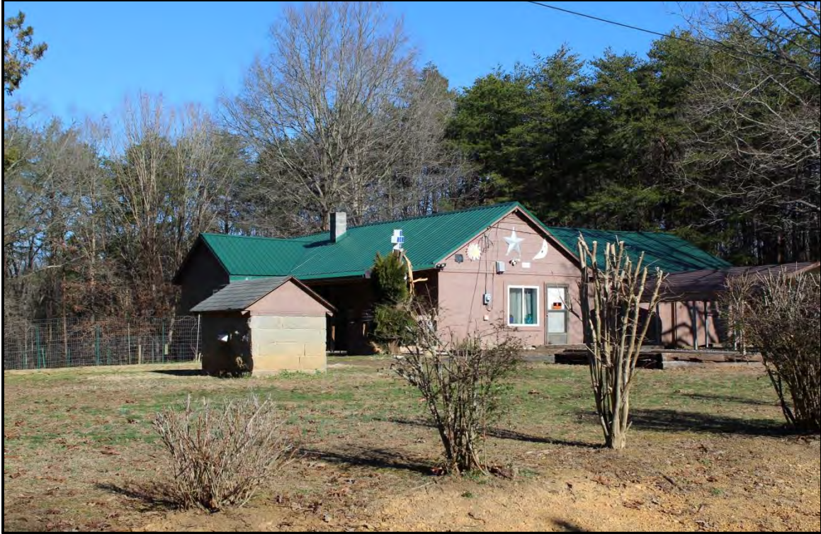
Figure 2.20. Architectural resource RK1788; view is northeast featuring the façade and the south elevation of the house with the pump shed in the foreground.
