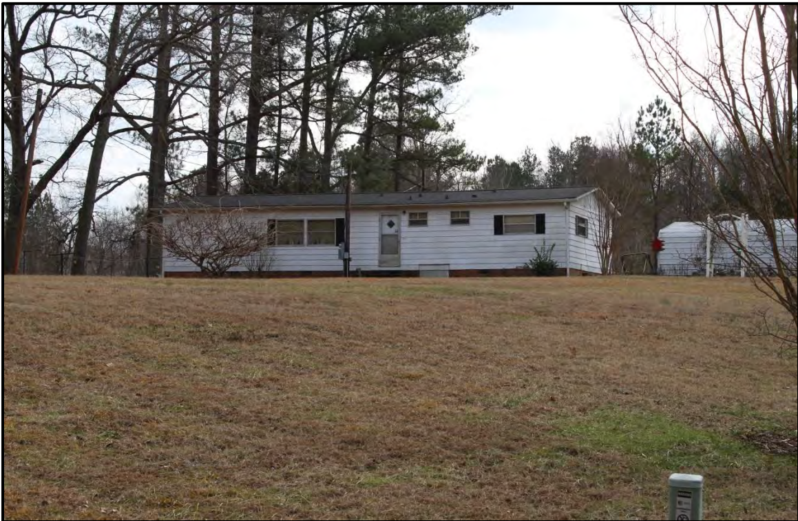
Figure 4.59. Architectural resource AM2629; view is southeast featuring the façade and west elevation of the ca. 1968 residence with the modern carport in the background.
