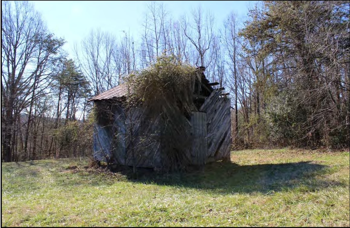
Figure 2.18. Architectural resource RK1787; view is south featuring the mid-twentieth century agricultural storage building.
