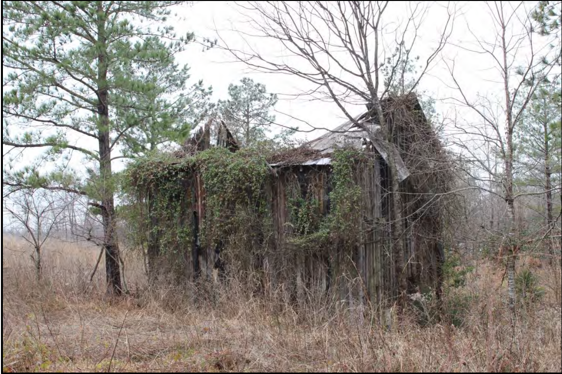
Figure 2.5. Architectural resource RK1086; view is northwest featuring the south (rear) and east elevations.
