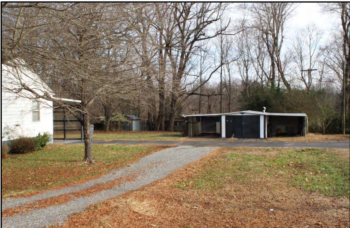
Figure 2.143. Architectural resource RK1812; view is east featuring the 1980 carport and storage building.
