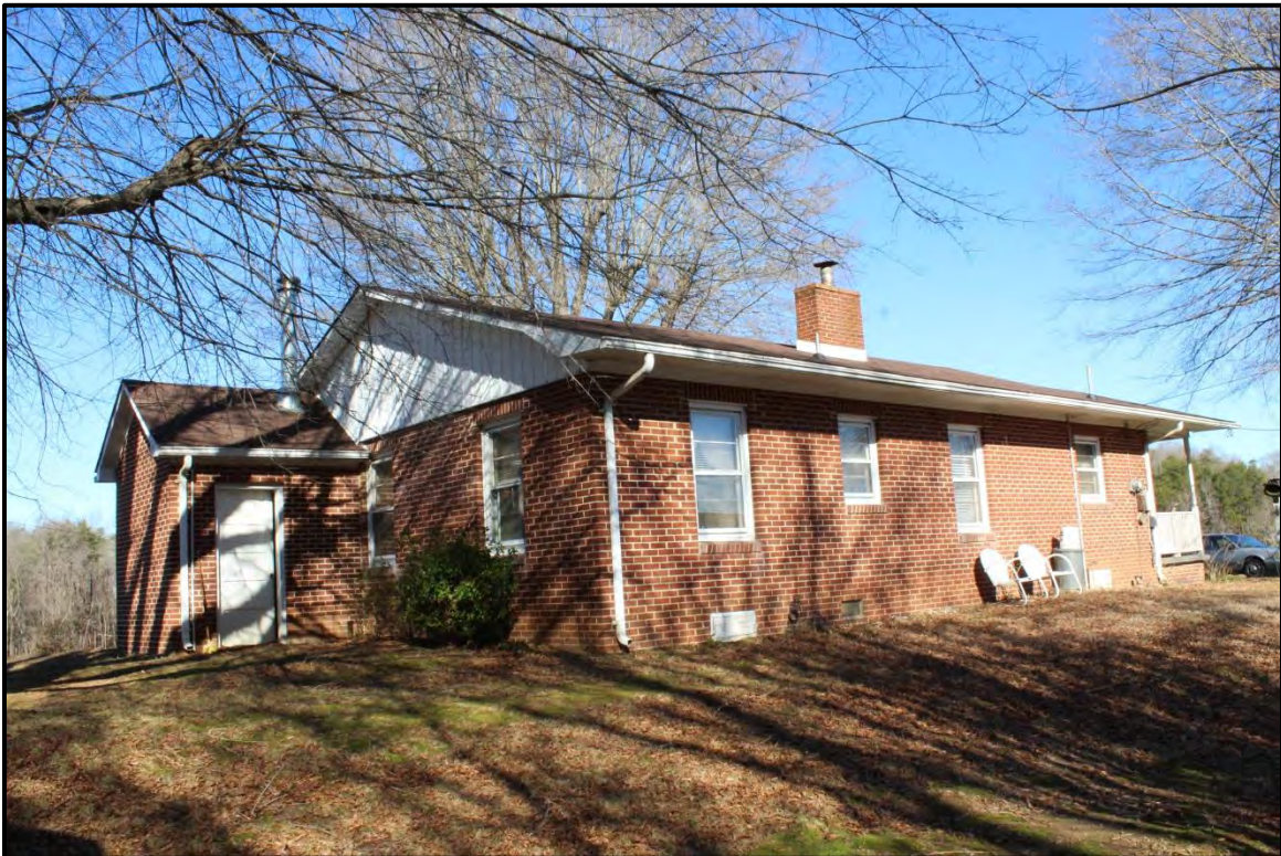
Figure 2.15. Architectural resource RK1787; view is northeast featuring the façade and west elevation.
