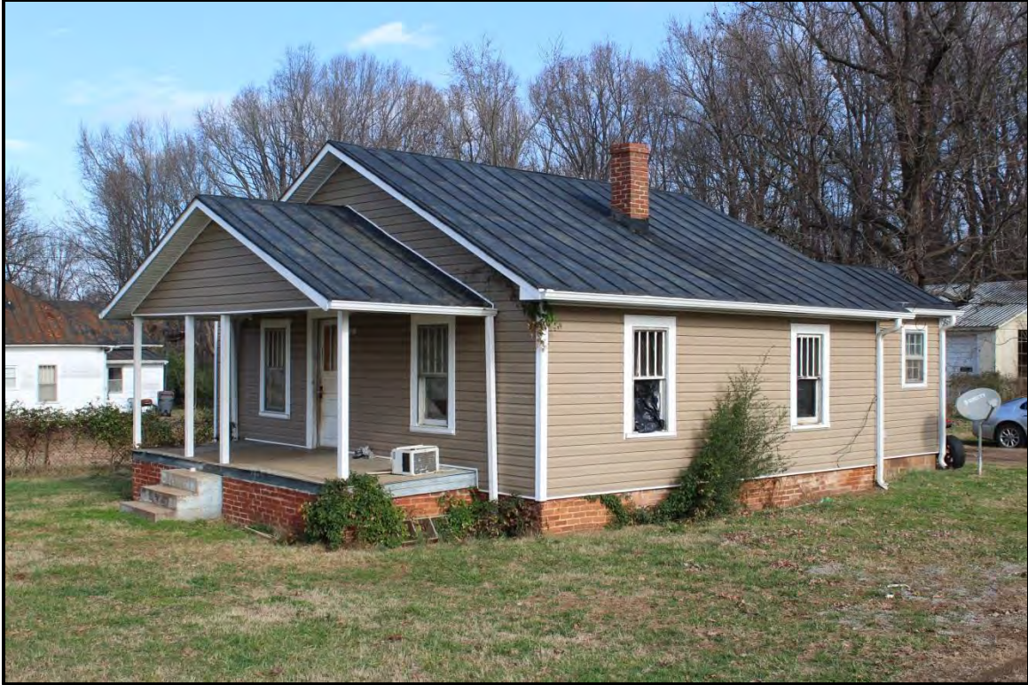
Figure 2.120. Architectural resource RK1805; view is northeast and features the façade and south elevation.
