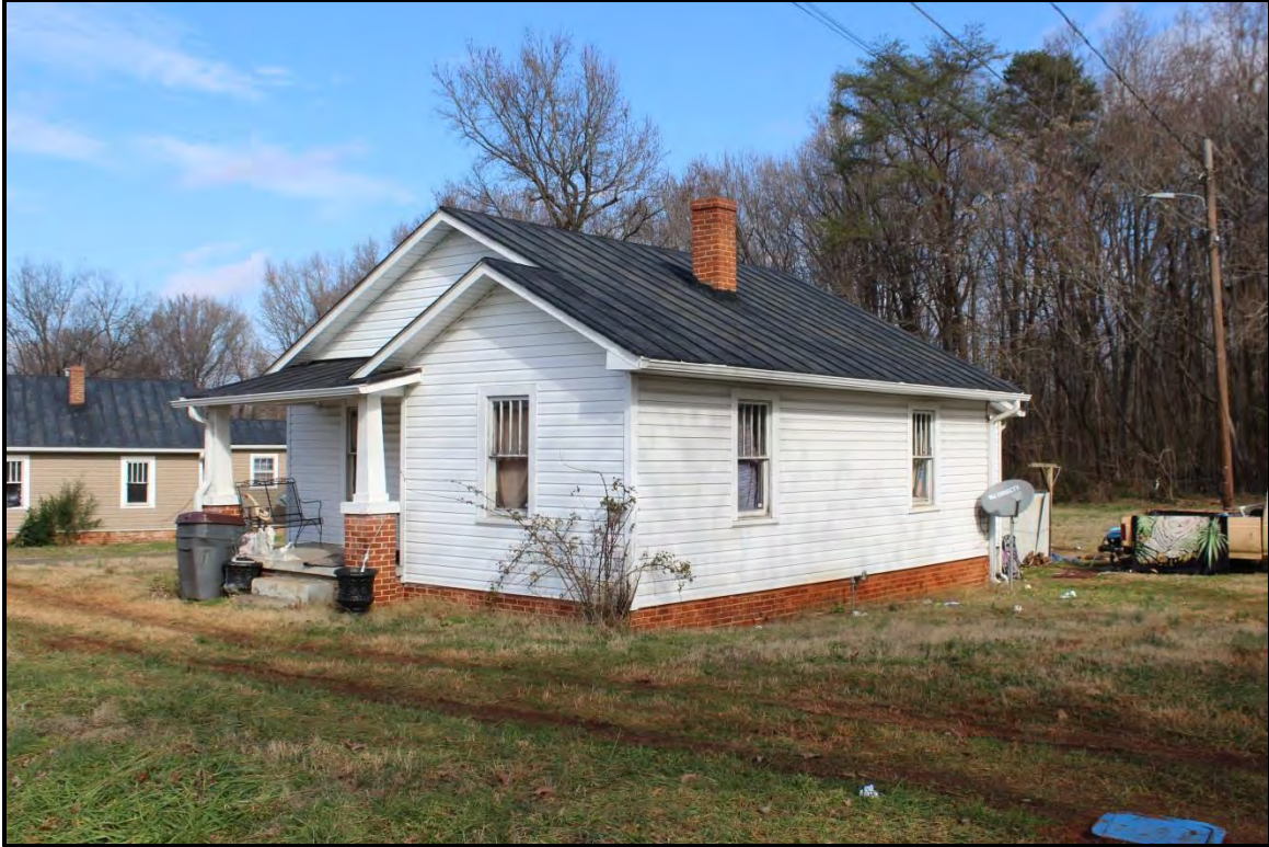
Figure 2.123. Architectural resource RK1806; view is southeast and features the façade and north elevation.
