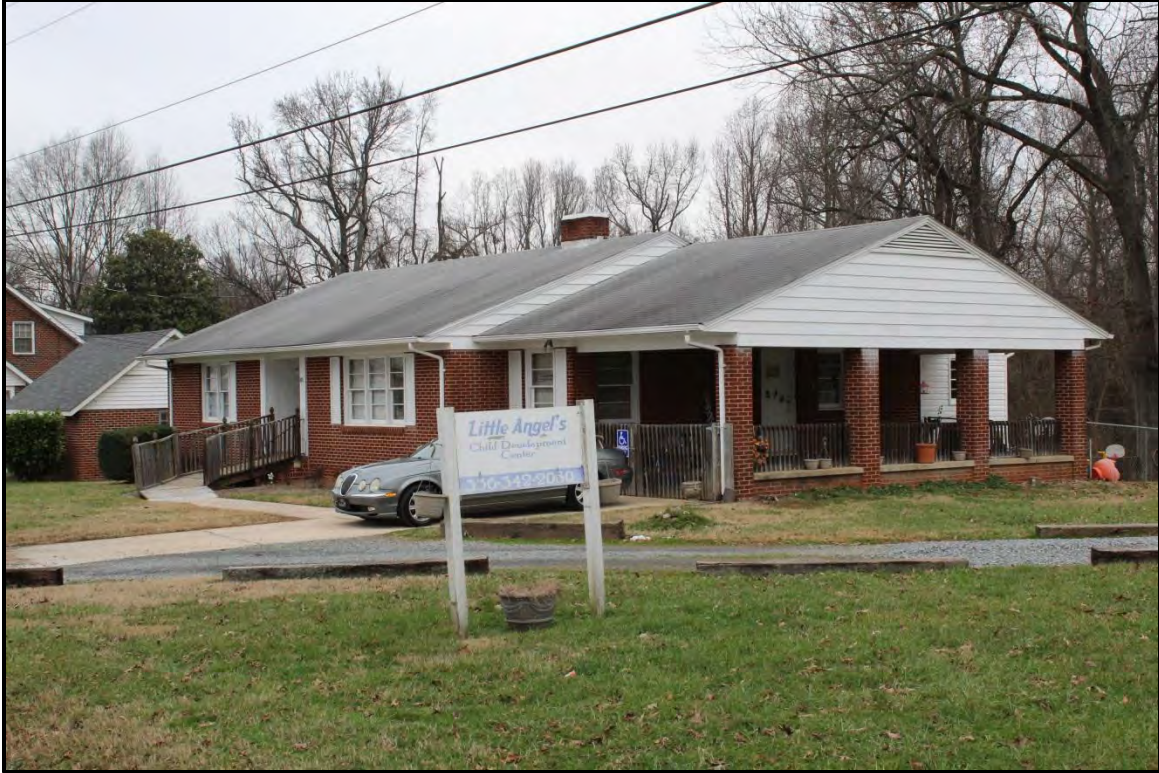
Figure 2.153. Architectural resource RK1815; view is northeast and features the façade and south elevation.
