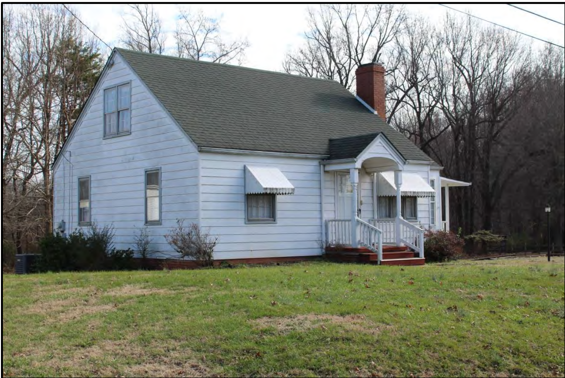
Figure 2.145. Architectural resource RK1813; view is southeast and features the façade and north elevation.
