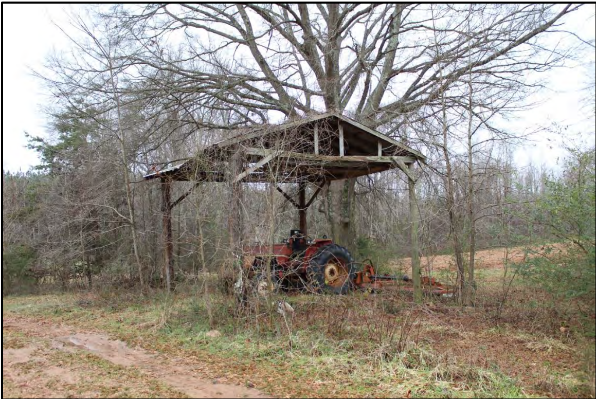
Figure 2.80. Architectural resource RK1818; view is north featuring the ca. 1970 pole shed.
