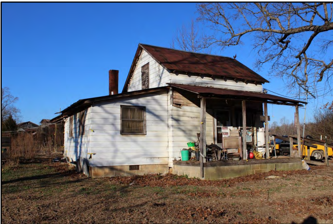
Figure 2.32. Architectural resource RK1792 farmhouse; view is northwest featuring the façade and south elevation.
