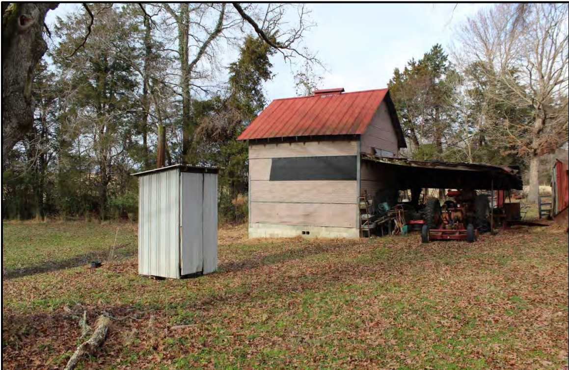
Figure 4.87. Architectural resource AM2631; view is northwest featuring the modern privy and the south and east elevations of the mid- to late twentieth century tobacco barn.
