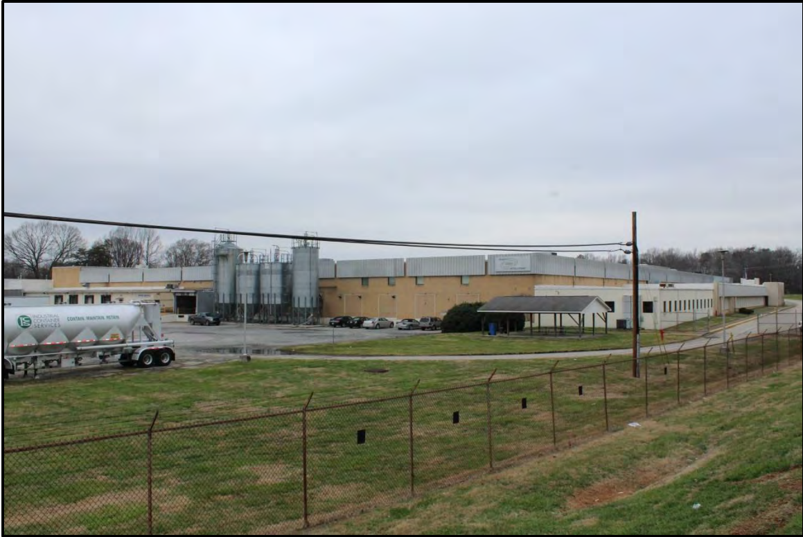
Figure 2.112. Architectural resource RK1803; view is northwest and features the south elevation of the manufacturing building, the storage silos, and the picnic shelter.
