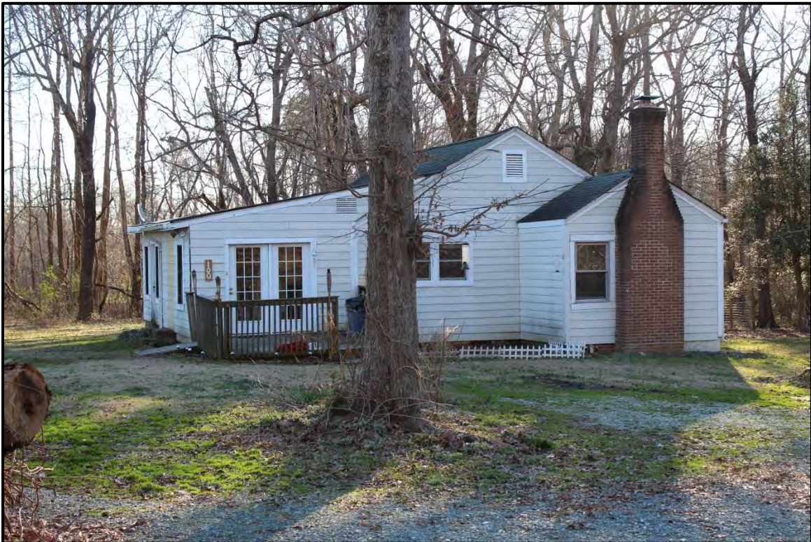
Figure 3.29. Architectural resource GF9117; view is southeast featuring the west and north (rear) elevations.
