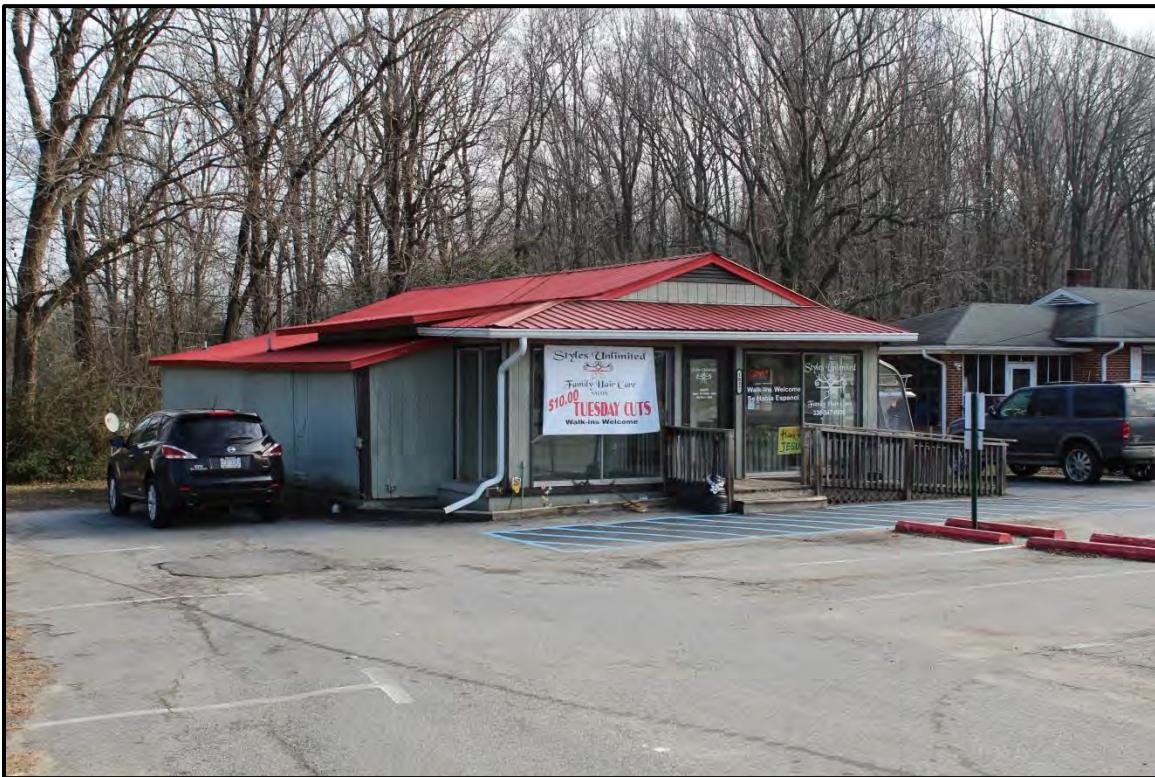
Figure 2.138. Architectural resource RK1811; view is southeast and features the façade and north elevation.
