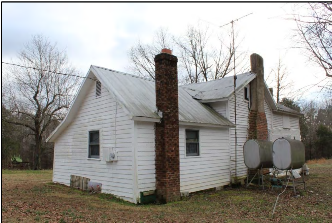
Figure 4.77. Architectural resource AM2631; view is south featuring the northeast and northwest (rear) elevations of ca. 1940 wood-frame wing addition.
