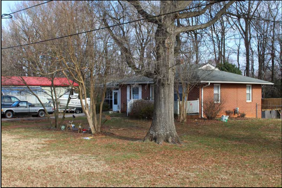
Figure 2.136. Architectural resource RK1810; view is northeast and features the façade and south elevation.
