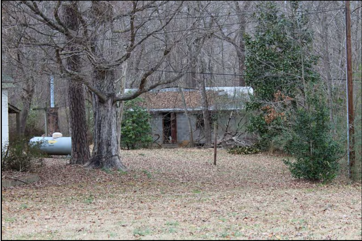
Figure 4.140. Architectural resource AM2645; view is north featuring the concrete block utility building.
