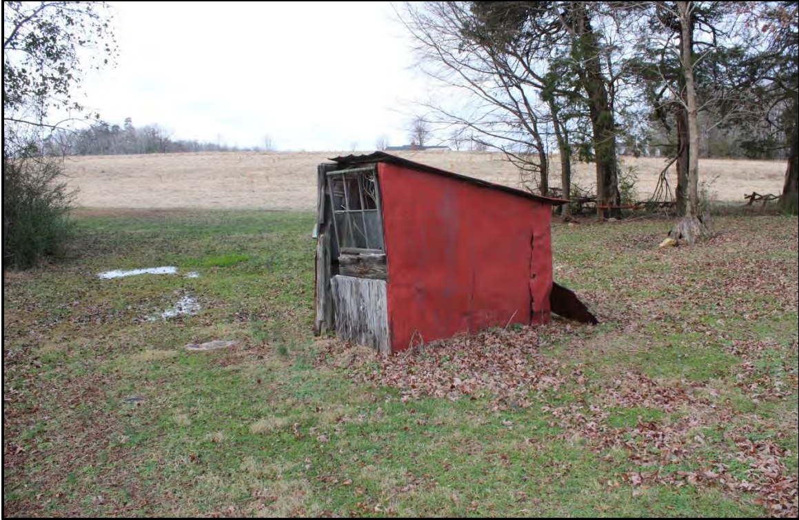
Figure 4.90. Architectural resource AM2631; view is northwest featuring the south and east elevations of the mid-twentieth century chicken house.
