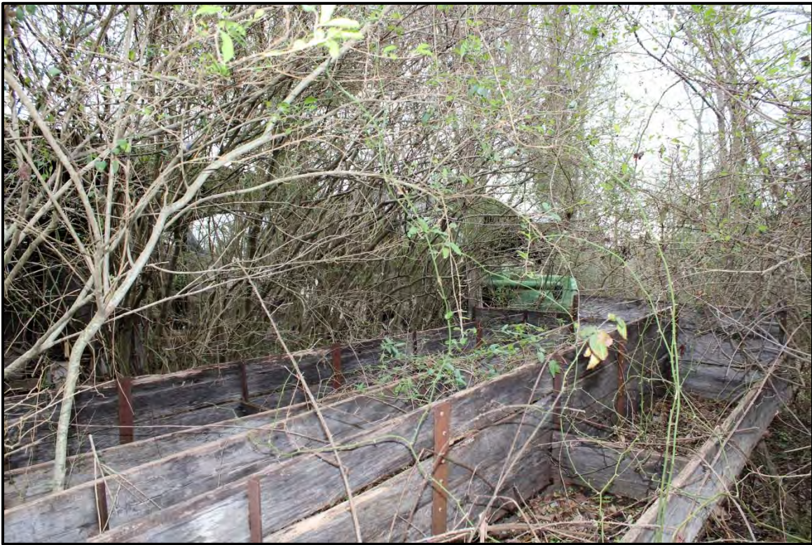
Figure 2.88. Architectural resource RK1818; view is west featuring the storage bins.
