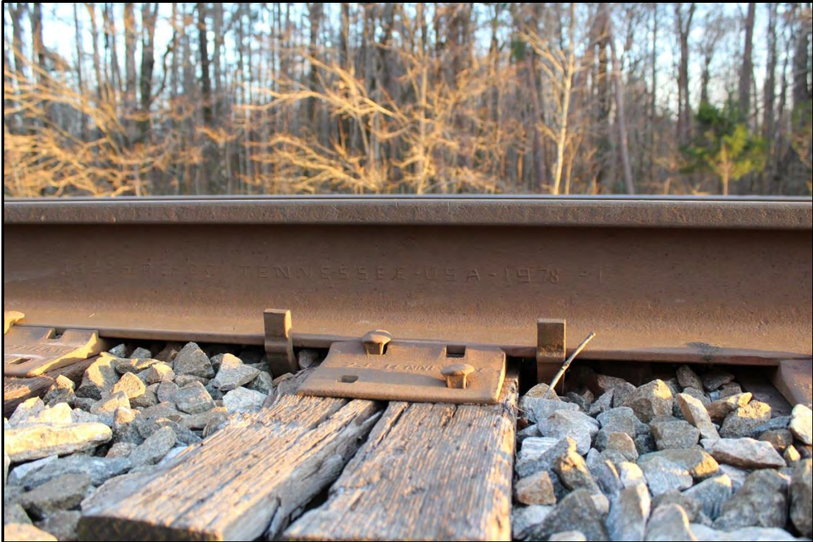
Figure 3.26. Architectural resource GF9116; “north track” featuring the 1978 manufacturing date.
