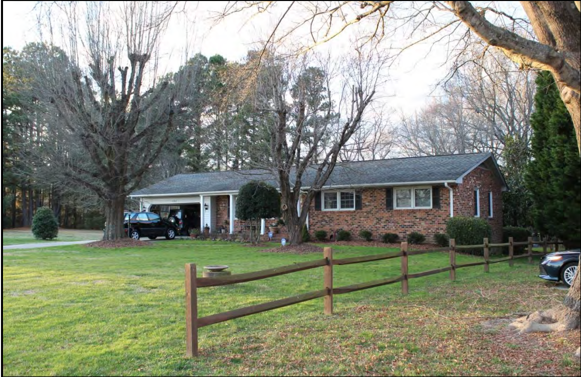
Figure 3.12. Architectural resource GF9110; view is northwest featuring the façade and east elevation.
