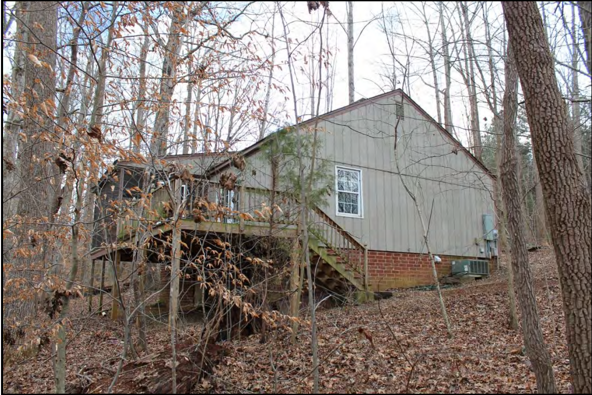
Figure 4.164. Architectural resource AM2649; view is east featuring the northwest (rear) and southwest elevations.
