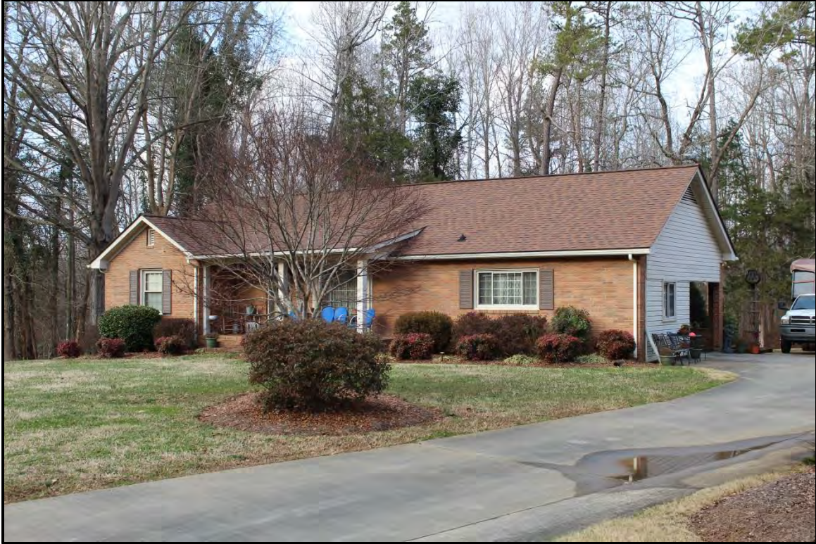
Figure 4.150. Architectural resource AM2651; view is northwest featuring the façade and east elevation.
