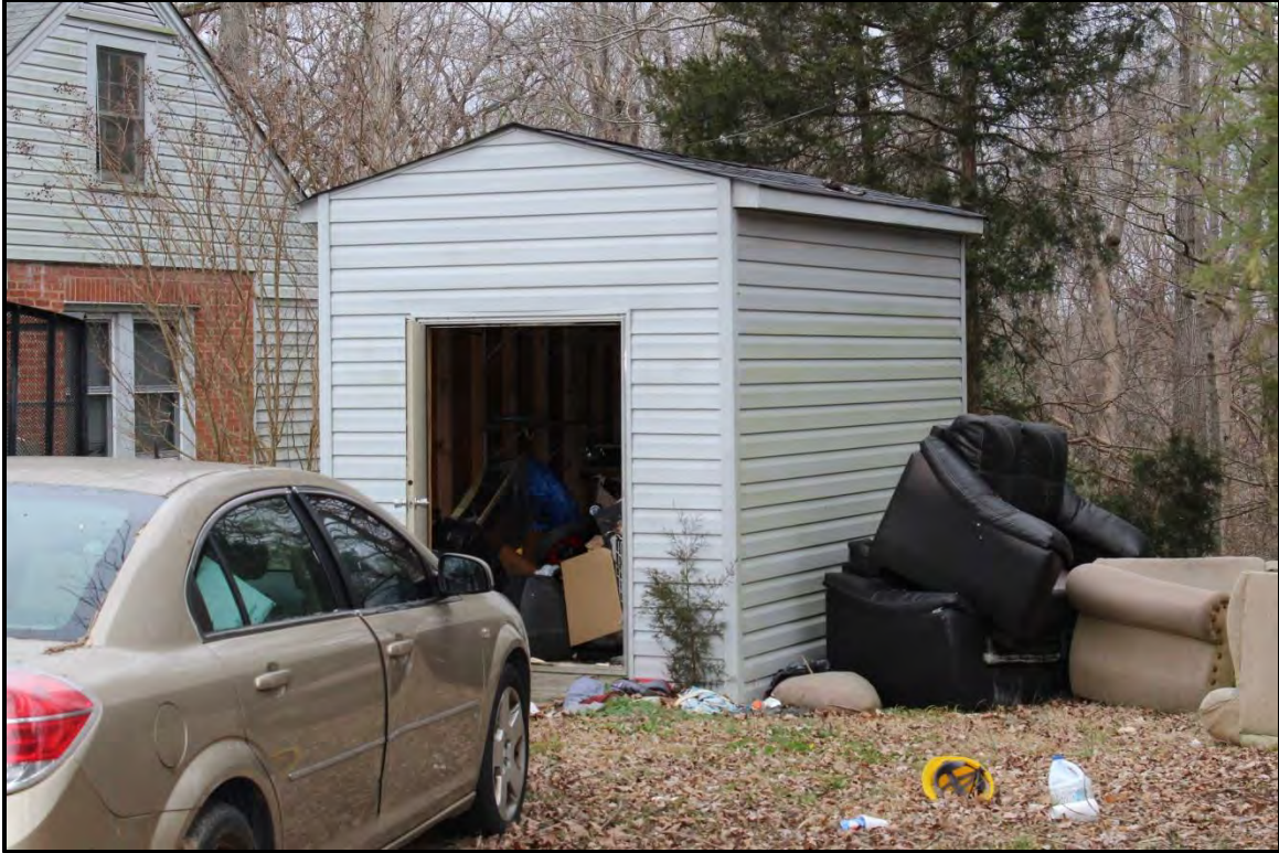
Figure 4.162. Architectural resource AM2648; view is west featuring the modern storage shed.
