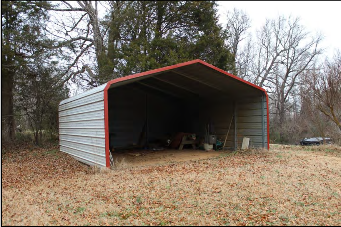
Figure 2.77. Architectural resource RK1818; view is northeast featuring the 2004 carport.
