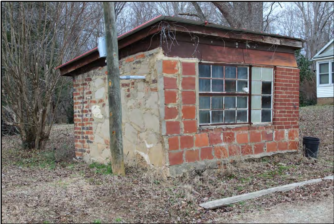
Figure 4.141. Architectural resource AM2645; view is northeast featuring the water pump shed.
