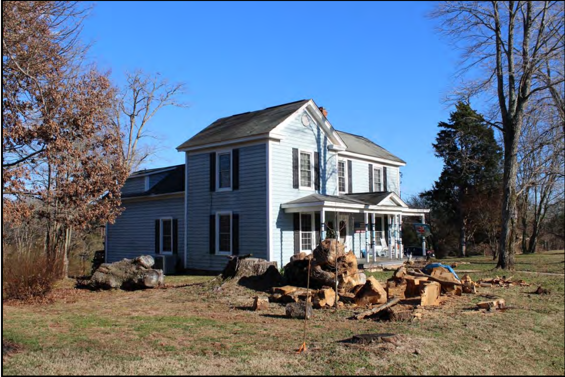
Figure 2.58. Architectural resource RK1796; view is east featuring the façade and west elevation.
