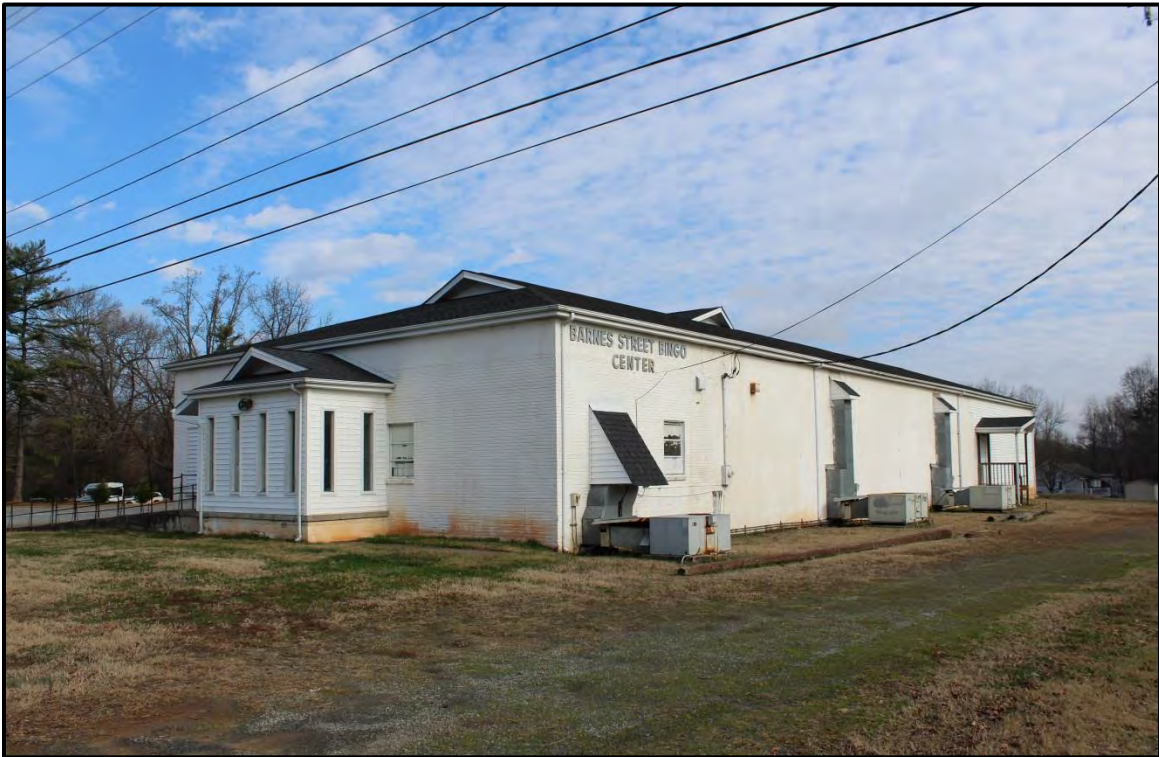
Figure 2.148. Architectural resource RK1814; view is northeast and features the façade and south elevation.
