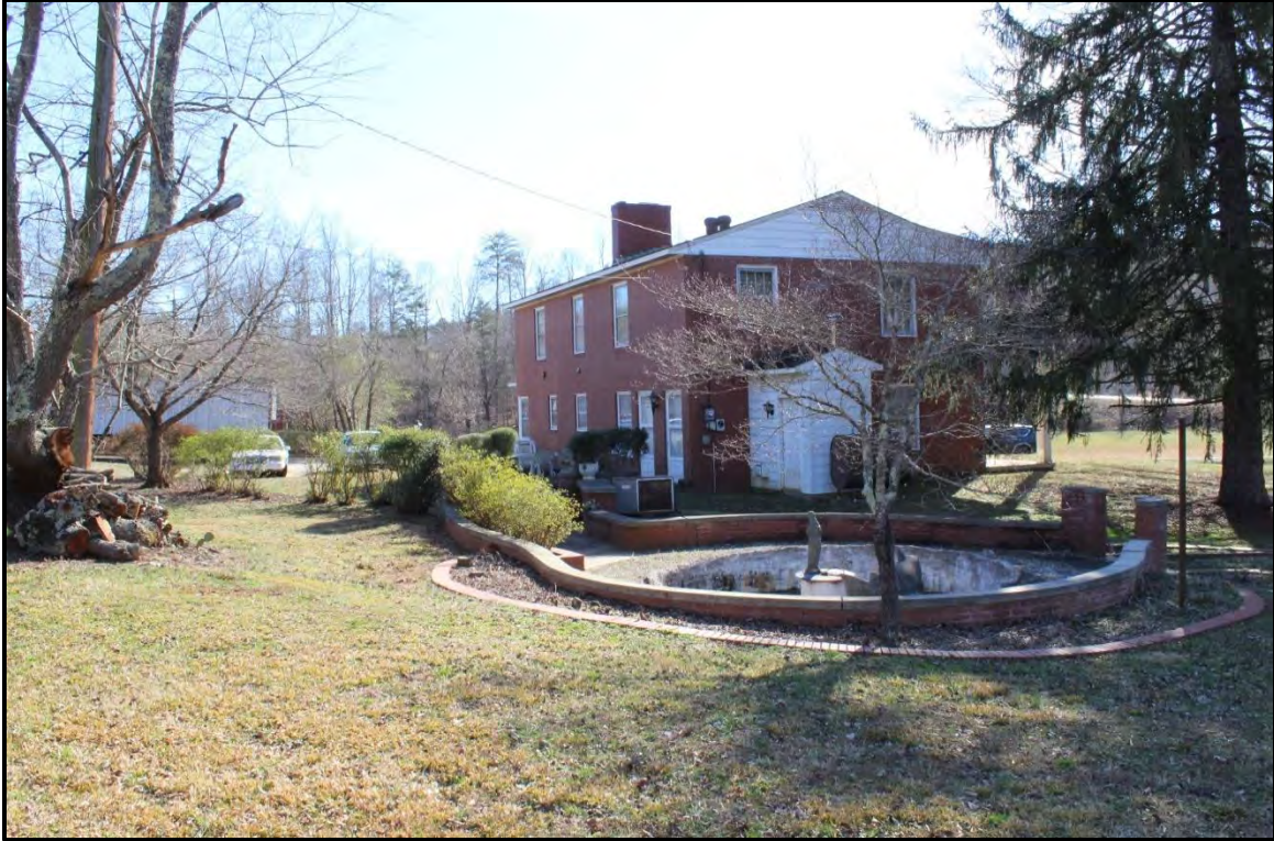
Figure 4.146. Architectural resource AM2644; view is southeast featuring the foundation and associated garden wall.
