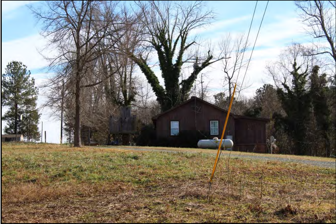
Figure 4.58. Architectural resource AM2629; view is south featuring the north and west (rear) elevations of the ca. 1952 house.
