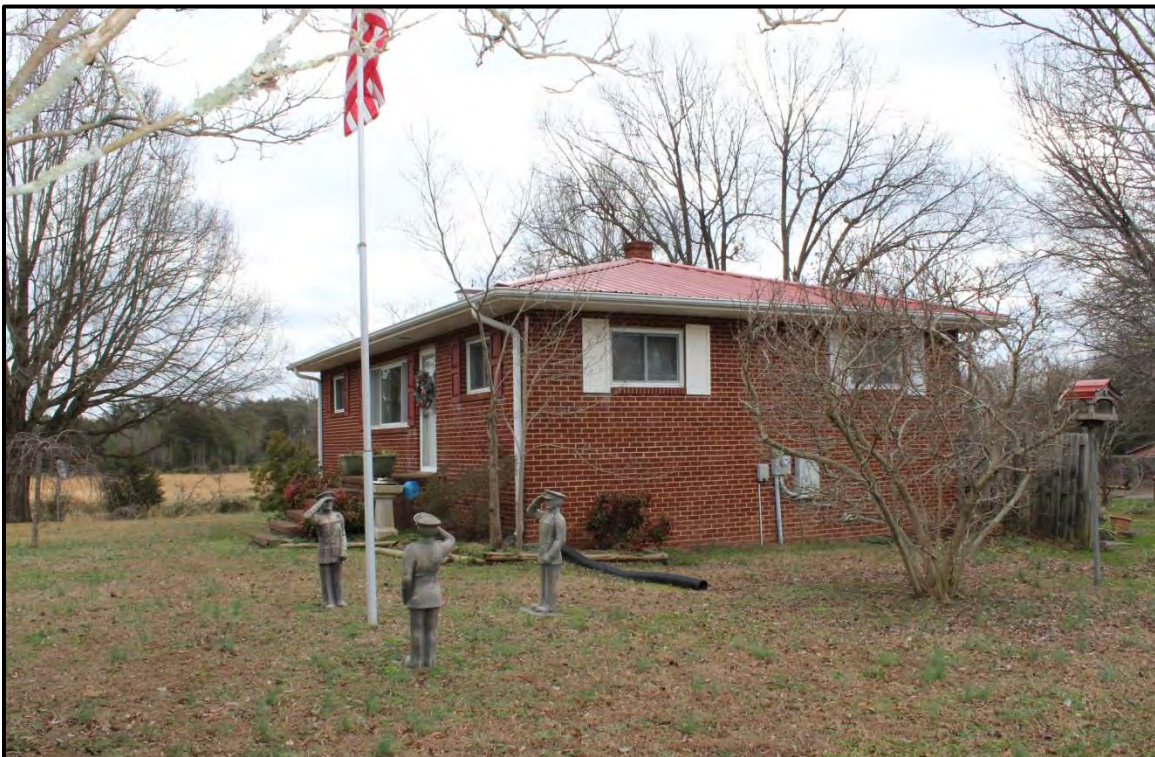
Figure 4.99. Architectural resource AM2652; view is southeast featuring the façade and west elevation of the farmhouse.
