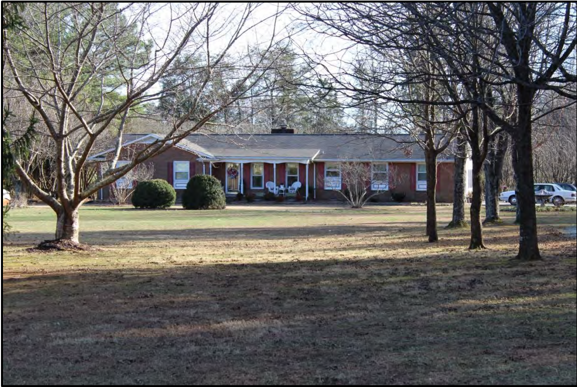
Figure 4.1. Architectural resource AM2617; view is south featuring the façade.
