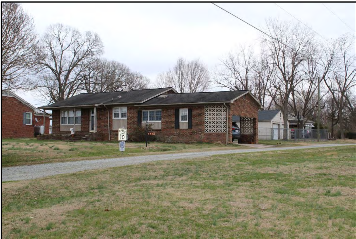
Figure 4.51. Architectural resource AM2640; view is southeast featuring the façade and west elevation.
