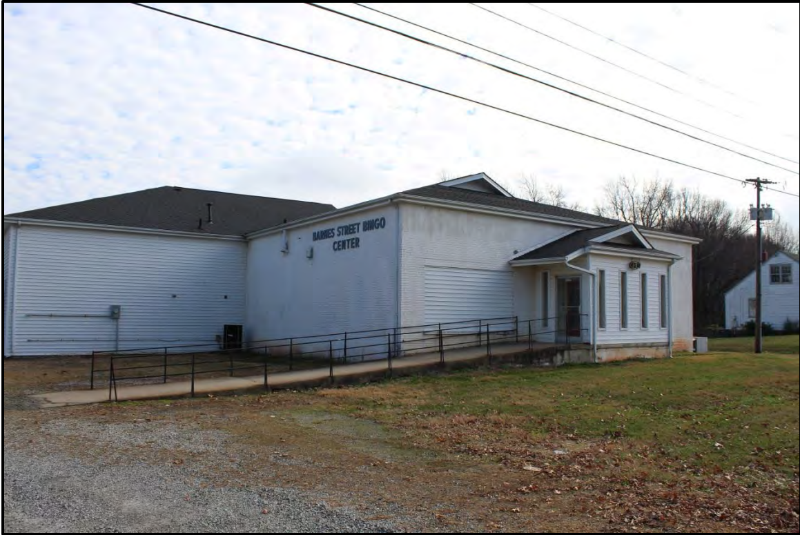
Figure 2.147. Architectural resource RK1814; view is southeast and features the façade and north elevation.
