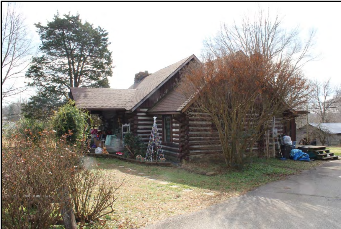
Figure 2.60. Architectural resource RK1820; view is southeast and features the façade and north elevation.
