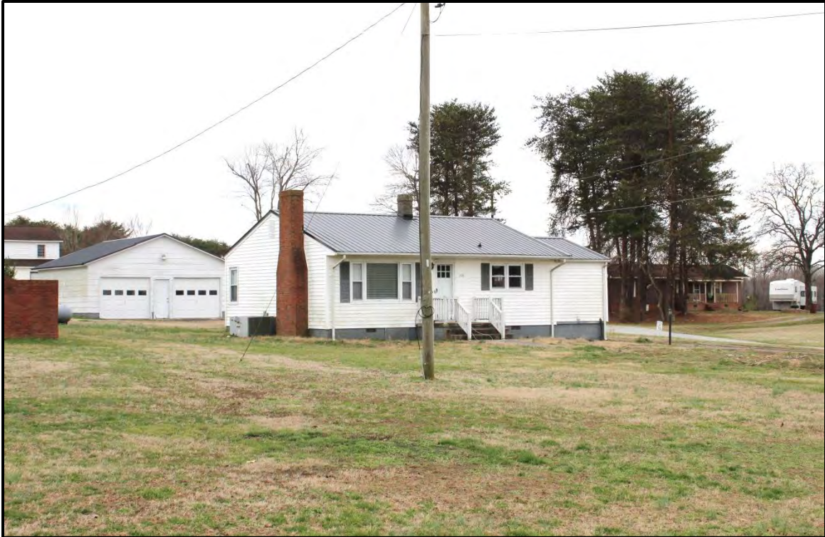
Figure 4.54. Architectural resource AM2642; view is southwest featuring the façade and east elevation of the house and associated garage.
