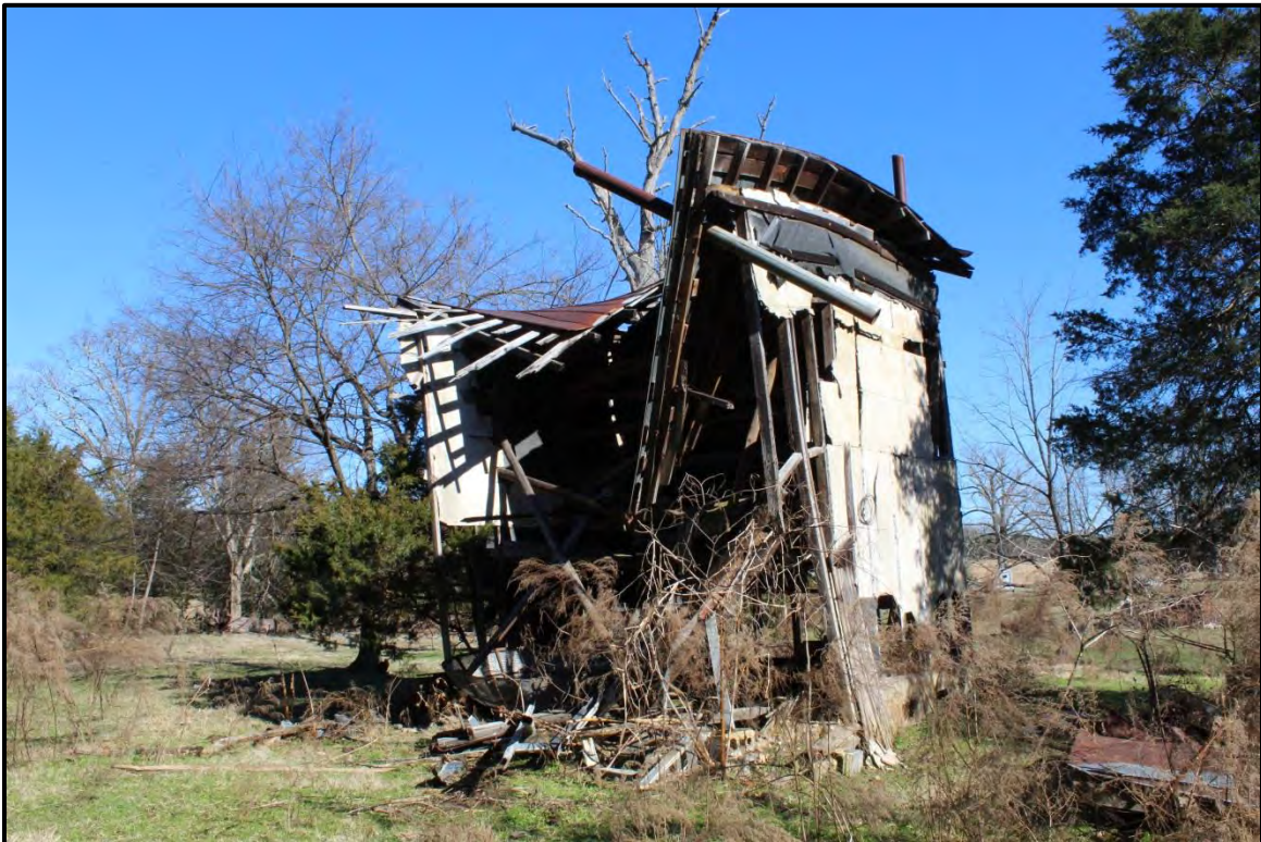
Figure 4.117. Architectural resource AM2635; view is southeast featuring the partially-collapsed tobacco barn.
