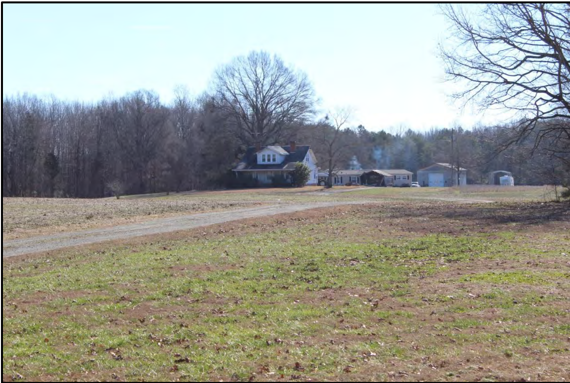
Figure 4.17. Architectural resource AM2622; view is southeast featuring the façade.
