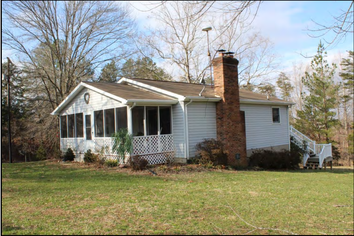
Figure 2.48. Architectural resource RK1794; view is northwest featuring the façade and east elevation.
