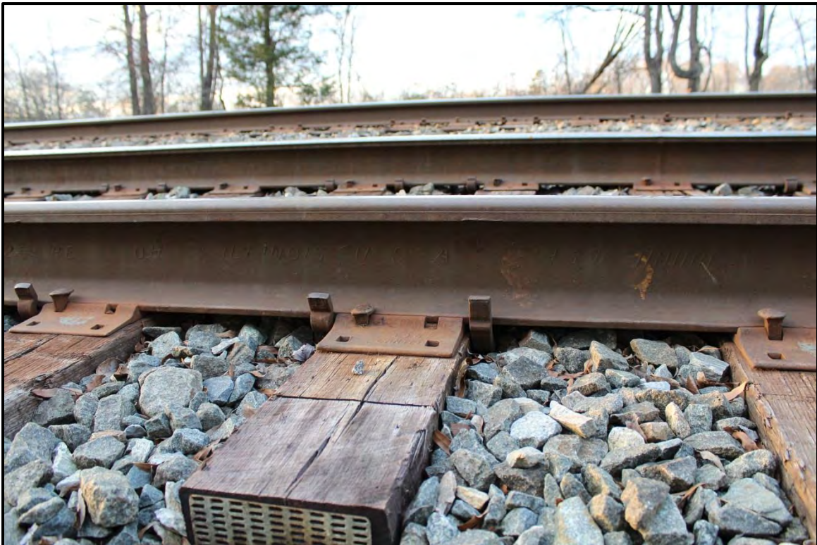
Figure 3.27. Architectural resource GF9116; “south track” featuring the 1939 manufacturing date.
